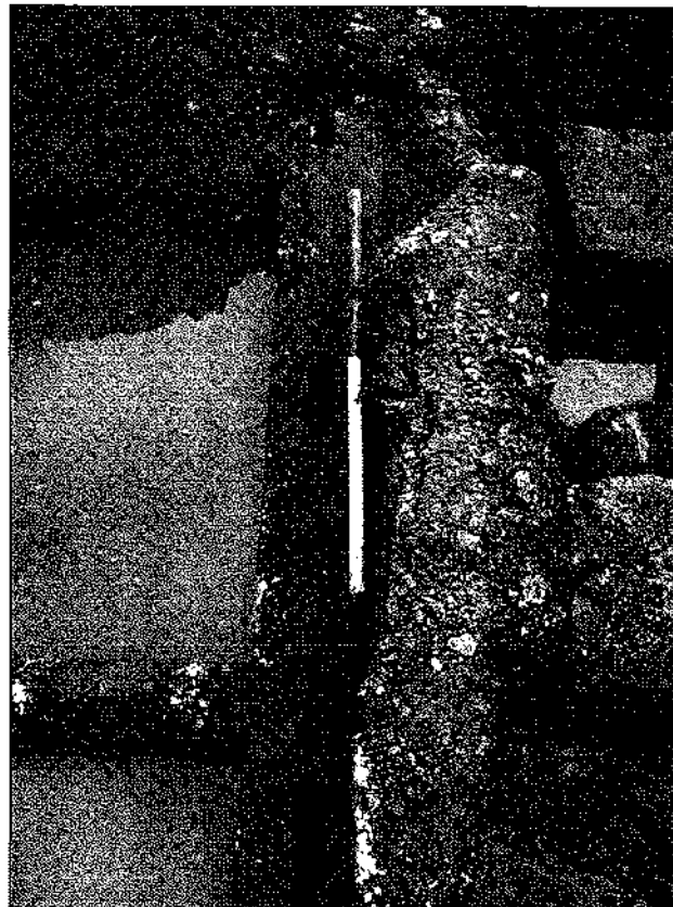
Plate 2: Mortise cut into F113.
