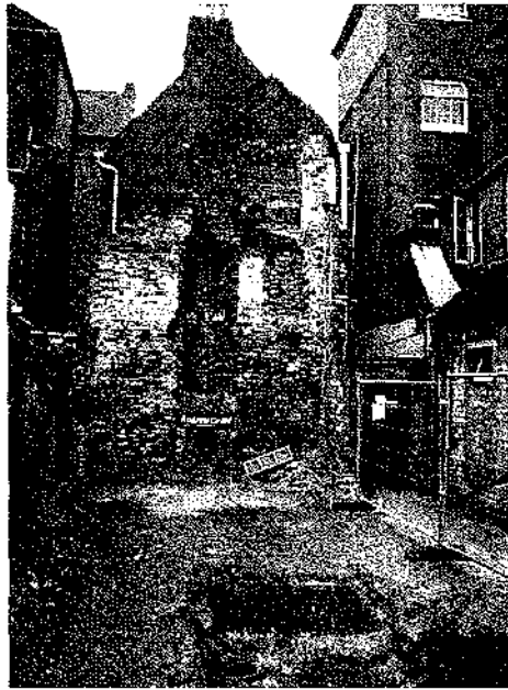
Plate 11: the rear of buildings fronting onto Foregate Street
