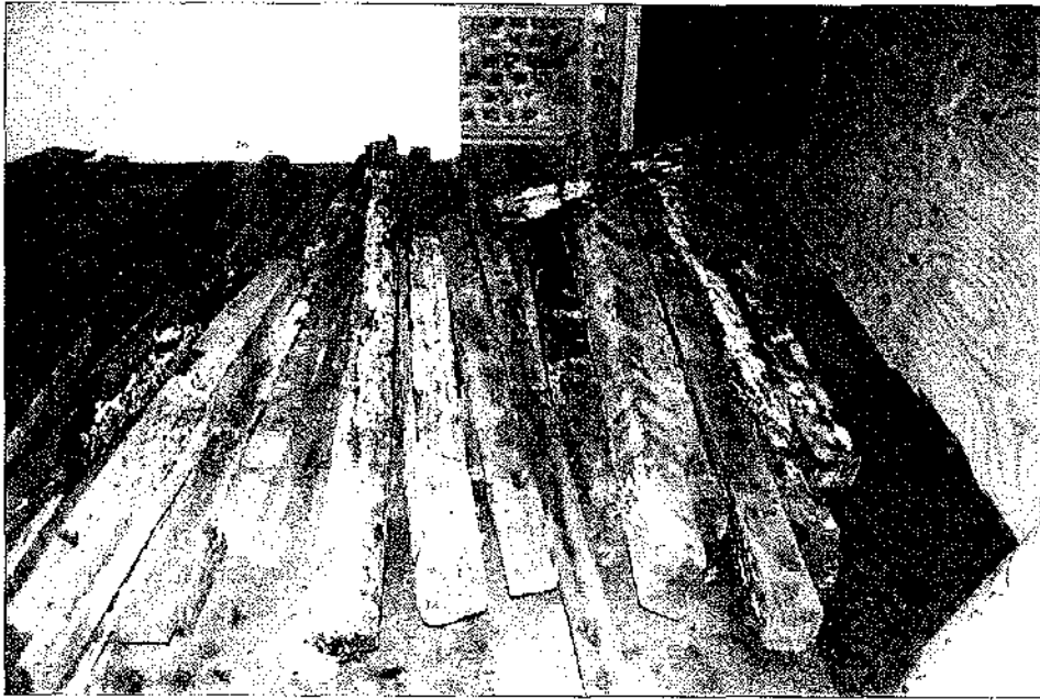
Plate 3. Floor joists from the cross-wing
