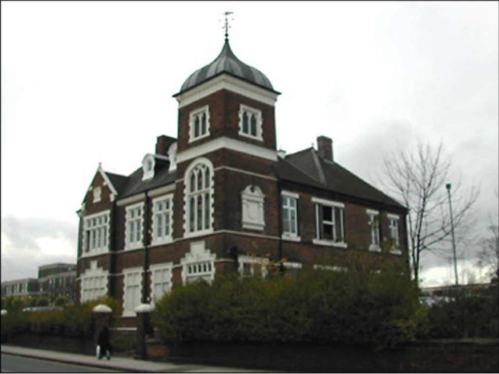
Plate 3: Former Workhouse Board of Guardian's office.
