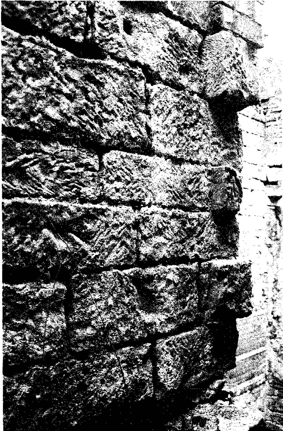
Plate 11. Keying for Former Cross-wall Opposite Wall Stub
