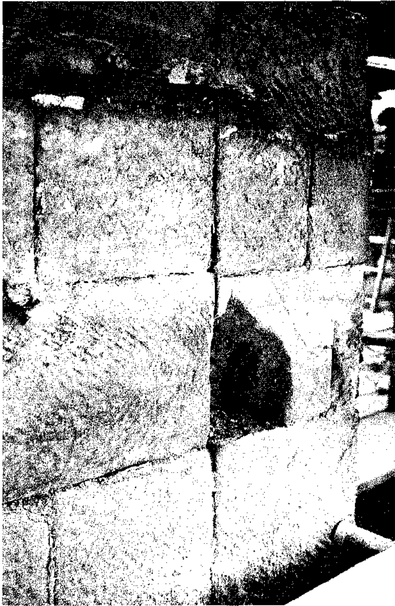
Plate 9. East Elevation, Vertical Joint in the Masonry Behind 19th-century Facing
