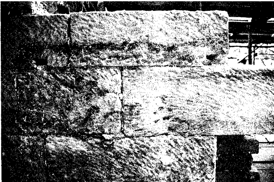
Plate 8. East Elevation , Masonry Behind the 19th-century Facing
