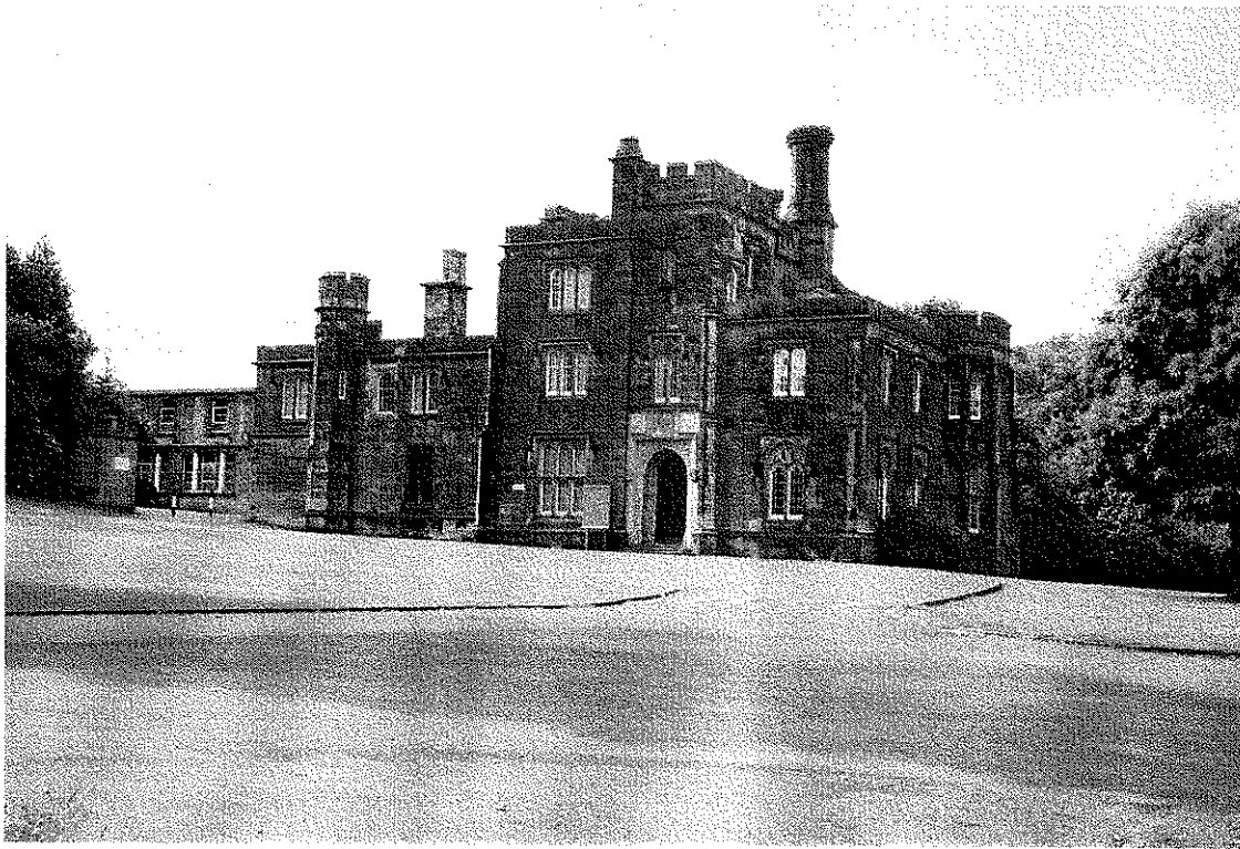
Plate 4 Priory Hall from the southeast
