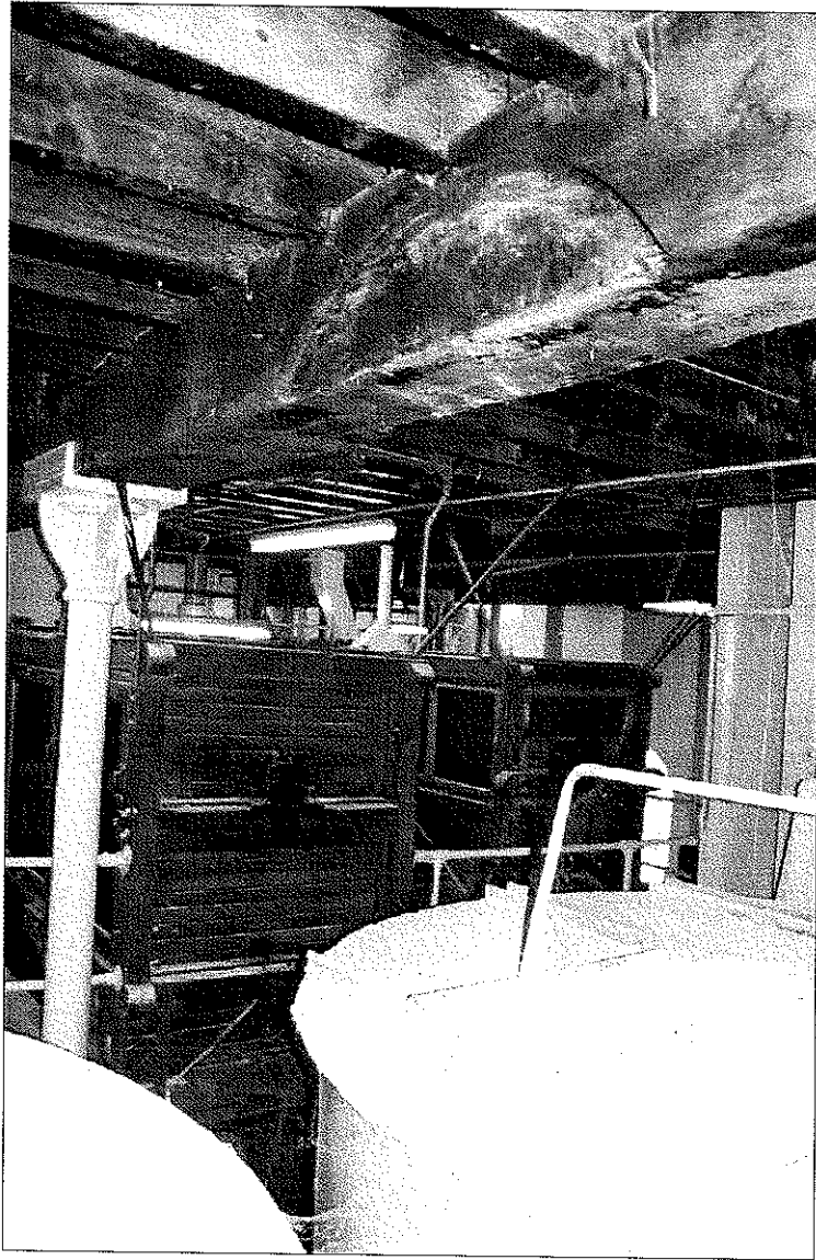
Plate 3 Mill room, arched recess in beam
