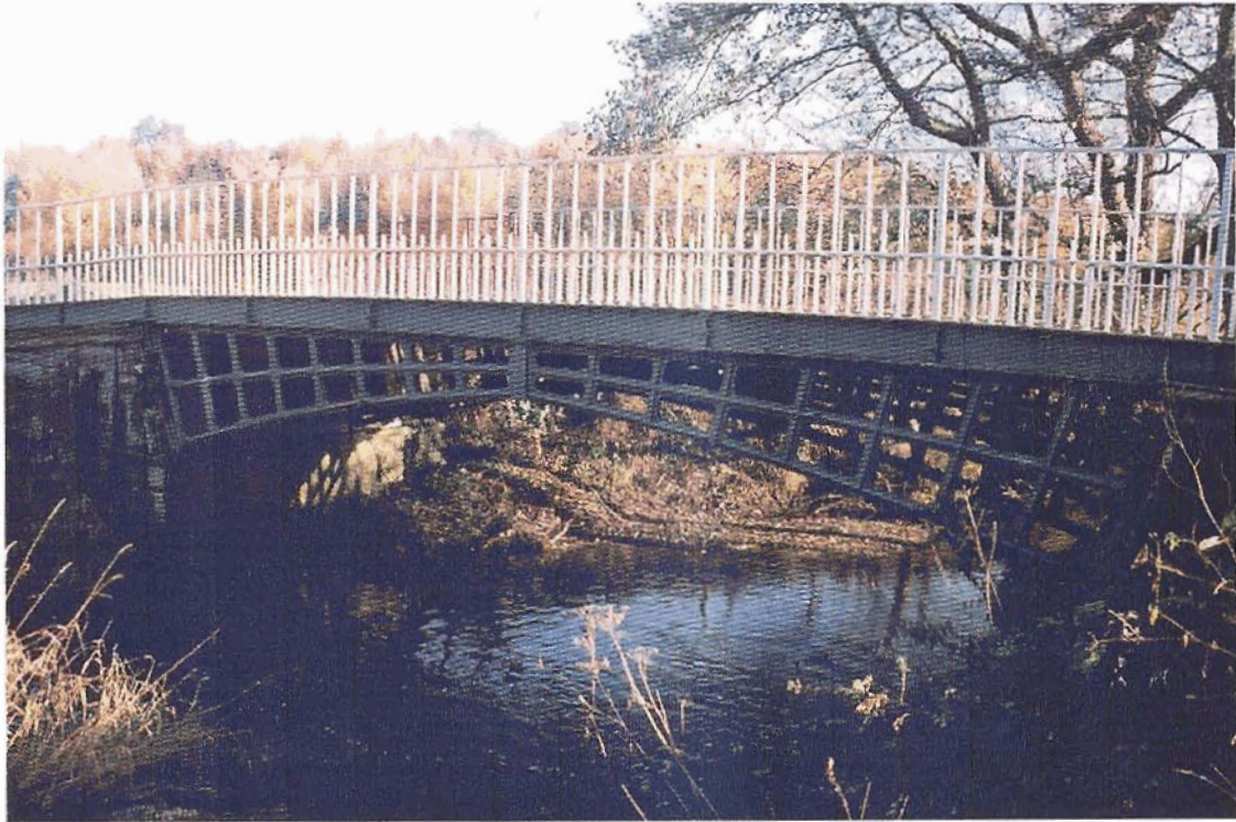
Plate 1 Cantlop Bridge from the west
