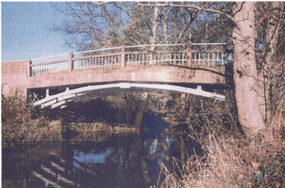
Plate 4 Boreton Bridge from the south
