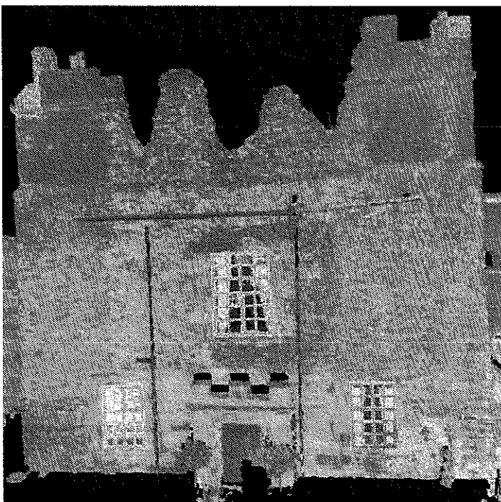
Fig. 9 Scan of building façade at 100mm resolution
