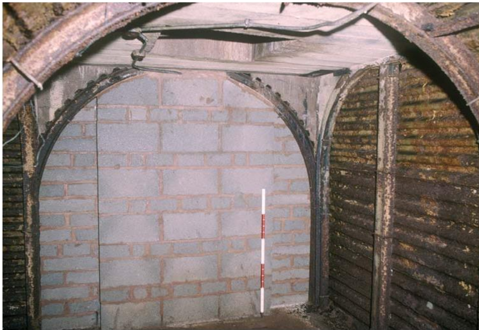
Plate 6 Junction of Two Tunnels Showing Blocking, with Emergency Exit
