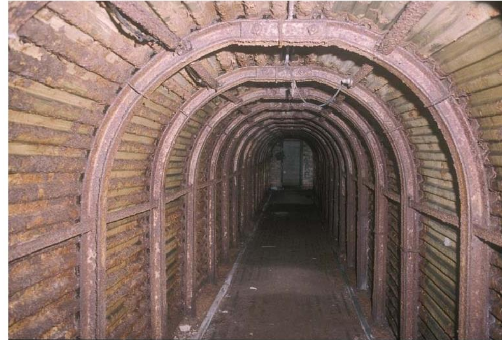
Plate 7 East-west Tunnel Looking back Towards the Entrance
