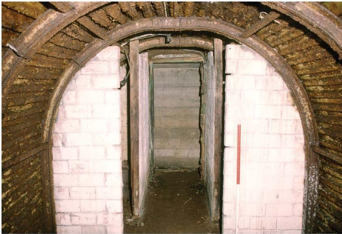
Plate 11 Blast Wall and Secondary Doorway
