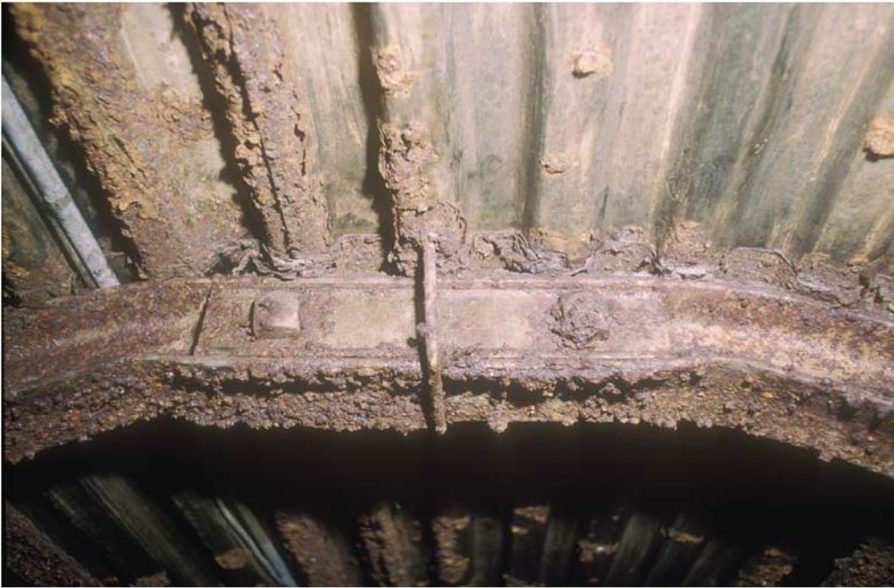
Plate 8 Detail of Fishplate
