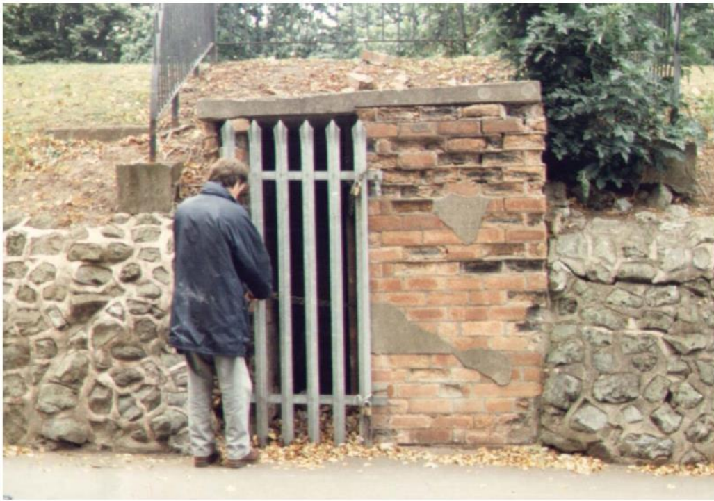
Plate 18 Entrance from Upper Green Road in 1996 (Whitehouse)
