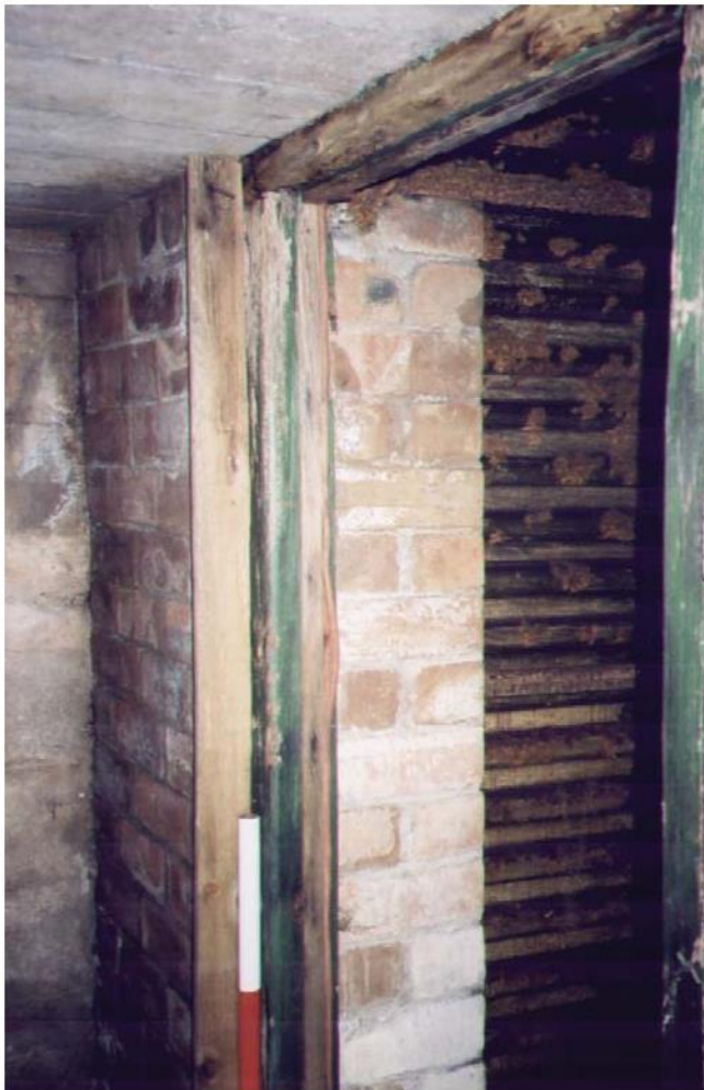
Plate 12 Detail of Door Frame with Rubber Tubing
