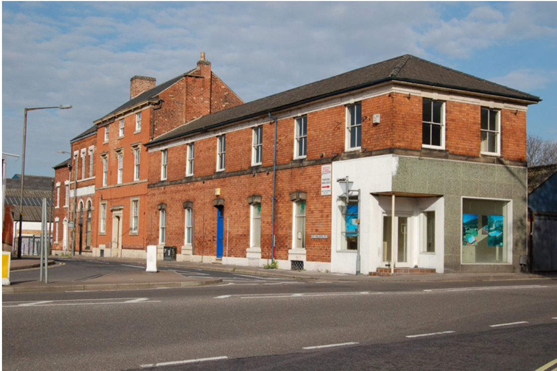
Plate 1: 2-8 St. Helen's Street, oblique view from the east.
