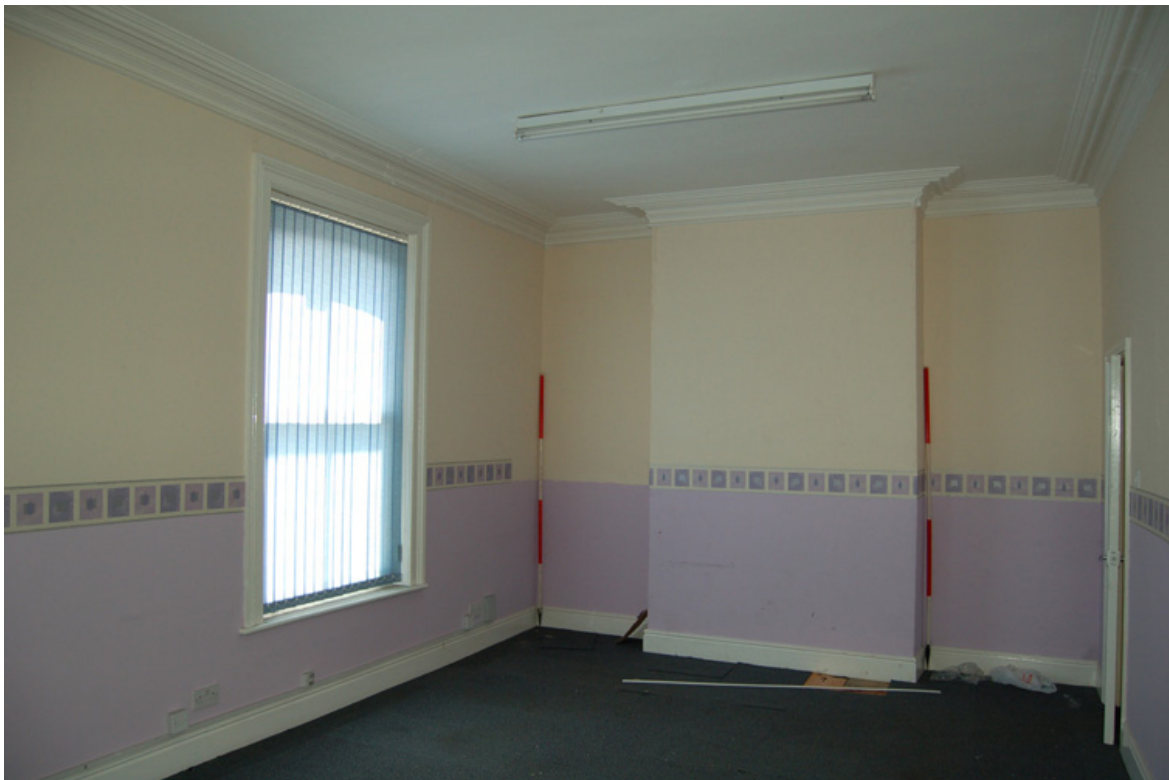
Plate 10: Room G1, looking west: projecting stack and moulded cornice.
