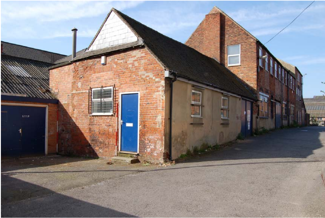
Plate 15: Unit 1, 71 King Street, oblique view from the east.
