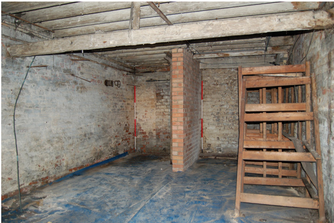
Plate 7: Basement Room B4, looking east, with inserted axial partition.
