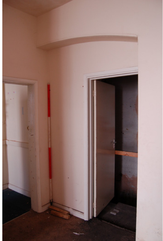
Plate 9: Segmental arch visible within Room G2.
