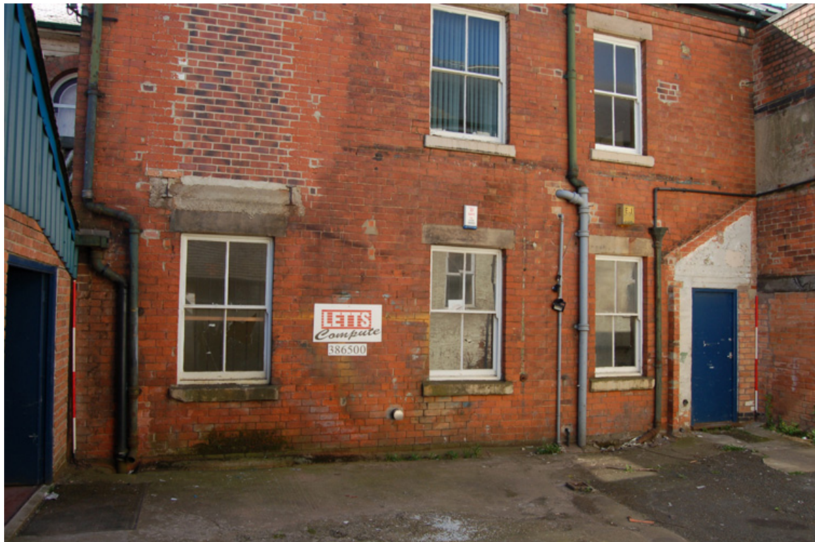
Plate 5: North (rear) extension to Nos. 2-8 St. Helen's Street.
