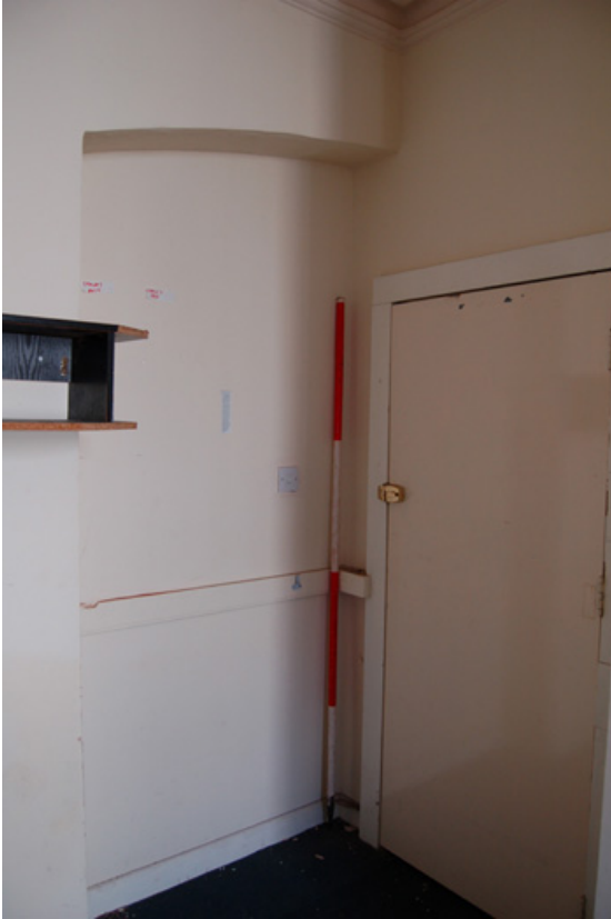
Plate 8: Segmental arch visible within Room G3.
