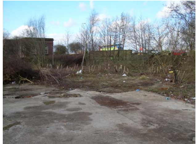
Plate 3 – Floor and foundations building 4
