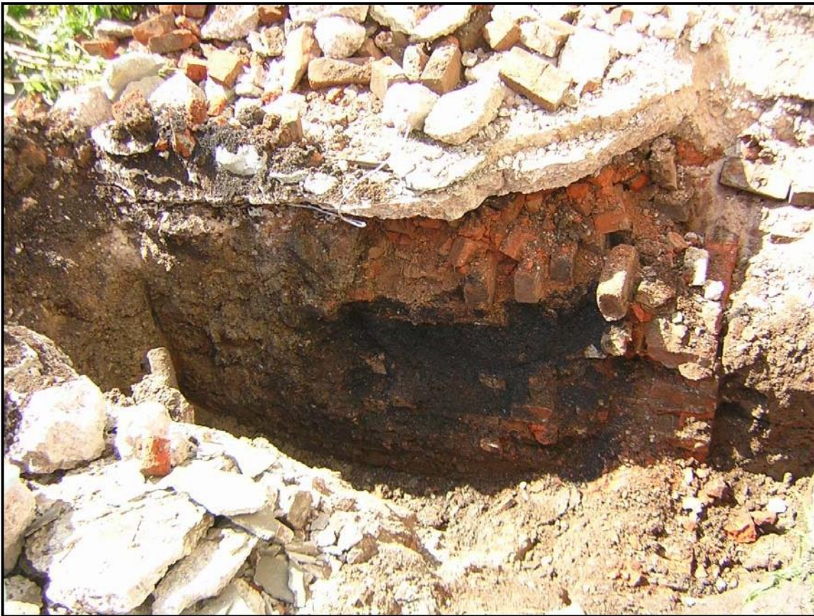
Plate 1 - Pit 4 showing wall foundation 1007
