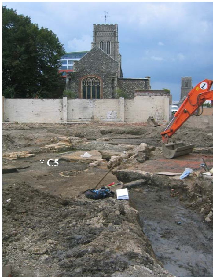
Figure 4: Looking west across the site, with Trench 2 visible to the right. The position of Core 5, located proximal to the building foundations, is highlighted.
