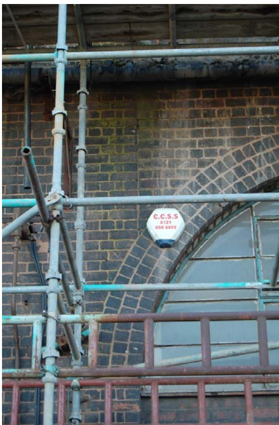
Plate 56: Bldg K; W elev., Level 1, straight joint.
