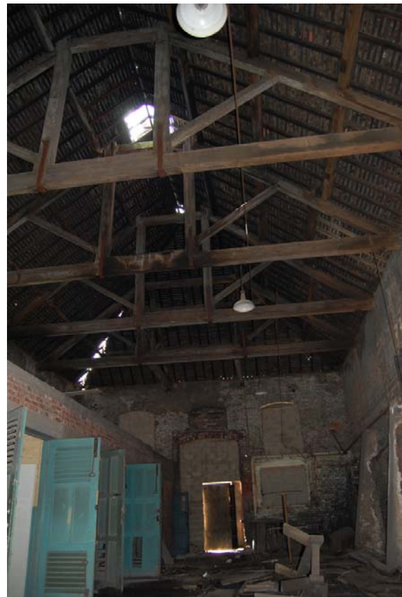
Plate 21: Building B, roof structure.
