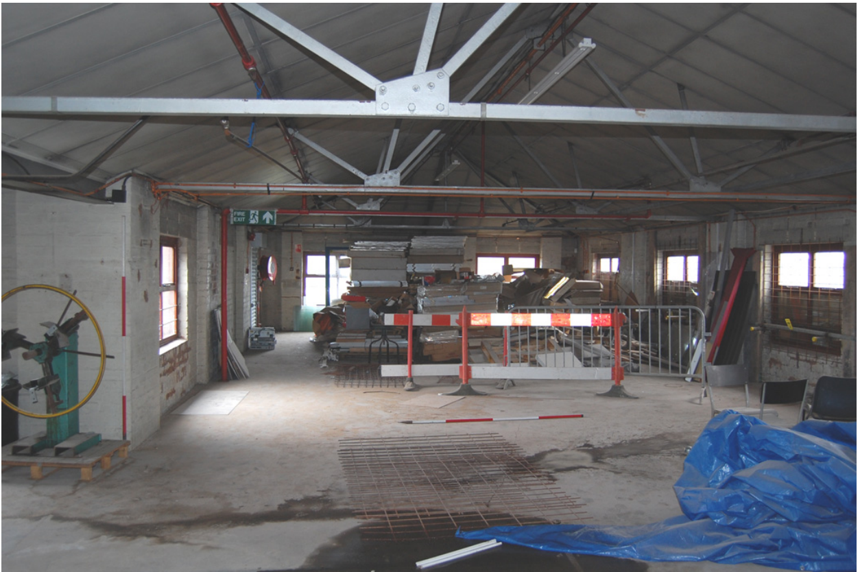
Plate 72: Building K; West Range, Level 7 looking south.
