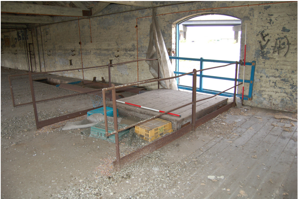
Plate 52: Building E; Level 3 hoist at Bay 3.
