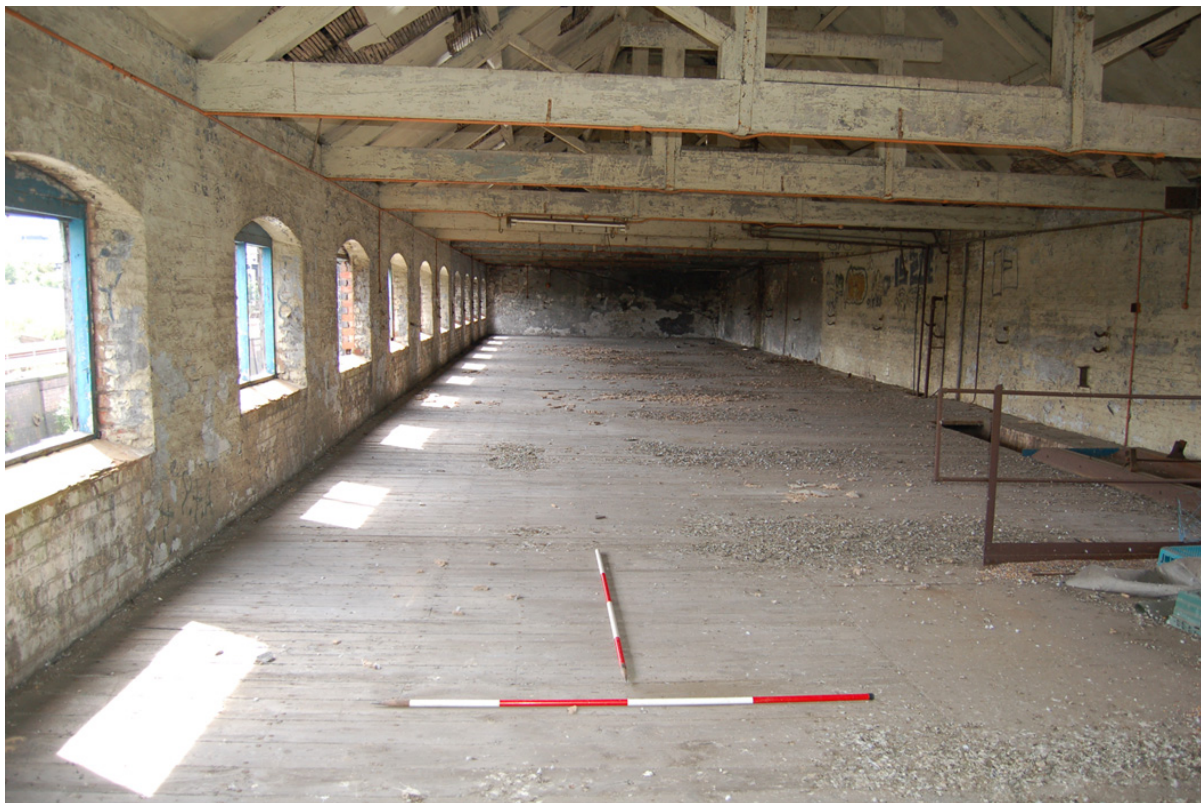
Plate 51: Building E; Level 3 looking west.
