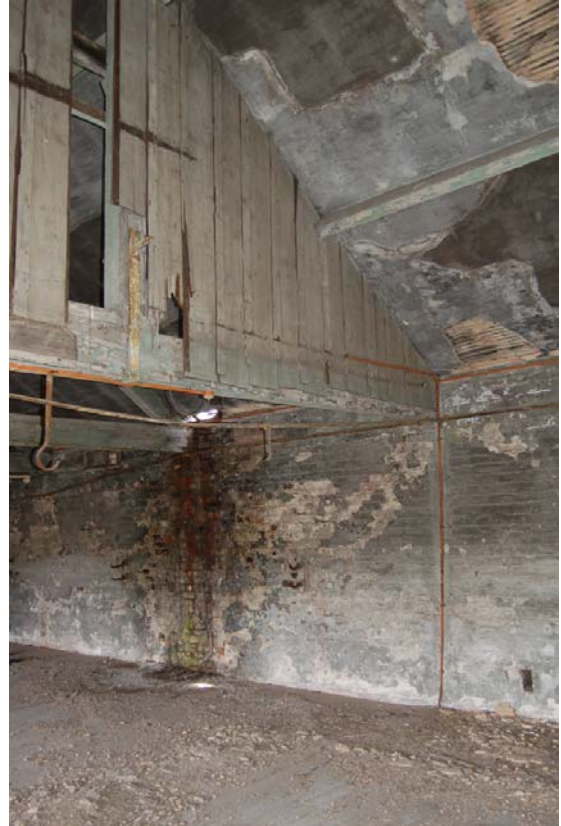
Plate 54: Building E, Level 3 former partitions.
