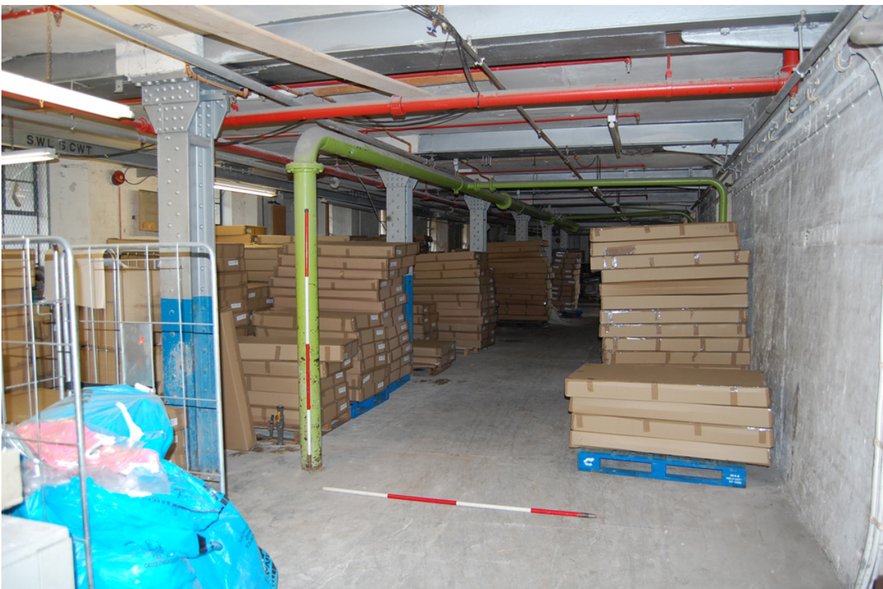
Plate 63: Building K; North Range, Level 2 looking east.
