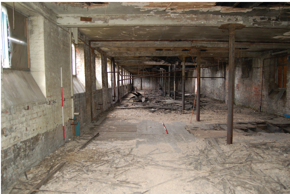
Plate 32: Building D; Level 2 looking west.
