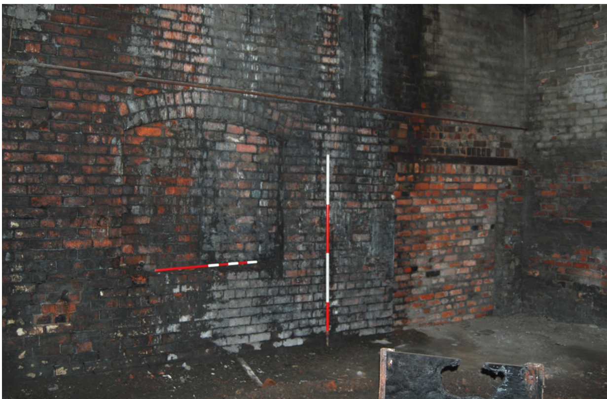
Plate 9: Building A: interior east wall; blocked window (left) and door (right).
