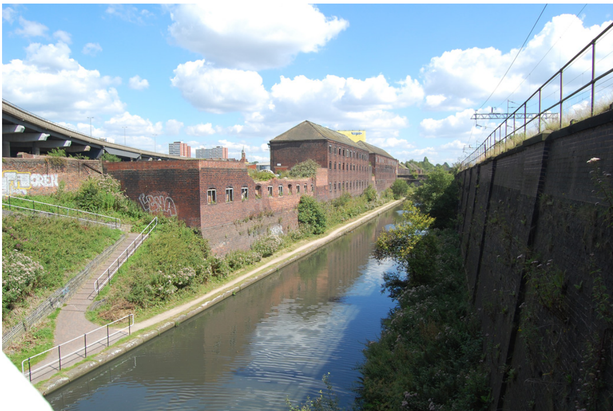
Plate 3: General view of site from west, looking along NML canal (Buildings F, E and D).
