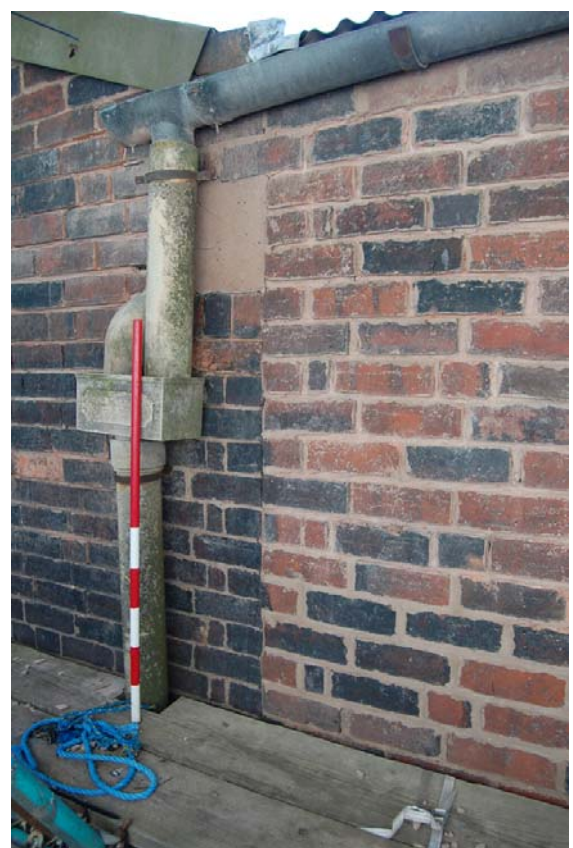
Plate 57: Bldg K, W elev., Level 7, straight joint.
