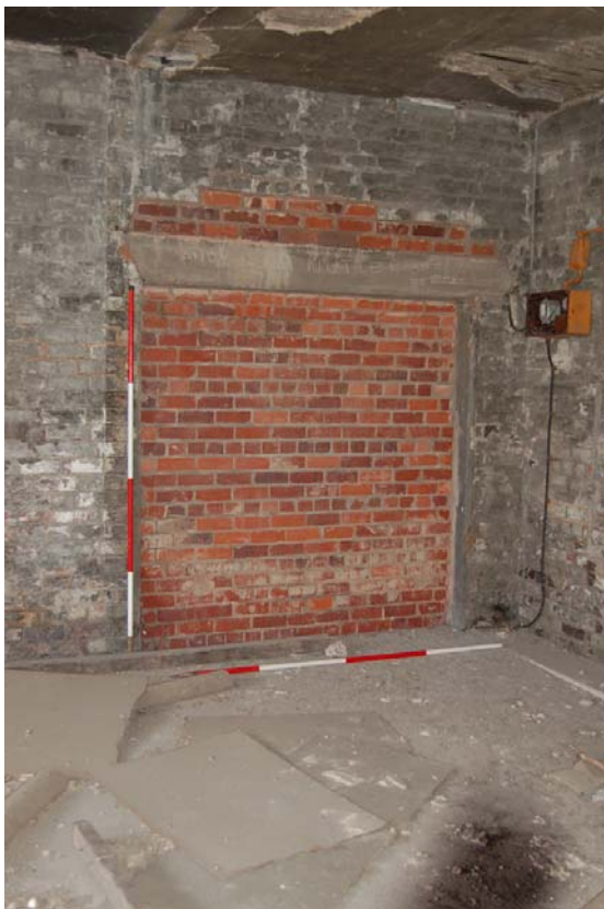
Plate 49: Bldg E; Level 2, blocked door in west wall.
