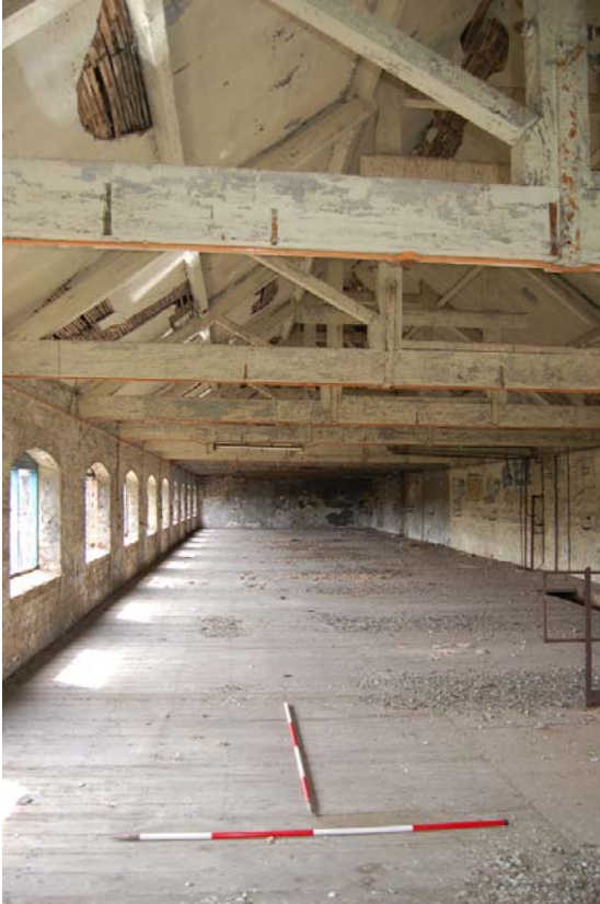
Plate 53: Building E, Level 3, roof structure.
