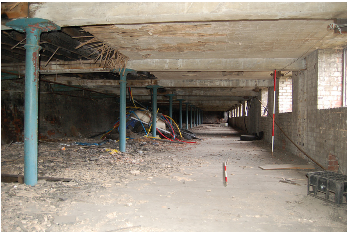
Plate 25: Building D; Level 1, looking east.
