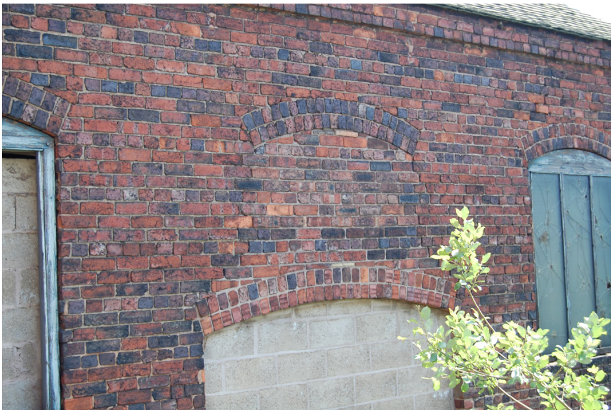
Plate 16: Building B, detail of west elevation; blocked window.
