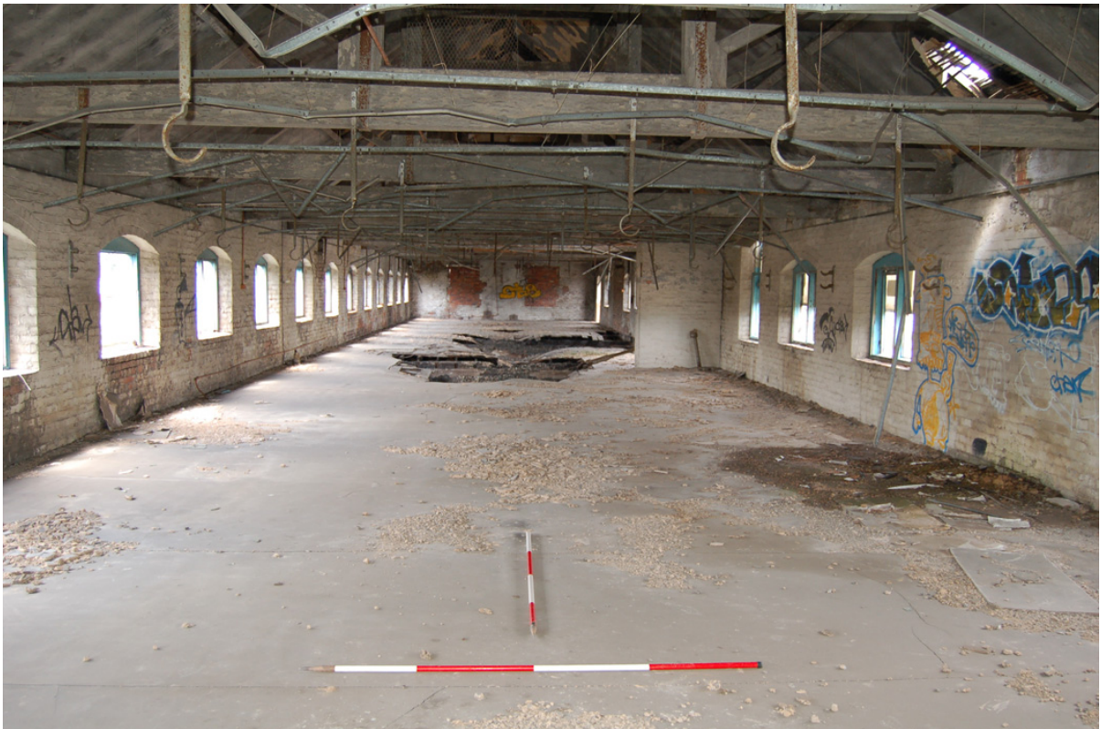
Plate 39: Building D; Level 3 looking west. Note hooked hangers below tie.
