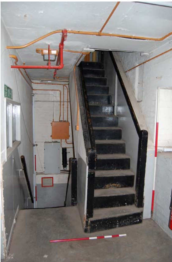
Plate 69: Building K; North Range, stair.
