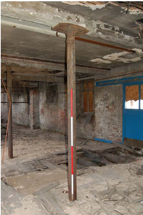
Plate 34 Bldg D; Level 2 central support column.
