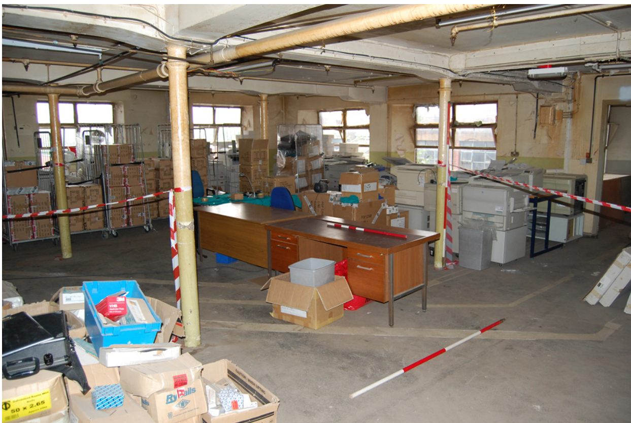
Plate 64: Building K; West Range, Level 4, looking south-east.
