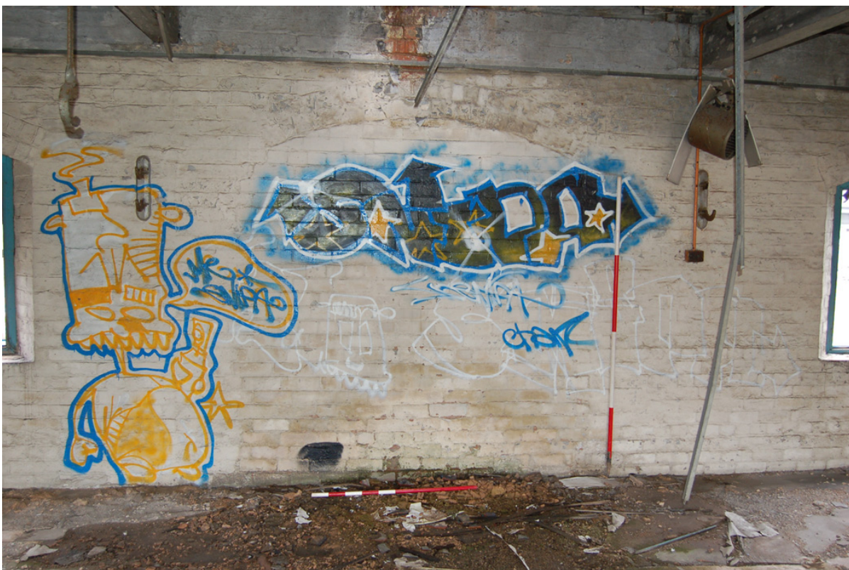
Plate 37: Building D; Level 3, blocked door in Bay 4 (north).
