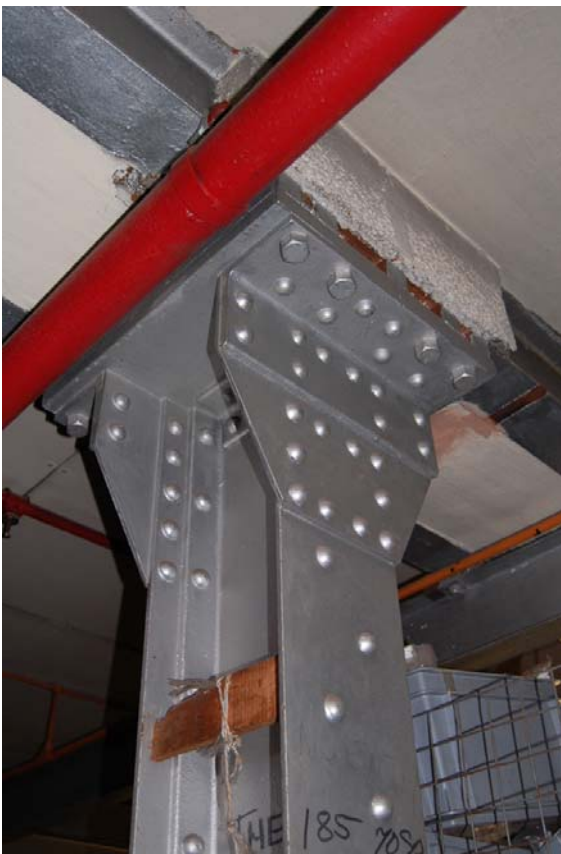
Plate 67: Building K; North Range, Level 1 inserted steel stanchion.
