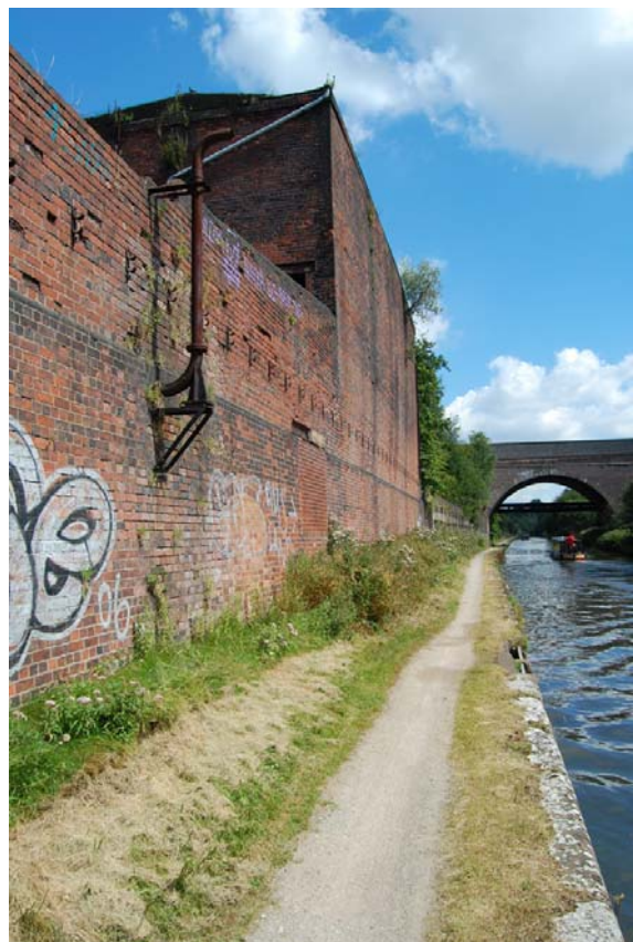
Plate 13: Building A, view from NML towpath.
