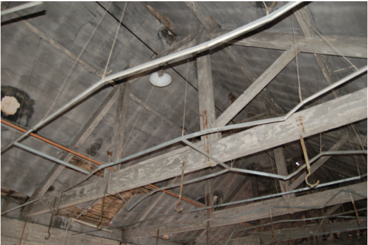
Plate 40: Building D; Level 3, roof structure.
