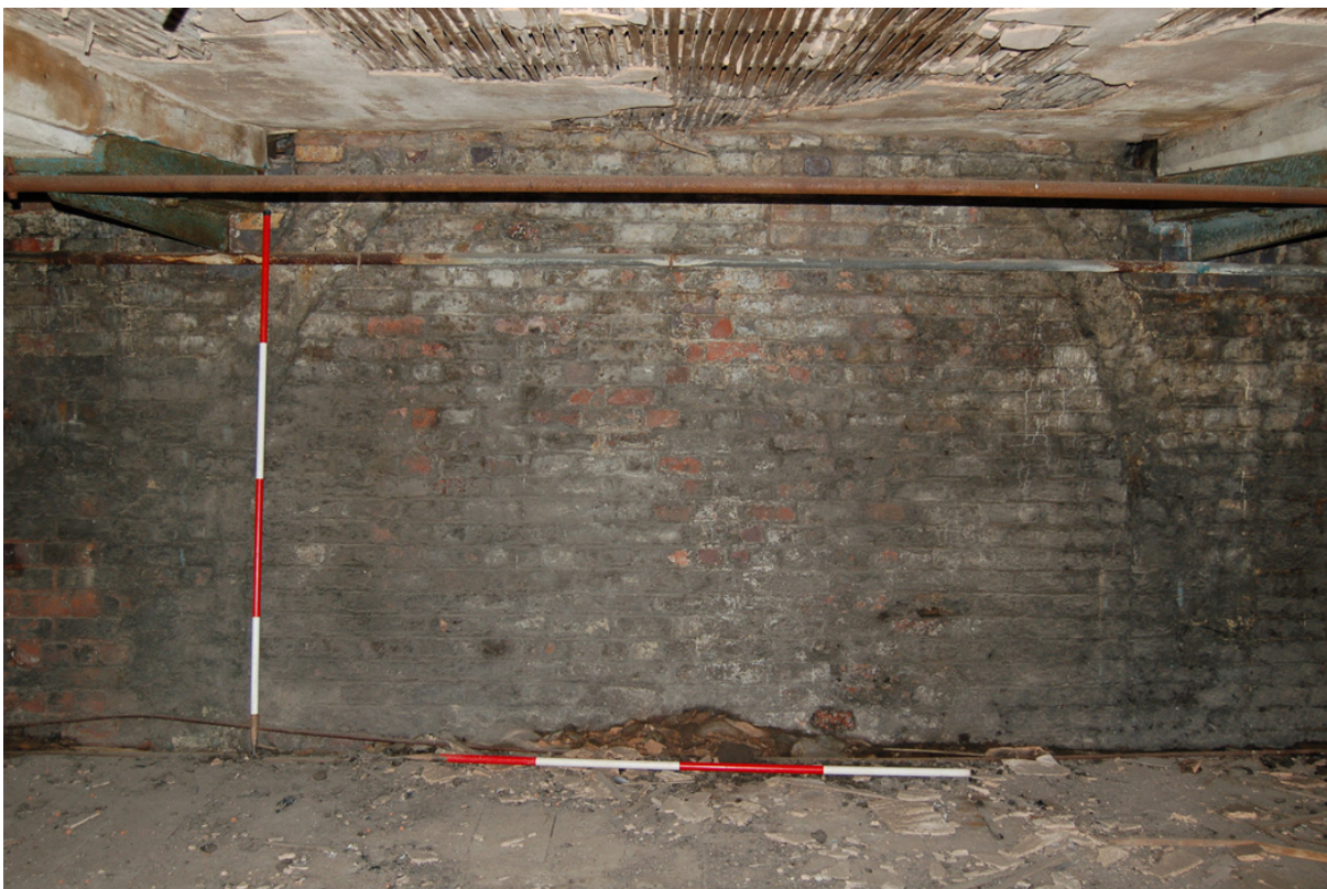
Plate 28: Building D; Level 1, blocked arched tunnel in north wall (Bay 9).
