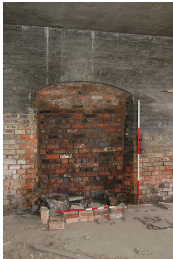
Plate 50: Bldg E; Level 2, blocked door in east wall.
