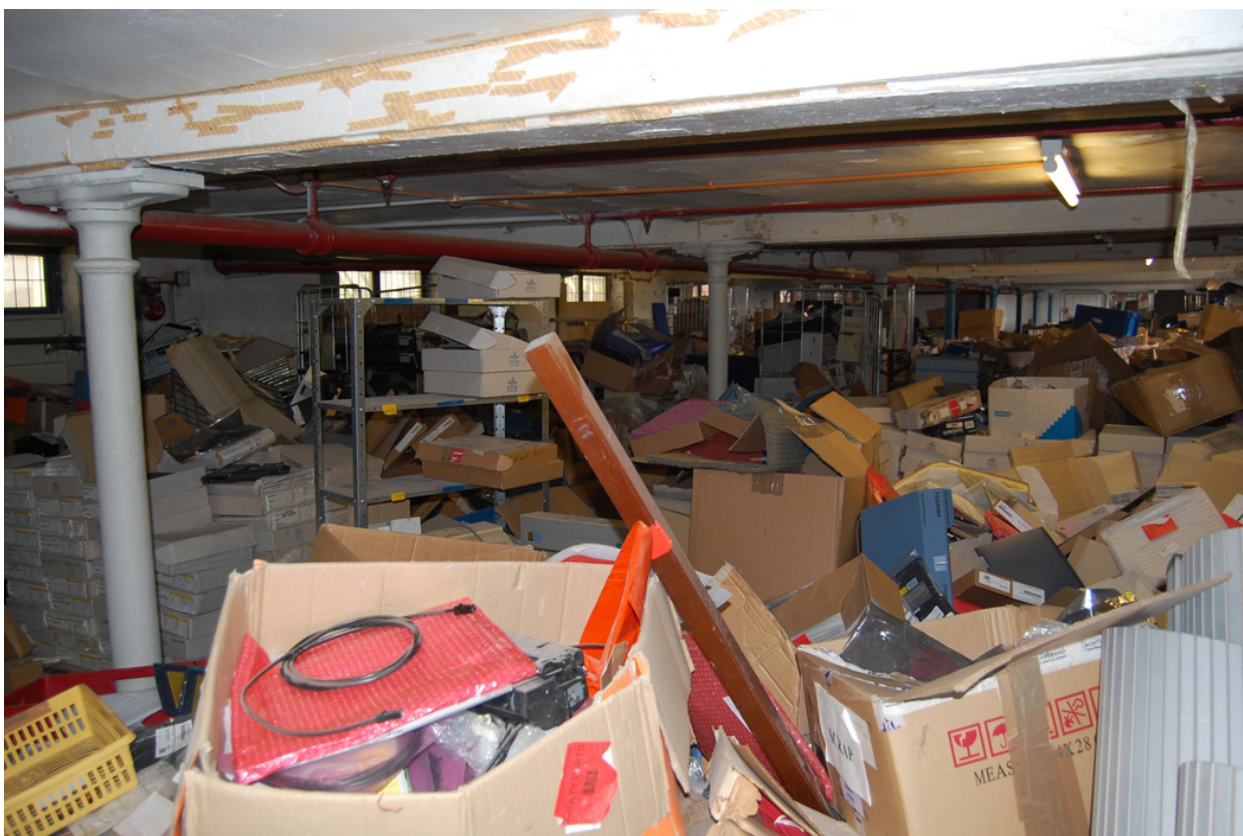
Plate 65: Building K; North Range, Level 6 looking east.
