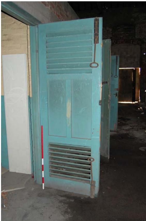
Plate 20: Building B, doors to plant rooms.
