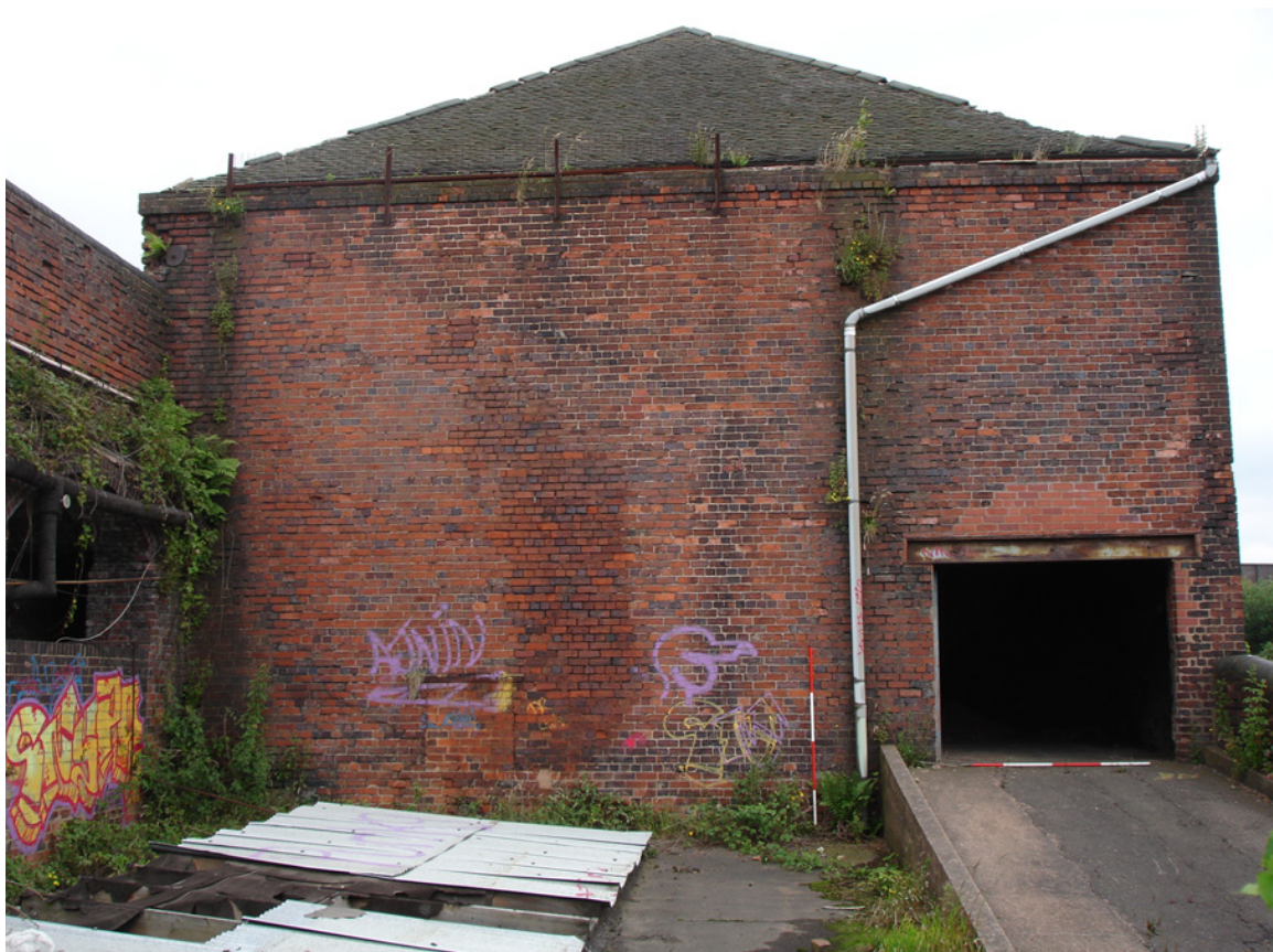
Plate 6: Building A, west elevation. Note shadow of former infill block (see Figure 14c).
