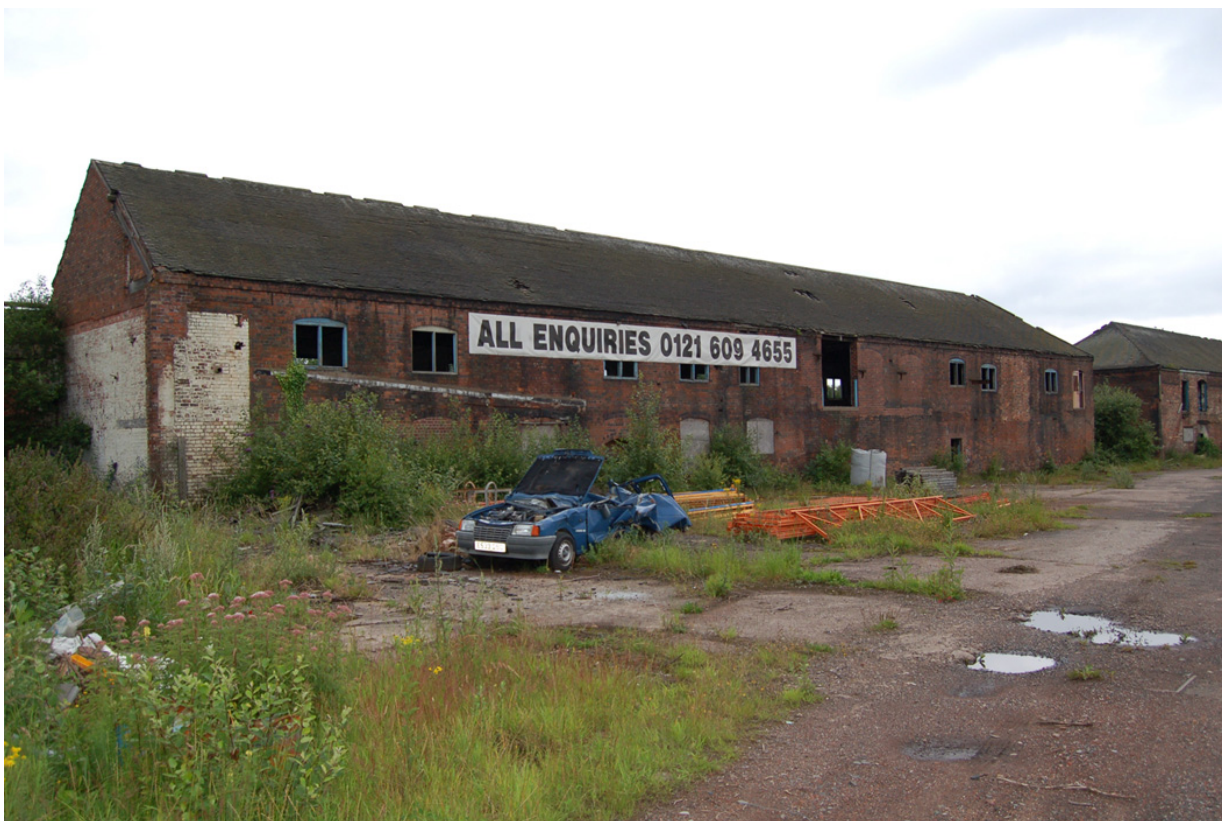
Plate 23: Building D: general view from the north-east.
