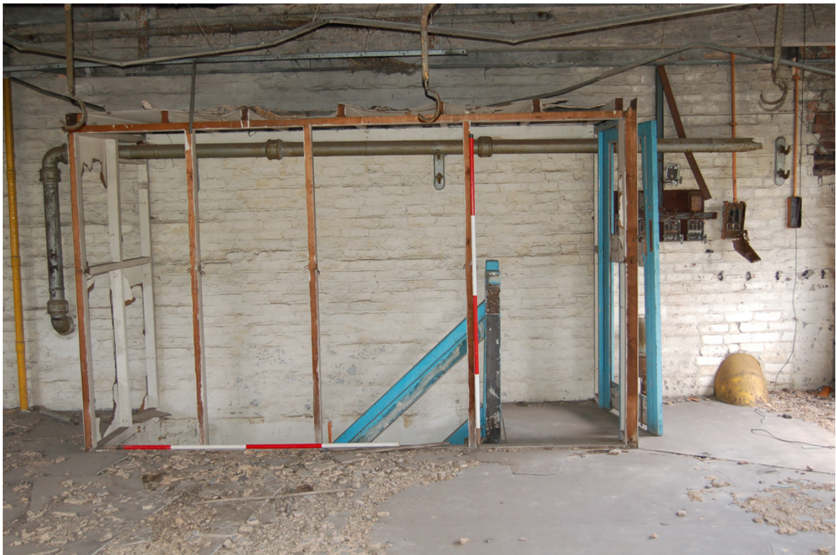
Plate 36: Building D; Level 3 stair rising in Bay 1 (east).
