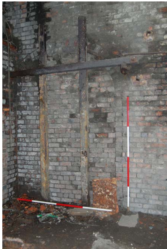
Plate 11: Building A, east wall, blocked archway.
