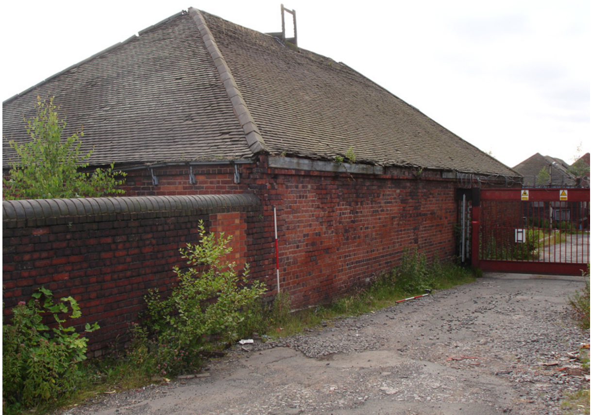
Plate 15: Building B, exterior view from the north-east.
