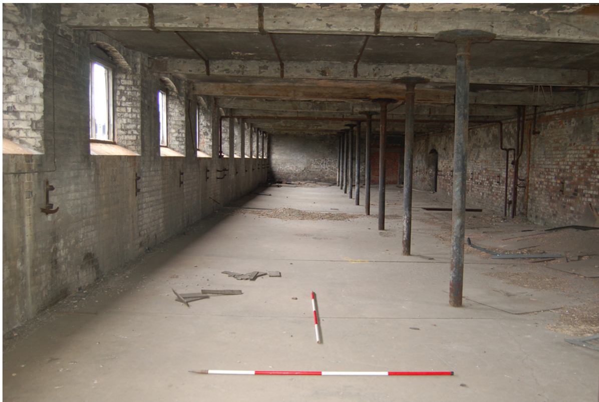
Plate 48: Building E; Level 2 looking west.
