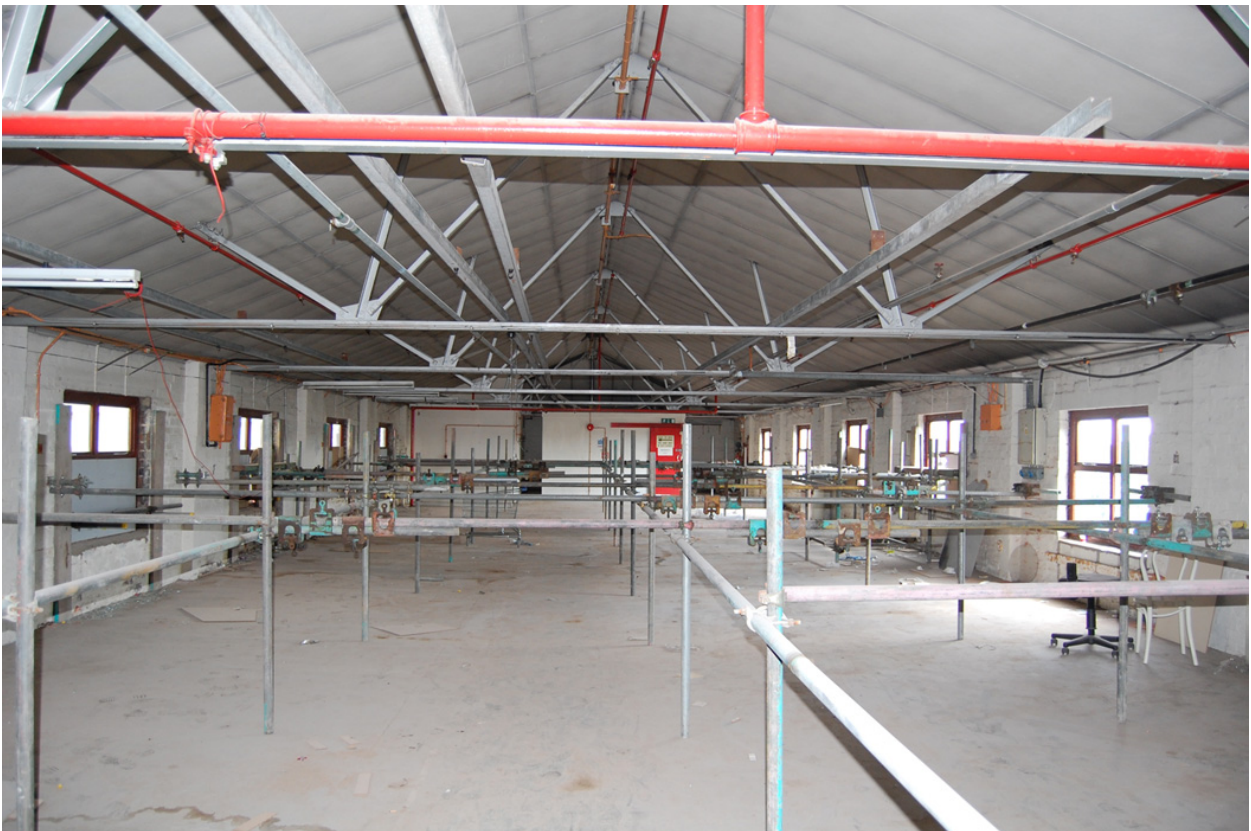
Plate 71: Building K; North Range, Level 7 looking east.
