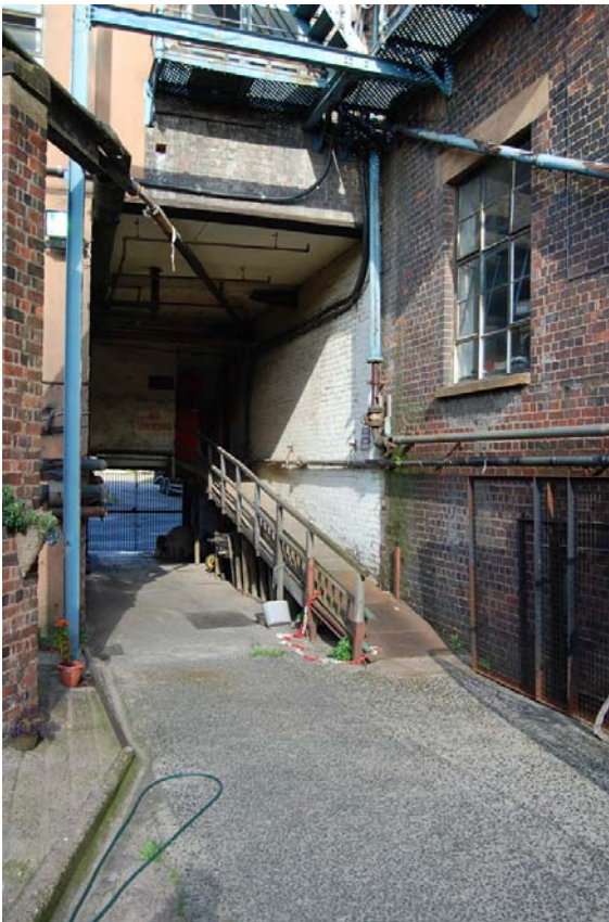
Plate 61: Bldg K, entranceway looking west.
