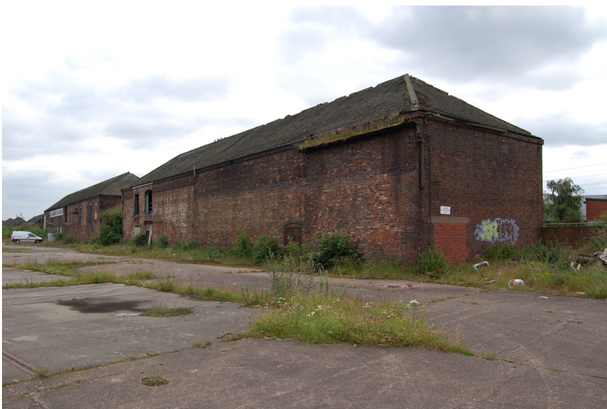
Plate 45 Building E; general view from the north-west.
