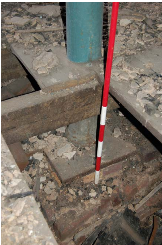
Plate 30: Bldg D; Level 1, detail of post base-plate.
