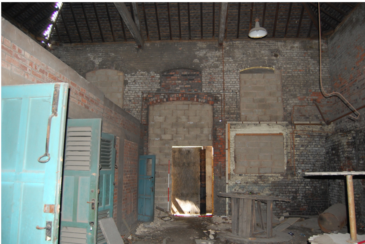
Plate 18: Building B, interior view looking west.
