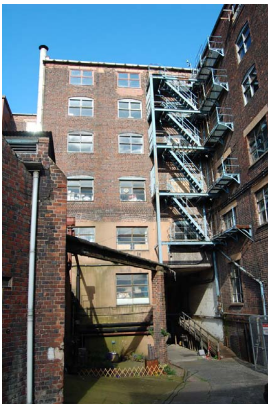
Plate 58: Bldg K, West Range, Yard elevation
