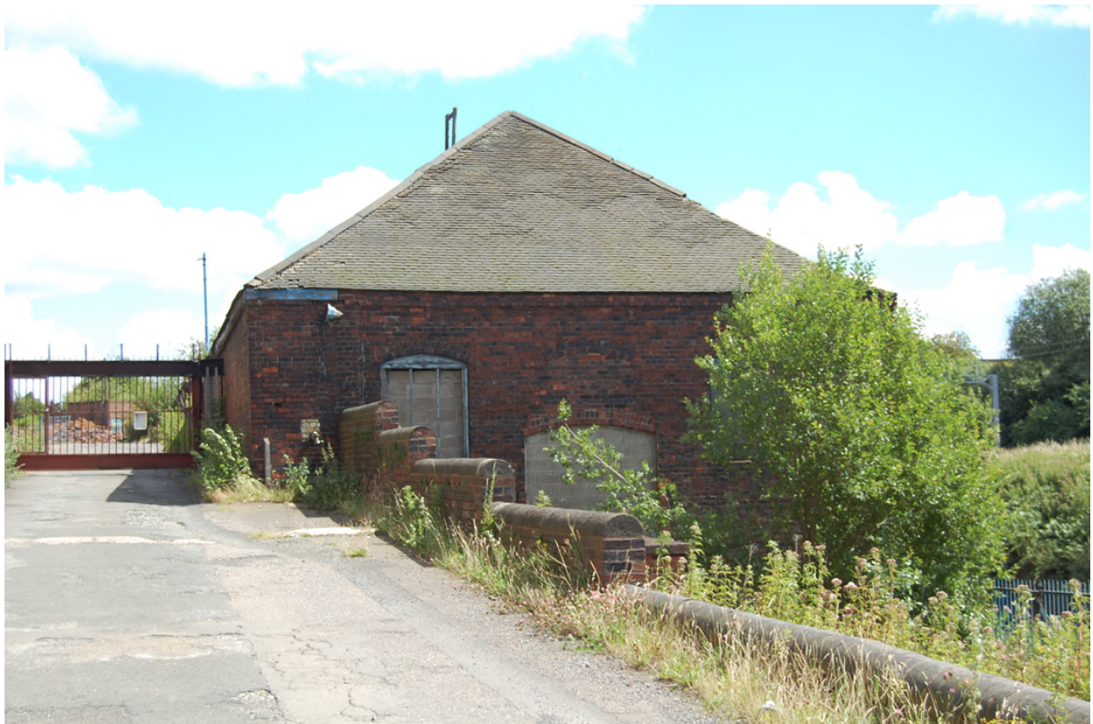
Plate 14: Building B, exterior view from the west.
