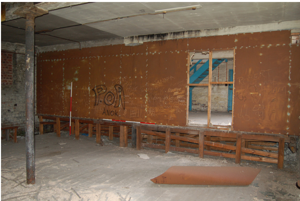
Plate 33: Building D; Level 2, raised floor level at east end (Bays 1 and 2).
