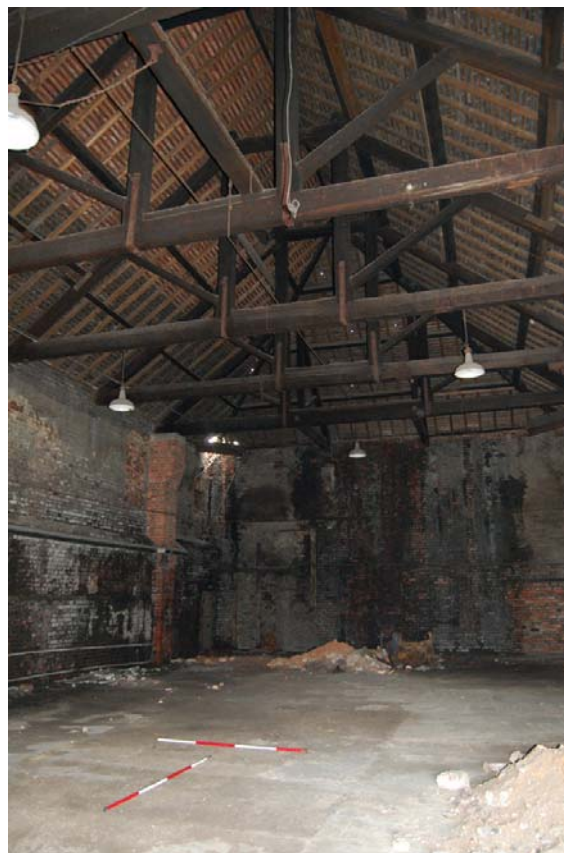
Plate 8: Building A, interior looking east.
