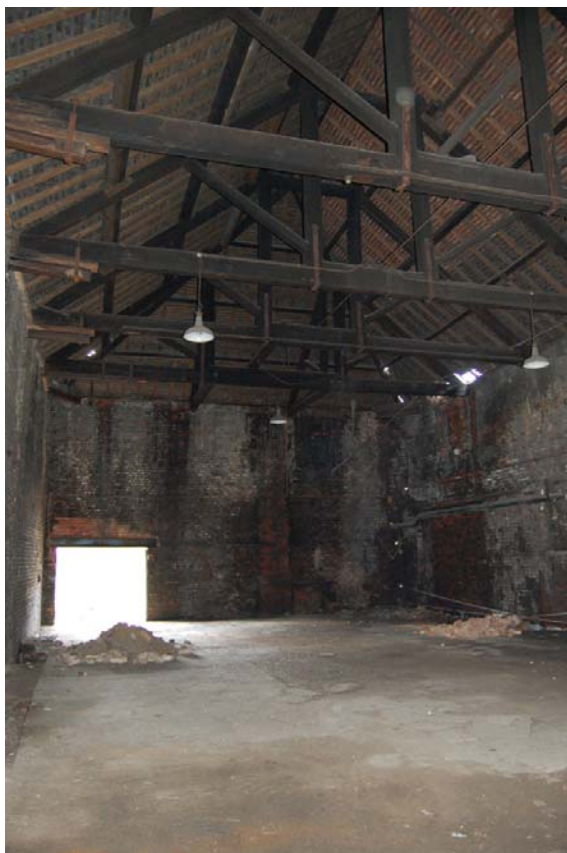
Plate 7: Building A, interior looking west.
