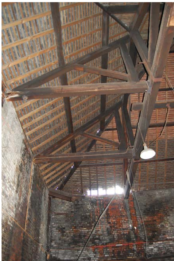
Plate 12: Building A, end 1/2 trusses.
