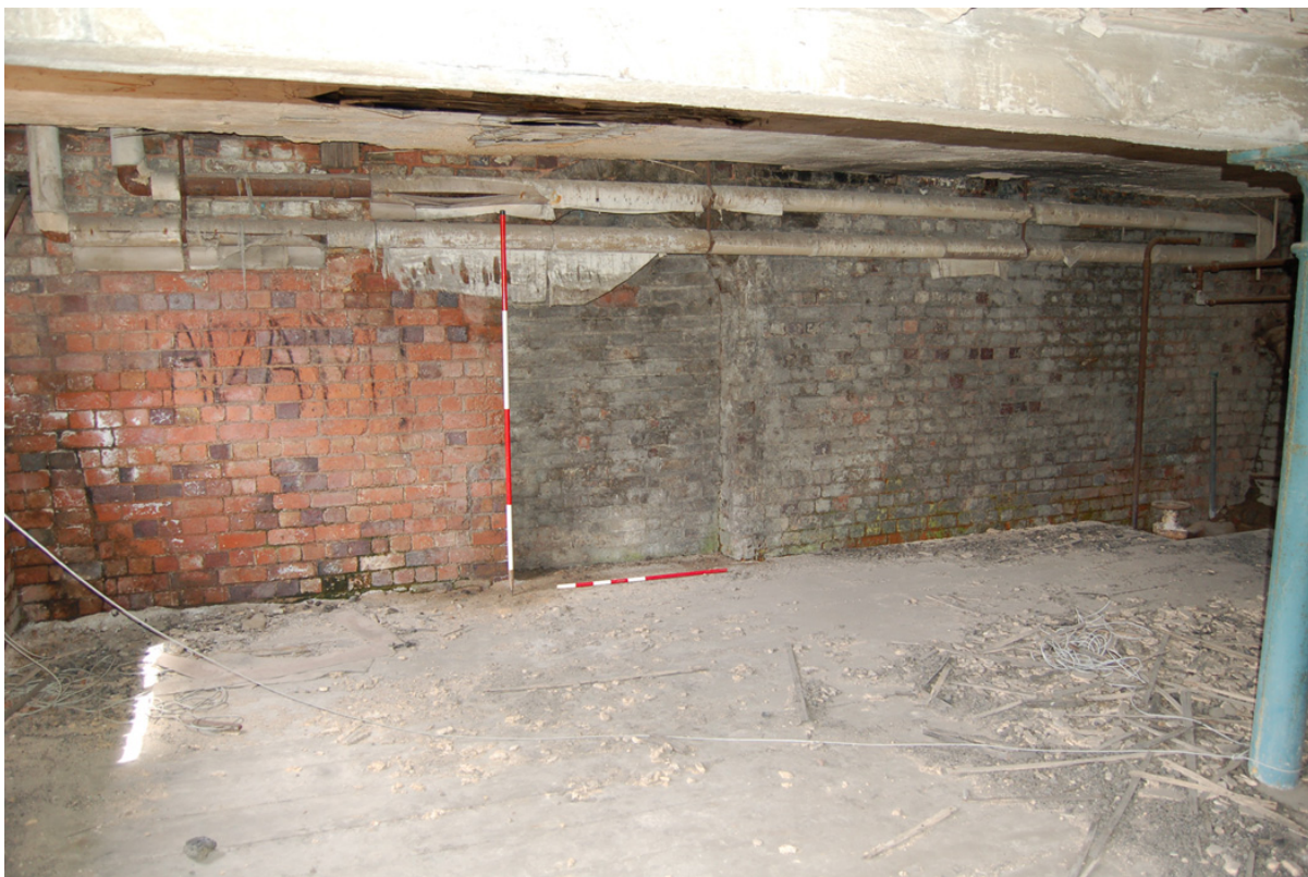
Plate 27: Building D; Level 1, blocked doorway in west wall.
