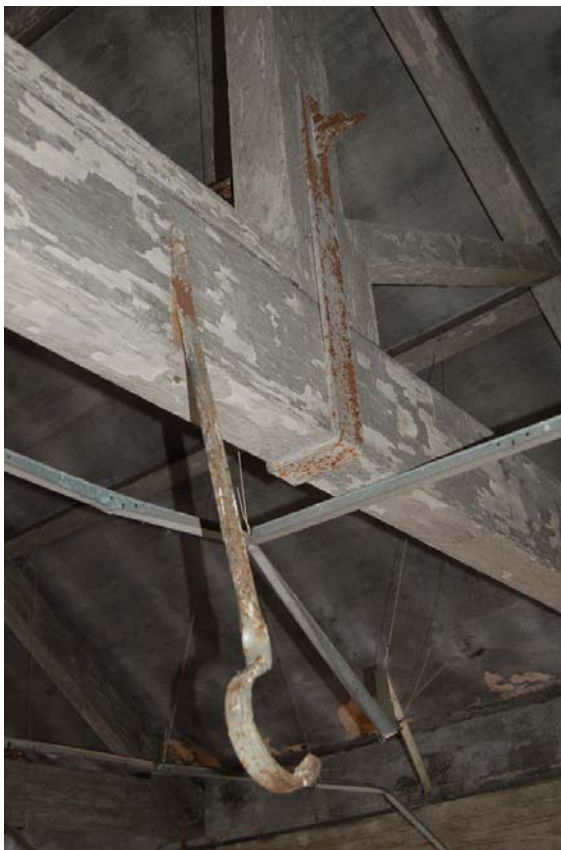
Plate 42: Bldg D; detail of hanger.
