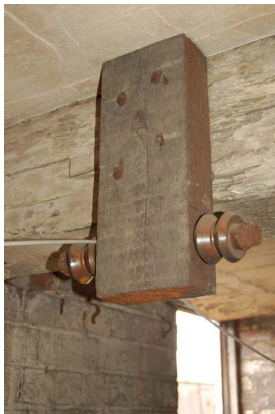
Plate 31: Pulley wheels to south side Building D, Level 1.
