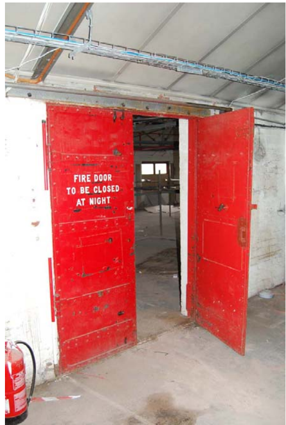
Plate 70: Building K; fire door between north and west range (Level 7).
