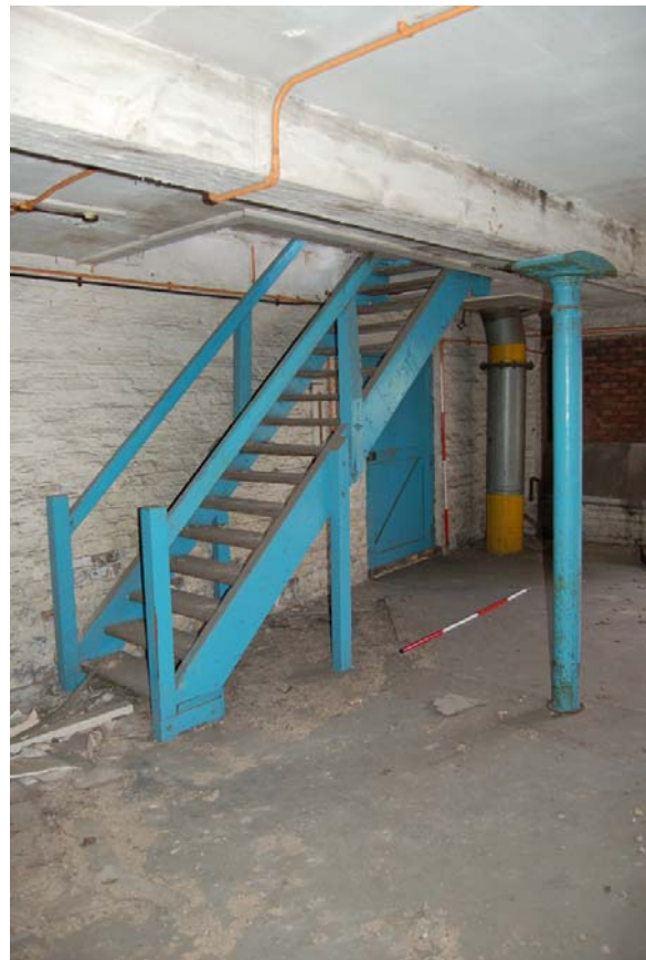
Plate 35: Bldg D, stair from Level 2 to 3.
