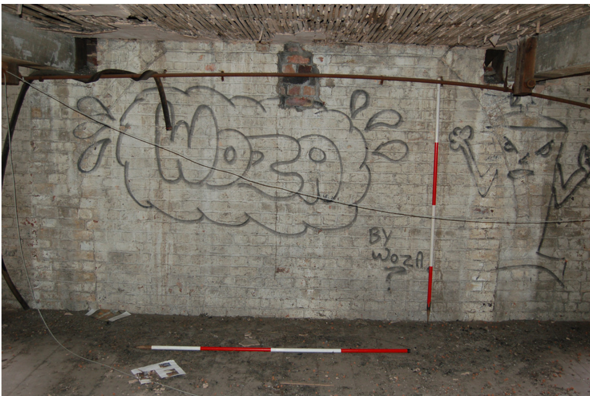
Plate 29: Building D; Level 1, blocked arched opening in south wall (Bay 9).
