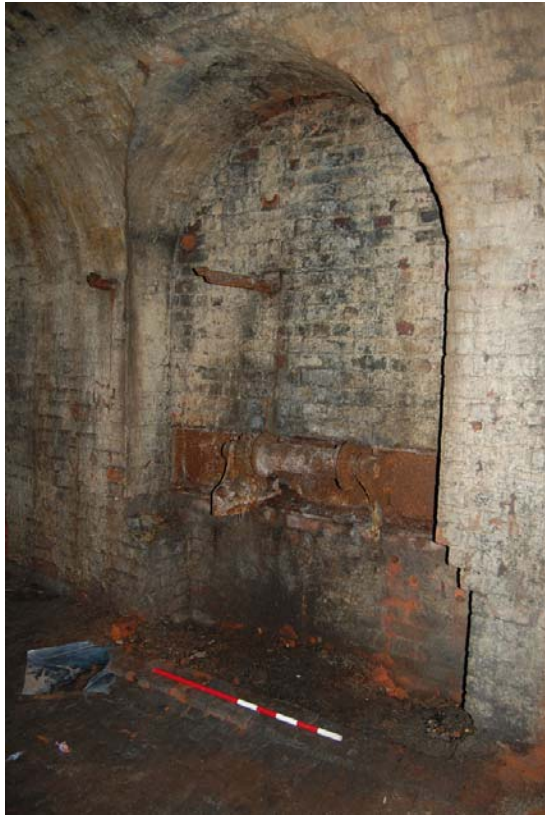
Plate 13: Arched recess with winch gear.
