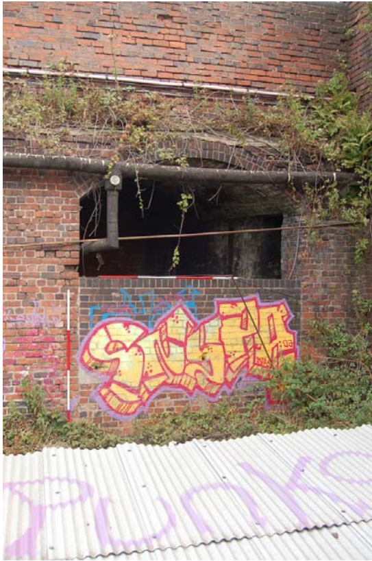
Plate 10: Entrance to central section (E).
