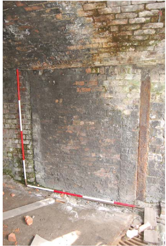
Plate 11: Blocking of east section.
