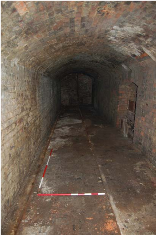
Plate 04: Tunnel, west section looking east.
