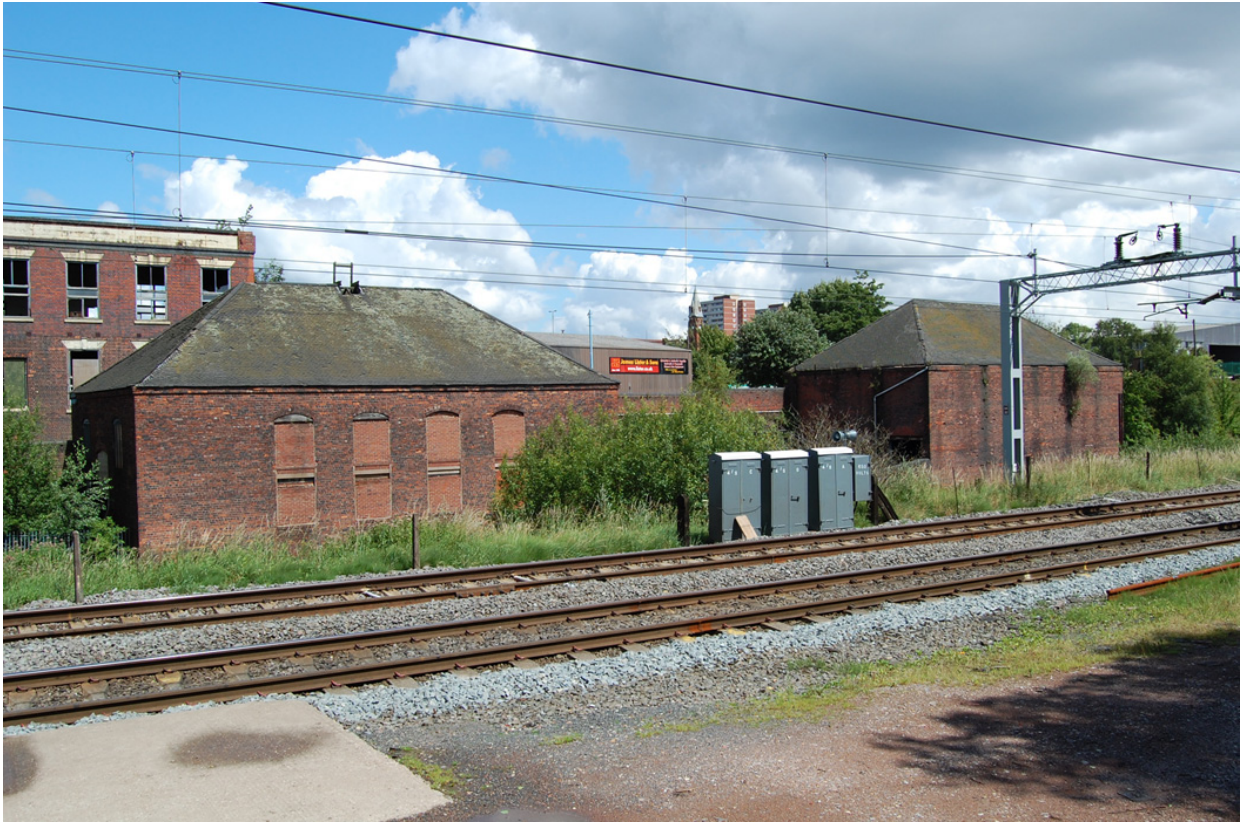
Plate 01: Buildings A and B seen from south side of NML canal.
