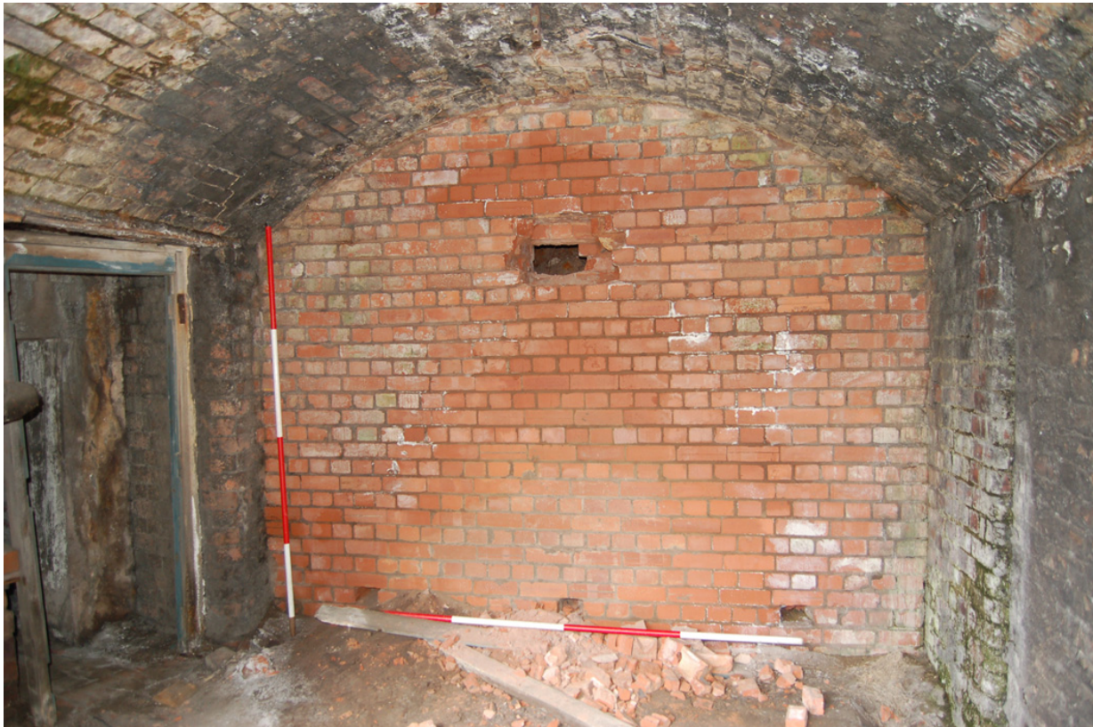
Plate 09: Central section, blocked tunnel leading north.
