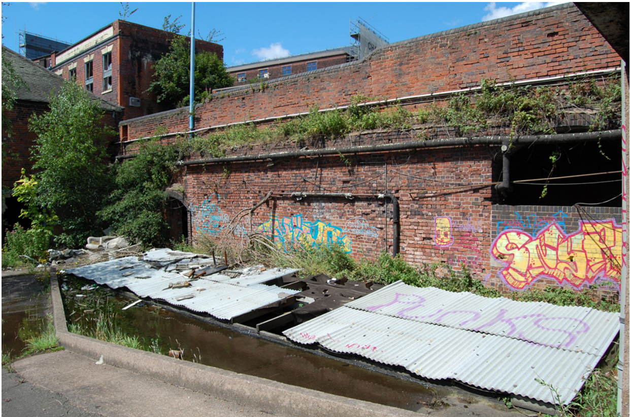
Plate 02: Entranceways to tunnels between Buildings A and B.
