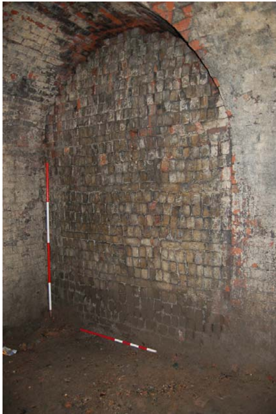
Plate 15: Blocked archway, east end.
