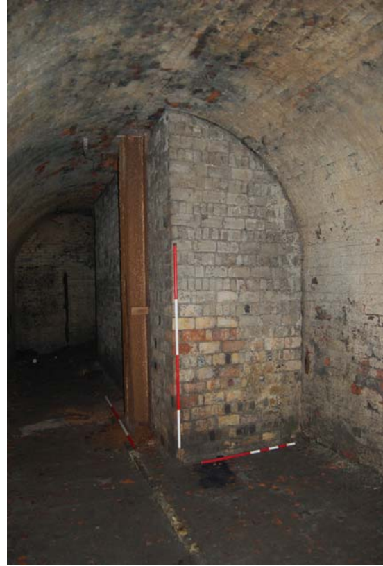
Plate 14: Inserted brickwork, east end.
