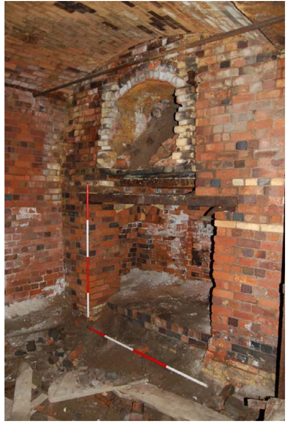
Plate 32: East end, openings in east wall.
