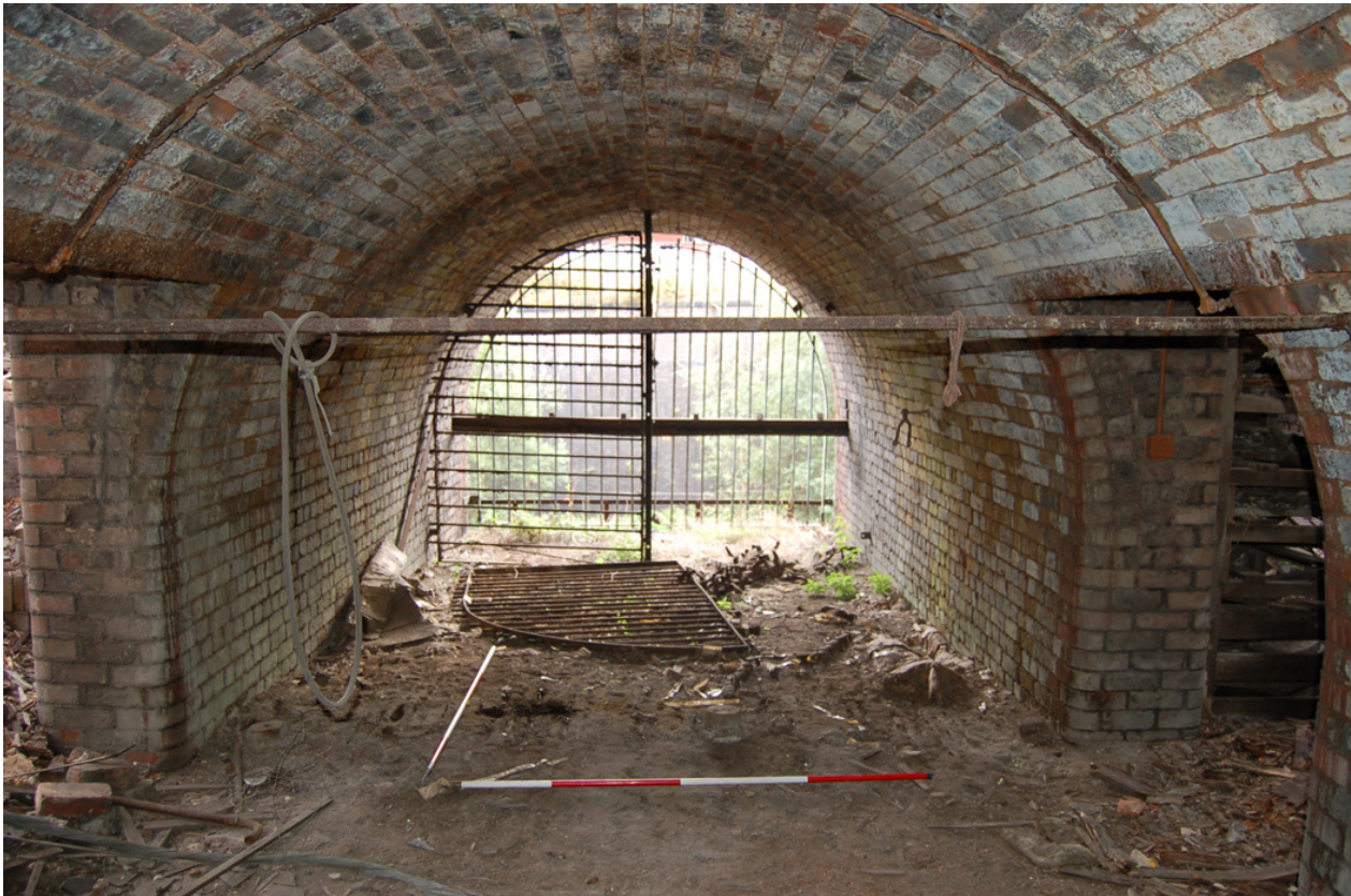
Plate 14: Building C, Level 1; central entrance tunnel looking south.
