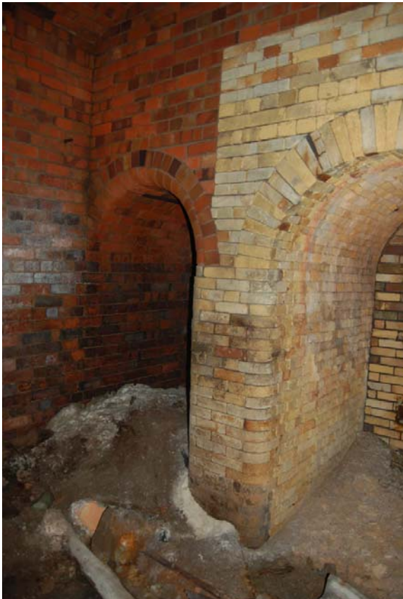
Plate 26: Tunnels F (right) and G (left).
