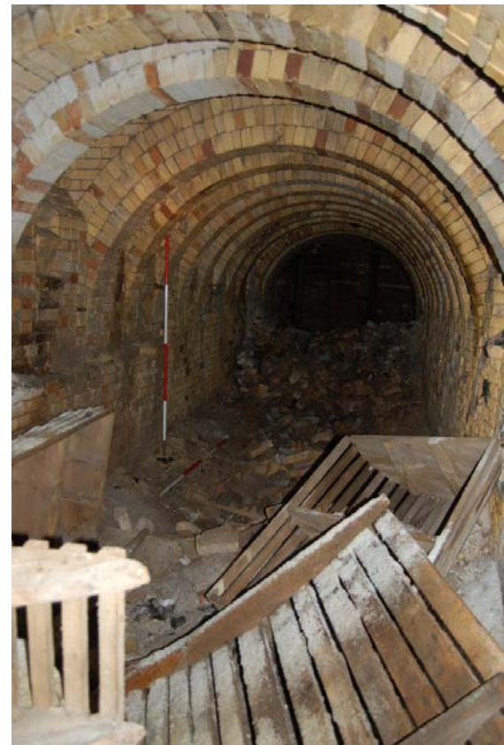
Plate 21: Tunnel C, looking east.
