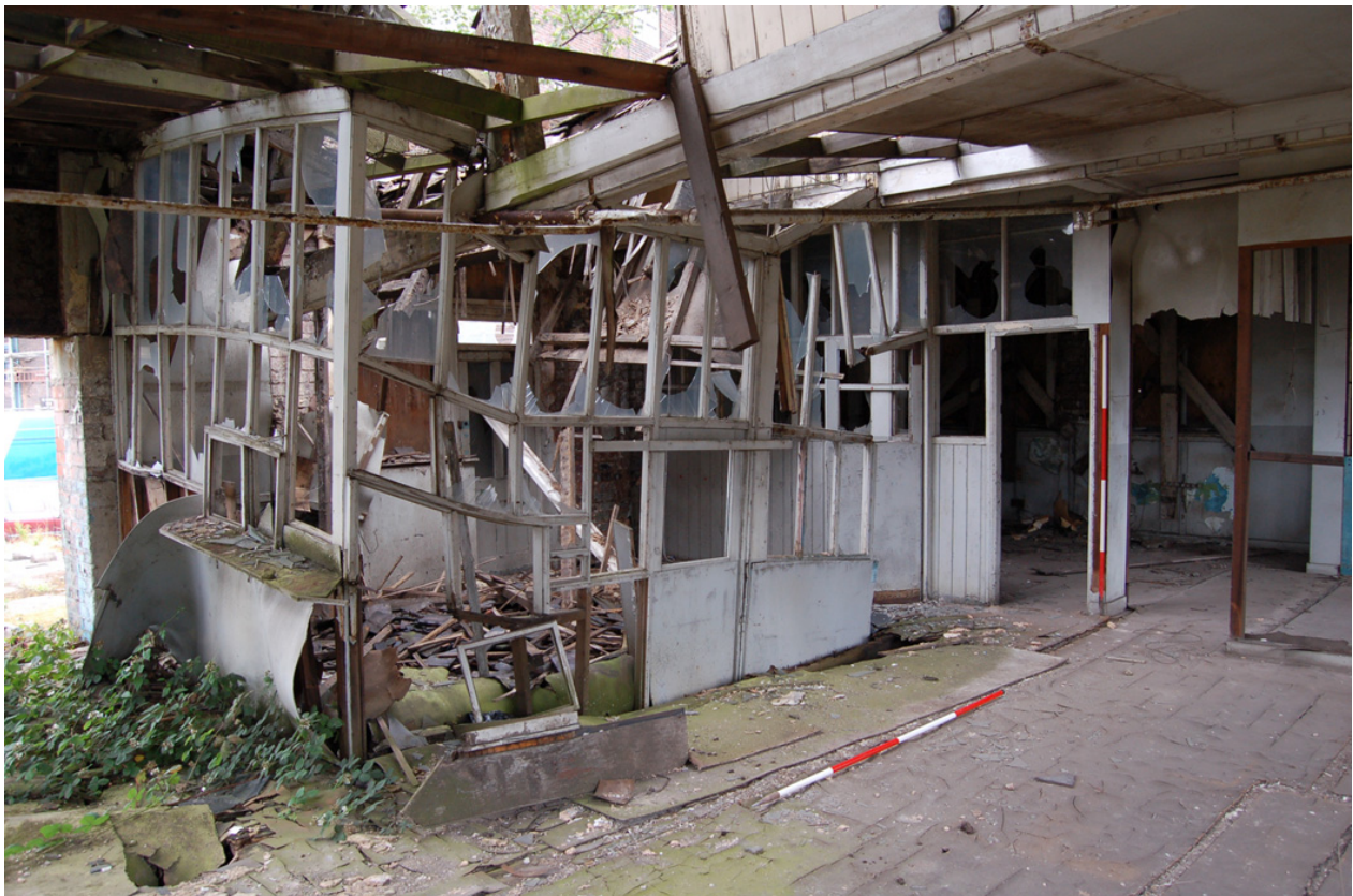
Plate 6: Building C, Level 2, east end; detail of office partitions.
