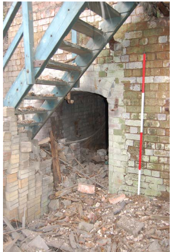
Plate 17: Entrance to furnace base (inserted).
