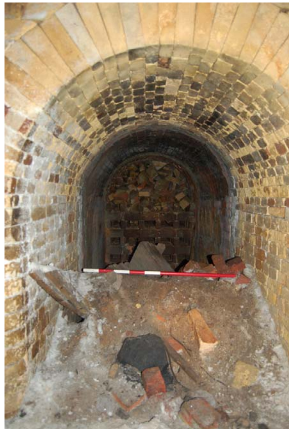
Plate 30: Tunnel B looking west, note packing.
