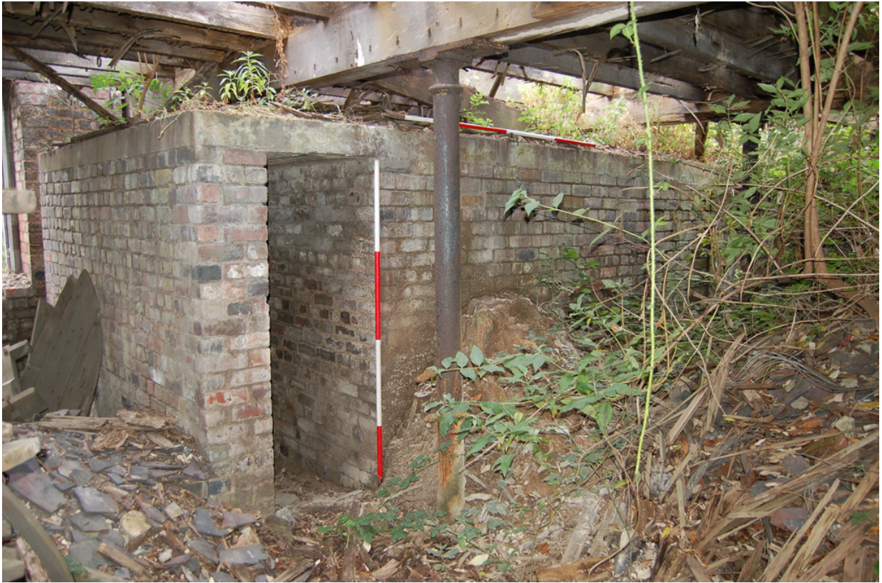
Plate 15: Building C, Level 1 (W); inserted store.
