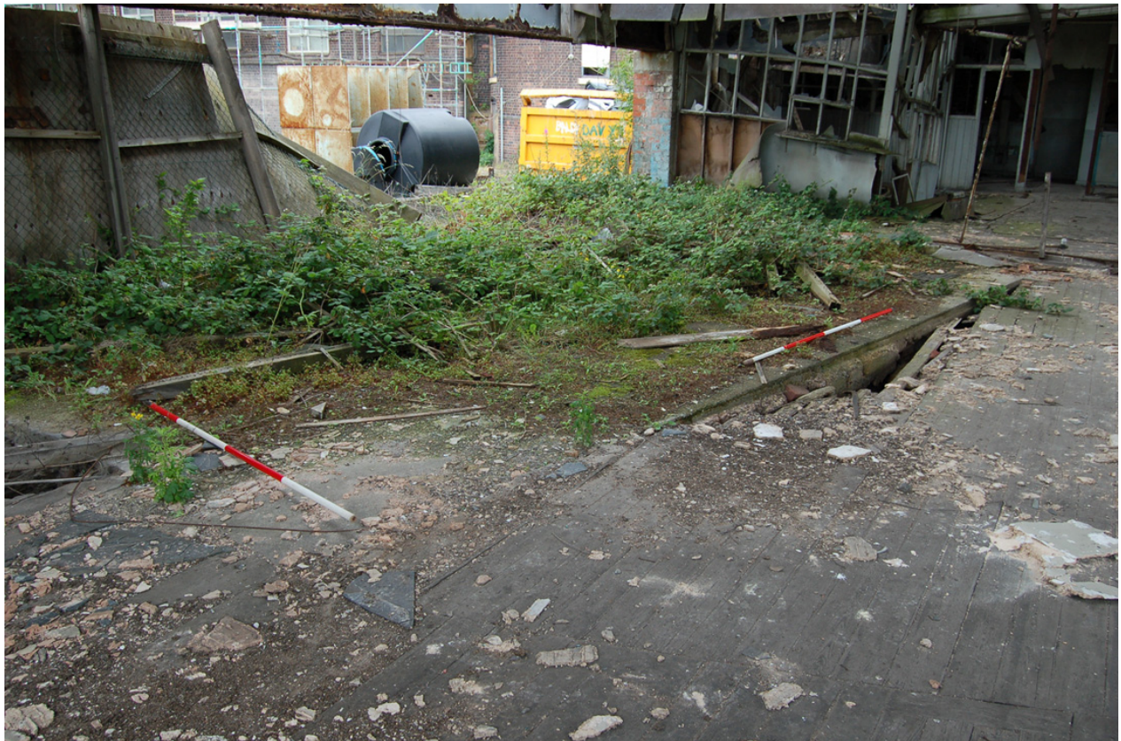
Plate 8: Building C, Level 2; concrete top of inserted Level 1 structure.
