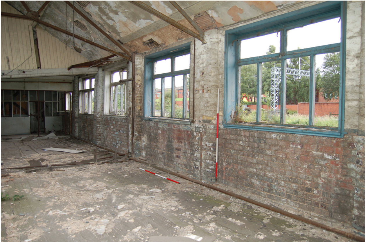
Plate 9: Building C, Level 2; fenestration of south elevation (E).
