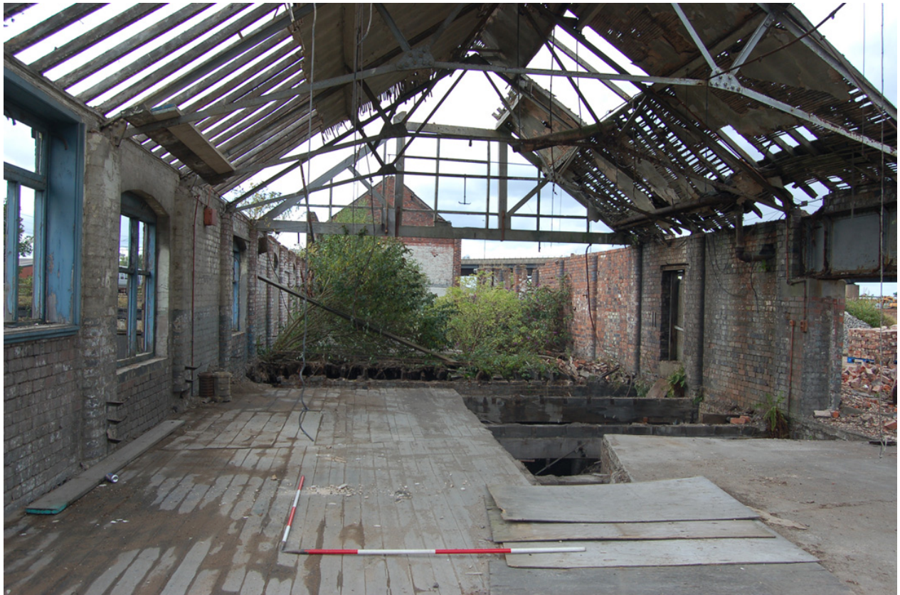
Plate 7: Building C, Level 2 looking west.
