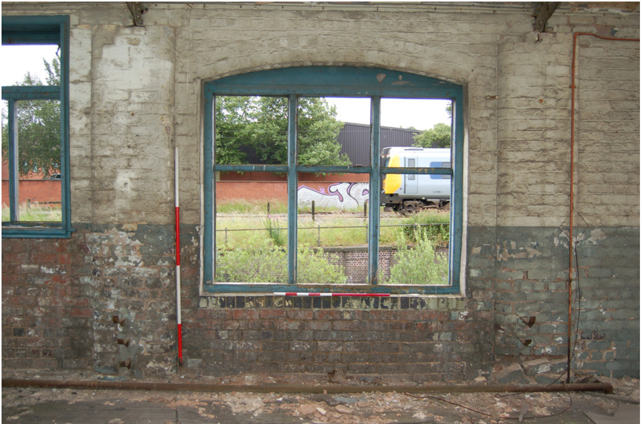
Plate 10: Building C, Level 2; fenestration of south elevation (W).
