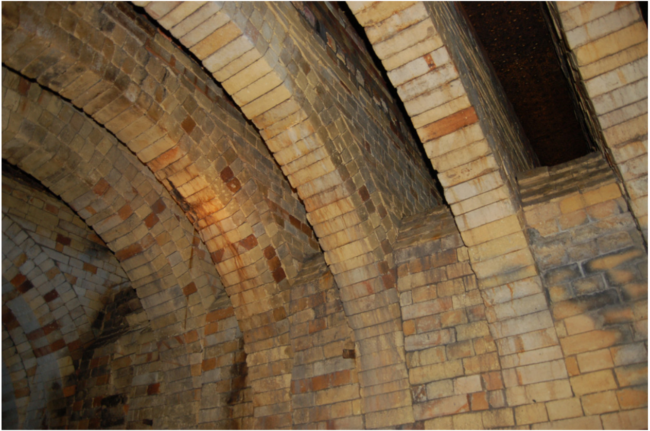
Plate 22: Tunnel C, detail of brick ribs.
