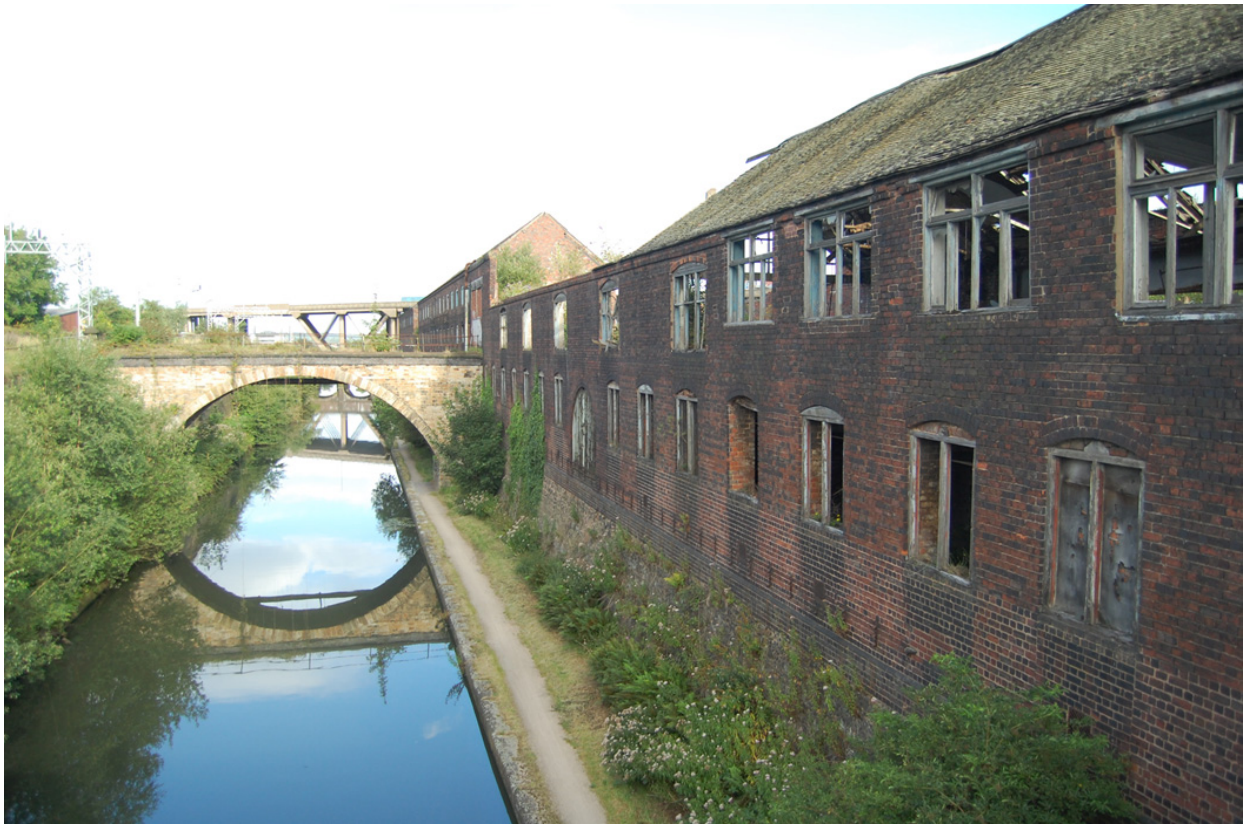
Plate 1: Building C, oblique view looking west from Canal Bridge.
