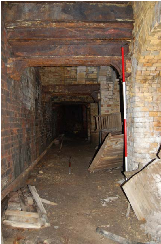
Plate 18: Western passage looking north.
