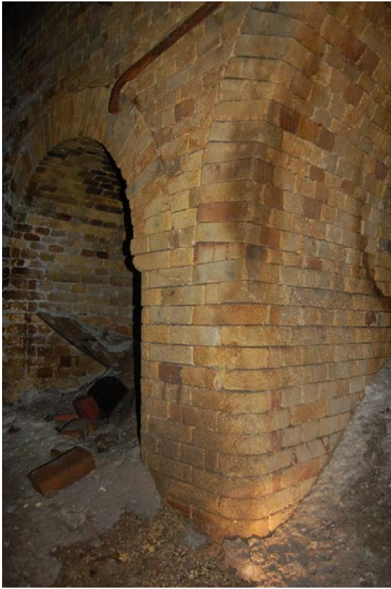
Plate 31: Brick detailing to east end arches.
