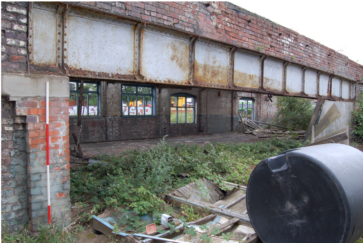
Plate 4: Building C, north elevation, inserted iron girder over wide opening.
