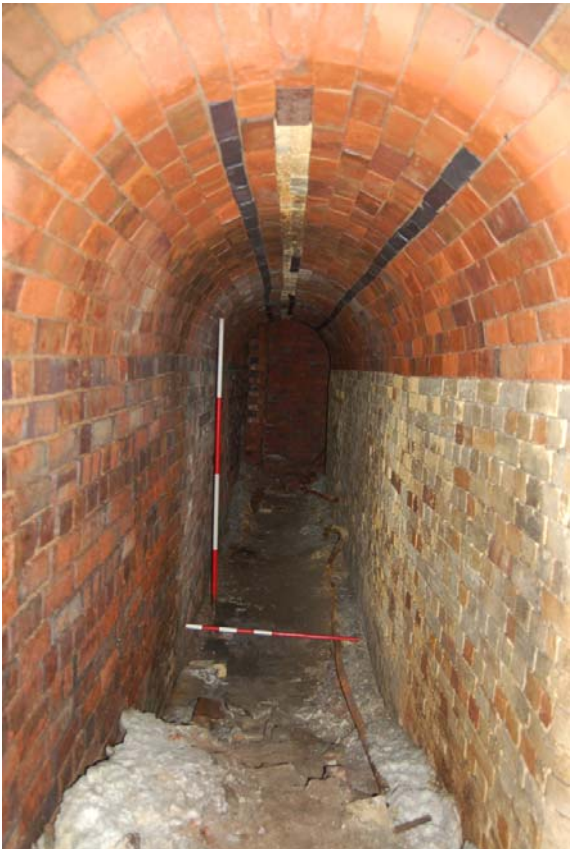
Plate 27: Tunnel G looking east.
