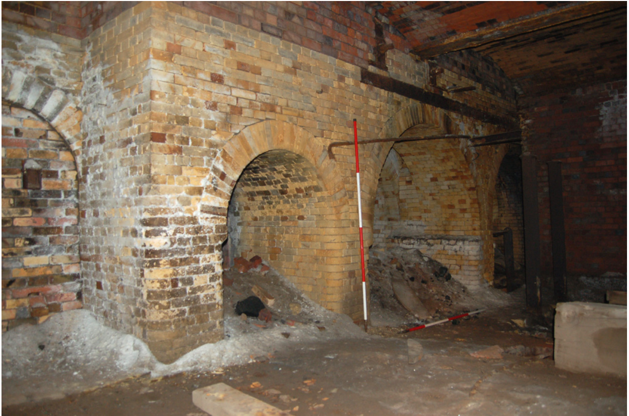
Plate 28: Furnace base, east end; tunnels A (left; blocked), B and C (middle), and D (far right).
