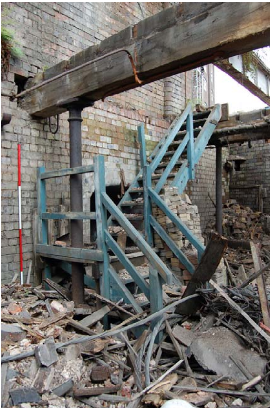
Plate 16: Stair against north wall.
