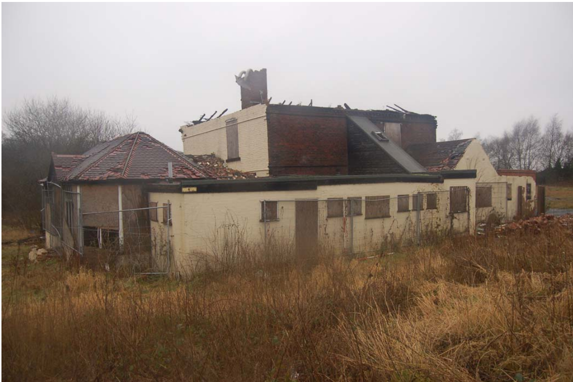
Plate 6: North-east elevation, oblique view.
