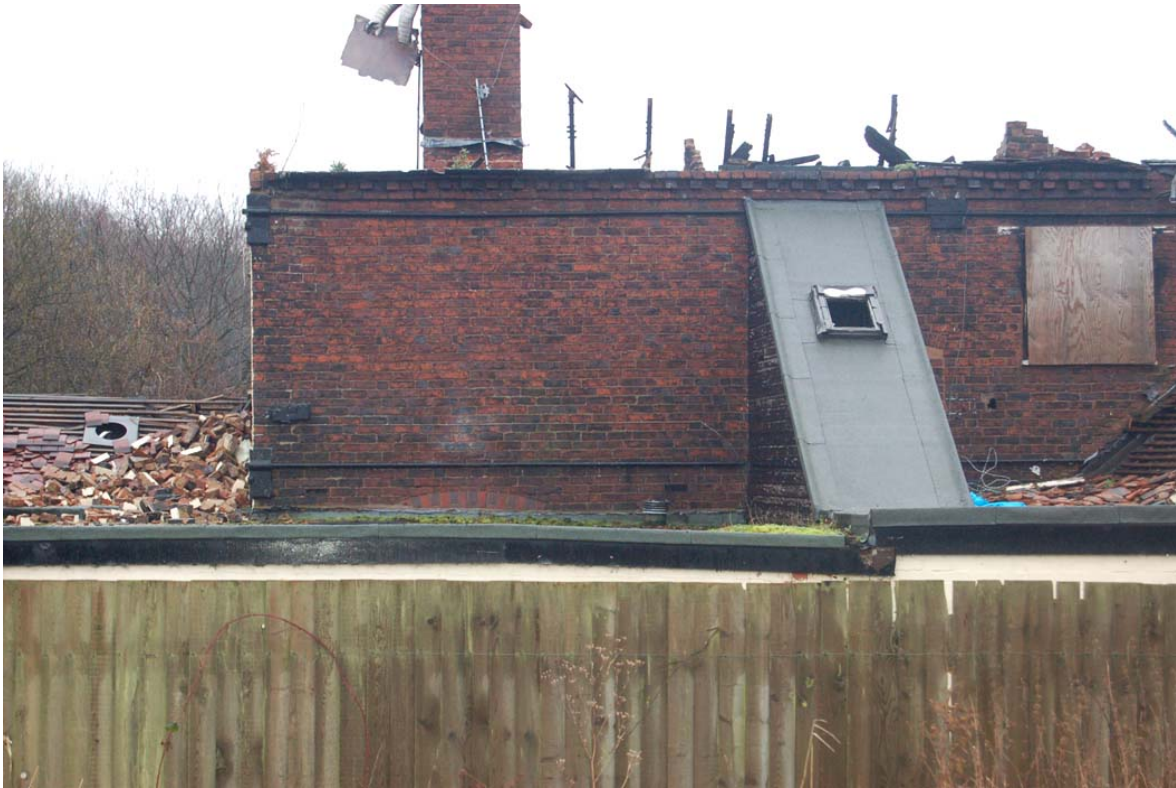
Plate 10: NE elevation, detail. Note brick arch below lower tie rod to left of stair.
