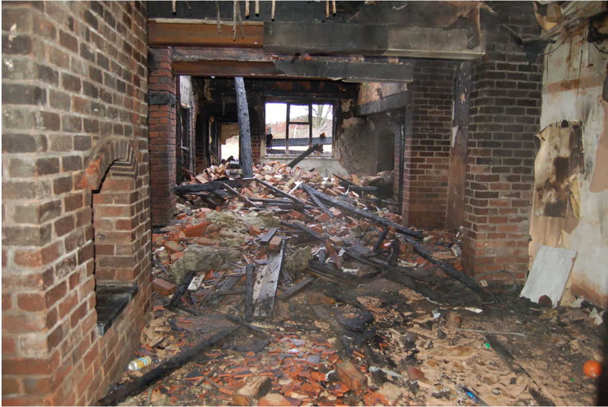
Plate 12: Ground floor interior, Rom G1 looking north-west.
