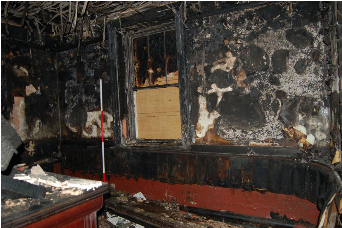
Plate 16: Ground floor interior Room G2, bar area looking south.
