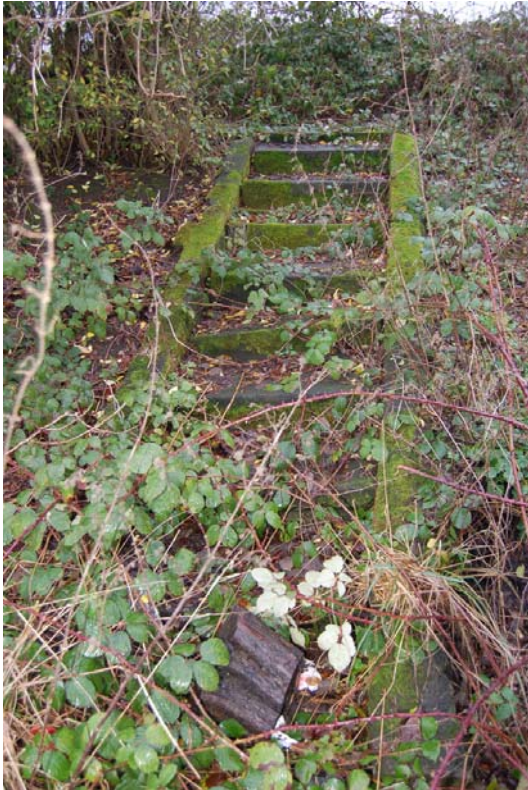
Plate 24: Surviving stone stair to south-east of The Wharf, formerly serving bowling green.
