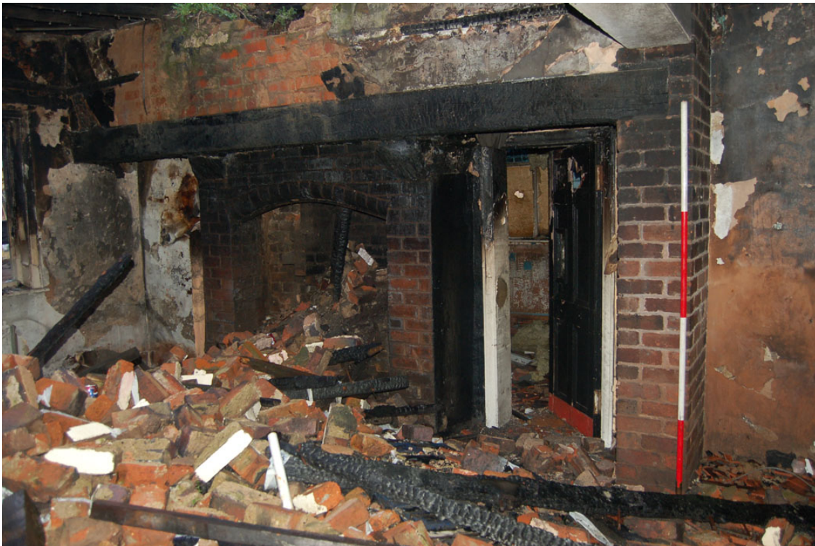
Plate 13: Ground floor interior, Room G1: fireplace.
