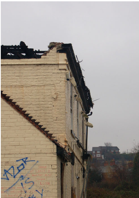
Plate 8: Rebuild of front wall (NW elevation).
