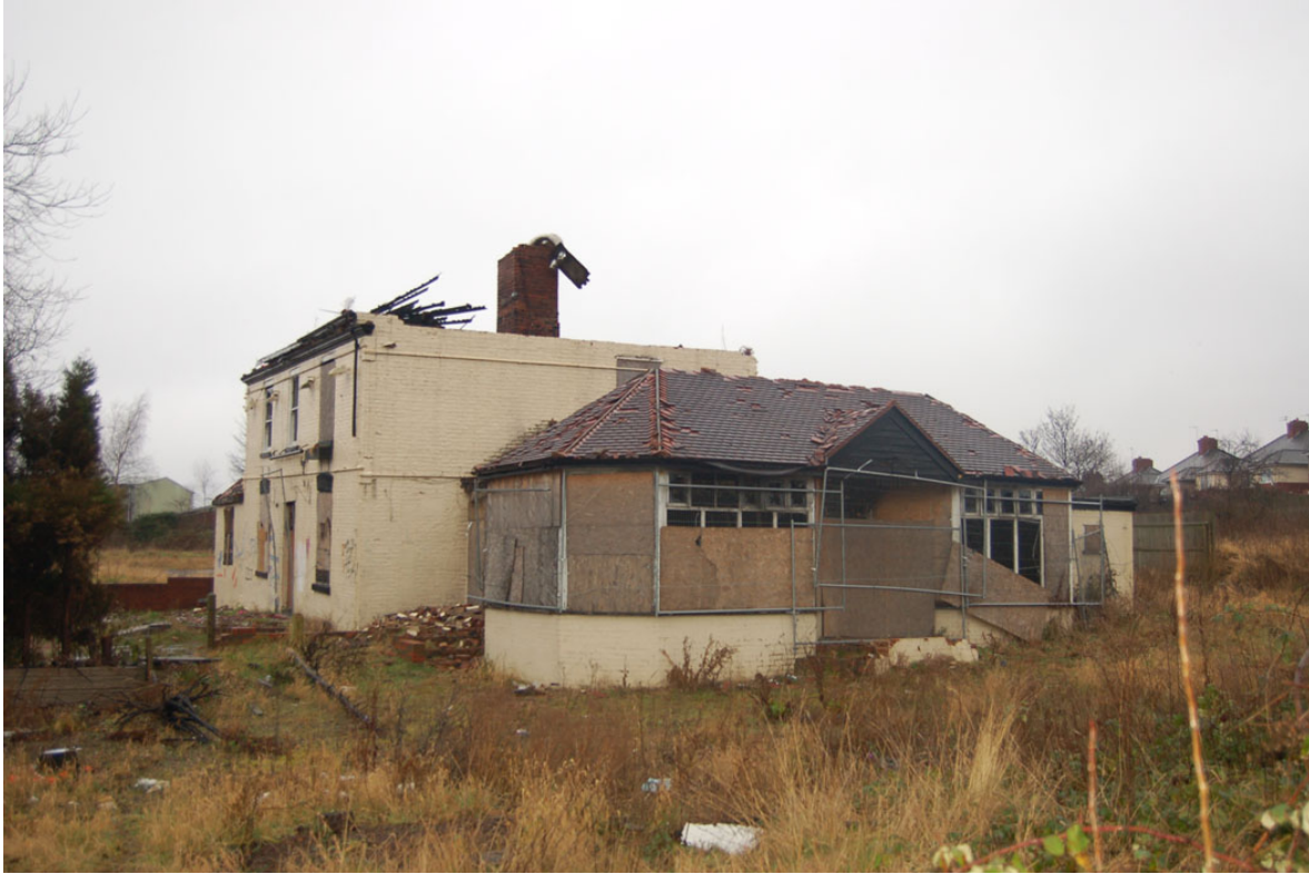
Plate 5: South-east elevation, oblique view.
