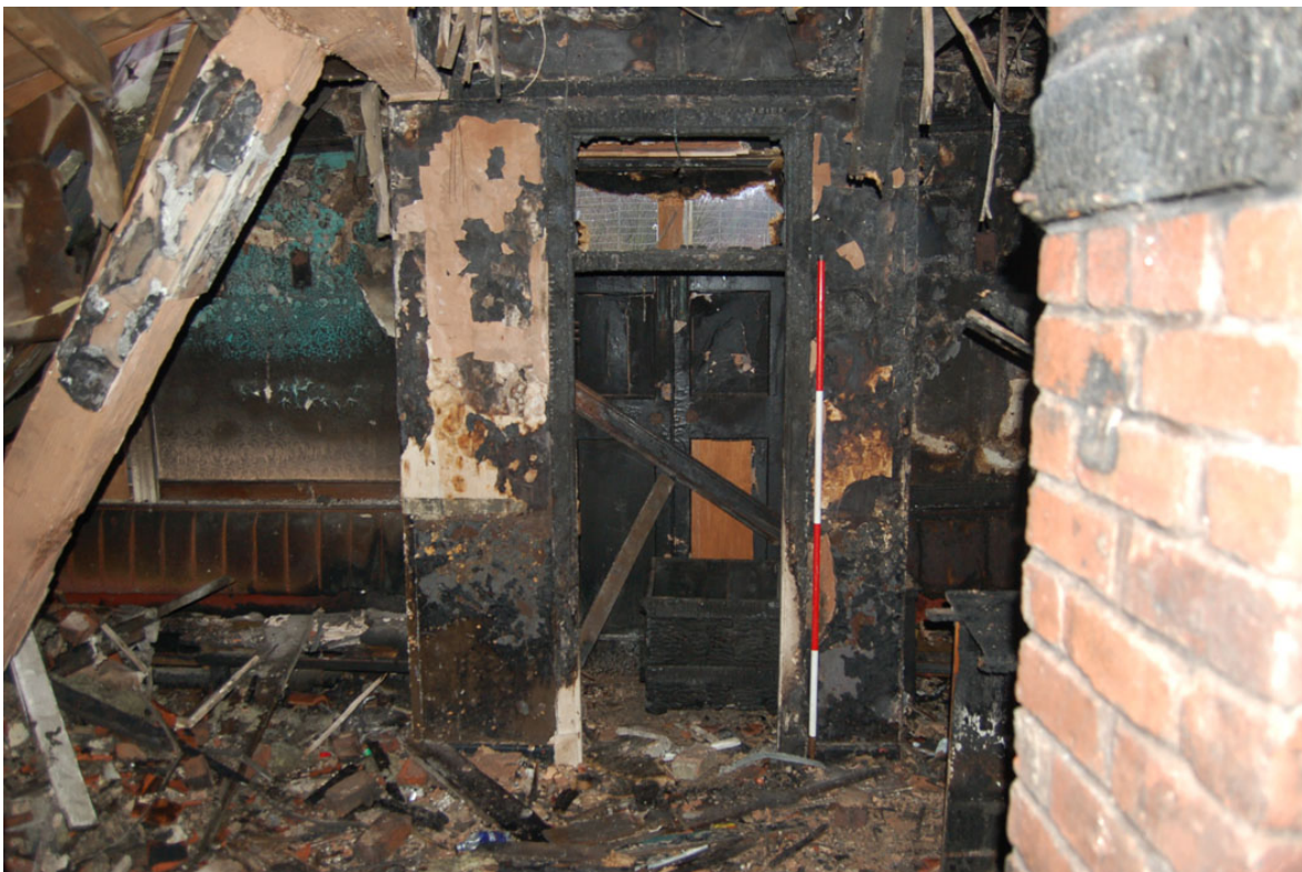
Plate 17: Ground floor interior, Room G2 entrance way.
