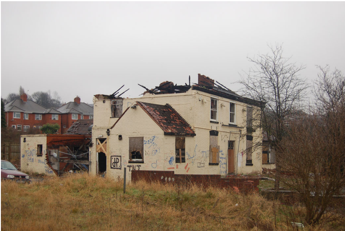
Plate 3: General view from the west.
