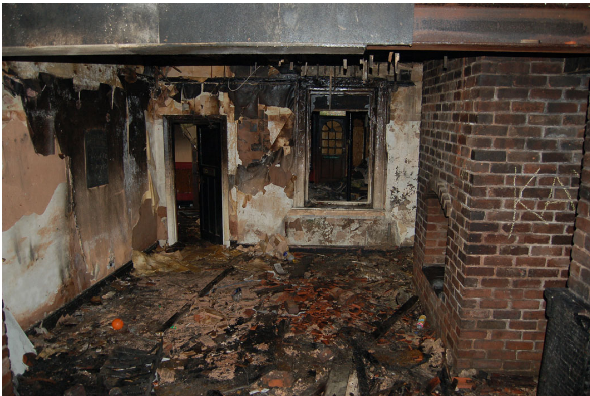
Plate 14: Ground floor interior. Room G1 looking south-east.
