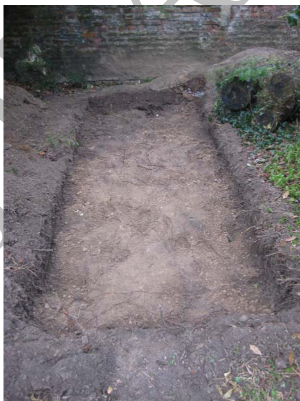
Figure 3: Photograph of Trench 9, identifying the shallow topsoil encountered overlying the natural deposits. The potential for palaeosol preservation was shown to be low.
