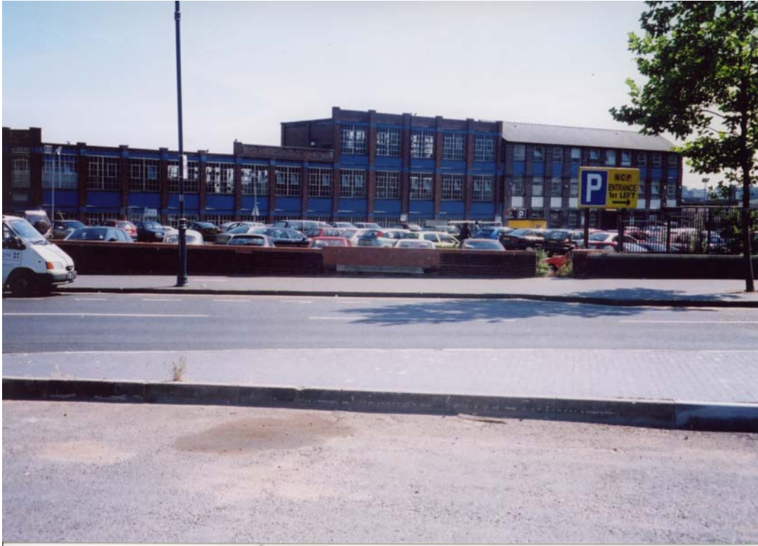
Plate 17: 20 th -century industrial buildings fronting onto Bartholomew Street, photographed in 2002 before demolition.
