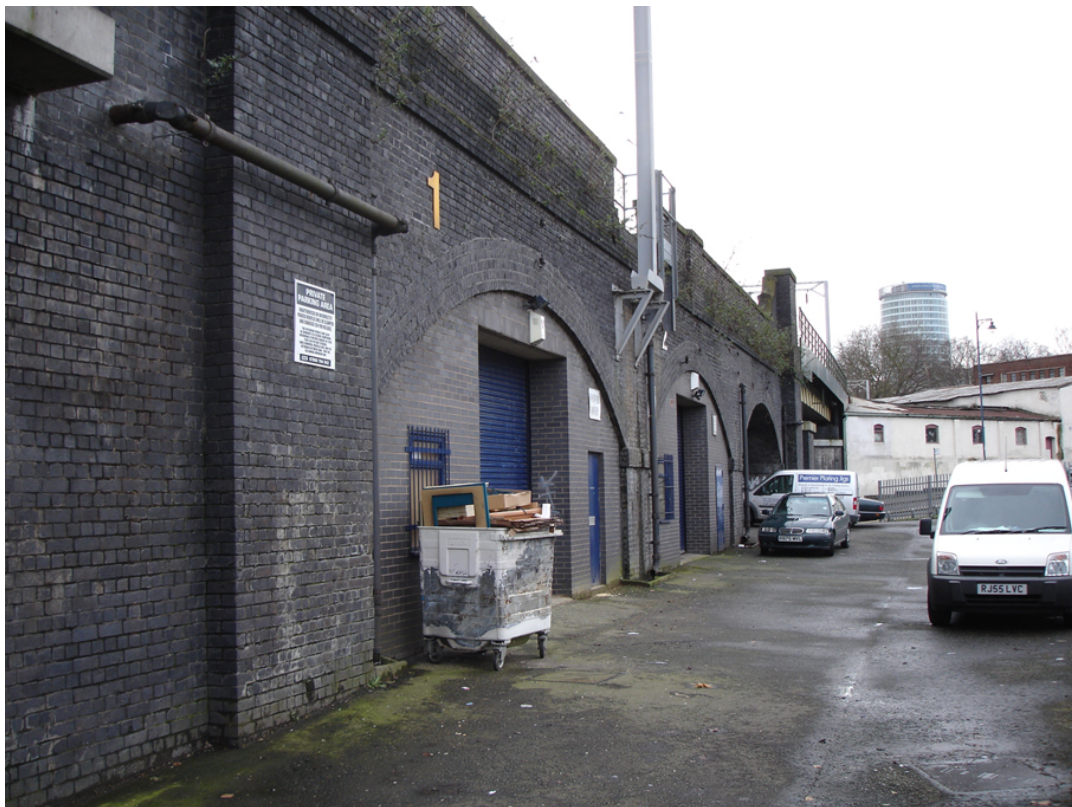
Plate 8: Arches of railway viaduct forming southern boundary of study area.
