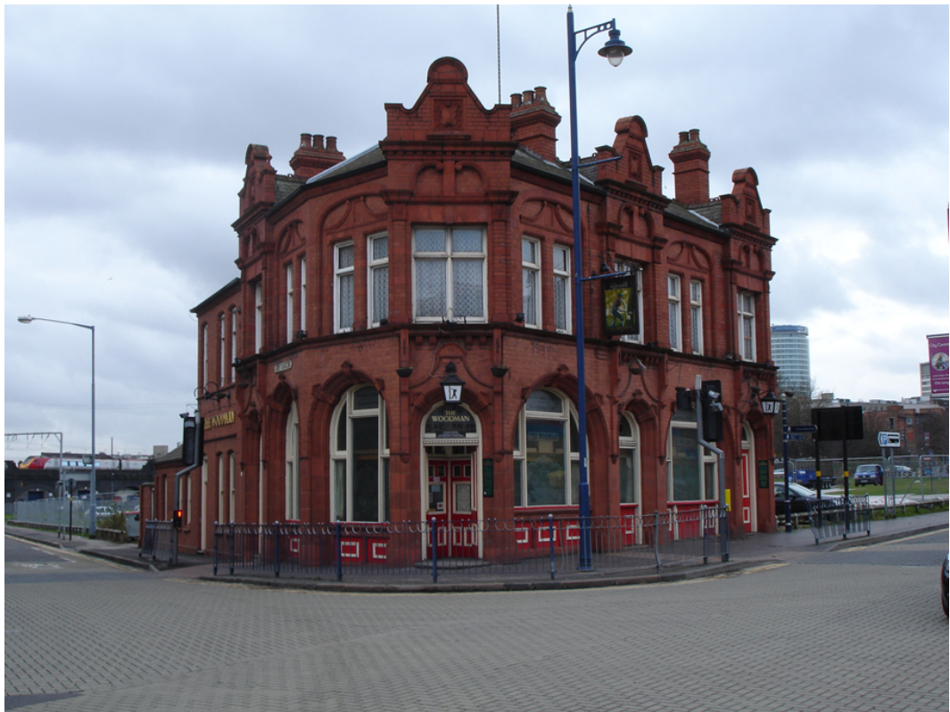
Plate 4: The Woodman Public House, Grade II Listed, SMR ref. 03922.
