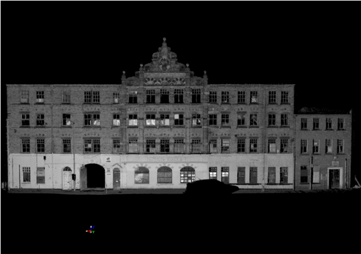
Plate 1: Point-cloud data of main western elevation.
