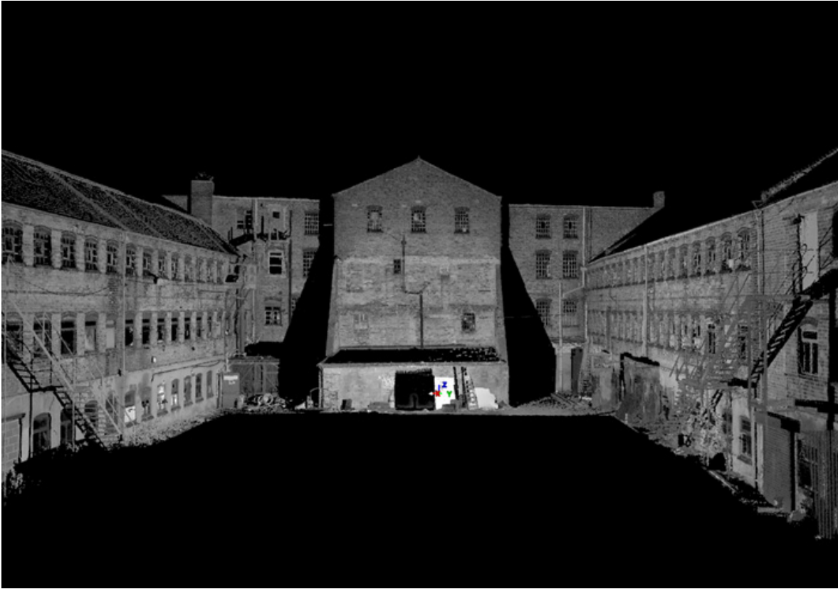
Plate 3: Point-cloud data for courtyard elevations.
