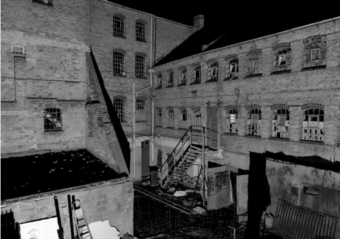
Plate 4: Detail of junction of north and west ranges.
