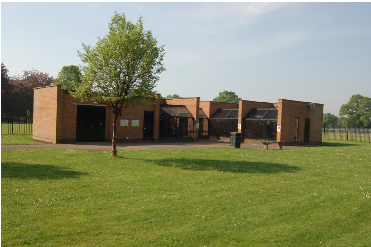
Plate 11: Red-brick aviary building looking south-west.
