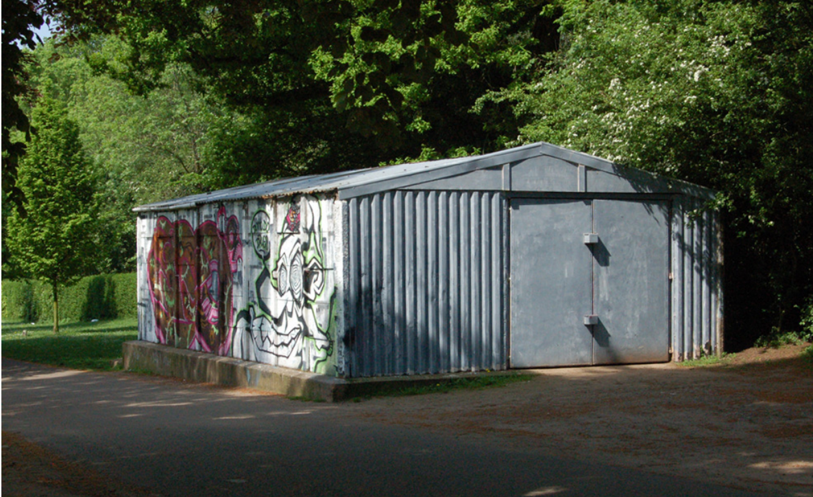
Plate 25: Unsympathetic tool store building against Kenilworth Road boundary.
