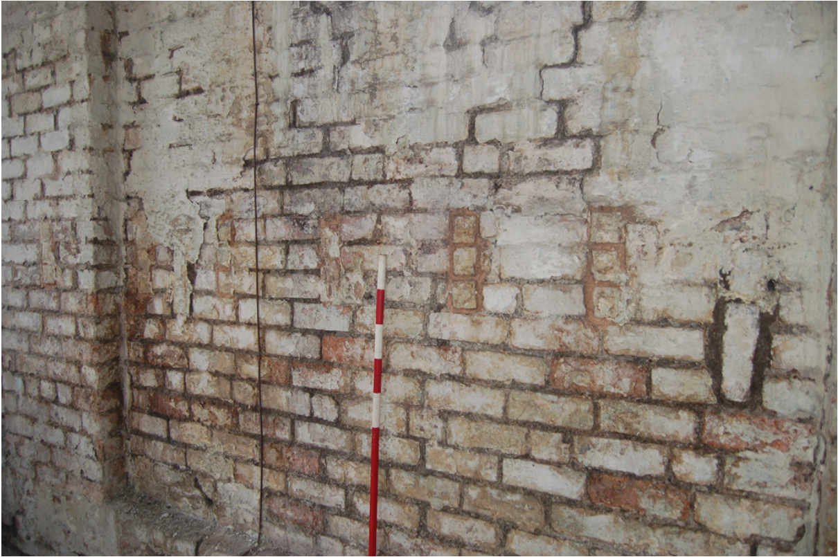
Plate 27: First floor, infilled joist sockets denoting former floor level.
