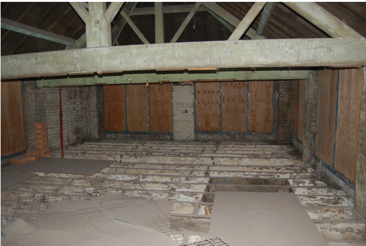
Plate 31: Second floor ventilation openings, looking east.
