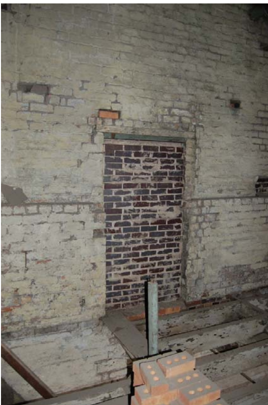
Plate 32: Second floor, blocked door.
