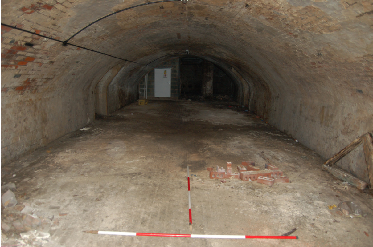
Plate 34: Main cellar, looking north towards brewery.
