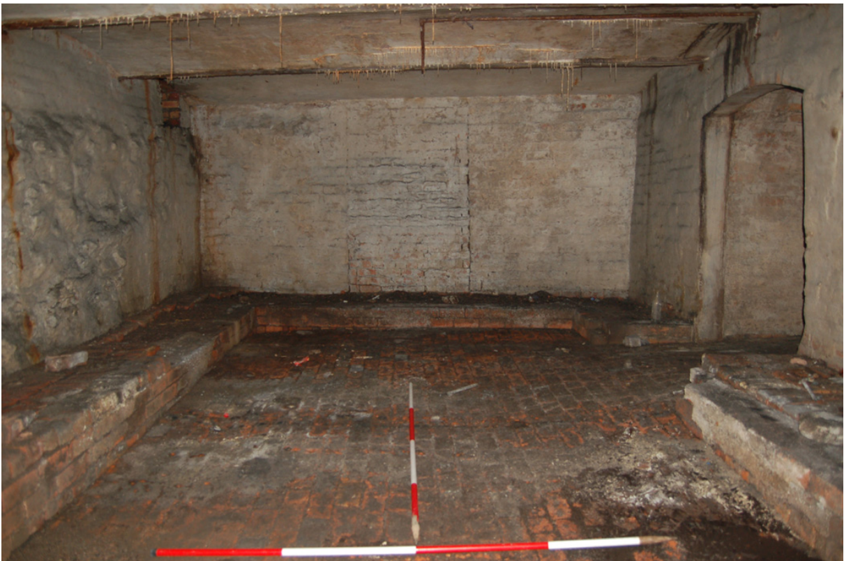
Plate 35: Side cellar to west, note stone wall to left.
