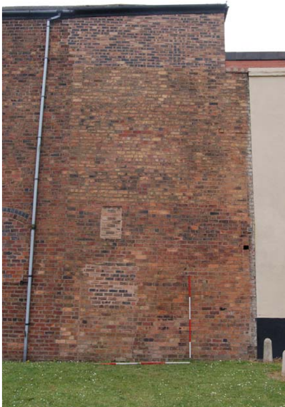
Plate 13: Stairwell/lift shaft; north elevation.
