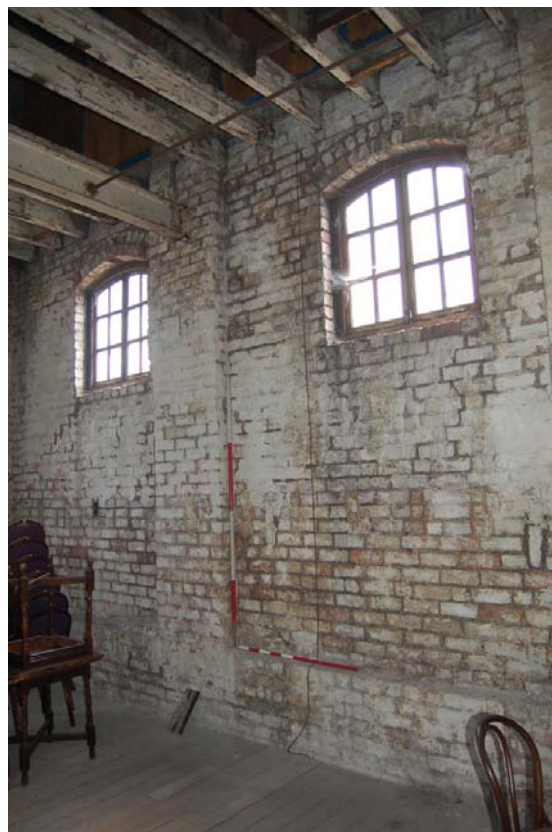
Plate 24: First floor; high level windows.
