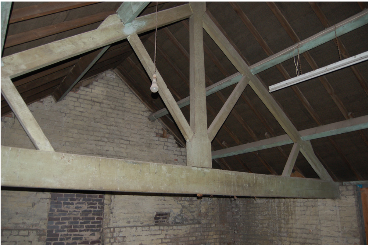
Plate 30: Second floor. roof structure.
