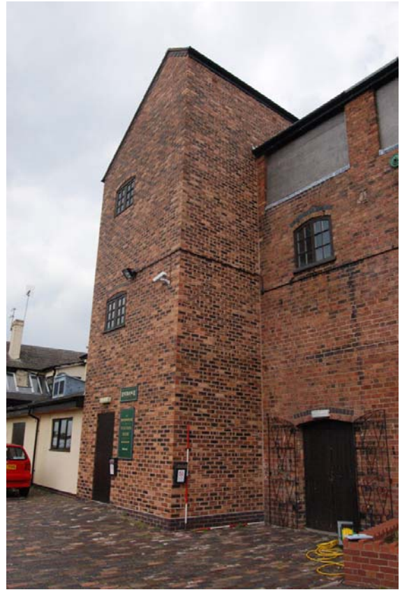
Plate 8: Stairwell/lift shaft; oblique view.
