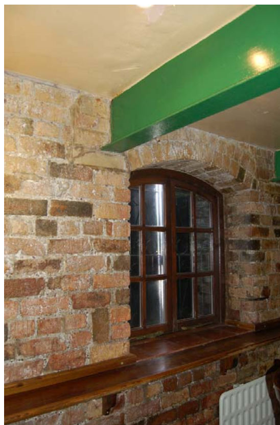
Plate 20: Patching around inserted joists.
