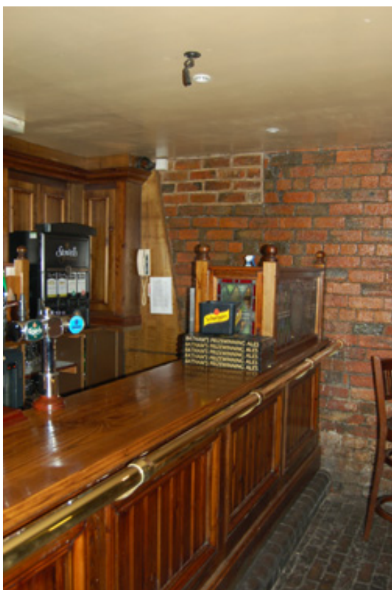
Plate 19: Blocked window behind bar area.
