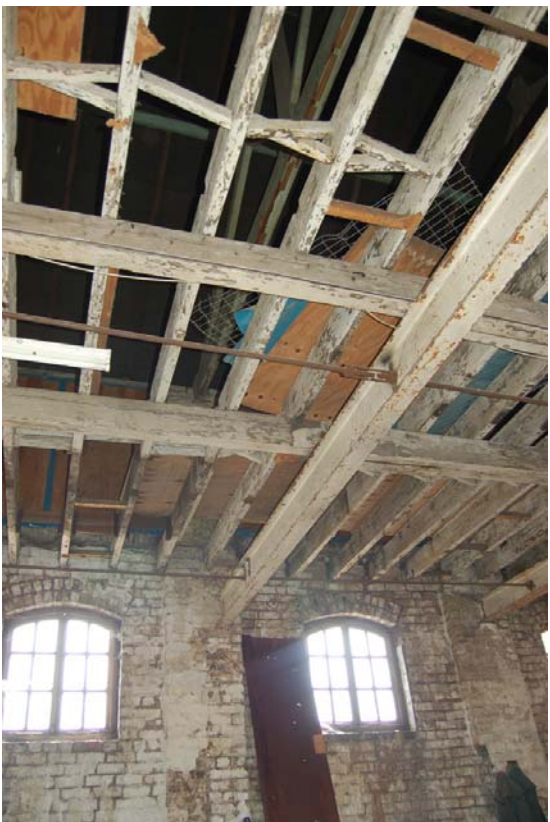
Plate 25: Second floor structure.
