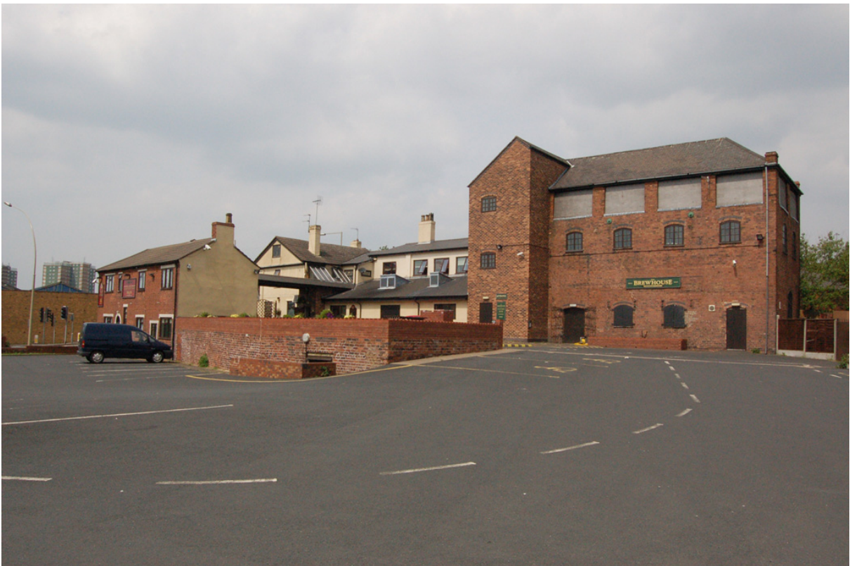
Plate 2: The former brewhouse range to rear of the Lamp Tavern, general view from the south.
