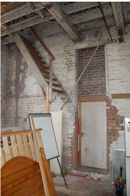
Plate 23: First floor, west wall and stair.
