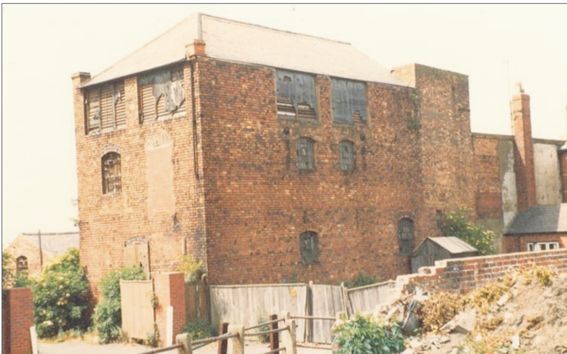
(b) Former Queens Cross Brewery photographed in 1981 (DALs P/1588). Note louvres to upper level and original iron-frame windows, also the related brewery building to left background, originally forming the southern boundary of the brewery yard.
