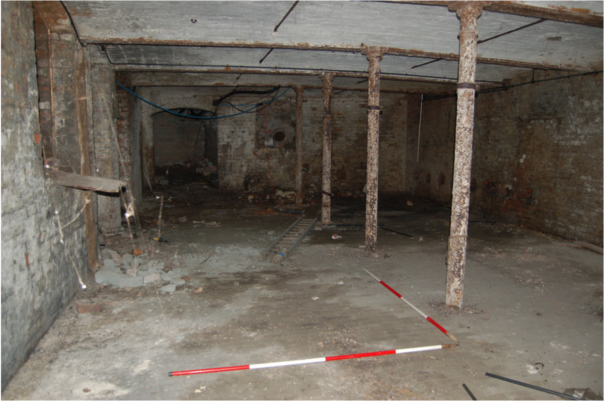
Plate 36: Cellar beneath brewery range, looking west.
