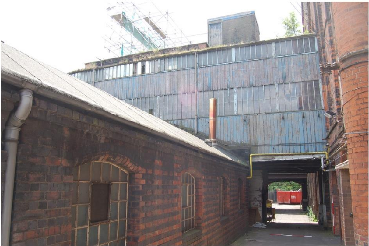
Plate 1: Link building from the north, note lift shaft projection.
