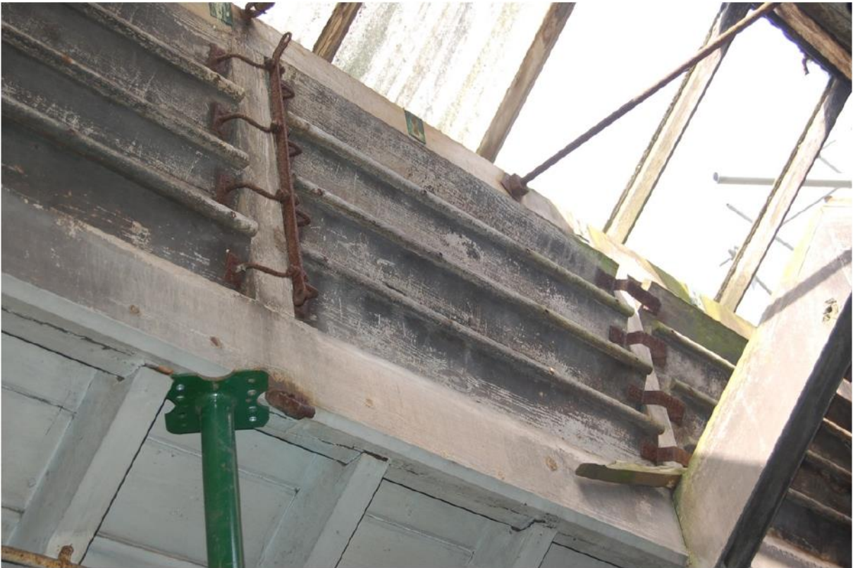
Plate 10: 2F level, timber roof louvres.
