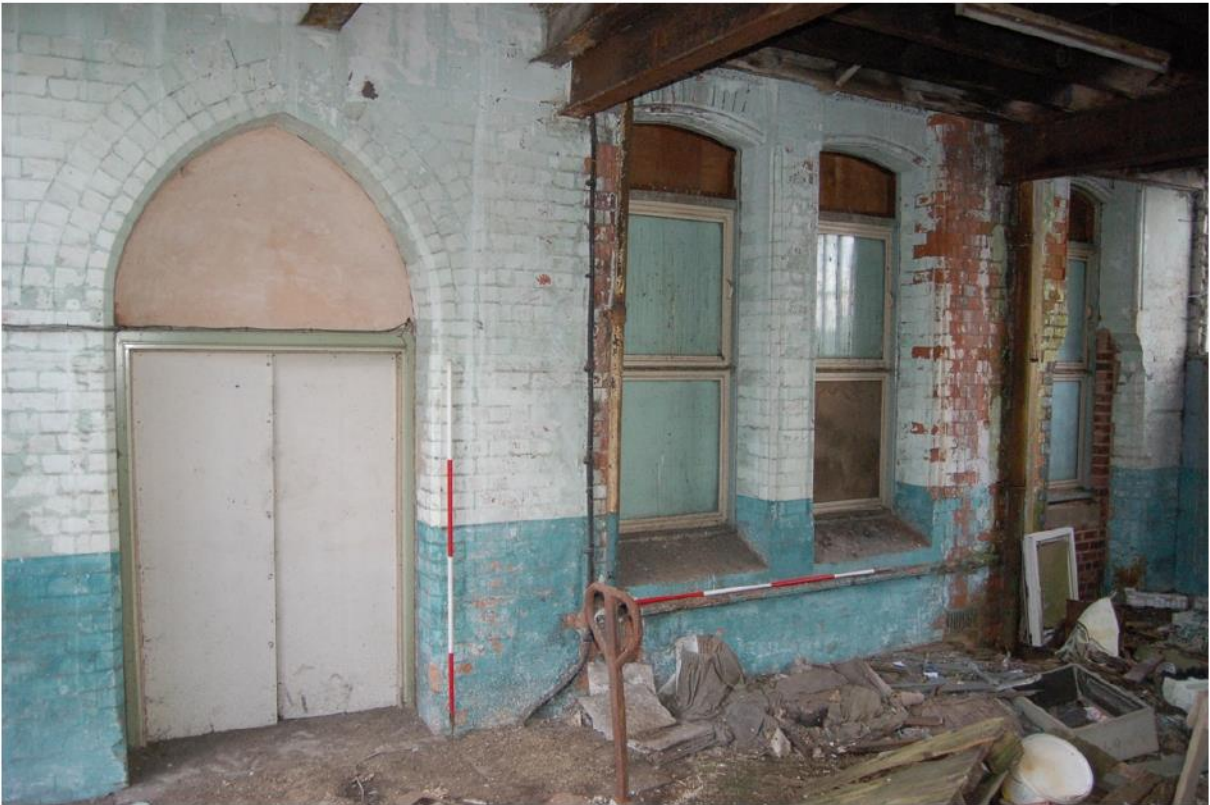
Plate 16: 1F level, west wall.
