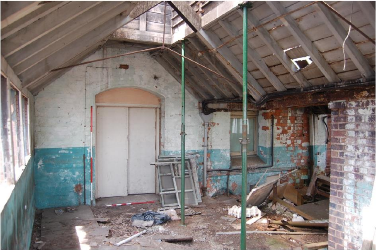
Plate 6: 2F level, looking west.
