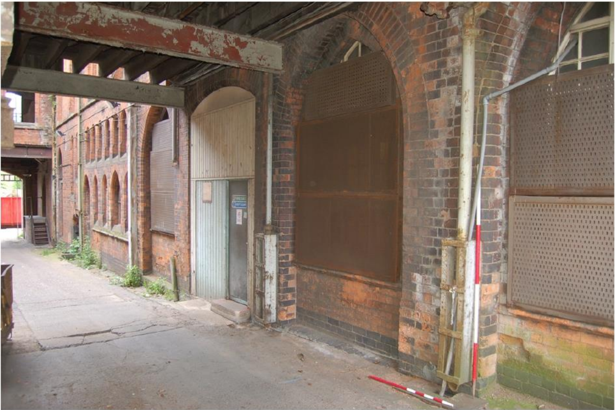
Plate 25: GF level, openings in east (office) range wall.
