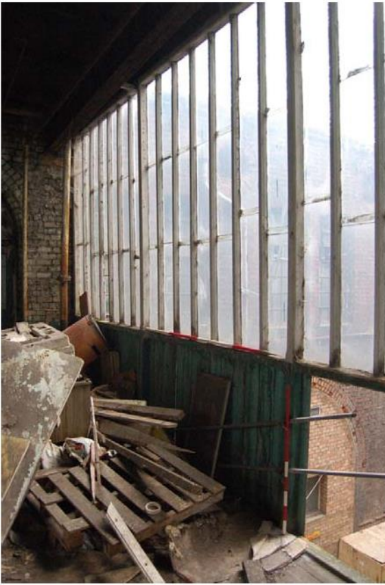
Plate 21: 1F, south wall.
