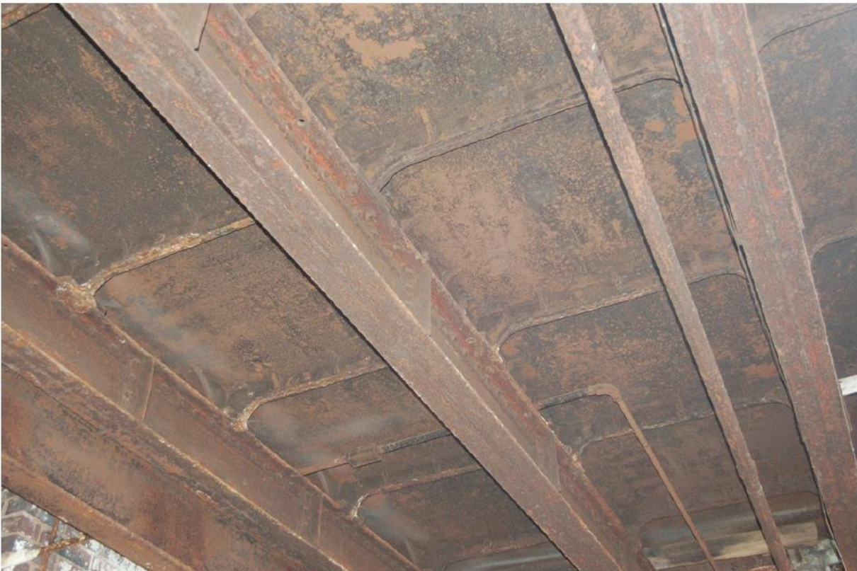
Plate 18: 2F floor structure, southern section.
