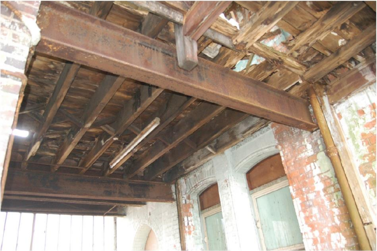
Plate 19: 2F floor structure, northern section.
