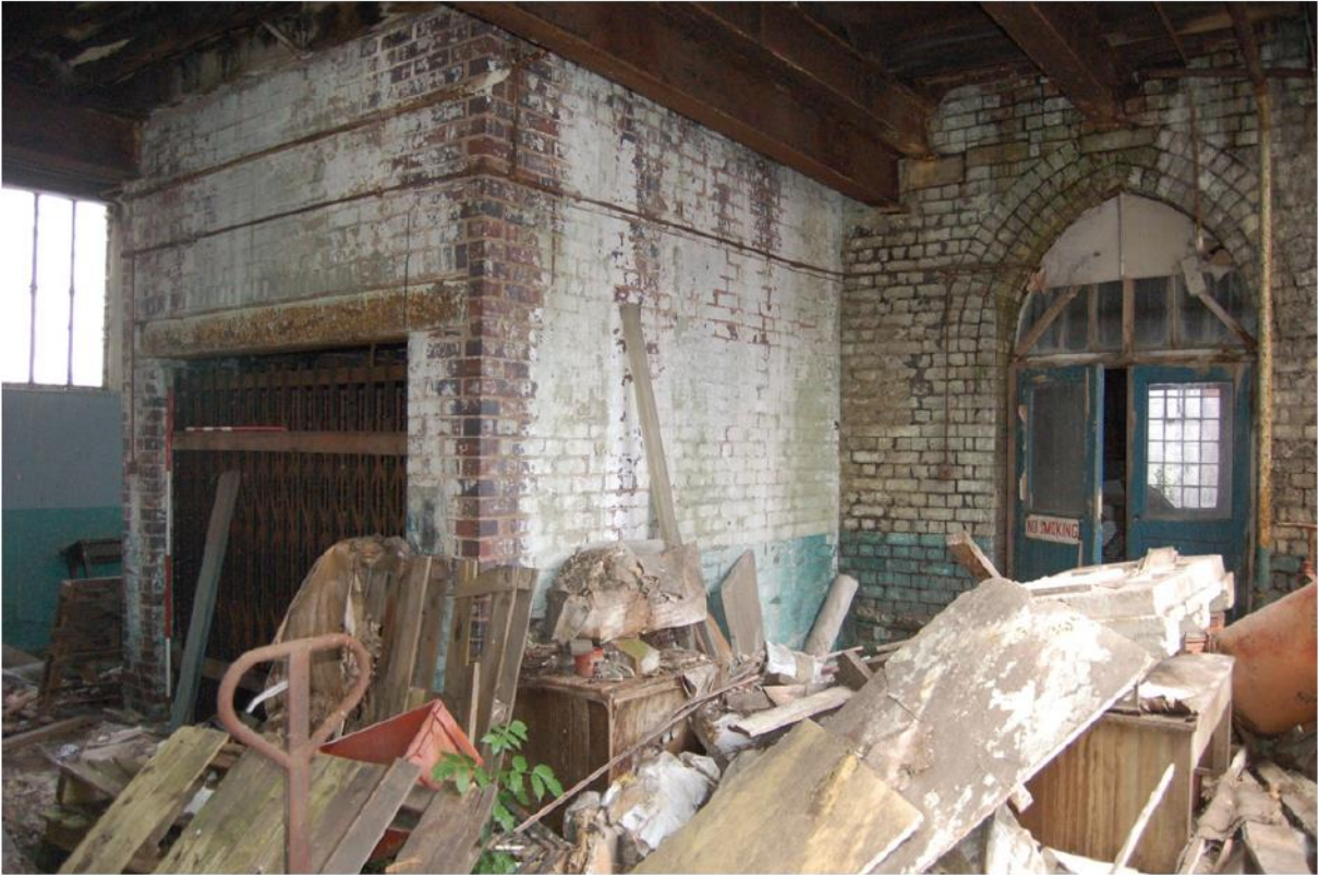
Plate 17: 1F level, east wall and inserted lift shaft.
