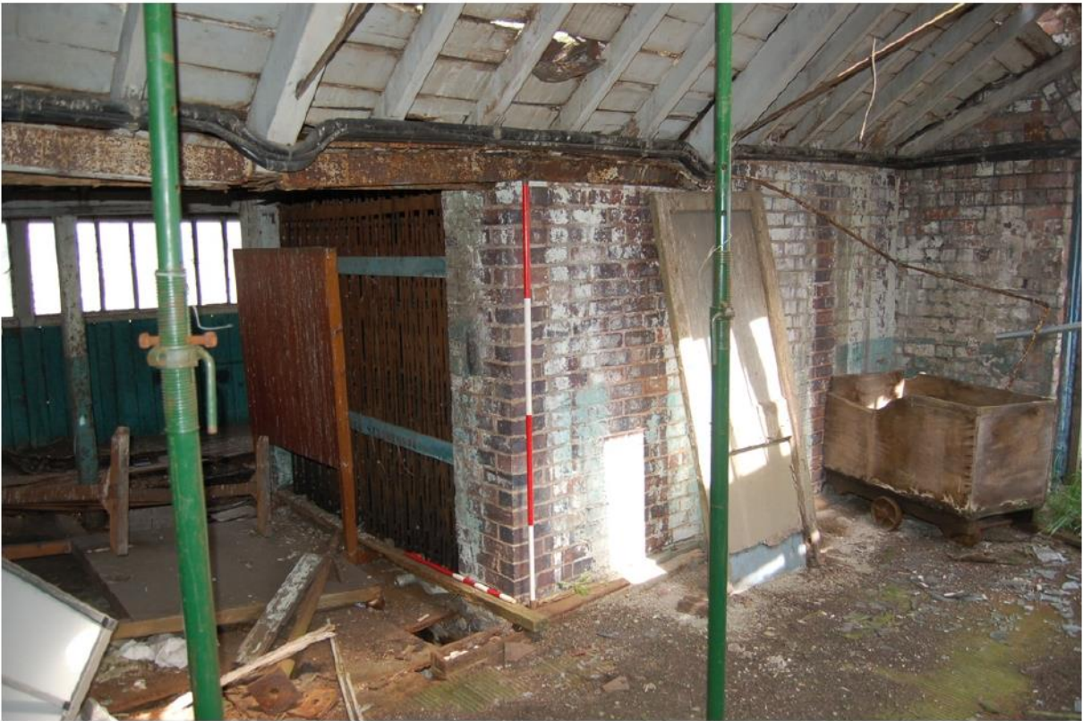
Plate 11: 2F level, inserted lift shaft.
