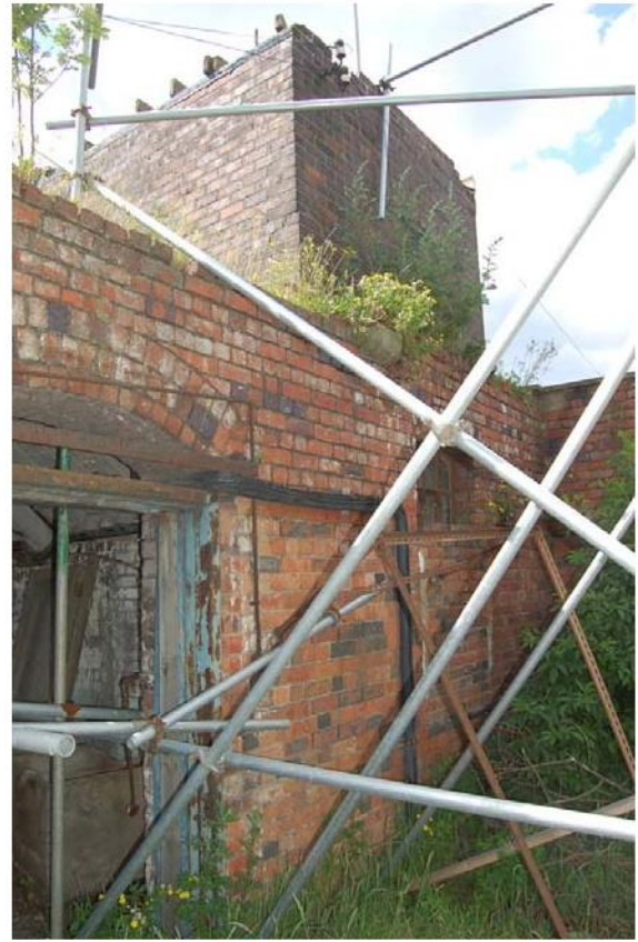
Plate 15: 2F, lift shaft blocking window.
