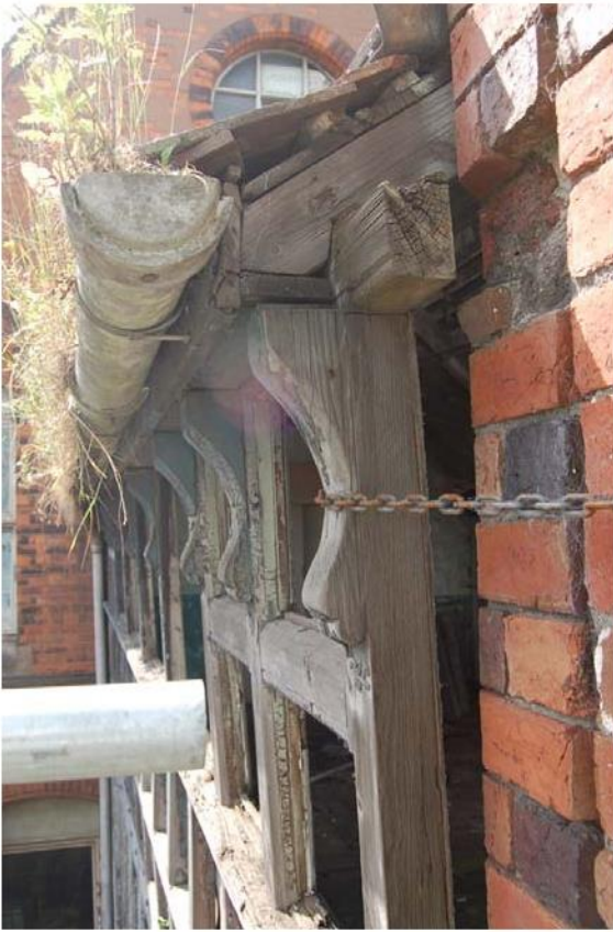
Plate 14: 2F, south wall structure.
