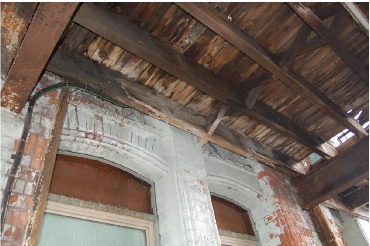
Plate 20: 1F, truncated windows in west wall (see also Plate 7).
