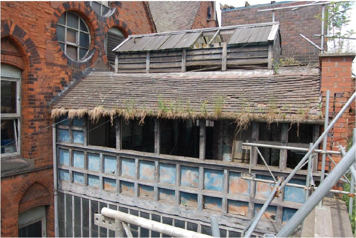
Plate 4: Link building from the south, 2F level.
