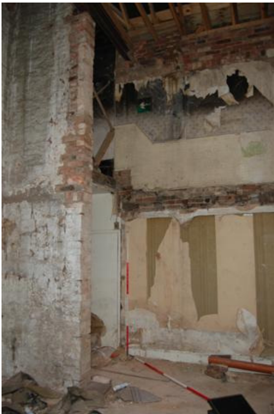
Plate 119: Bldg B, Block B1; Rm BG2/BF10 looking north-west.
