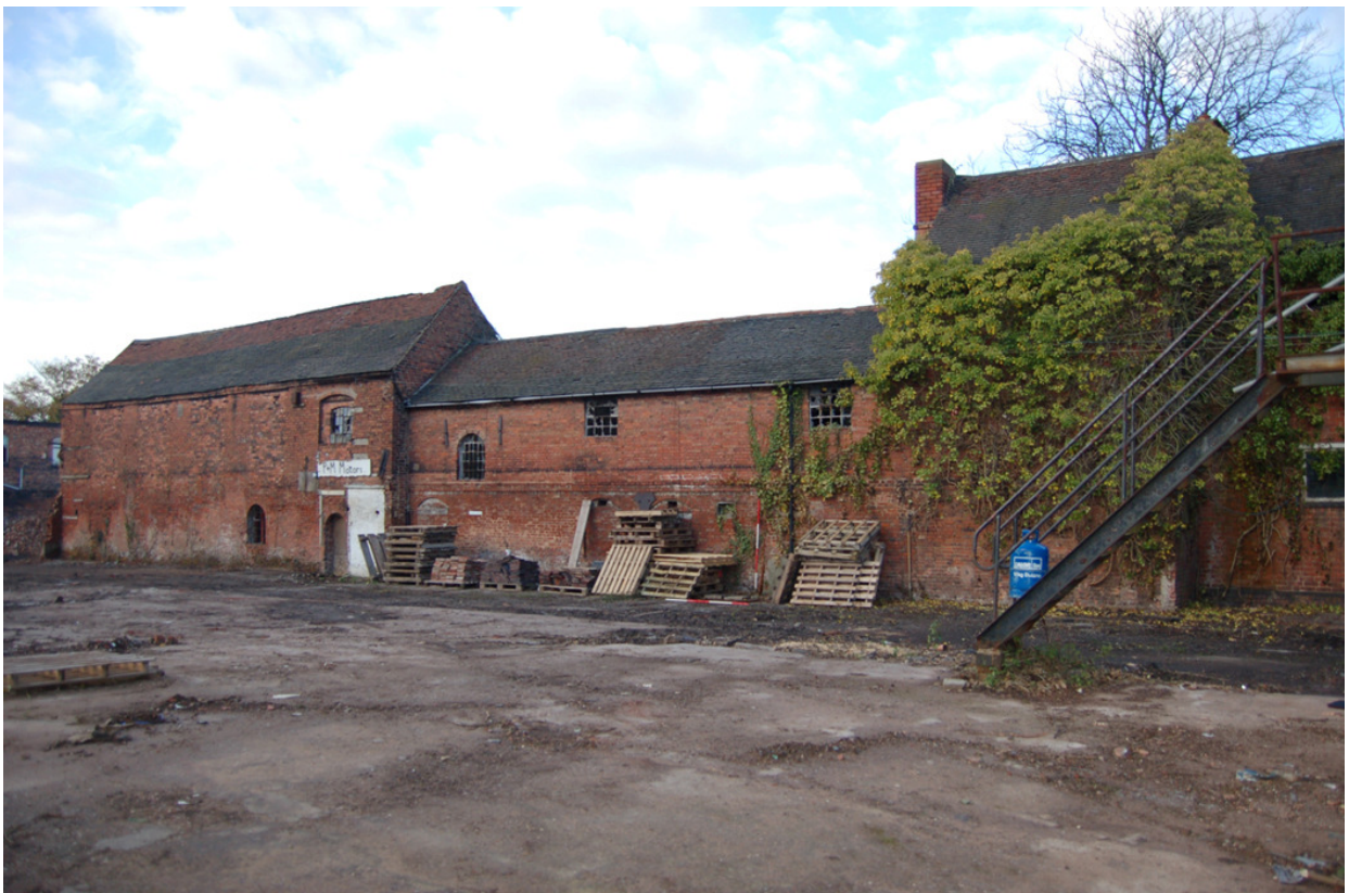
Plate 176 : Building B; rear range south elevation (Bldg. D to left).
