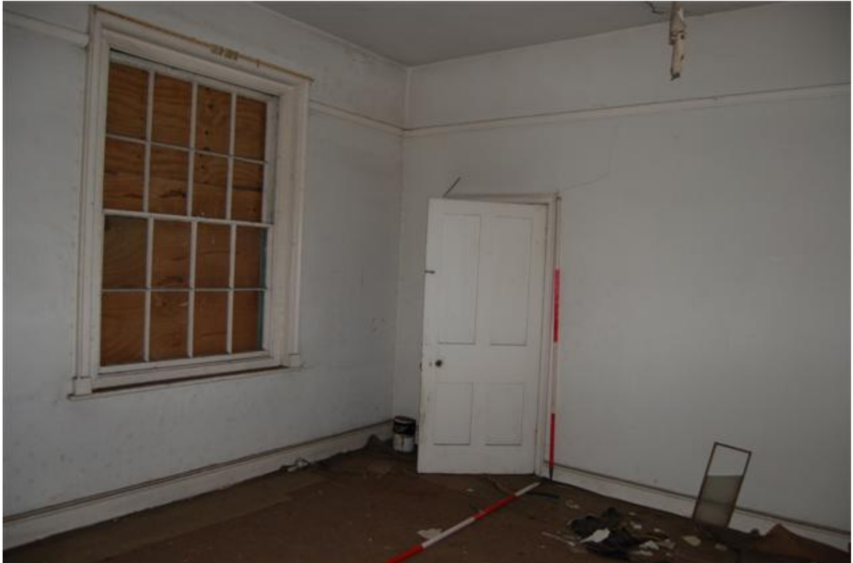
Plate 183: Building B, Block B5; Room BF16 looking north-east.
