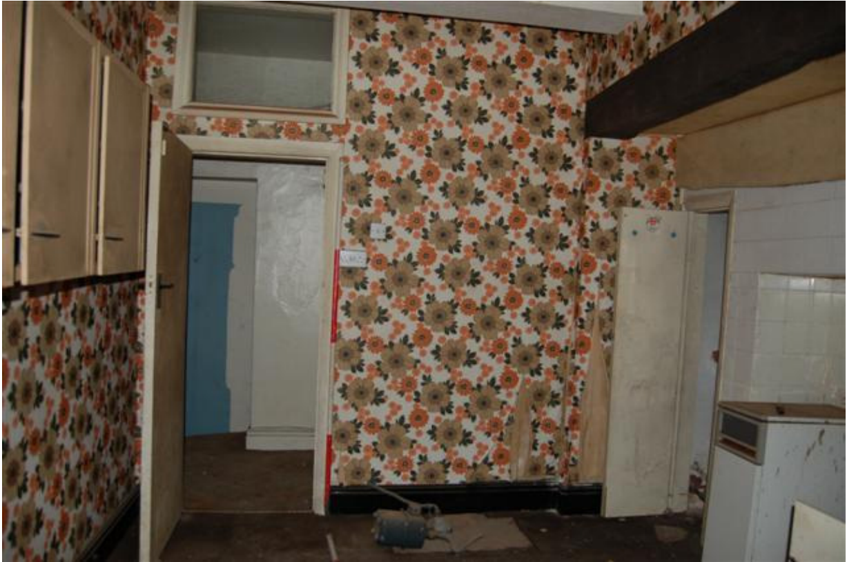
Plate 158: Building B, Block B3; Room BG14 looking east.
