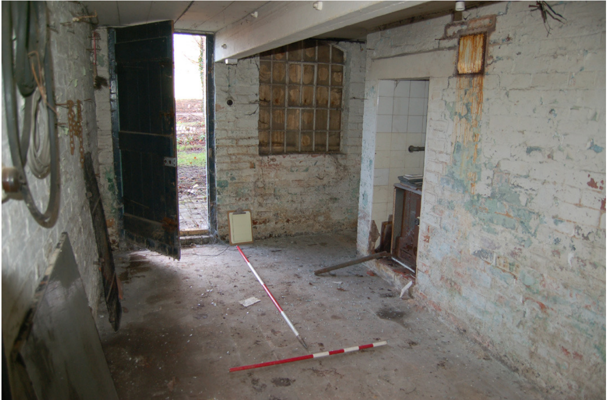
Plate 199: Building B, Block B7; Room BG21, looking north.
