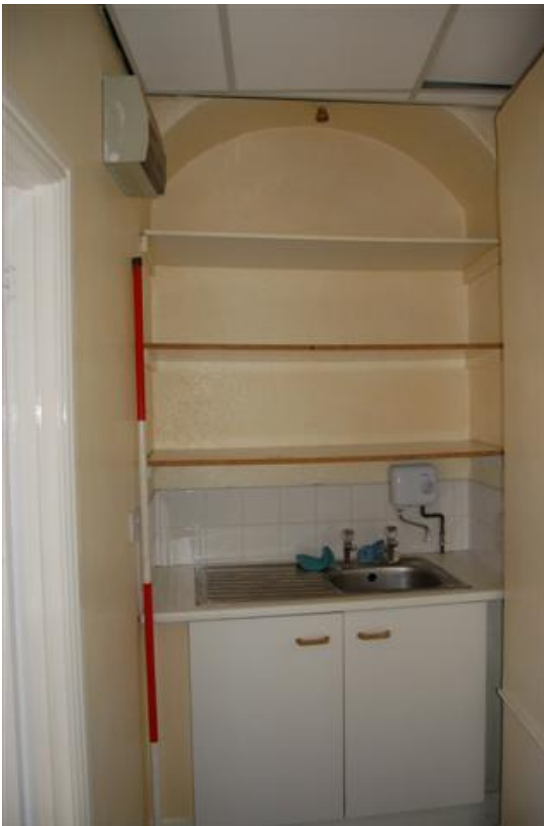
Plate 27: Building A, Block A3; Room AG5 (W), looking north.
