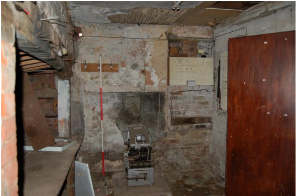
Plate 54: Building A, Block A4; Room AG9 looking north.
