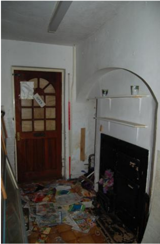
Plate 257: Bldg C, Block C2; Room CG8 range.
