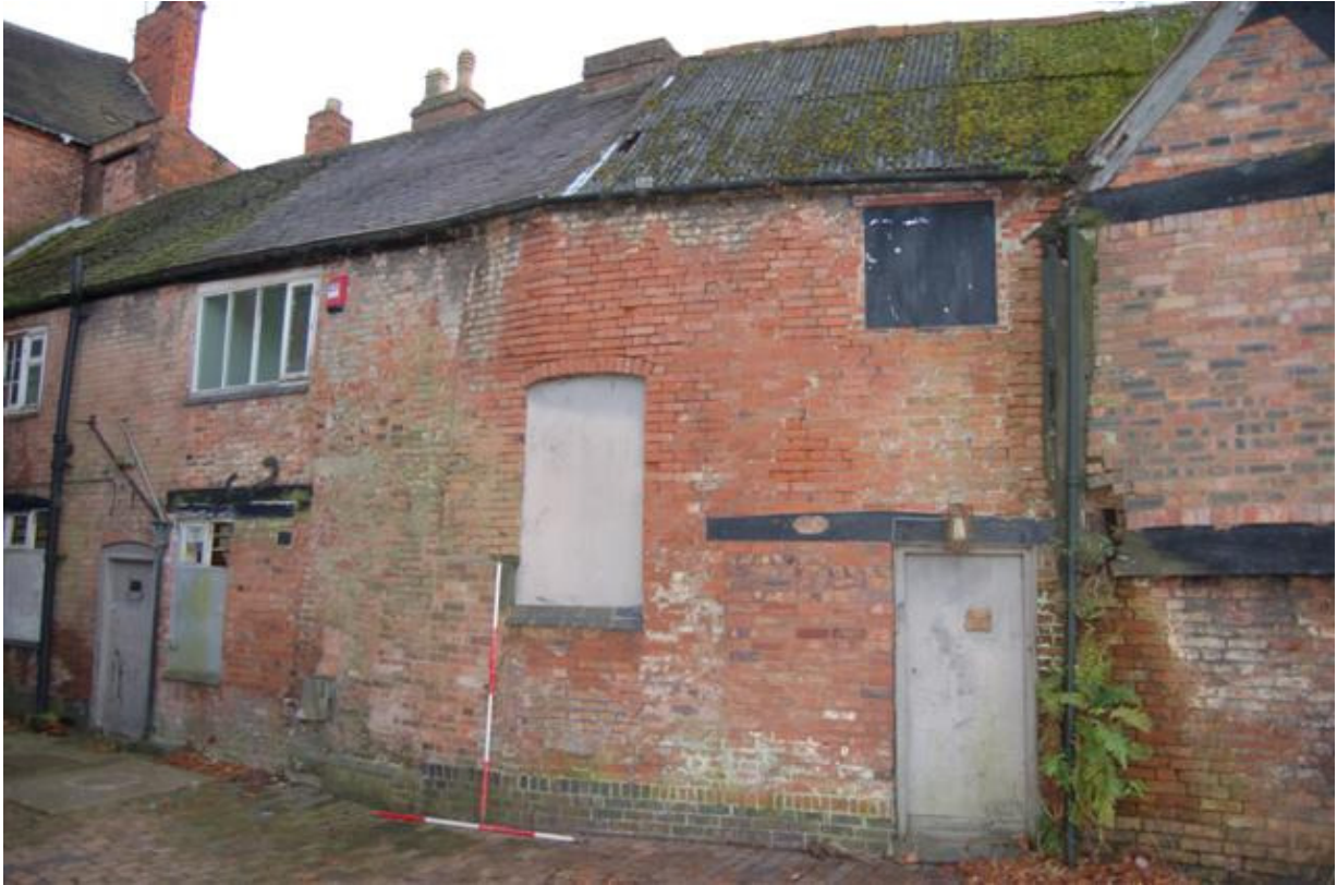
Plate 65: Building A north exterior Block A5.
