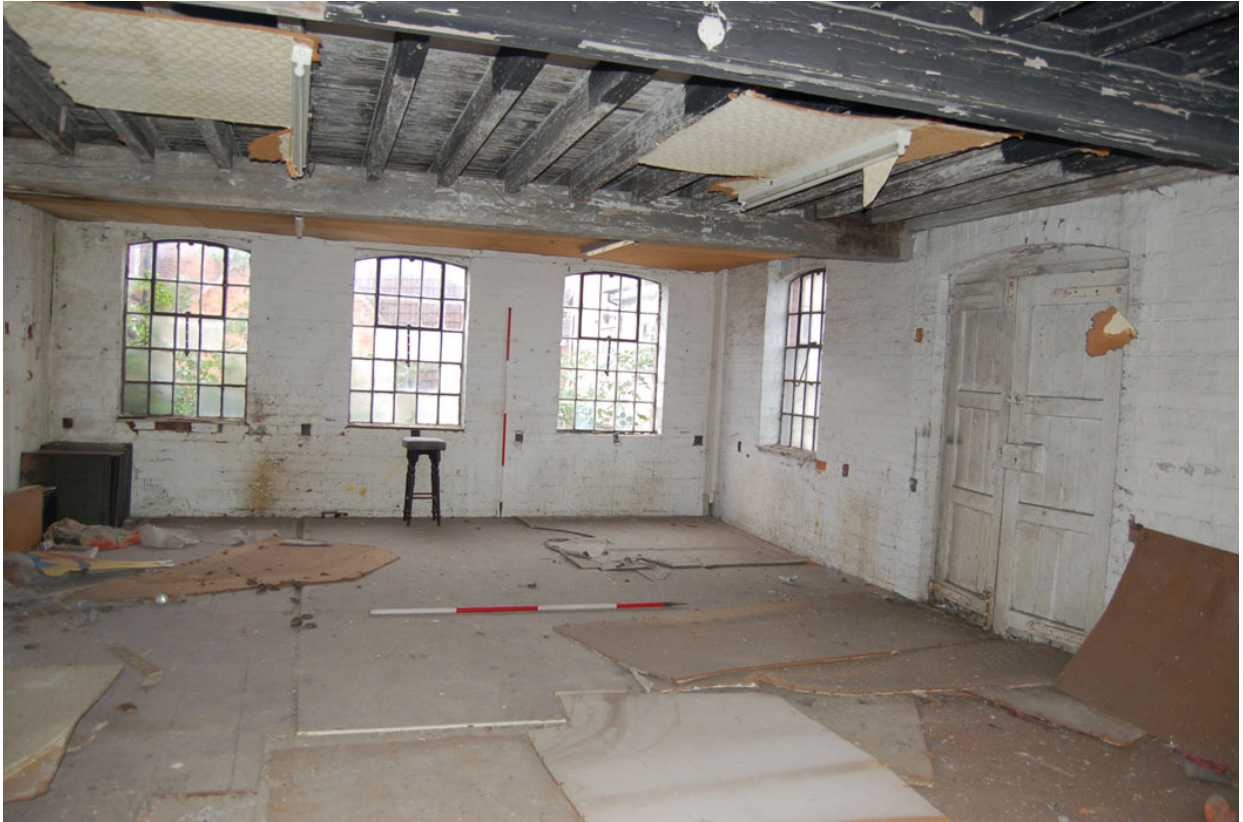
Plate 326: Building G, 1 st floor, looking south (note fixings for former work benches below windows).
