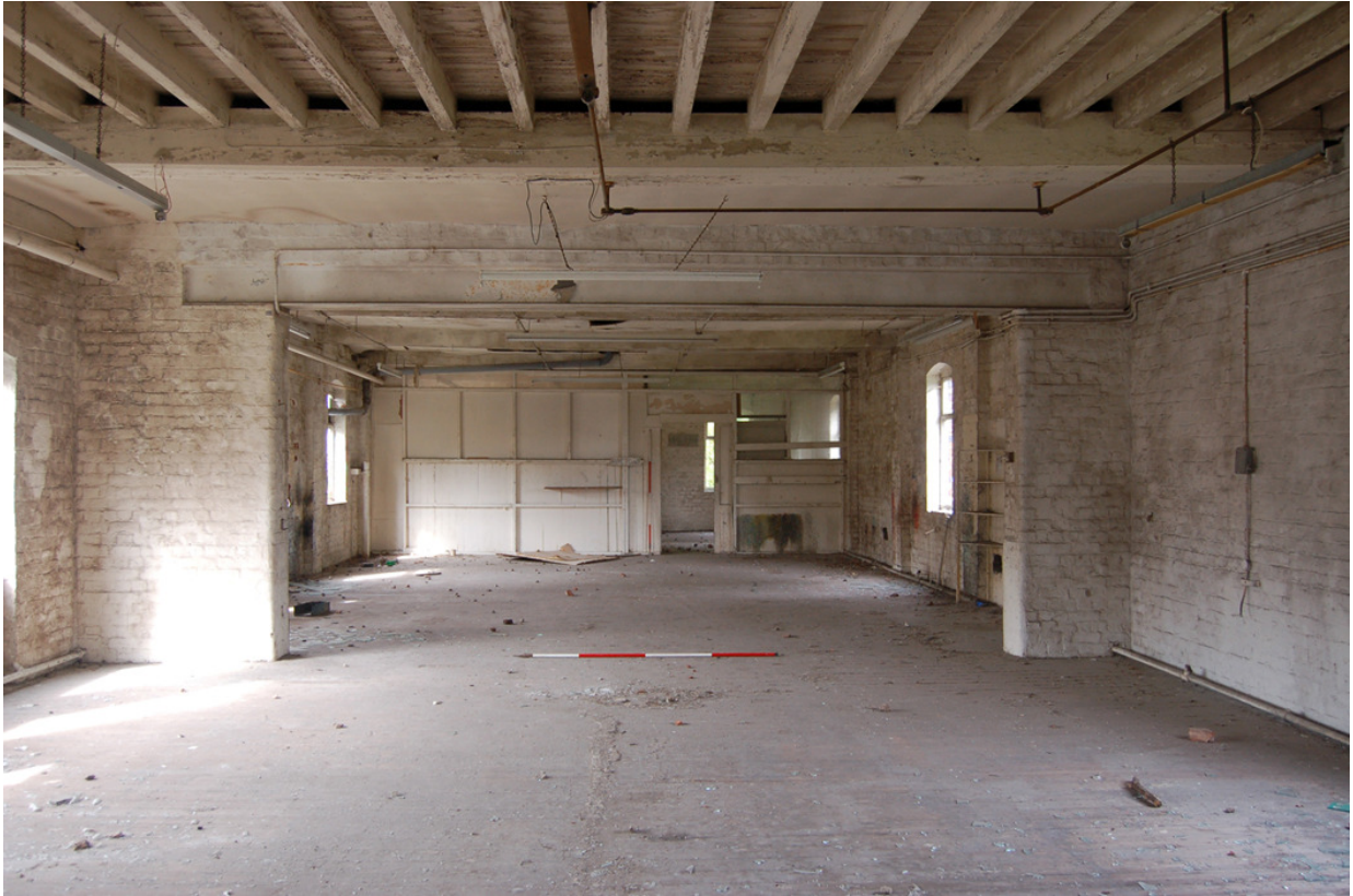
Plate 345: Building H, 1 st floor looking west.
