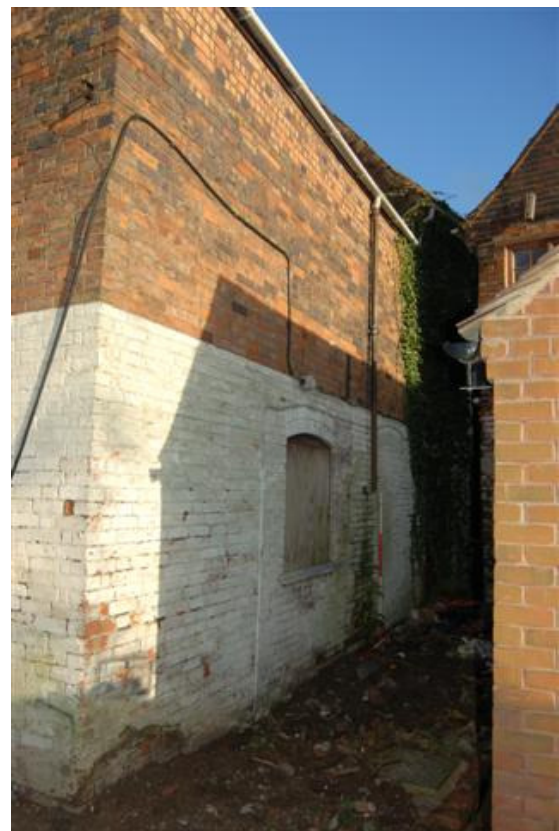
Plate 266: Bldg C, Block C3, south elevation.
