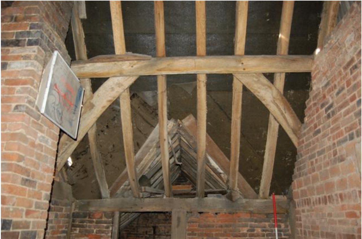
Plate 94: Building A, Block A6; Room AF14, roof structure looking west.
