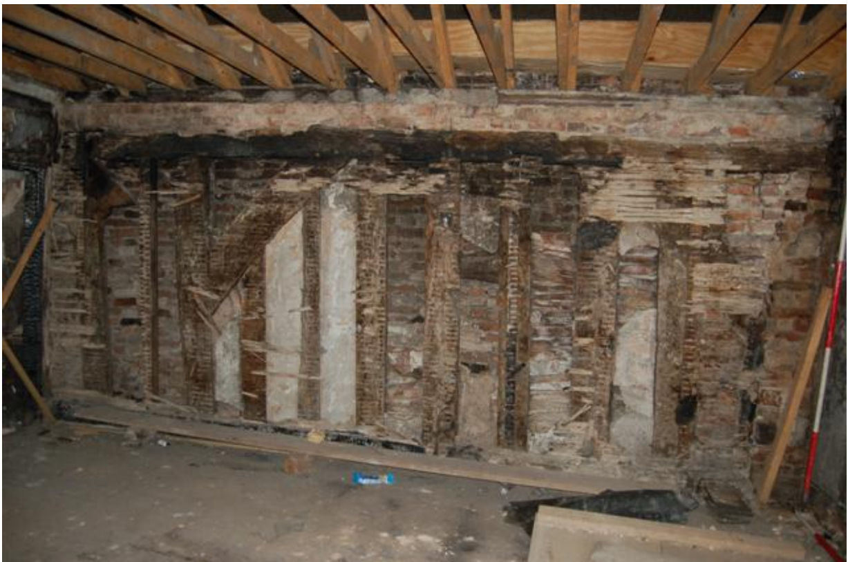
Plate 132: Building B, Block B1; Room BF1 north wall exposed framing.
