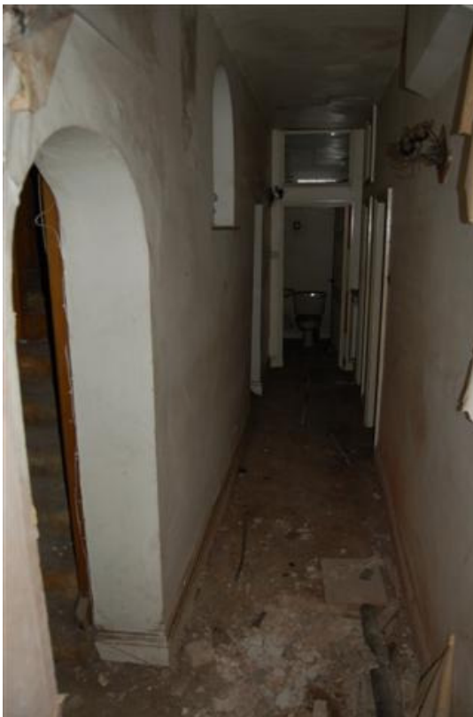
Plate 152: Bldg B, Block B3; Rm BG6 looking S.
