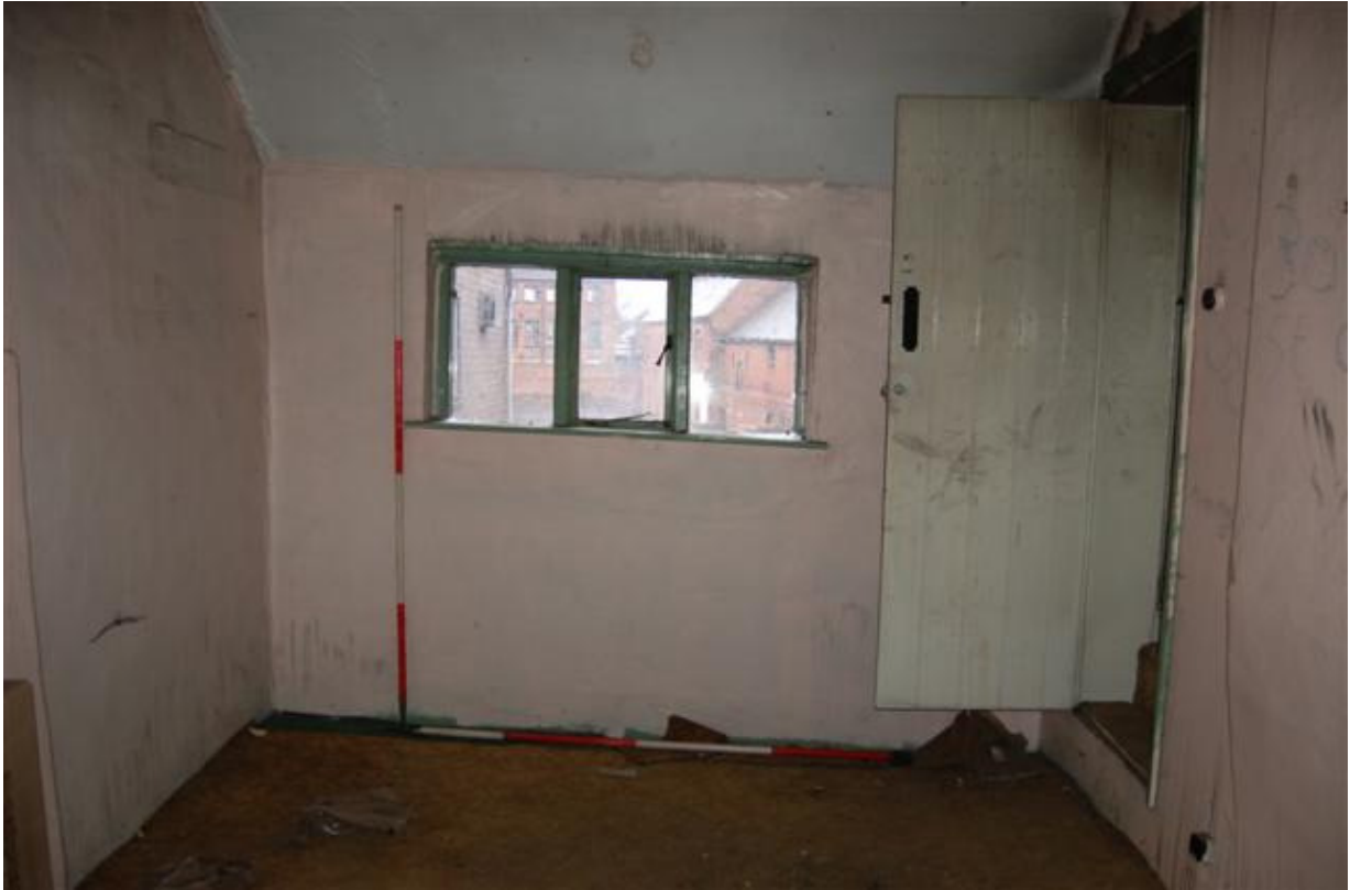
Plate 148: Building B, Block B2; Room BF4 looking west.
