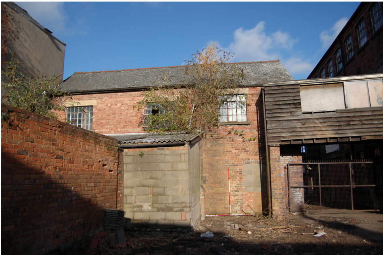
Plate 311: Building F, south elevation.
