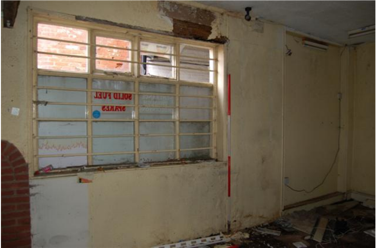
Plate 49: Building A, Block A4; Room AG7 looking north.
