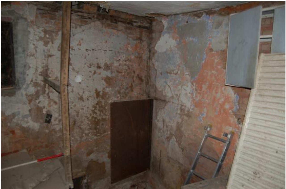
Plate 70: Building A, Block A5; Room AF13 looking north-east.
