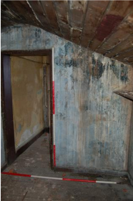
Plate 32: Bldg. A, Block A8; Room AF6 looking E.
