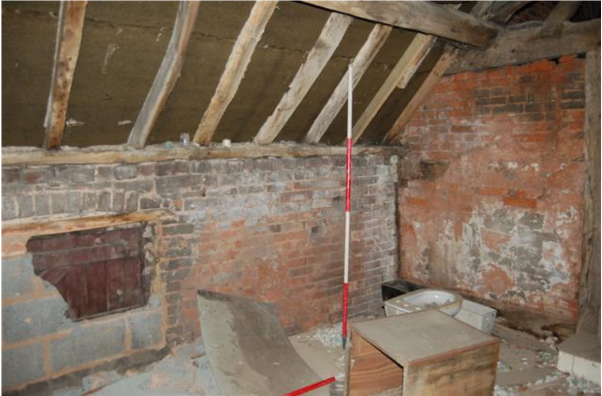
Plate 105: Building A, Block A7; Room AF15 looking north-east.
