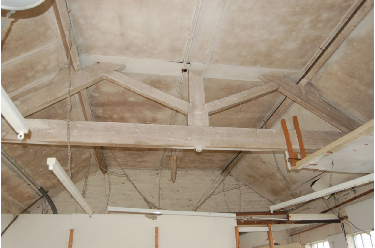
Plate 321: Building F 1 st floor, detail of King-post roof truss.
