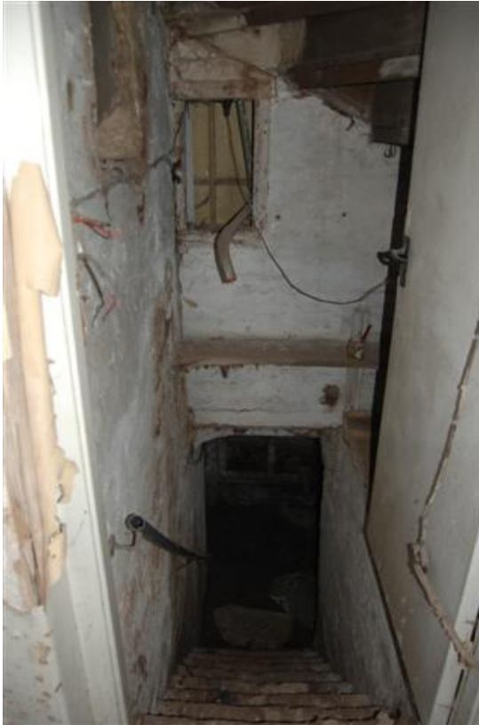
Plate 168: Bldg B, Block B4; Rm BG3 looking S (cellar)
