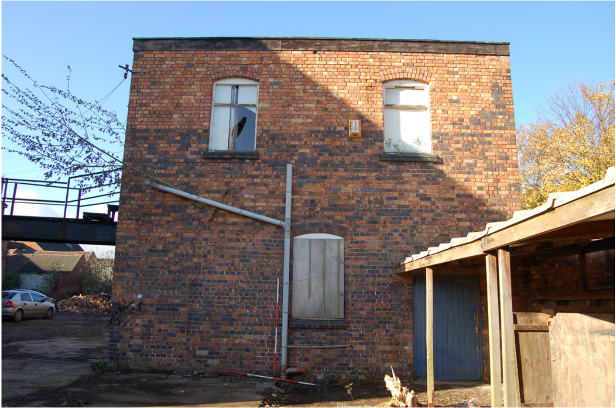
Plate 338: Building H, east elevation.
