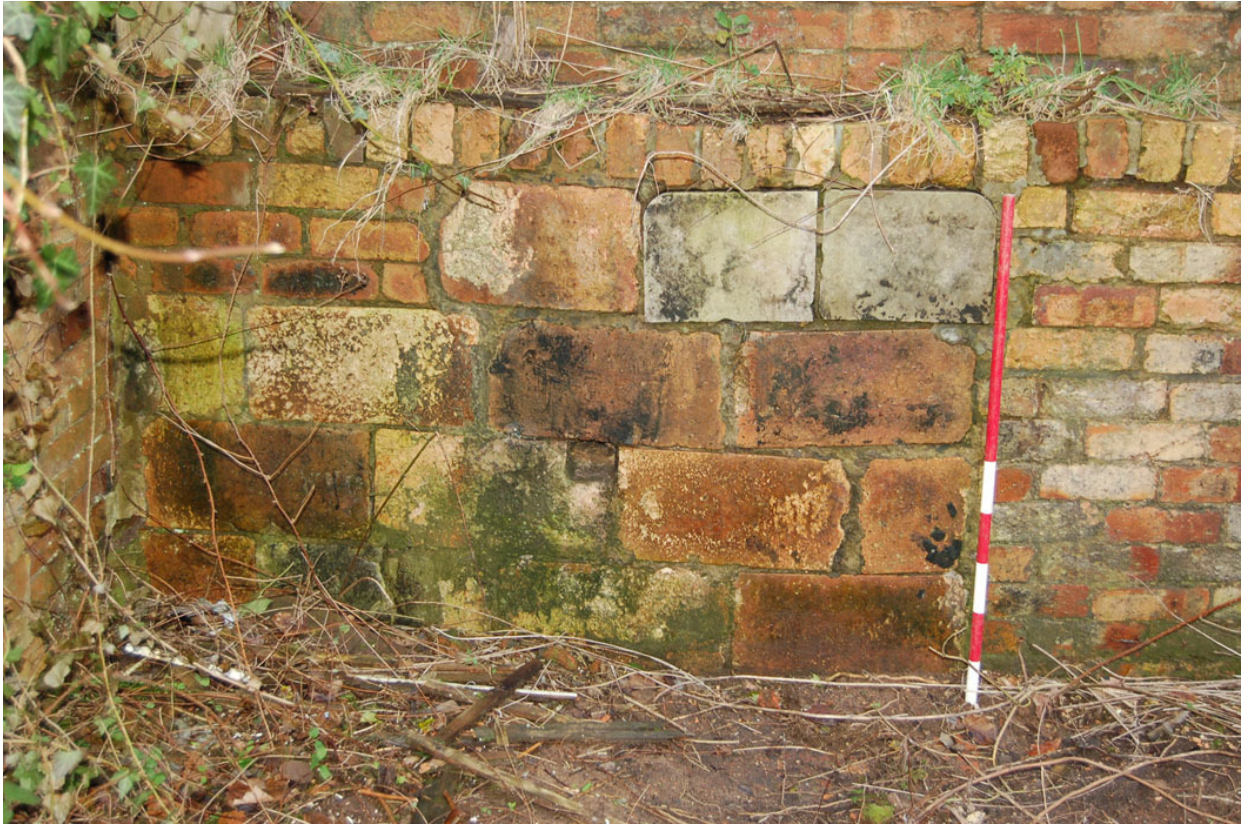
Plate 294: Boundary wall (south section); detail of ashlar masonry.
