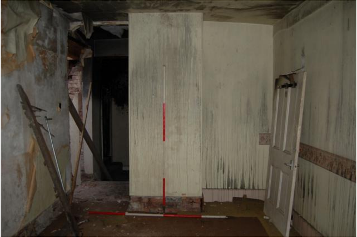
Plate 165: Building B, Block B3; Room BF12 looking east.
