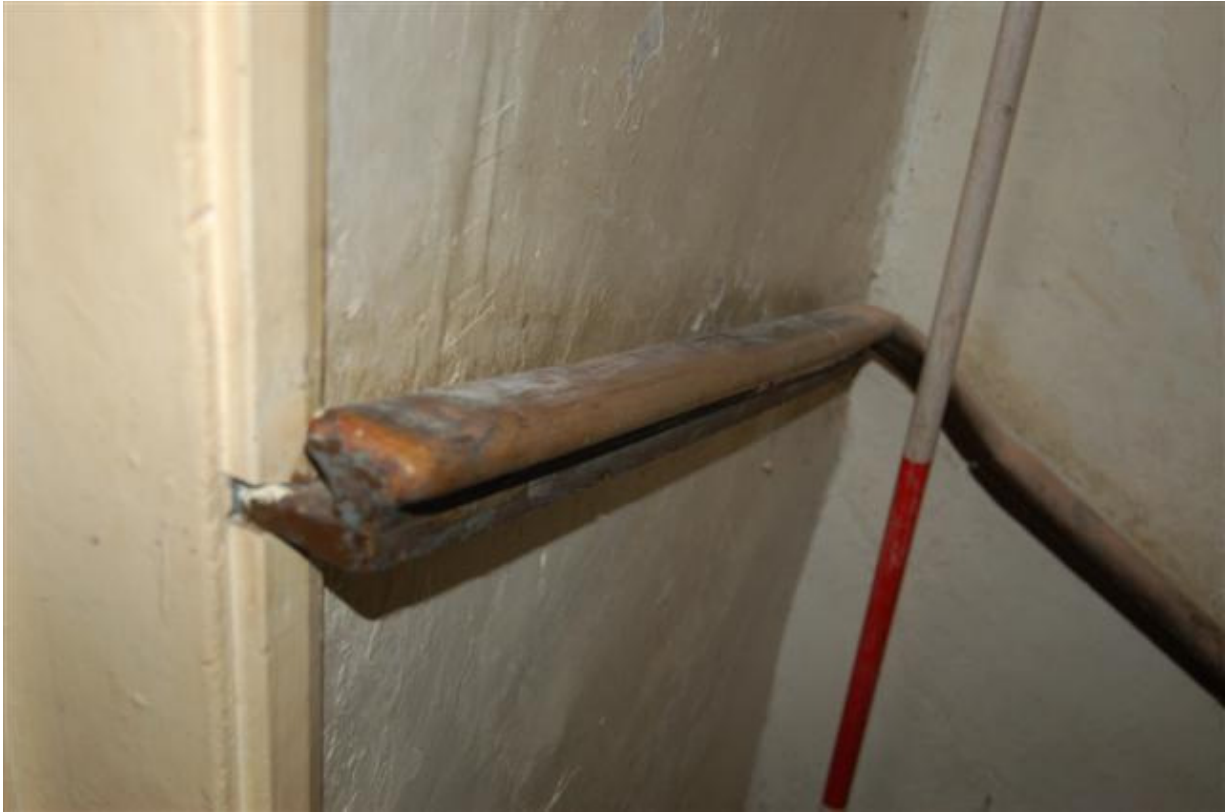
Plate 228: Building C, Block C1; Stair CG7/CF9 detail of handrail.
