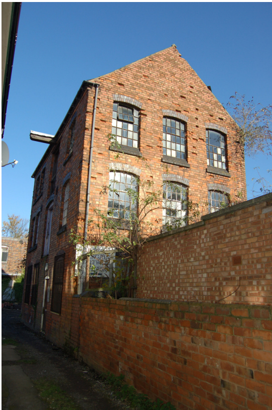
Plate 322: Building G, exterior looking north.
