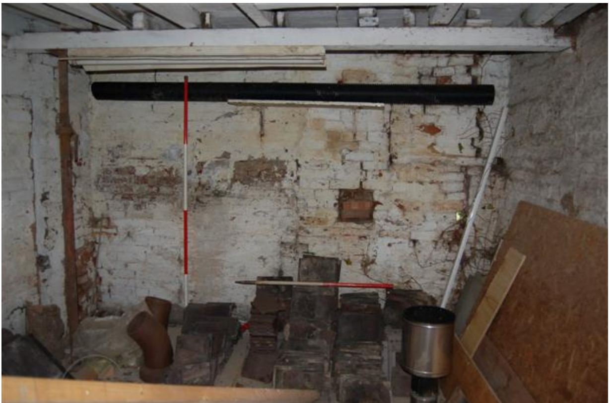
Plate 102: Building A, Block A7; Room AG14 looking west.
