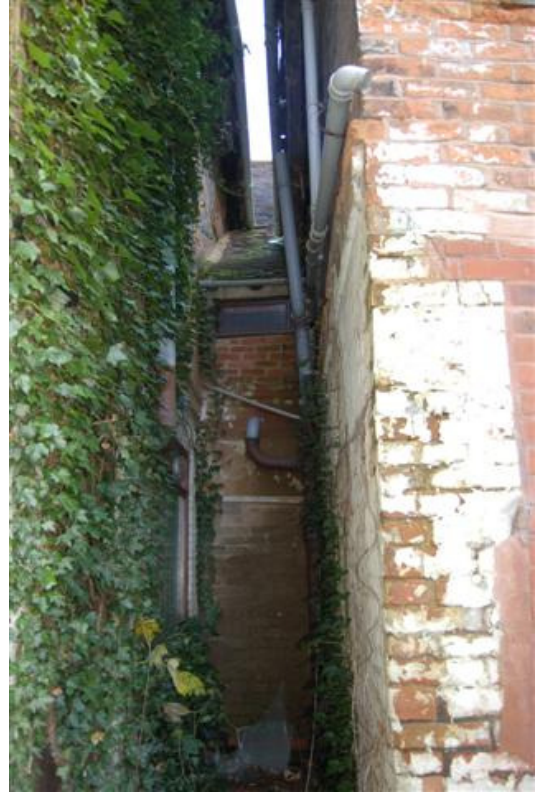
Plate 272: Gap between Blocks C5 (r.) and C2 (l.).
