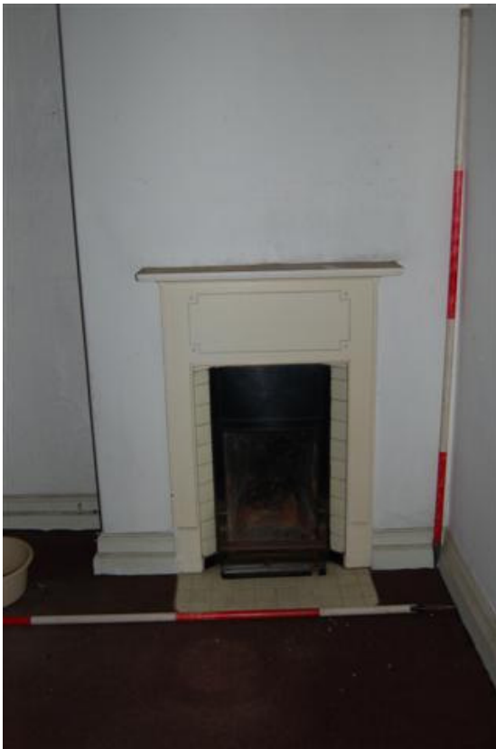
Plate 20: Bldg A, Block A2; Room AF4 fireplace.
