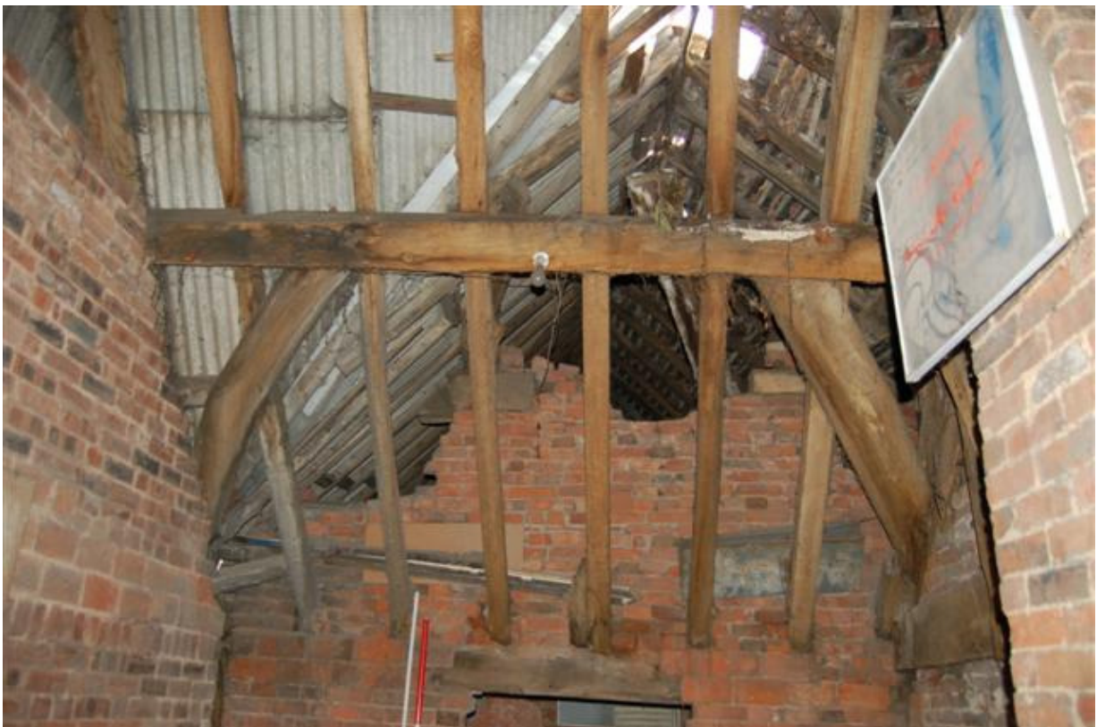
Plate 89: Building A, Block A6; Room AF14, roof structure looking east.
