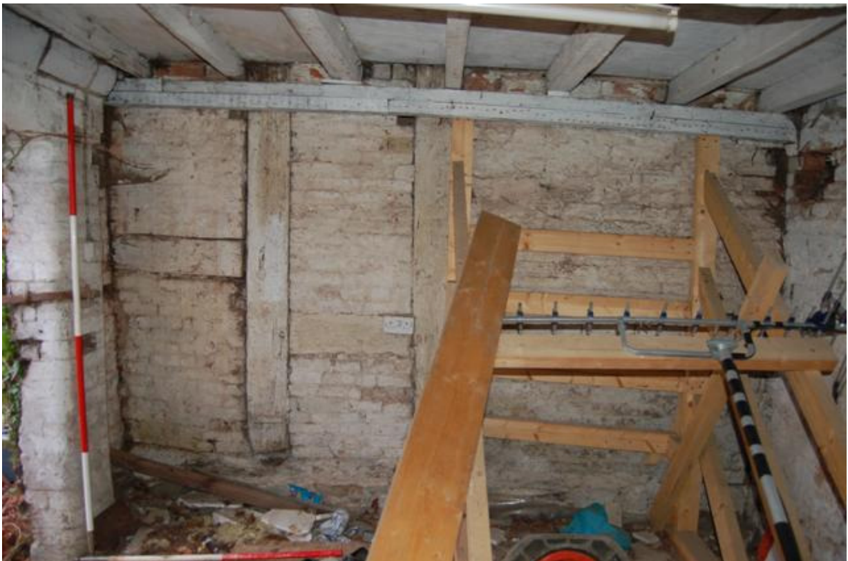
Plate 100: Building A, Block A7; Room AG14 looking east.
