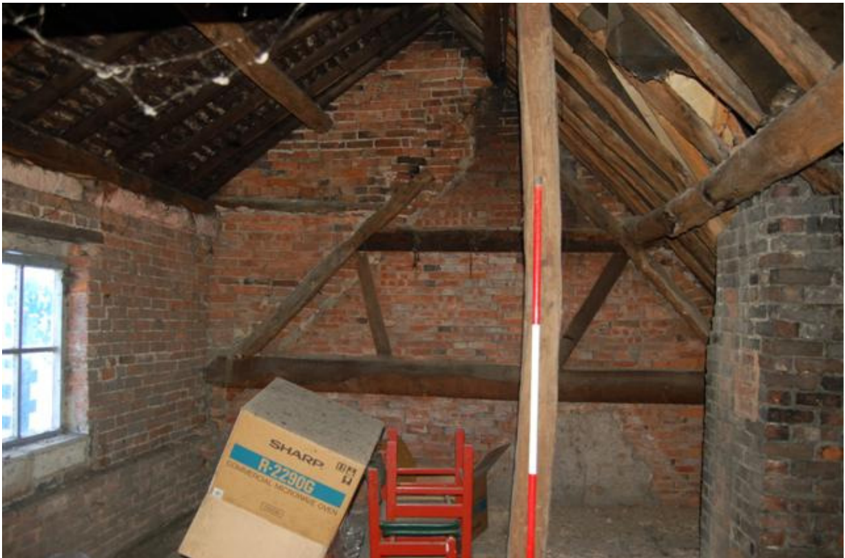
Plate 252: Building C, Block C1; Room CS2 roof structure looking south.
