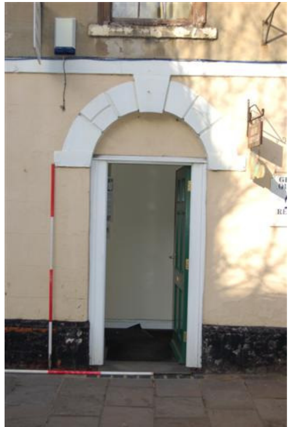
Plate 221: Building C, door detail.
