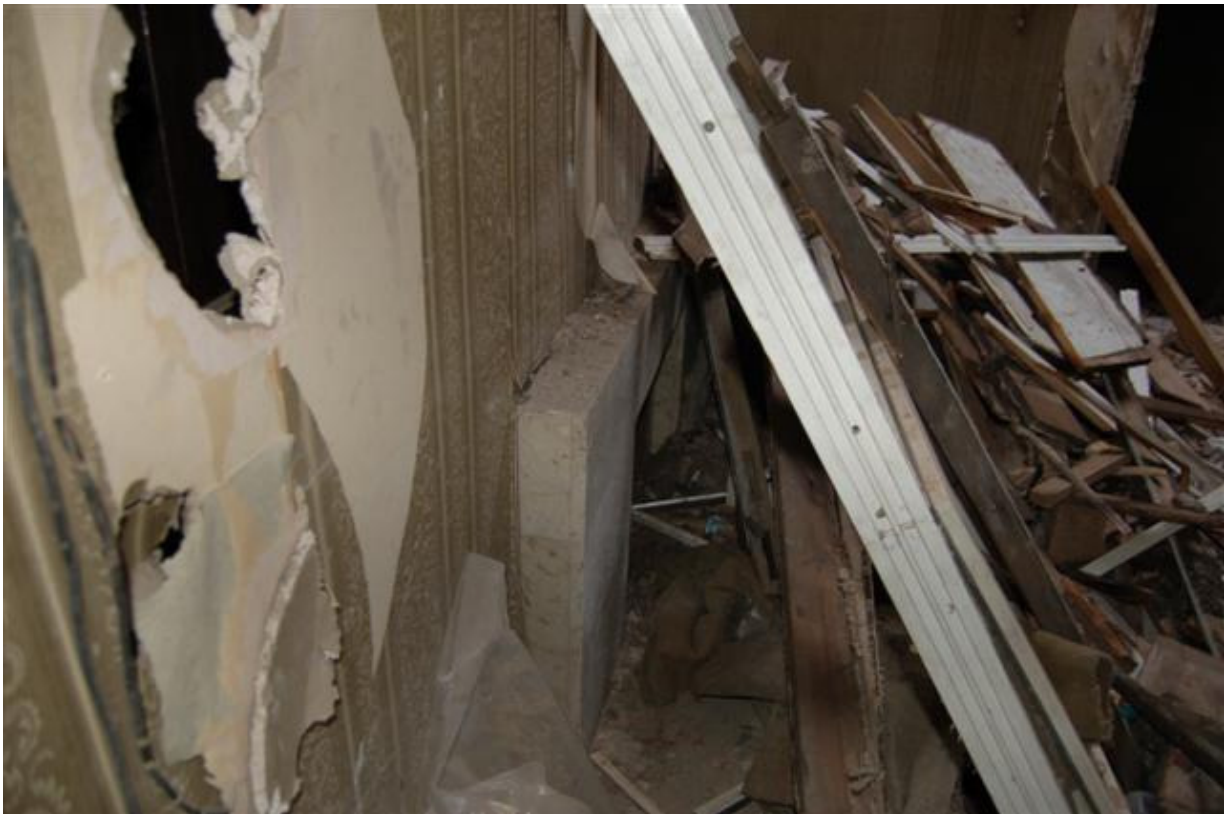
Plate 123: Building B, Block B1; Room BG2 fireplace.
