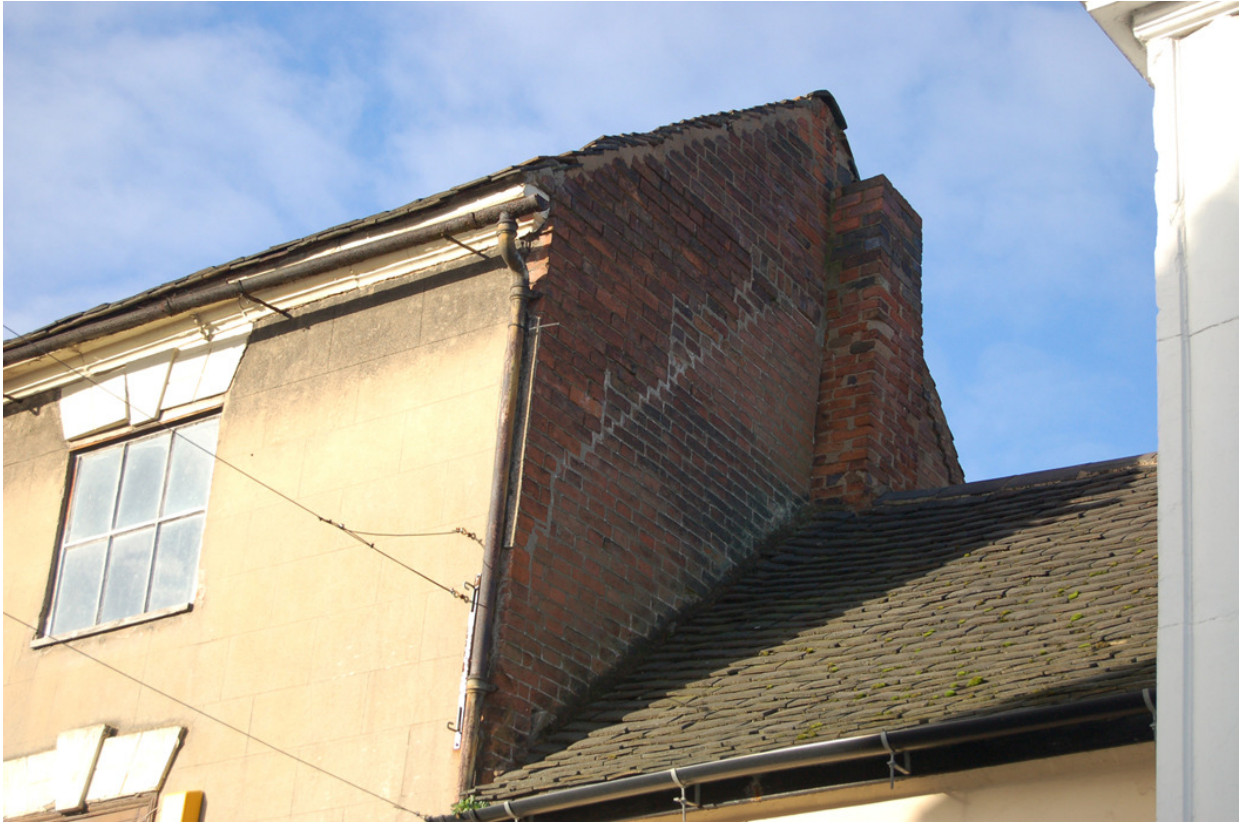
Plate 219: Building C, north elevation; detail of raised brickwork.
