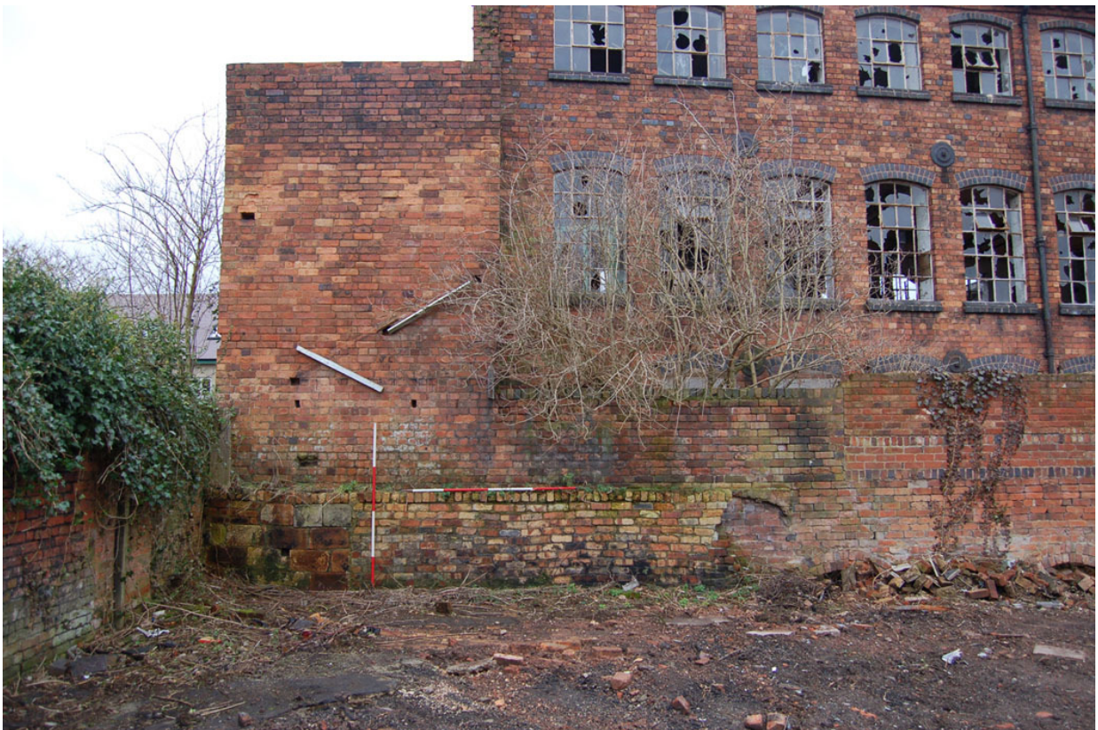
Plate 293: Boundary wall (south section) looking west, Building E beyond.
