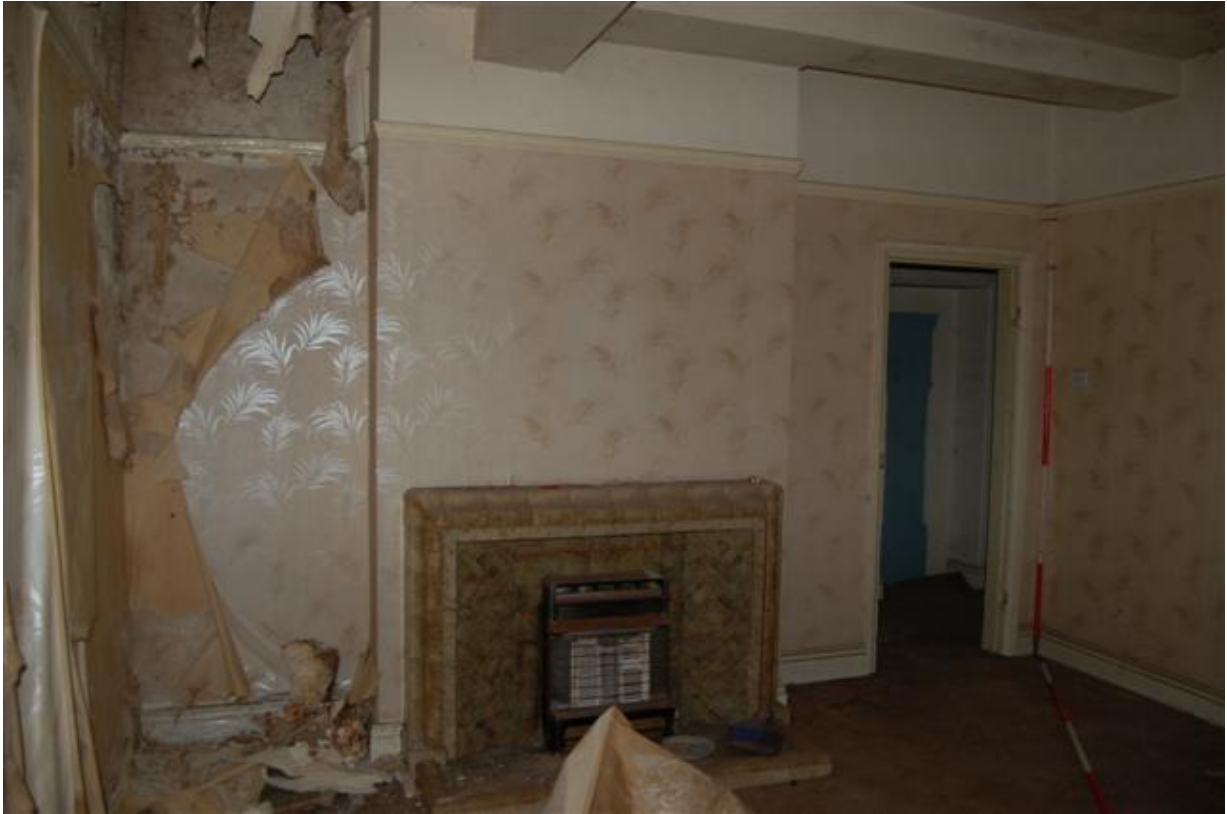
Plate 156: Building B, Block B3; Room BG13 looking east.
