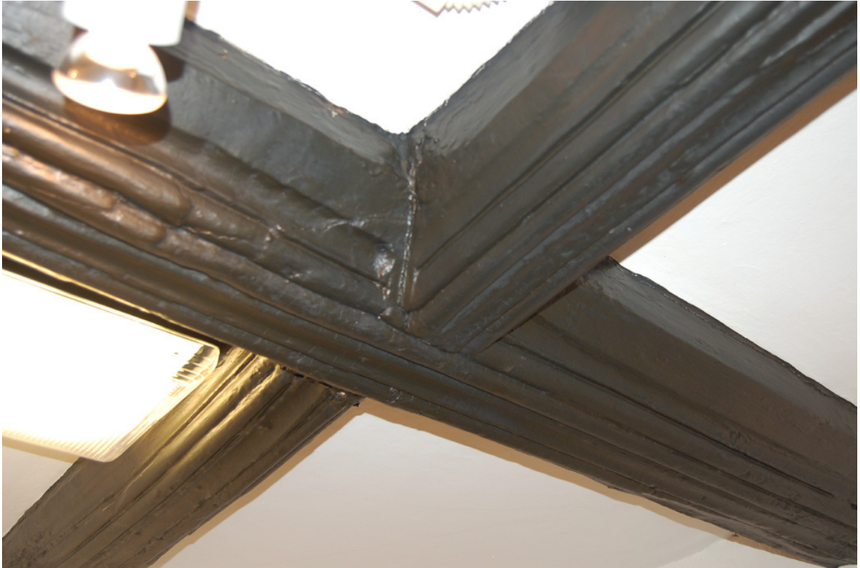
Plate 111: Building B, Block B1; Room BG12 detail of moulded ceiling beams.
