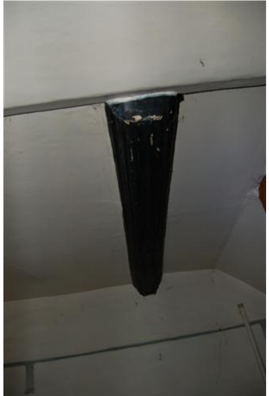
Plate 125: Room BG5, moulded ceiling beam.
