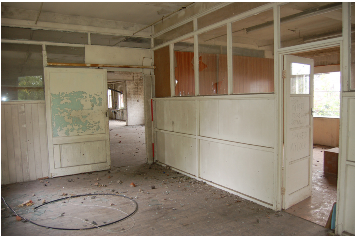
Plate 346: Building H, 1 st floor; inserted studwork walls at Bays 8/9.
