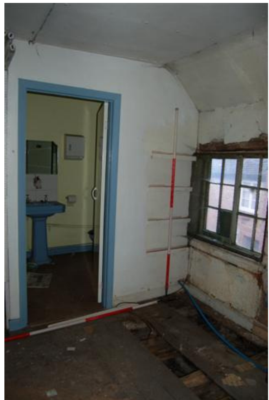
Plate 64: Bldg.A, Block A4; Rm AF8 looking W.
