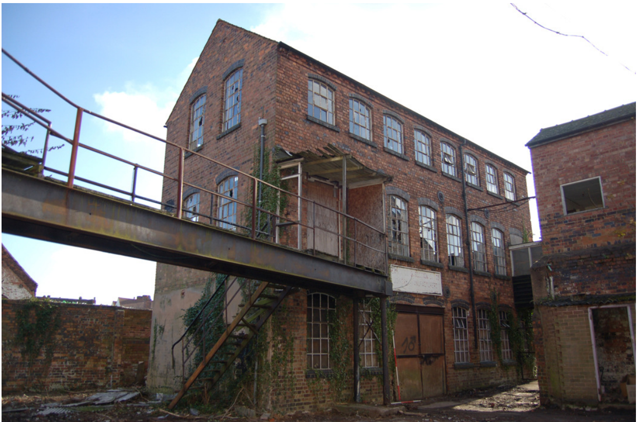
Plate 302: Building E, west elevation, oblique view. Note raised 1 st floor access to building H (left).
