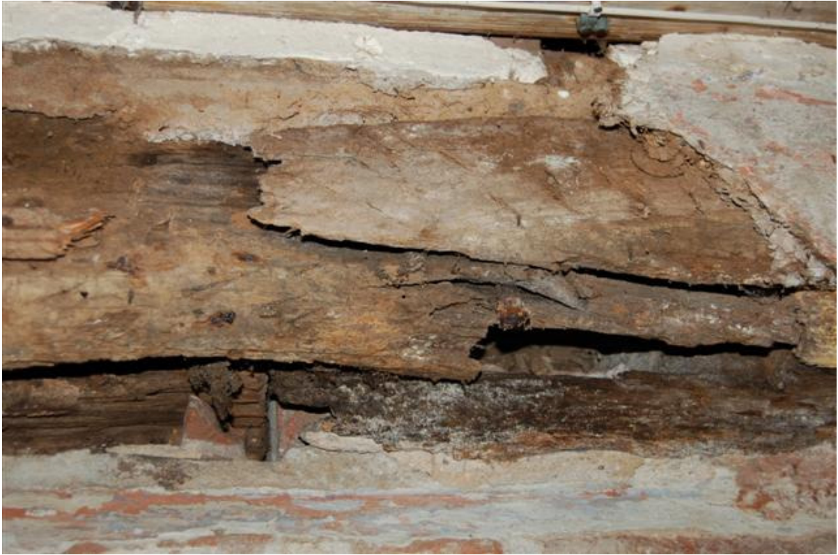
Plate 69: Building A, Block A5; Room AG11, detail of mortise holes.
