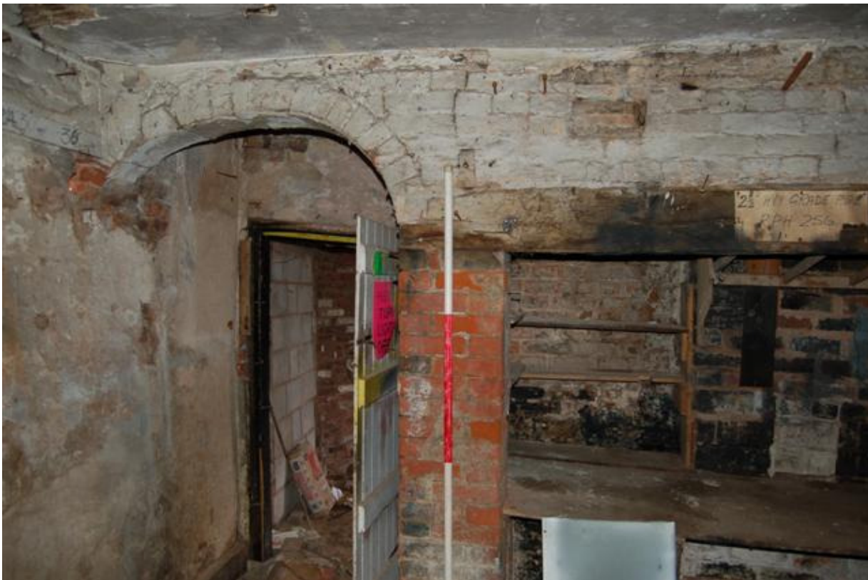
Plate 55: Building A, Block A4; Room AG9, doorway to AG10-12.
