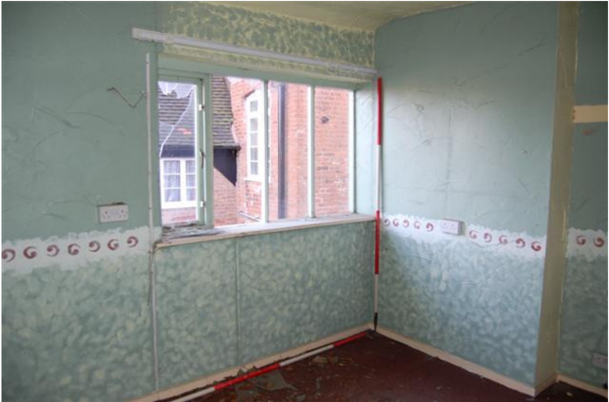
Plate 62: Building A, Block A4; Room AF12 looking north-east.
