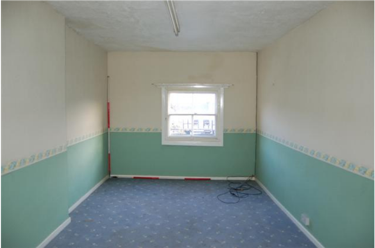
Plate 41: Building A, Block A3; Room AS5 looking east.
