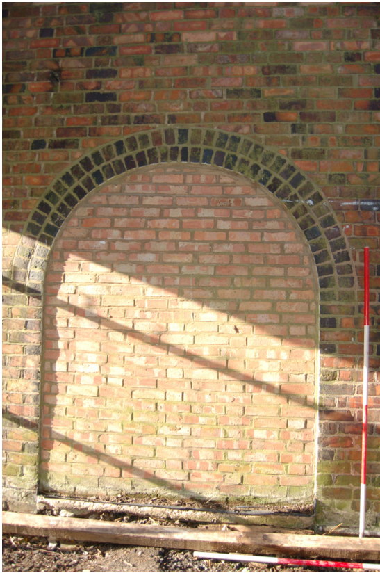
Plate 314: Building F, east elevation; door.
