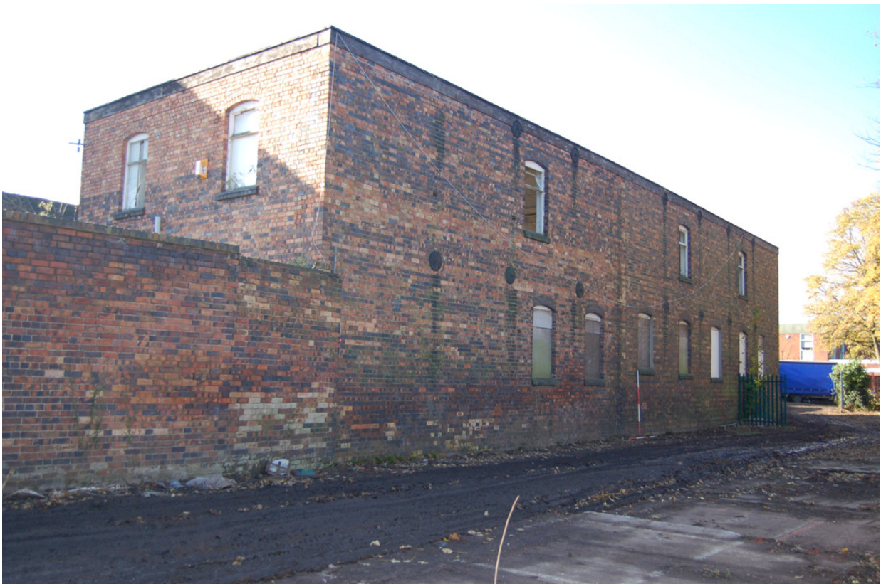
Plate 337: Building H, north elevation.
