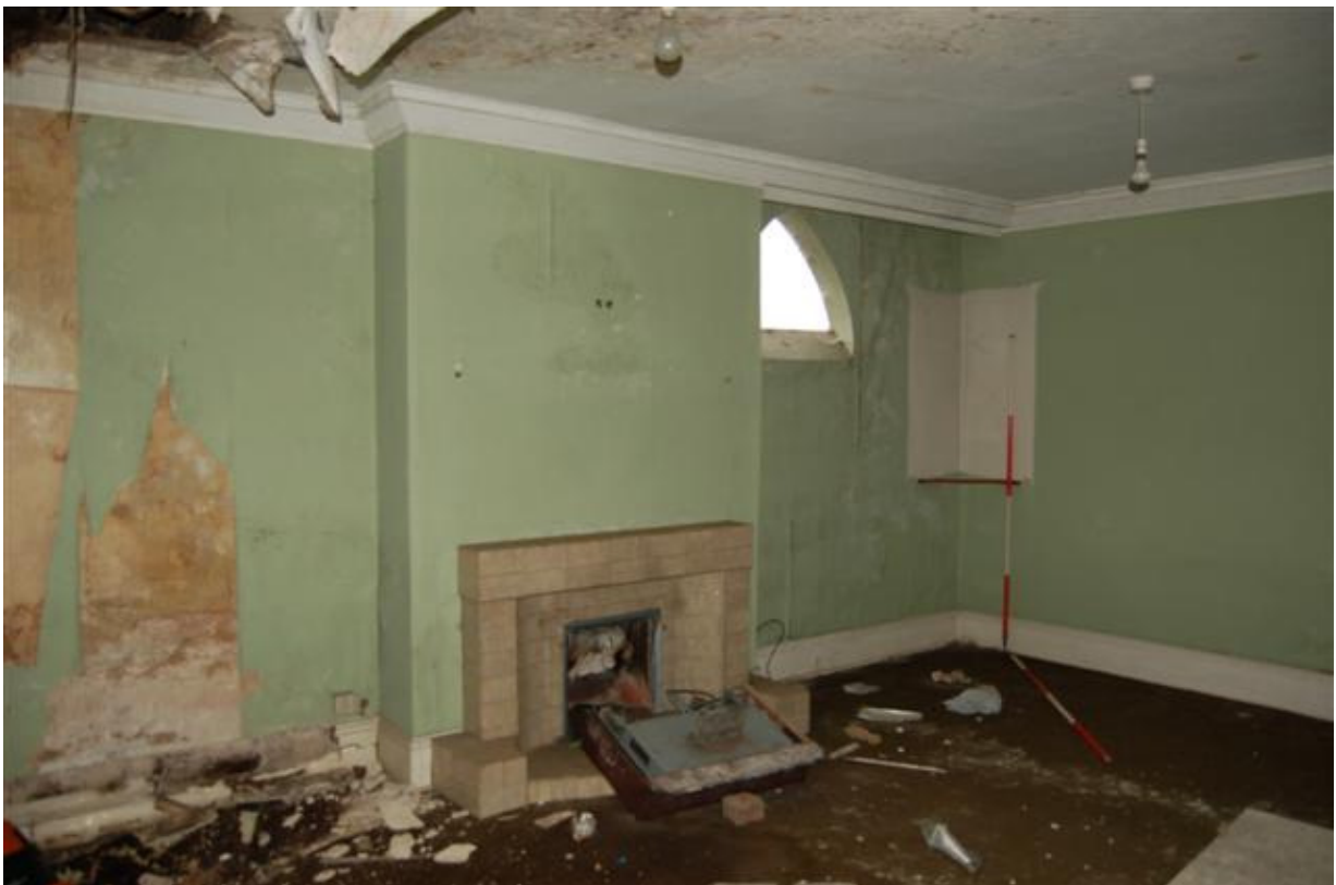
Plate 180: Building B, Block B5; Room BG16 looking south-west..
