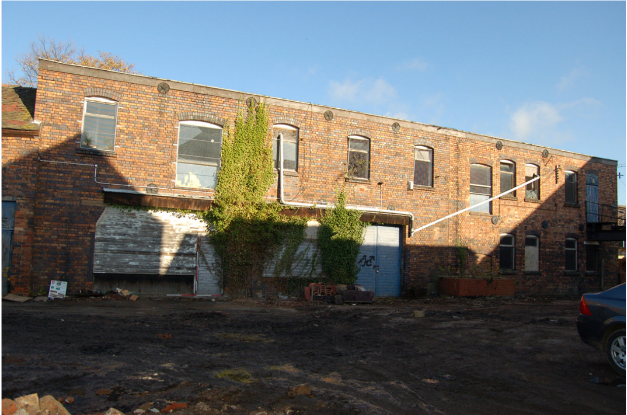
Plate 330: Building H, south elevation (oblique).
