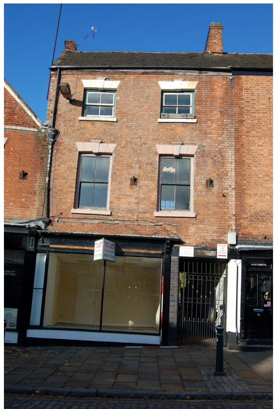
Plate 21: Building A Block A3; exterior (east).
