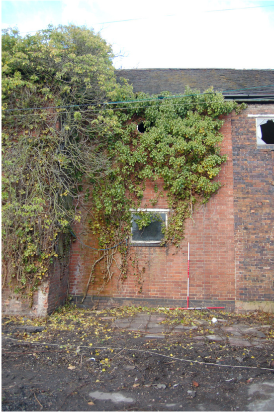
Plate 185: Building B Block B6; exterior south elevation.
