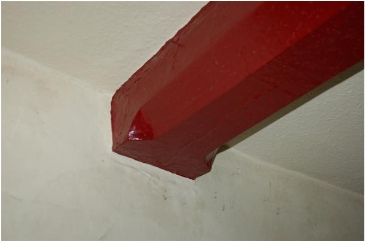
Plate 239: Building C, Block C1; Room CF3 detail of ceiling beam..
