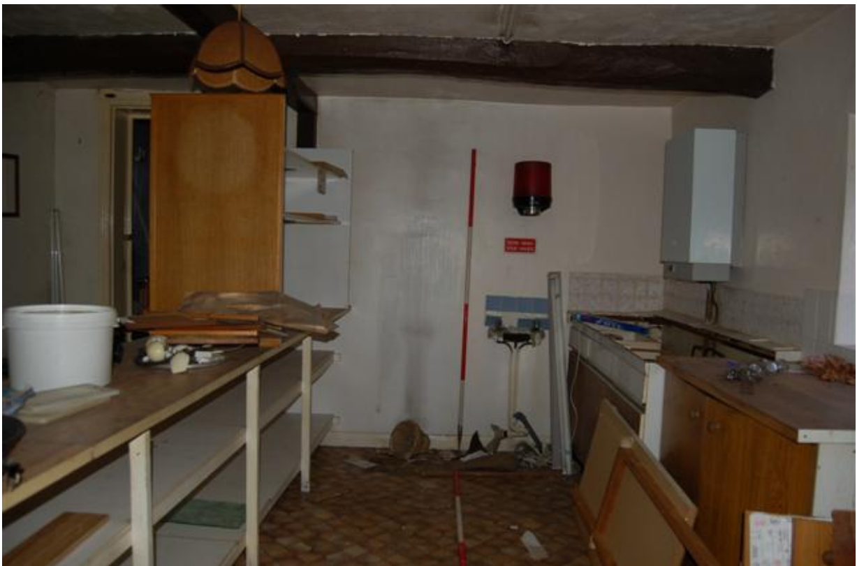
Plate 263: Building C, Block C2; Room CF11 looking west.
