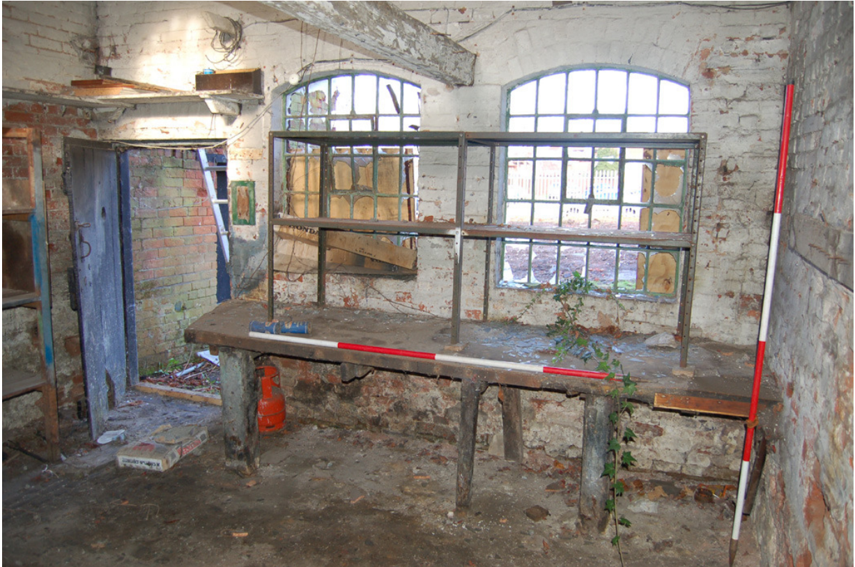
Plate 213: Building B, Block B7; Room BG25, north wall.
