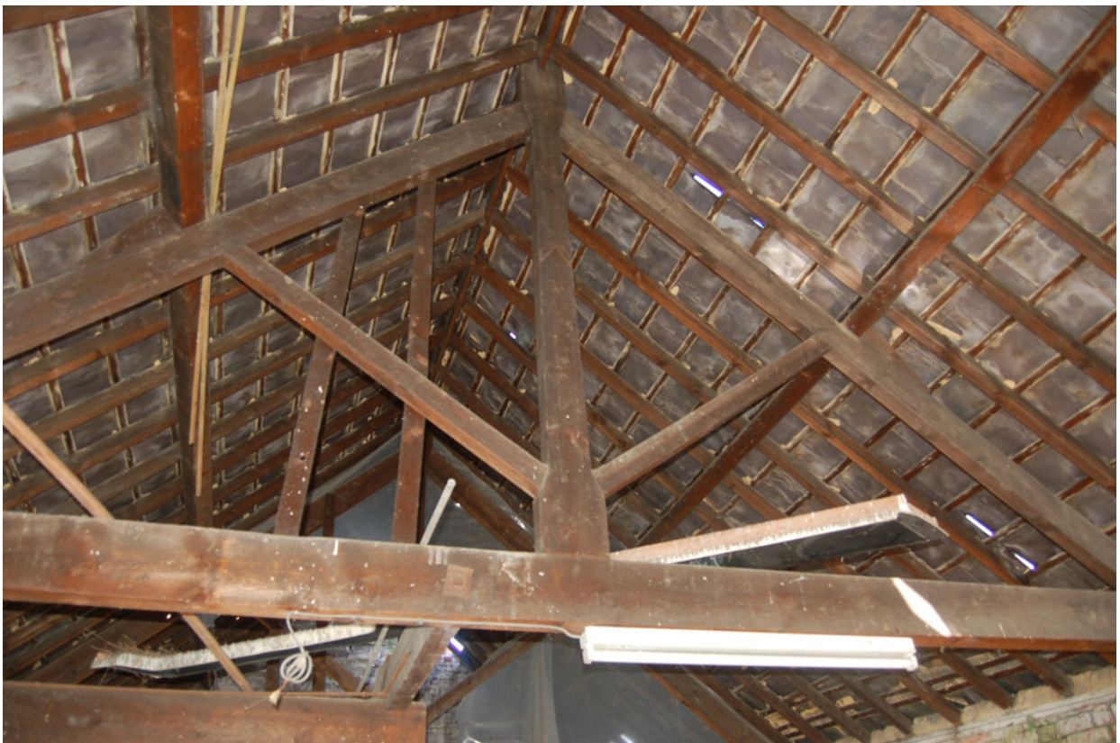
Plate 329: Building G, 2 nd floor, detail of King-post roof.
