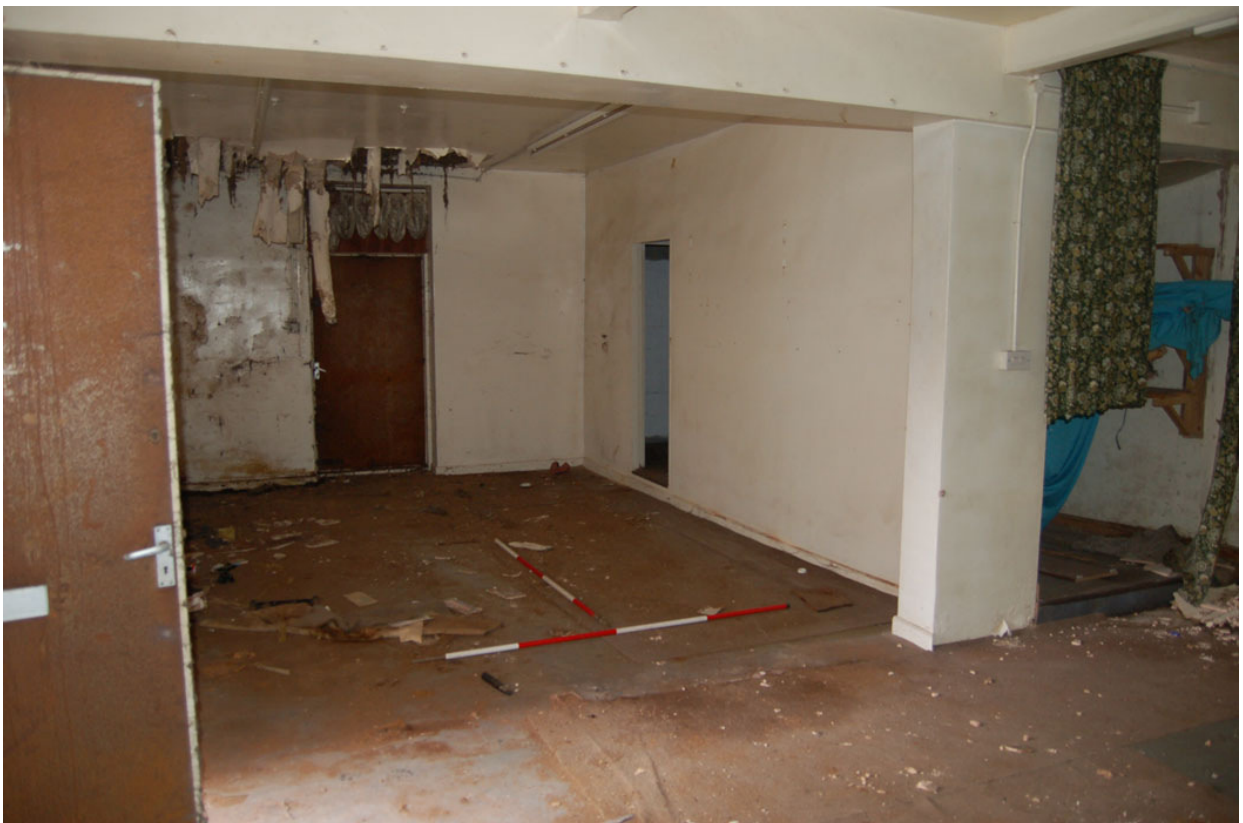
Plate 325: Building G, ground floor looking north.
