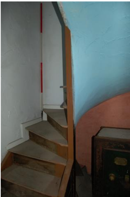
Plate 56: Bldg A Block A5; Room AF7 stair detail.
