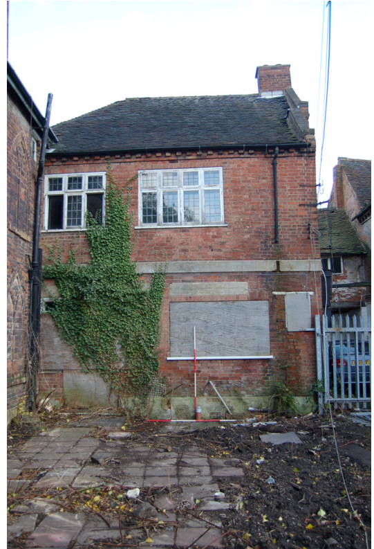
Plate 151: Building B (No.14) Block B3, W elev.
