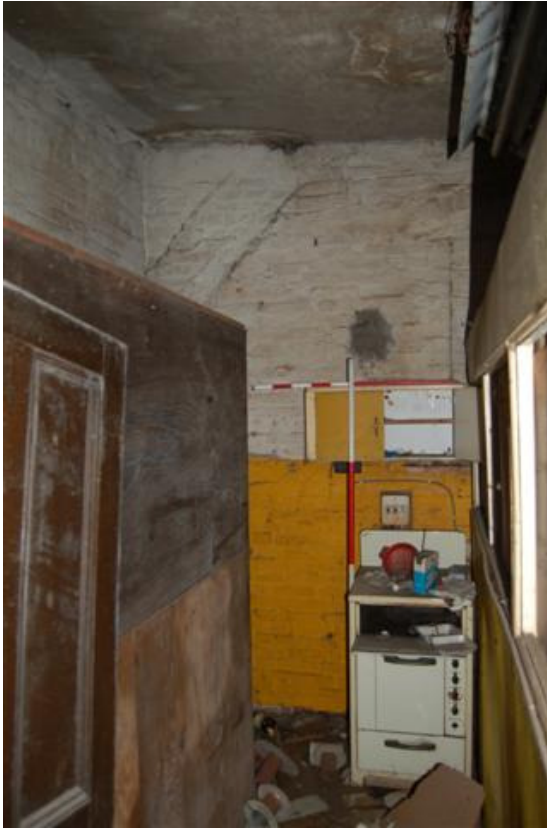
Plate 284: Building D, Room D6 looking east.
