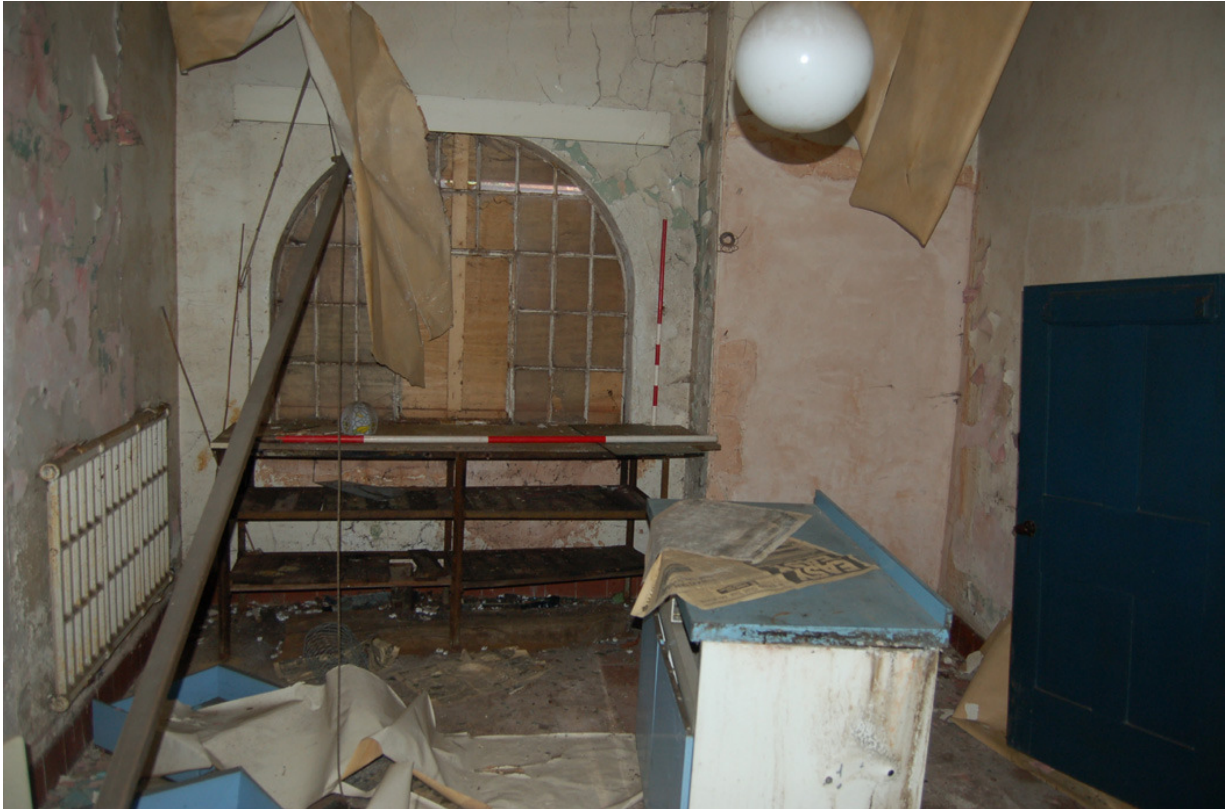
Plate 201: Building B, Block B7; Room BG20, looking north.
