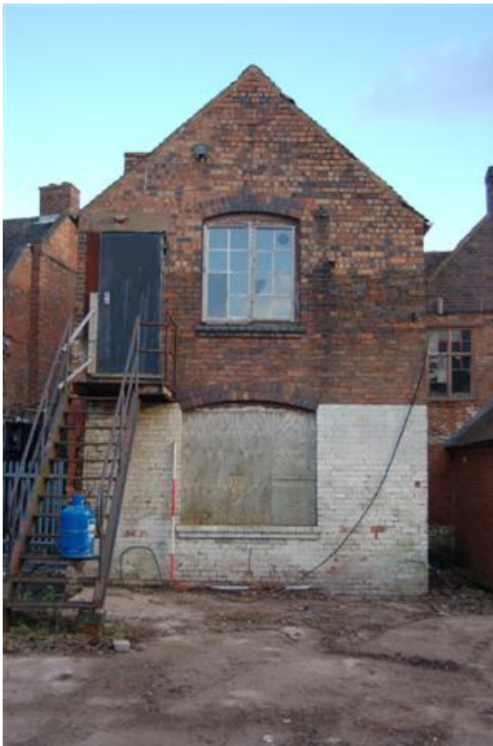
Plate 265: Bldg C, Block C3, west elevation.
