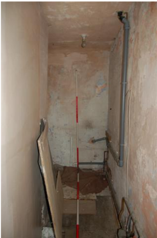
Plate 60: Bldg.A, Block A4; Rm AF10 looking N.
