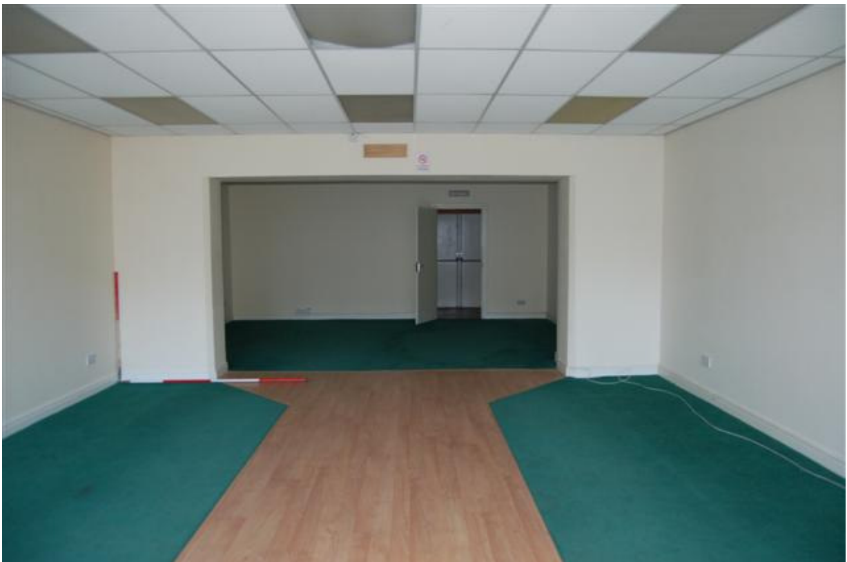
Plate 7: Building A, Block A1; Room AG1, looking west.
