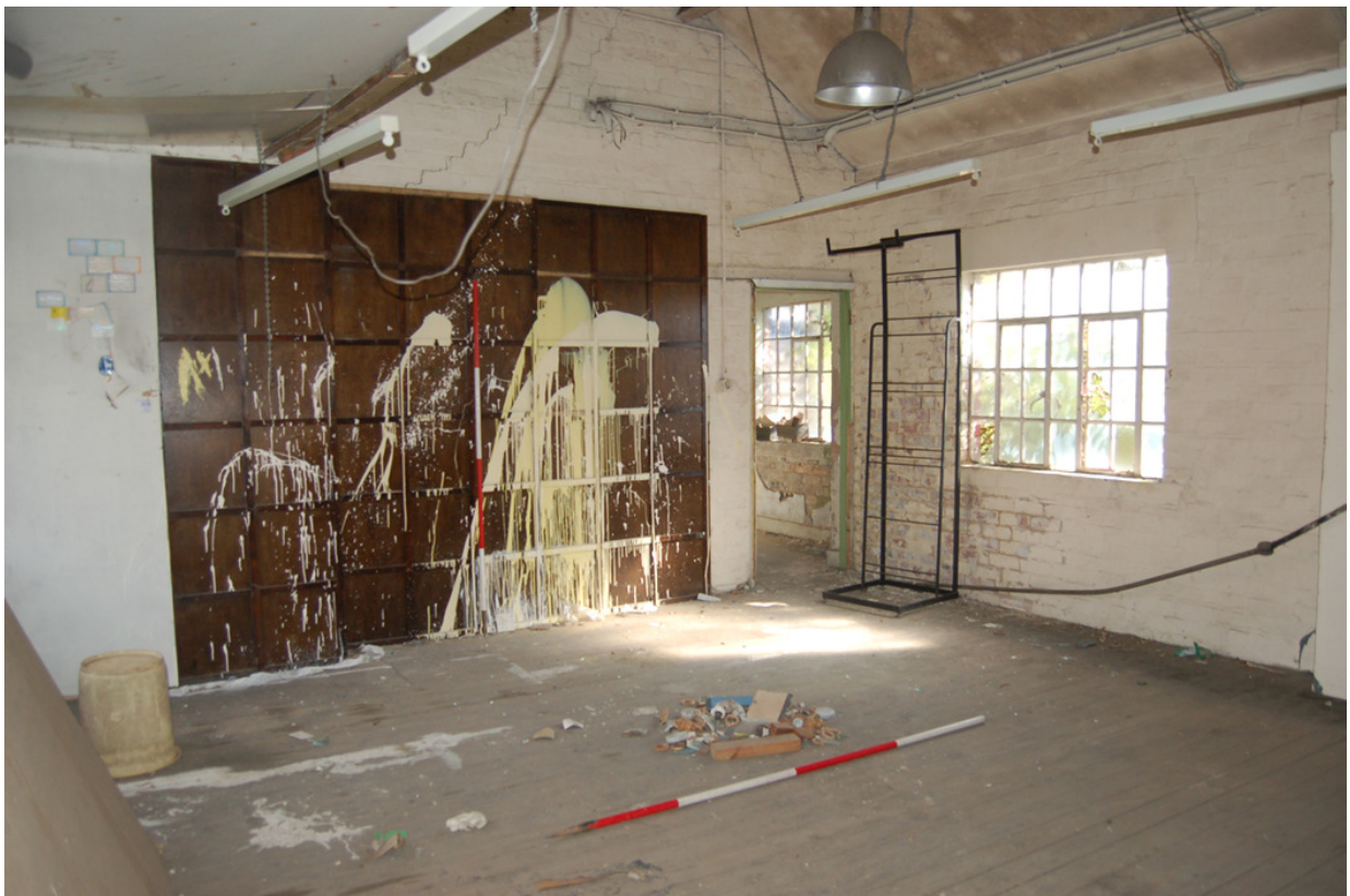
Plate 320: Building F, 1 st floor looking north-west.
