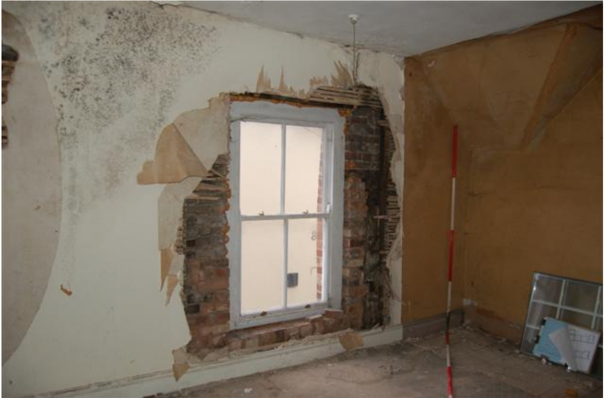
Plate 141: Building B, Block B1; Room BF3 looking east.
