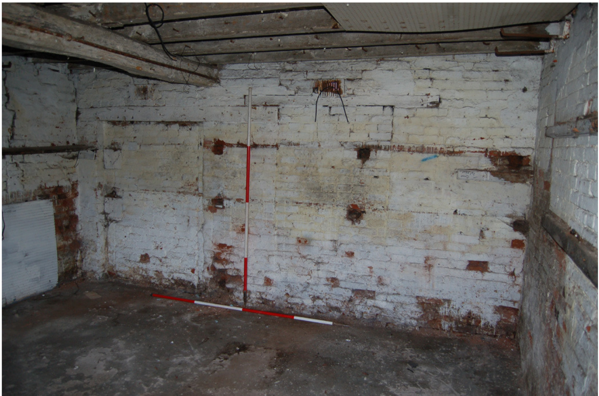
Plate 208: Building B, Block B7; Room BG24, south wall.
