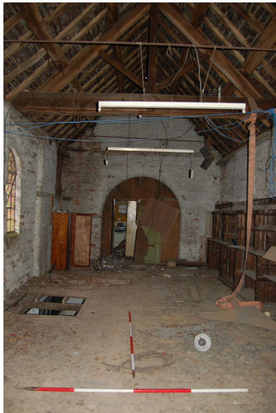
Plate 286: Building D, Room D7 looking east.
