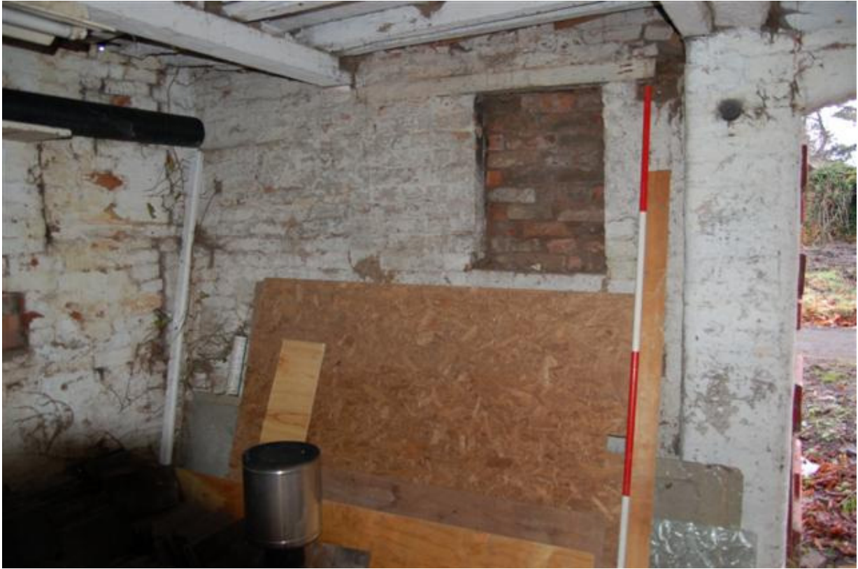
Plate 99: Building A, Block A7; Room AG14 looking north.
