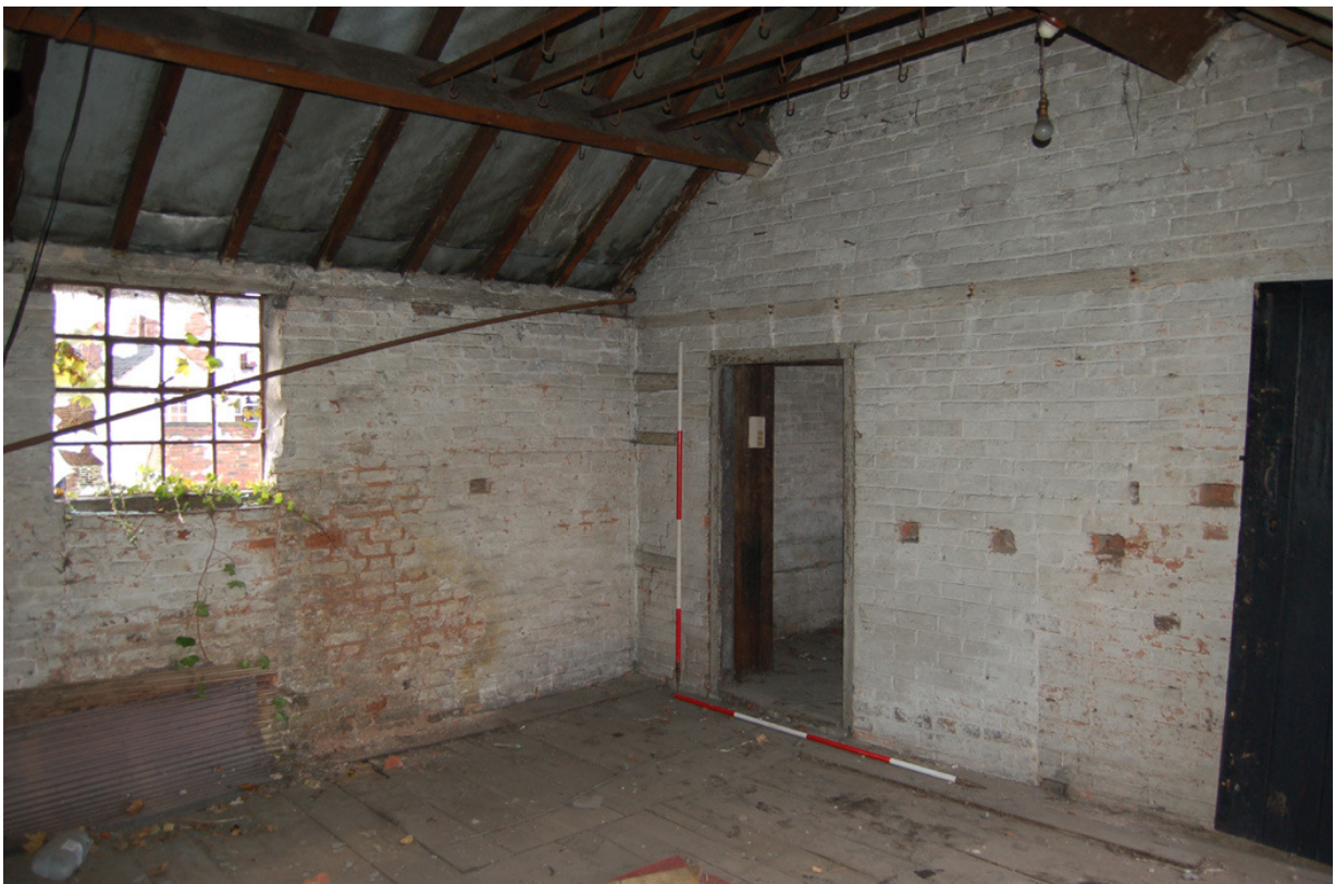
Plate 210: Building B, Block B7; Room BF21 looking south-west.
