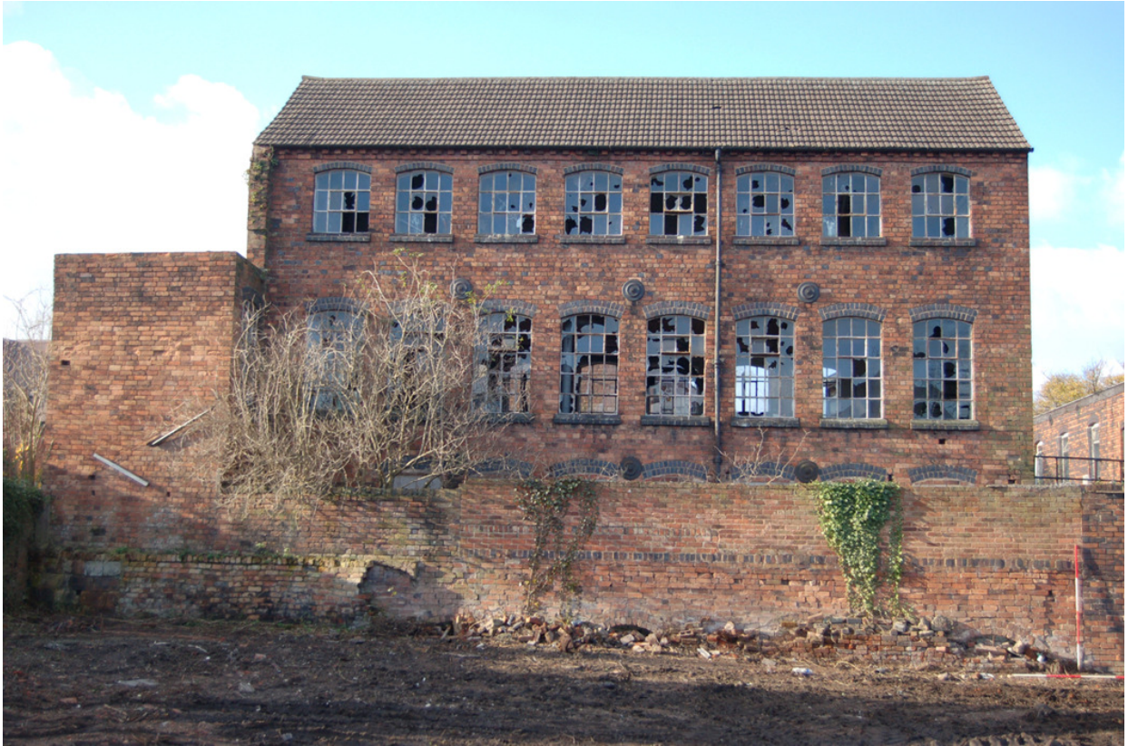
Plate 301: Building E, east elevation. Note stair turret (left) and manufactory boundary wall (foreground).
