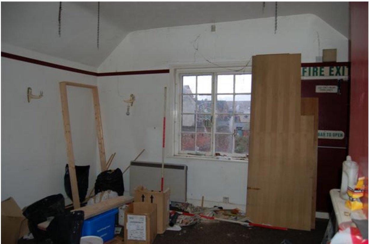
Plate 268: Building C, Block C3; Room CF14 looking west.
