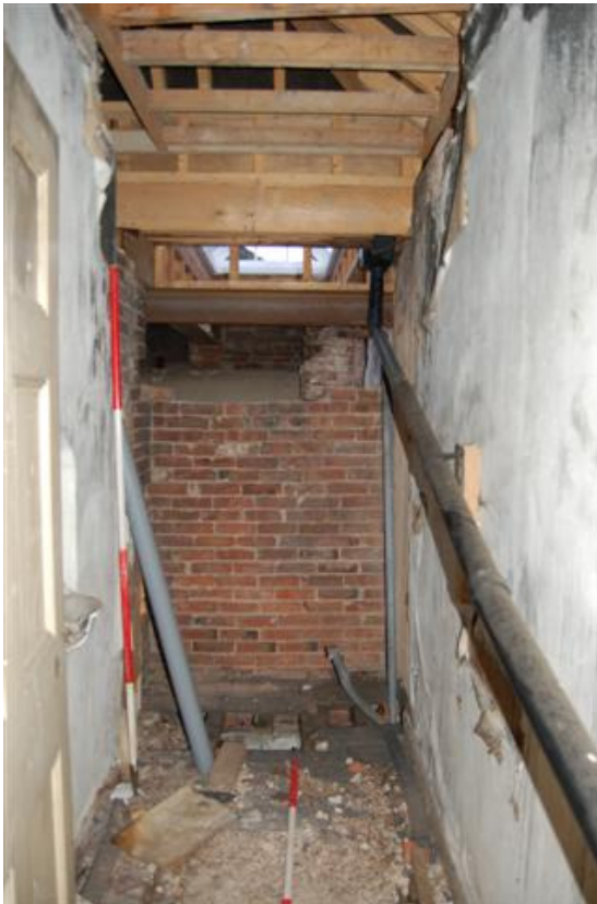
Plate 173: Bldg B, Block B4; Rm BF13 looking E.
