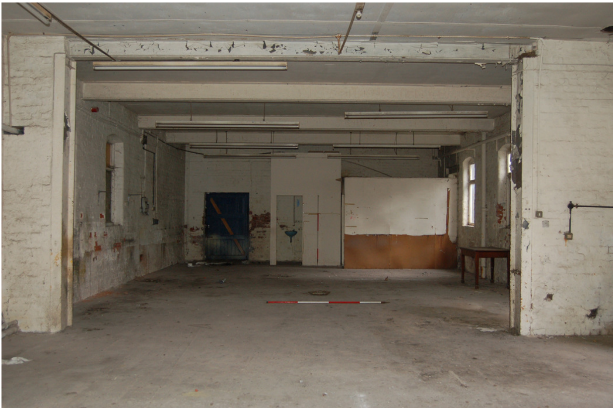
Plate 339: Building H, ground floor looking east.
