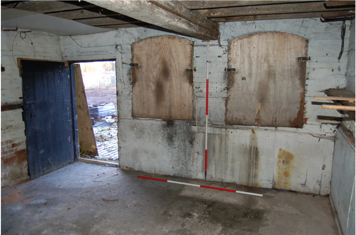
Plate 207: Building B, Block B7; Room BG24, north wall.
