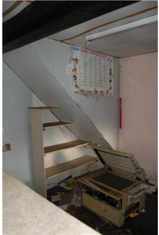
Plate 278: Building D, Room D1 looking NE.
