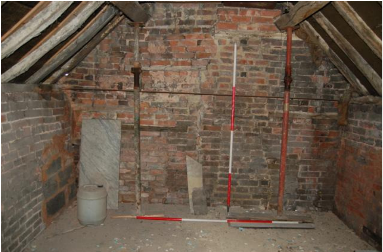
Plate 104: Building A, Block A7; Room AF15 looking west.
