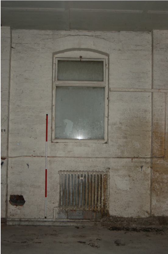
Plate 342: Building H, GF window detail.
