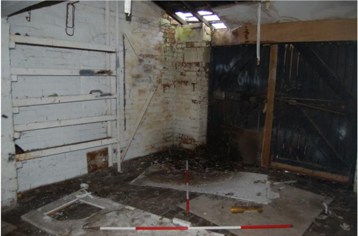
Plate 282: Building D, Room D4b looking north-west.
