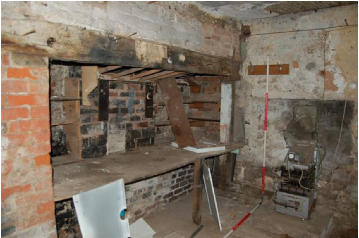
Plate 52: Building A, Block A4; Room AG9 looking north.
