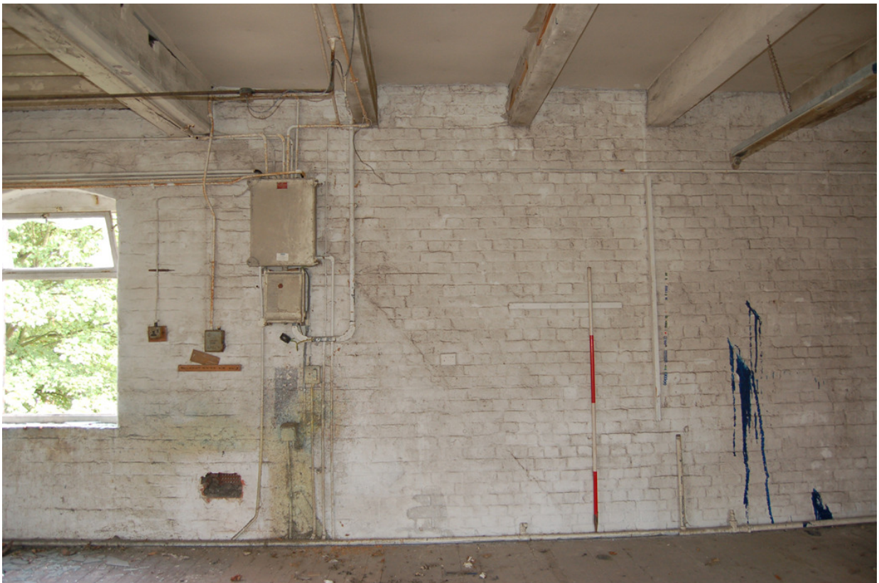
Plate 348: Building H, 1 st floor' scar of former stair at Bay 2, (north).
