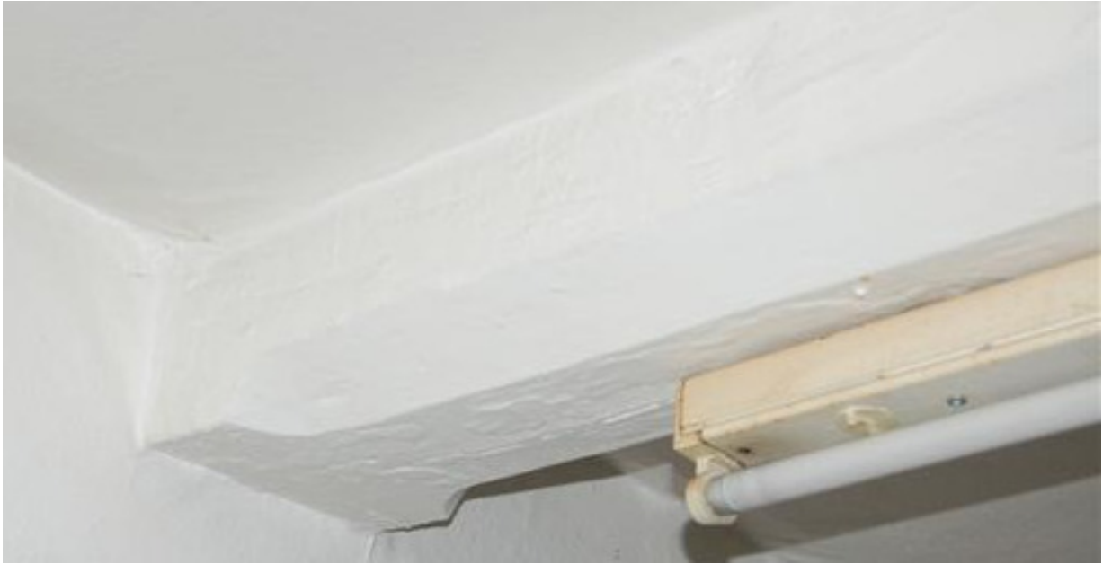
Plate 233: Building C, Block C1; Room CF1 detail of ceiling beam.
