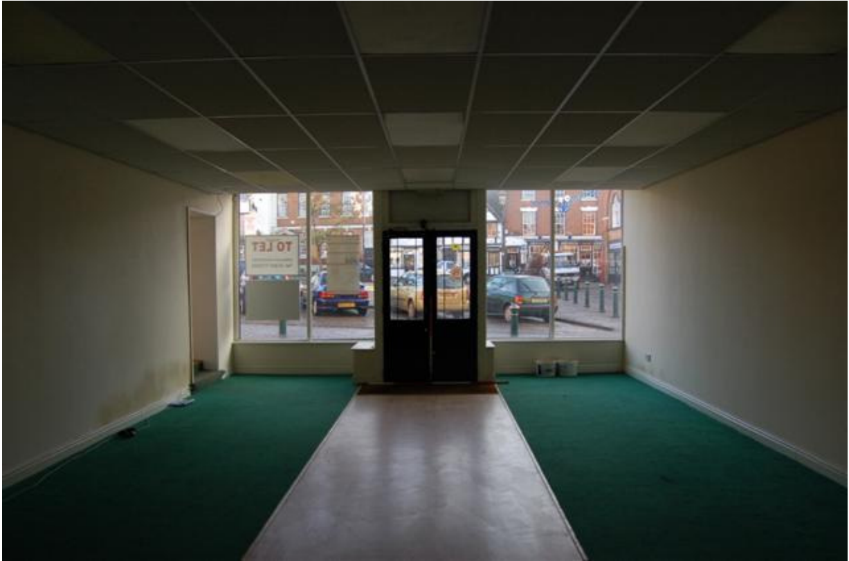
Plate 6: Building A, Block A1; Room AG1 looking east.
