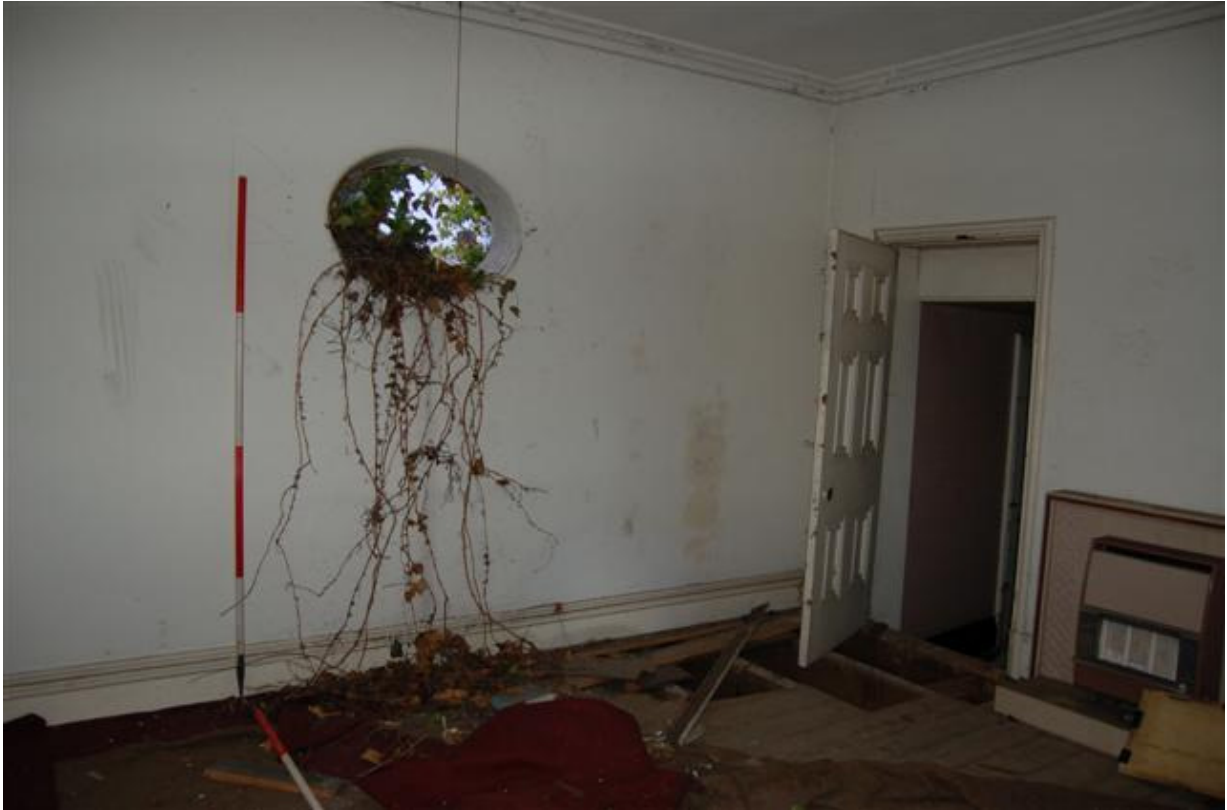
Plate 191: Building B, Block B6; Room BF17 looking south-west.
