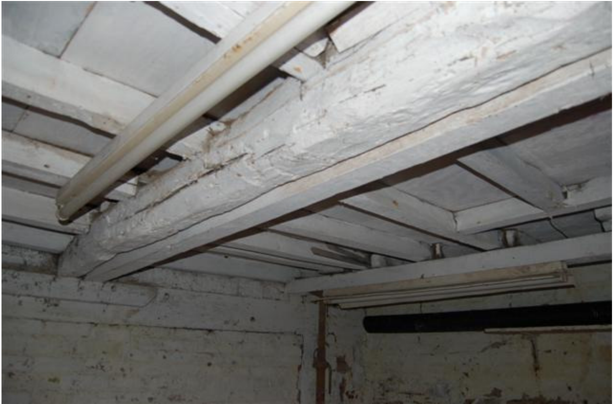
Plate 103: Building A, Block A7; Room AG14 ceiling structure looking south-west.
