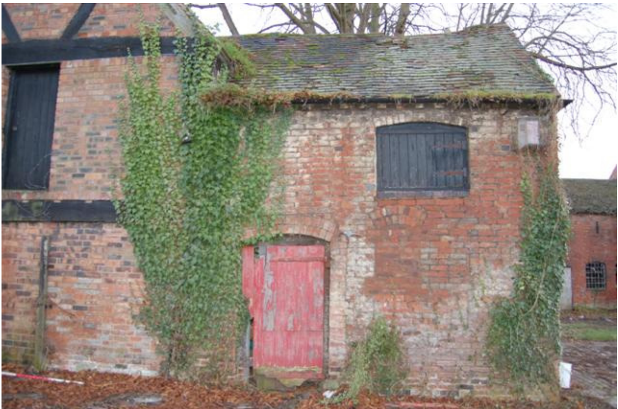
Plate 95: Building A, Block A7; north elevation.
