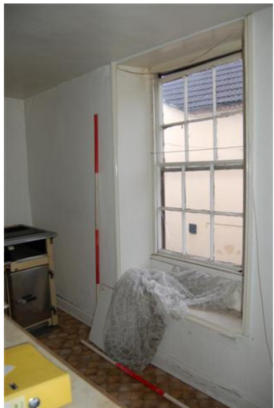
Plate 230: Bldg C, Block C1; Rm CF1 → NE.
