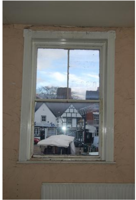
Plate 11: Building A Block A1; Room AF1 window detail.
