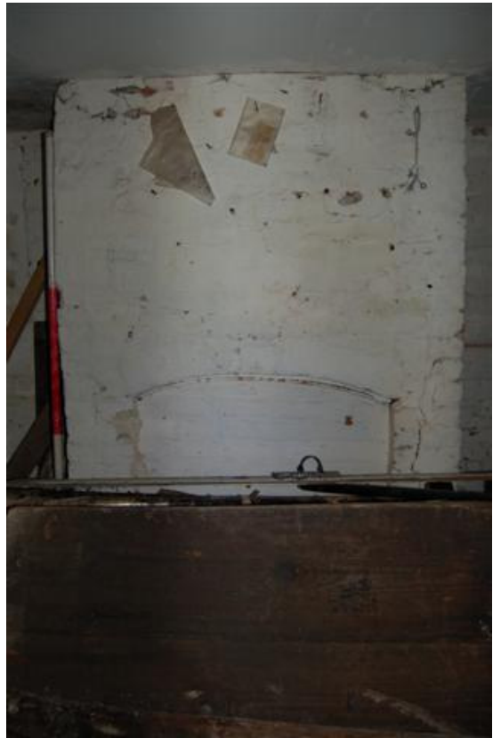
Plate 82: Bldg A, Block A6; Rm AG13 fireplace.
