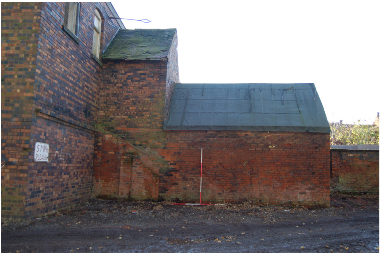
Plate 335: Building H, north elevation (extensions).
