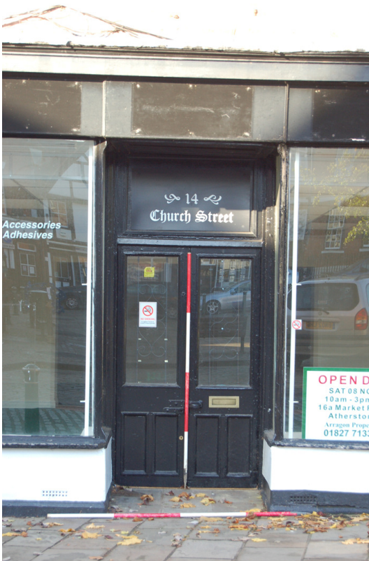
Plate 5: Building A Block A1, No. 14 Church St.
