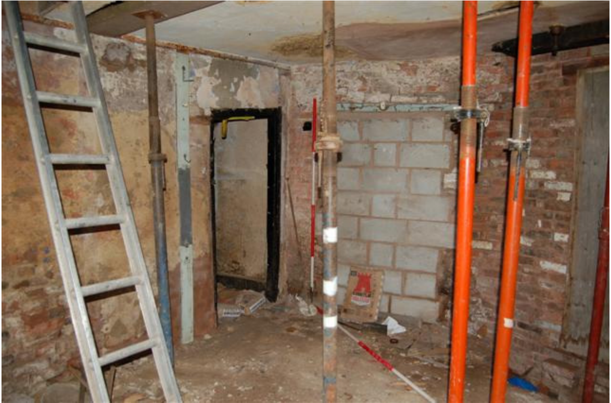
Plate 67: Building A, Block A5; Room AG10/12 looking south-east.
