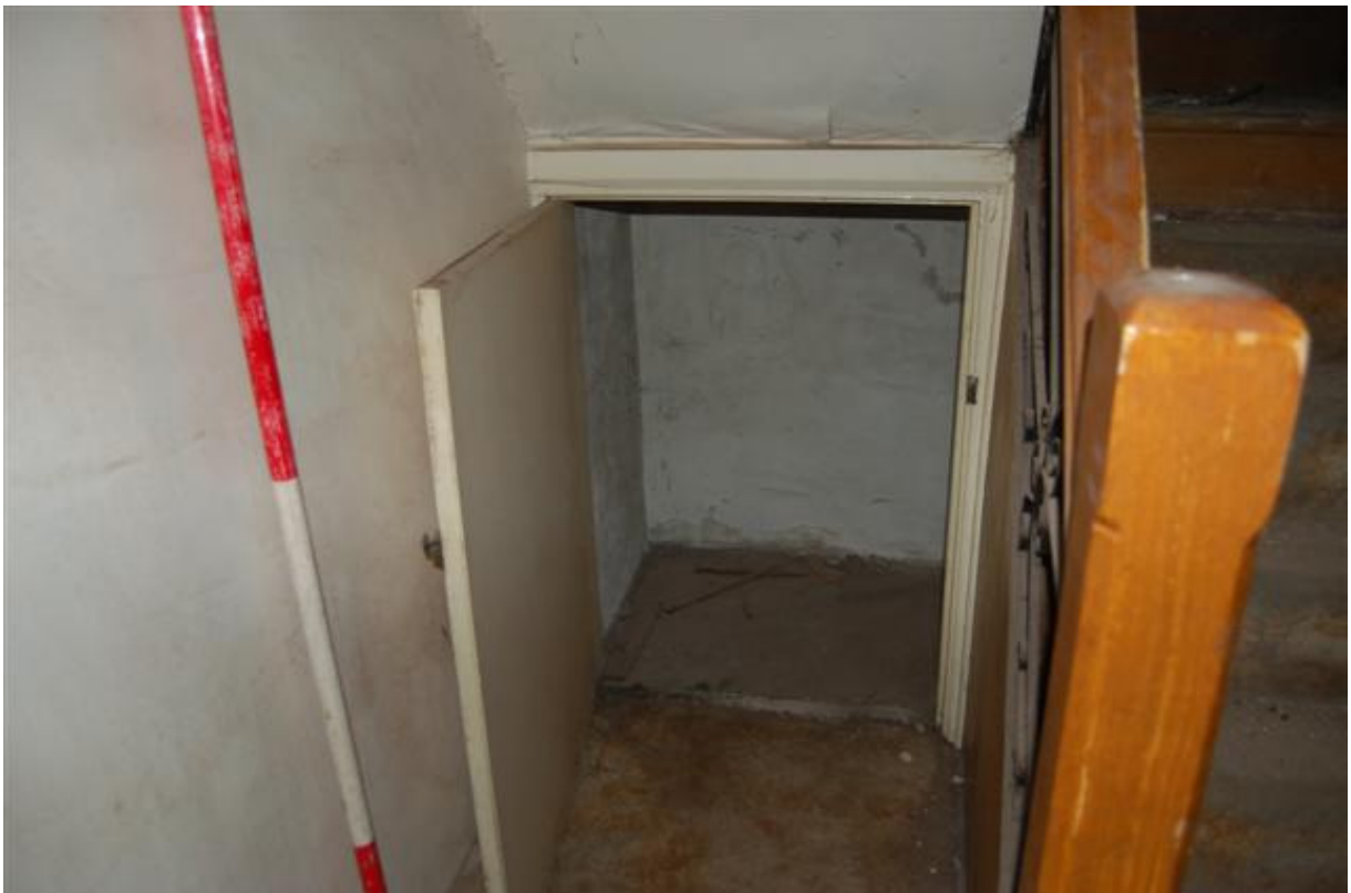
Plate 126: Building B, Block B1, Room BG5 looking south.
