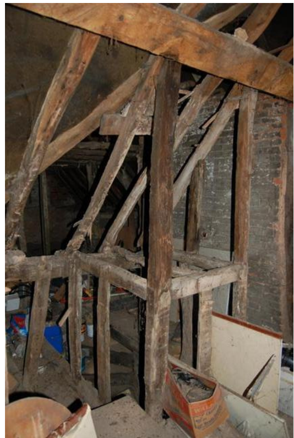
Plate 250: Bldg C, Block C1, Room CS1 stair.
