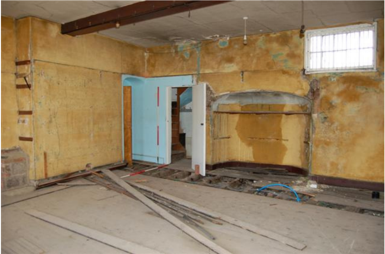
Plate 28: Building A, Block A3; Room AF5 looking south-west.
