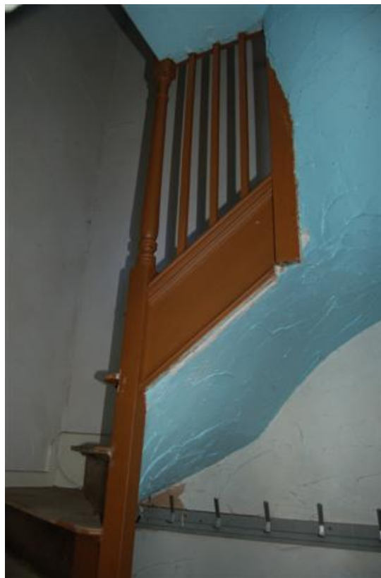
Plate 57: Bldg A, Block A5; Room AF7 stair detail.
