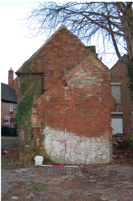
Plate 97: Building A, Block A7; west elevation.
