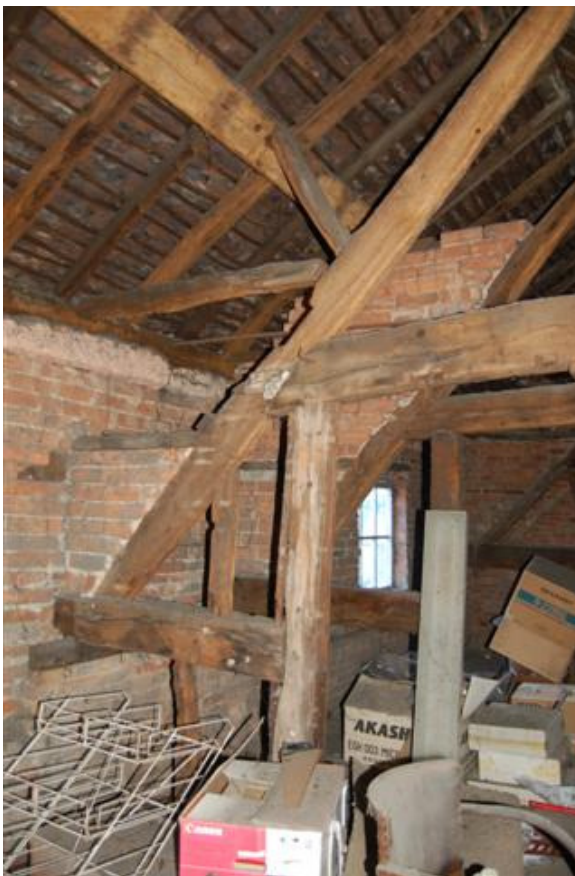
Plate 249: Bldg C, Block C1, Roof structure.
