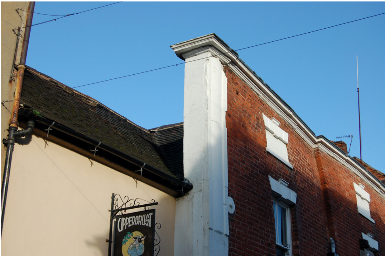
Plate 108: Building B (No 12 Church Street), parapet wall masking original gables.
