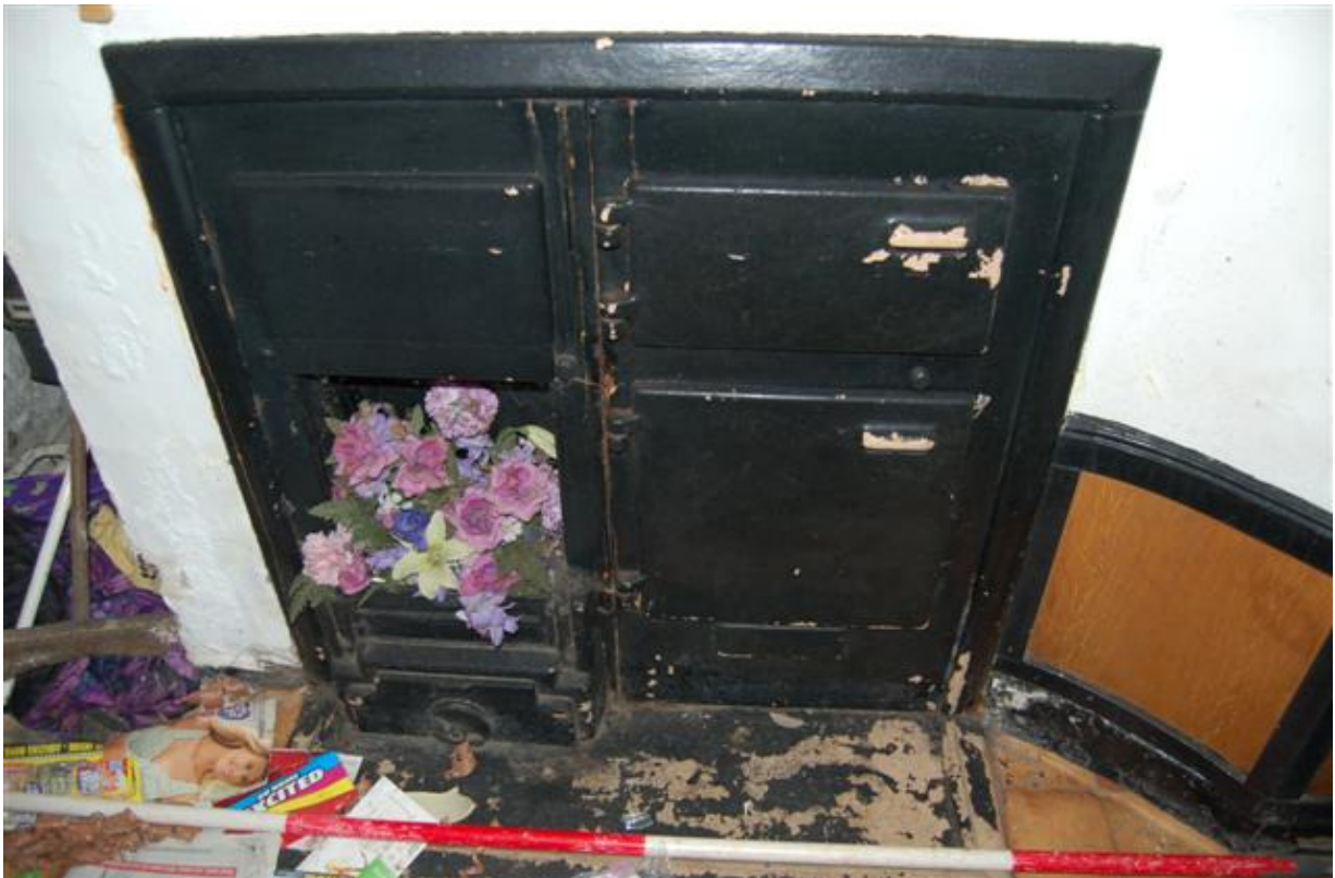
Plate 258: Building C, Block C2; Room CG8 detail of range
