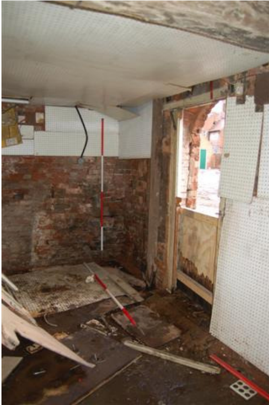
Plate 277: Building D, Room D1 looking SE.
