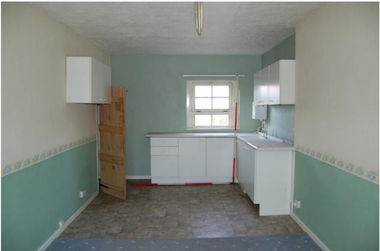
Plate 42: Building A, Block A3; Room AS5 looking west.
