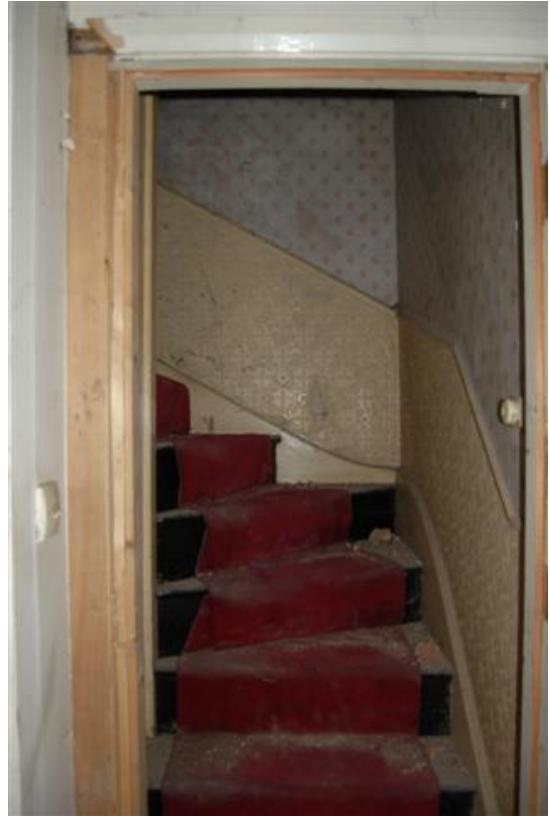
Plate 169: Bldg B, Block B4; stair GF-1F.
