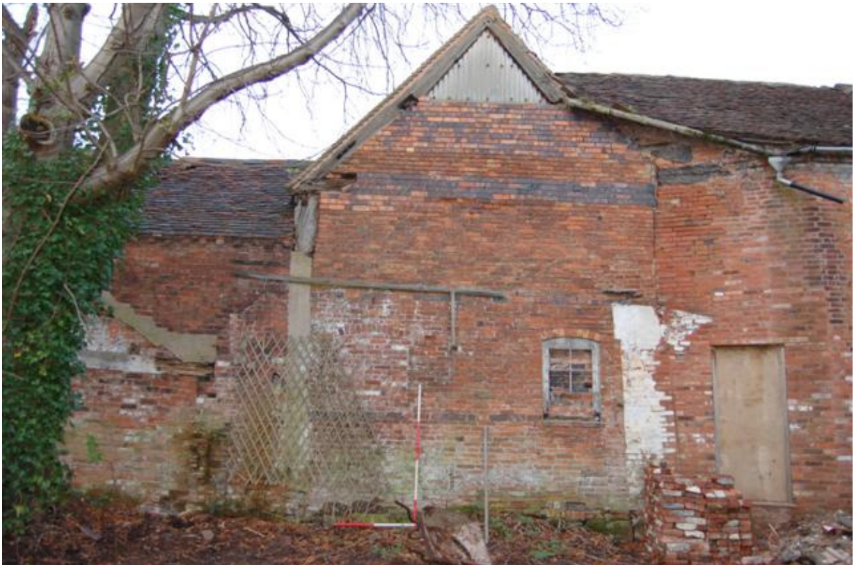
Plate 77: Building A, Block A6; south elevation.
