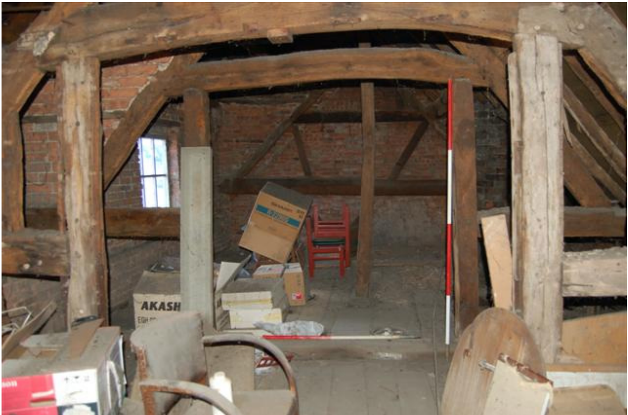
Plate 245: Building C, Block C1; Room CS2 roofspace looking south.
