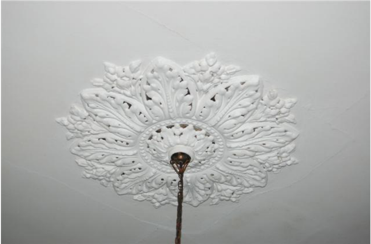
Plate 189: Building B, Block B6; Room BG17 ceiling rose.
