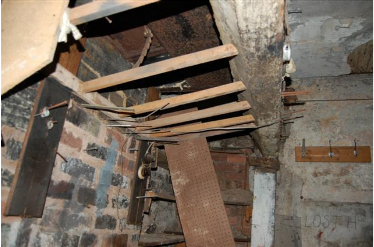
Plate 53: Building A, Block A4; Room AG9, fireplace bressummer from south.
