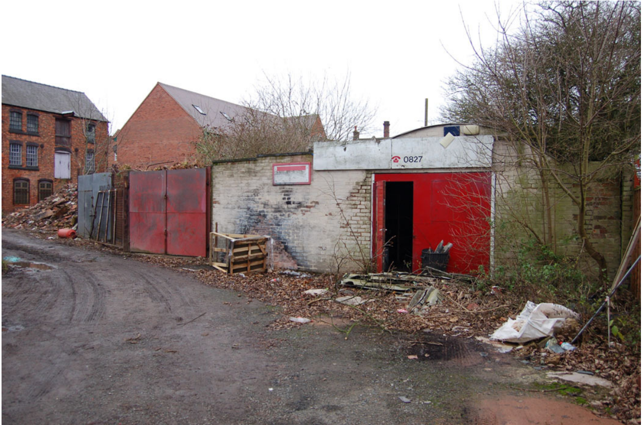
Plate 349: Building I and associated yard, north elevation, oblique.
