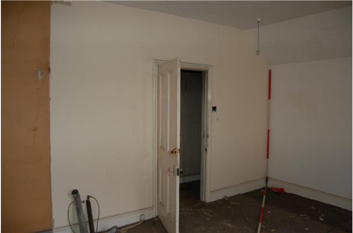
Plate 139: Building B, Block B1; Room BF3 looking west.
