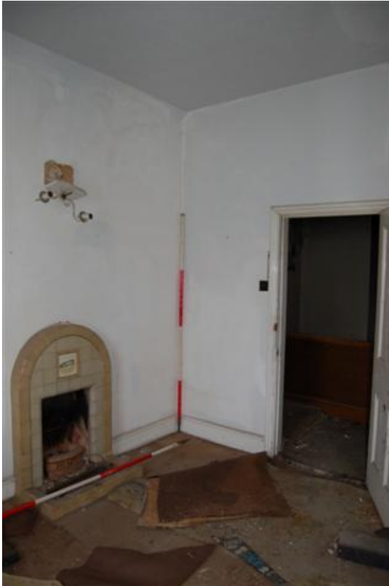
Plate 136: Bldg B, Block B1; Rm BF2 looking SW.
