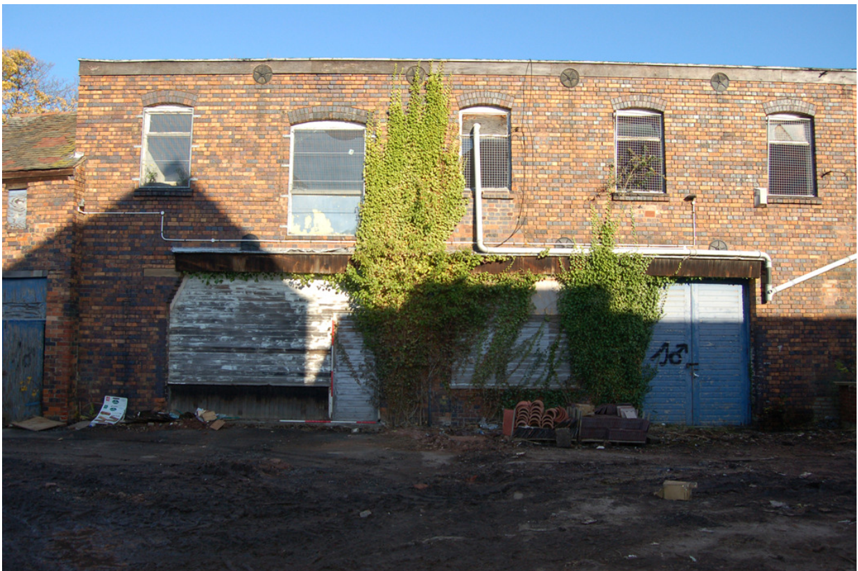
Plate 331: Building H, south elevation (west).
