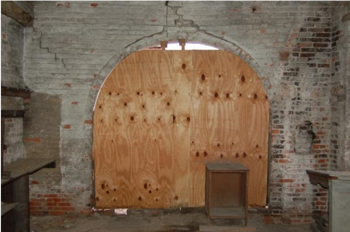
Plate 290: Building D, Room D7 western archway.
