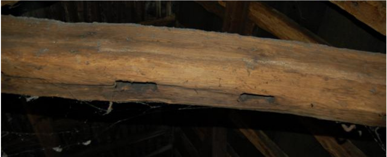
Plate 248: Building C, Block C1; Room CS1 stud mortises to collar soffit
