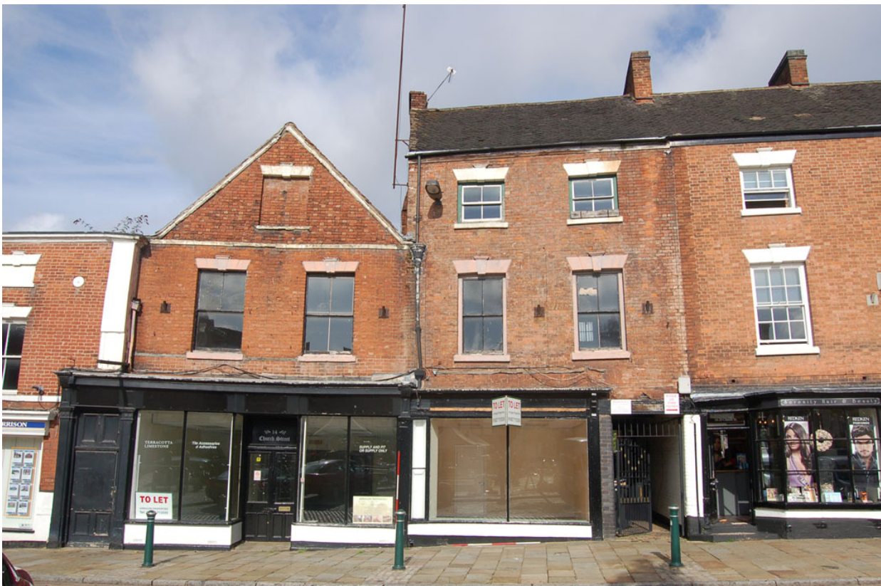
Plate 2: Building A; Nos. 14 [left] and 16 [right] Church Street, north (street) elevation.
