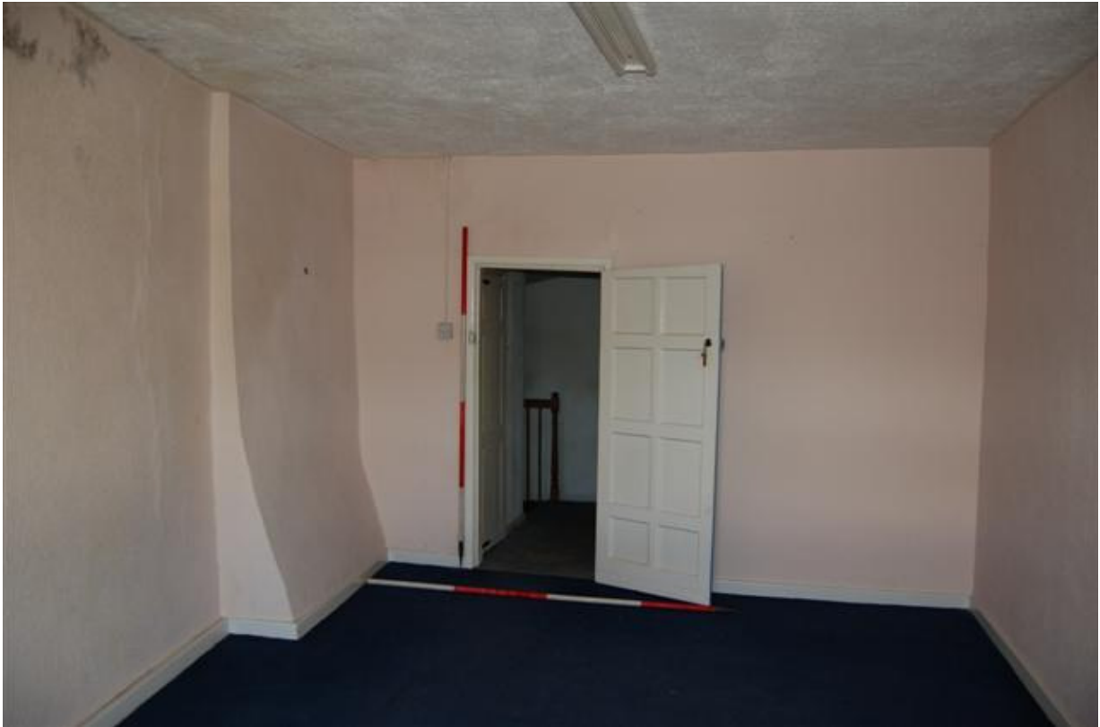
Plate 39: Building A, Block A3; Room AS4 looking west.
