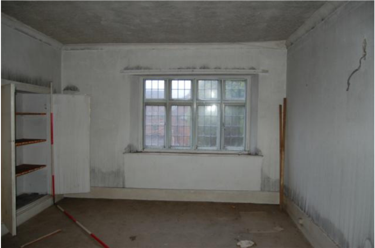
Plate 163: Building B, Block B3; Room BF11 looking west.
