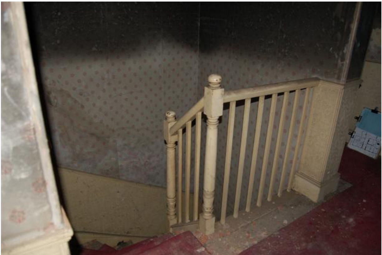
Plate 170: Building B, Block B4; stair 1F-GF.
