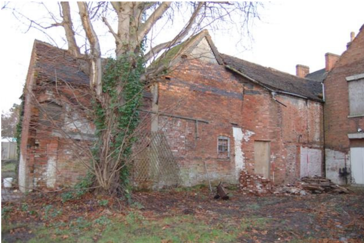
Plate 96: Building A, Block A7; south elevation.
