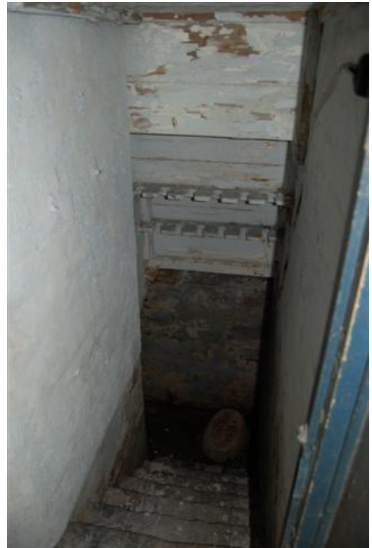
Plate 195: Bldg B, Block B7; Rm BG18 stair to cellar
