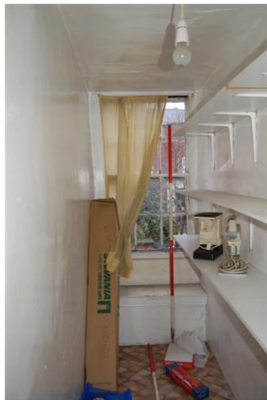
Plate 235: Bldg C, Block C1; Rm CF2 looking E.
