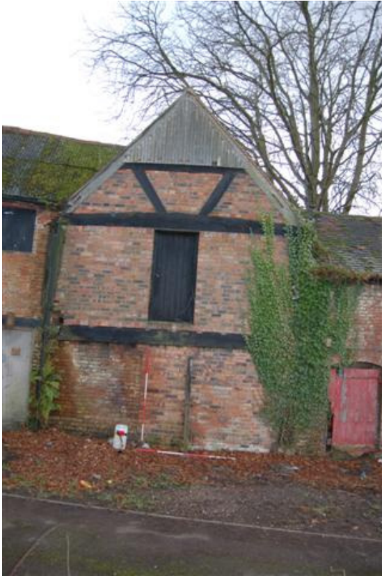
Plate 76: Building A, Block A6; north elevation.
