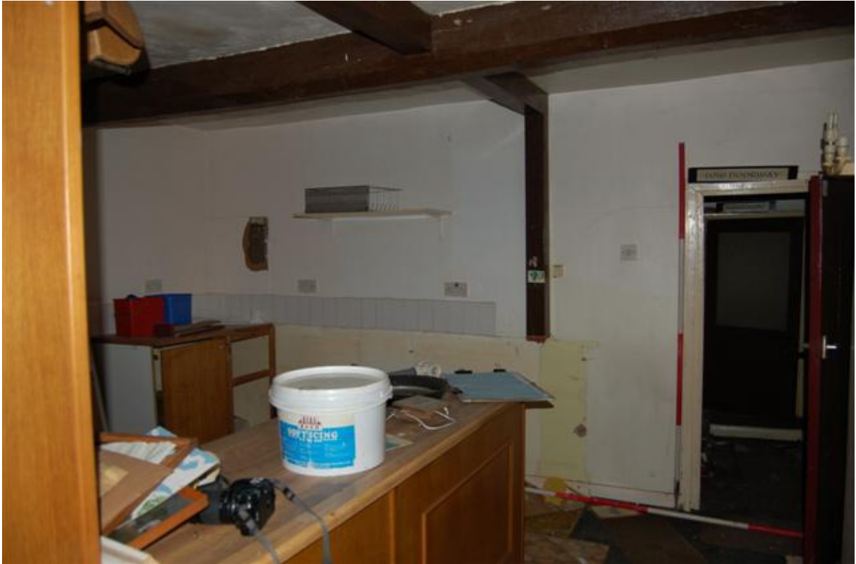
Plate 262: Building C, Block C2; Room CF11 looking east.
