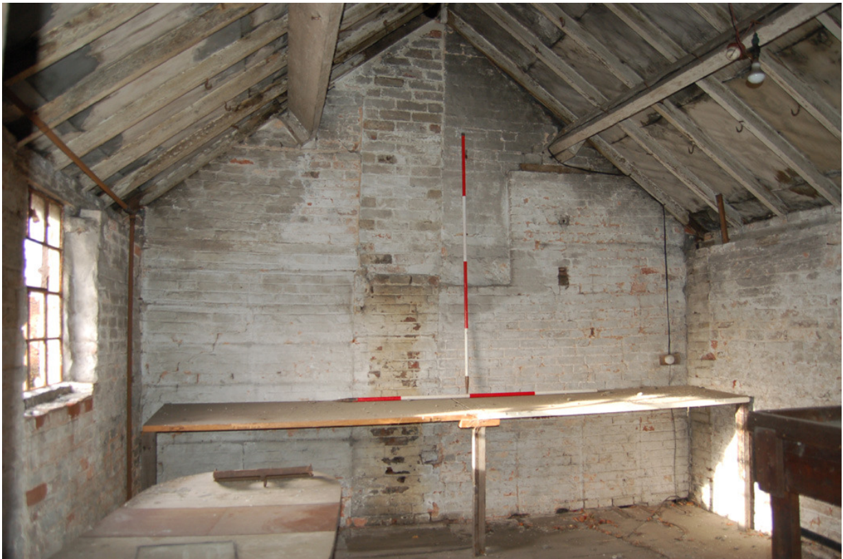
Plate 212: Building B, Block B7; Room BF22 looking west.
