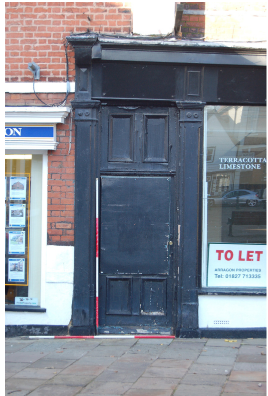
Plate 4: Building A Block A1, No.14/12 Church St.
