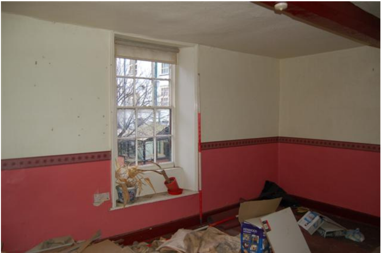
Plate 237: Building C, Block C1; Room CF3 looking south-east.
