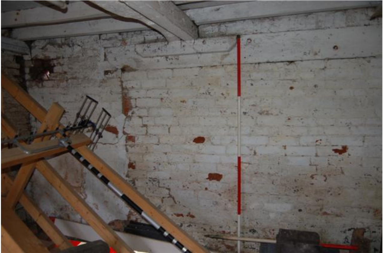
Plate 101: Building A, Block A7; Room AG14 looking south.
