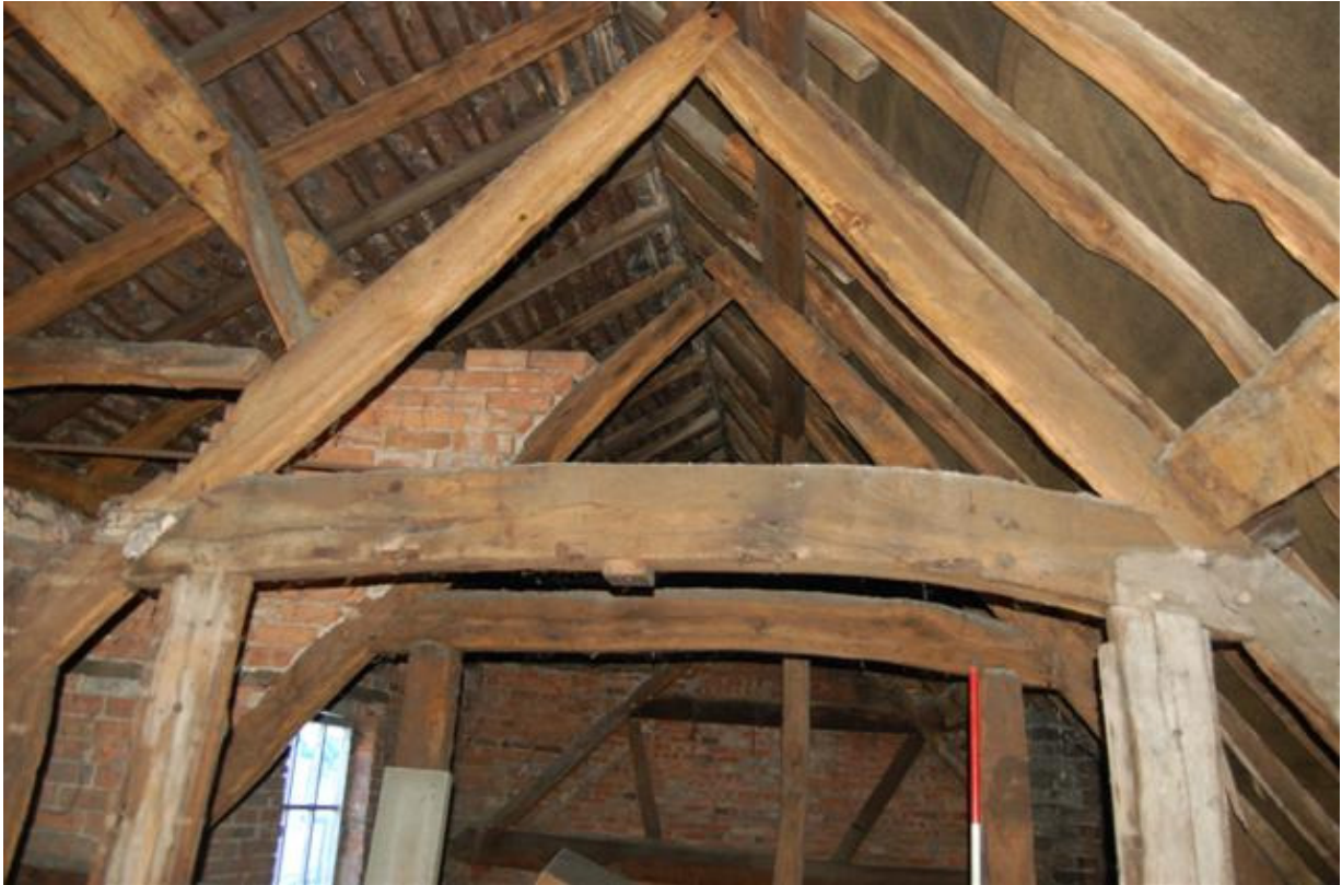
Plate 246: Building C, Block C1; Room CS1/2 roofspace looking south.
