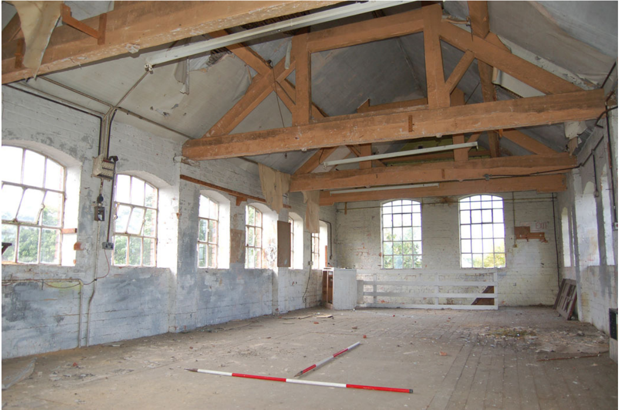
Plate 307: Building E, 2 nd floor looking north.
