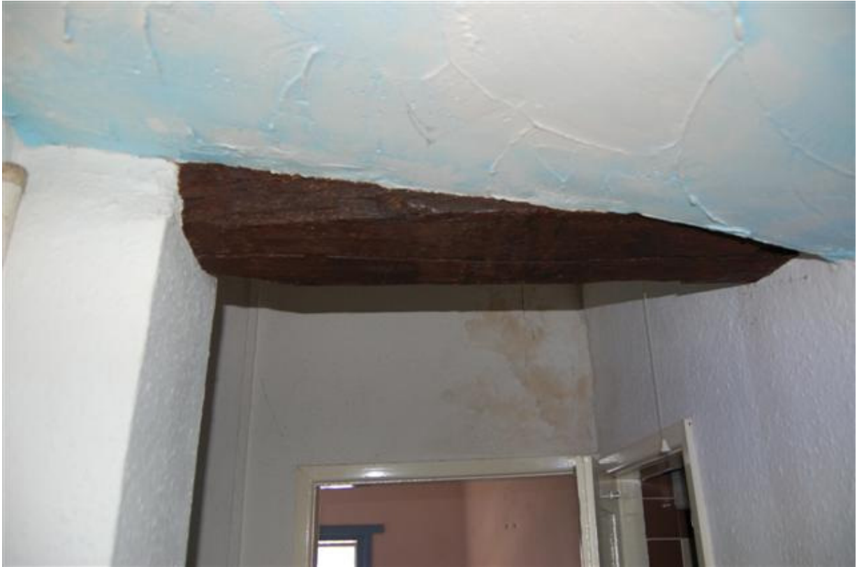
Plate 35: Building A, Block A3; Room AS1, beam at head of stair.
