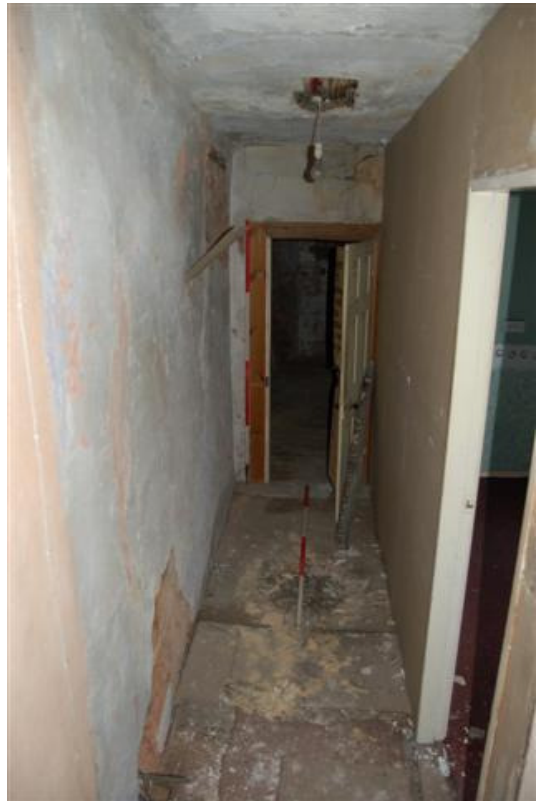
Plate 61: Bldg.A, Block A4; Rm AF11 looking W.
