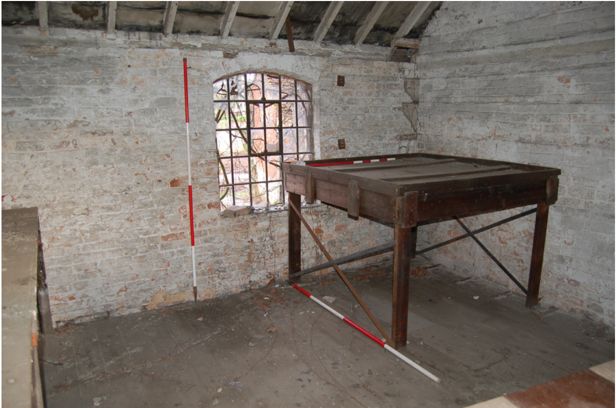
Plate 211: Building B, Block B7; Room BF22 looking north-east.
