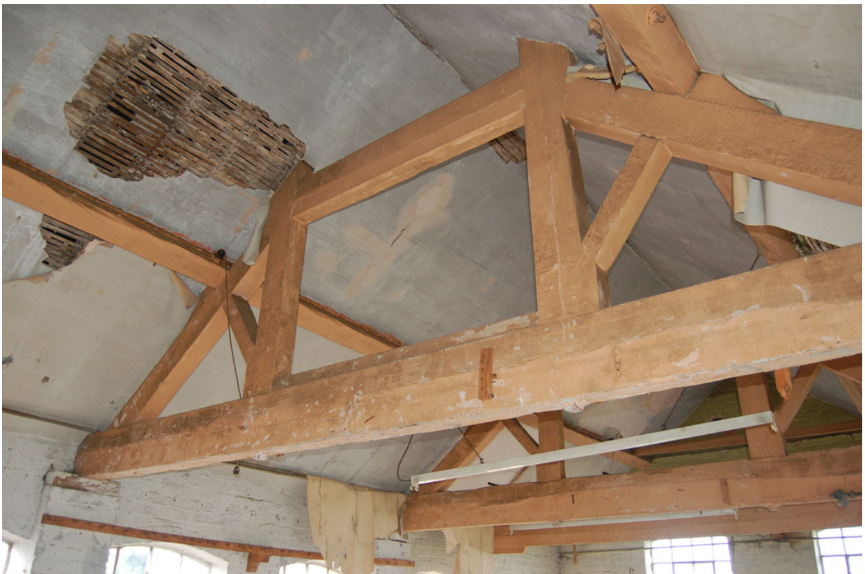
Plate 308: Building E, 2 nd floor; detail of Queen-post truss.
