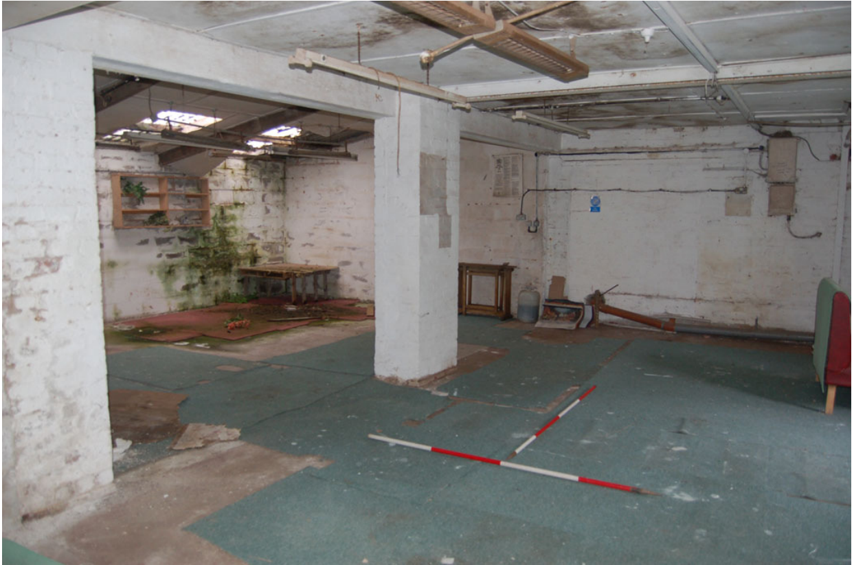
Plate 317: Building F, interior looking south-west: 1970s lean-to extension to left.
