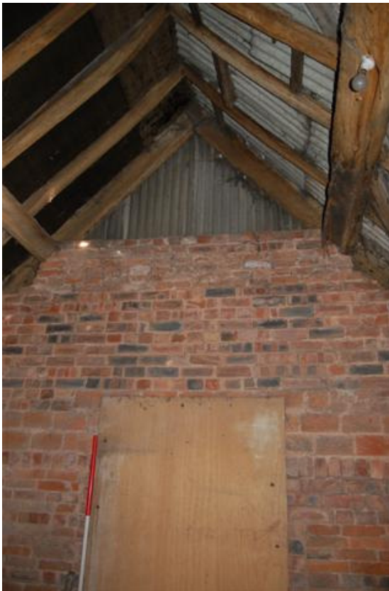
Plate 83: Building A, Block A6; Room AF14, N wall.
