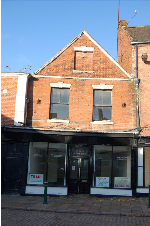
Plate 3: Building A Block A1, No.14 Church St.
