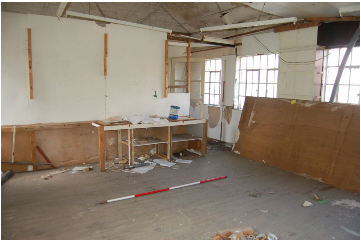
Plate 318: Building F 1 st floor looking east.
