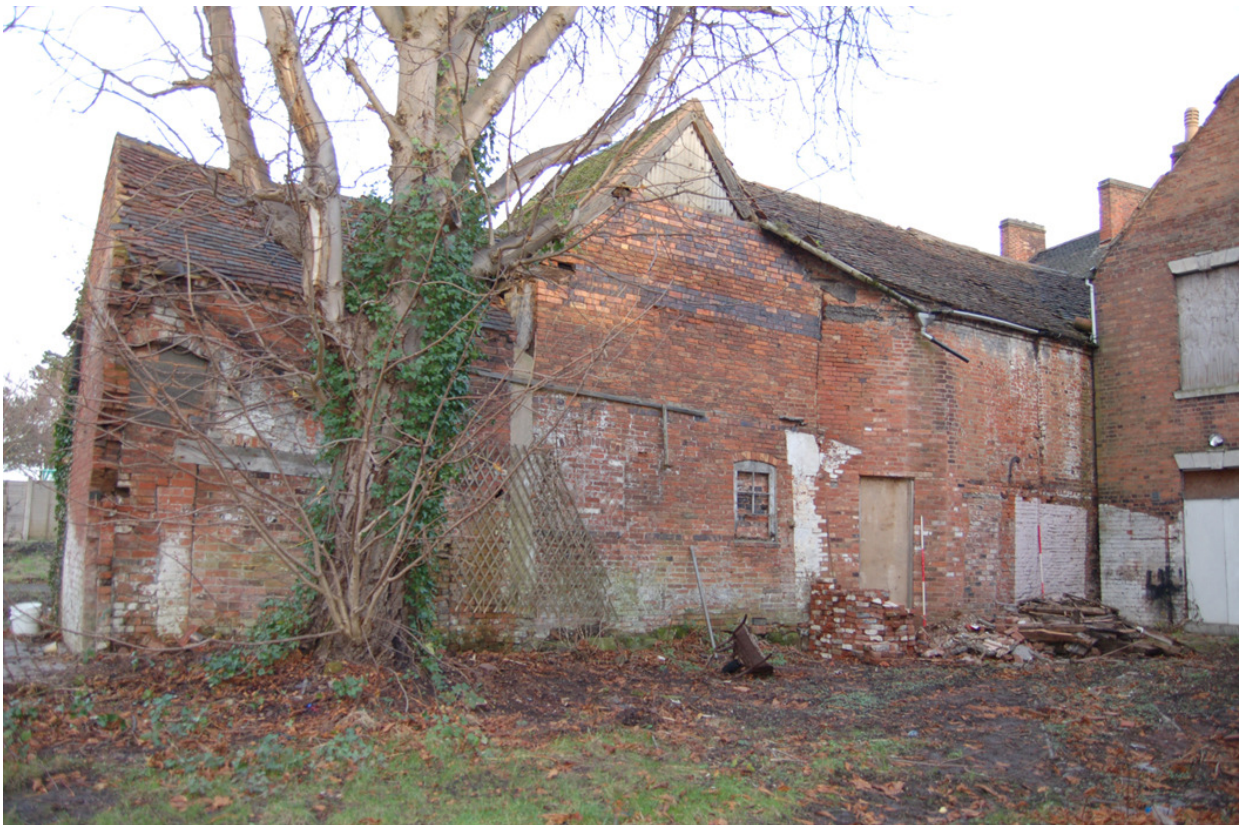
Plate 44: Building A (No. 16) rear range south elevation (oblique).
