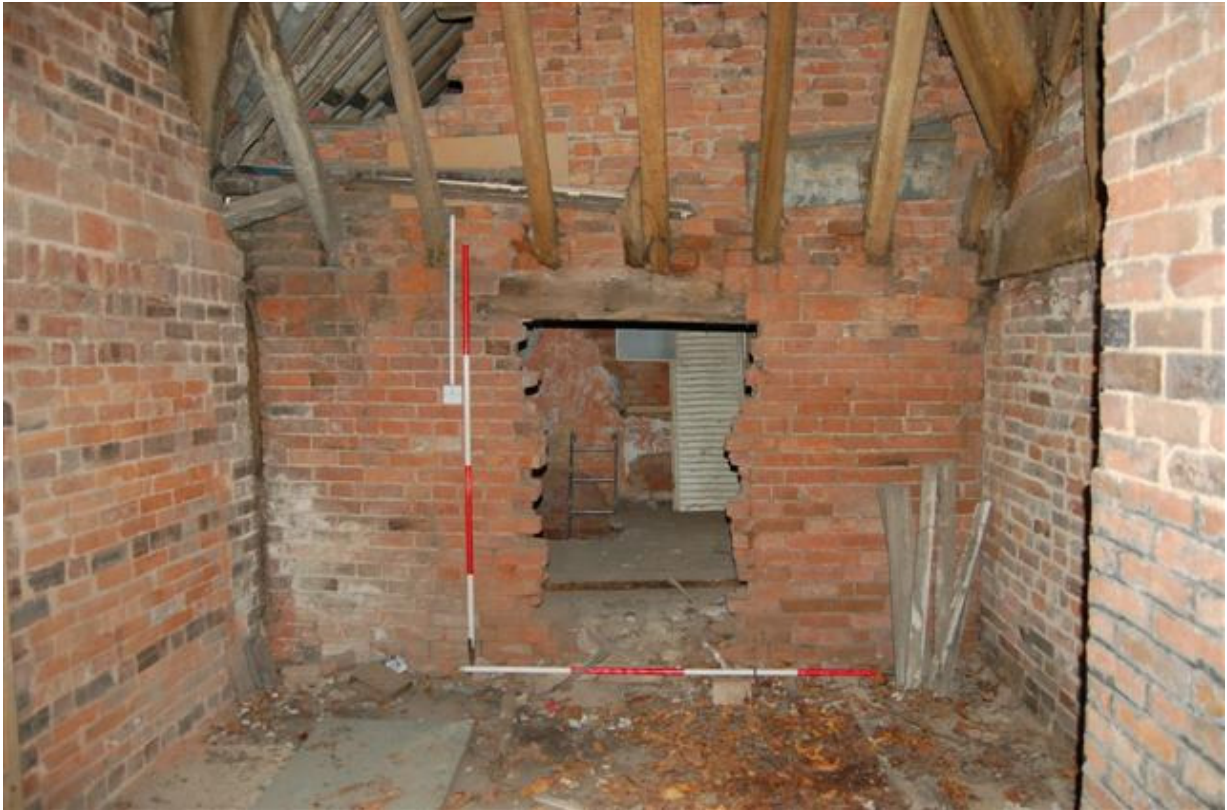
Plate 88: Building A, Block A6; Room AF14, east wall.
