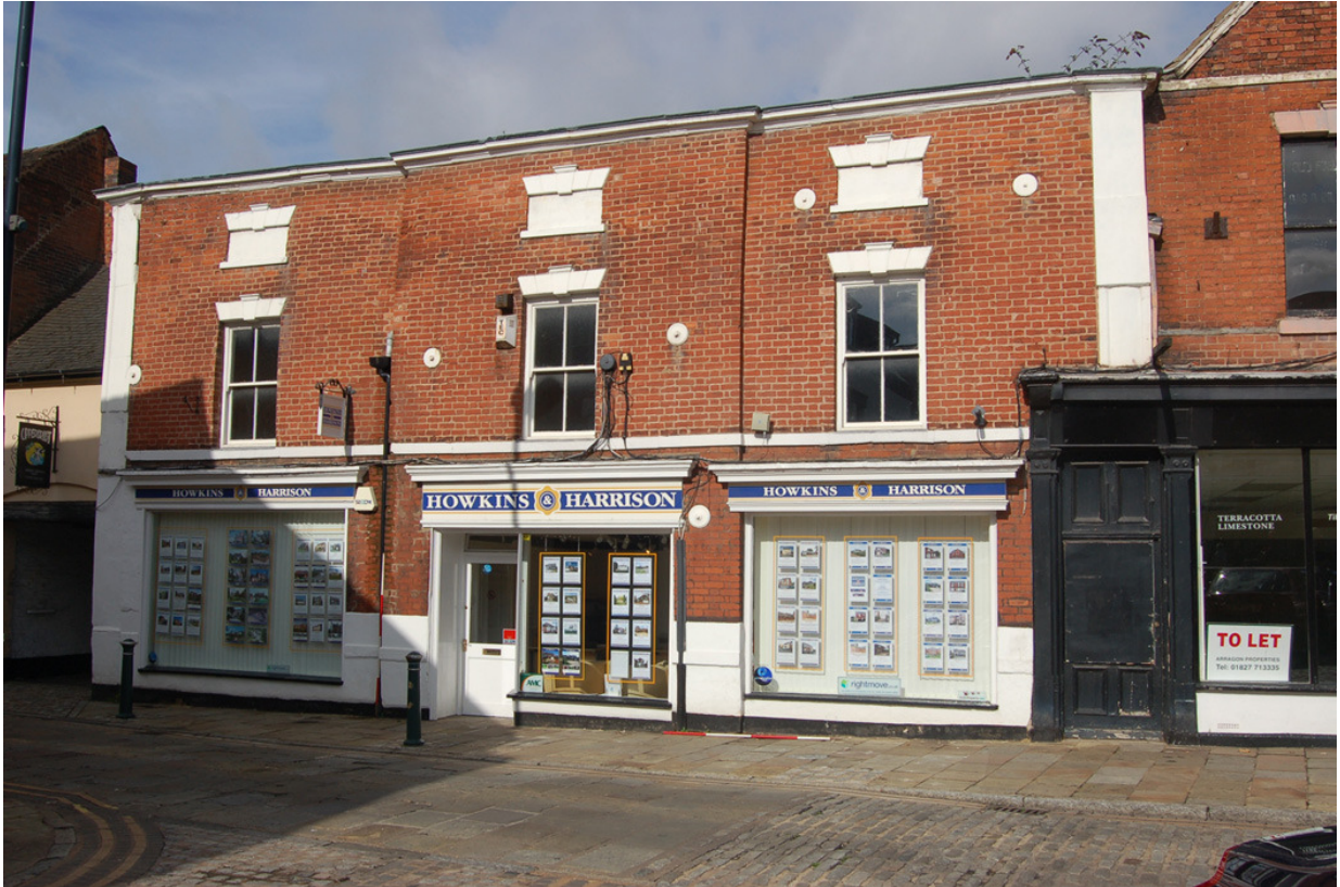
Plate 107: Building B (No 12 Church Street), north (street) elevation.
