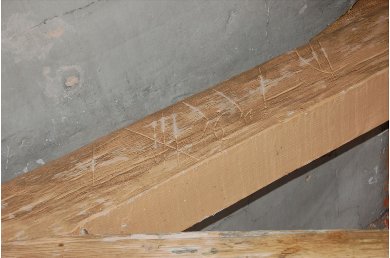
Plate 309: Building E, 2 nd Floor; detail of Baltic importer's marks on northernmost truss.
