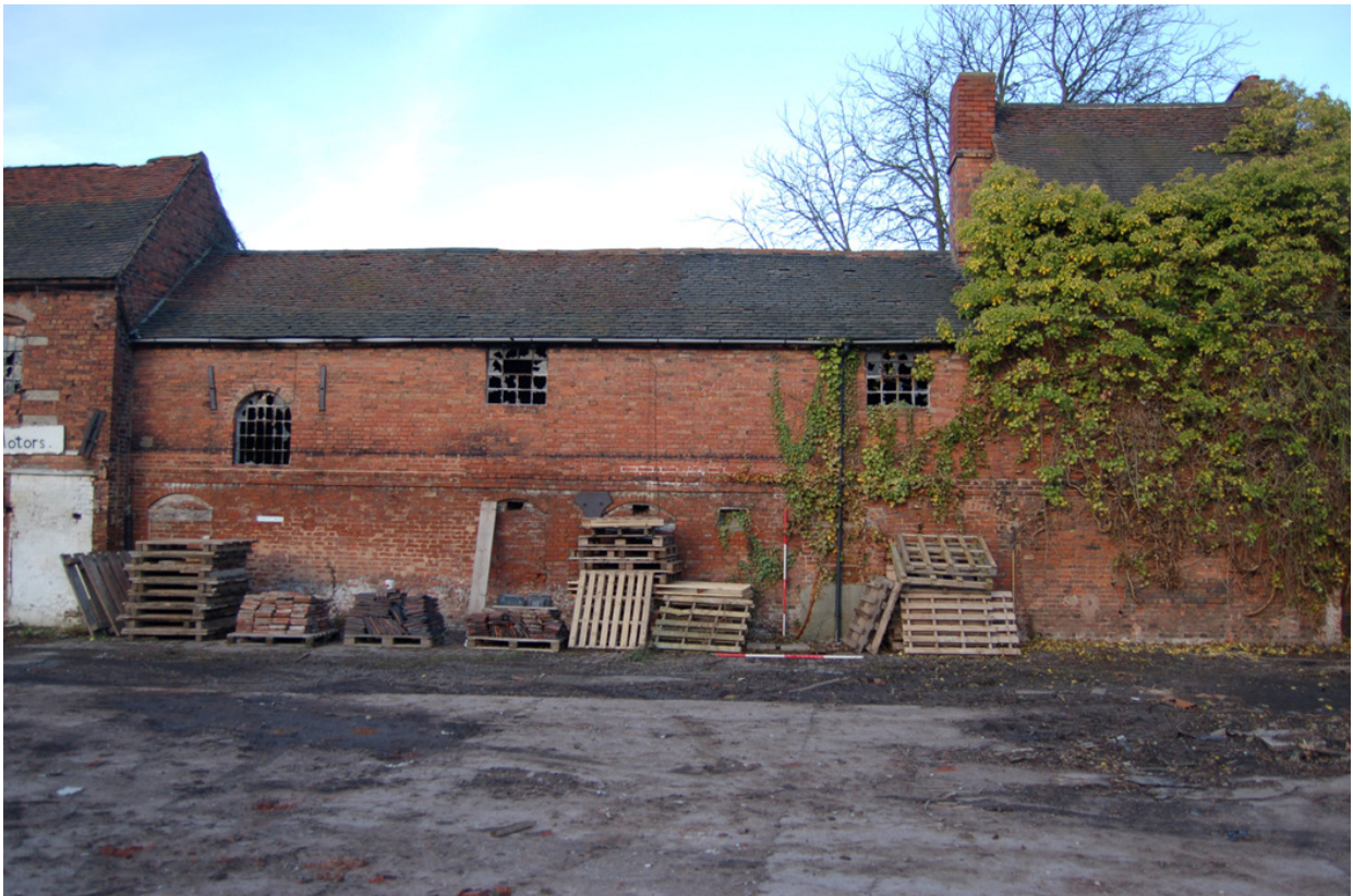
Plate 192: Building B; rear range south elevation (Bldg. D to left).
