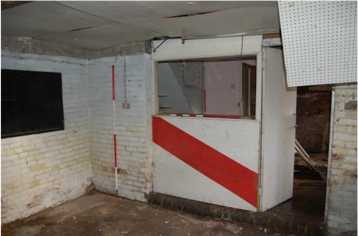
Plate 279: Building D, Room D2 looking east.
