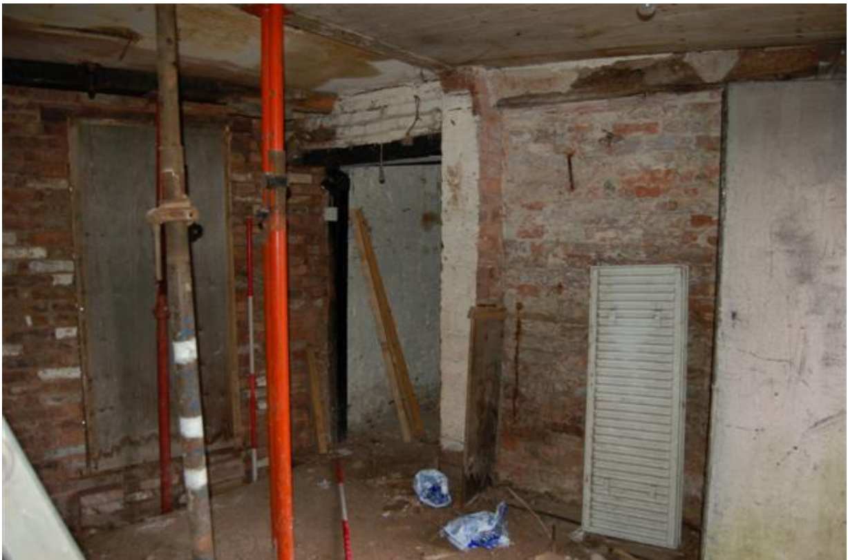
Plate 68: Building A, Block A5; Room AG11/12 looking south-west.
