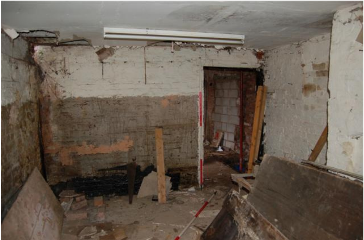
Plate 78: Building A, Block A6; Room AG13 looking east.
