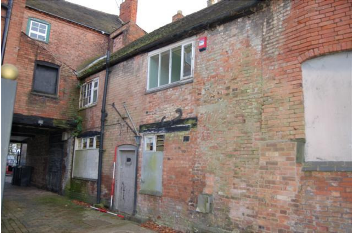
Plate 45: Building A, Blocks A4 and A5, north exterior.
