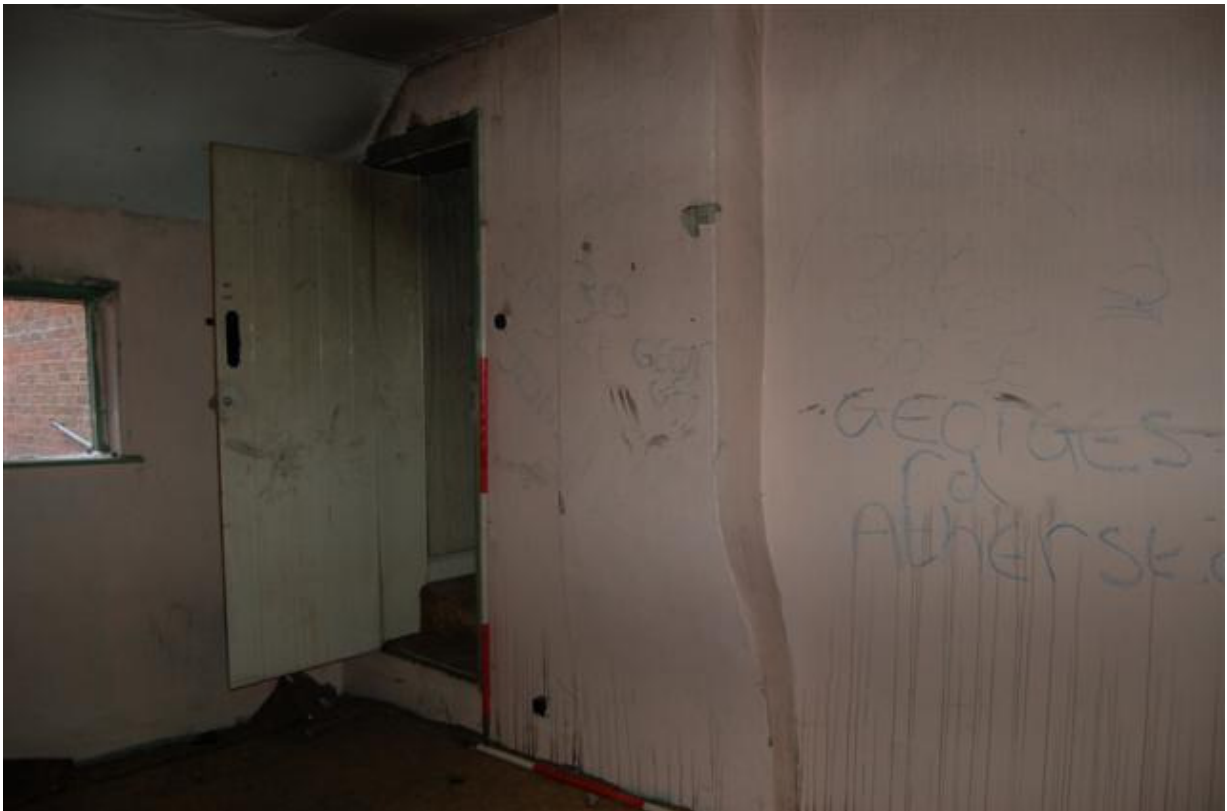
Plate 147: Building B, Block B2; Room BF4 looking north-west.
