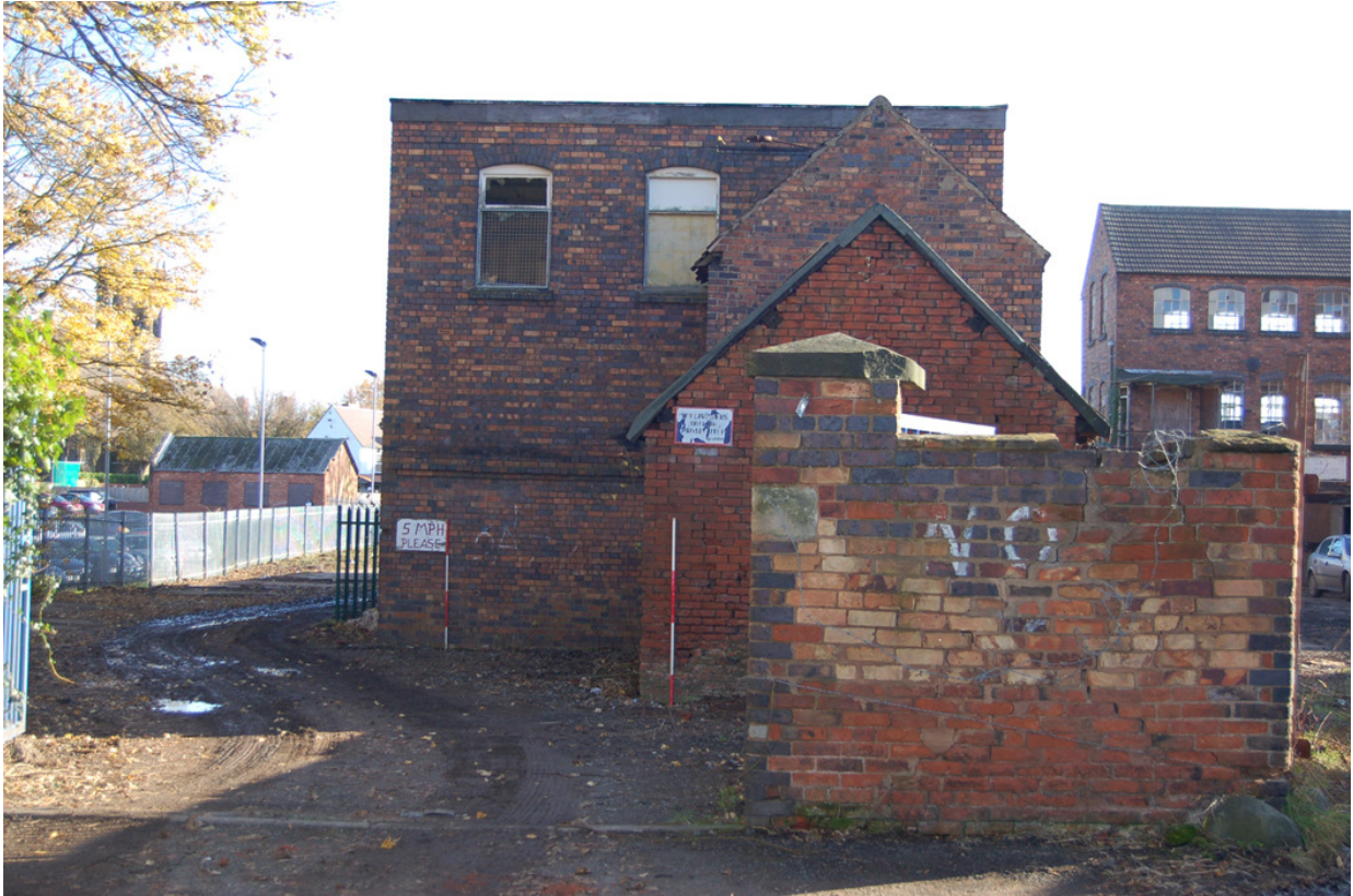
Plate 334: Building H, west elevation.
