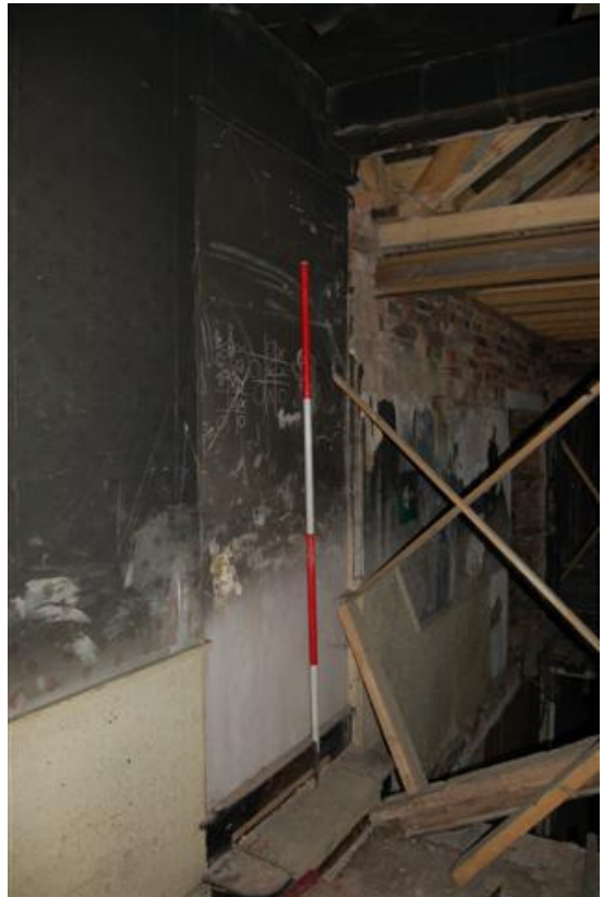
Plate 172: Bldg B, Block B4; Rm BF14 looking E.
