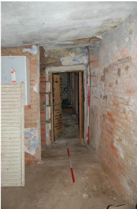
Plate 72: Bldg. A, Block A5; Rm AF13 → E.
