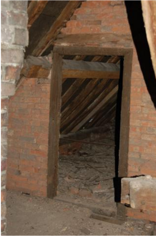
Plate 253: Bldg C, Block C1; Room CS2, door to CS3.
