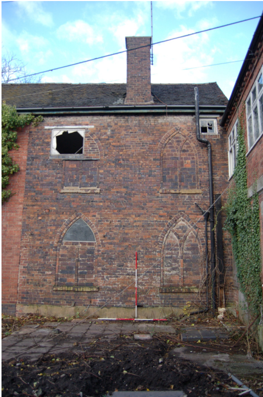
Plate 177: Building B, Block B5 exterior: south elevation.
