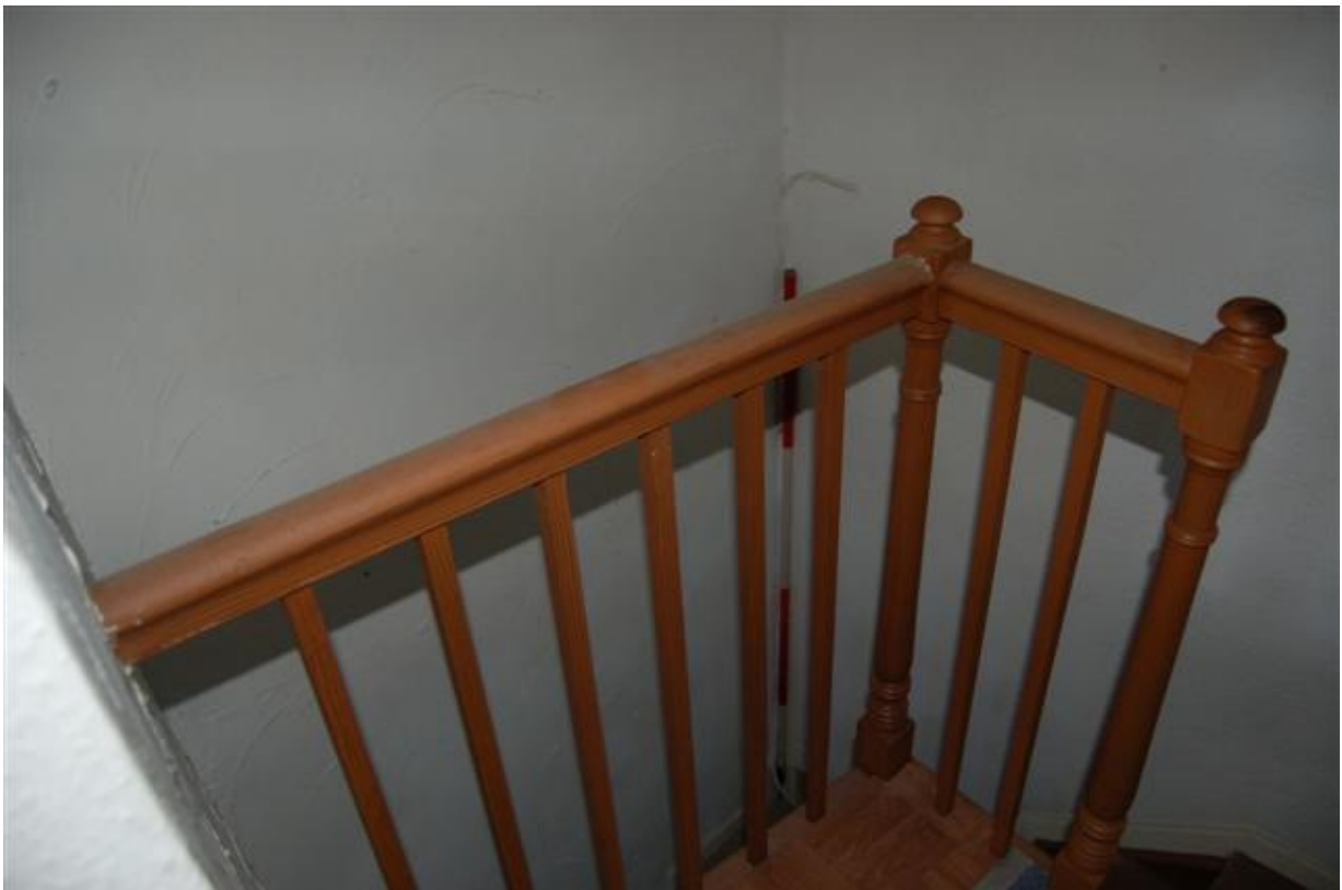
Plate 34: Building A, Block A4; Room AF7, stair.
