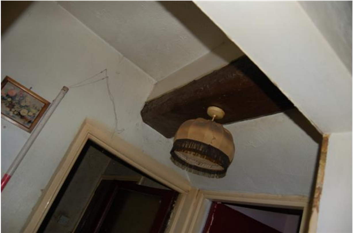
Plate 240: Building C, Block C1; Room CF4 ceiling beam.
