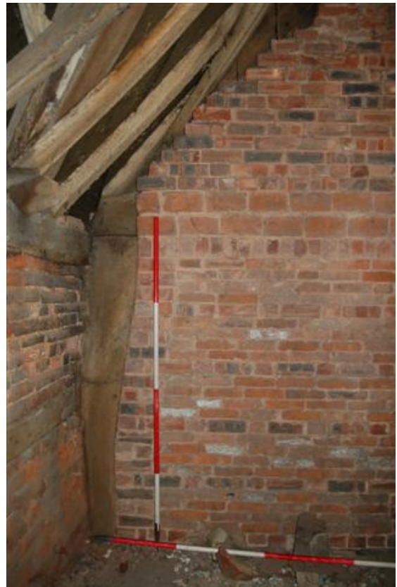
Plate 84: Building A, Block A6; Room AF14, N wall.
