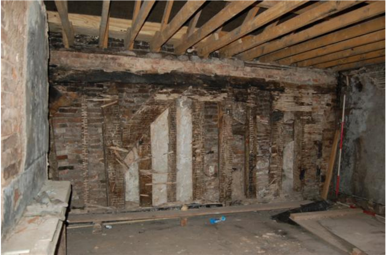
Plate 131: Building B, Block B1; Room BF1 north wall exposed framing.
