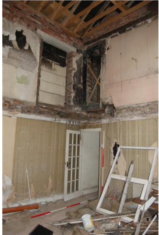
Plate 118: Bldg B, Block B1; Rm BG2/BF10 looking north-east.
