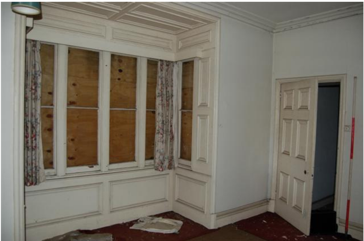
Plate 190: Building B, Block B6; Room BF17 looking north-east.
