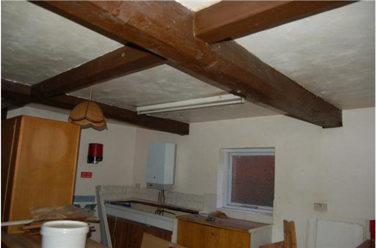
Plate 264: Building C, Block C2; Room CF11 ceiling structure.
