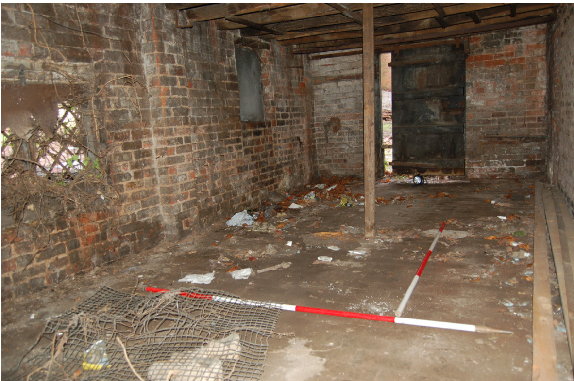
Plate 291: Building D, Room D5 interior looking east.
