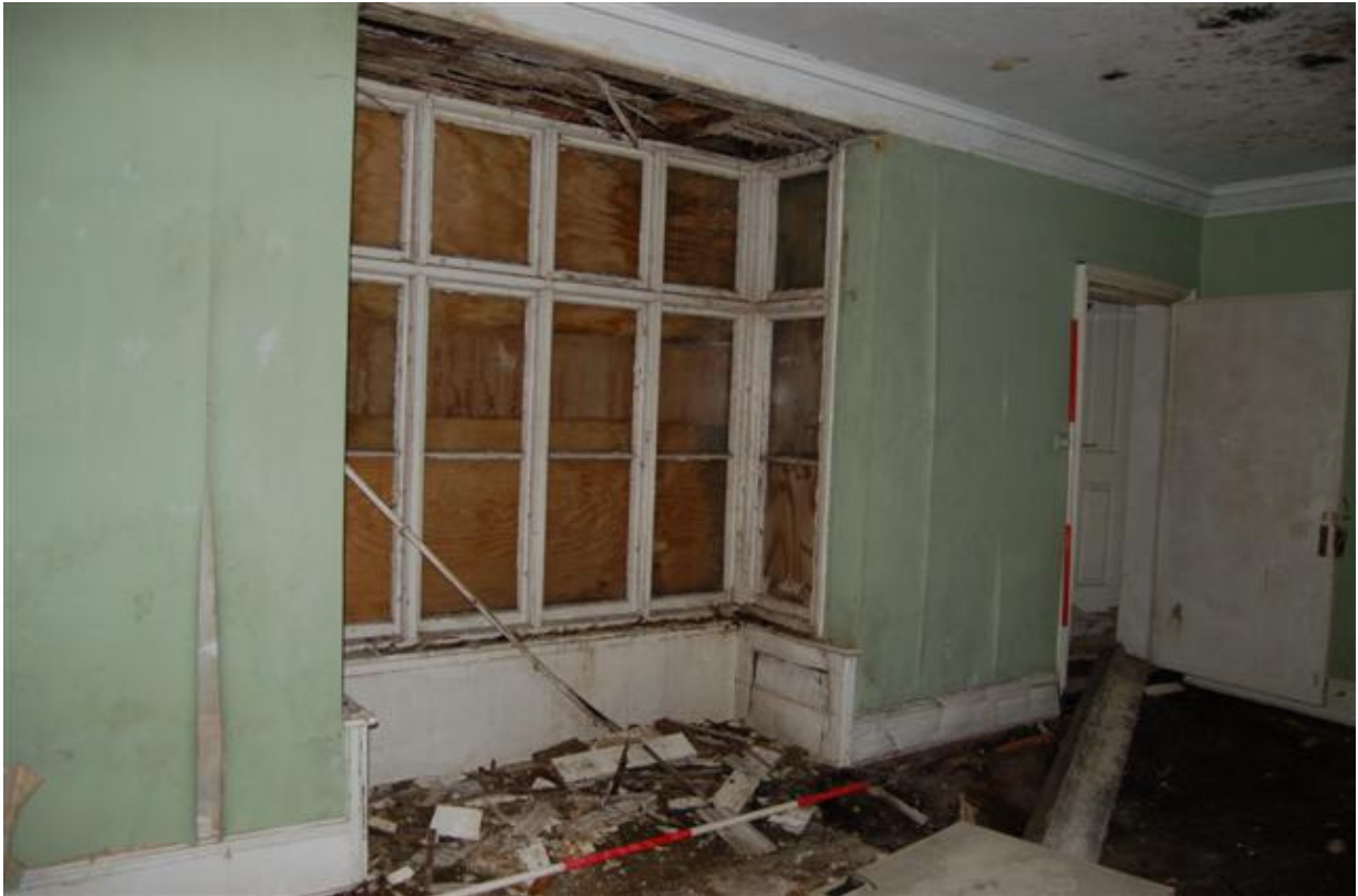
Plate 179: Building B, Block B5; Room BG16 looking north-east.
