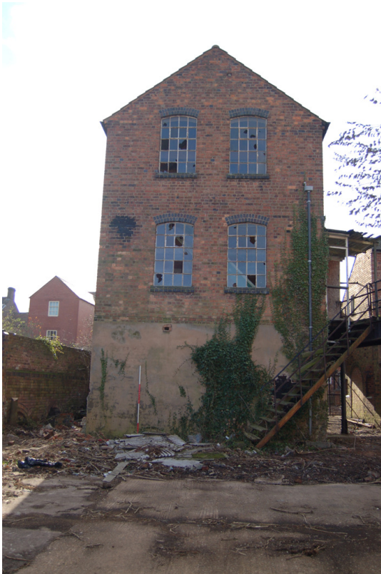
Plate 299: Building E, north elevation.
