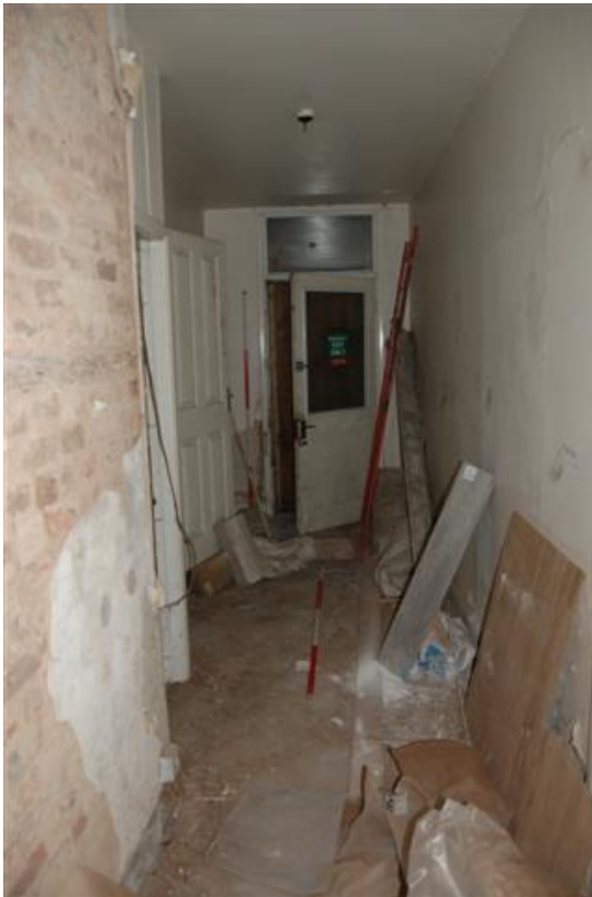
Plate 166: Bldg B, Block B4; Rm BG3 looking W.
