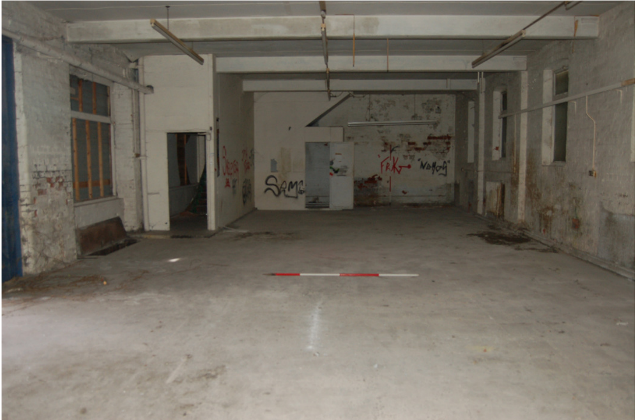
Plate 340: Building H, ground floor looking west.
