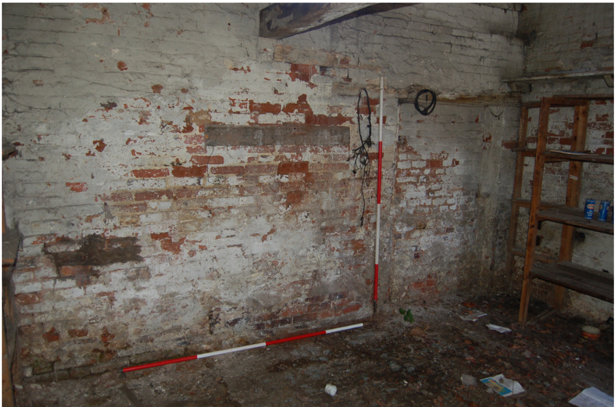
Plate 214: Building B, Block B7; Room BG25, south wall, blocked door.
