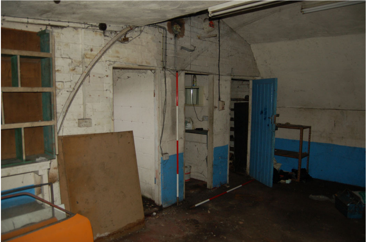
Plate 351: Building I, interior, south; note exposed semi-circular rib.
