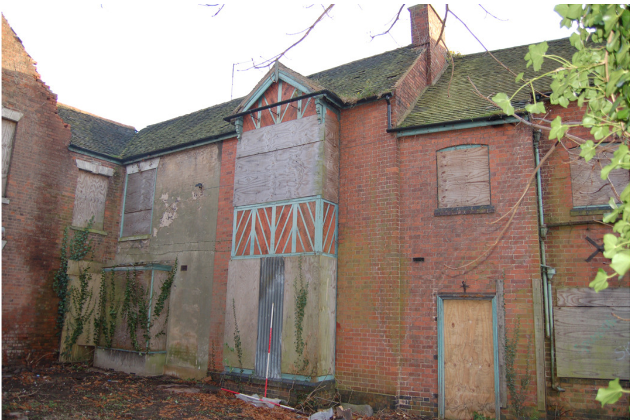
Plate 178: Building B Blocks B5 and B6 north elevation.
