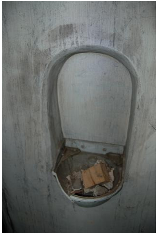
Plate 174: Bldg B, Block B4; Rm BF13 basin.
