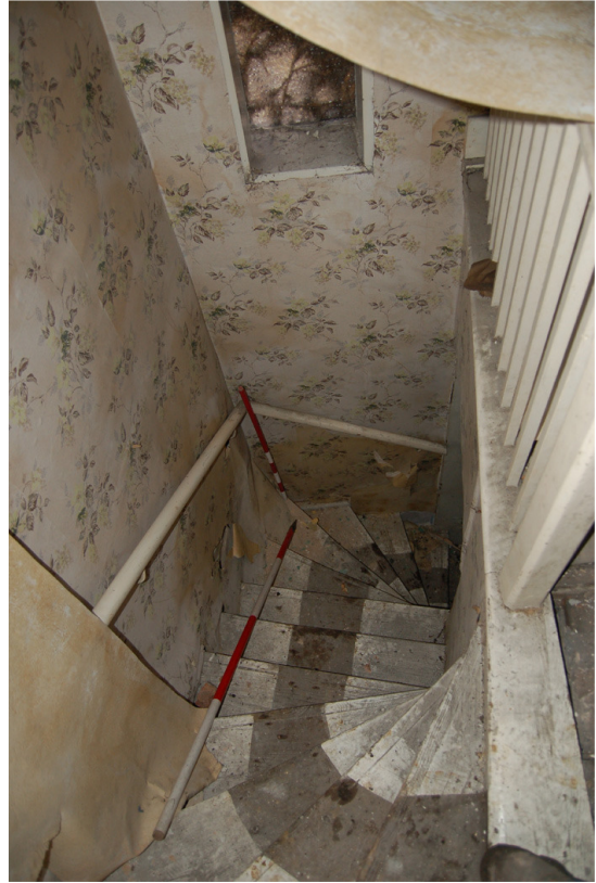
Plate 204: Bldg. B, Block B7; stair BG19/BF19.
