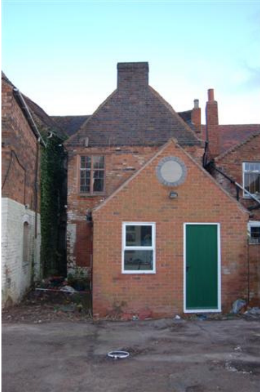
Plate 271: Bldg C, Blocks C4/5 west elevation.
