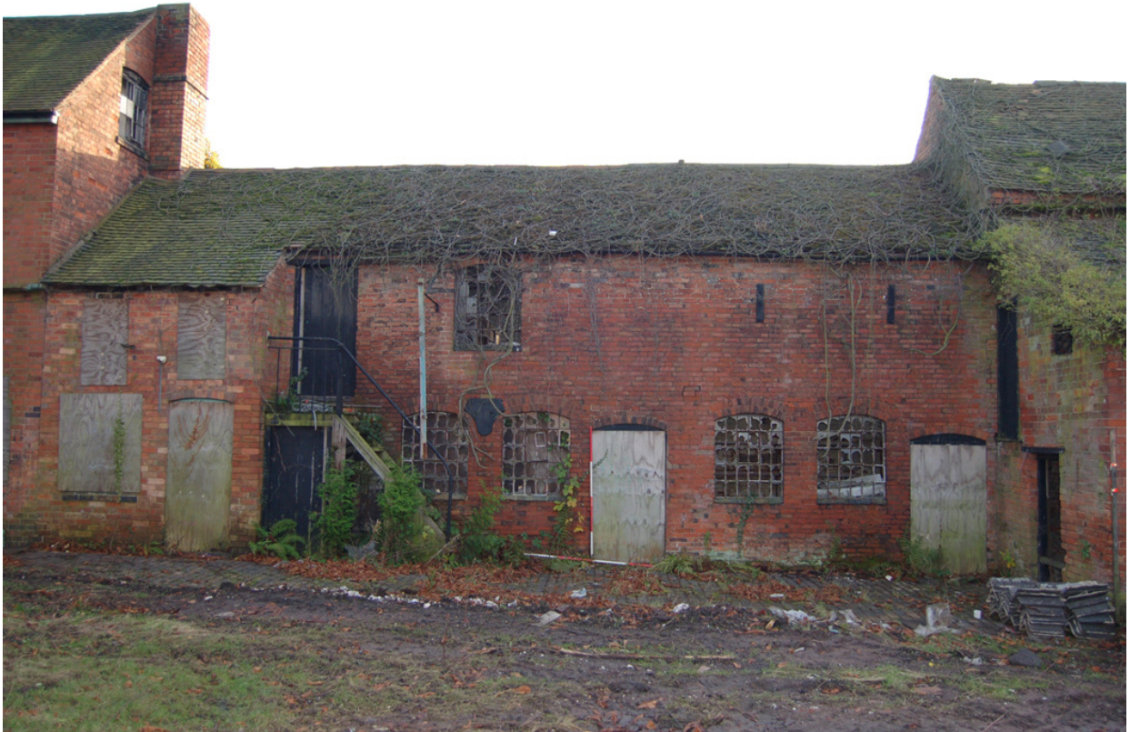
Plate 193: Building B; rear range north elevation, centre (Bldg. D to right).
