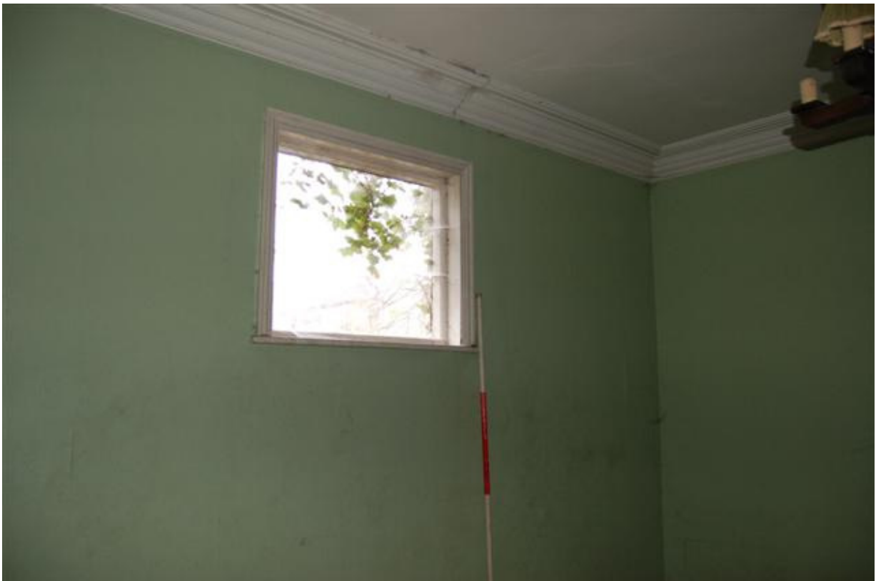
Plate 188: Building B, Block B6; Room BG17 looking south-west.
