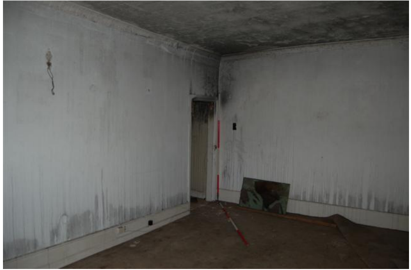
Plate 161: Building B, Block B3; Room BF11 looking north-east.
