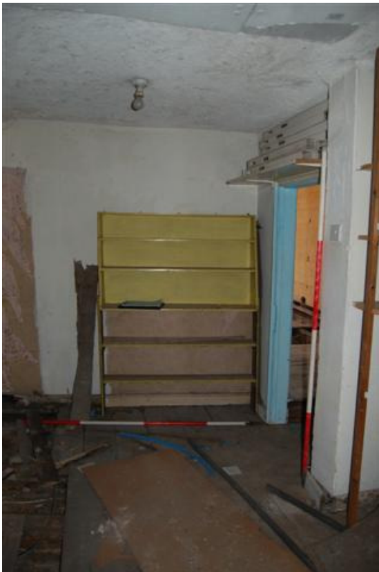
Plate 63: Bldg.A, Block A4; Rm AF12 looking W
