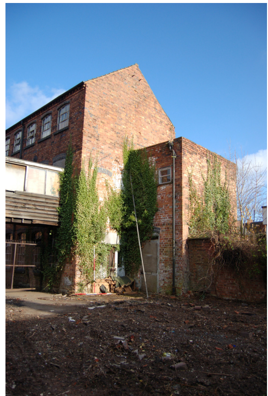
Plate 300: Building E, south elevation and stair.
