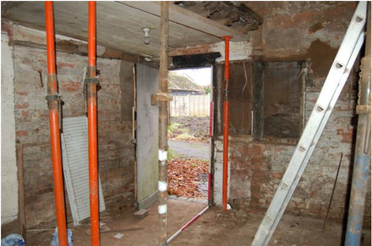
Plate 66: Building A, Block A5; Room AG12 looking north-west.
