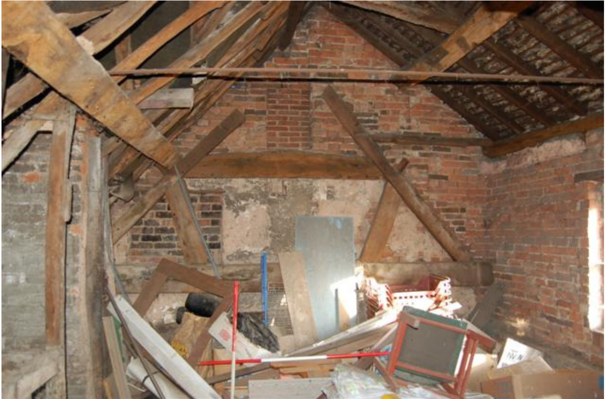
Plate 242: Building C, Block C1; Room CS1 roofspace looking north.
