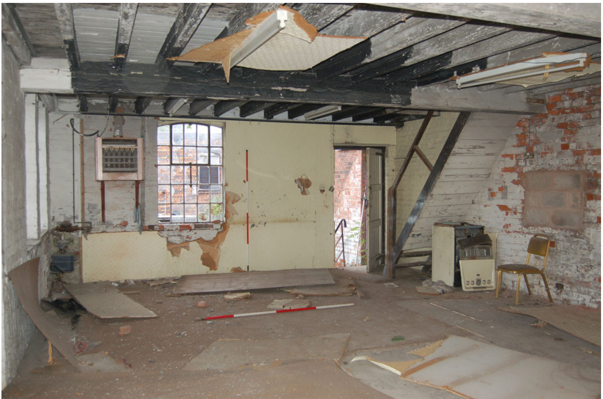
Plate 327: Building G, 1 st floor, looking north.
