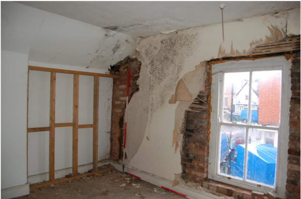
Plate 140: Building B, Block B1; Room BF3 looking north-east.
