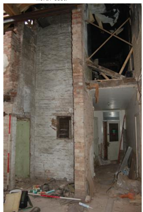
Plate 120: Bldg B, Block B1; Rm BG2/BF10 looking west.
