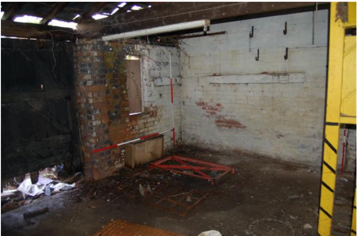
Plate 281: Building D, Room D3 looking north-east.
