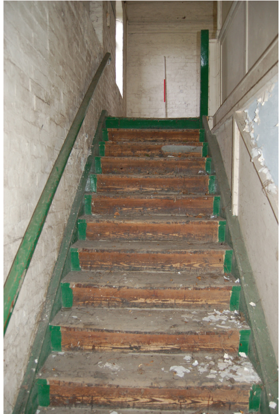
Plate 343: Building H, stair.
