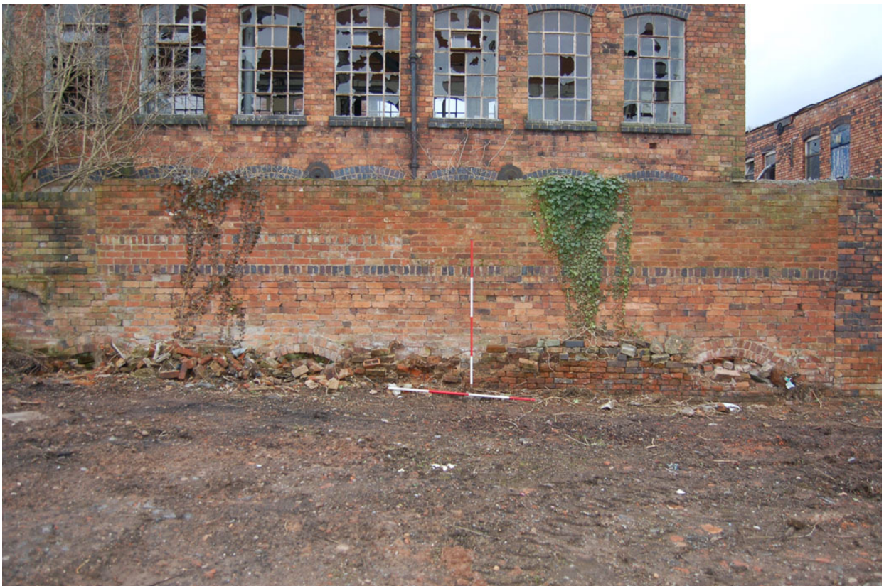
Plate 295: Boundary wall (central section) looking west.
