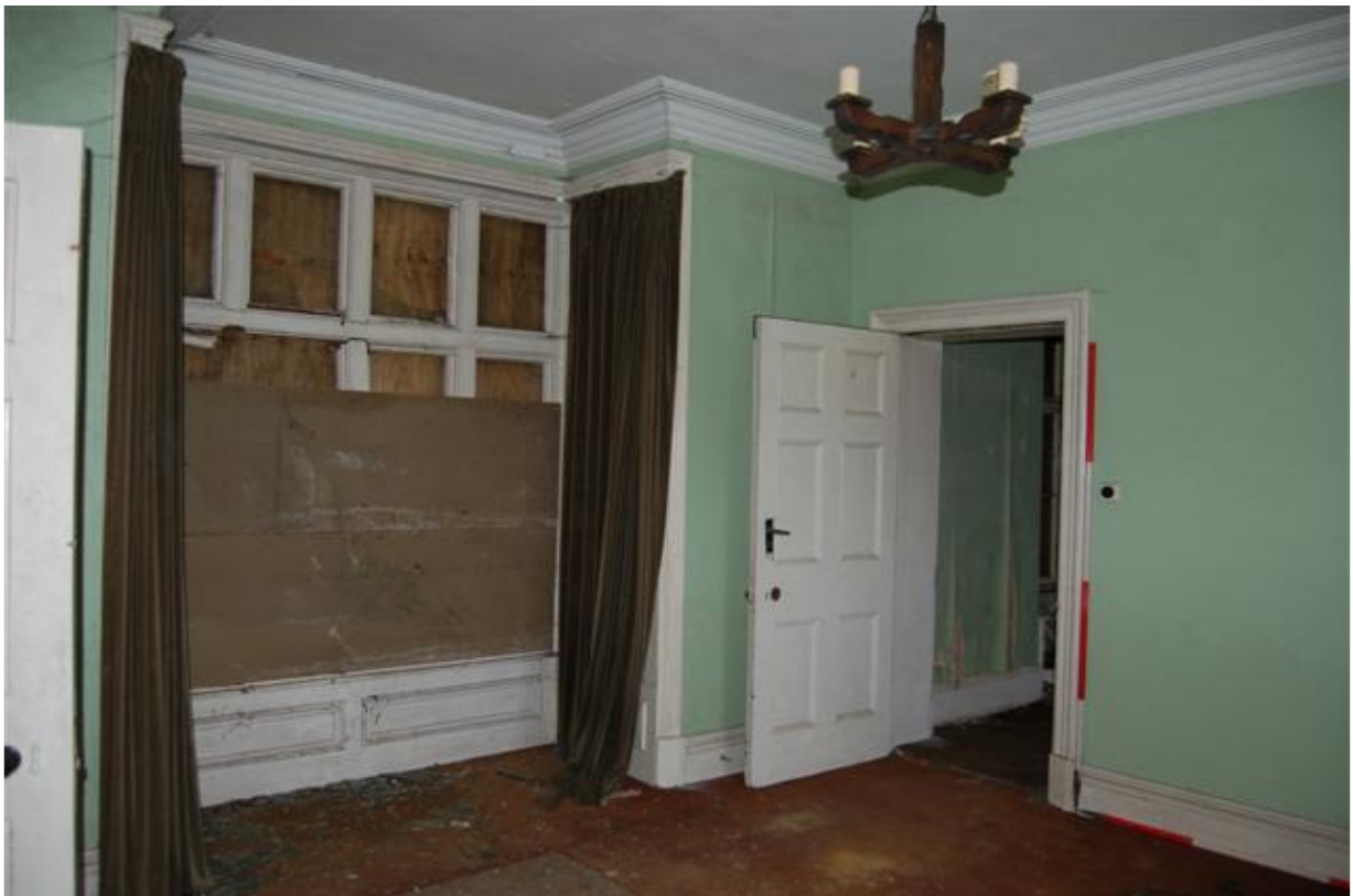
Plate 186: Building B, Block B6; Room BG17 looking north-east.
