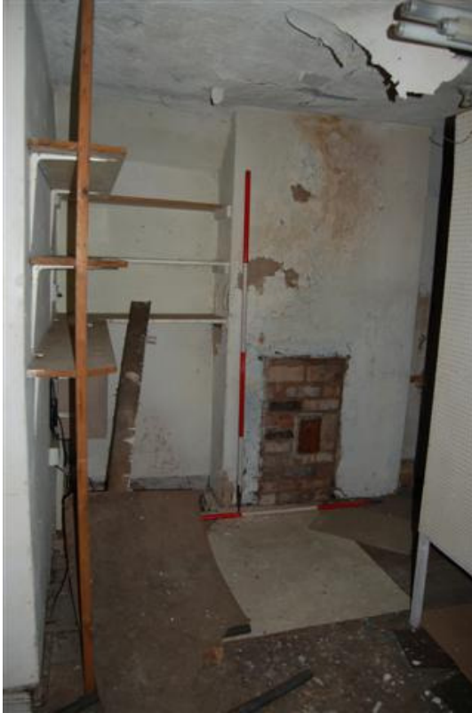
Plate 58: Bldg.A, Block A4; Rm AF8 looking S.
