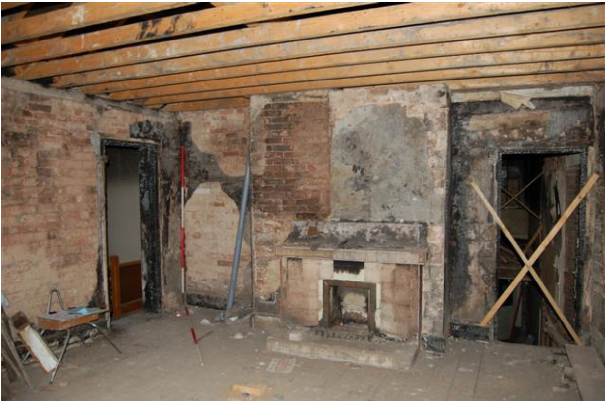
Plate 130: Building B, Block B1; Room BF1 west wall.
