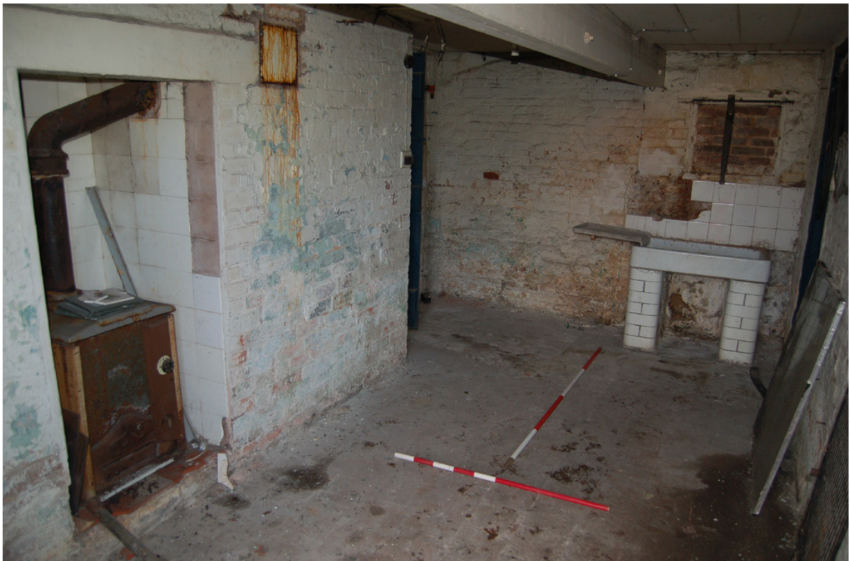
Plate 200: Building B, Block B7; Room BG21, looking south.
