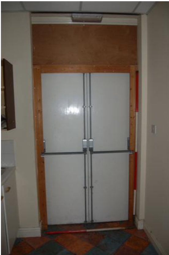
Plate 14: Building A, Block A2; Rm AG3 doorway.
