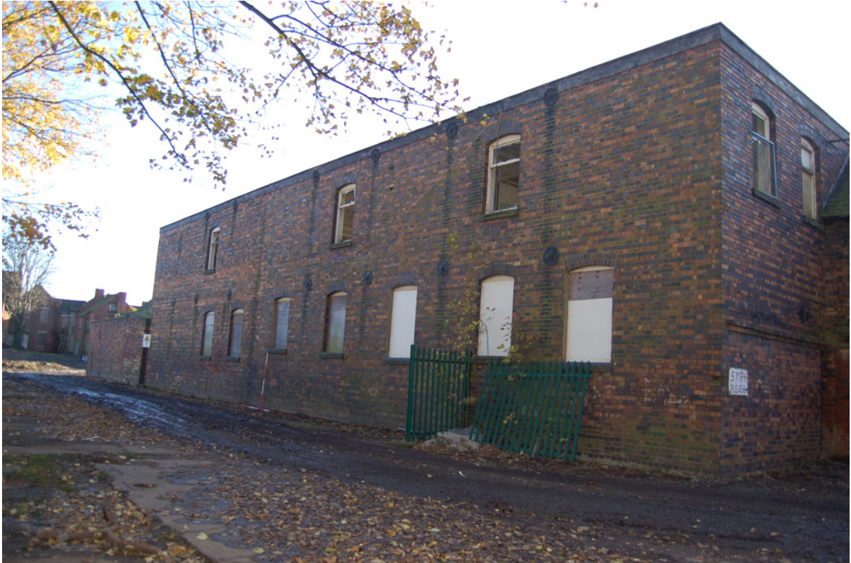
Plate 336: Building H, north elevation.
