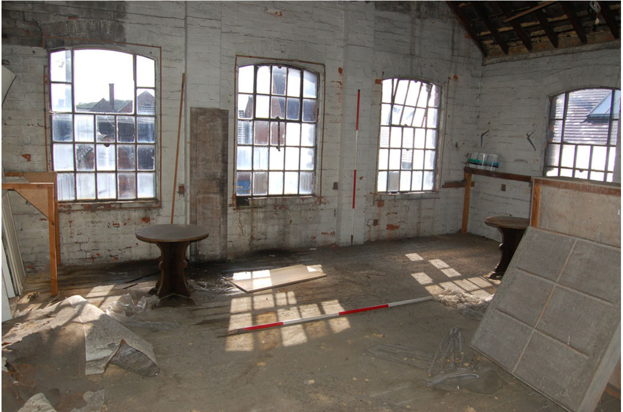
Plate 328: Building G, 2 nd floor looking south.
