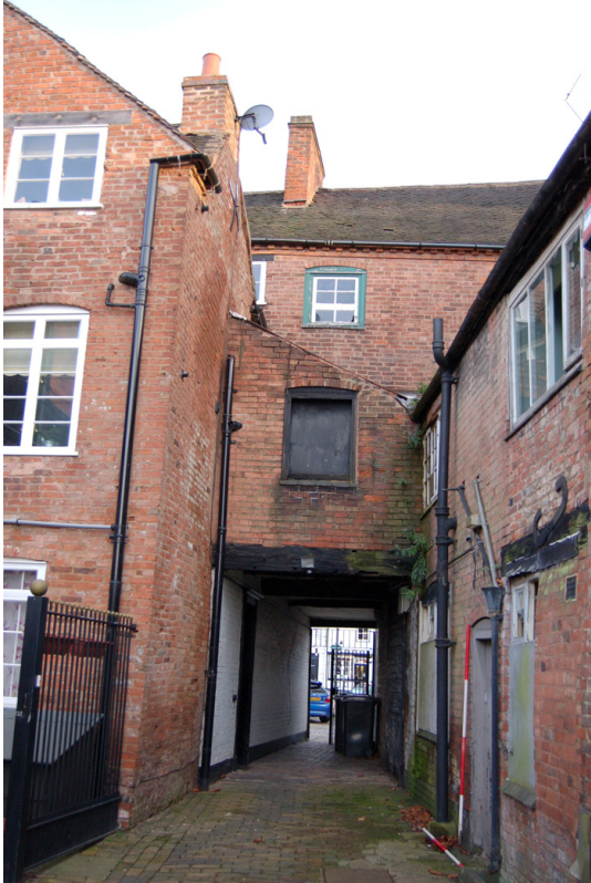
Plate 24: Building A Block A3 (No.16) rear elevation.
