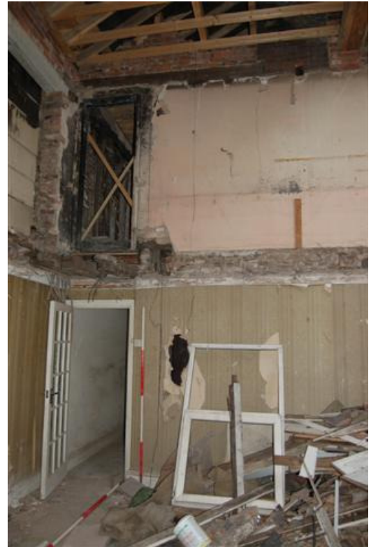
Plate 122: Bldg B, Block B1; Rm BG2/BF10 looking east.
