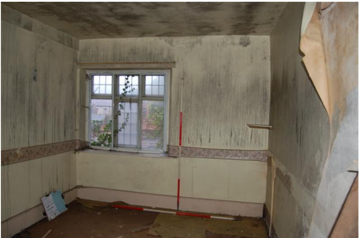
Plate 164: Building B, Block B3; Room BF12 looking west.
