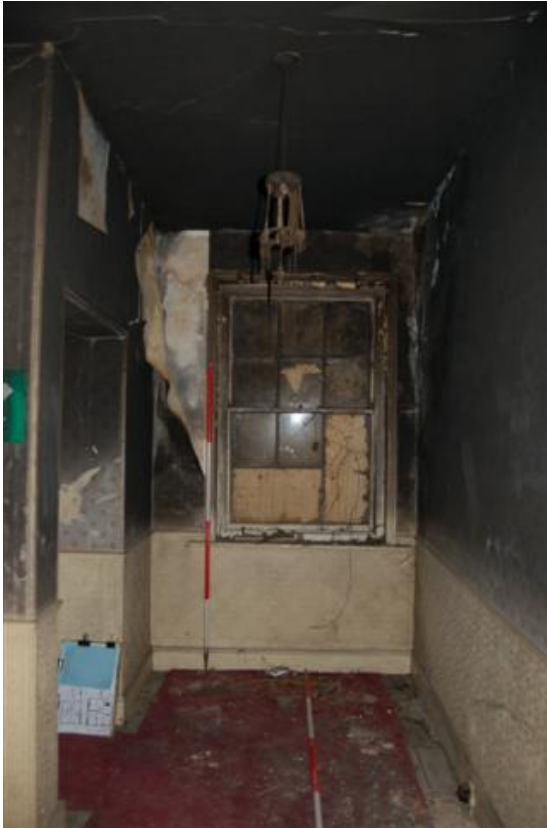
Plate 171: Bldg B, Block B4; Rm BF14 looking W.
