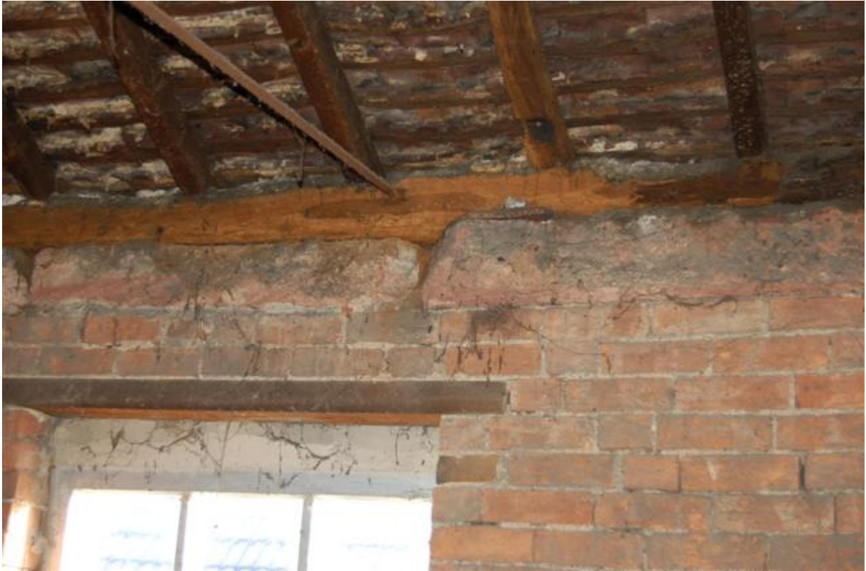
Plate 244: Building C, Block C1; Room CS1 detail of east wall.
