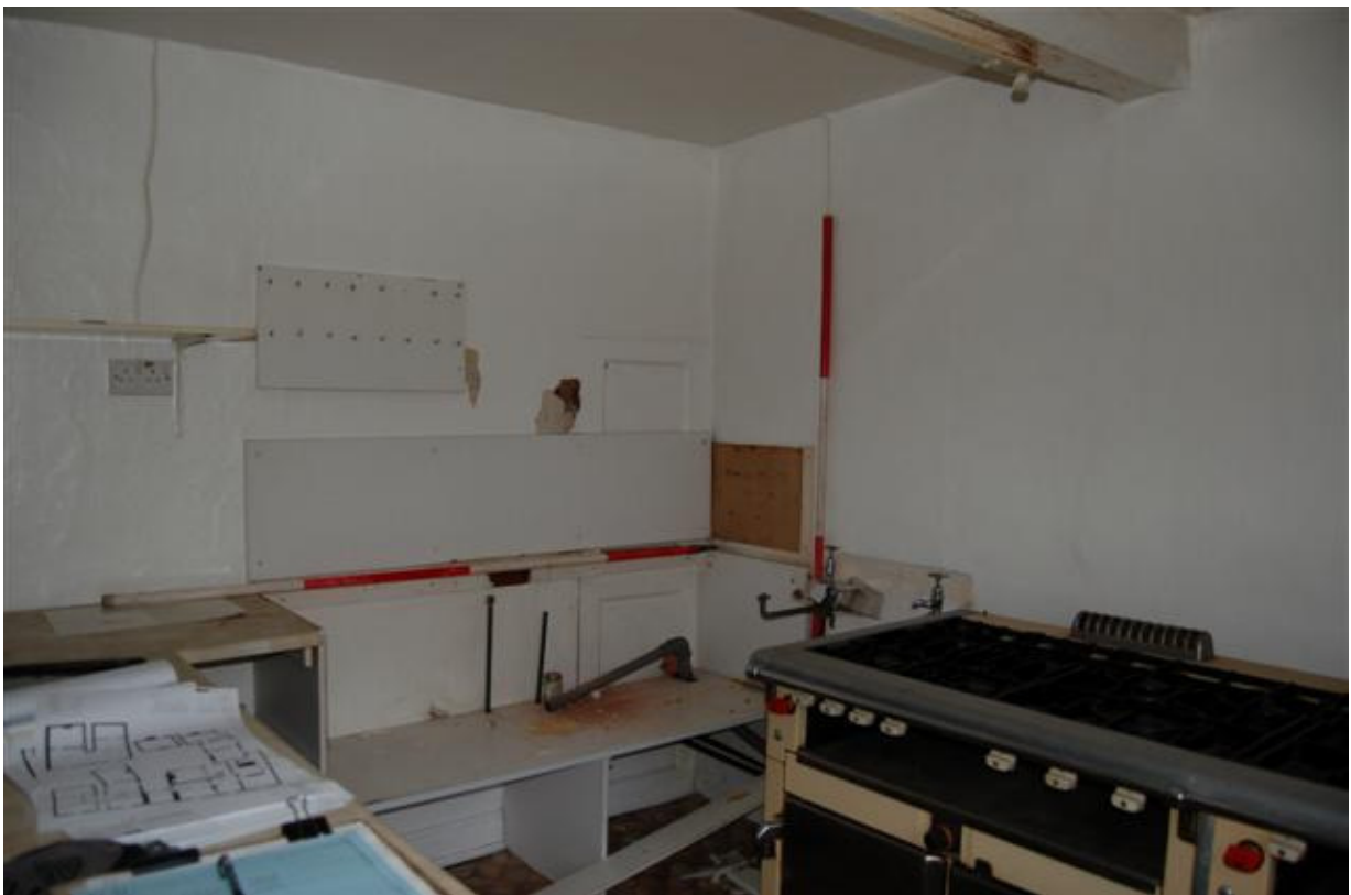
Plate 232: Building C, Block C1; Room CF1 looking north-west.
