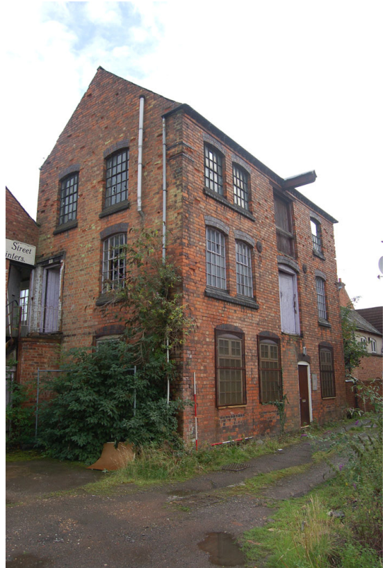
Plate 323: Building G, exterior looking SE.
