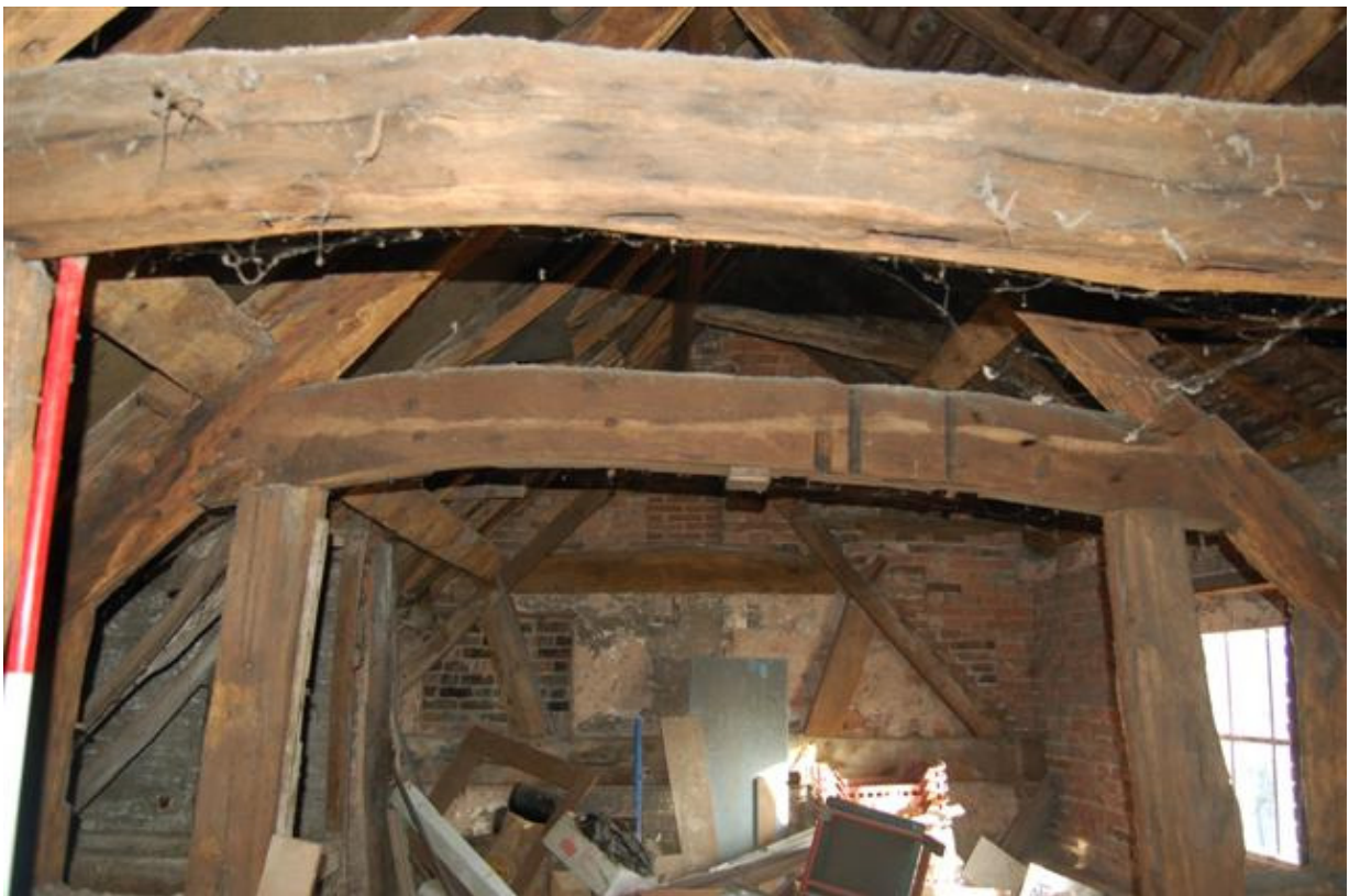
Plate 247: Building C, Block C1; Room CS1 roofspace looking north.
