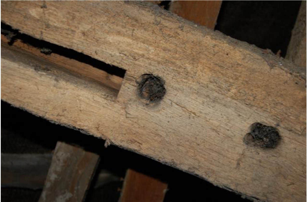
Plate 92: Building A, Block A6; Room AF14, detail of east wallplate soffit, stud mortise and stave holes.
