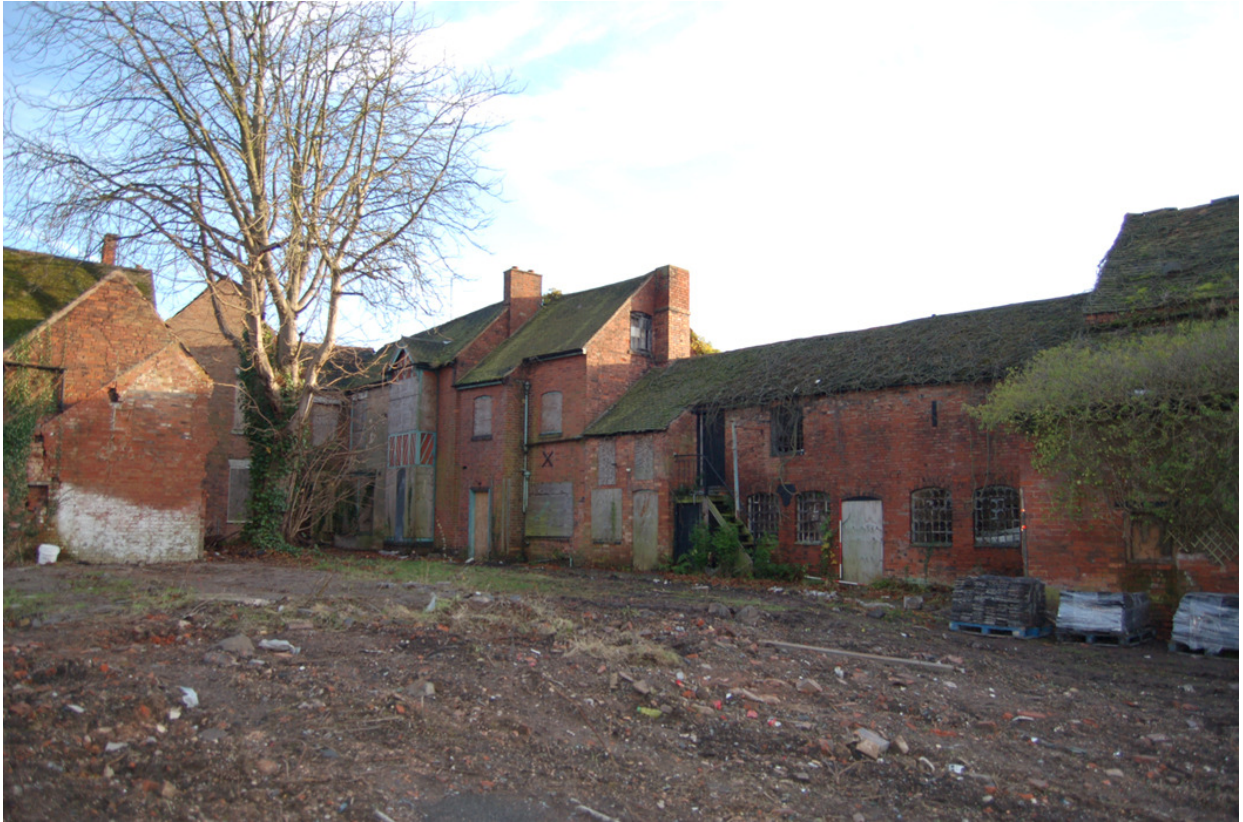
Plate 175: Building B; rear range north elevation (Bldg. D to right).
