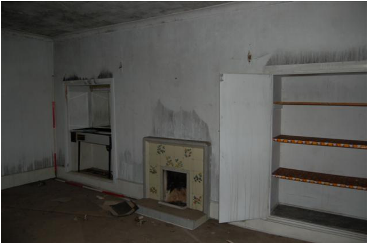
Plate 162: Building B, Block B3; Room BF11 looking south-east.
