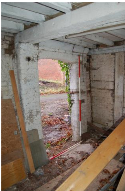
Plate 98: Bldg. A, Block A7; Rm AG14 looking NE.
