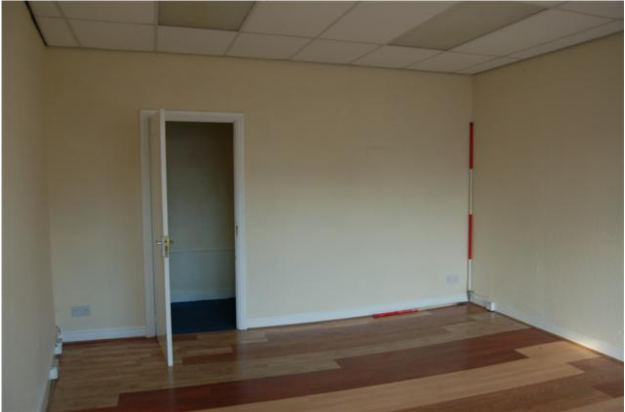
Plate 26: Building A, Block A3; Room AG5 looking west.
