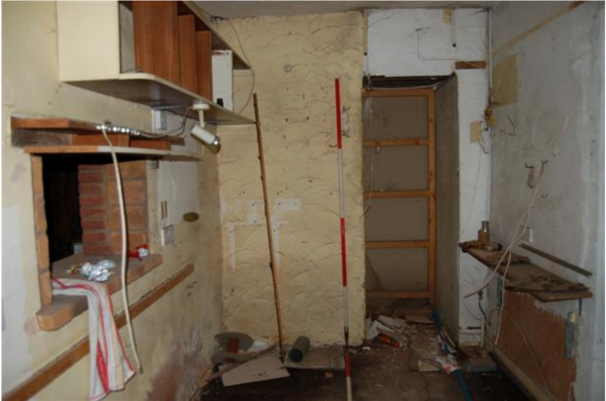
Plate 51: Building A, Block A4; Room AG8 looking south.
