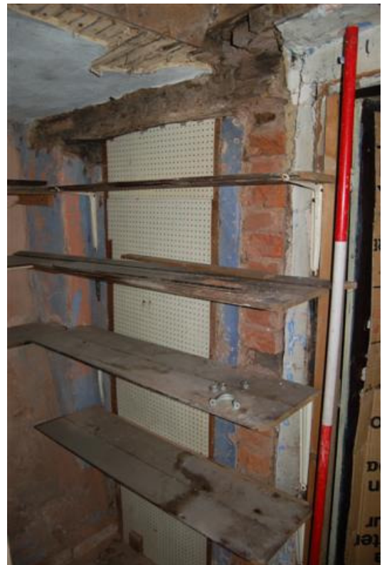
Plate 73: Bldg. A, Block A5; Rm AF13
