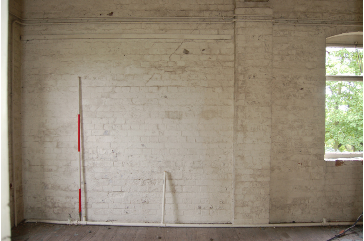
Plate 347: Building H, 1 st floor' scar of former stair at Bay 9, (north).
