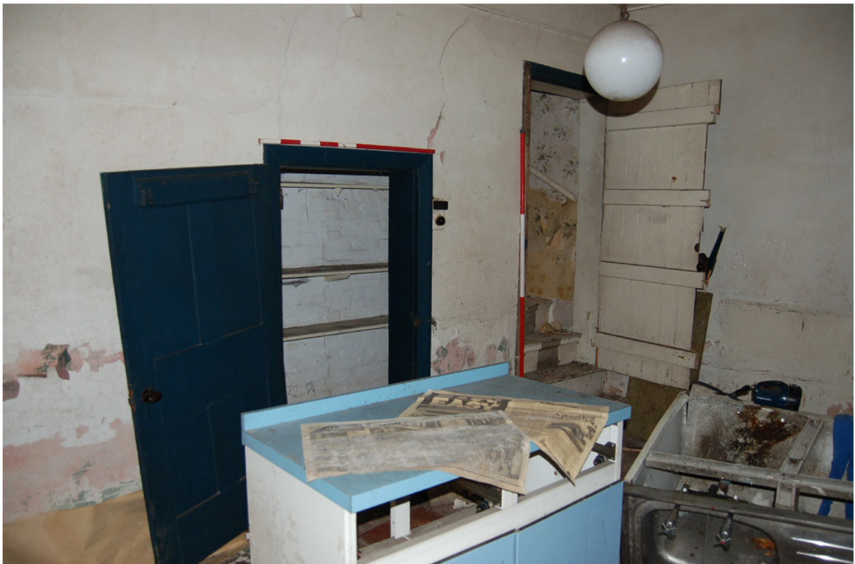
Plate 202: Building B, Block B7; Room BG20, looking south-east.
