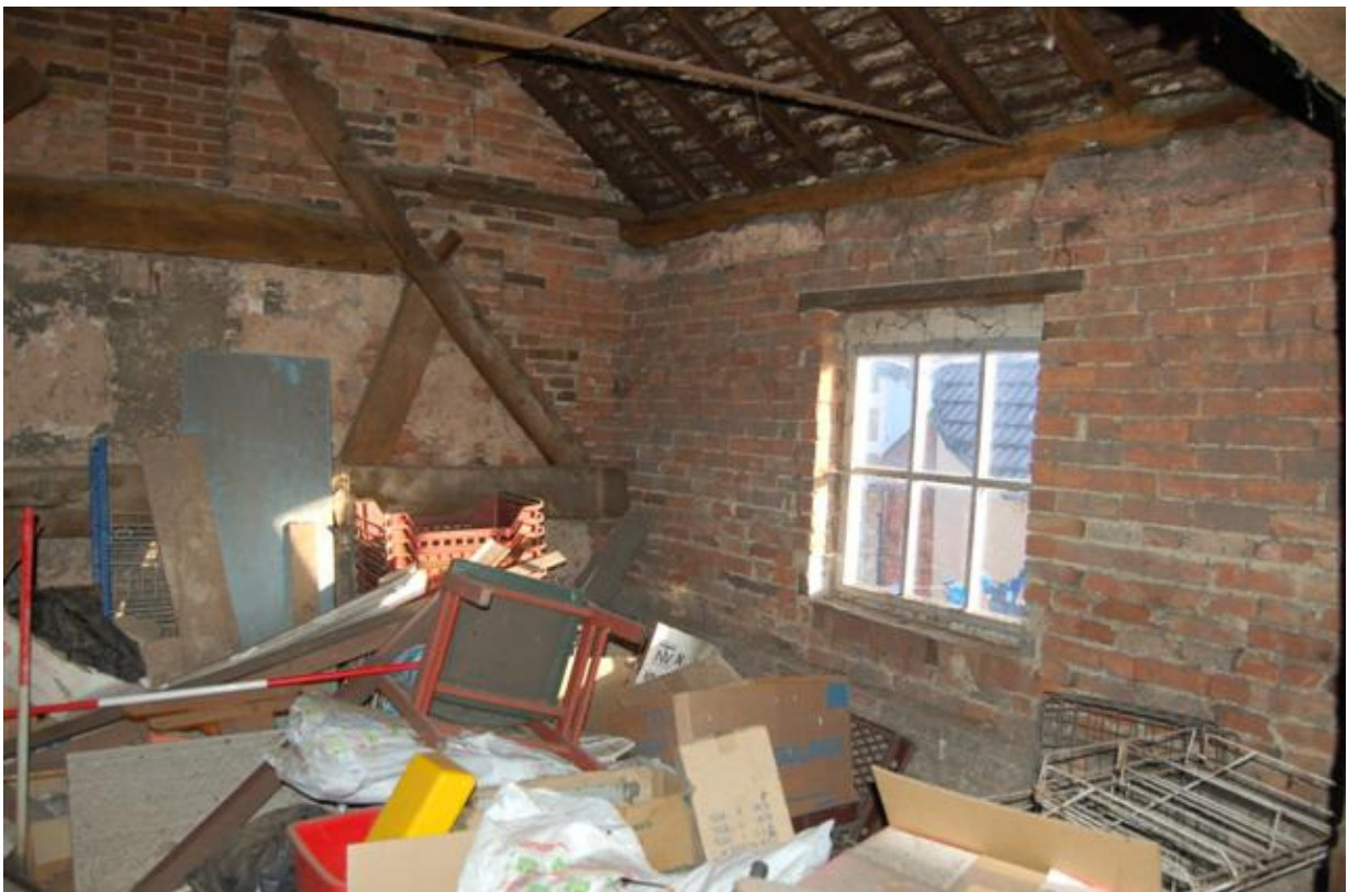
Plate 243: Building C, Block C1; Room CS1 roofspace looking north-east.
