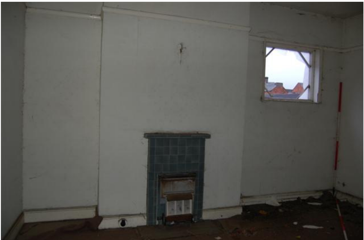
Plate 184: Building B, Block B5; Room BF16 looking south-west.
