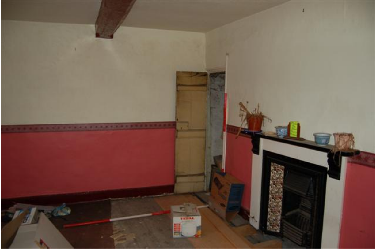
Plate 238: Building C, Block C1; Room CF3 looking south-west.
