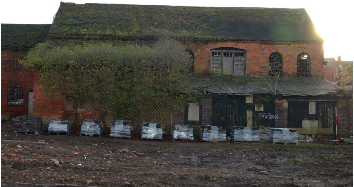
Plate 274: Building D, north elevation.
