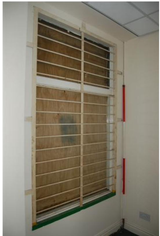
Plate 15: Building A, Block A2; Rm AG4 window.
