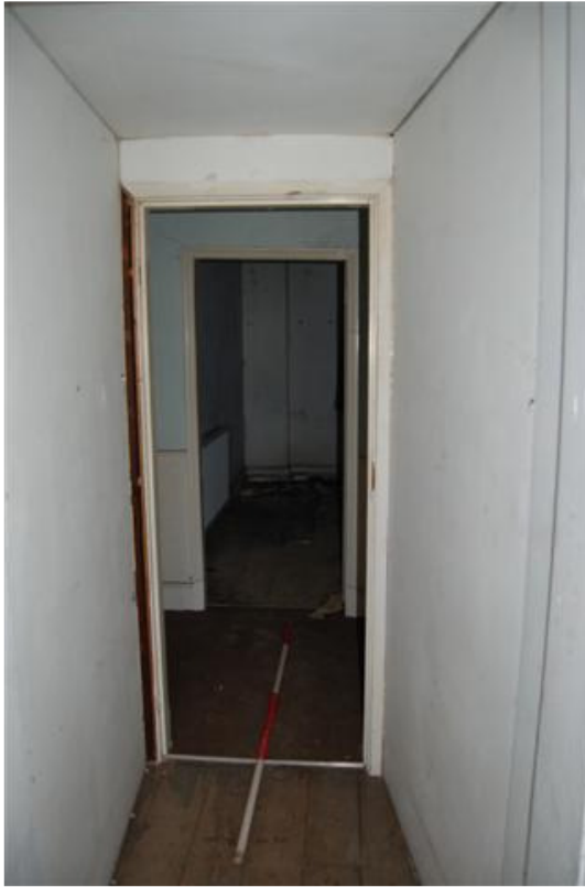
Plate 16: Bldg A, Block A2; Rm AF2 from east.
