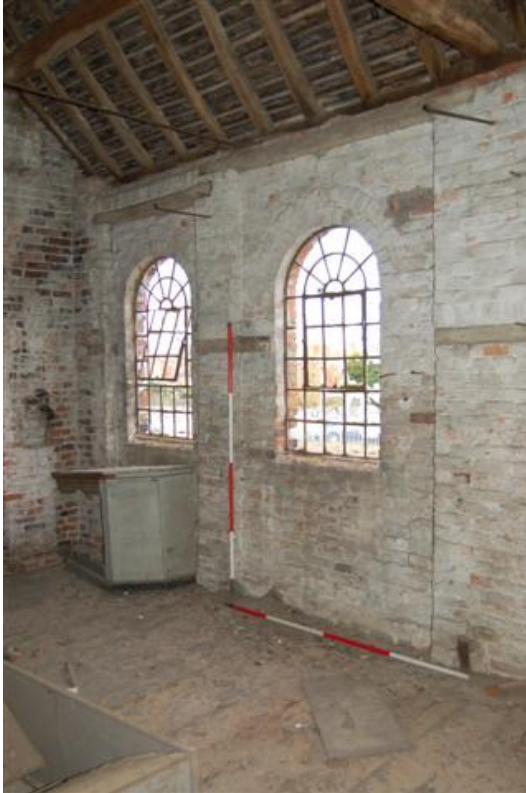
Plate 287: Bldg D, Rm D7 looking north-west.
