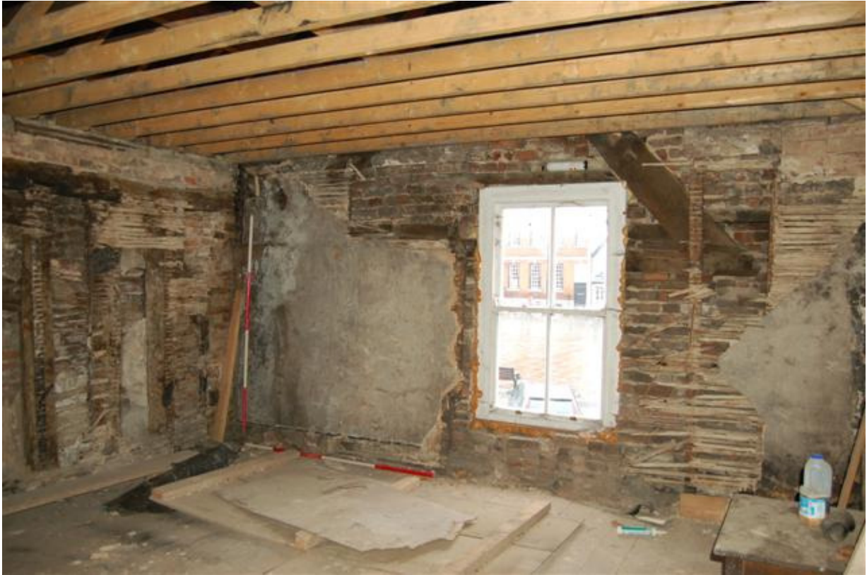
Plate 133: Building B, Block B1; Room BF1 looking north-east.
