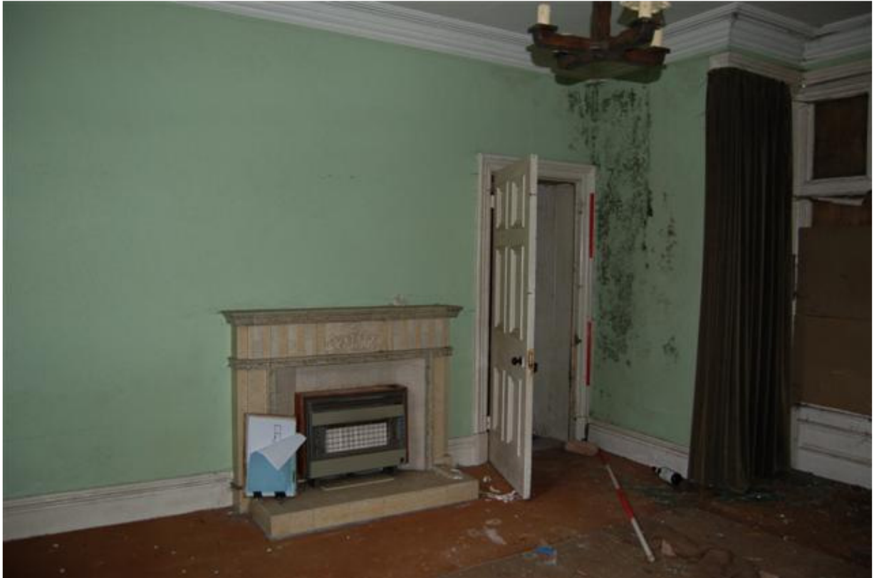
Plate 187: Building B, Block B6; Room BG17 looking north-west
