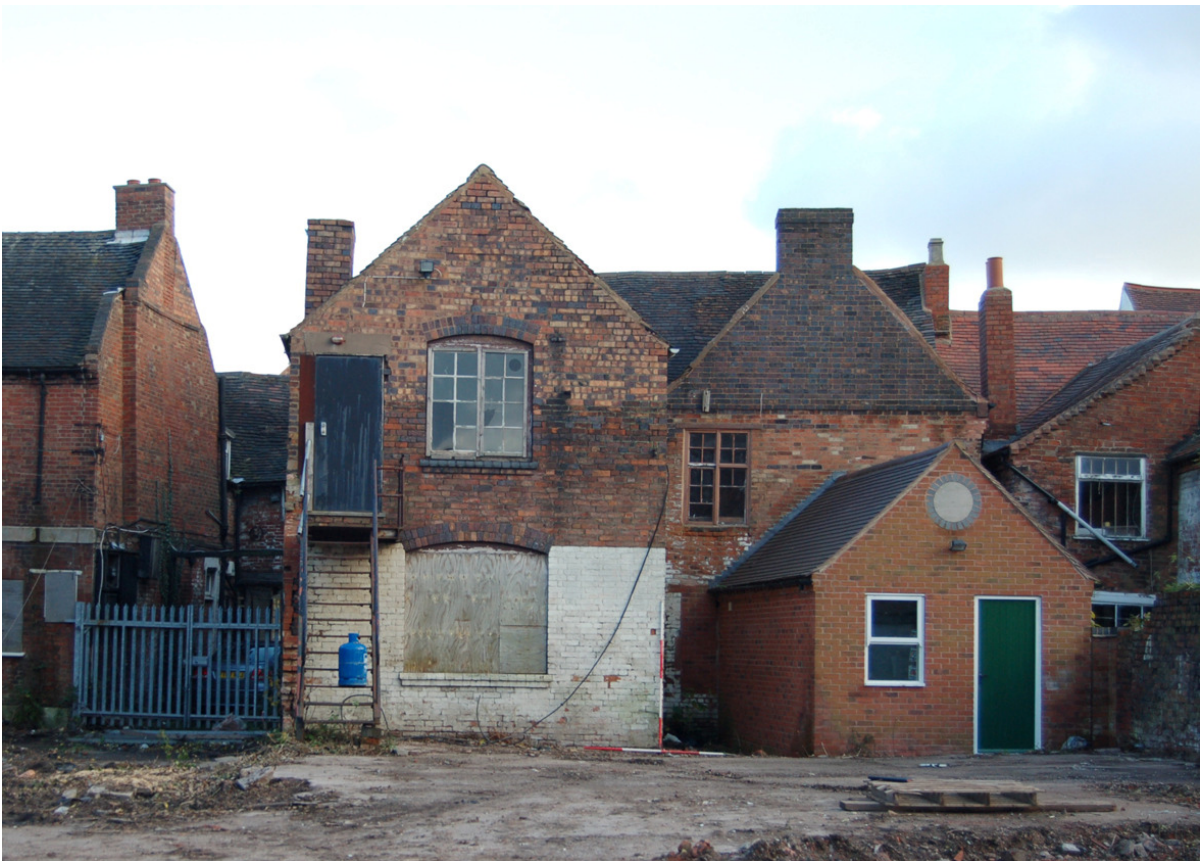
Plate 254: Building C, rear elevation from west.
