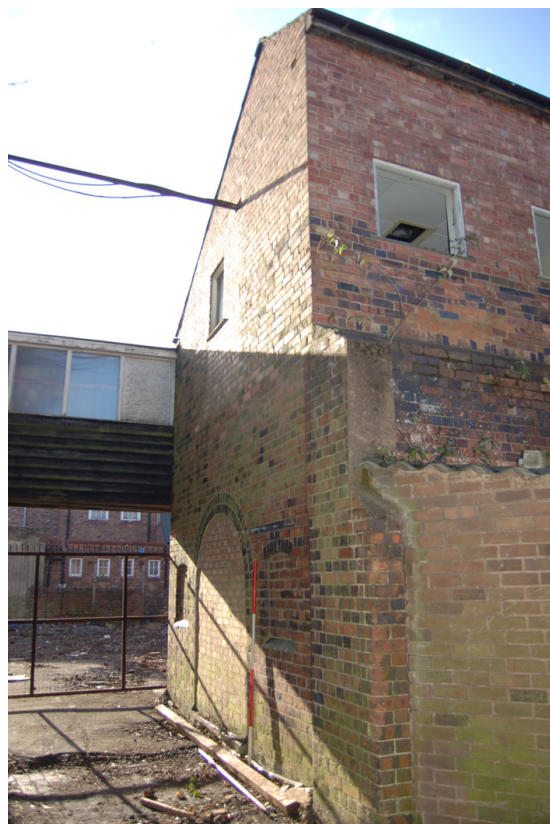
Plate 313: Building F, east elevation (oblique).
