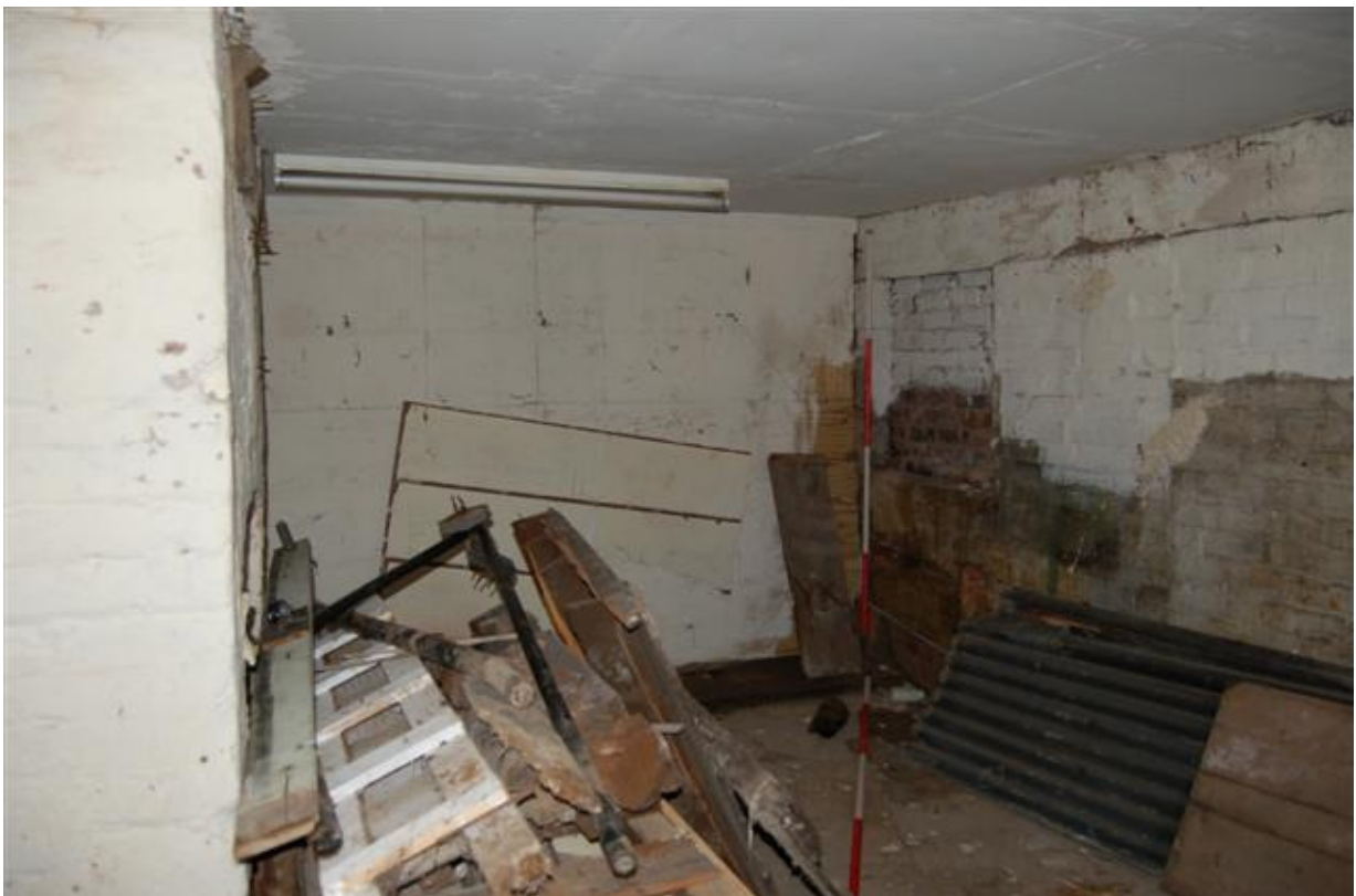
Plate 79: Building A, Block A6; Room AG13 looking west.
