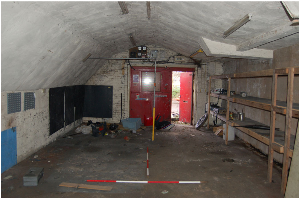
Plate 350: Building I (Room I1), interior looking north.
