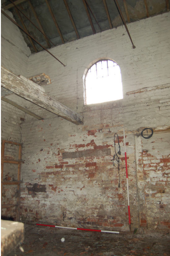
Plate 215: Bldg B, Block B7; Rm BG25, north wall window.
