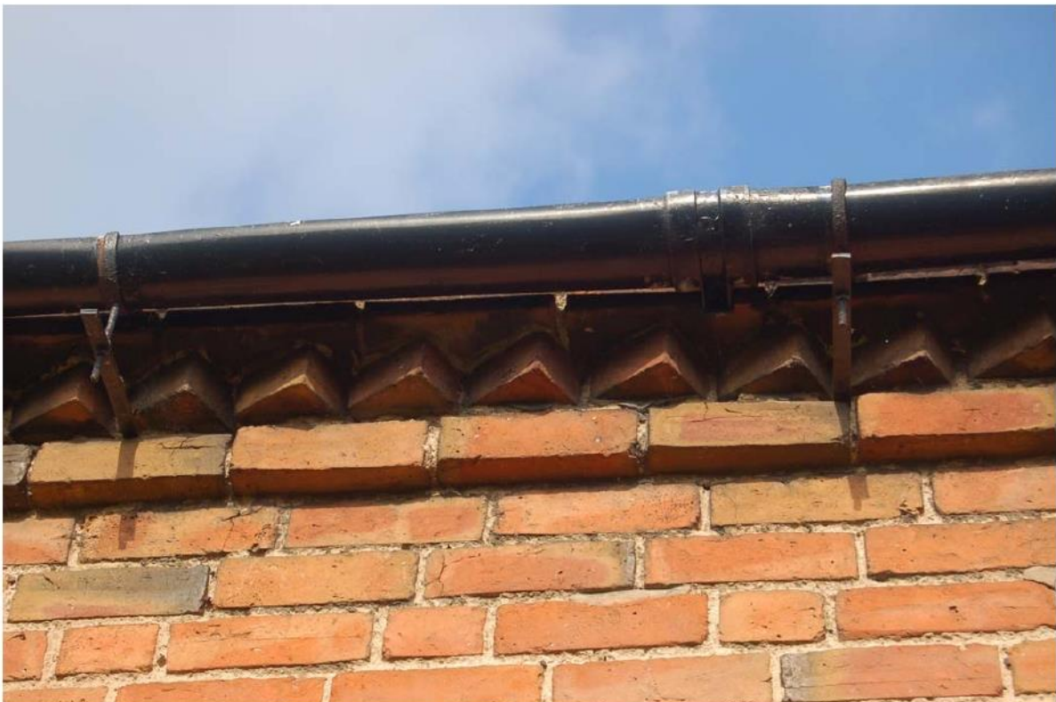
Plate 14: Detail of projecting string and dog-tooth eaves band.
