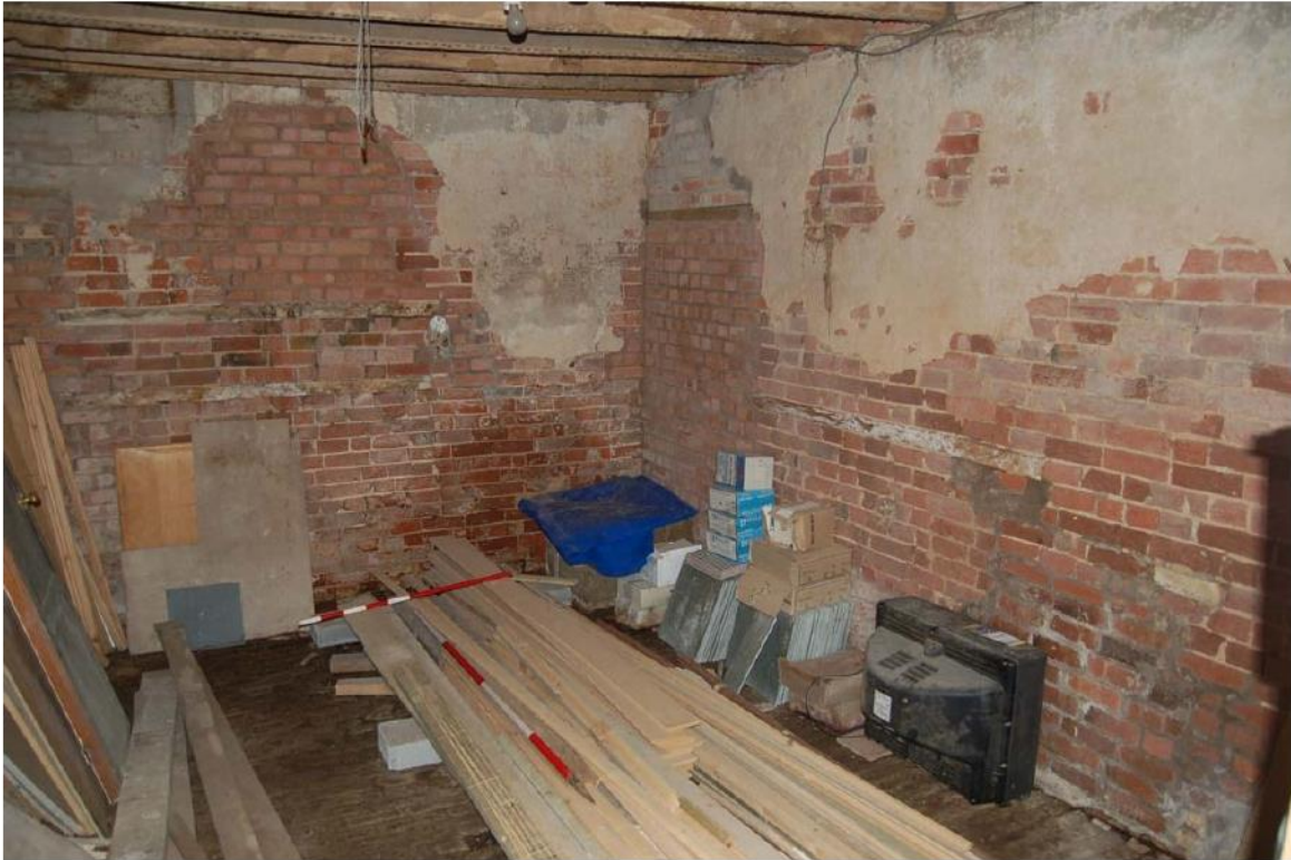
Plate 33: South range, interior; Room GF03 looking north-west, NB. blocked window (left) and door (right).
