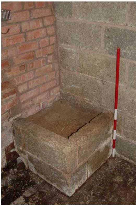
Plate 36: GF04 Breeze-block 'trough' to NE corner.
