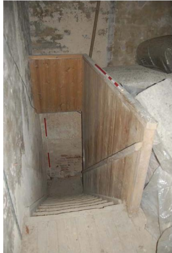
Plate 25: 1F01 - GF01 stair detail.
