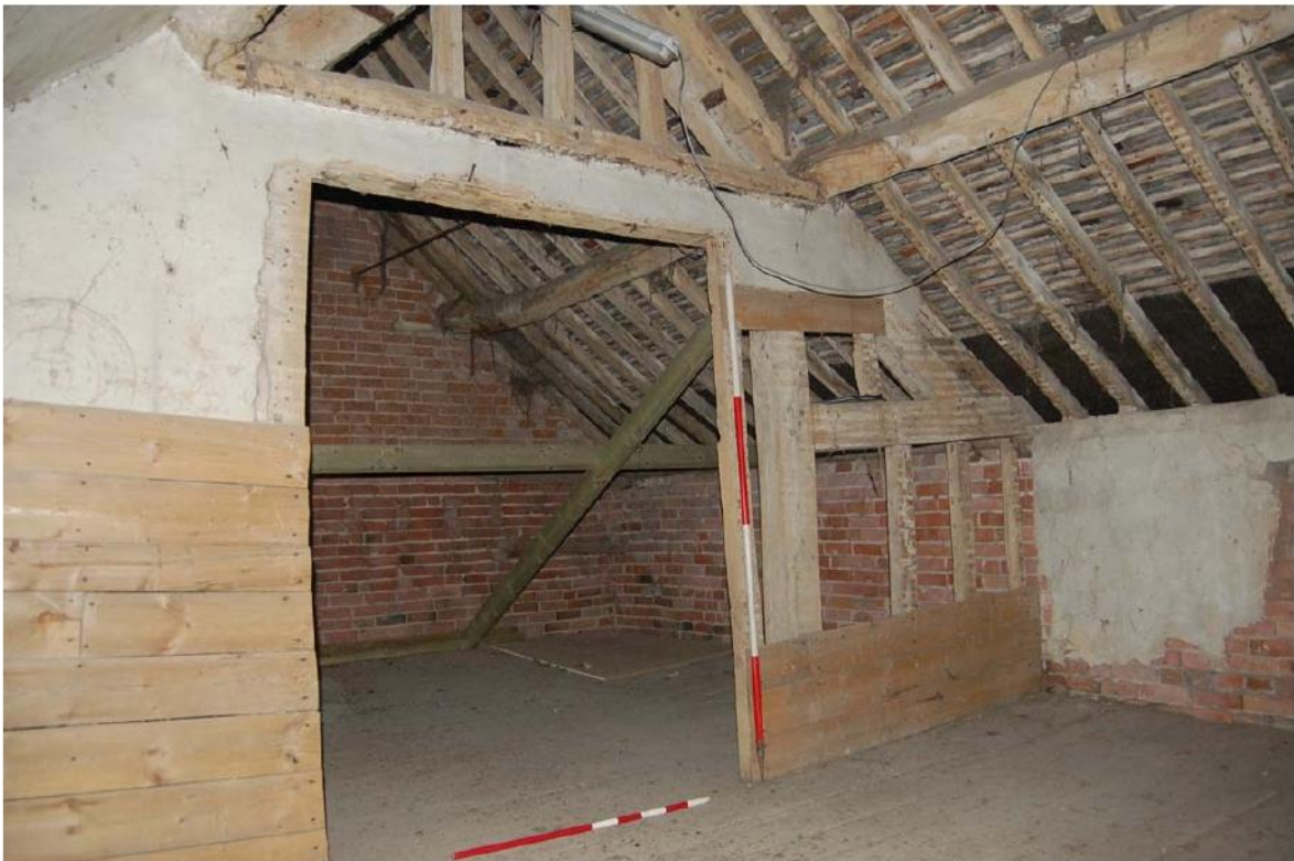
Plate 39: North range, interior; Room 1F03 central truss looking south-west.
