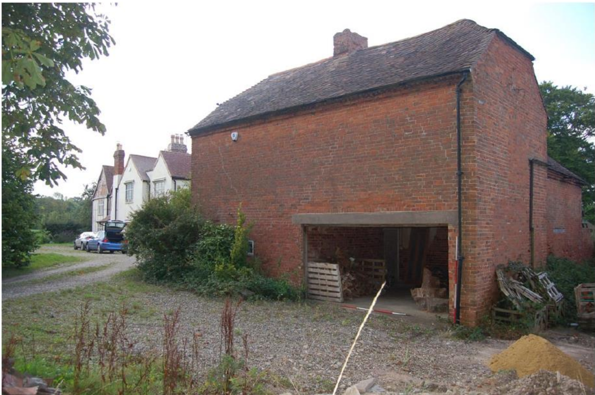
Plate 4: Contextual view from the north-west, Hill Top Farmhouse to left.
