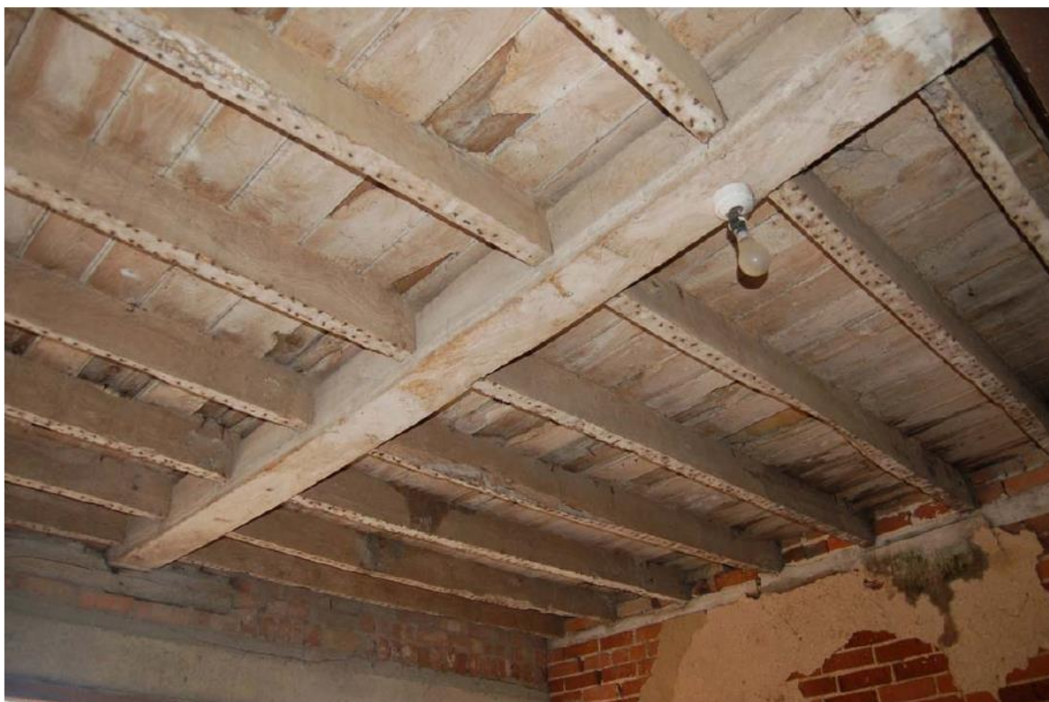
Plate 23: North range, interior; Room GF02 ceiling structure.
