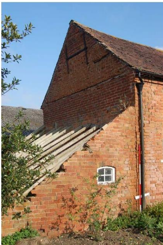
Plate 9: South range, south elevation.
