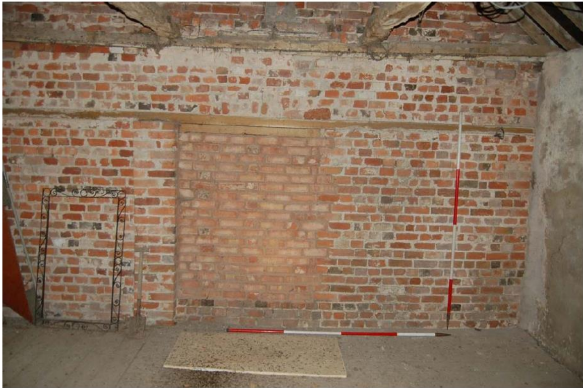
Plate 30: North Range, interior; Room 1F02 looking west; note central window/pitching door.
