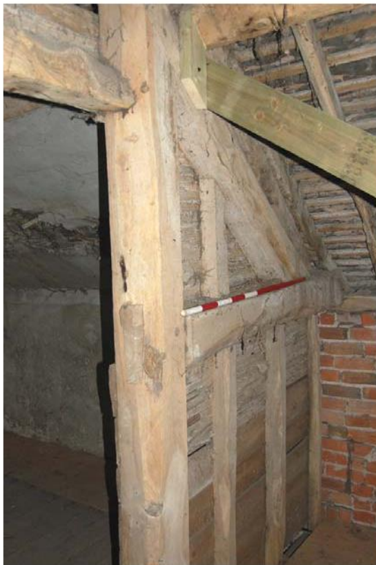
Plate 42: Room 1F03, interrupted tie.
