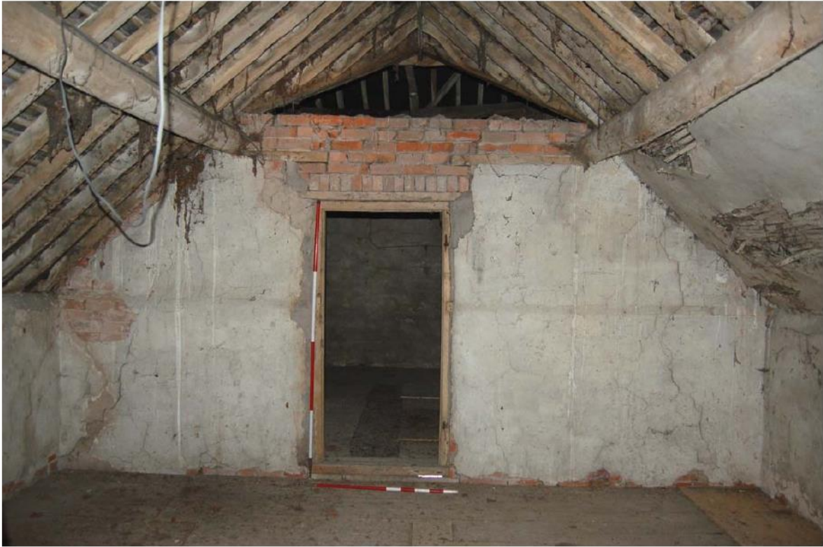
Plate 38: North range, interior; Room 1F03 looking north.
