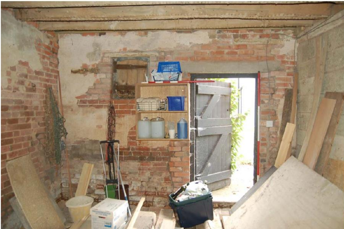
Plate 34: South range, interior; Room GF03 looking east.
