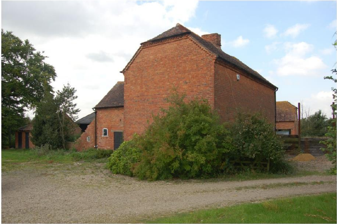
Plate 3: General view from the east.
