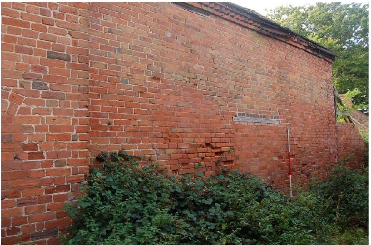
Plate 12: South range, west elevation blocked windows and central door.
