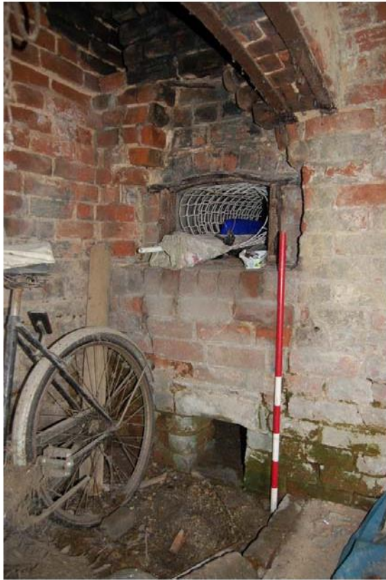
Plate 17: GF01; detail of bread oven.
