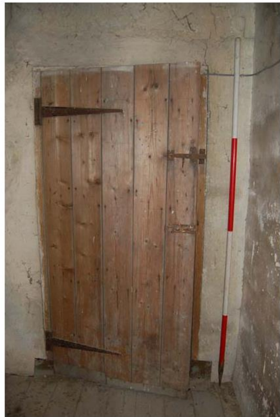
Plate 29: Room 1F01; door to 1F02.
