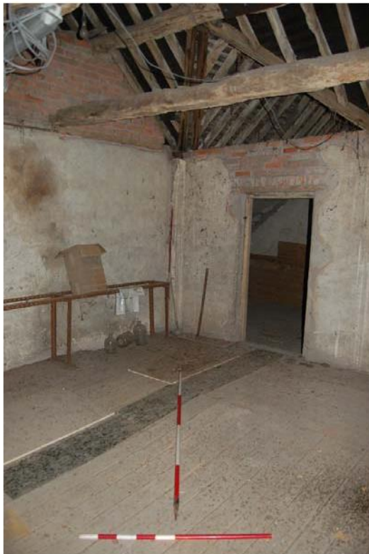
Plate 31: 1F02 looking south-east.
