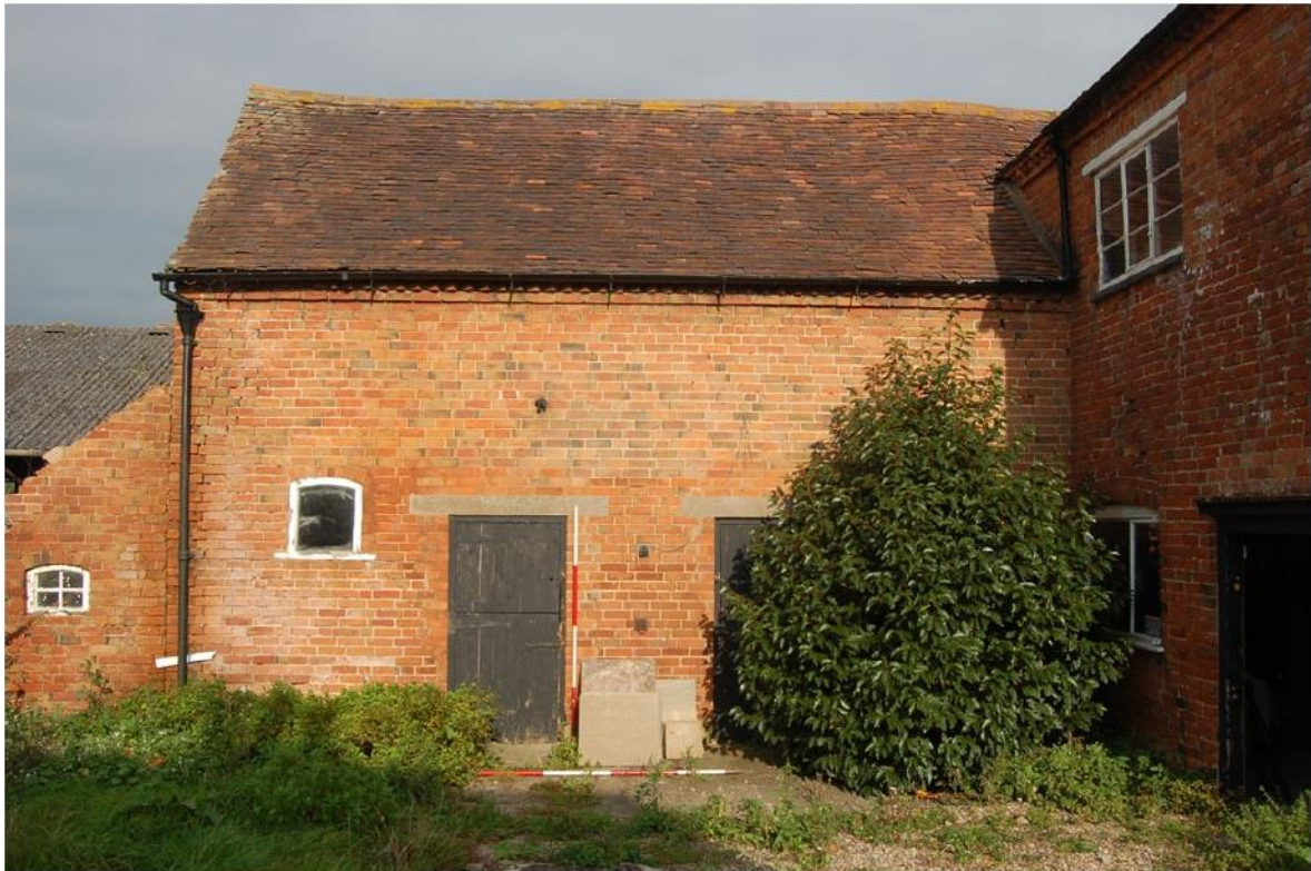
Plate 8: South range, east elevation.
