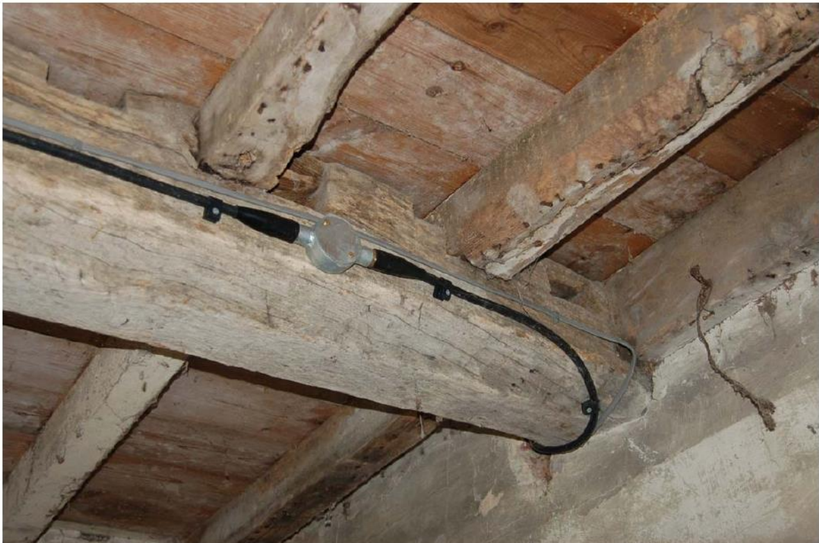
Plate 19: North range, interior; Room GF01 ceiling structure.
