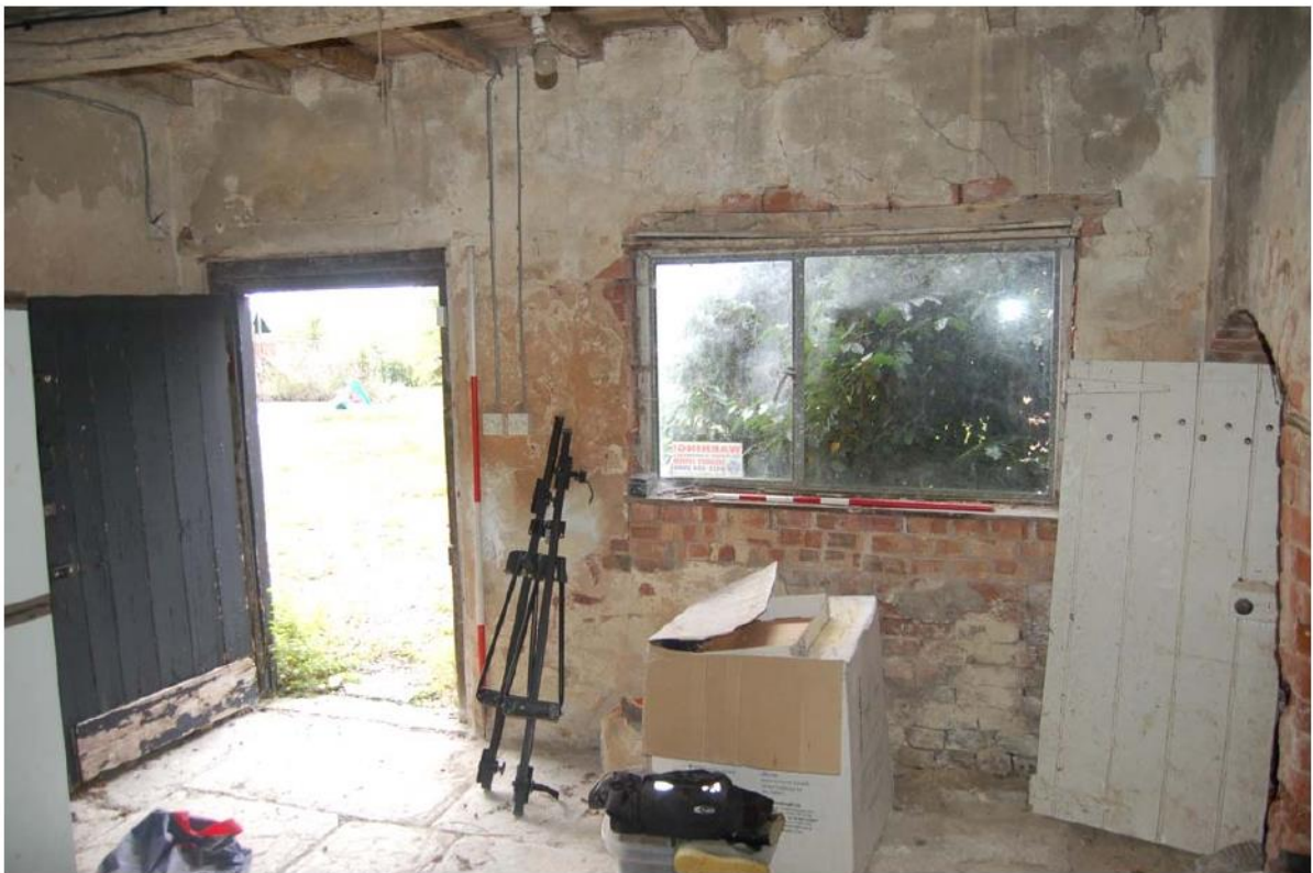
Plate 16: North range, interior; Room GF01 looking south.
