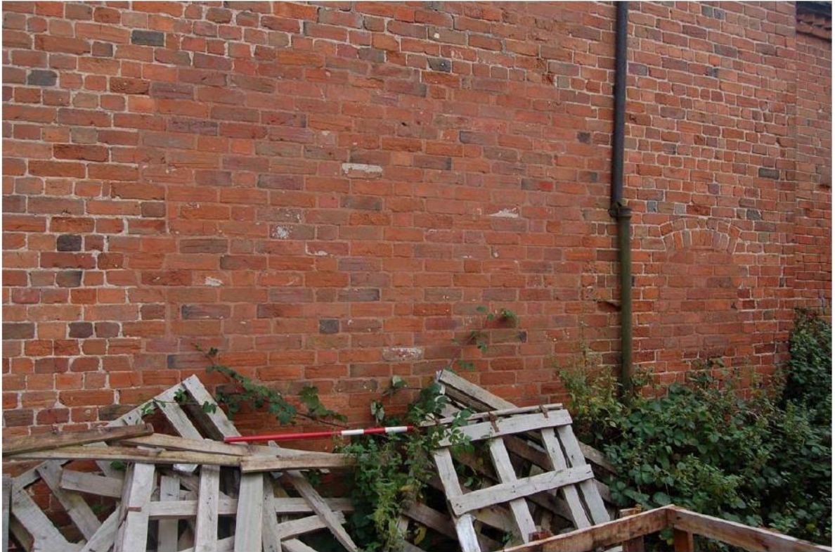
Plate 11: North range, west elevation; blocked door and window.
