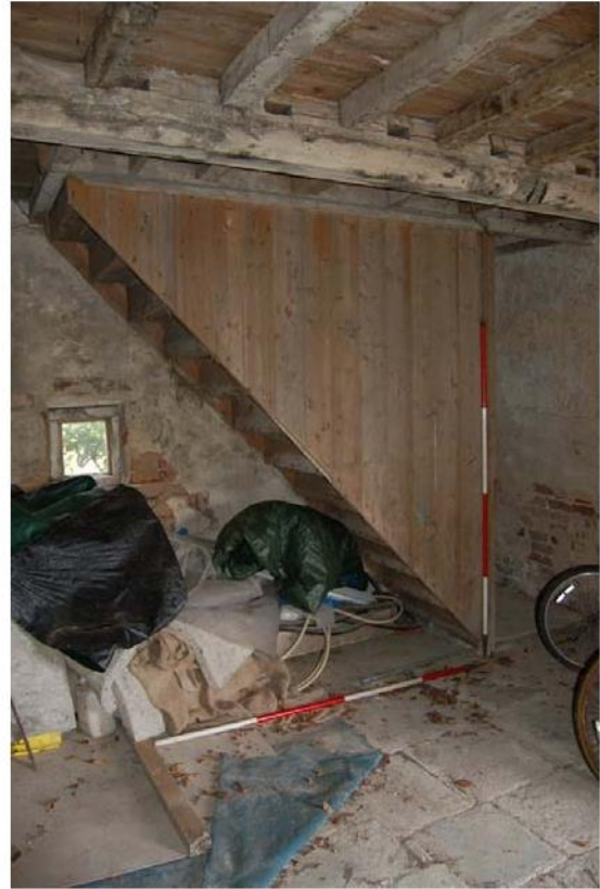
Plate 18: GF01; stair rising at NE corner.
