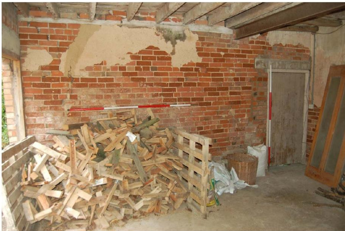
Plate 20: North range, interior; Room GF02, east wall.
