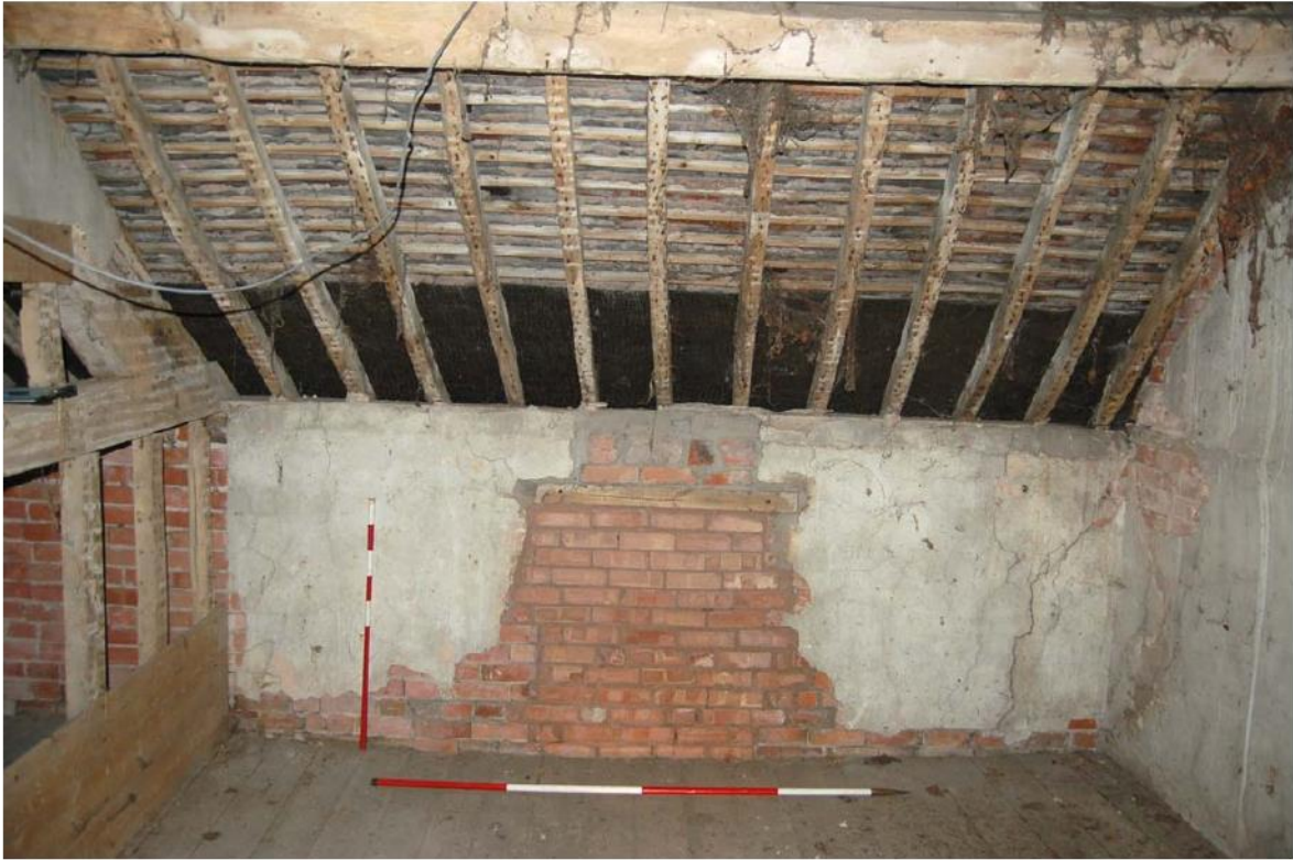
Plate 40: North range, interior; Room 1F03, west wall; blocked window/pitching door.
