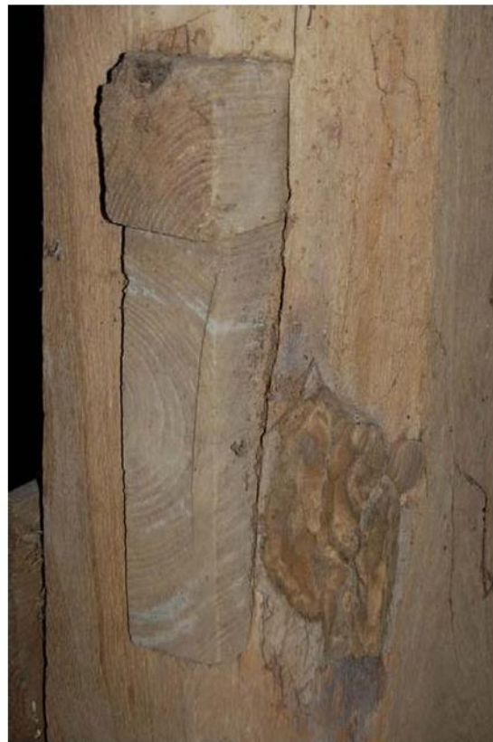
Plate 43: Room 1F03; detail of wedged joint.
