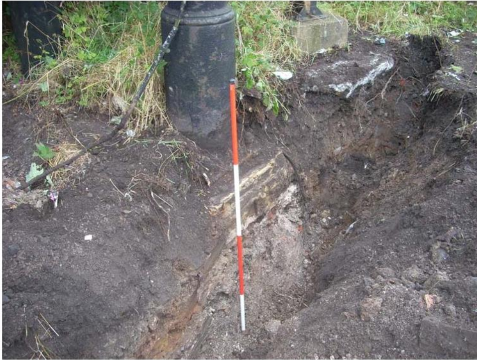
Plate 1: Foundation Trench 1 showing the footing of the footbridge.
