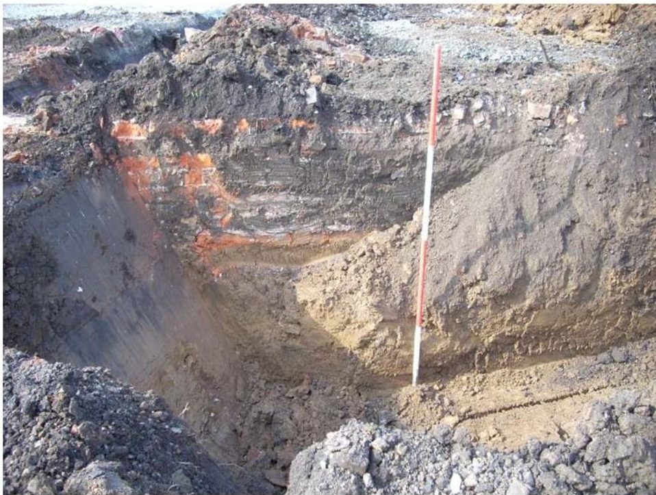
Plate 2: Foundations visible during the balancing pond excavations.
