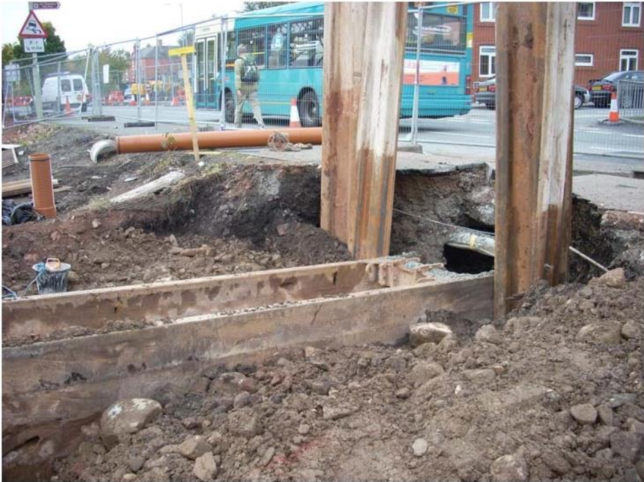
Plate 4: Shoring the trenches to prevent collapse.
