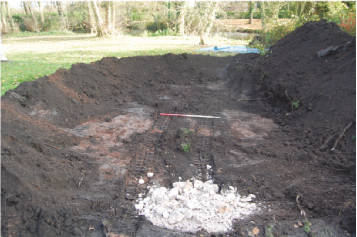
Mound construction after excavation, from the south
