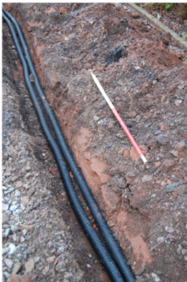
Service trench; course of sandstone blocks, from the southeast
