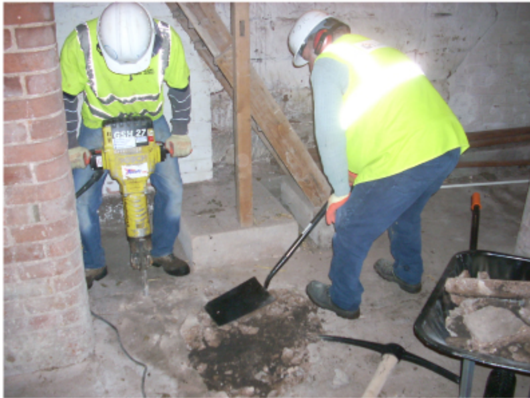
Malthouse floor groundworks, from the east
