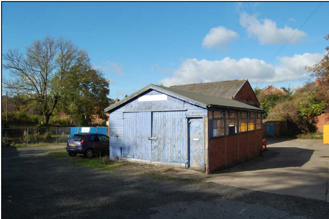
Plate 10: Building 4 from the Southeast
