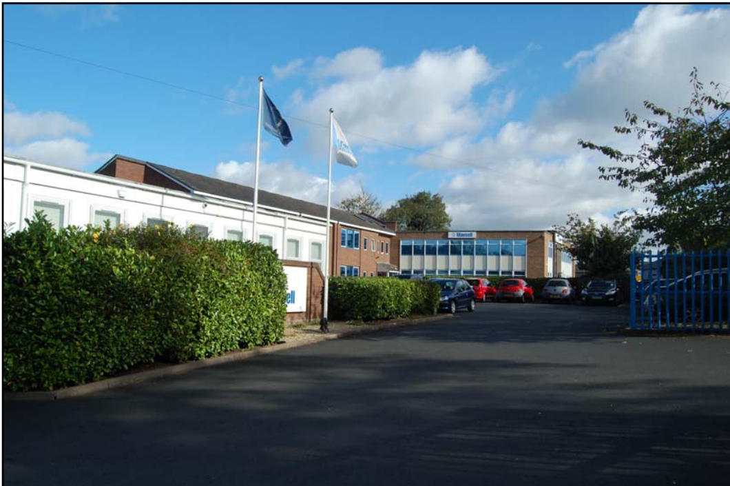
Plate 4: Current Office of Mansell Construction Ltd. from Southwest
