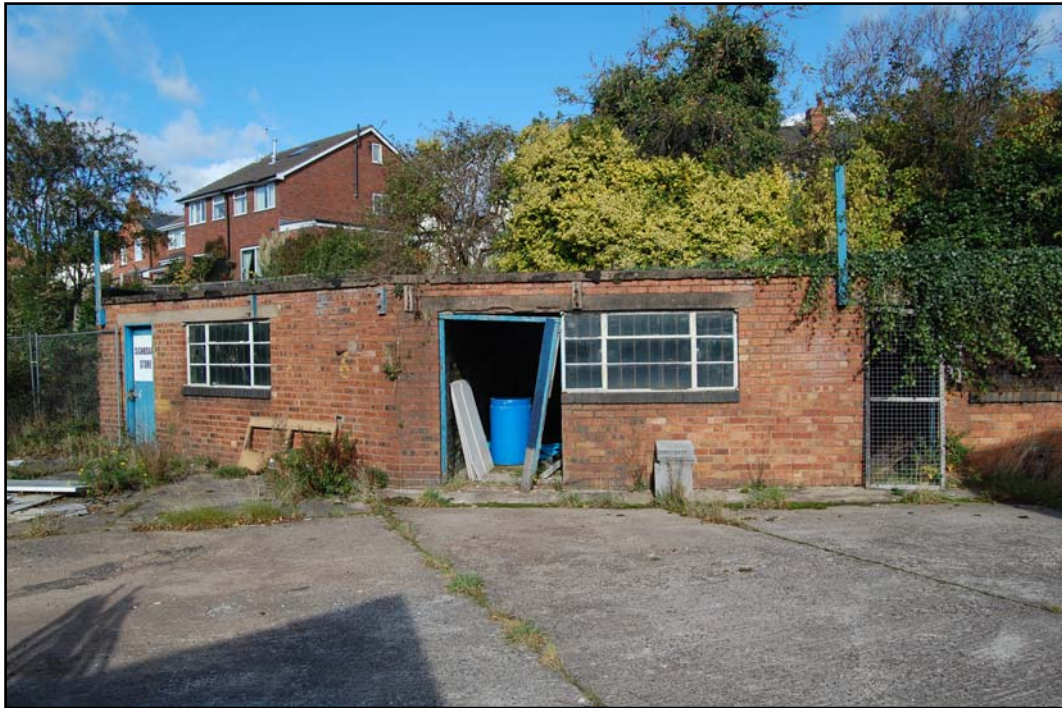
Plate 7: Building 1 from the South
