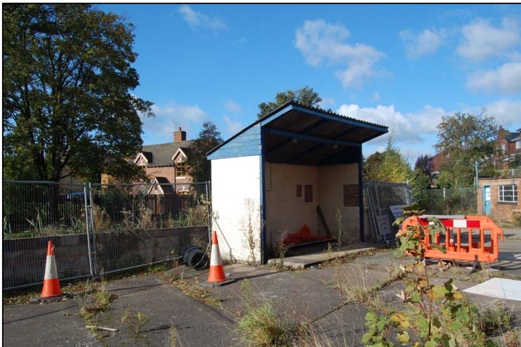
Plate 8: Building 2 from the Southeast
