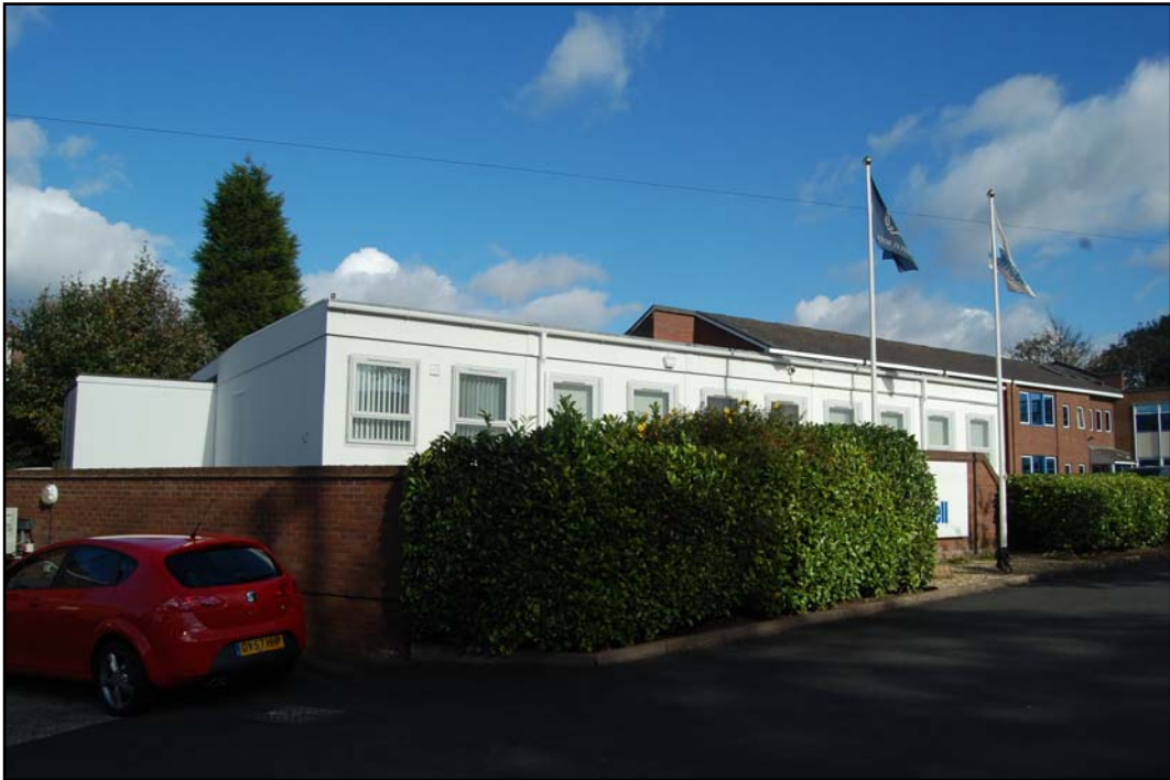
Plate 5: Late 20th-Century Prefab Building from the Southwest
