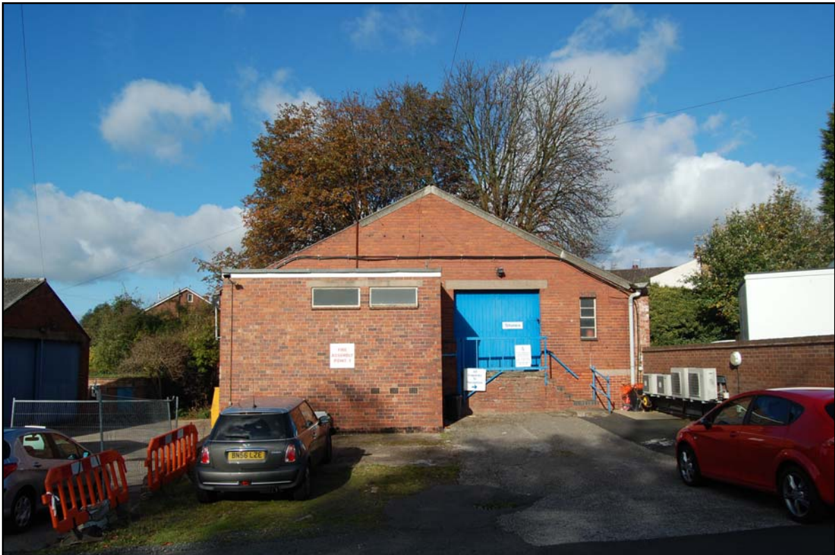
Plate 11: Building 5 from the South
