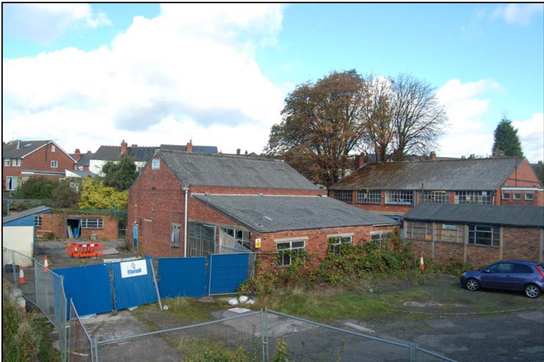
Plate 6: Western Portion of the Site from the Southwest
