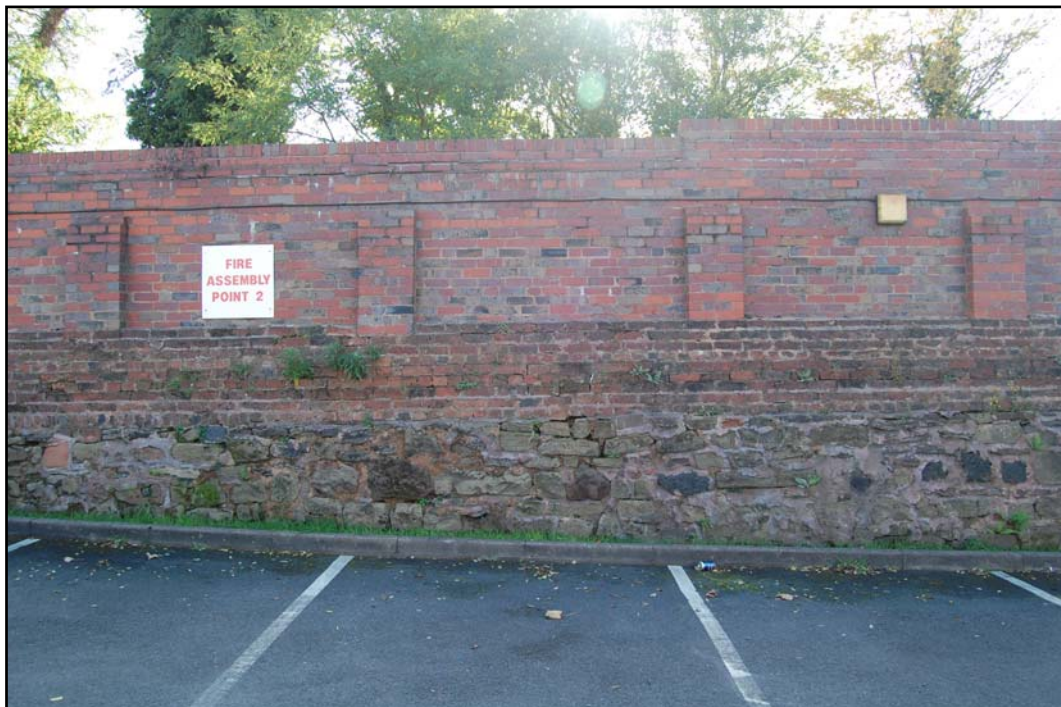
Plate 2: South Boundary Wall from the North
