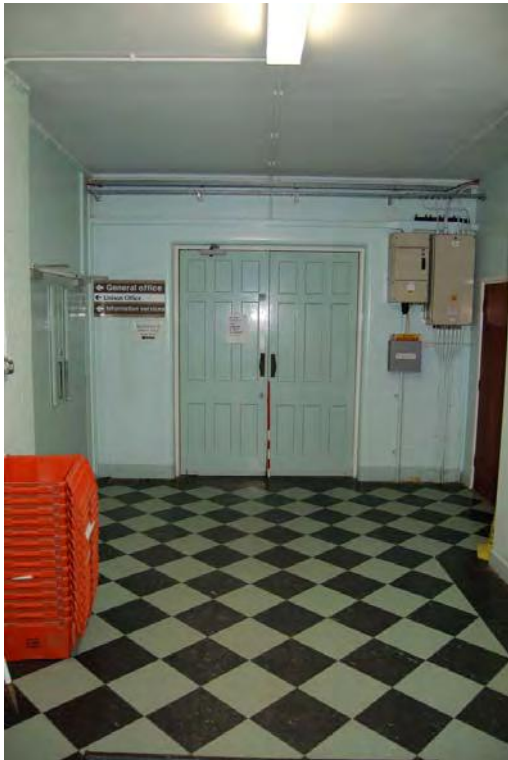
Plate 55: Bldg 28: East entrance (GF89).
