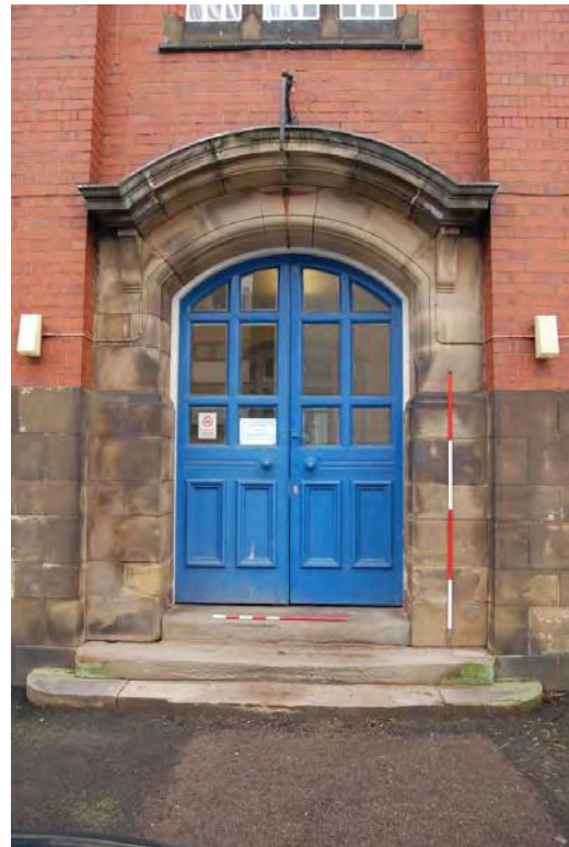
Plate 28: Building 28: main entrance.
