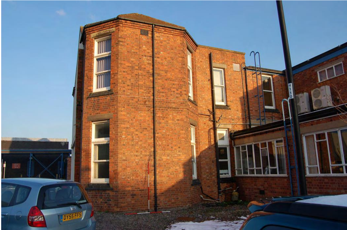
Plate 136: Building 52: north-west elevation.
