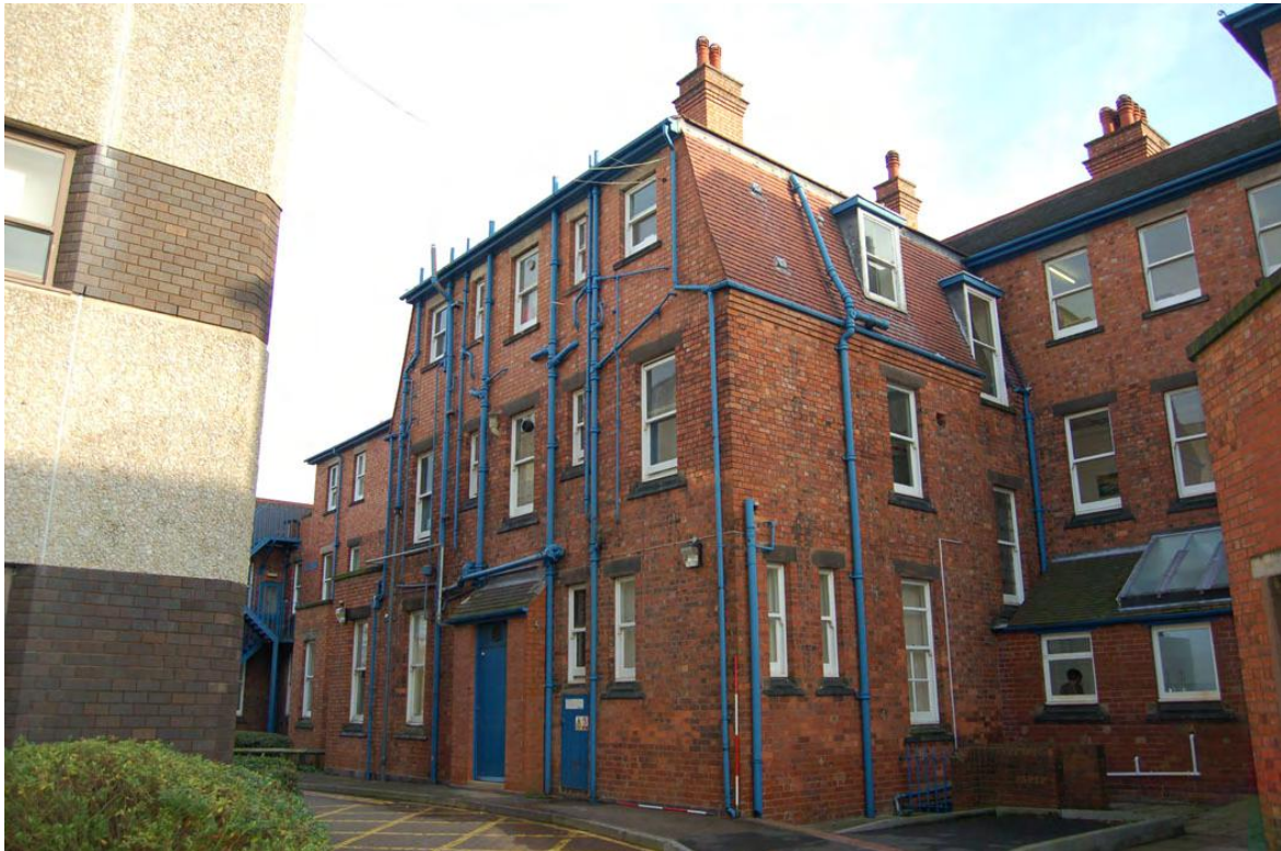
Plate 11: Building 23: north elevation (centre).
