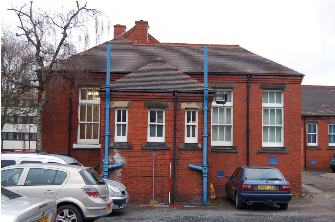
Plate 101: Building 36: west range, south elevation.
