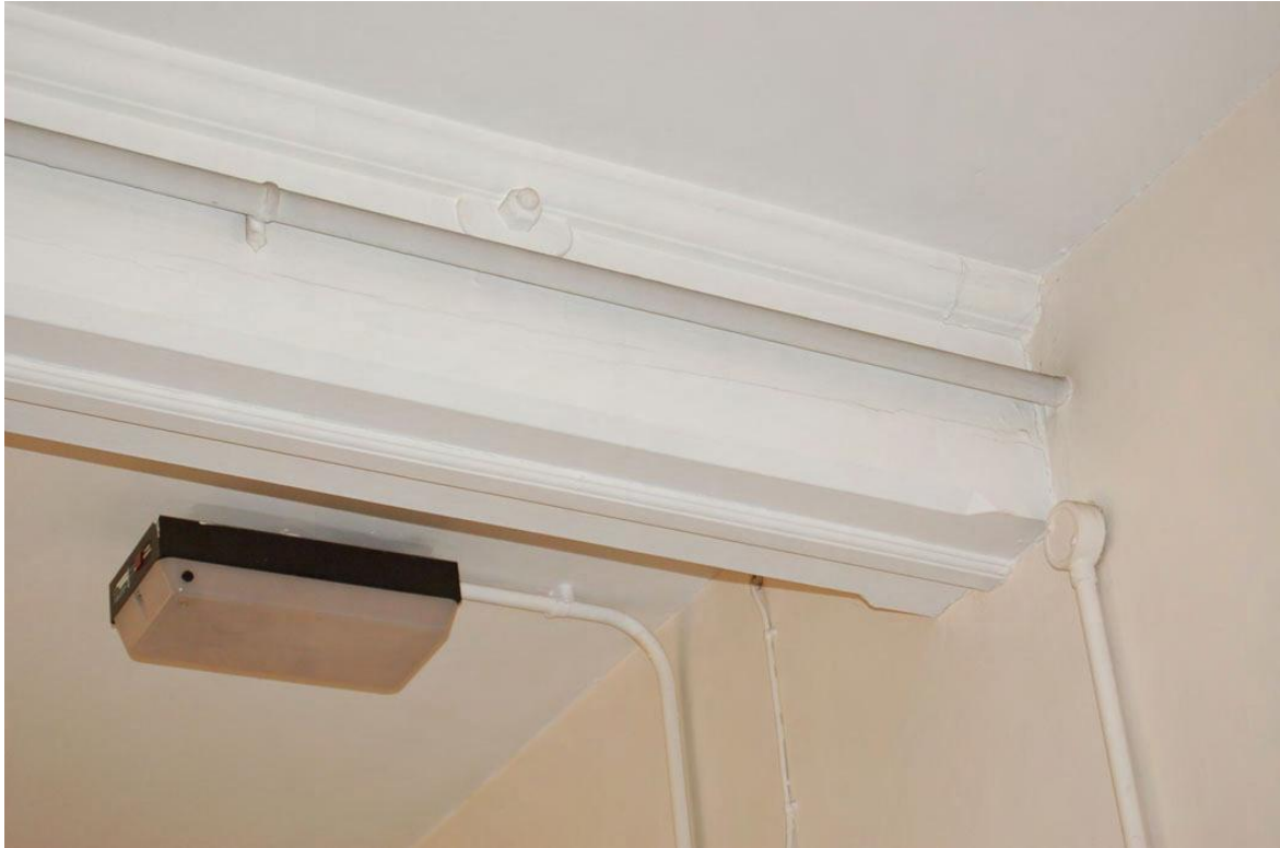
Plate 126: Building 37: Ground floor, stop-chamfered beam.
