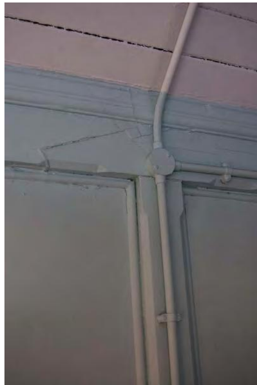
Plate 85: Bldg 29: walkway detail.
