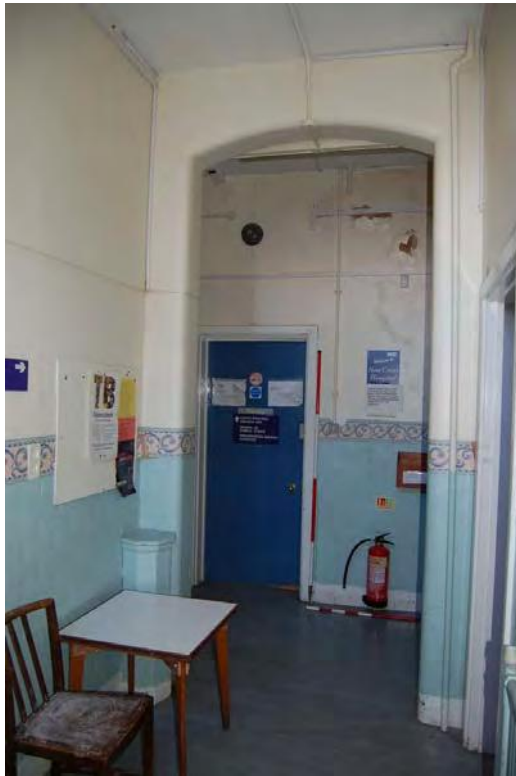
Plate 109: Bldg 36, lobby GF15.
