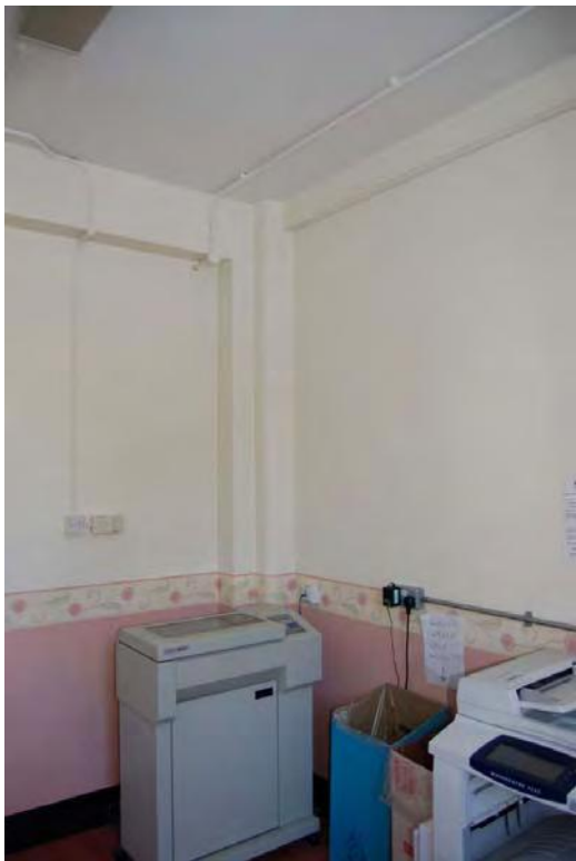
Plate 80: Bldg 29: GF room detail.
