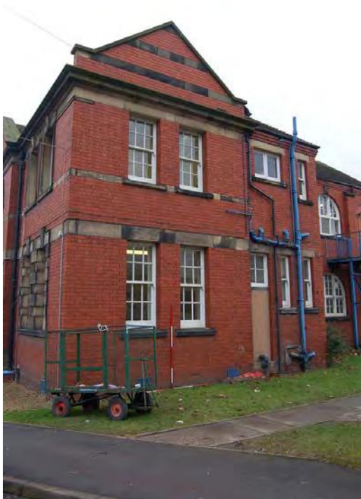
Plate 121: Building 37; north elevation, east gable.
