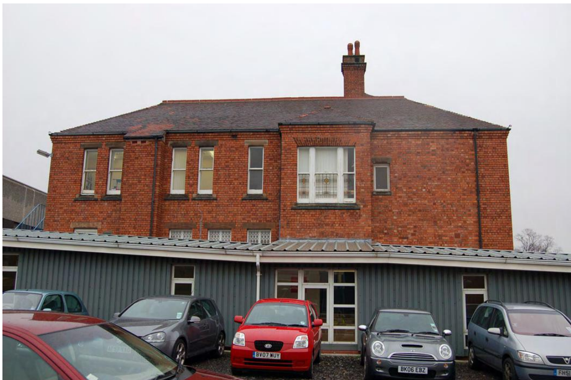
Plate 7: Building 23: west elevation.
