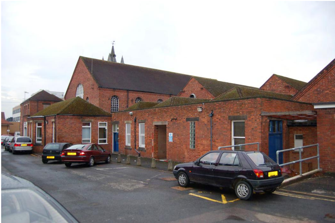
Plate 34: Building 28: east flanking range and northern ranges looking south-west.
