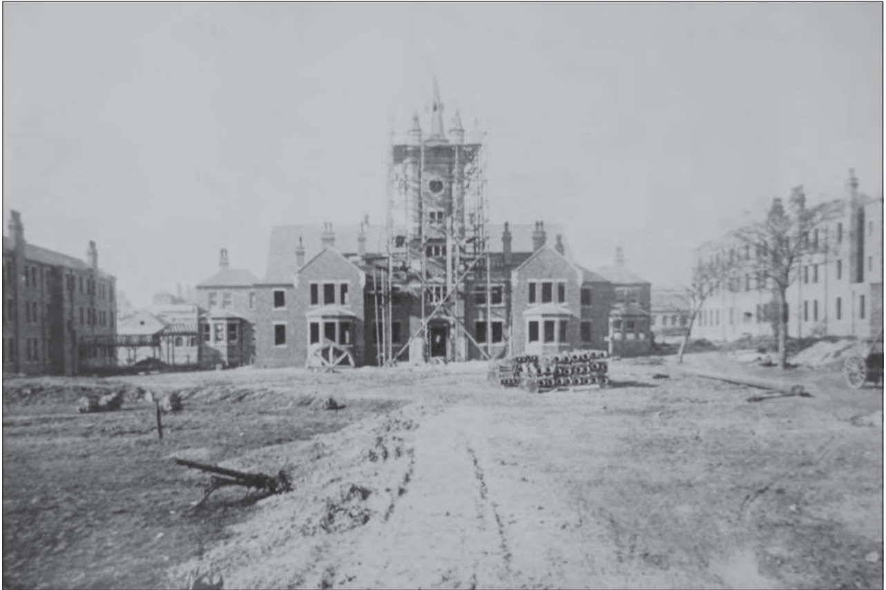
(a) Under construction
