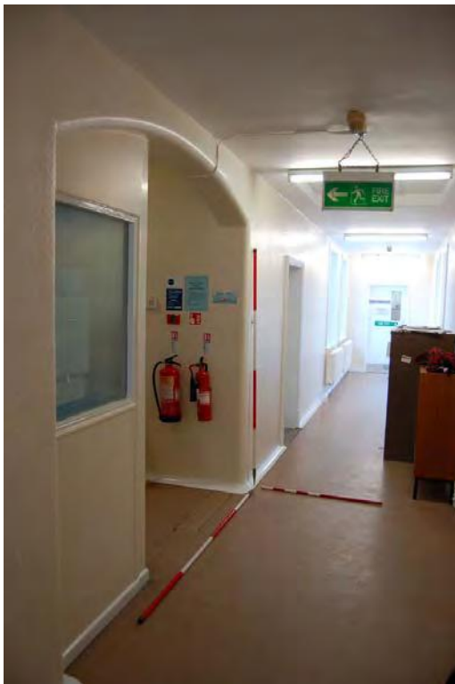
Plate 23: Bldg 23: 2F corridor.
