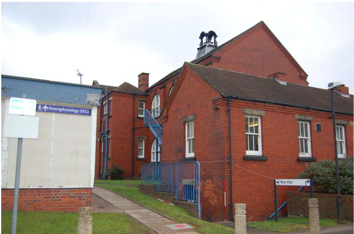
Plate 119: Building 37; oblique view looking south-east.
