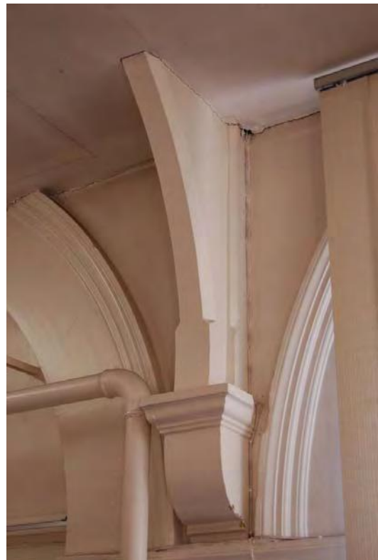
Plate 131: Bldg 37: roof bracket.
