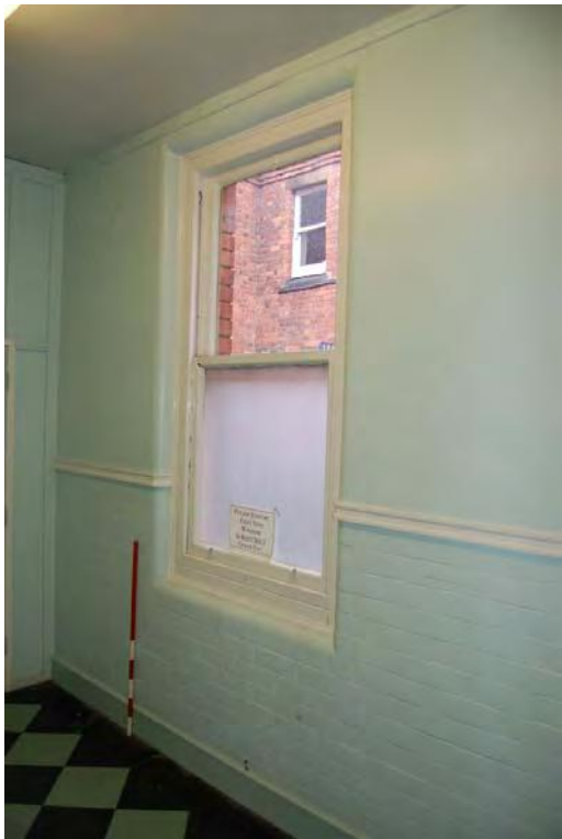
Plate 53: Bldg 28: GF window detail.
