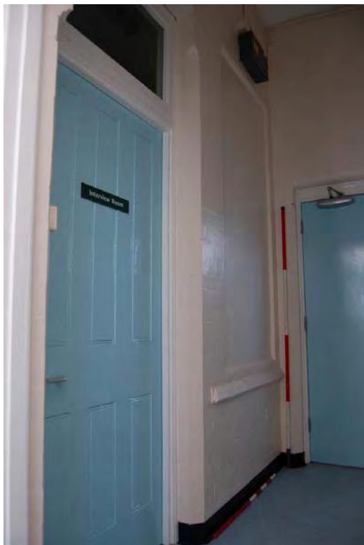
Plate 113: Bldg 36, lobby GF22.
