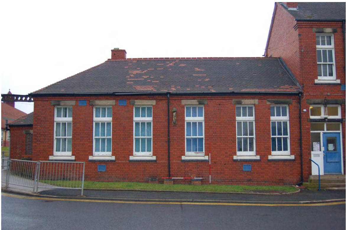
Plate 98: Building 36: west elevation (north).
