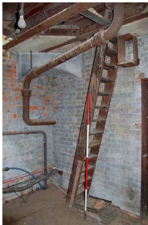
Plate 50: Bldg 28: Clock tower stair 2/3F.
