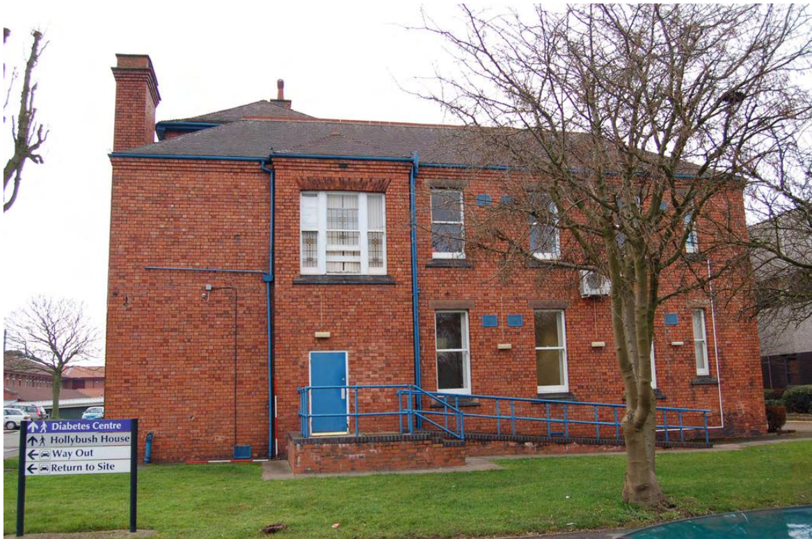
Plate 6: Building 23: east elevation.
