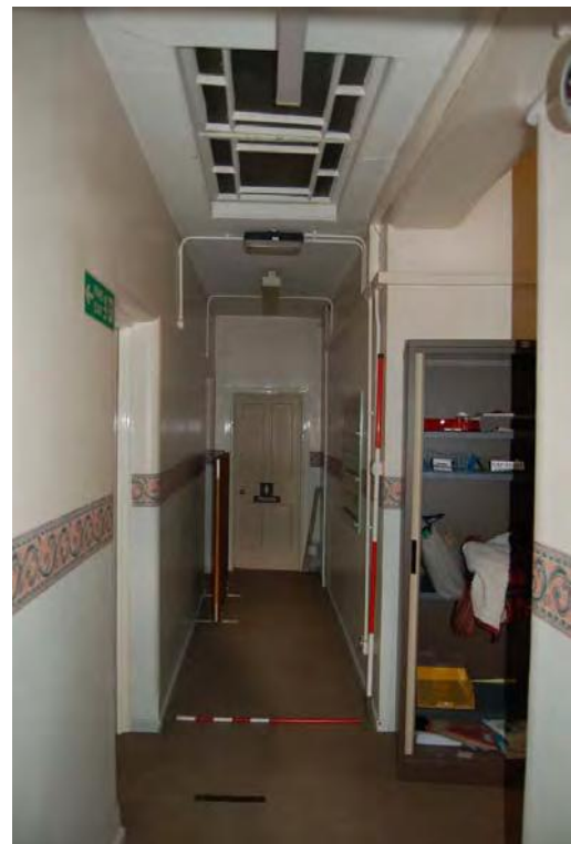
Plate 125: Bldg 37: GF05 (NB Skylight).
