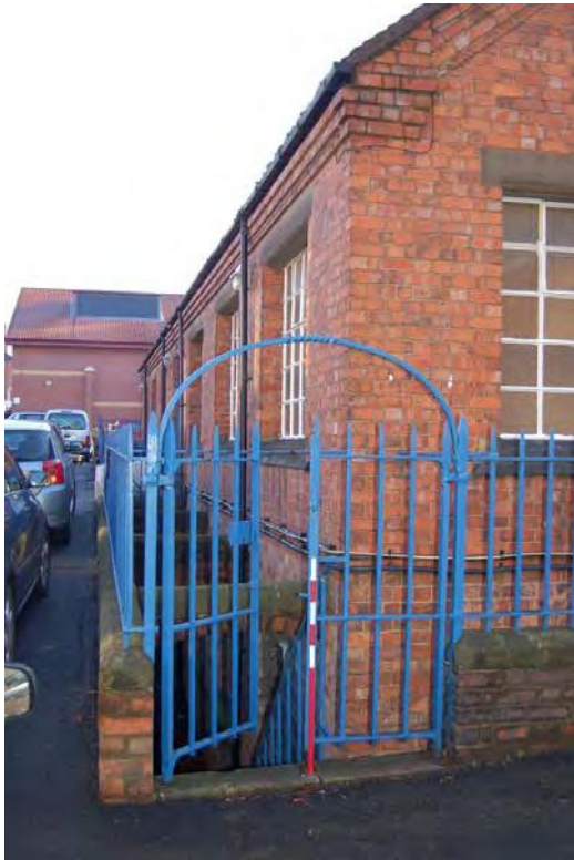
Plate 36: Bldg 28: stair to basement level.
