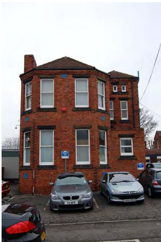
Plate 87: Bldg 29: S elevation.
