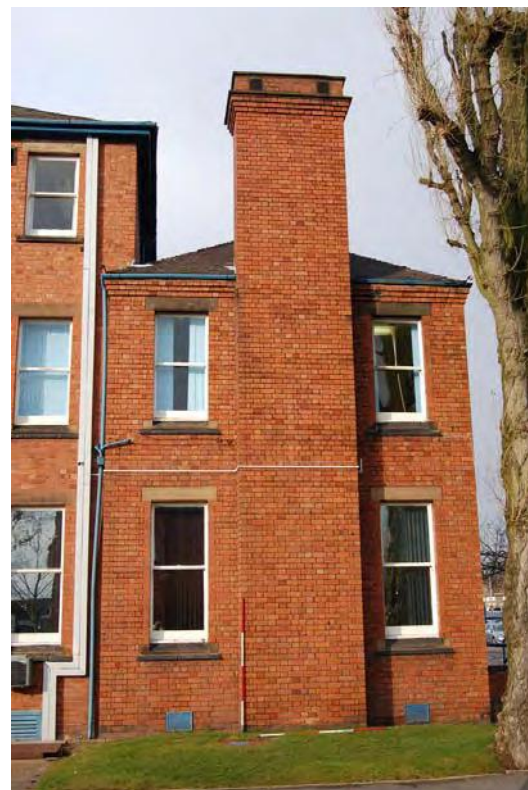
Plate 5: Building 23: south elevation eastern terminal block.
