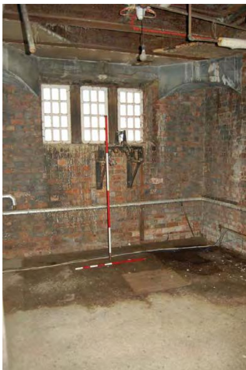
Plate 49: Bldg 28: Clock tower 2F.
