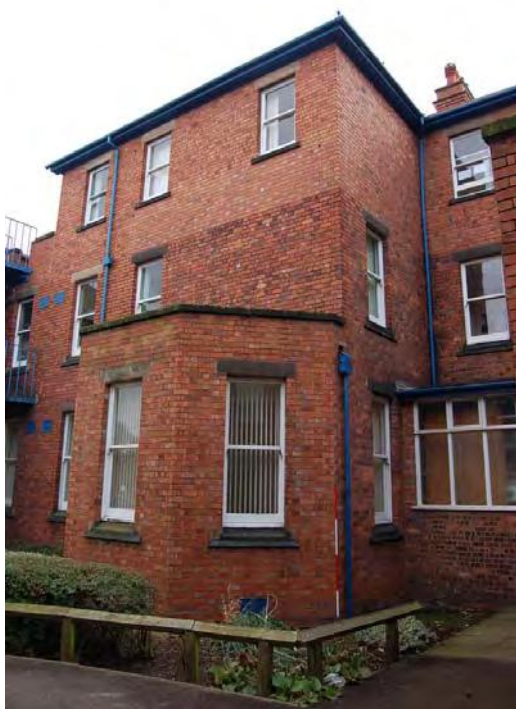
Plate 9: Building 23: north elevation, centre section looking SE.
