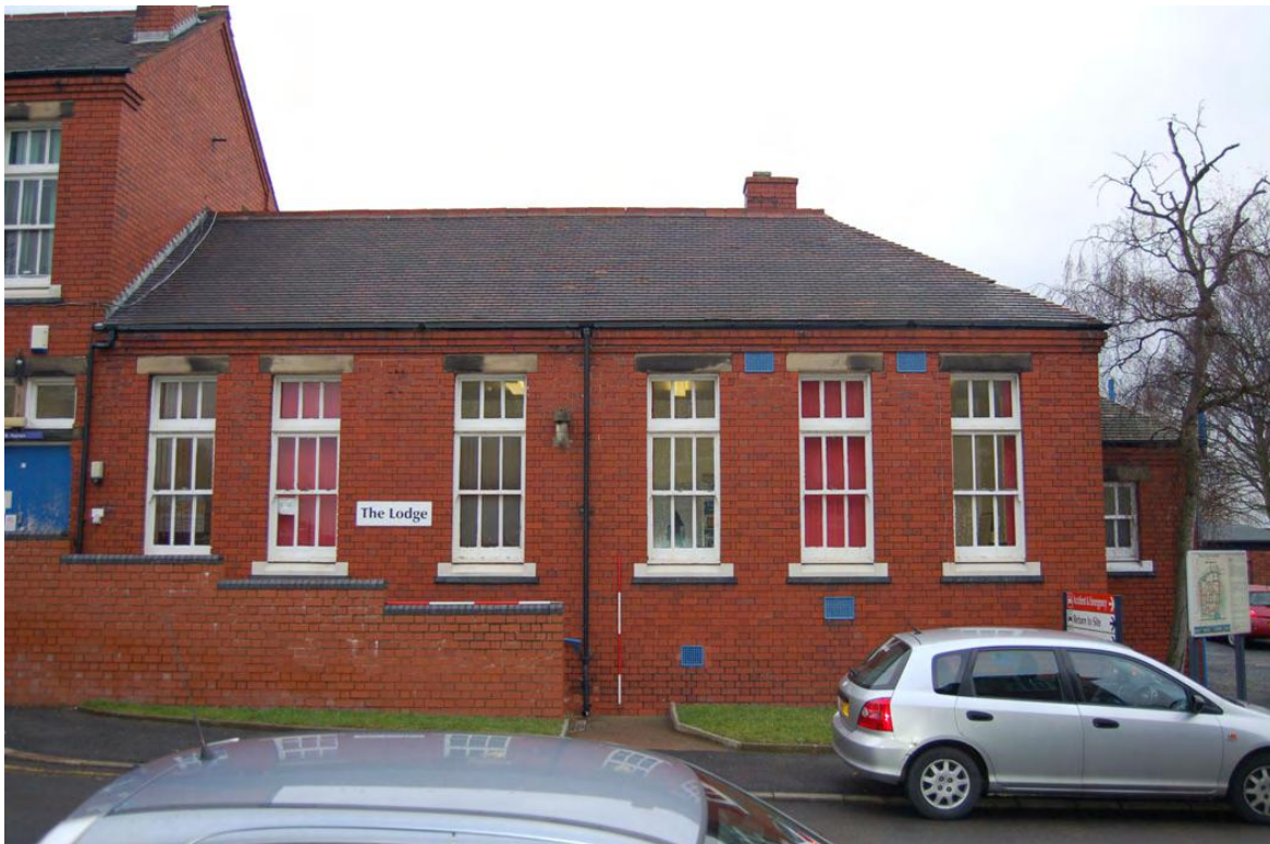
Plate 100: Building 36: west elevation (south).
