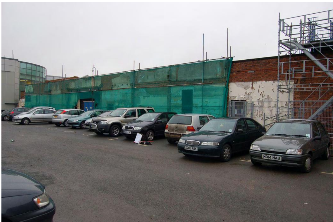
Plate 145: Building 52; southern elevation of transverse passage.
