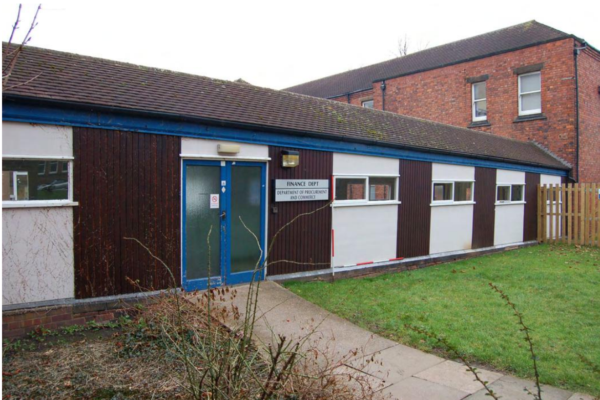
Plate 83: Building 29: covered walkway, north side linking to former nursery to right.
