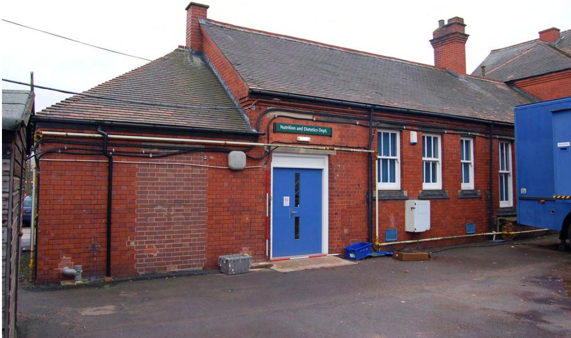
Plate 105: Building 36: east range, north elevation (east end).
