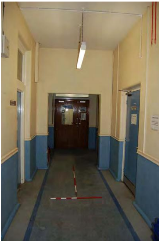
Plate 143: Bldg 52: 1F corridor (N).
