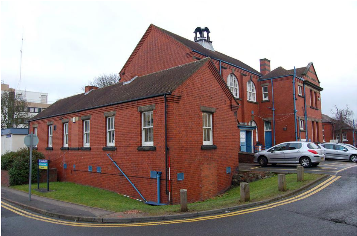
Plate 118: Building 37; oblique view looking north-east.
