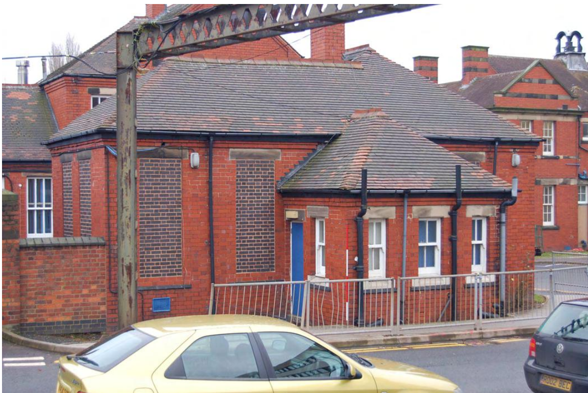
Plate 108: Building 36: north elevation.
