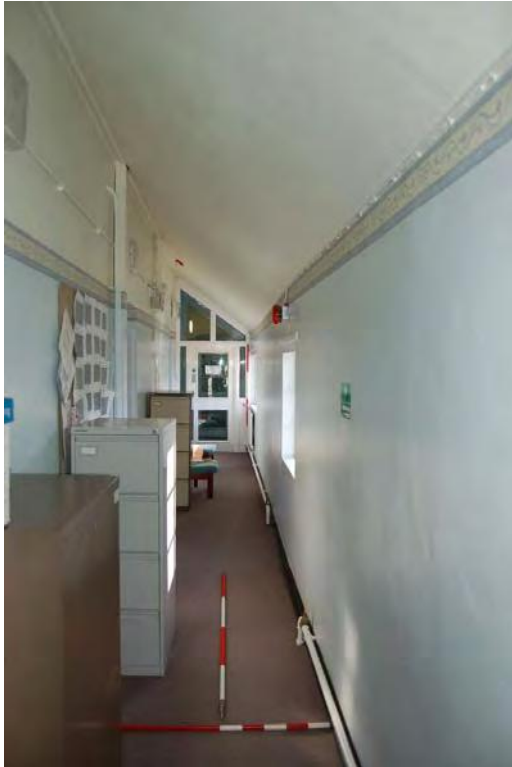
Plate 82: Bldg 29: 1F corridor.
