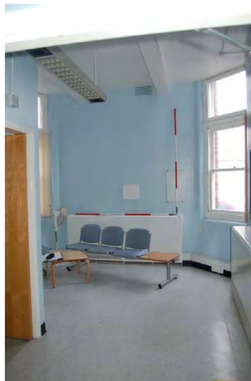
Plate 140: Bldg 52: GF, room GF21.
