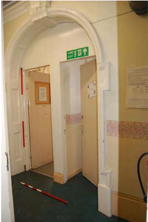
Plate 128: Bldg 37: arched door to 1F03.
