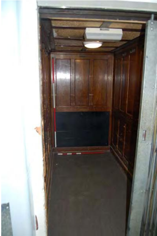
Plate 141: Bldg 52: Waygood-Otis lift.
