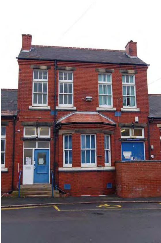
Plate 99: Bldg 36: west elevation, main block.
