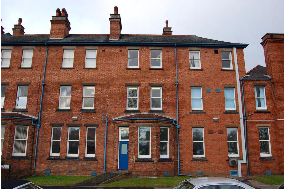
Plate 3: Building 23: south elevation (east).
