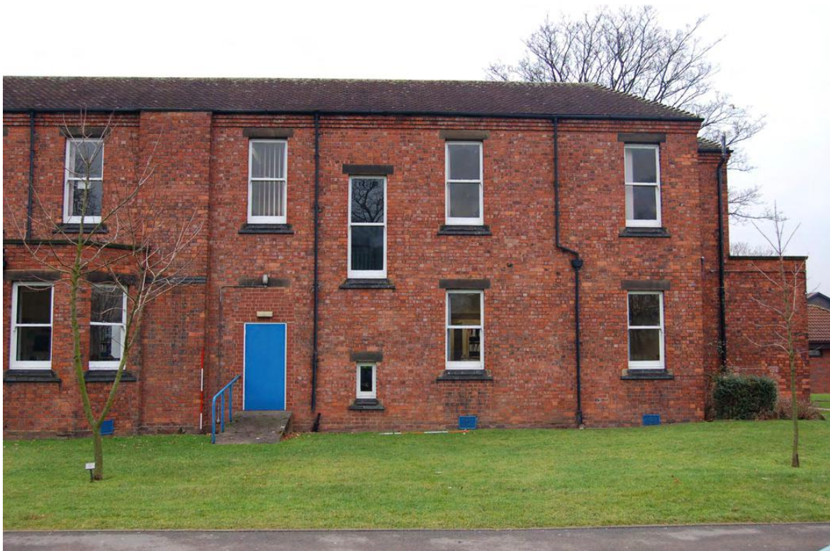
Plate 70: Building 29: east elevation, north end.
