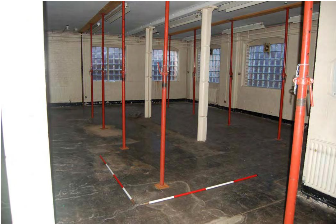
Plate 67: Building 28: rear range basement (B1) looking north-west.
