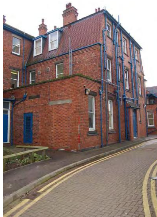
Plate 10: Building 23: north elevation, centre section looking SW.
