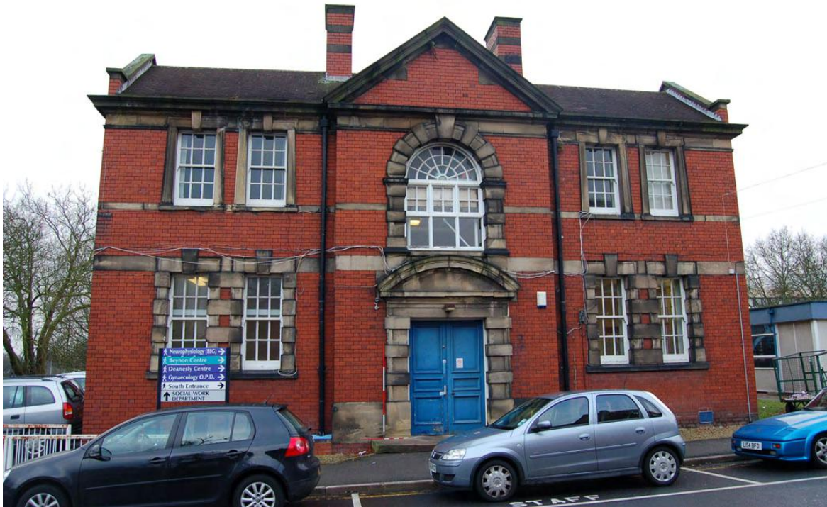
Plate 116: Building 37; west elevation.
