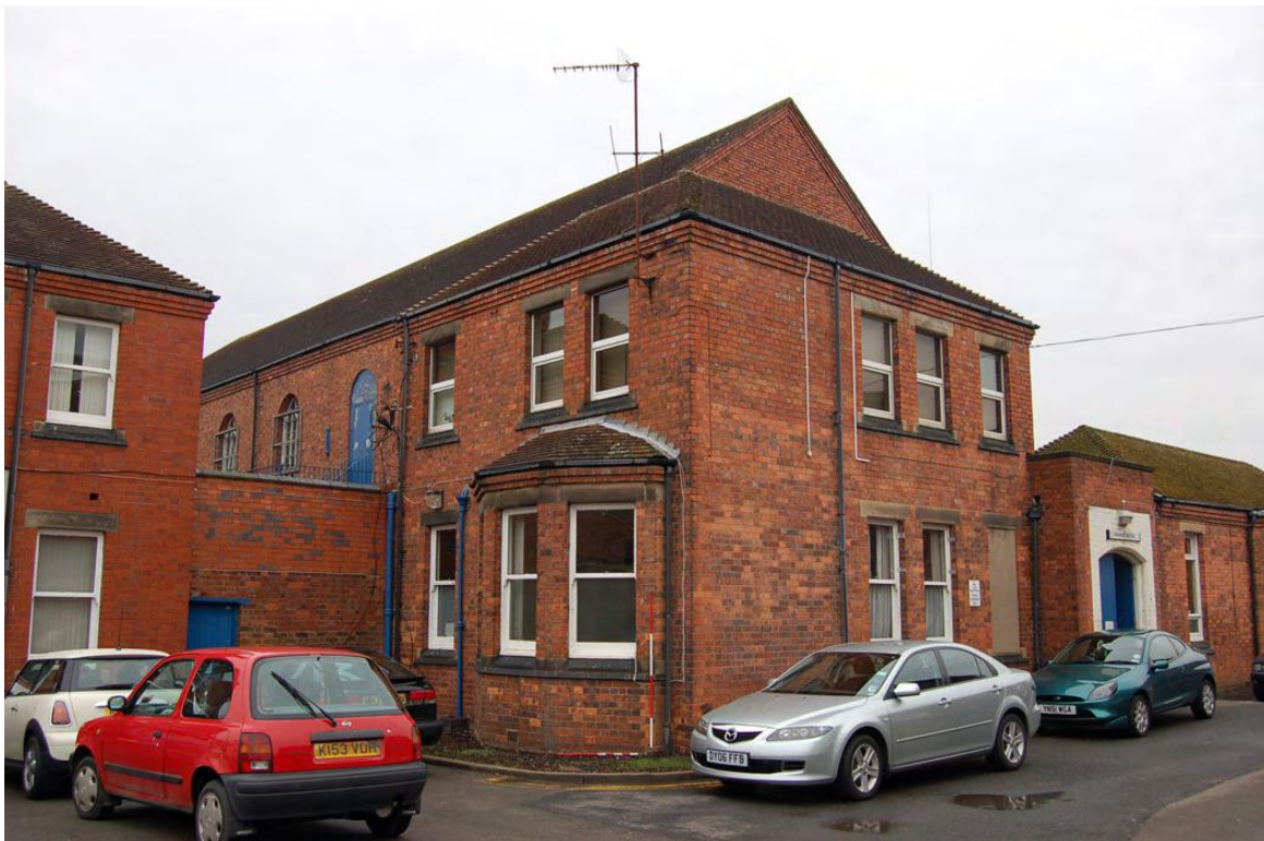
Plate 31: Building 28: eastern flanking range, main hall beyond.
