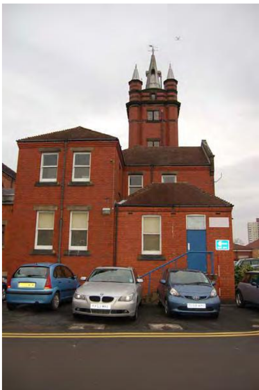
Plate 42: Bldg 28: clock tower range (W).
