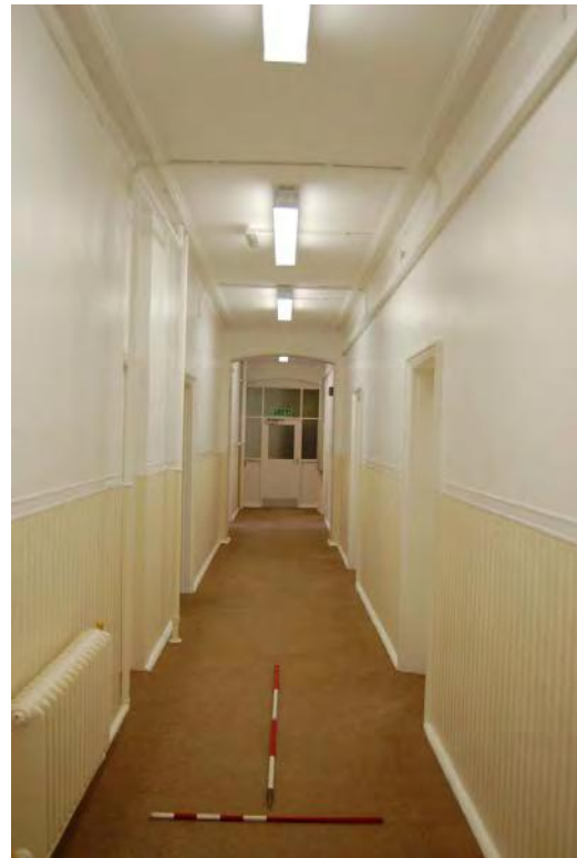
Plate 16: Bldg 23: GF corridor, E (GF26).
