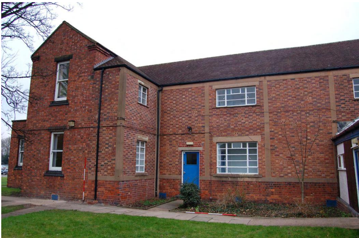
Plate 72: Building 29: west elevation, north end (note infill of veranda / balcony).
