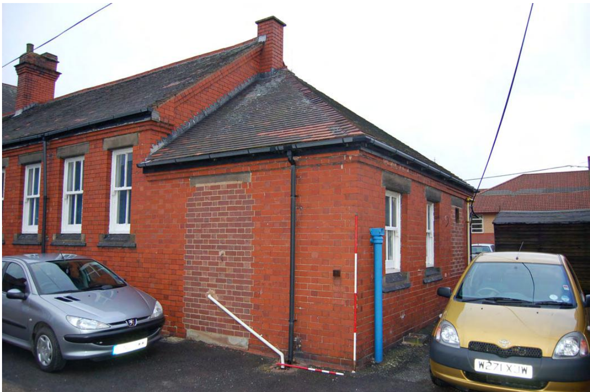
Plate 104: Building 36: east range, east end.
