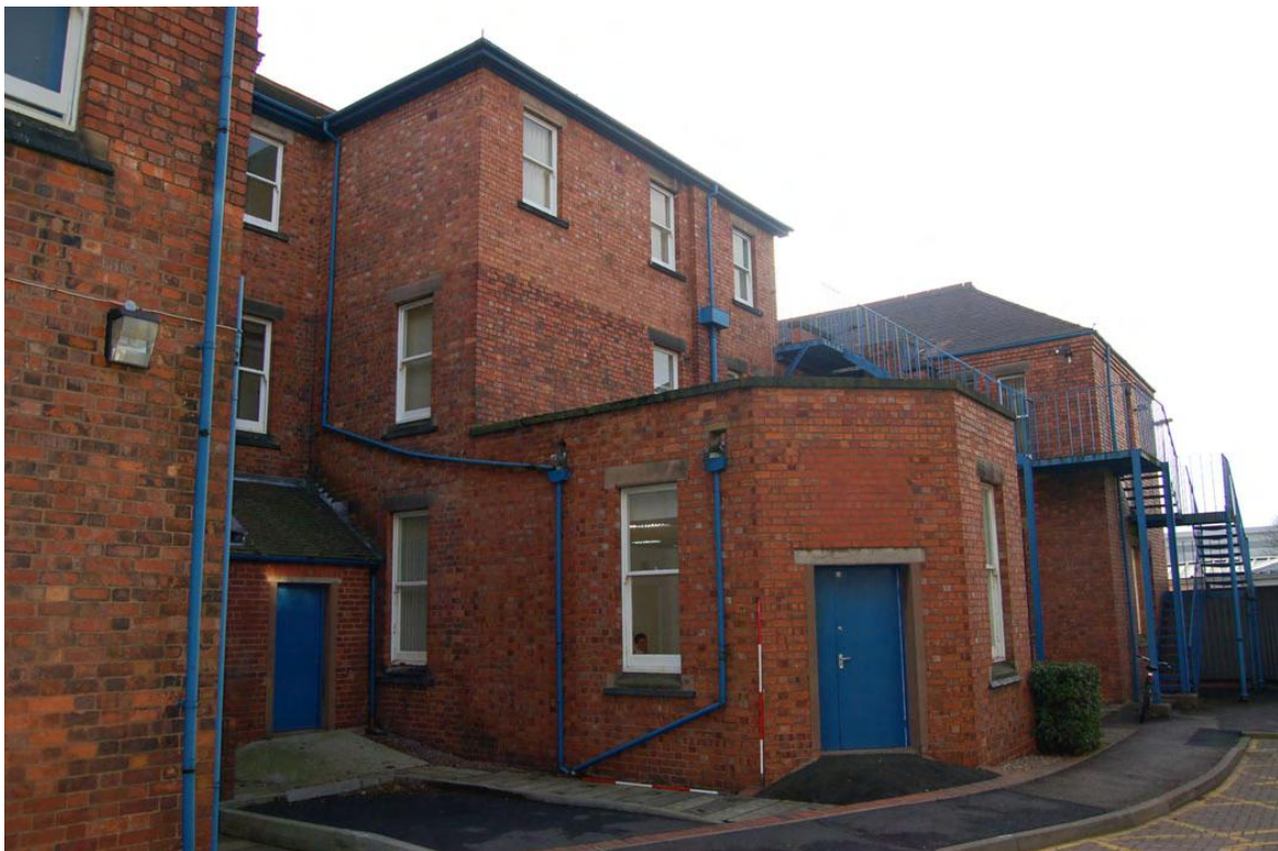
Plate 12: Building 23: north elevation (west).
