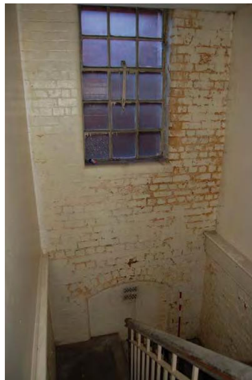
Plate 66: Bldg 28: rear range, stair to basement.
