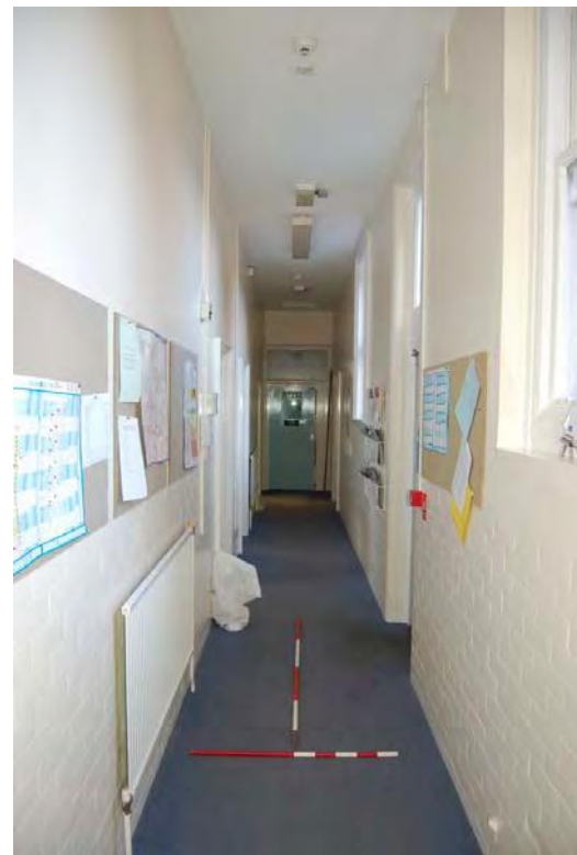
Plate 112: Bldg 36, corridor GF31.
