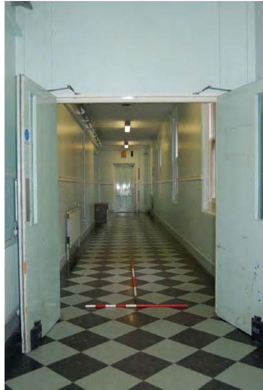
Plate 52: Bldg 28: Corridor GF92.
