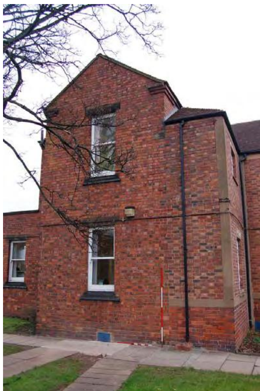
Plate 74: Bldg 29: north-west gable note infill of veranda / balcony).
