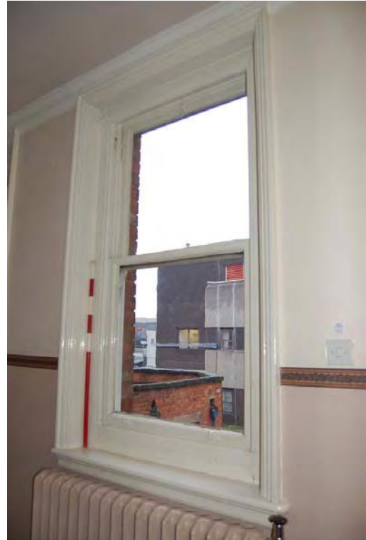
Plate 22: Bldg 23: typical window detail (1F).
