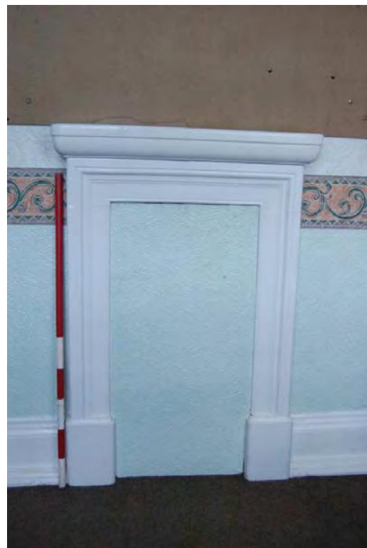
Plate 61: Bldg 28: 1F11, FP surround.
