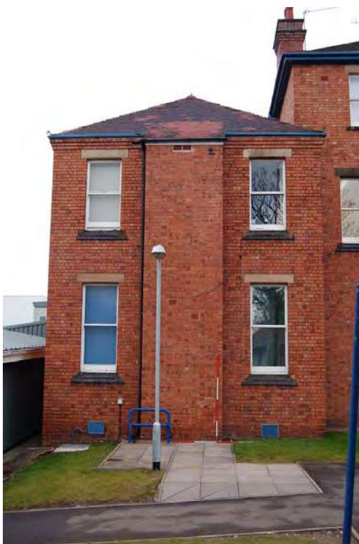
Plate 4: Building 23: south elevation, western terminal block.
