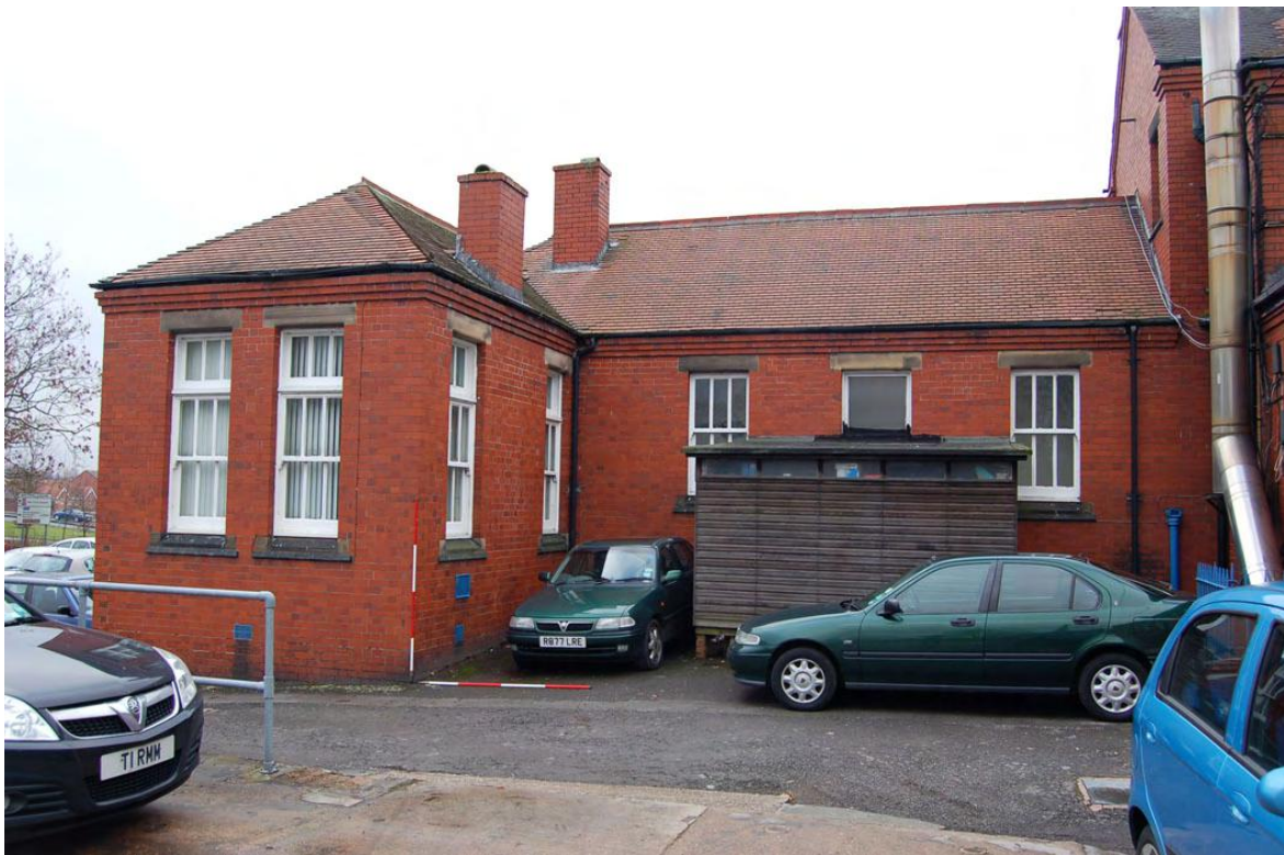
Plate 102: Building 36: west range, east elevation (south end).
