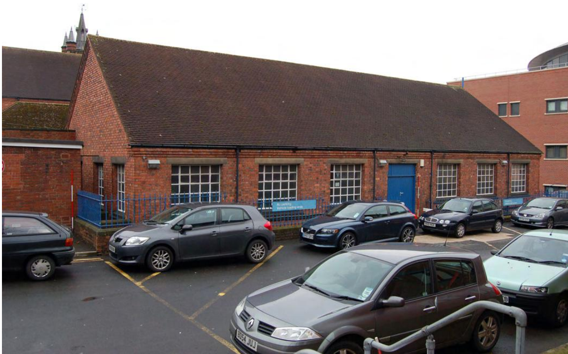
Plate 35: Building 28: northern block, oblique view looking south-west.
