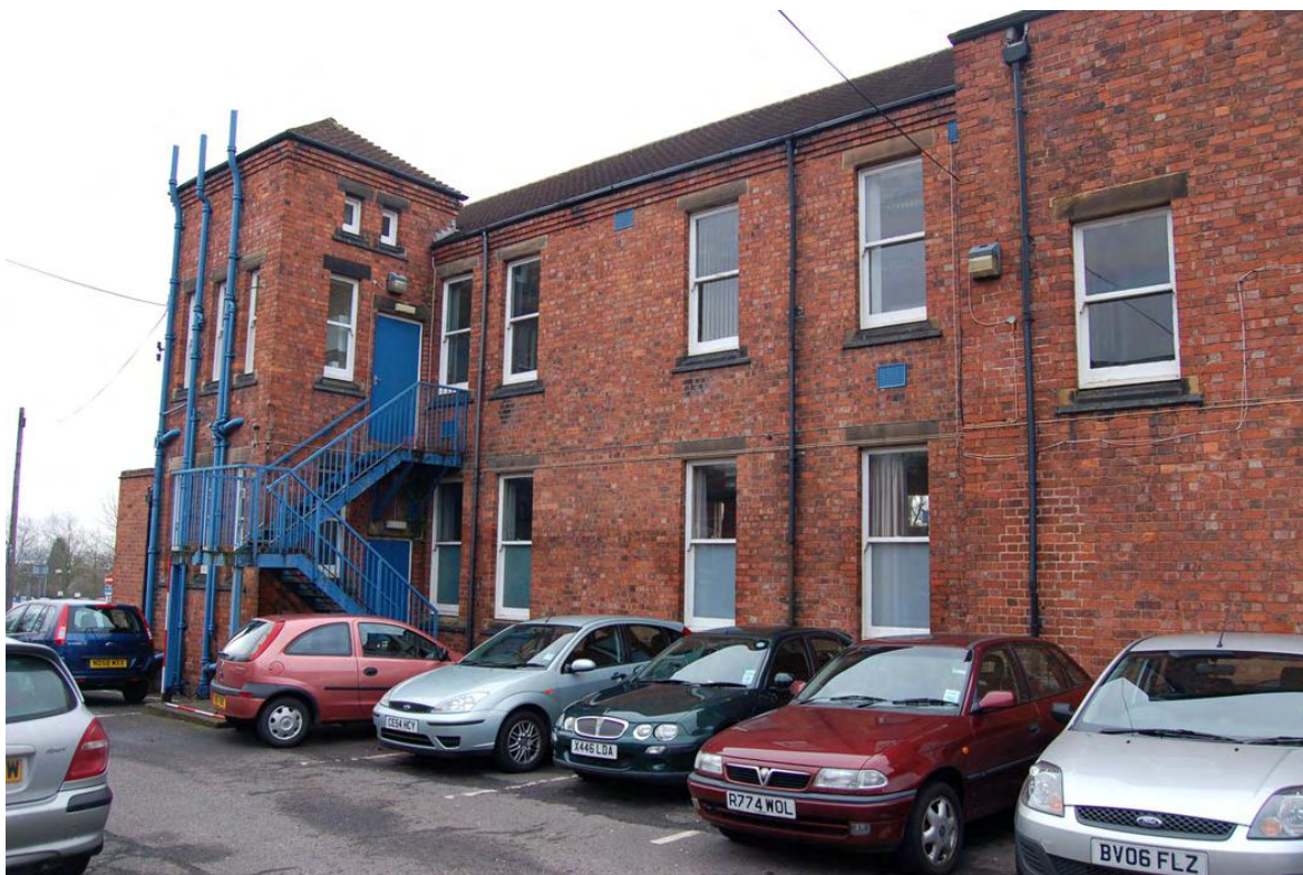
Plate 89: Building 29, east elevation looking south-east.
