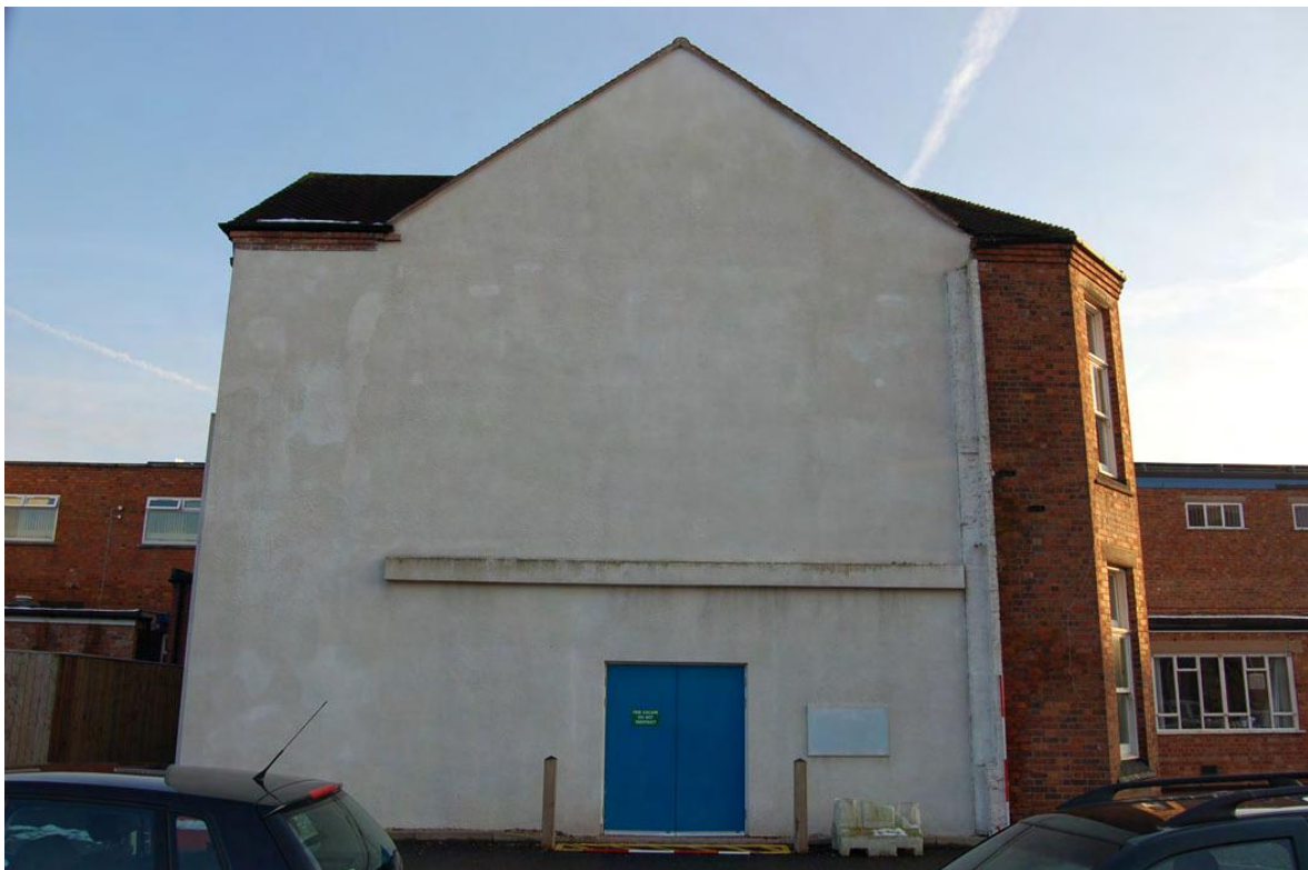
Plate 135: Building 52: truncated north elevation, note wall stub to right.
