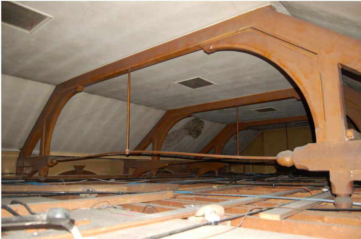
Plate 132: Building 37: centre block; hammerbeam roof (compare Plates 58/9).
