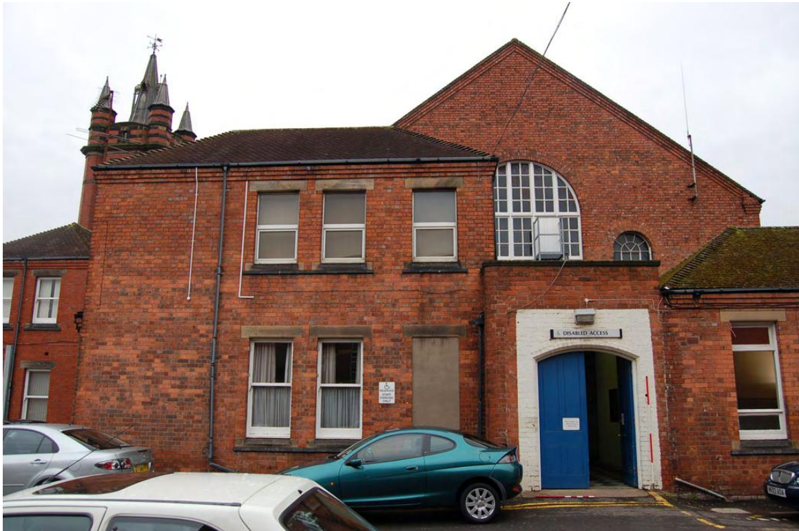
Plate 32: Building 28: east flanking range, main hall beyond.
