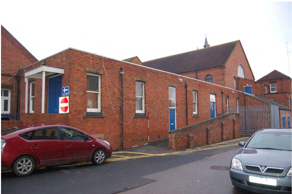
Plate 38: Building 28: north-eastern perimeter corridor, main hall beyond.
