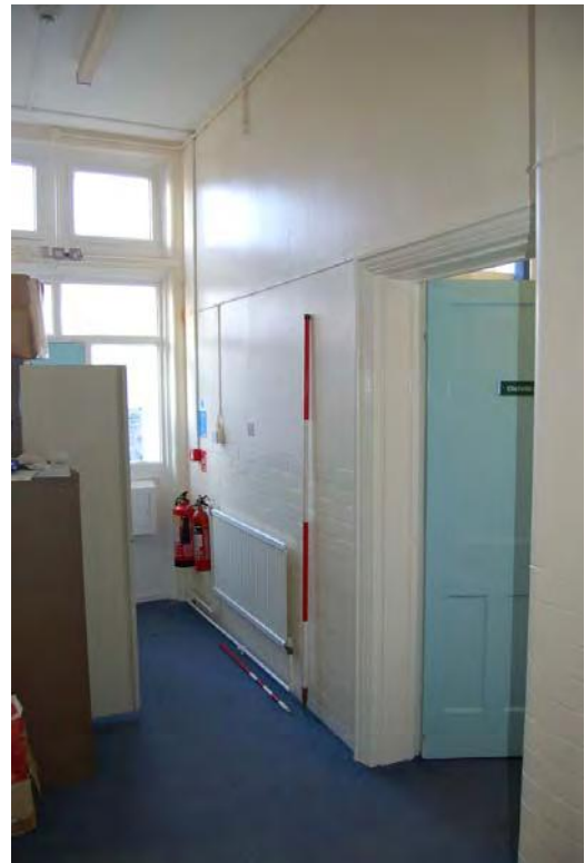
Plate 110: Bldg 36, lobby GF27.
