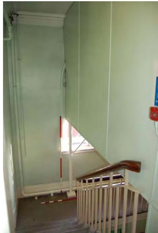
Plate 123: Bldg 37: inserted mezzanine.
