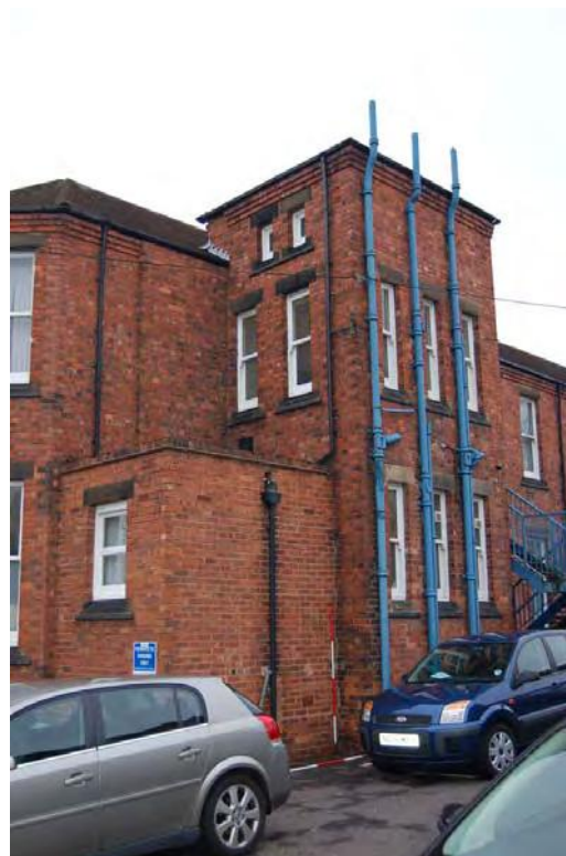
Plate 88: Bldg 29: projecting toilet block.
