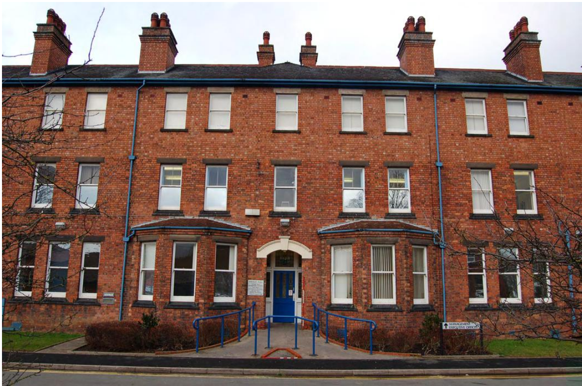
Plate 2: Building 23: south elevation (centre).
