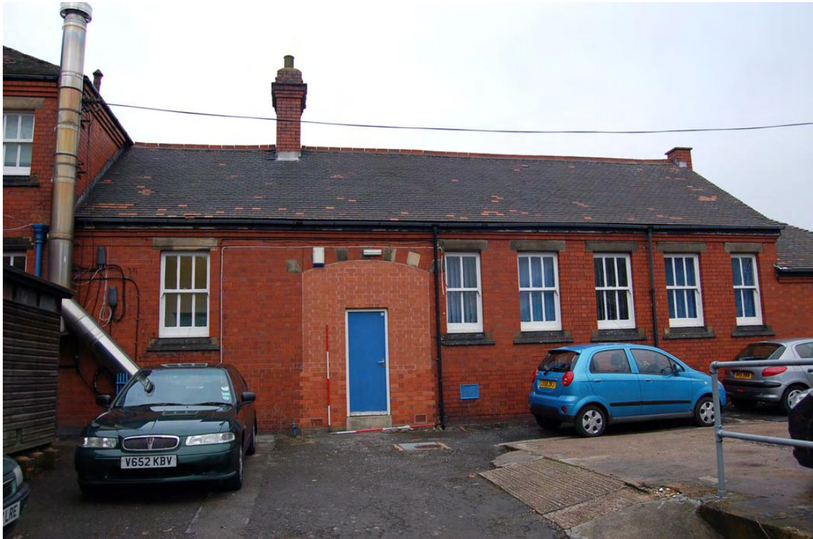
Plate 103: Building 36: east range, south elevation.
