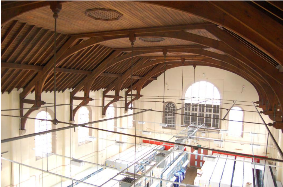
Plate 59: Building 28: main hall (GF90), hammerbeam roof, looking west.
