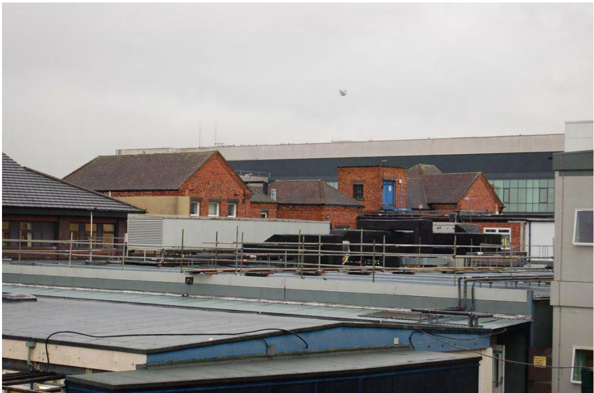
Plate 133: Building 52: long view from the south-east.
