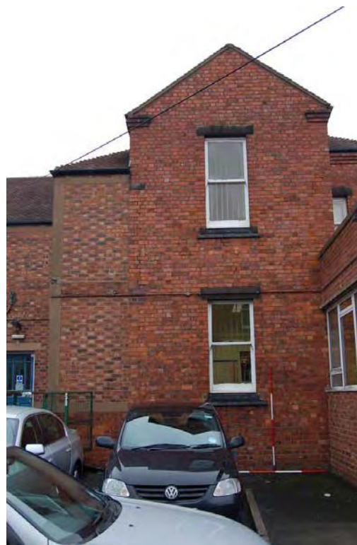
Plate 75: Bldg 29: south-west gable (note infill of veranda / balcony).
