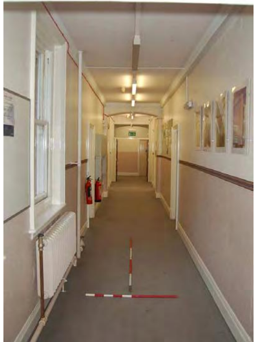
Plate 20: Bldg 23: 1F corridor (1F11).
