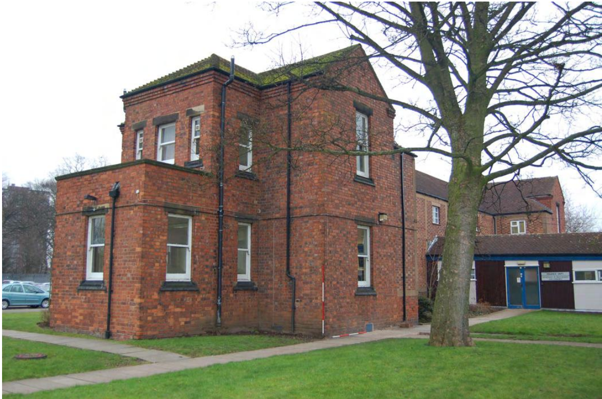
Plate 71: Building 29: north end and north-west gable.
