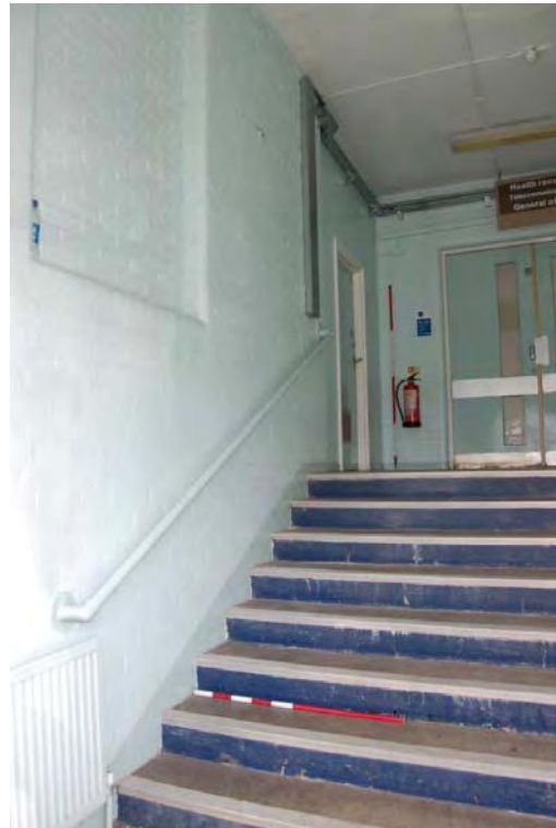
Plate 56: Bldg 28: West entrance (GF26).
