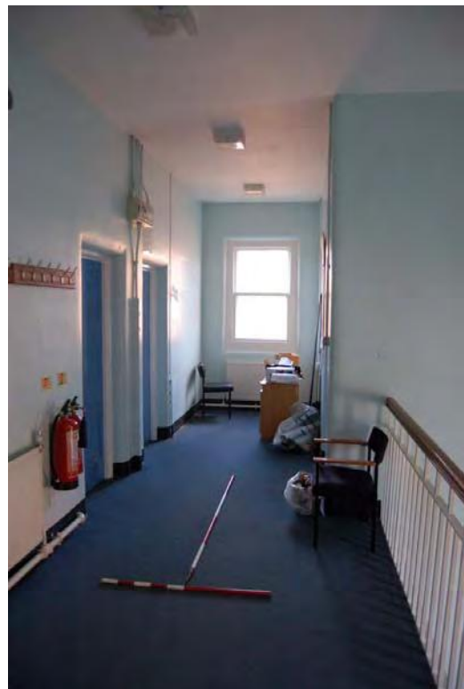
Plate 94: Bldg 29, 1F landing.
