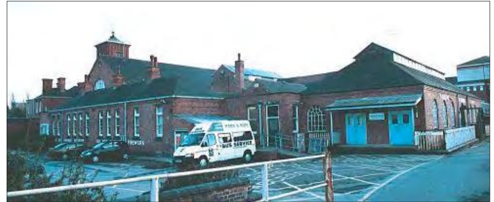
(c) Main Administration Block (compare Plate 34)
