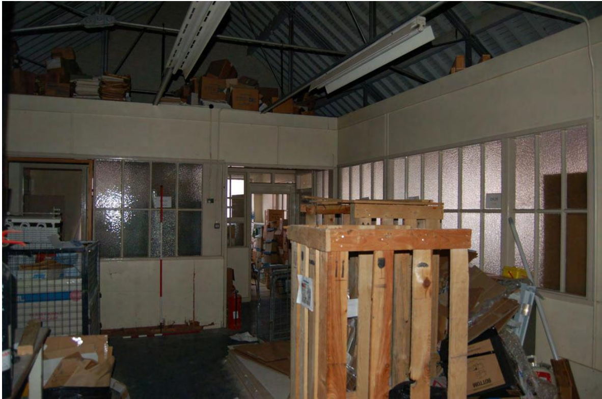
Plate 62: Building 28: rear range, partitioned area to west.
