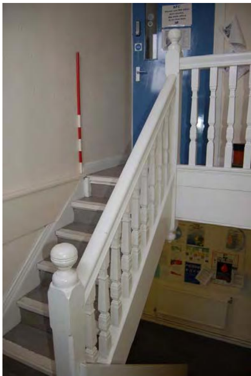
Plate 47: Bldg 28: stair at GF08/1F20.
