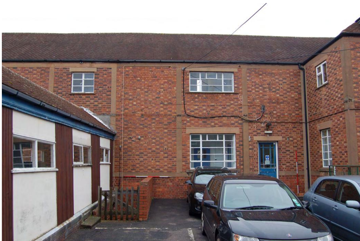
Plate 73: Building 29: west elevation, south end (note infill of veranda / balcony).
