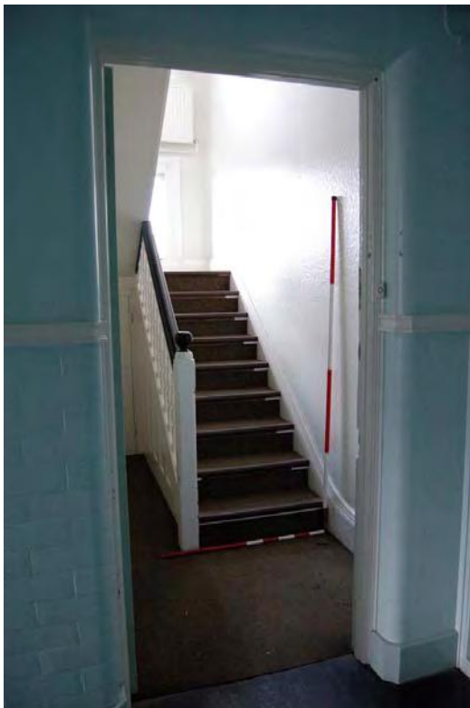
Plate 60: Bldg 28: stair GF25.
