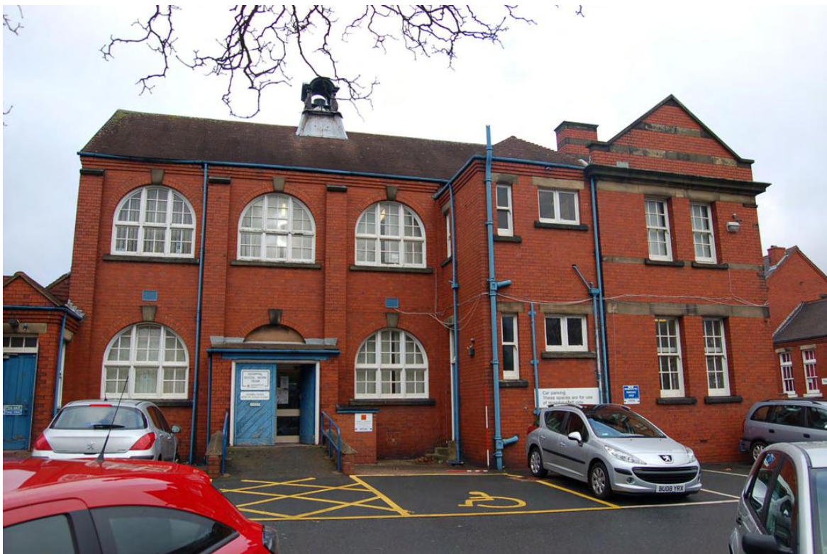
Plate 117: Building 37; south elevation.
