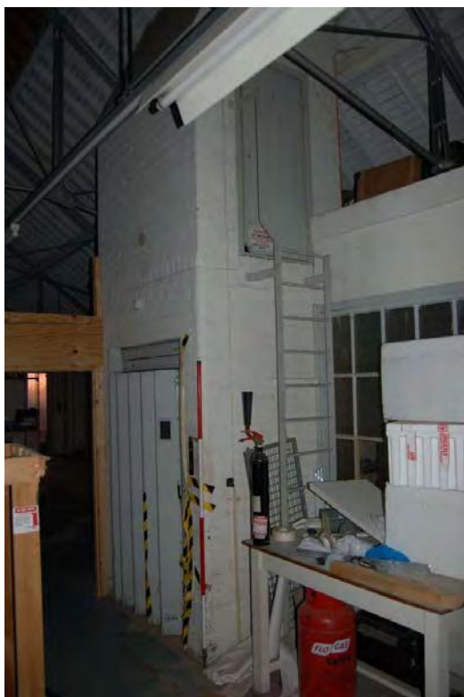
Plate 65: Bldg 28: rear range, lift.
