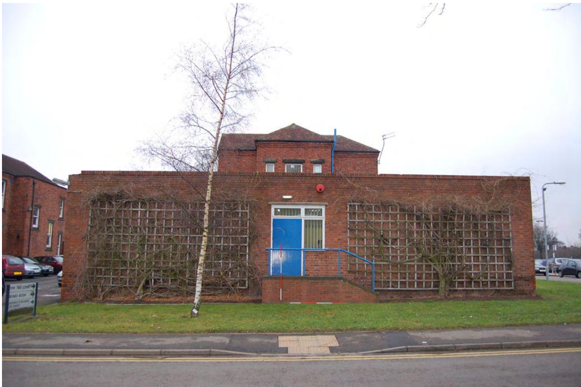
Plate 77: Building 29: south elevation.
