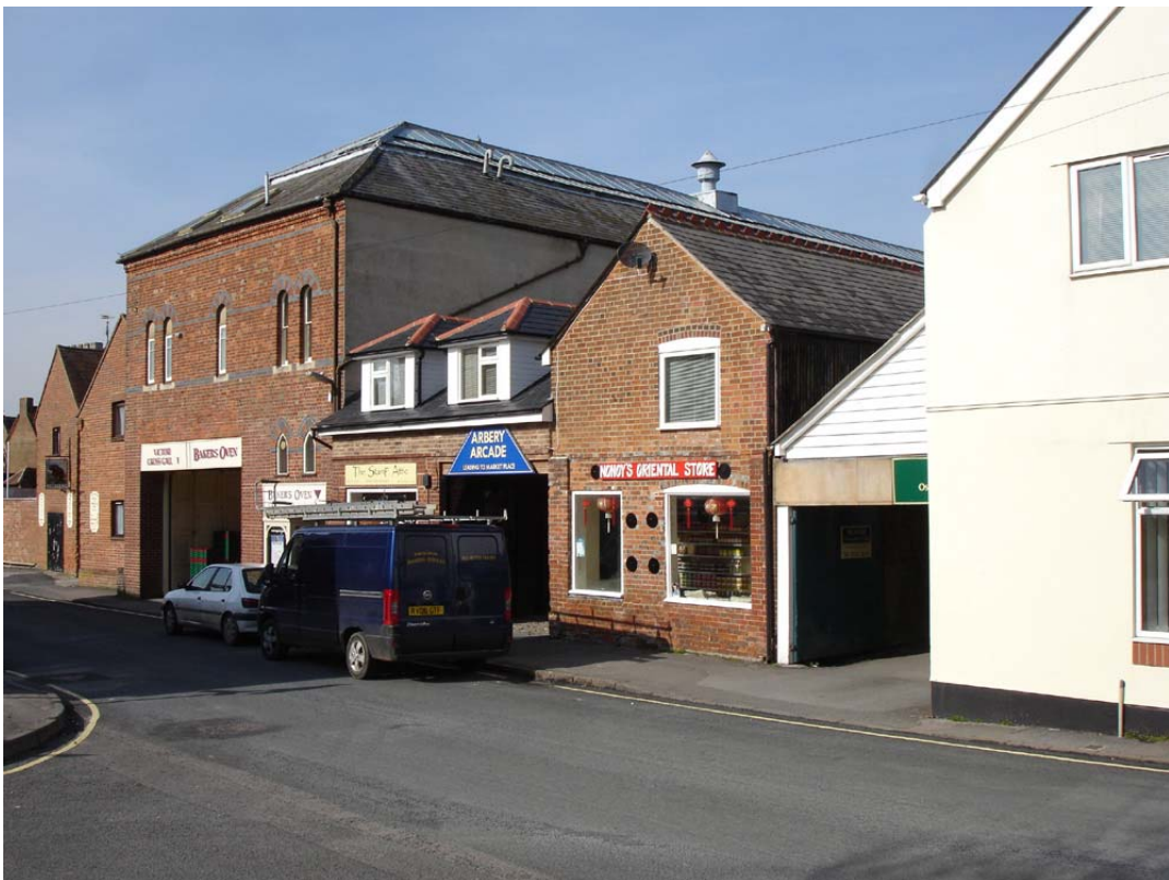
Plate 2: Church Street entrance to yard, note former Corn Exchange to left.
