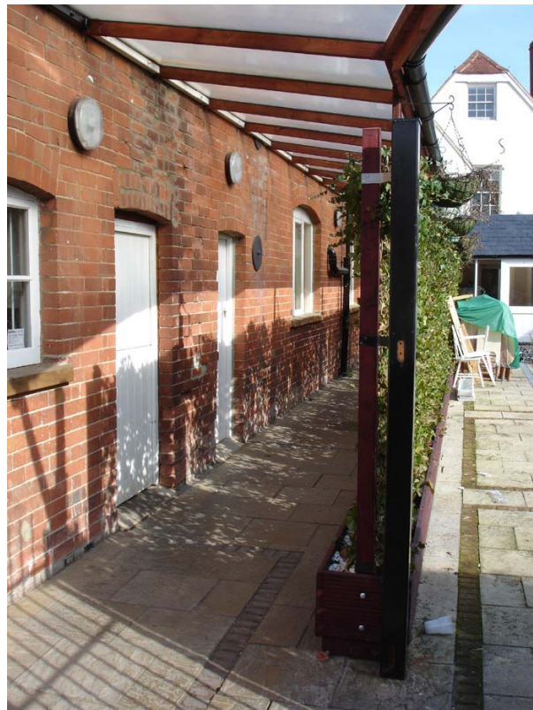
Plate 8: Passage looking north.
