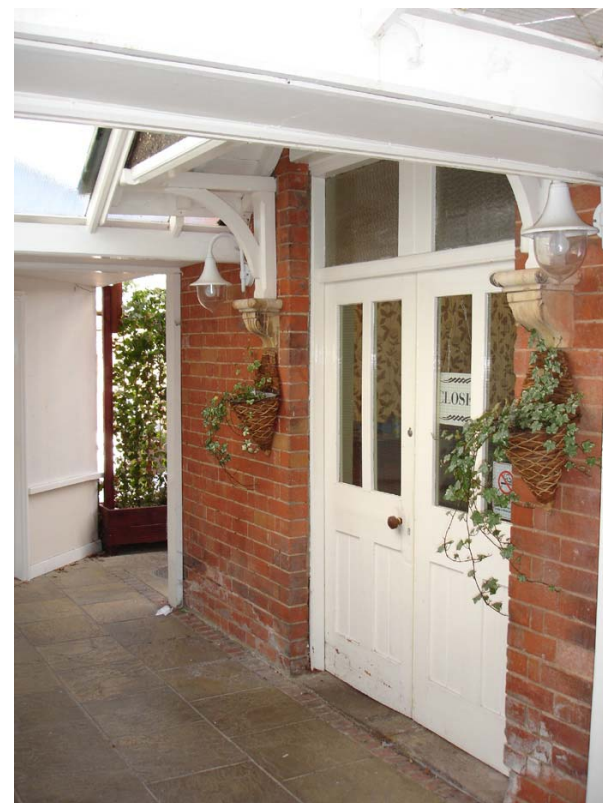
Plate 10: Workshop block, north end.
