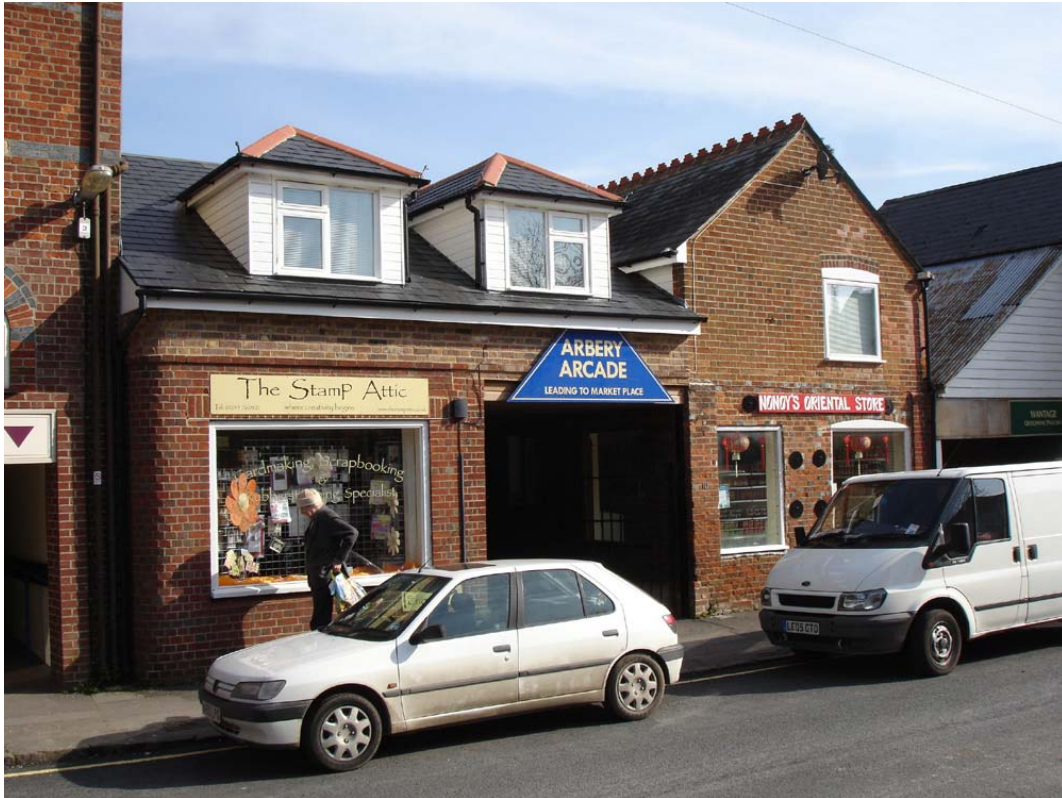
Plate 3: Detail of Church Street entrance.
