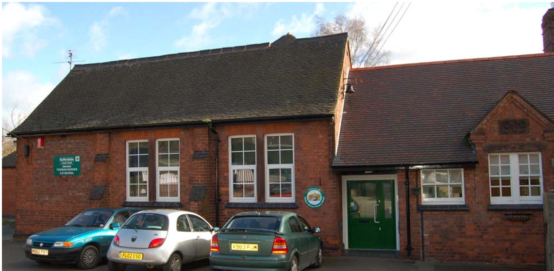
School 56: Thomas Barnes Primary School, School Lane, Hopwas, Tamworth (1875).
