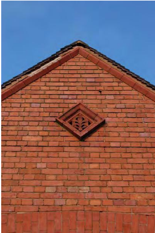
Plate 21: Terra-cotta panel in gable.
