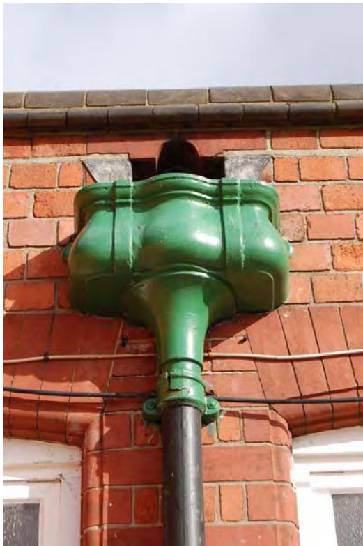
Plate 23: Primary rainwater hopper.
