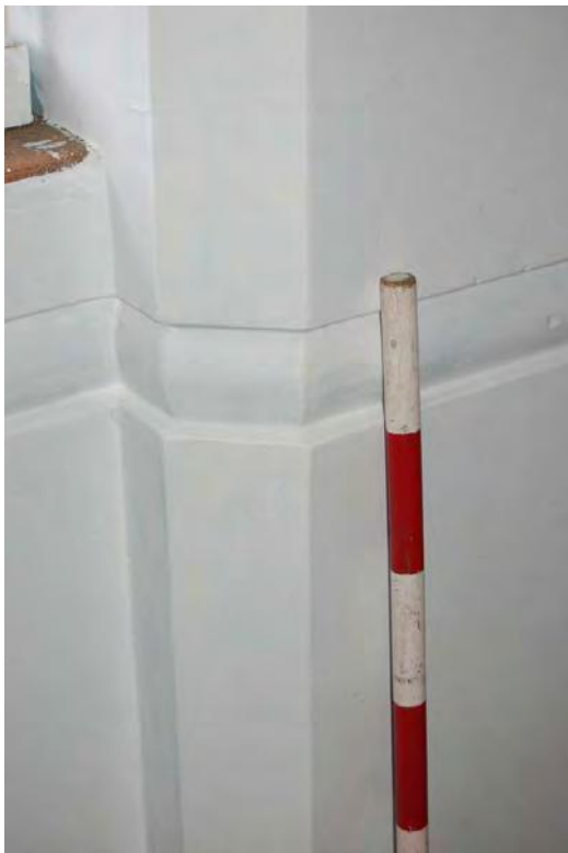
Plate 51: 1937/8, recessed dado detail.
