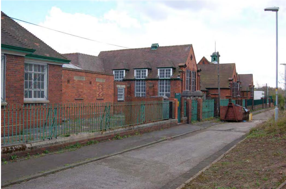
Plate 6: West elevation (L:1937-8/R:1905/6), oblique view looking south-west.
