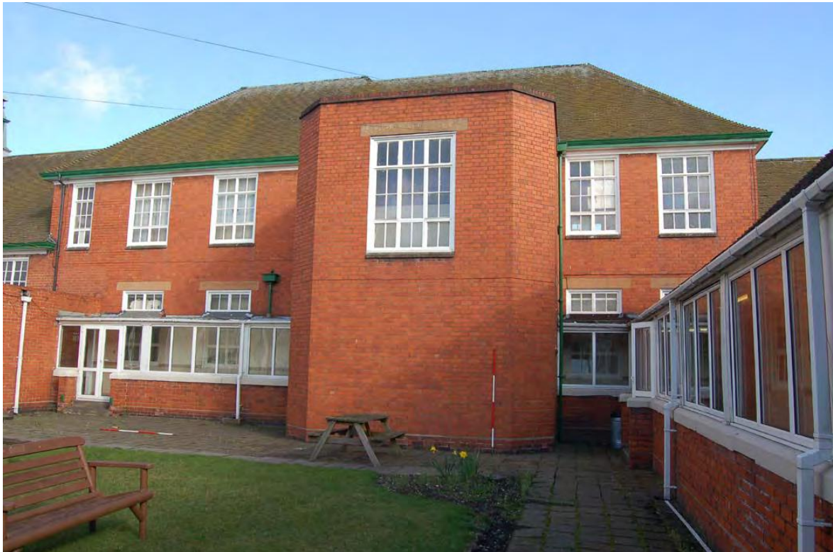
Plate 43: 1937/8 range, east block; rear elevation including stair.
