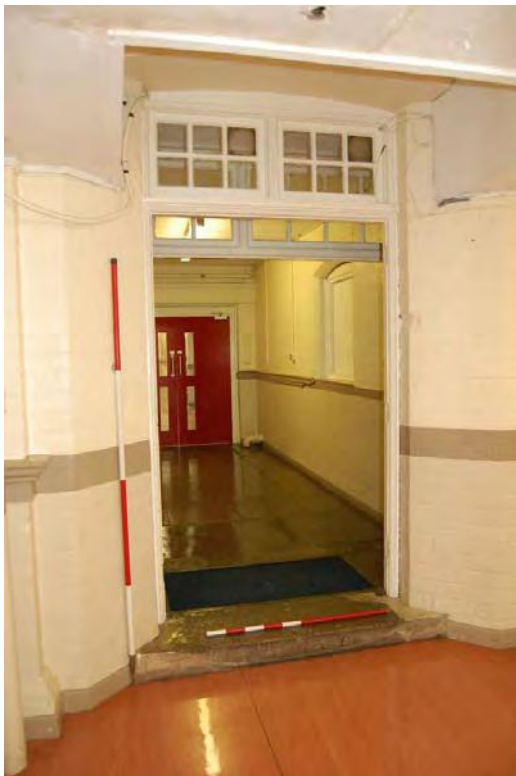
Plate 31: West range; former exterior door.
