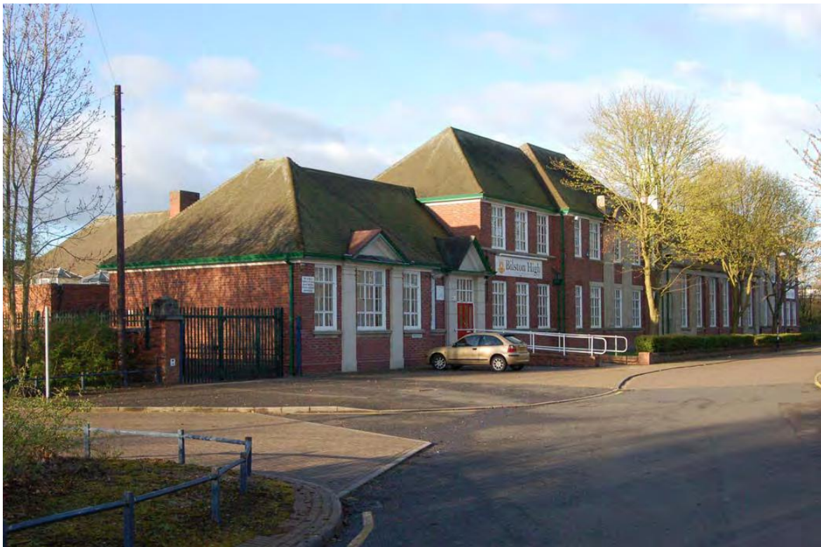
Plate 37: Prosser Street elevation (1937/8), oblique view looking south-east.
