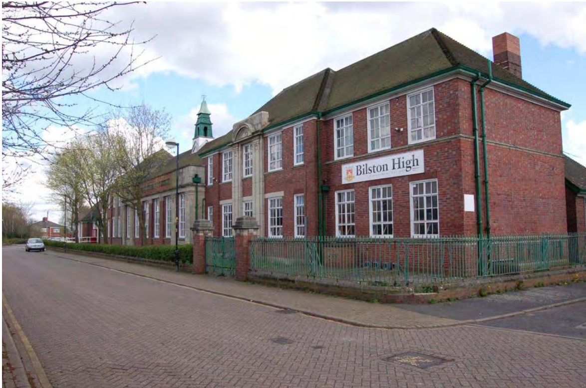
Plate 38: Prosser Street elevation (1937/8), oblique view looking south-west.
