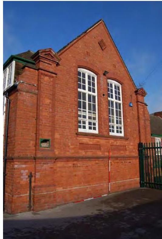
Plate 15: Eastern block, east elevation.
