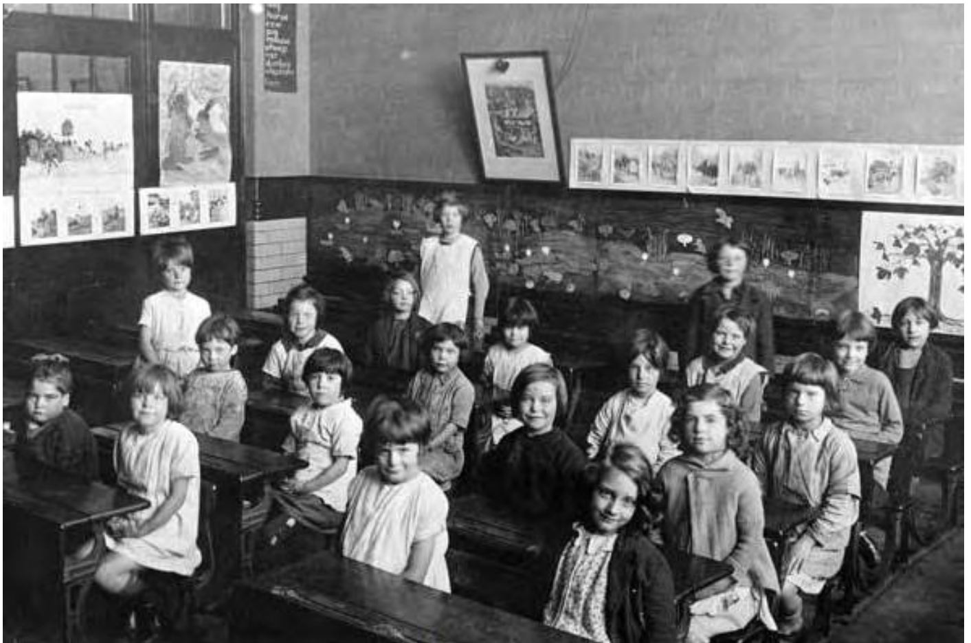
(b) Interior view of one of classrooms opening off girls hall. Note original glazed brick dado and half glazed hinged partitions (WALS P/6001).
