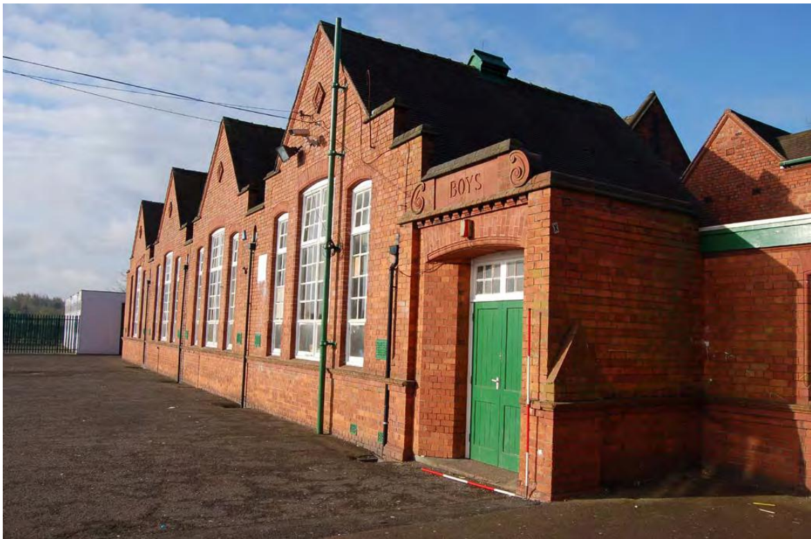
Plate 17: Western range; playground elevation, oblique view looking south-west.
