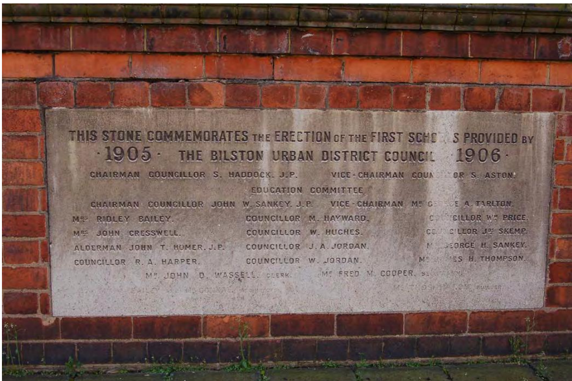
Plate 5: Dated foundation stone; north range, north elevation.
