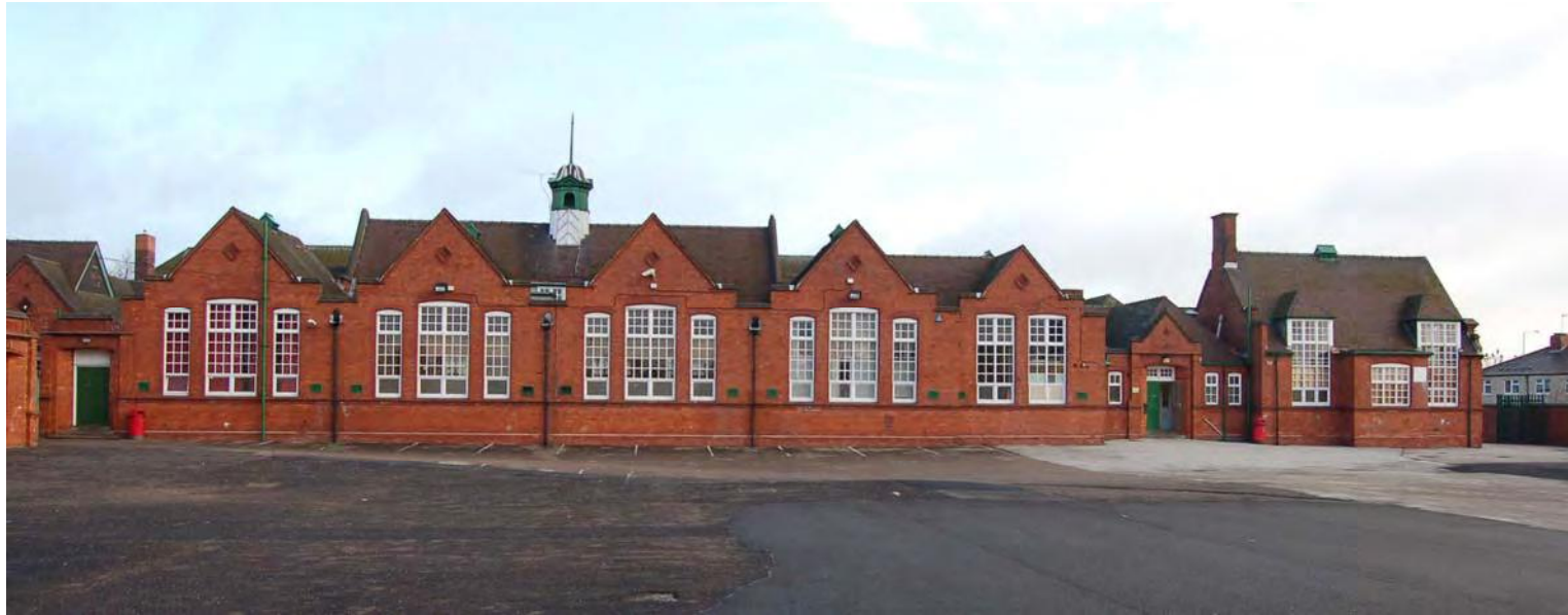
Plate 11: North range, playground elevation.
