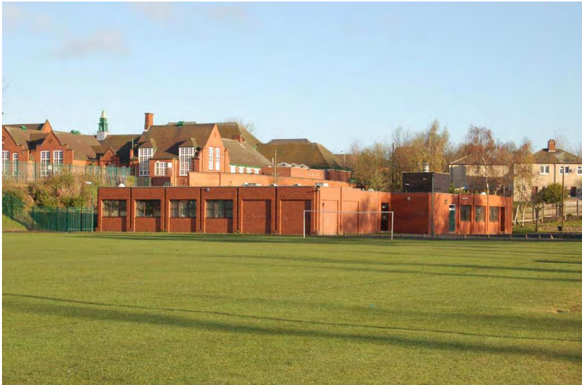
Plate 60: Modern science block, primary school buildings beyond, atop bank.
