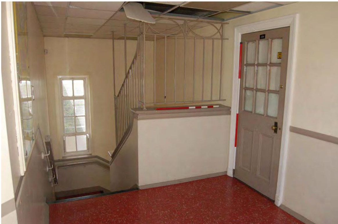
Plate 54: 1937/8 range; secondary stair at 1F level (064).
