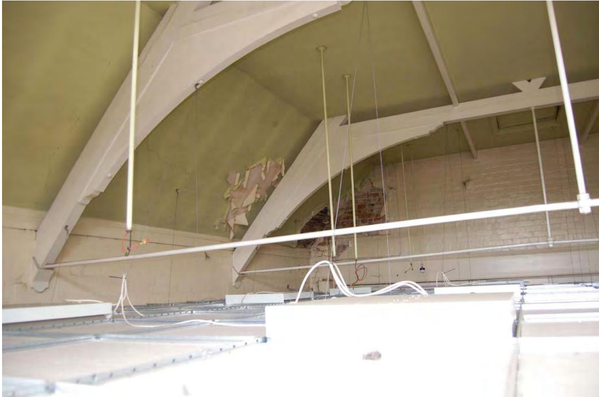
Plate 36: Primary roof structure above suspended ceiling.
