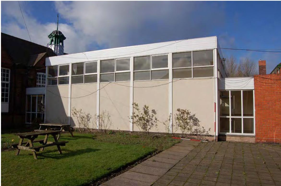
Plate 55: Unsympathetic infill block between 1938 range and northern 1905/6 range.
