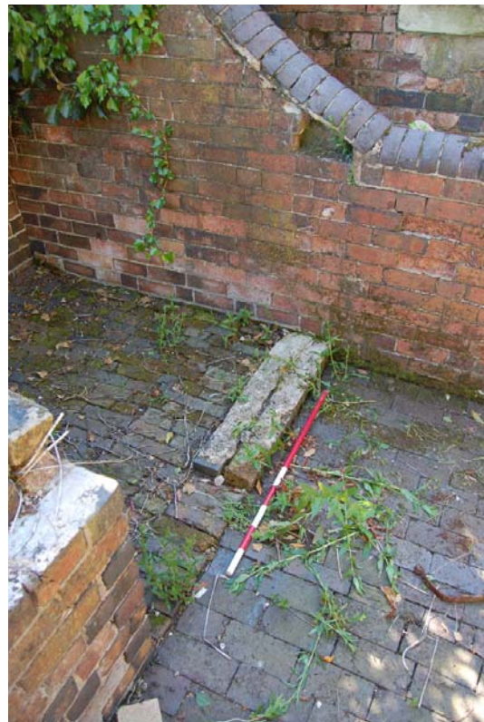
Plate 12: Former partition wall, 04/05.
