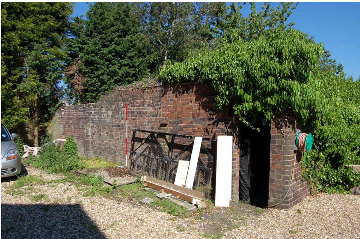
Plate 4: Outbuilding; south elevation oblique view from south-east.
