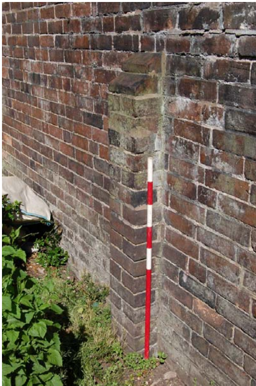
Plate 6: South elevation buttress detail.
