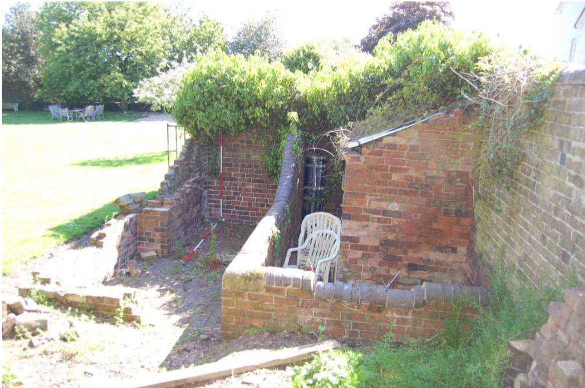
Plate 10: Outbuilding; west elevation; cells 04/05 to left, 01-03 to right.
