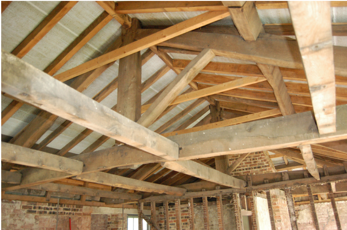
Plate 93: King-post roof structure over Room F4.
