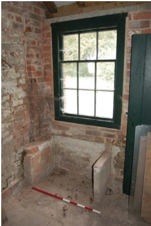
Plate 77: Room G8, looking north.
