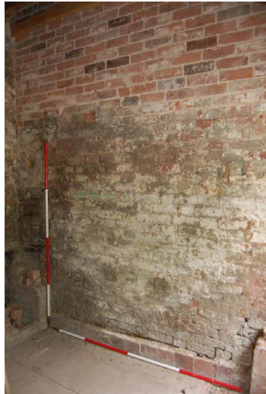
Plate 78: Room G8, west wall.
