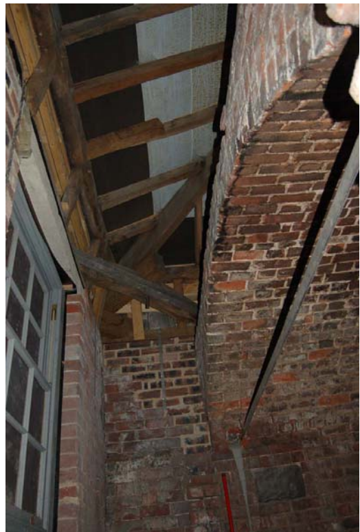
Plate 98: Room F2, brick vault.
