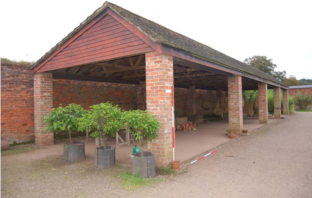
Plate 22: North garden, south wall (west); general oblique view looking south-west.
