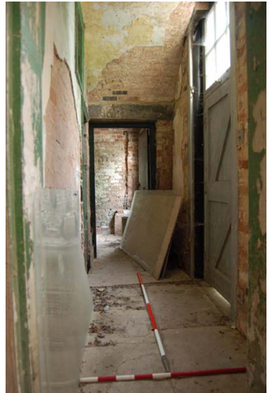
Plate 71: Room G6, looking west.
