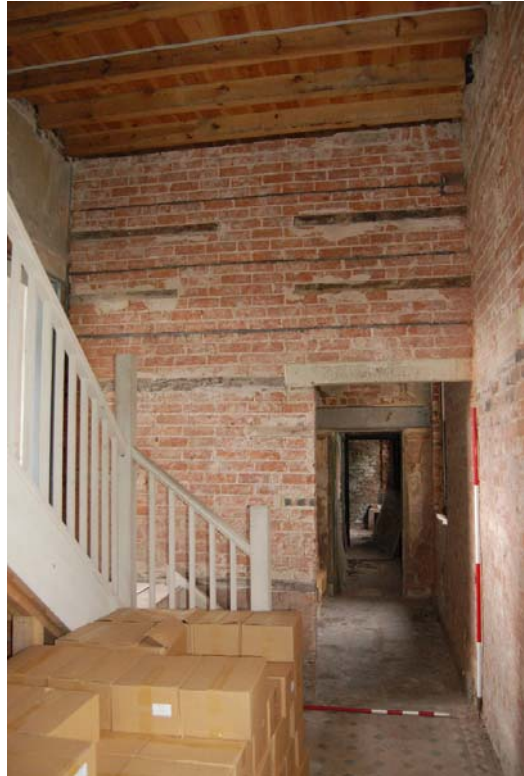
Plate 52: Room G3, looking west.
