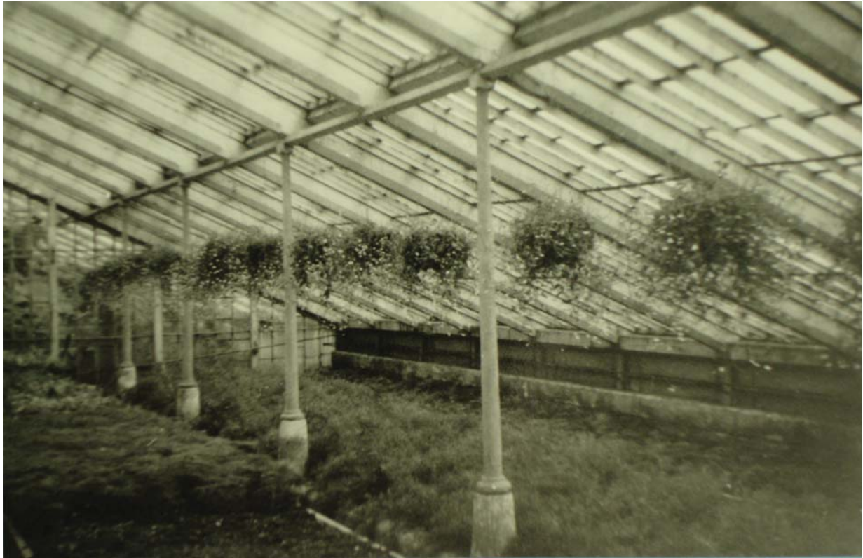
(a) North-east vinery; interior looking south-east c.1940 (SAMS Acc. No. FP11.3.84)
