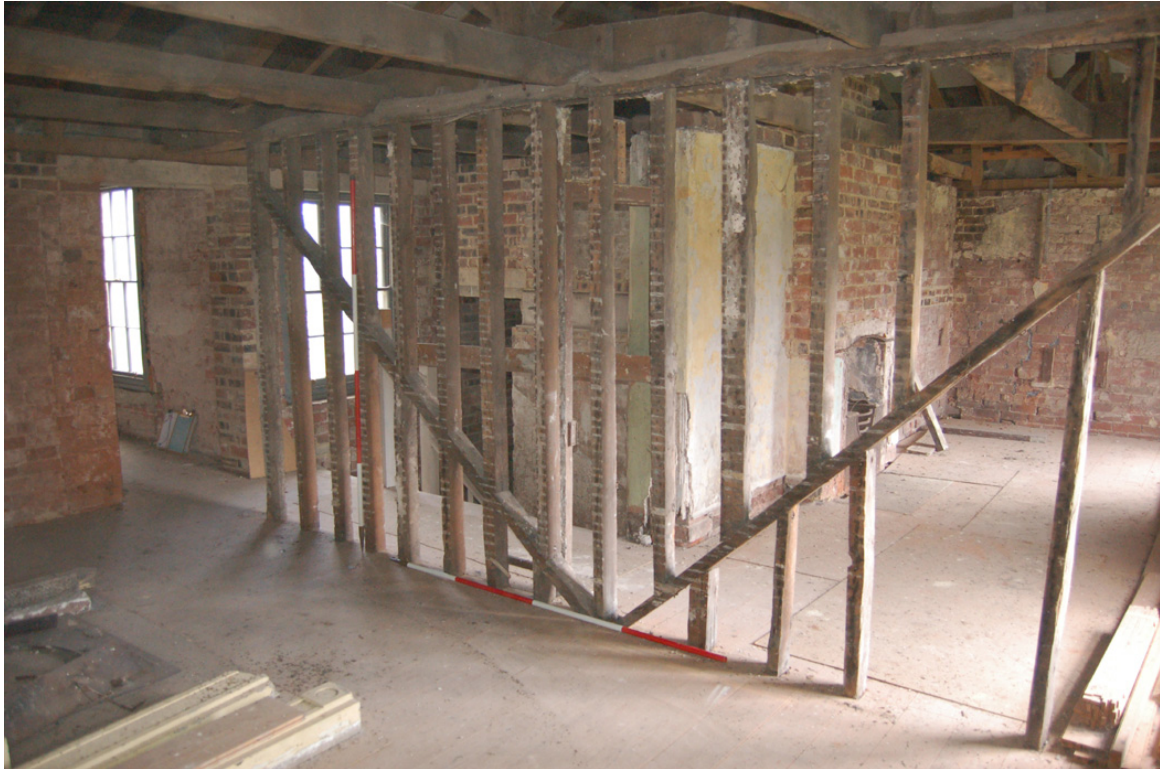
Plate 85: Room [F4], east studwork wall.
