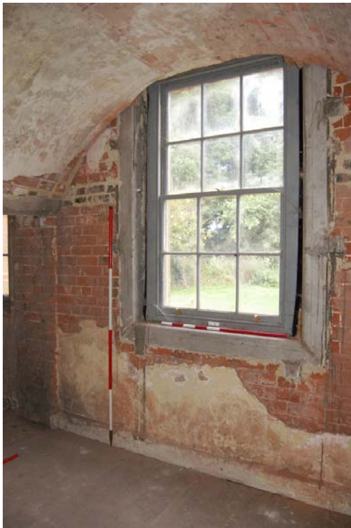
Plate 58: Room G2, north wall.
