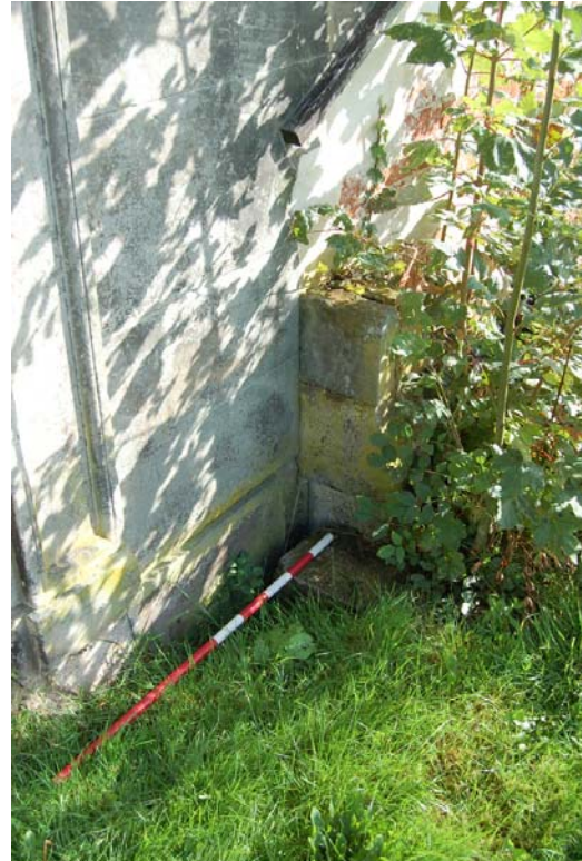
Plate 34: Stub of stone glasshouse wall.
