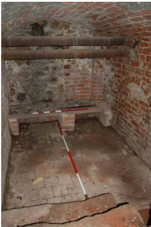
Plate 74: Basement Rm B7, looking south.
