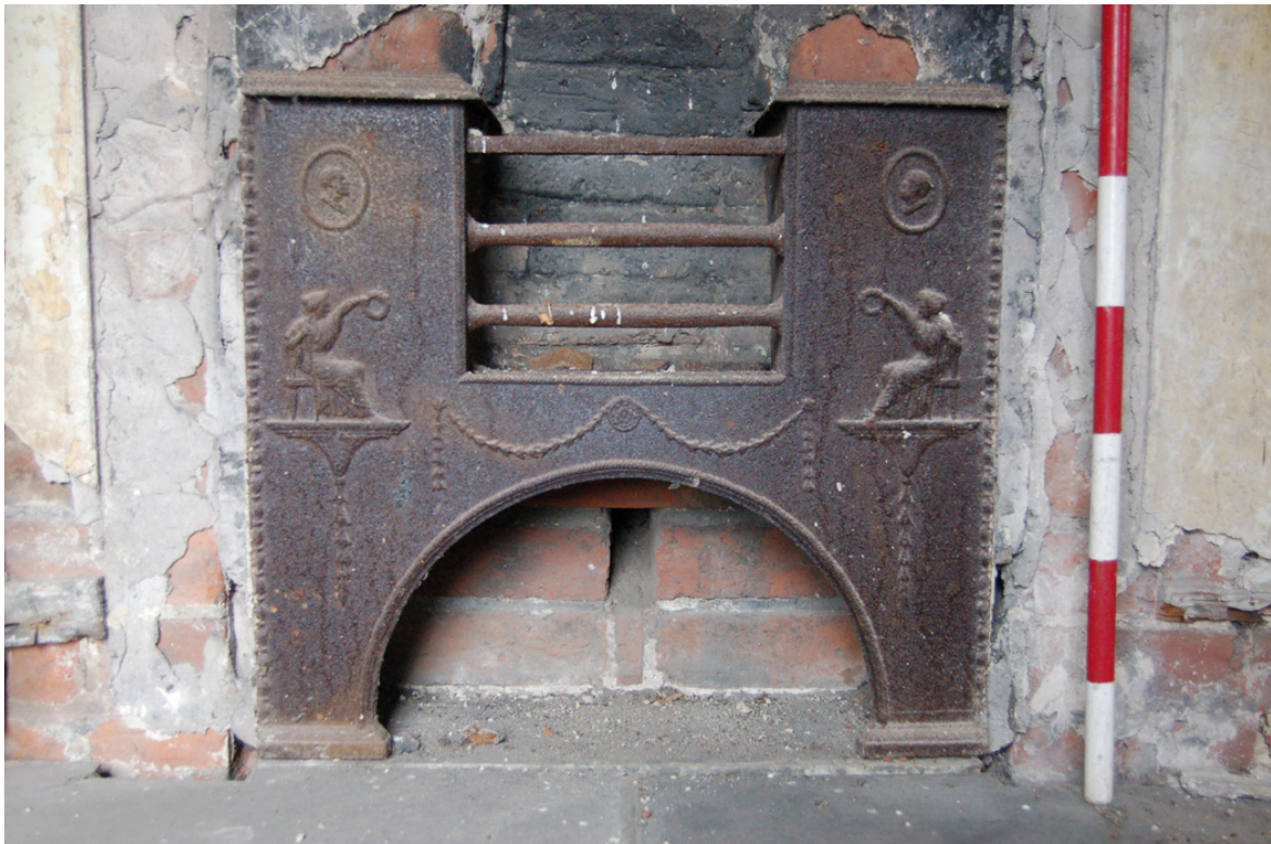
Plate 89: Room F5, detail of early-19 th -century hob-grate [f11].
