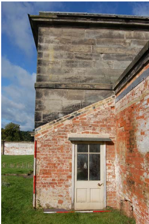
Plate 31: Gardener's House, east elevation.
