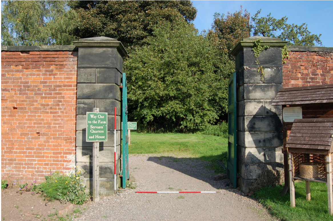
Plate 15: North Garden, east wall; gateway.
