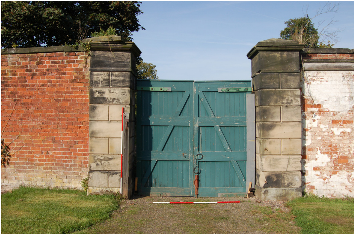
Plate 7: North garden, west wall; gateway.
