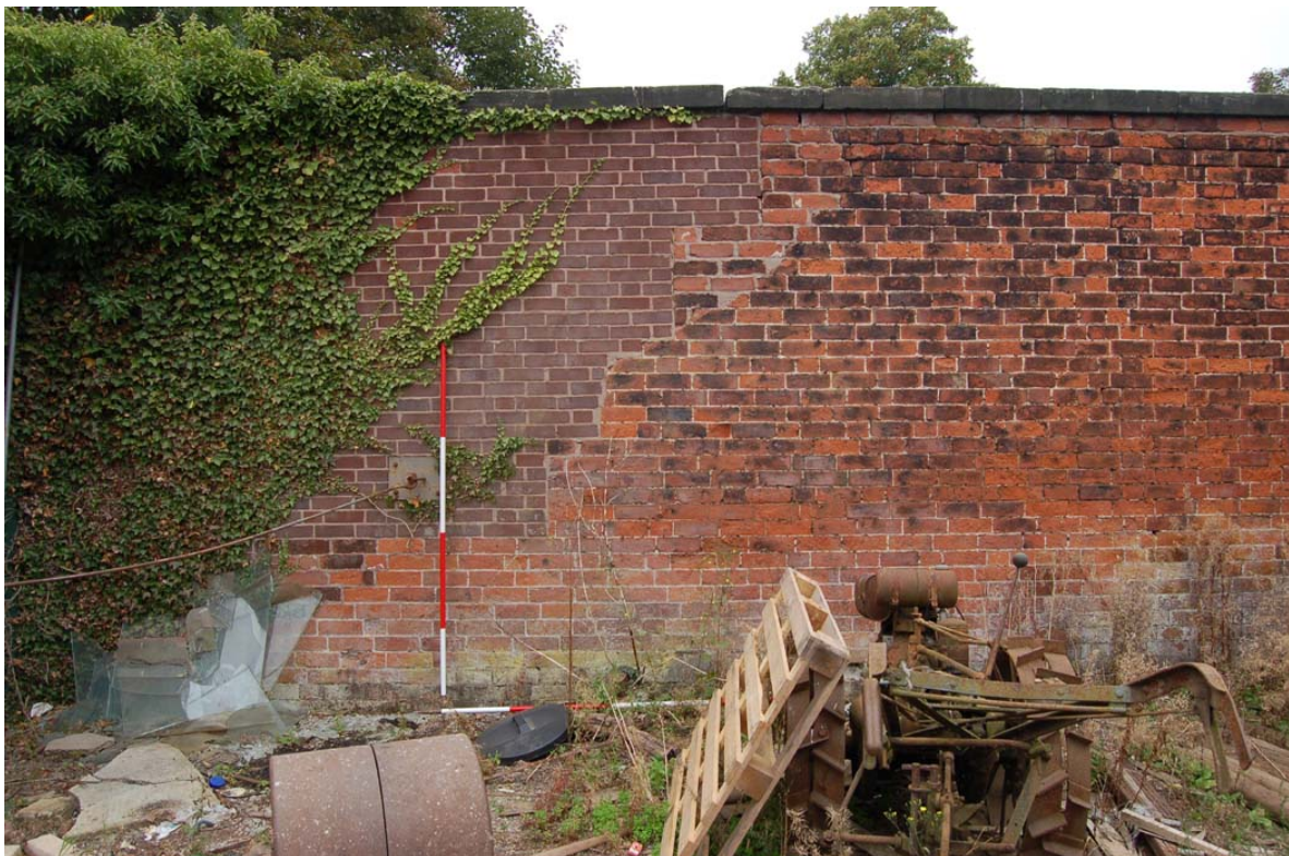
Plate 143: South garden, west wall; rebuilt wall north of gateway.
