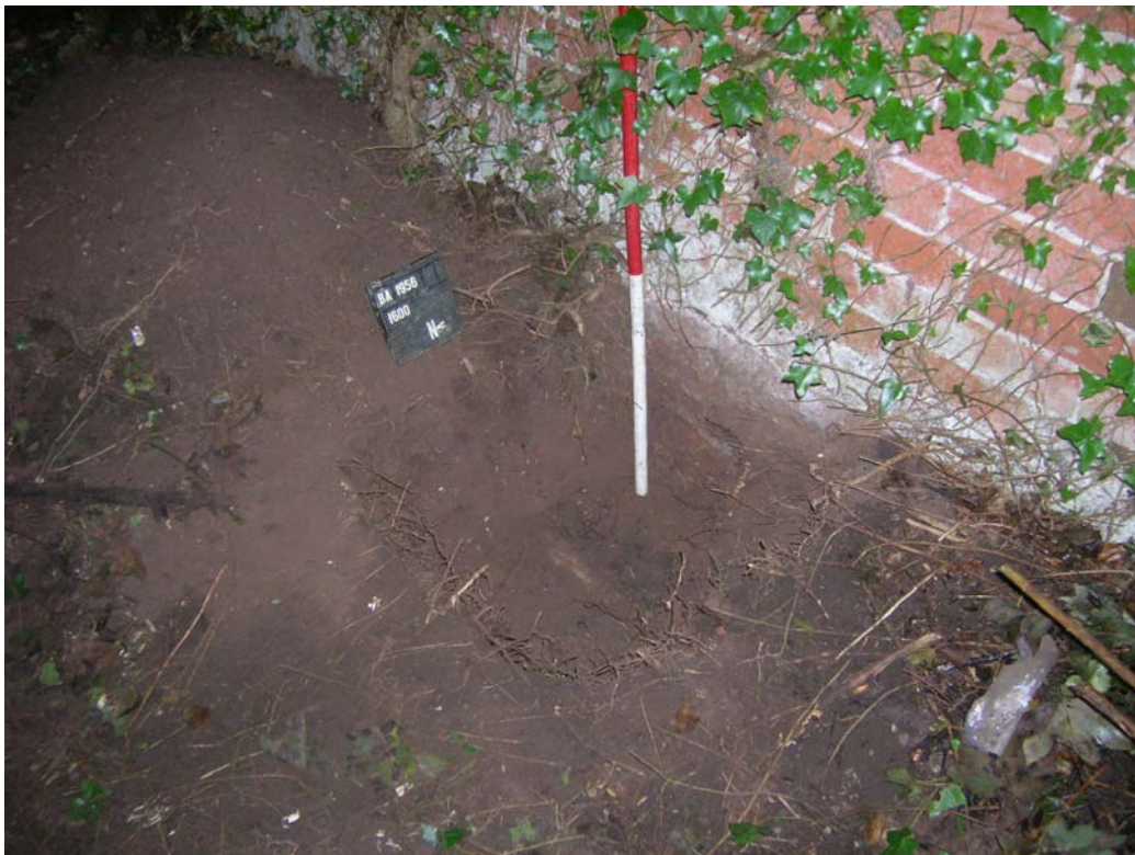
Plate 187: TP16; foundation of annex garden, north wall.
