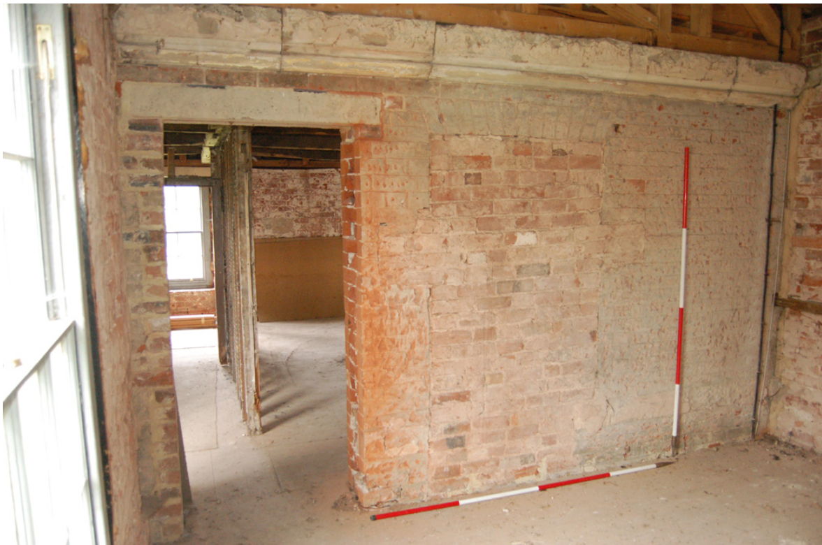
Plate 103: Rm. F6, south wall, note former exterior cornice detail.
