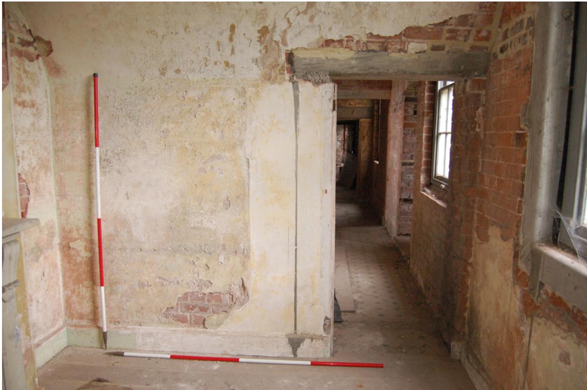
Plate 57: Room G2, west wall.
