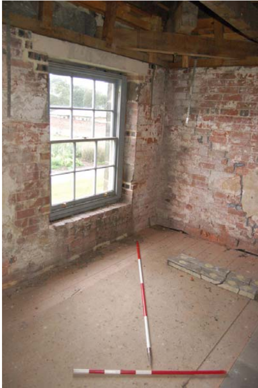
Plate 87: Room F5 looking south-west
