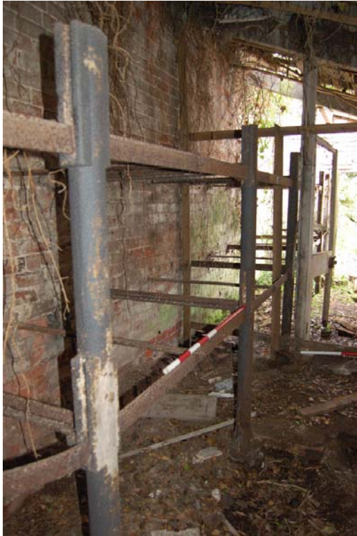
Plate 155: Potato Store, iron racking.
