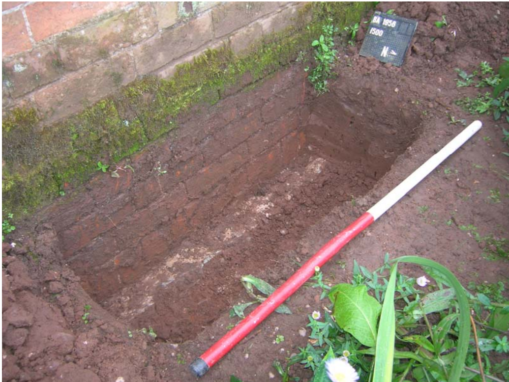
Plate 186: TP15; foundation of north walled garden, south wall.
