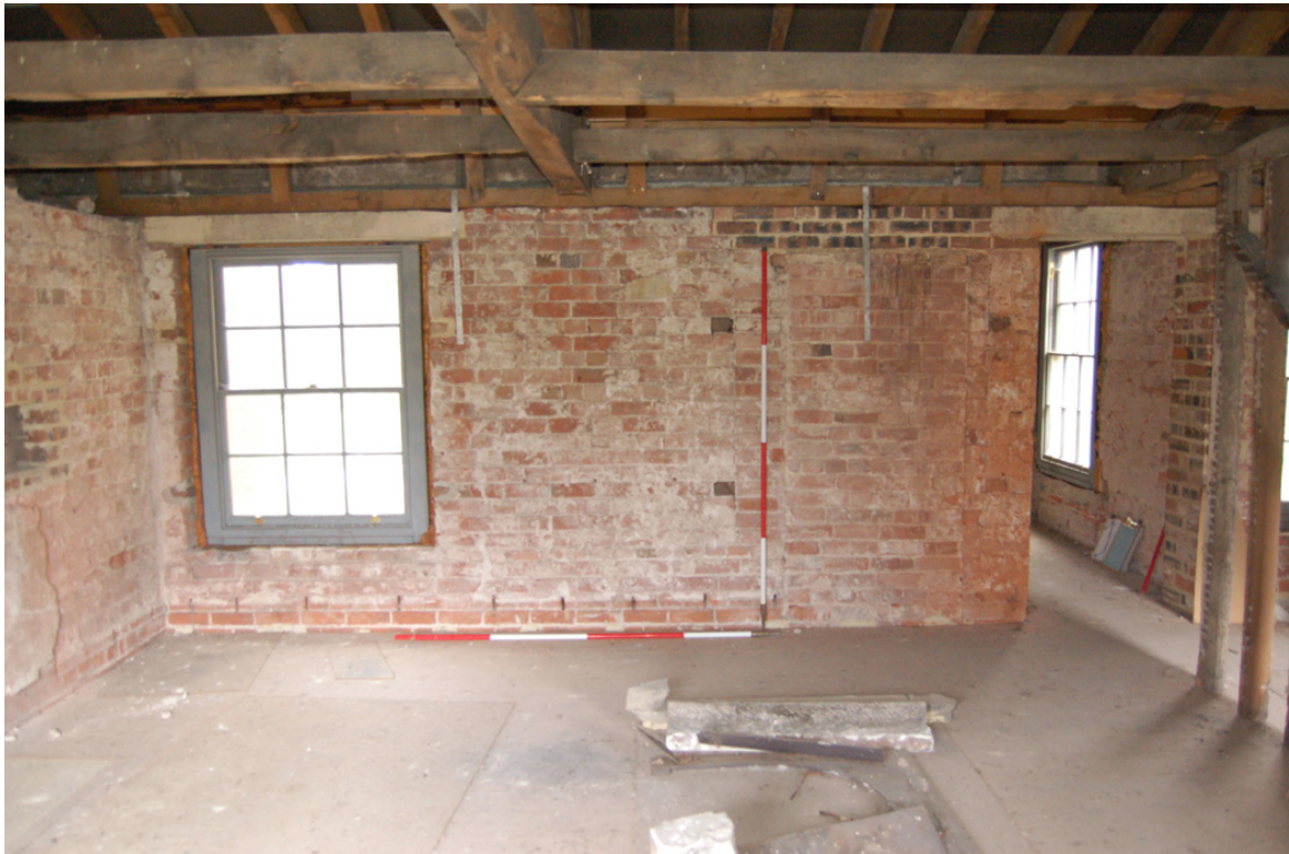
Plate 83: Room [F4], north wall.
