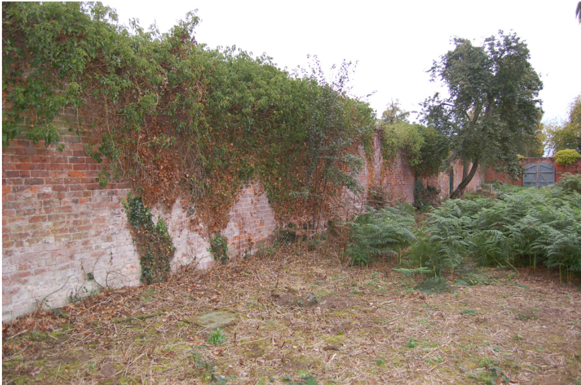
Plate 146: East annex garden, west wall general view looking north-west.
