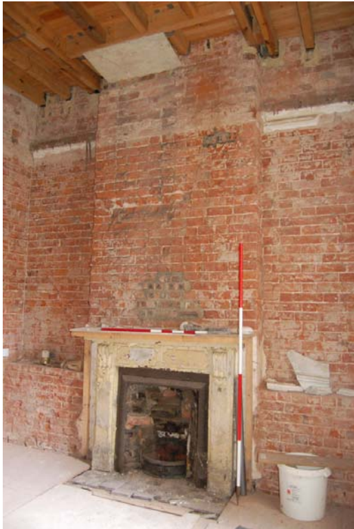
Plate 64: Room G5, north wall.
