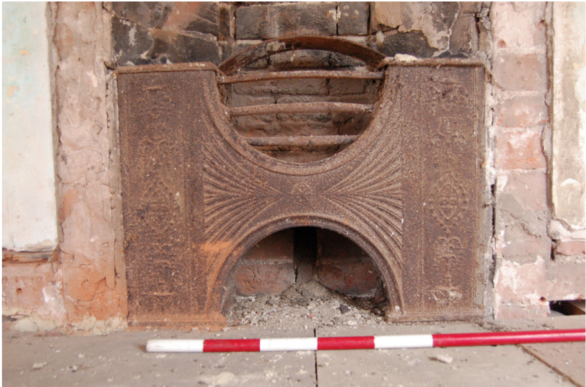
Plate 92: Room F3/7, detail of early-19 th -century hob-grate [f10].
