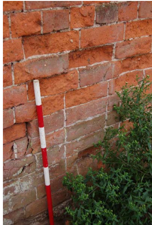
Plate 20: Flue access point.
