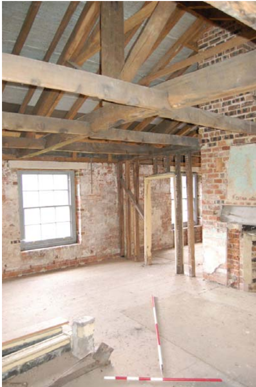
Plate 81: Room [F4] looking south-west.
