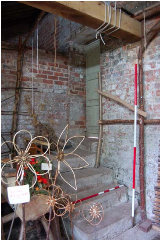
Plate 112: Rm G11; stair at SE corner.
