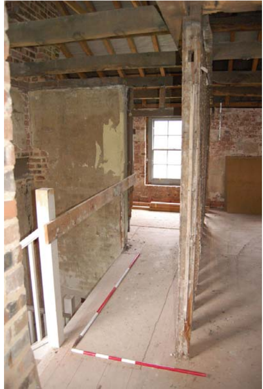
Plate 80: Landing at head of stair.
