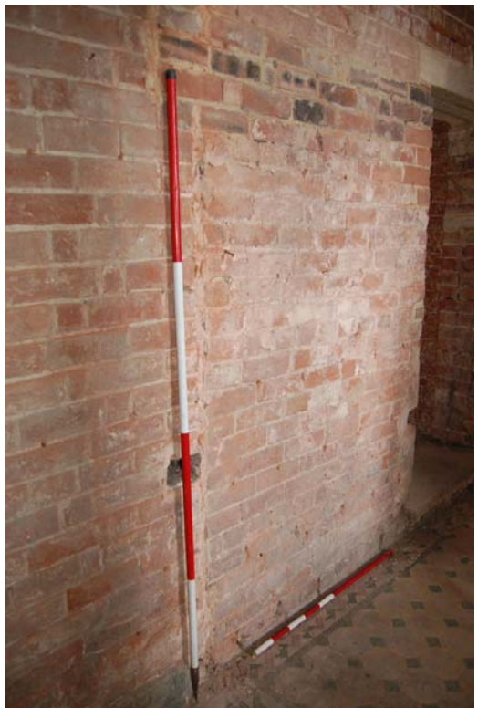
Plate 54: Room G3, blocked door.
