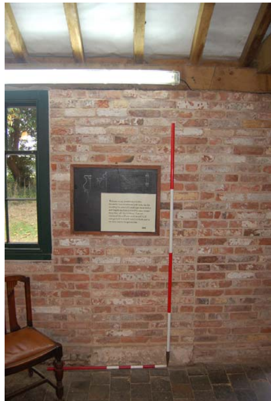
Plate 128: Rm G17 blocked door (N wall).
