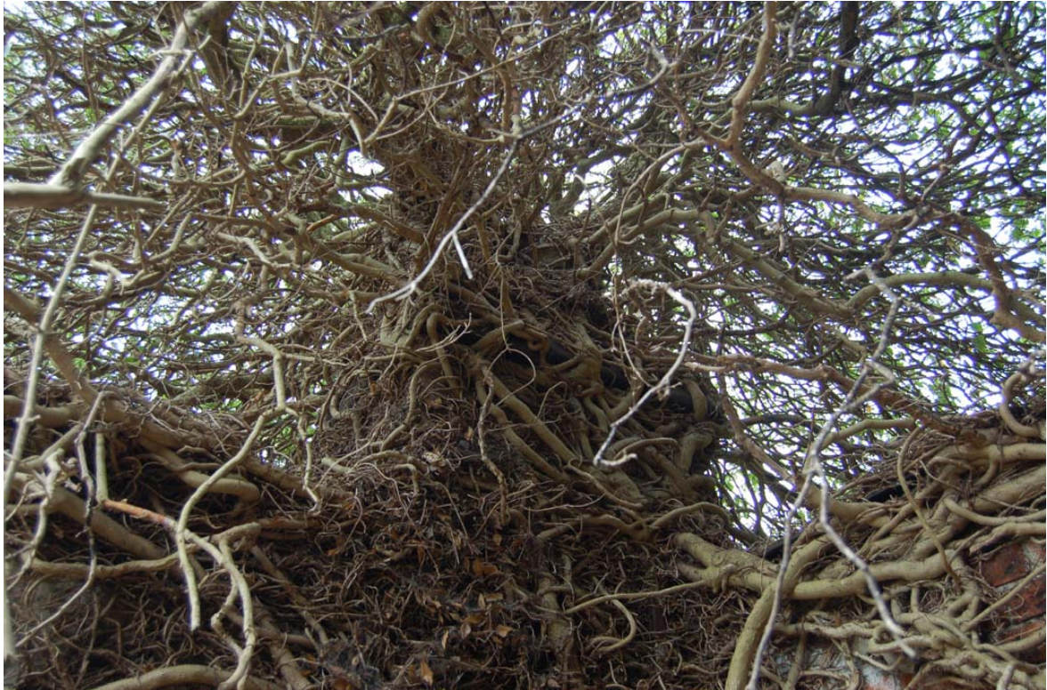
Plate 164: Stack at east end of wall, heavily obscured by vegetation.
