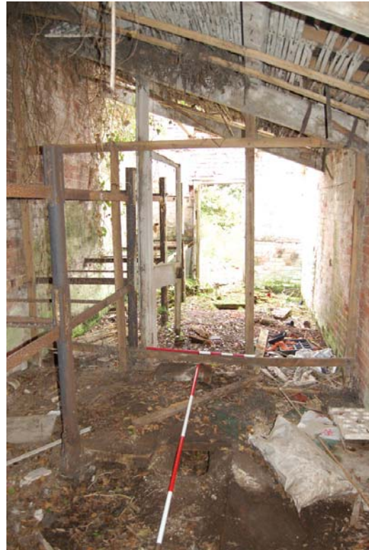
Plate 154: Potato Store, interior looking W.
