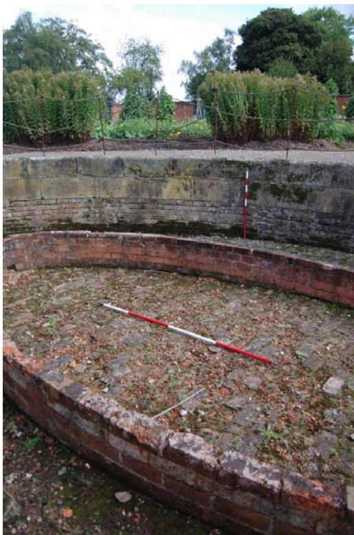
Plate 25: North dipping pool looking NE.
