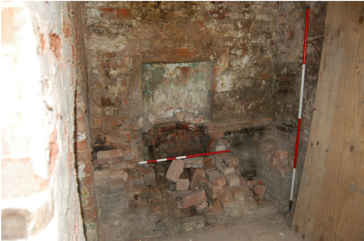
Plate 76: Room G8, south wall; setting for copper.
