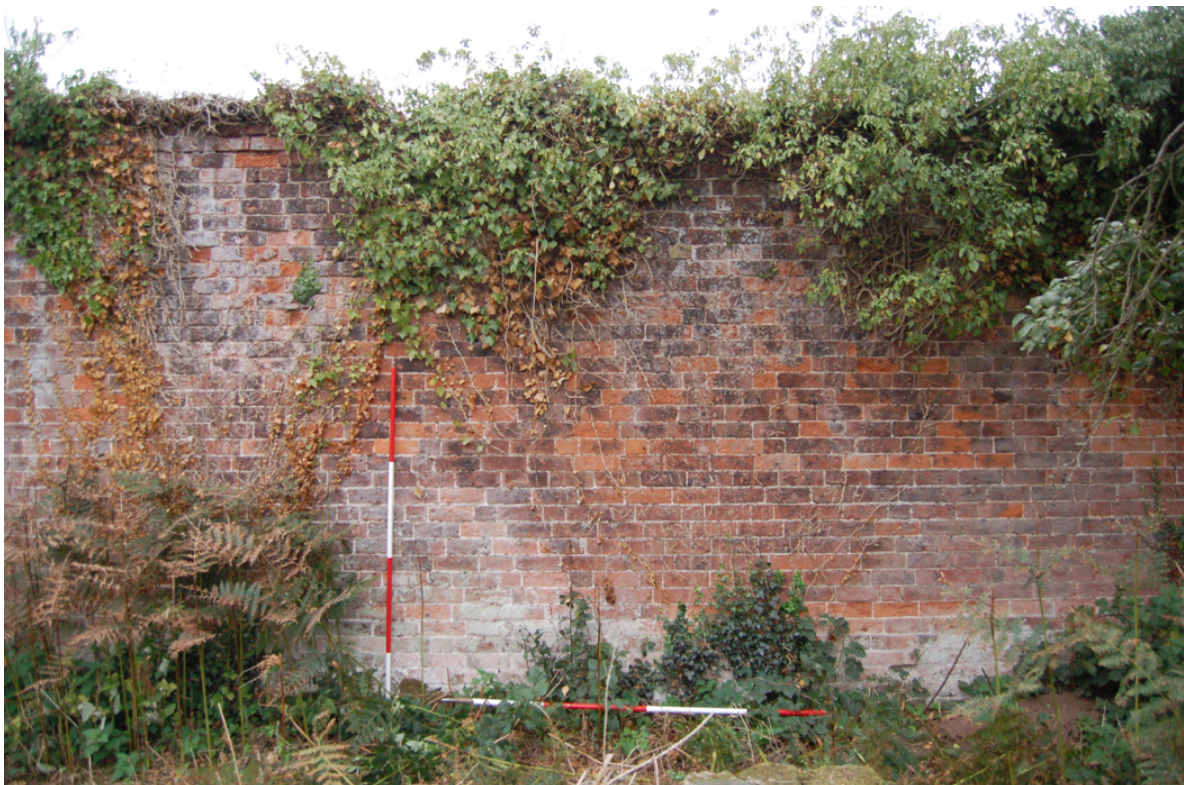
Plate 147: East annex garden, west wall; representative section of walling.
