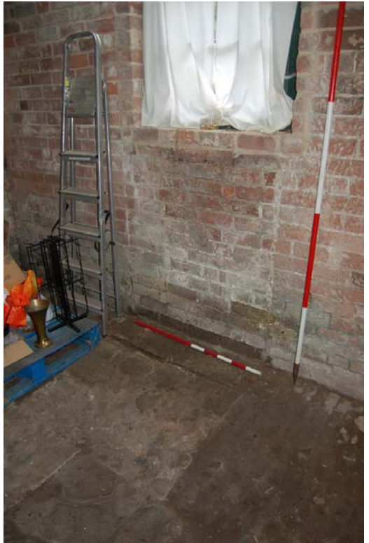
Plate 121: Rm G13, semi-blocked doorway.
