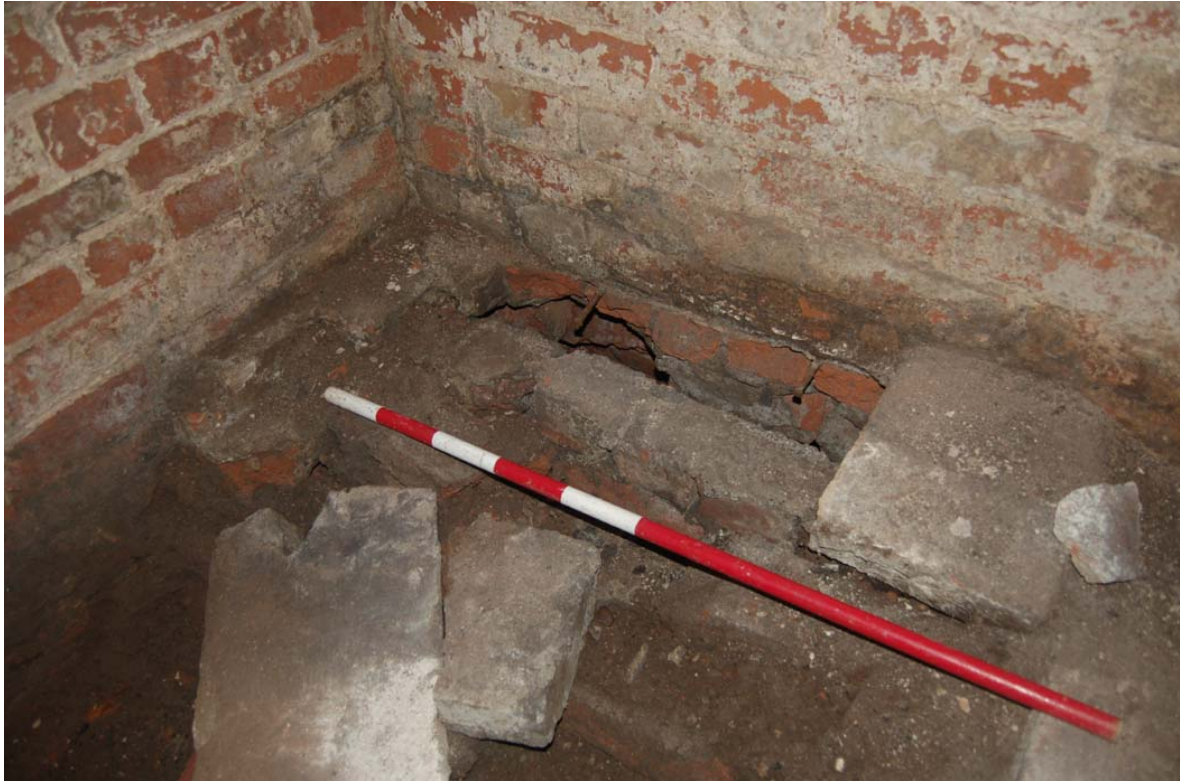
Plate 44: Room B1; primary flue at western end.
