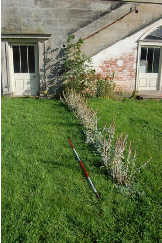
Plate 33: Line of western glasshouse wall.
