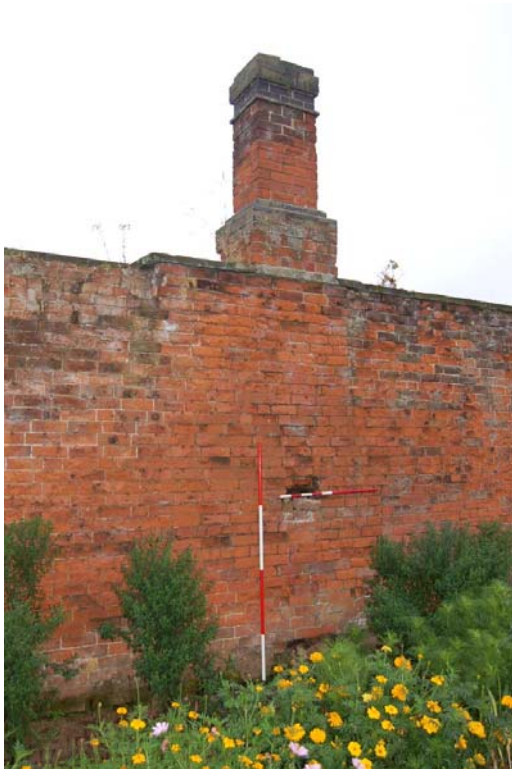
Plate 19: Stack in hot wall.
