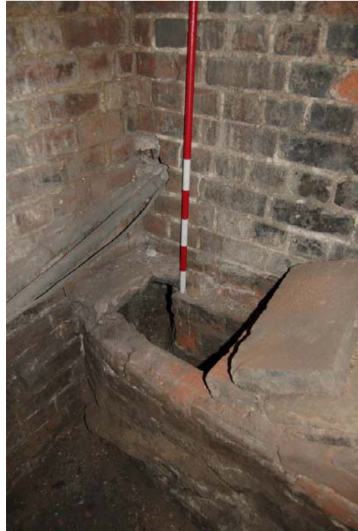
Plate 100: Room F2, flue to E of stack.
