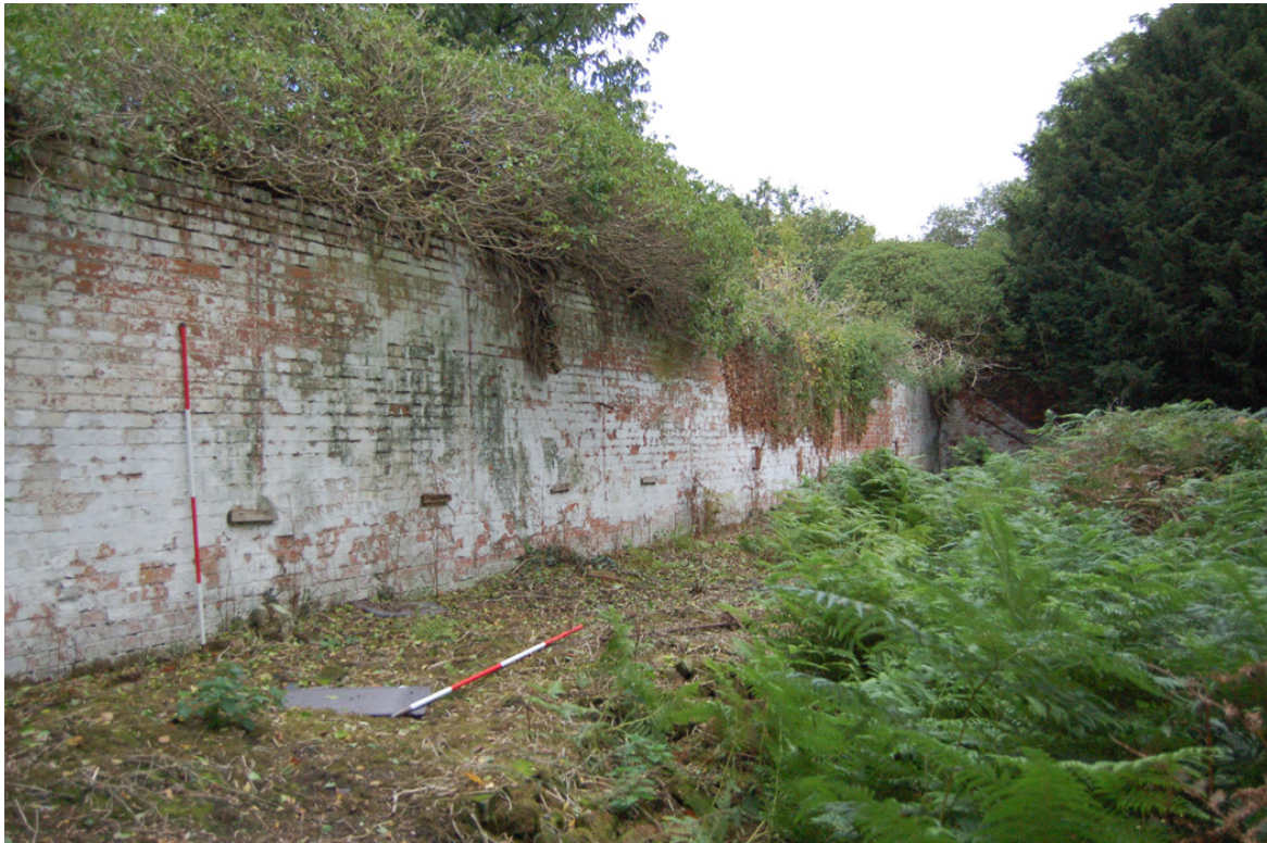
Plate 162: South-east garden, north wall; oblique view looking north-east.
