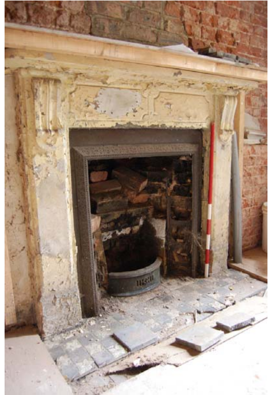
Plate 69: Room G5, fireplace.
