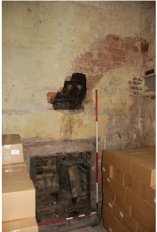
Plate 63: Room G4, south wall range.
