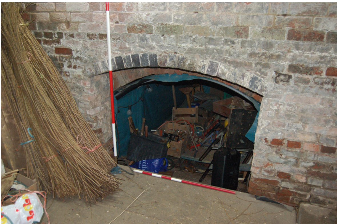
Plate 115: Rm B5; arched opening to coal store.
