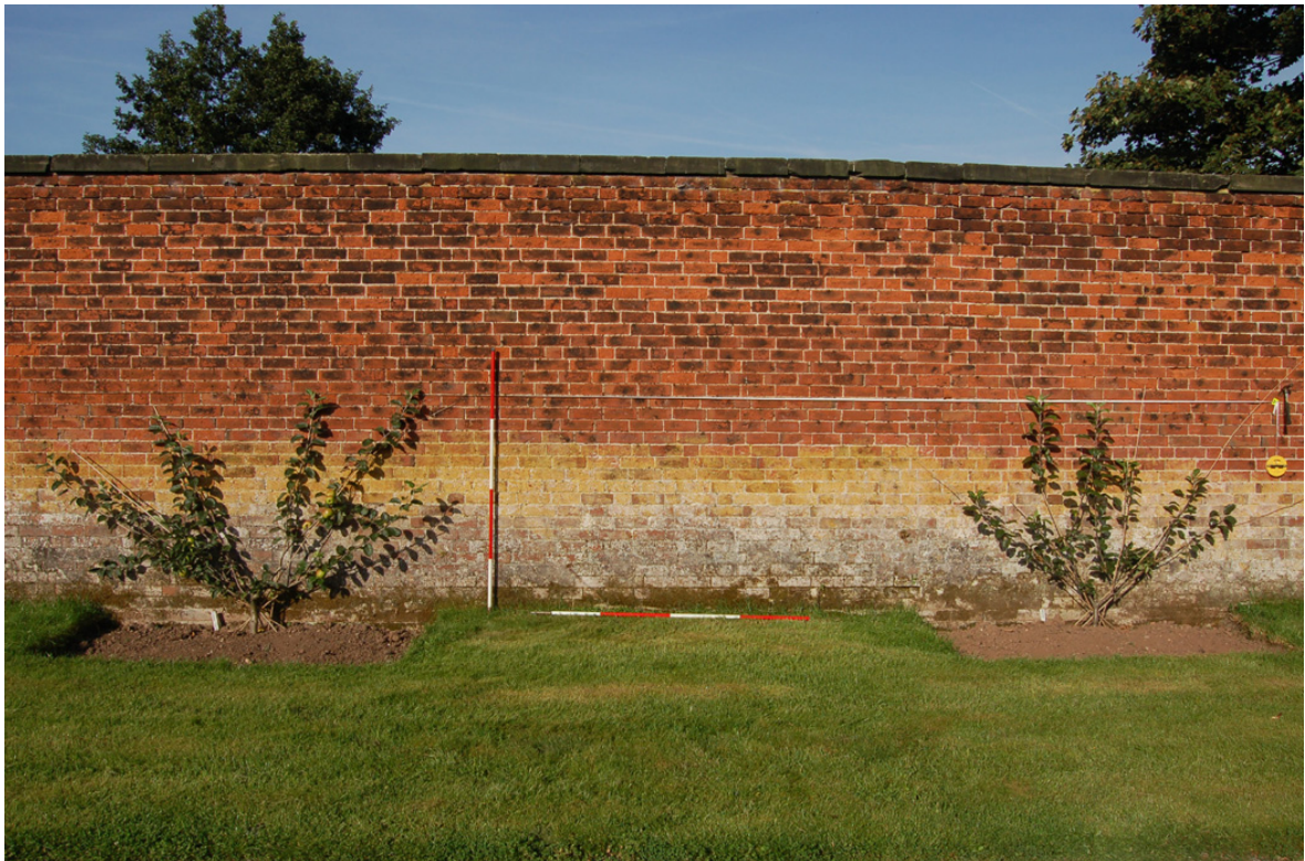
Plate 6: North garden, west wall; representative section of brickwork.
