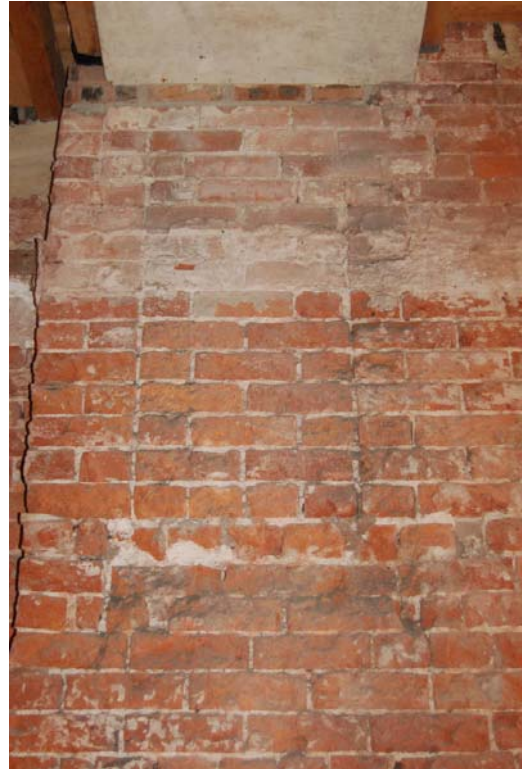
Plate 65: Room G5, upper flue (blocked).
