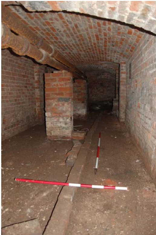
Plate 41: Room B1, looking west.
