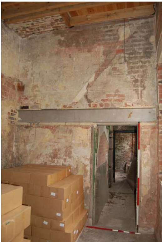
Plate 62: Room G4, west wall.
