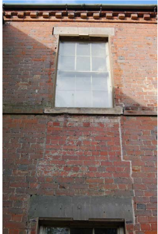
Plate 39: N Extension; blocking in east wall.
