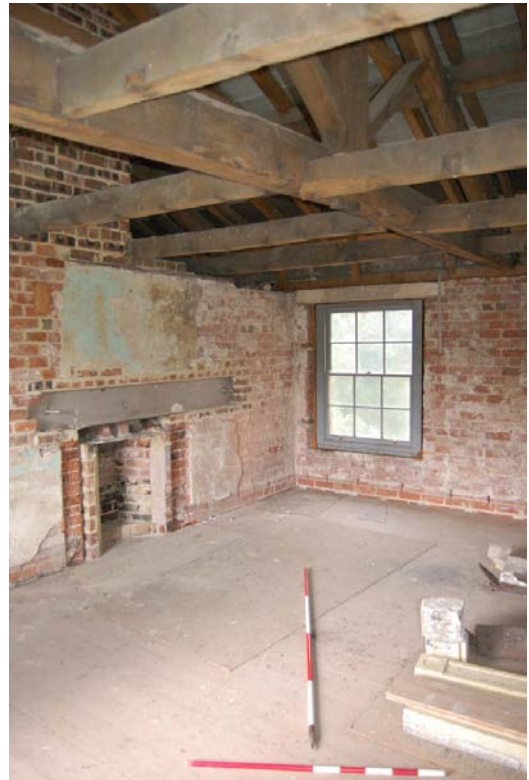
Plate 82: Room [F4] looking north-west.
