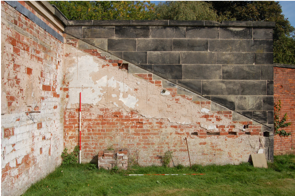
Plate 13: North-east vinery: profile of glasshouse visible in west wall
