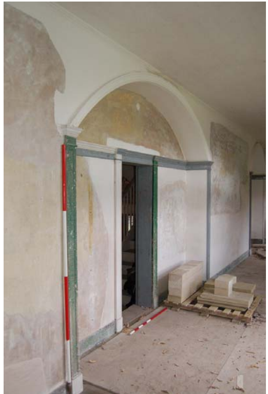
Plate 50: Room G1, doorway to G3.
