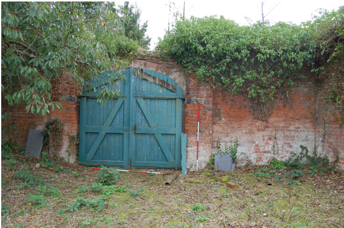
Plate 159: Potato Store, detail of brick-lined ducting with ceramic capping.
