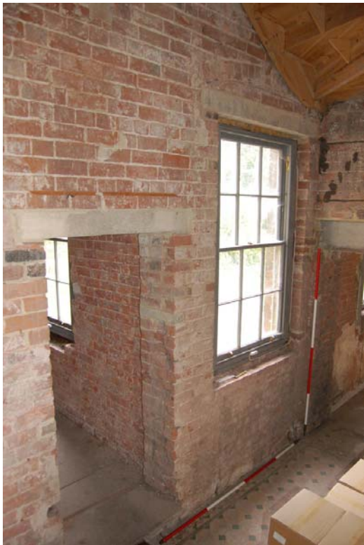
Plate 53: Room G3, looking north-east
