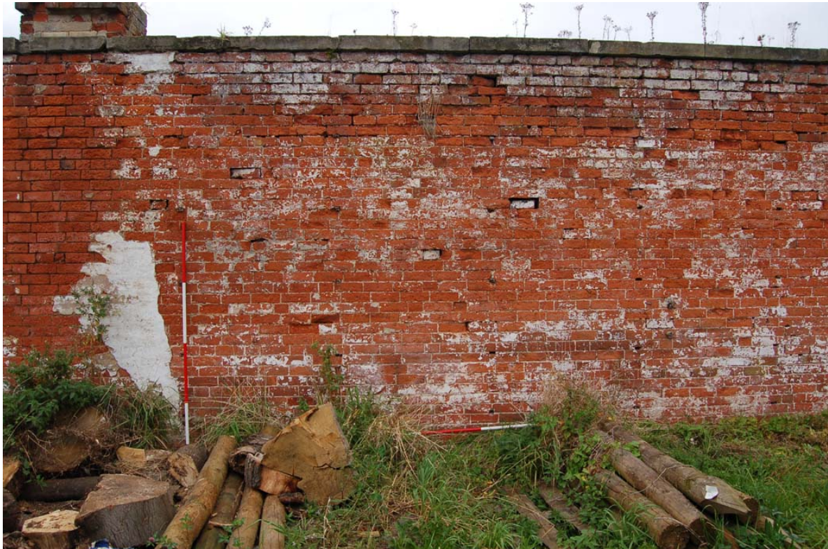
Plate 133: South garden, north wall; representative section of walling.
