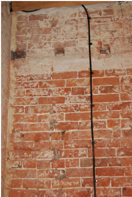
Plate 66: Room G5, former joist sockets.
