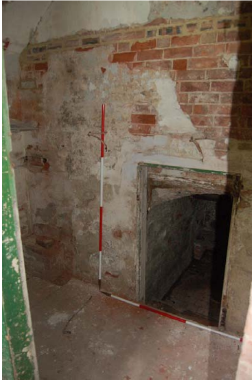
Plate 72: Room G7, looking south-east.
