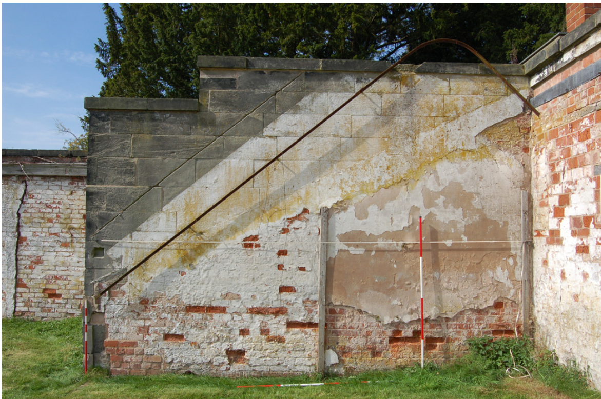
Plate 10: North-west vinery: profiles of successive glasshouses visible in west wall.
