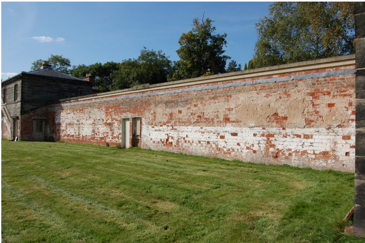
Plate 12: North-east vinery, rear wall general view looking north-west.
