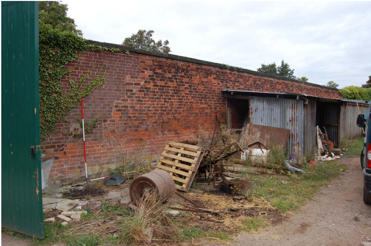
Plate 144: South garden, west wall; oblique view looking north-west.
