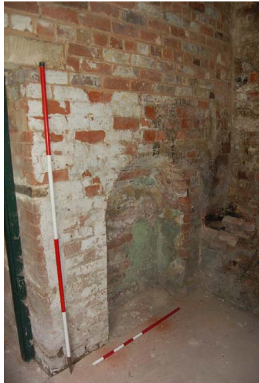
Plate 75: Room G8, east wall recess.
