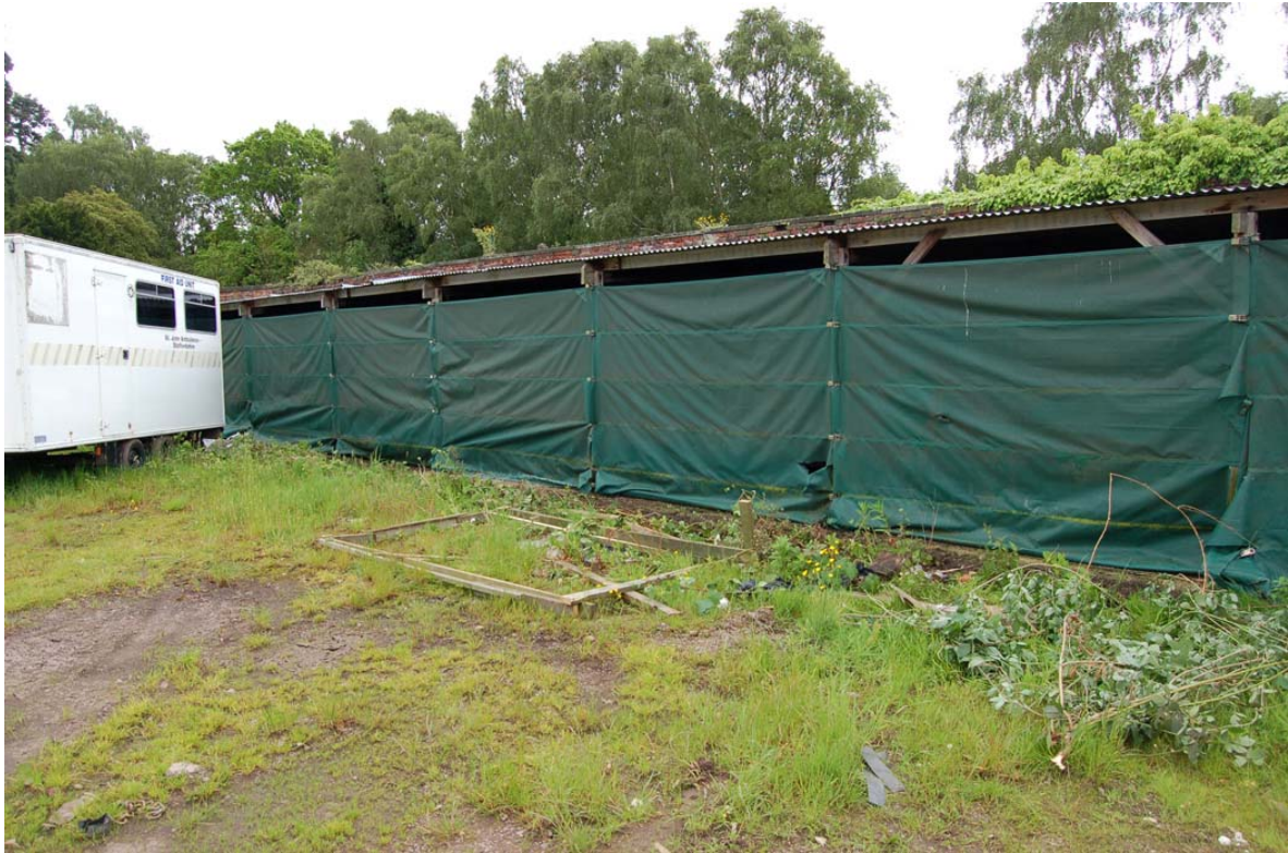
Plate 138: South garden, south wall, east end obscured by storage sheds.
