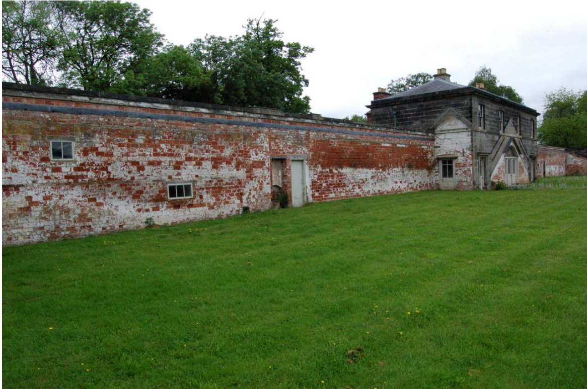
Plate 11: North-west vinery, rear wall general view looking north-east.
