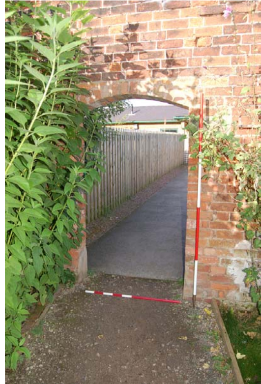
Plate 5: Pedestrian doorway, west wall (ins).
