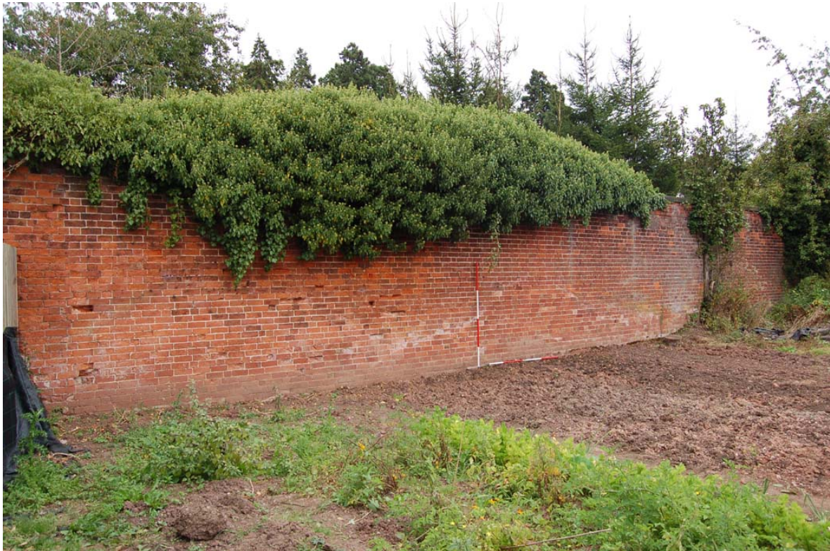
Plate 136: South garden, east wall; north end.
