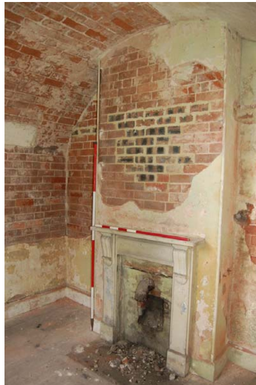
Plate 59: Room G2, south wall.
