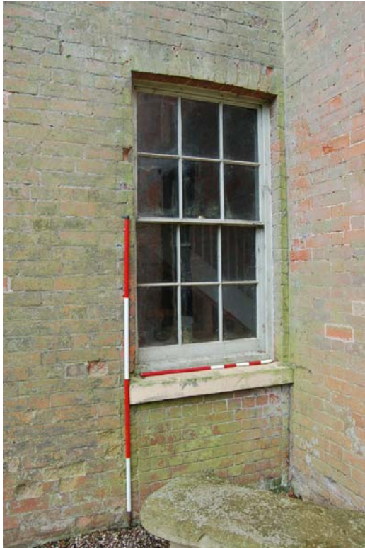
Plate 38: Main block, converted door.
