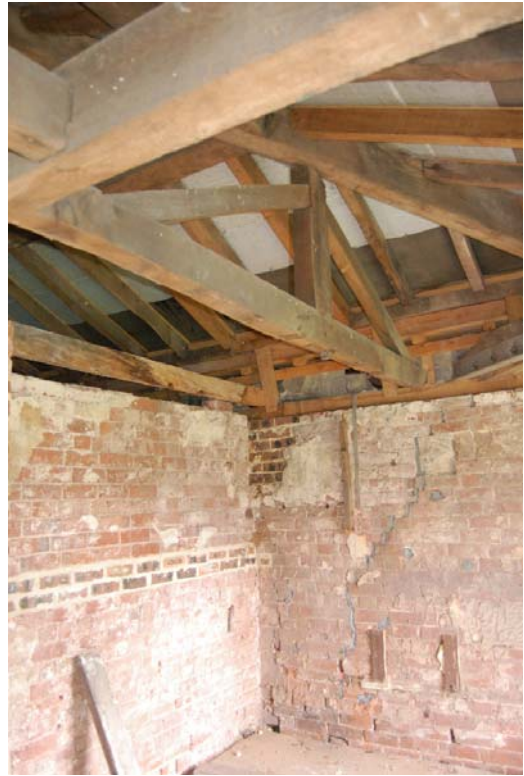
Plate 96: Subsidiary KP truss at Rm. F3/7.
