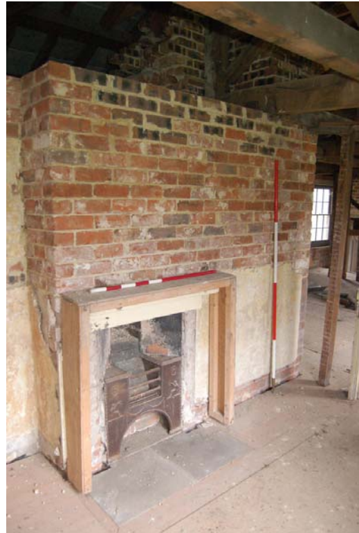
Plate 88: Room F5 looking north-east.
