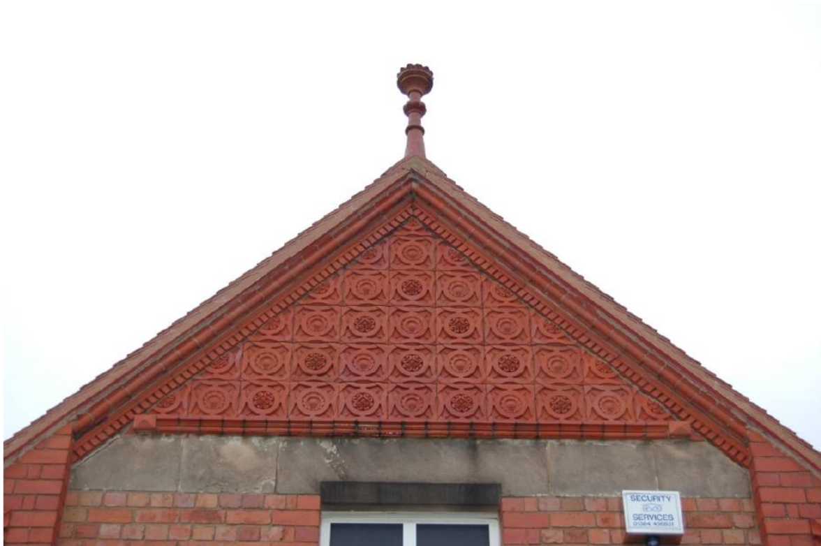
Plate 47: Central gable; terra-cotta apex detail.
