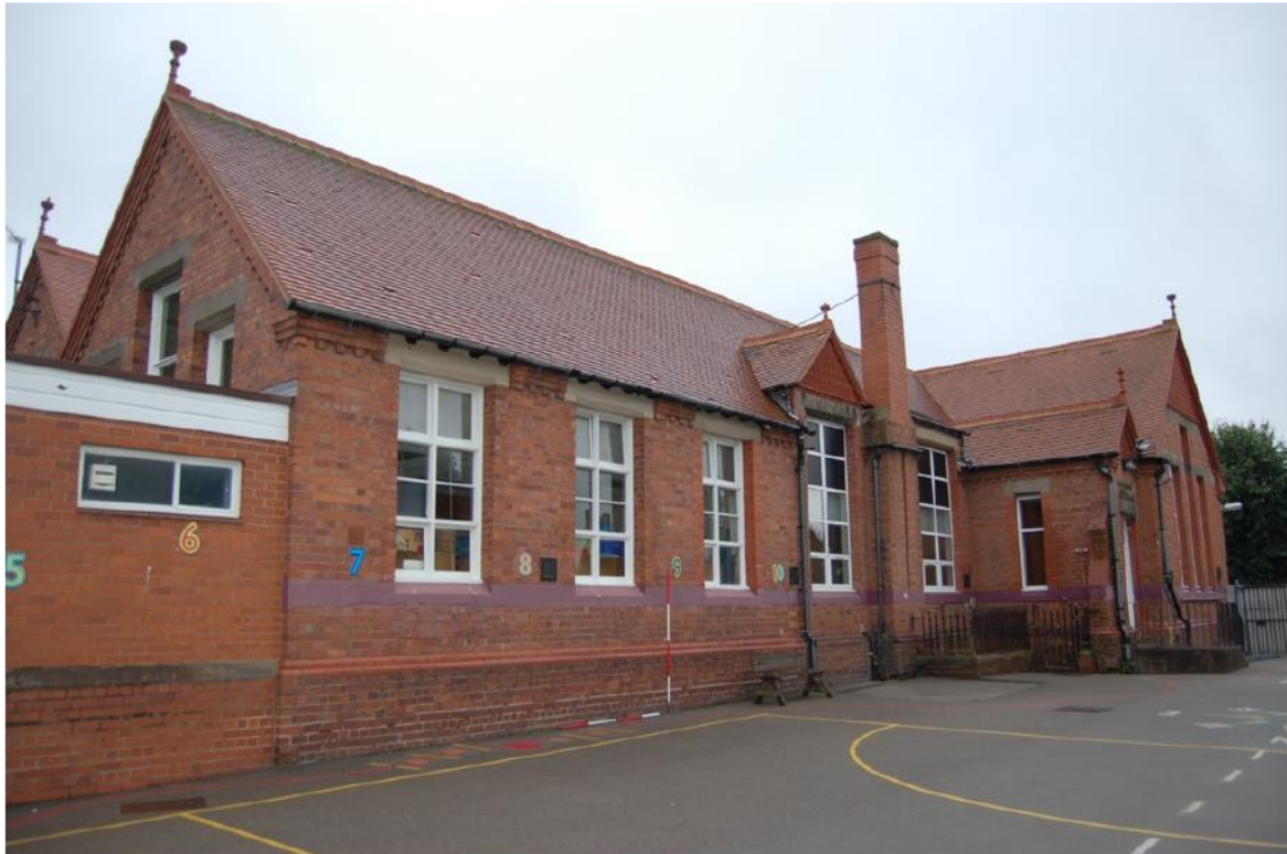
Plate 53: North school buildings, west elevation oblique.
