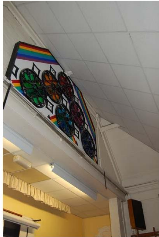
Plate 62: Re-used ceiling vents.
