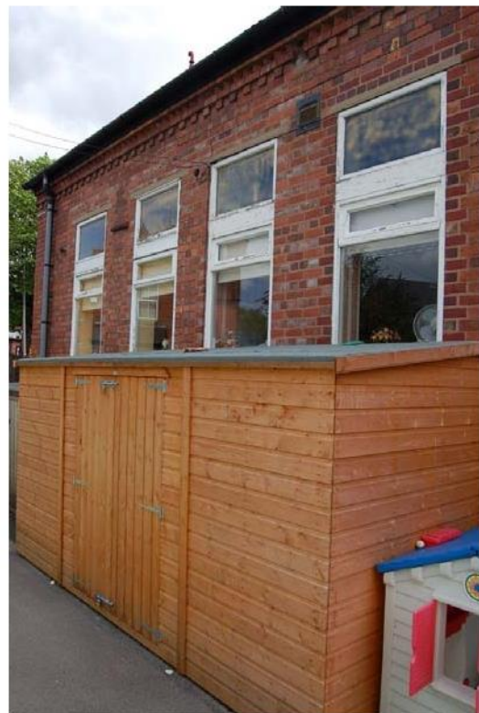
Plate 19: West elev.; inserted windows.
