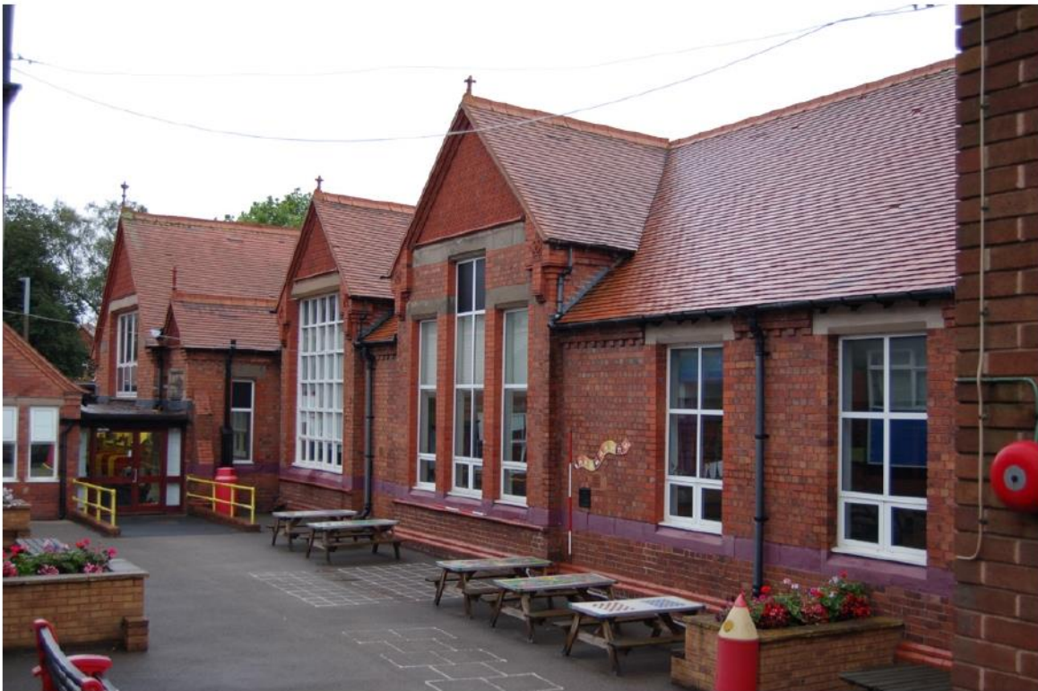
Plate 49: South School, main block east elevation.
