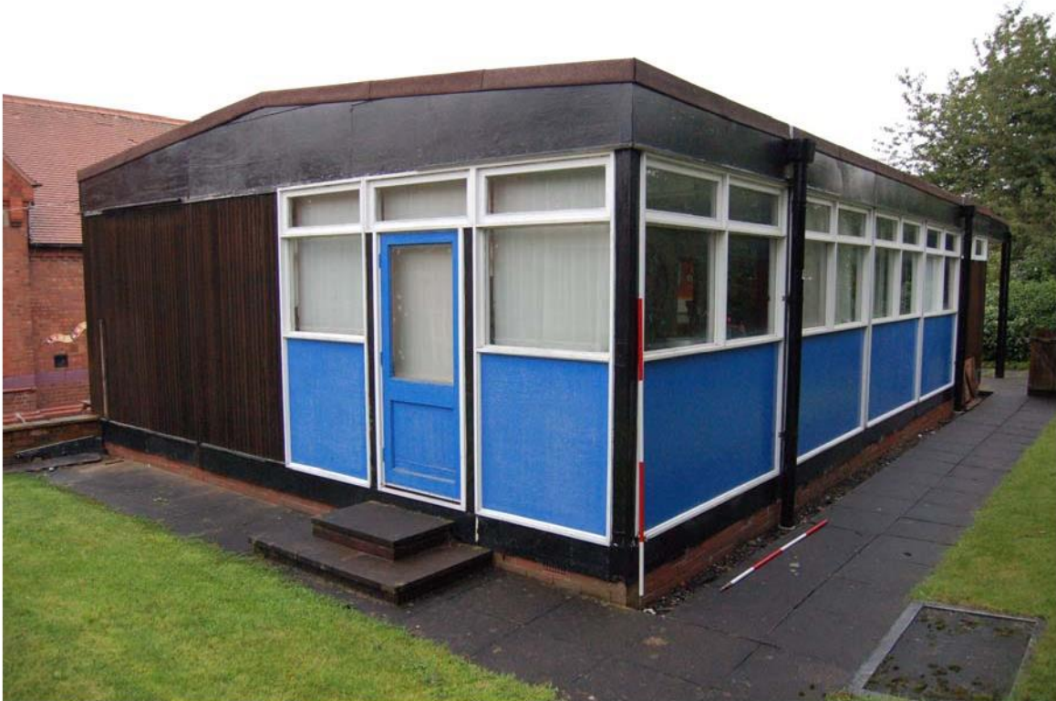
Plate 75: Technology Block (1972); south/east elevation oblique.
