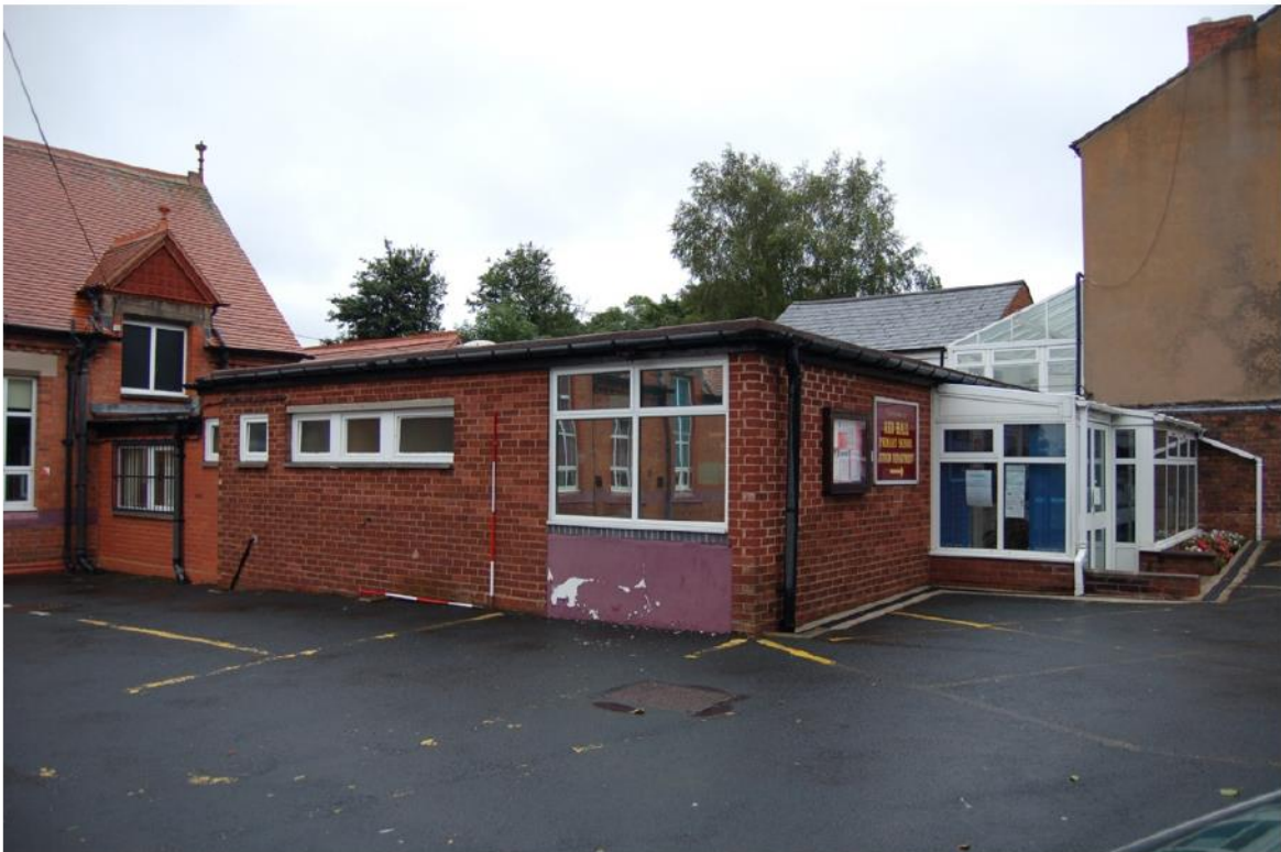
Plate 69: Single-storey entrance block, added 1958 (see also Figure 15b).
