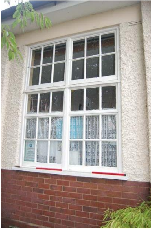
Plate 39: Nursery; window detail.
