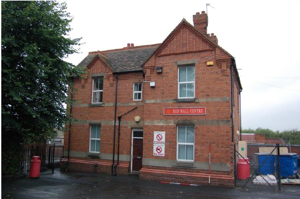
Plate 79: No.11 Zoar Street; east elevation overlooking school yard.
