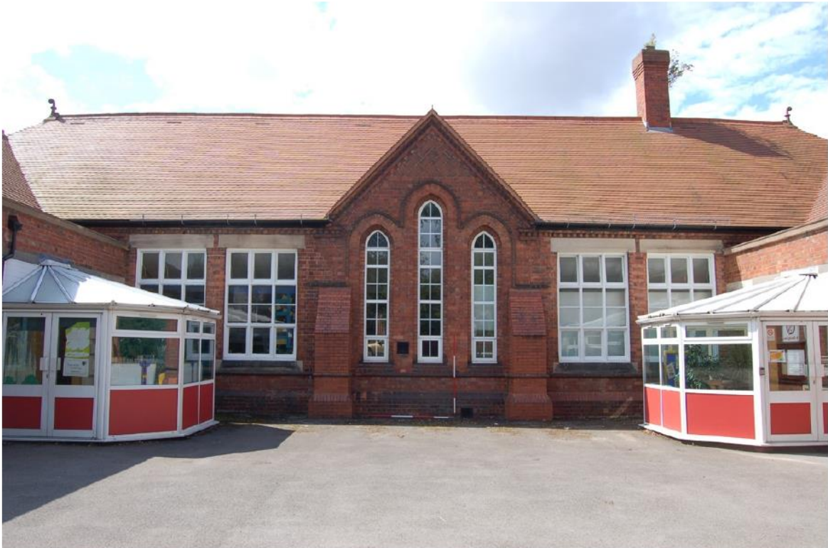
Plate 4: South school building; north (Zoar St.) elevation, central section.
