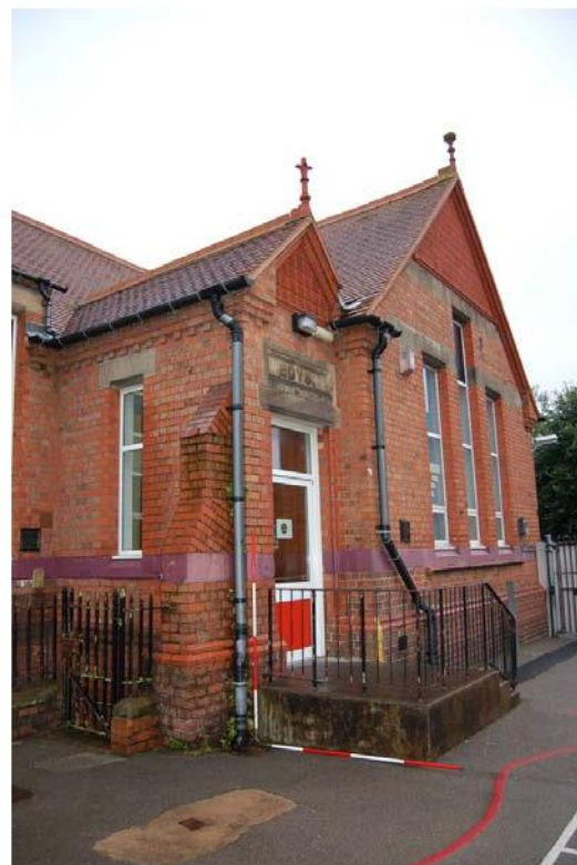
Plate 55: Boys entrance door (west).
