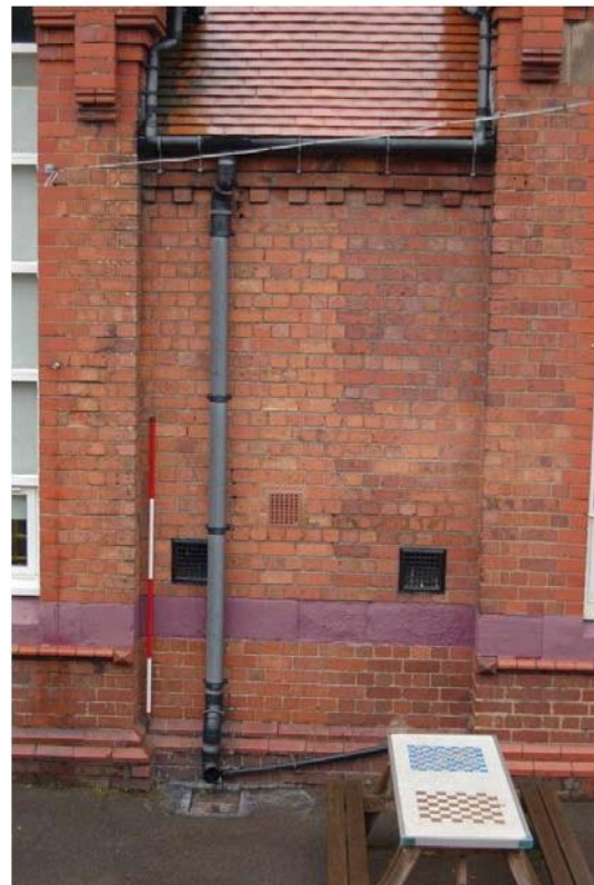
Plate 52: Phase break in brickwork.
