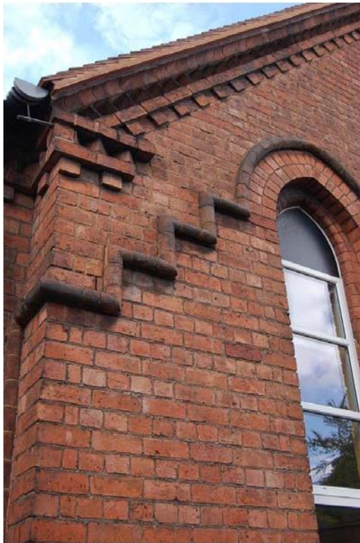
Plate 15: East elevation; stepped string.
