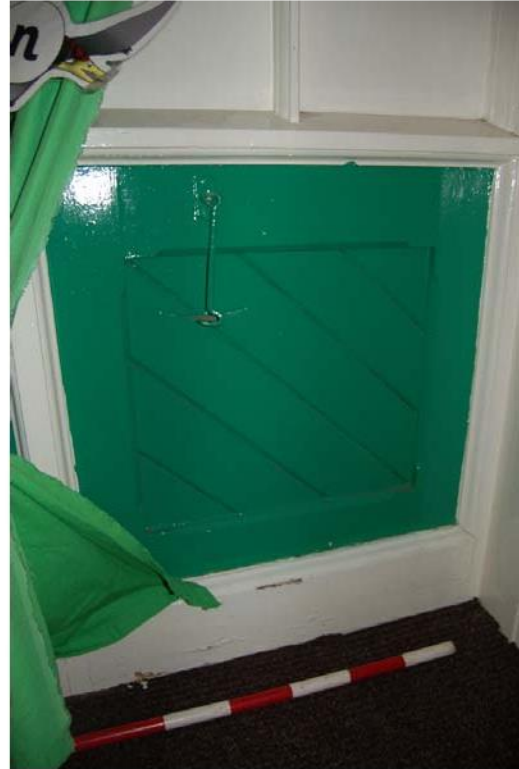
Plate 25: Timber boarding detail.
