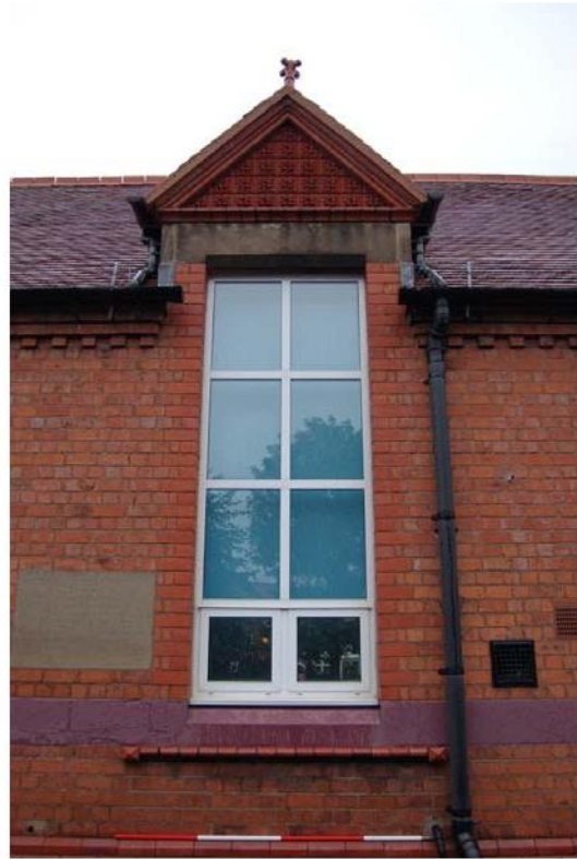
Plate 46: South elevation, window detail.
