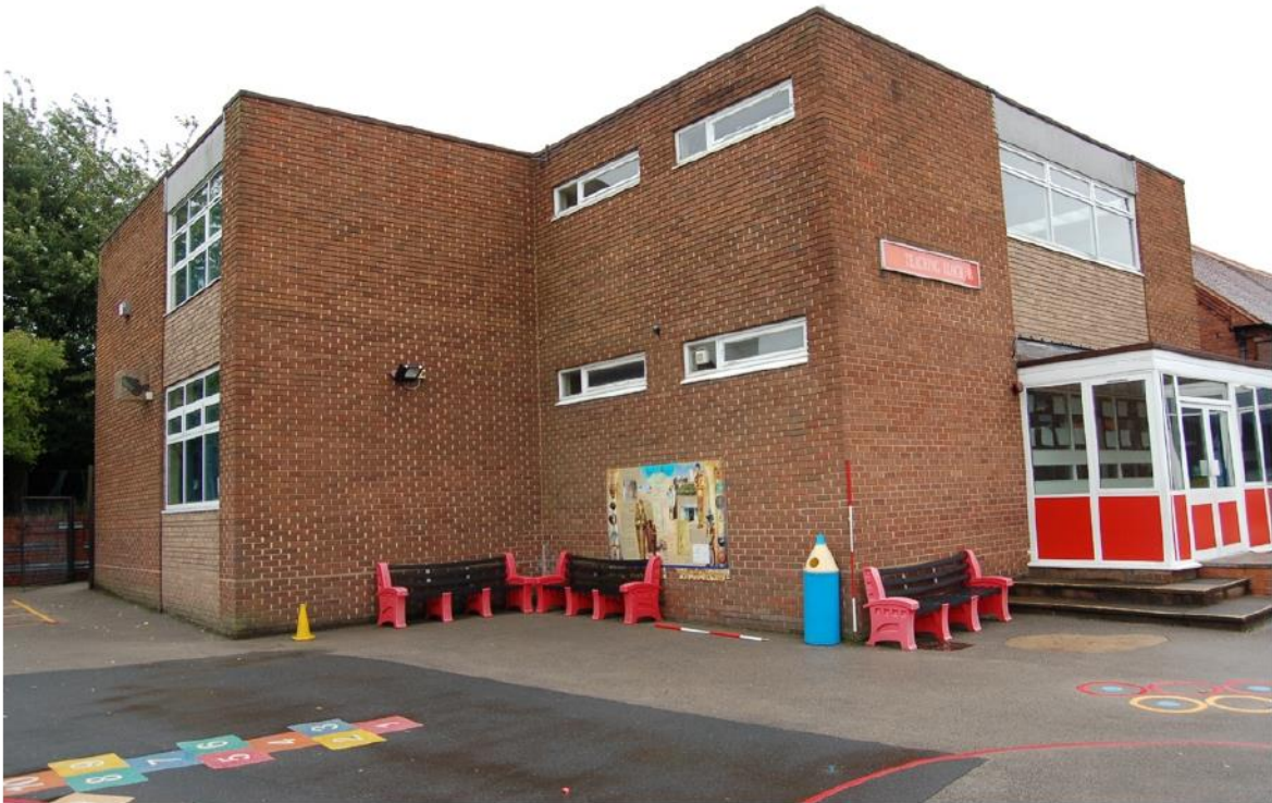
Plate 70: Two-storey entrance block, added 1968.
