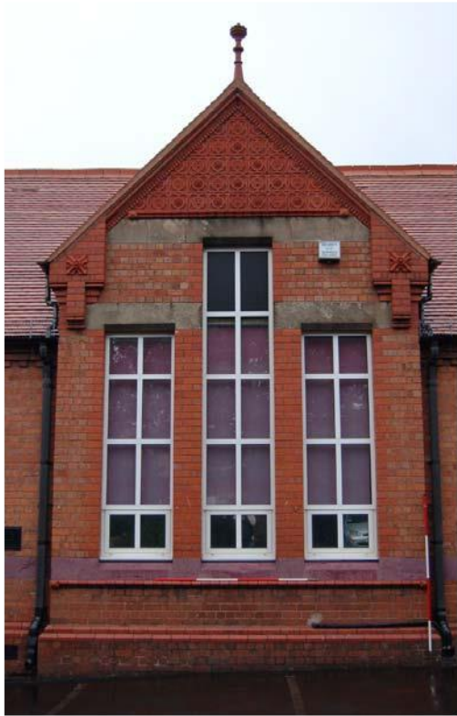
Plate 45: South elevation, central gable.
