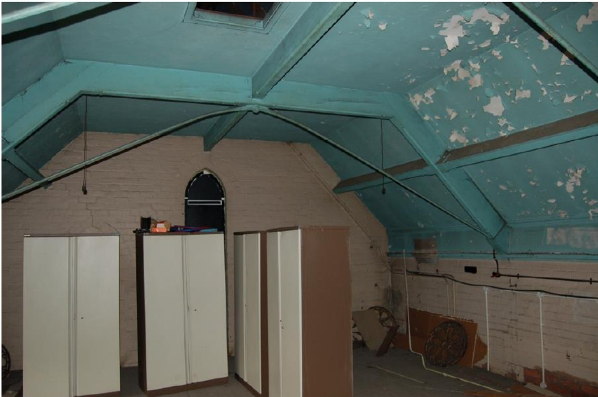
Plate 33: Secondary roof structure over Rms. [03/01].
