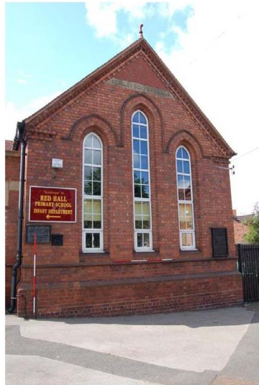
Plate 3: Western projecting gable.
