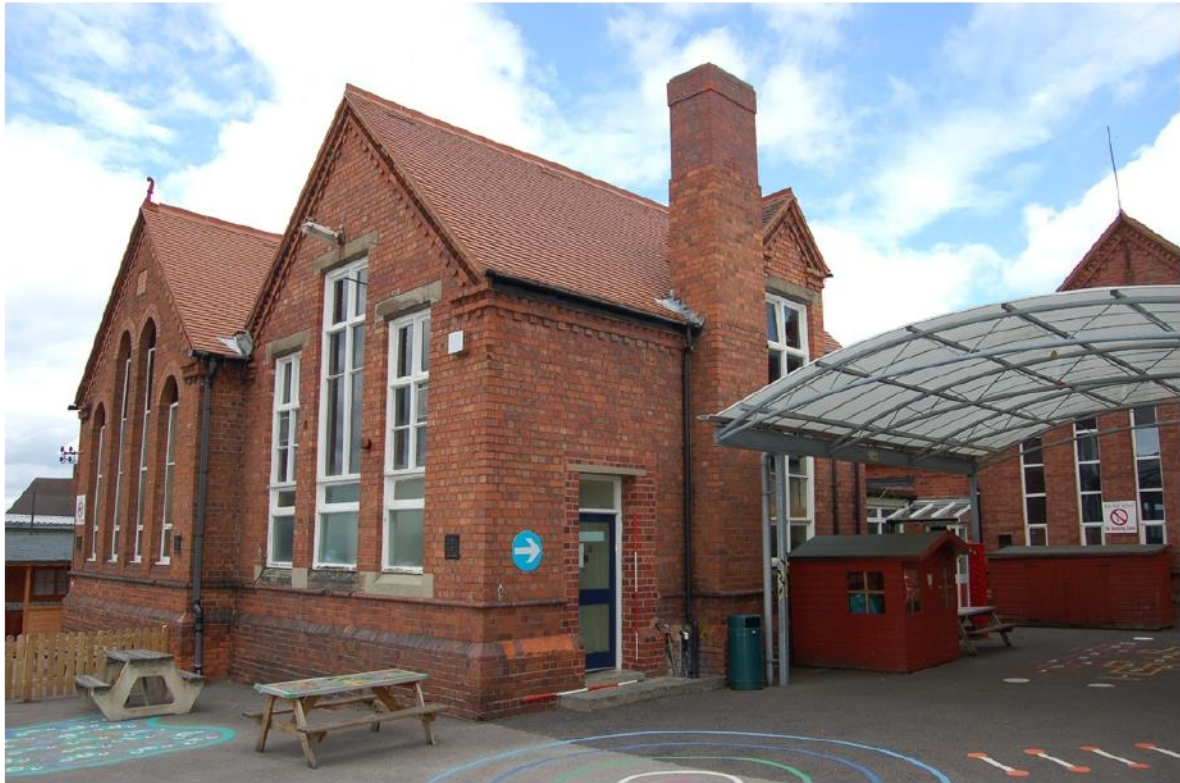
Plate 12: South school building; south elevation (west) oblique view.
