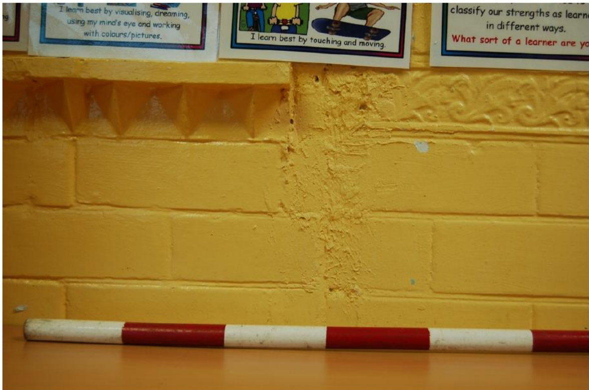
Plate 65: Junction of dado rails at Phase I/II boundary (Rm. [07]).
