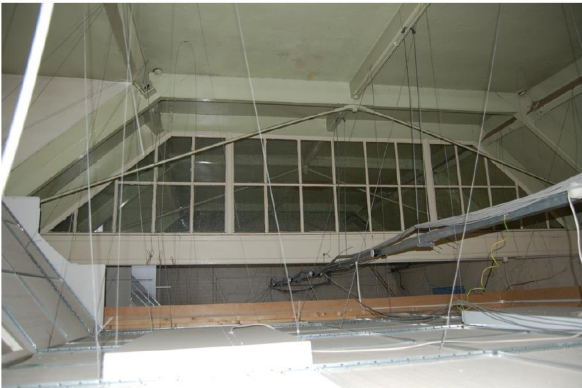
Plate 67: Surviving upper section of glazed partition (1 of 2), above suspended ceiling Rm. [07].
