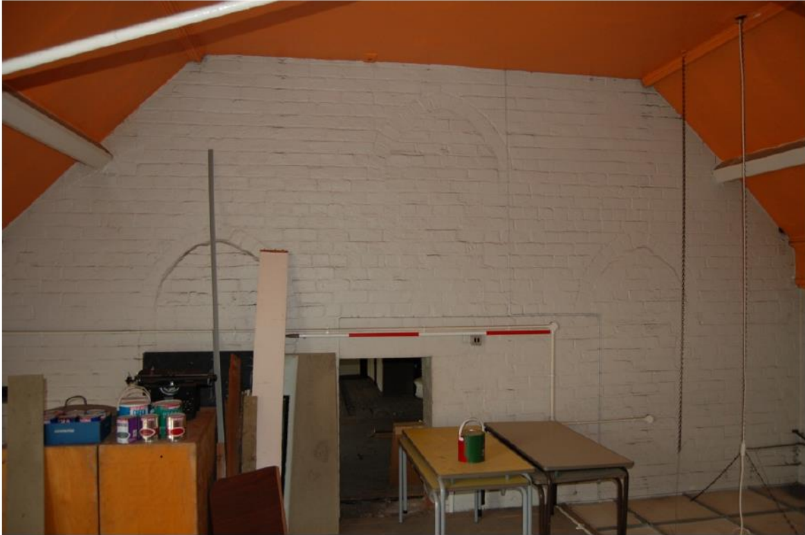
Plate 32: Blocked windows in former front wall (Rms. [04-07]).
