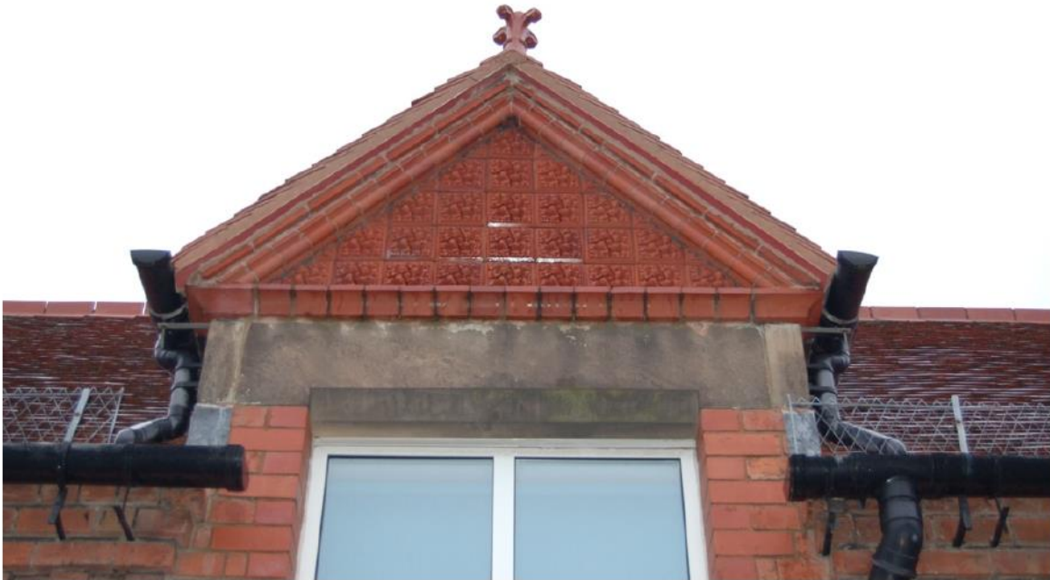
Plate 48: Smaller window gable - terra-cotta apex detail.
