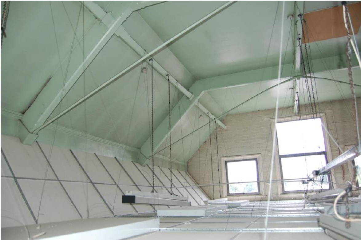
Plate 66: Roof structure above inserted ceiling in Rm. [10].
