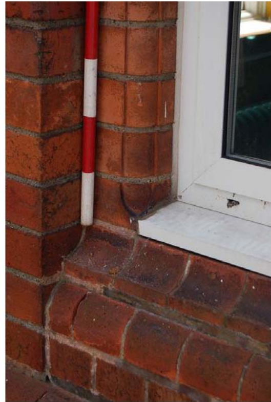
Plate 10: Secondary window jamb detail.
