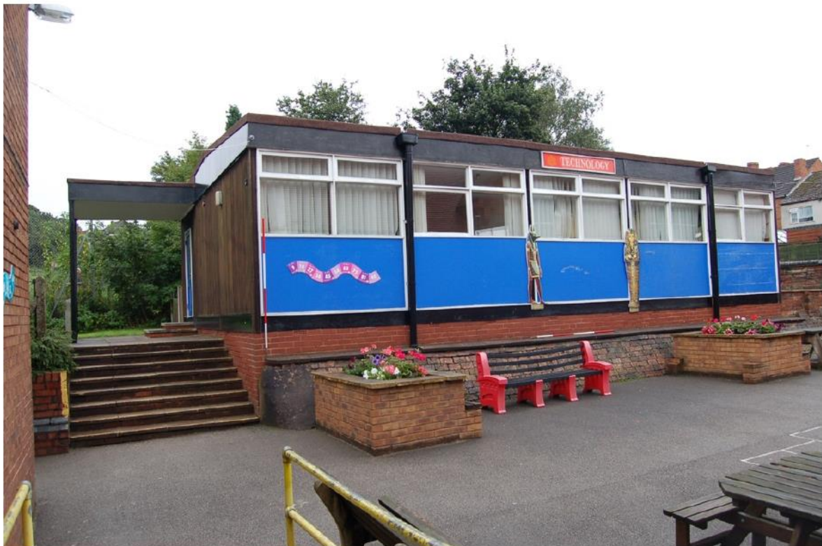
Plate 74: Technology Block (1972); west elevation.
