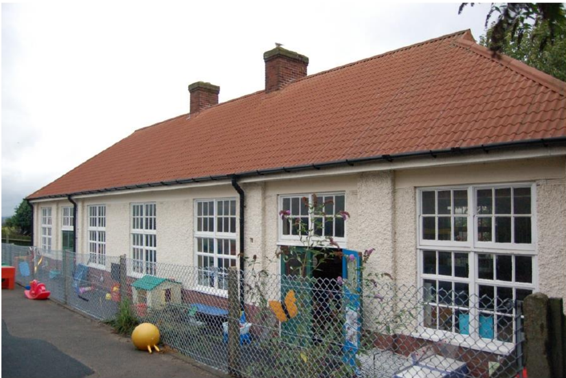
Plate 38: Nursery; east elevation looking south-west.
