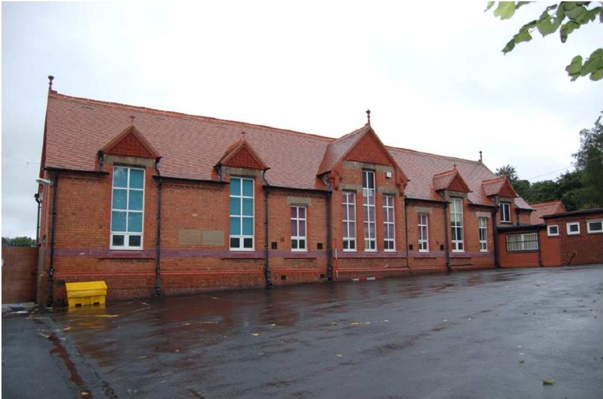
Plate 43: North School Buildings, south (Zoar St) elevation; 1890/1.
