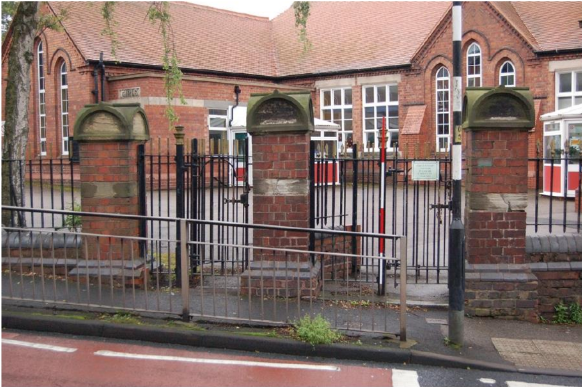
Plate 77: South school; double gate detail.
