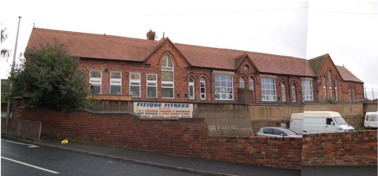
Plate 17: South school building; western elevation viewed from Zoar Street.
