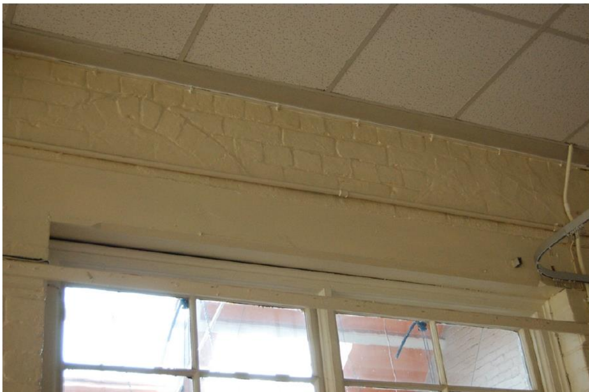
Plate 29: Former lancet window openings Rm. [23].
