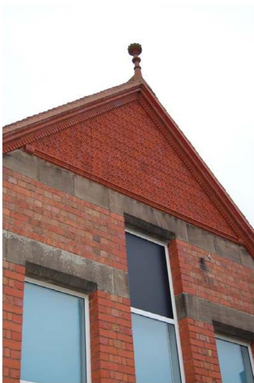
Plate 54: Main west gable; apex detail.
