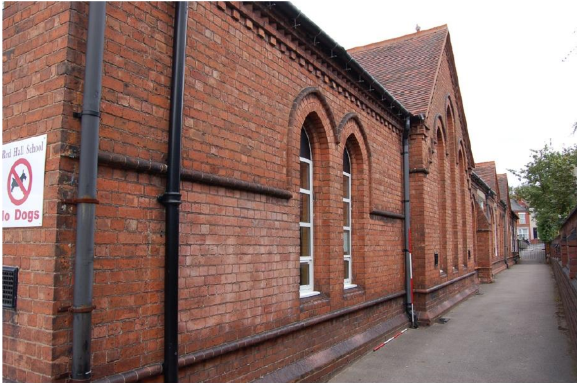
Plate 14: South school building; eastern elevation oblique view.
