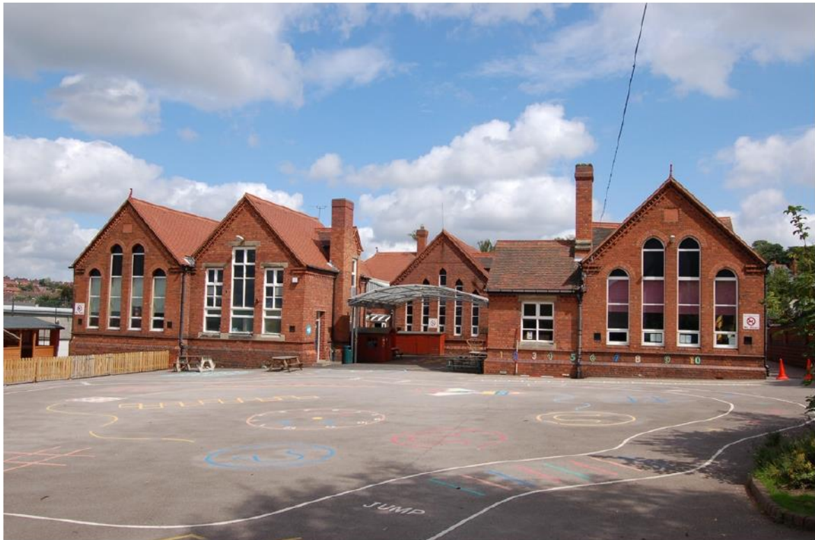
Plate 11: South school building; south elevation - 1880 with later additions.
