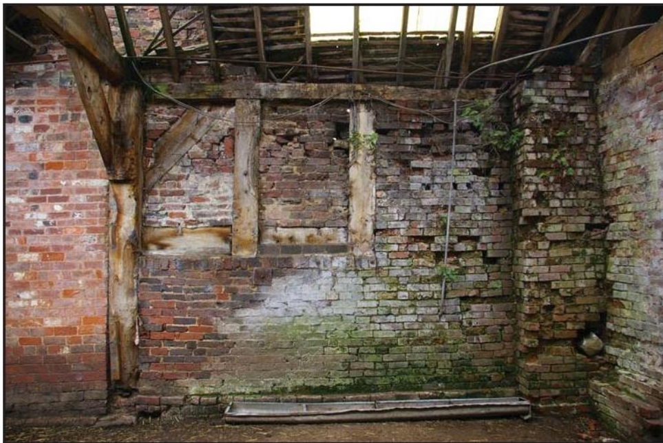
Plate 8: Timber wall framing inside the barn from the southwest
