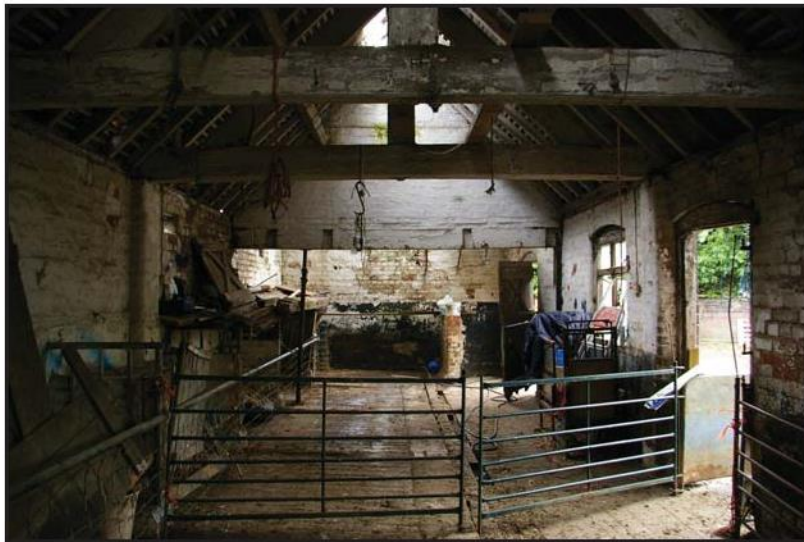
Plate 11: Stable wing interior from the southwest
