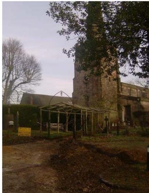
Excavation for the footpath to the south of the church
