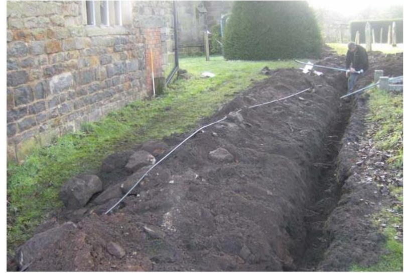
Sandstone block demolition rubble to the north of 1026
