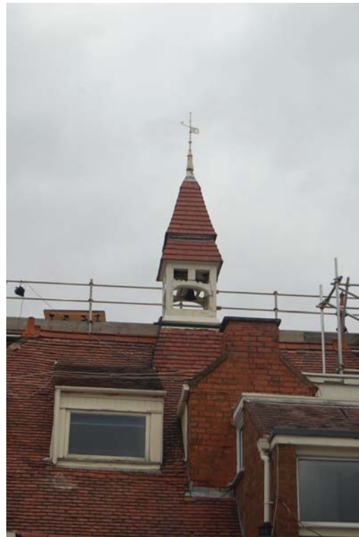
Photo 22: Original pavilion roof structure bell tower from southeast.
