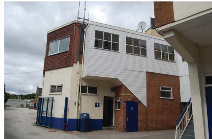
Photo 19: Centre Pavilion (road side) from east.
