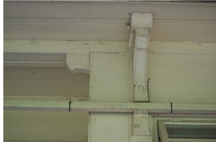
Photo 38: Partially embedded original stanchion and bracket (west) from north.
