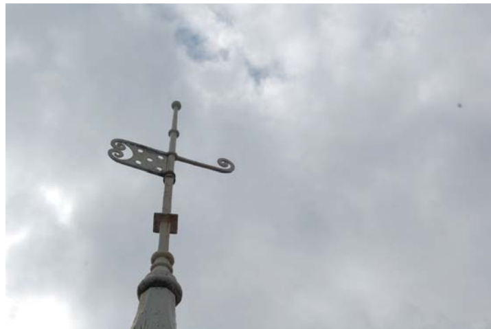
Photo 28: Original pavilion roof structure bell tower weather vane from north.
