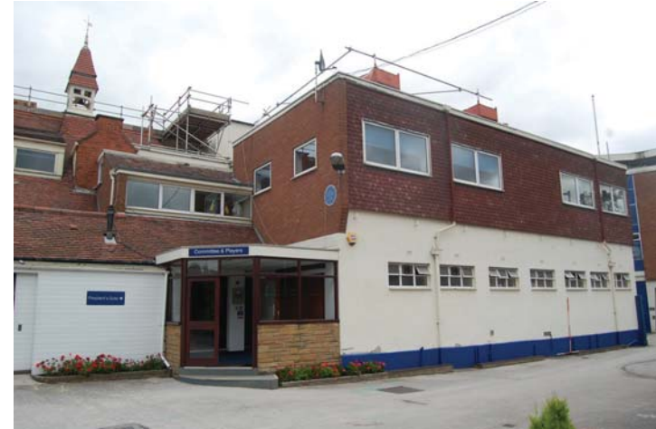
Photo 18: Centre Pavilion (east, road side) from southwest.
