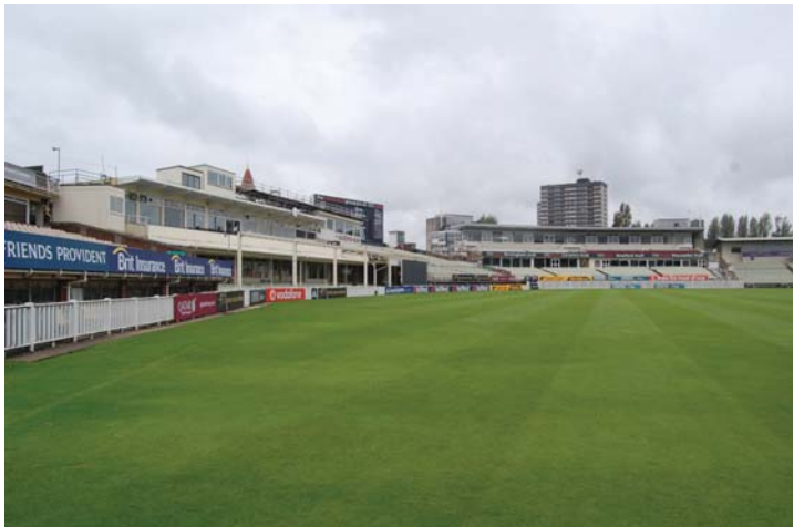
Photo 3: Centre Pavilion (field side) from northeast.
