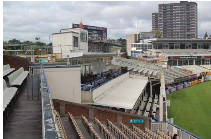
Photo 12: Centre Pavilion (field side) upper stand from east.
