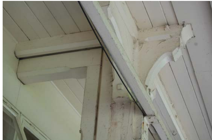
Photo 34: Sole surviving complete original stanchion and bracket from east.
