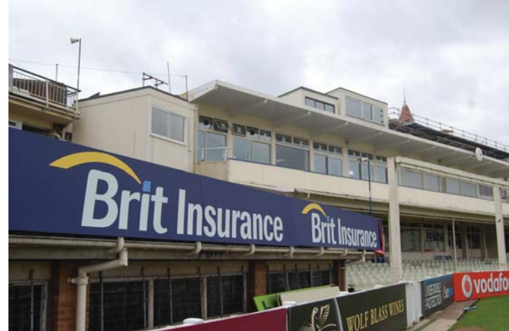
Photo 8: Centre Pavilion (field side) from northeast.
