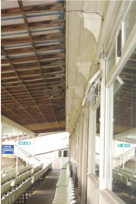
Photo 29: Original upright/stanchion brackets from west.
