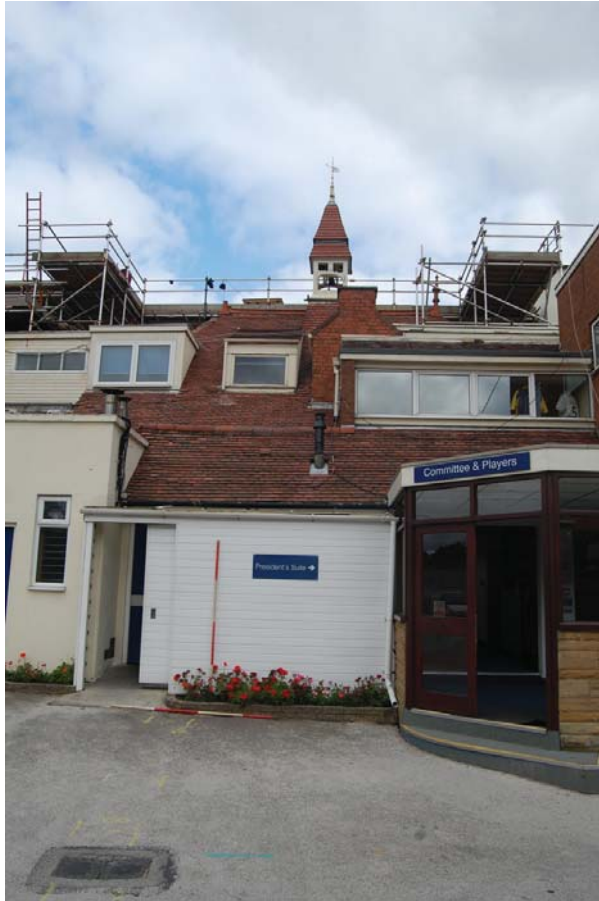
Photo 17: Centre Pavilion (centre east, road side) from south.
