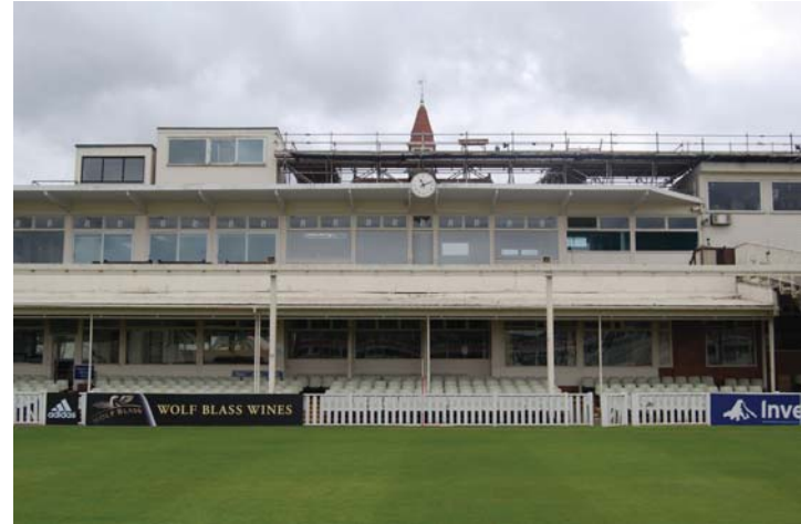
Photo 6: Centre Pavilion (centre, field side) from north.
