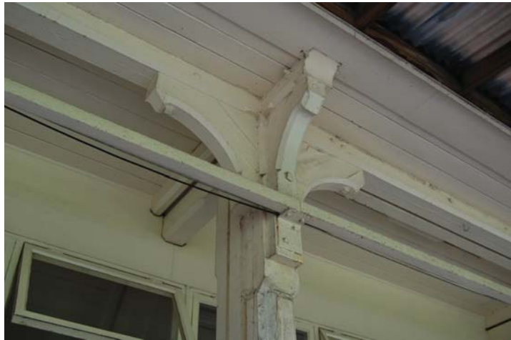
Photo 33: Sole surviving complete original stanchion and bracket from northeast.
