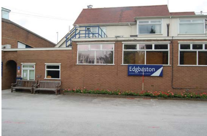
Photo 15: Centre Pavilion (west, road side) from south.
