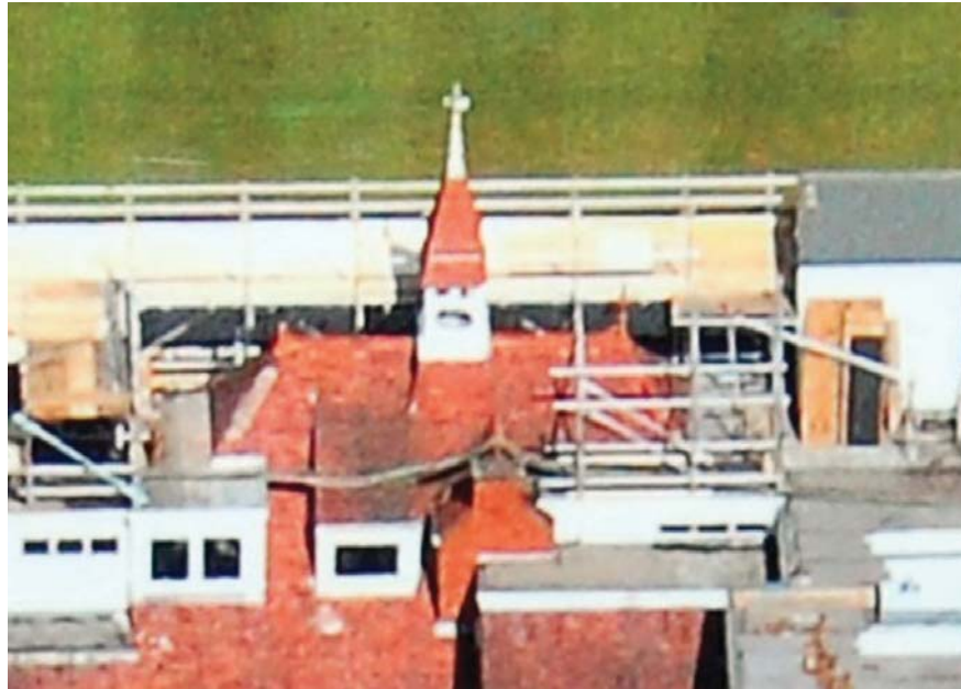
Photo 20: Original pavilion roof structure oblique aerial from south.
