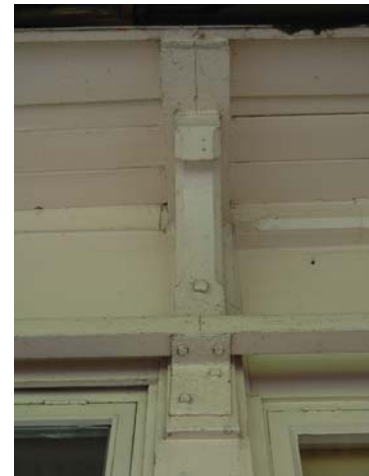
Photo 40: Embedded original stanchion and bracket from north.
