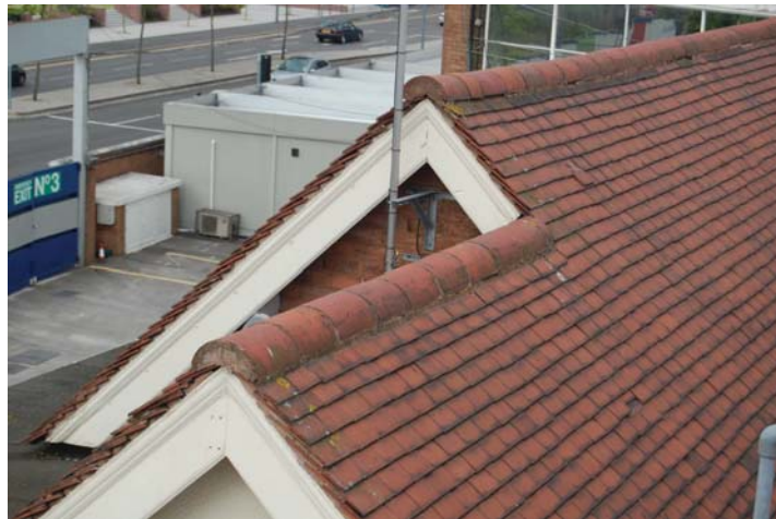
Photo 43: Gabled structure roof from northeast.
