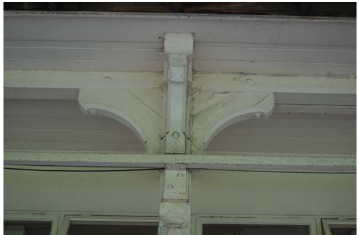
Photo 32: Sole surviving complete original stanchion and bracket from north.
