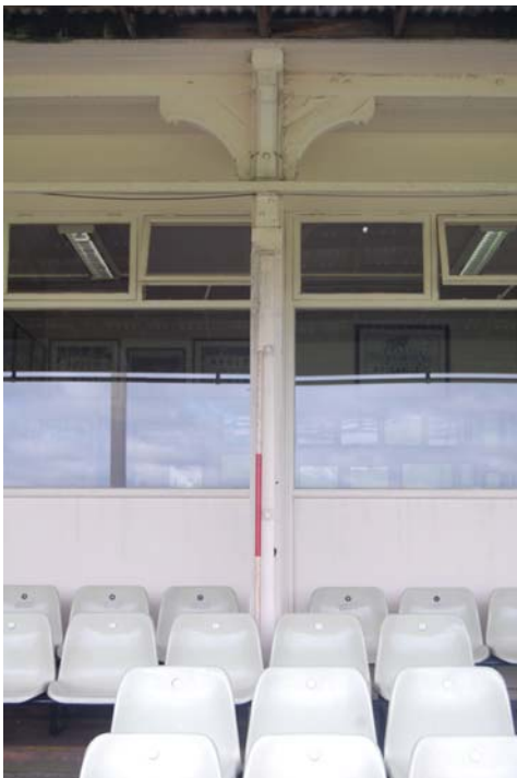
Photo 31: Sole surviving complete original stanchion and bracket from north.
