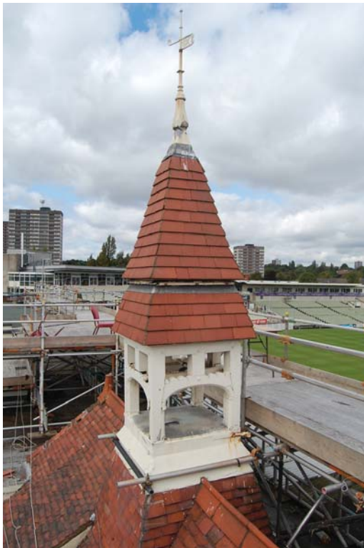
Photo 21: Original pavilion roof structure from south.
