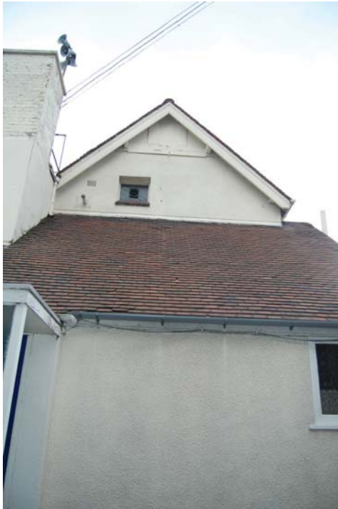
Photo 44: Gabled structure from west.
