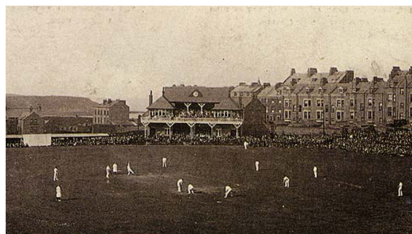
Plate 12: New Marine Road, Scarborough, built 1897
