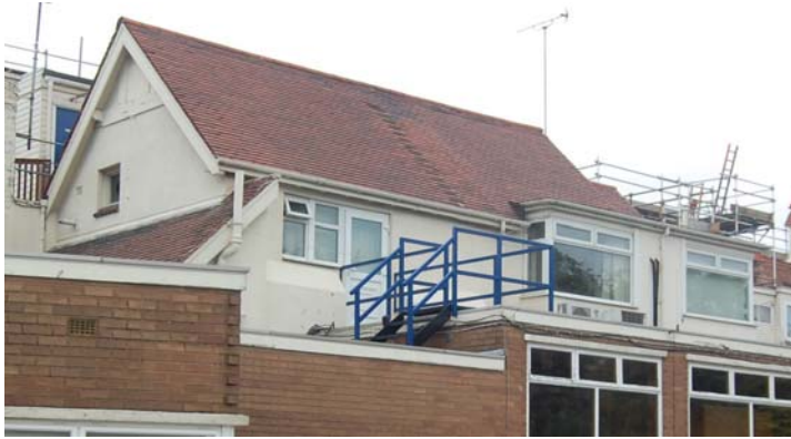
Photo 41: Gabled structure from southwest.
