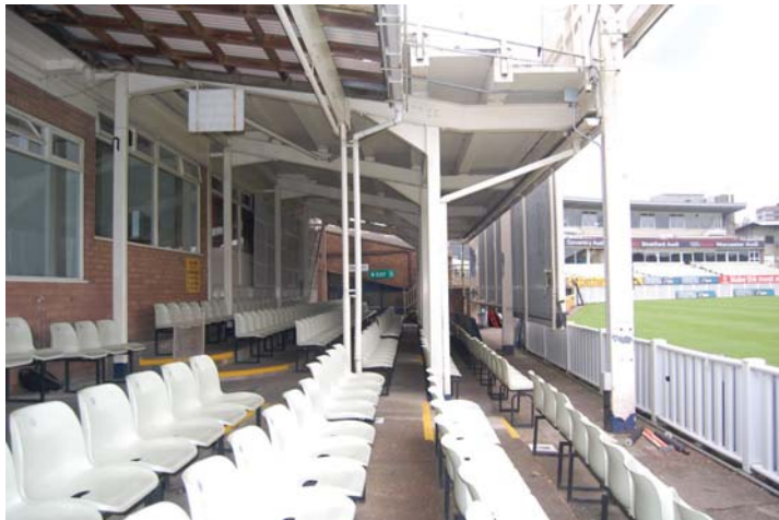
Photo 11: Centre Pavilion (field side) lower stand from east.
