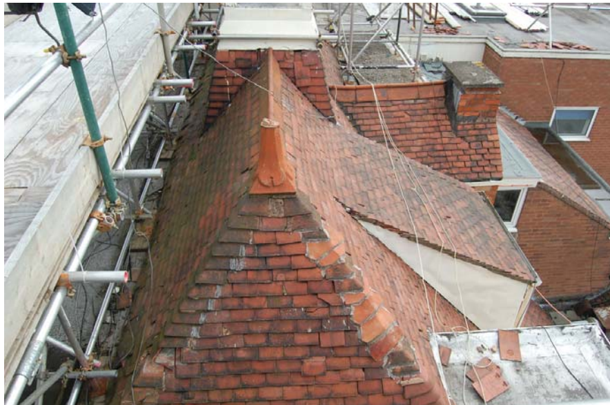
Photo 25: Original pavilion roof structure from west.
