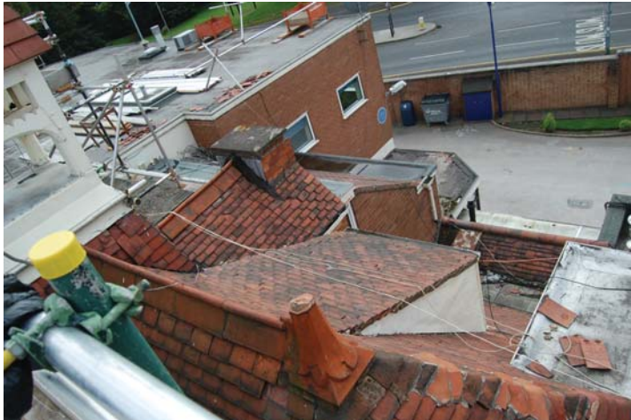
Photo 26: Original pavilion roof structure from northwest.
