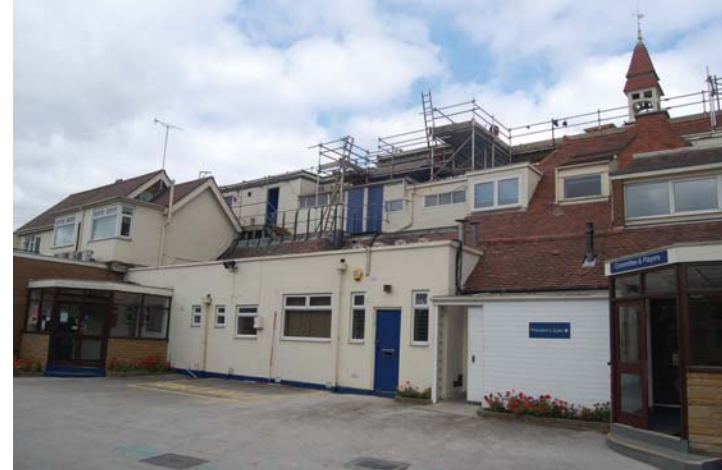
Photo 16: Centre Pavilion (centre west, road side) from southeast.
