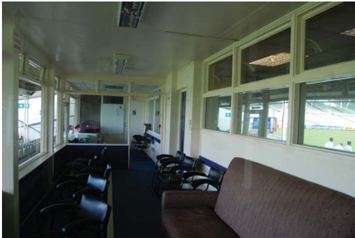
Photo 56: Players' Viewing Rooms from west (interior ground floor).
