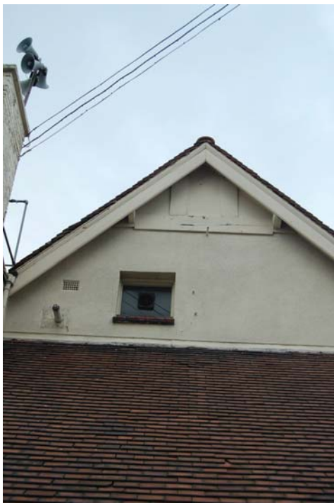
Photo 46: Gabled structure detail from west.
