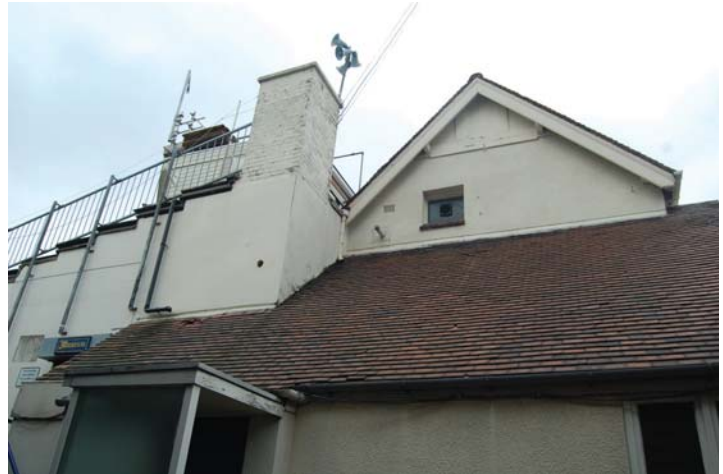
Photo 45: Gabled structure from southwest.
