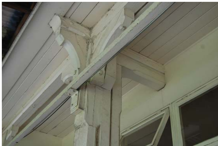
Photo 35: Sole surviving complete original stanchion and bracket from northwest.
