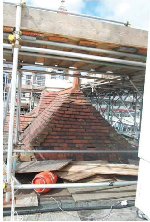
Photo 24: Original pavilion roof structure from east.
