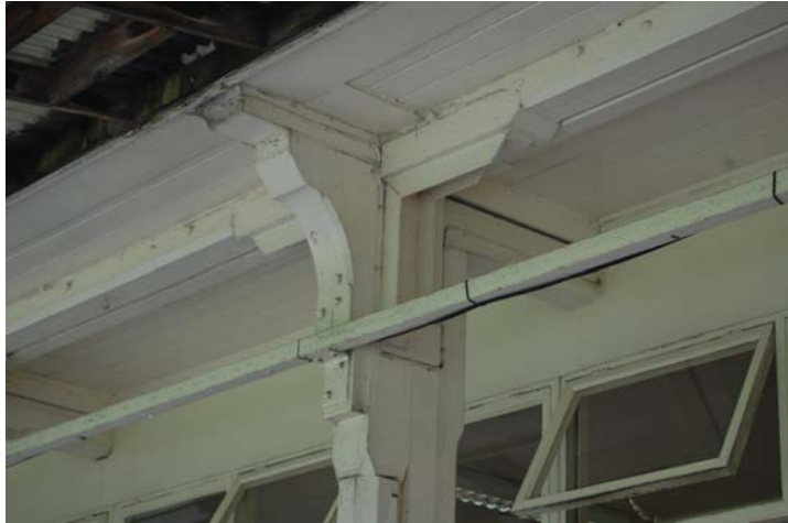
Photo 37: Partially surviving original stanchion and bracket from northwest.
