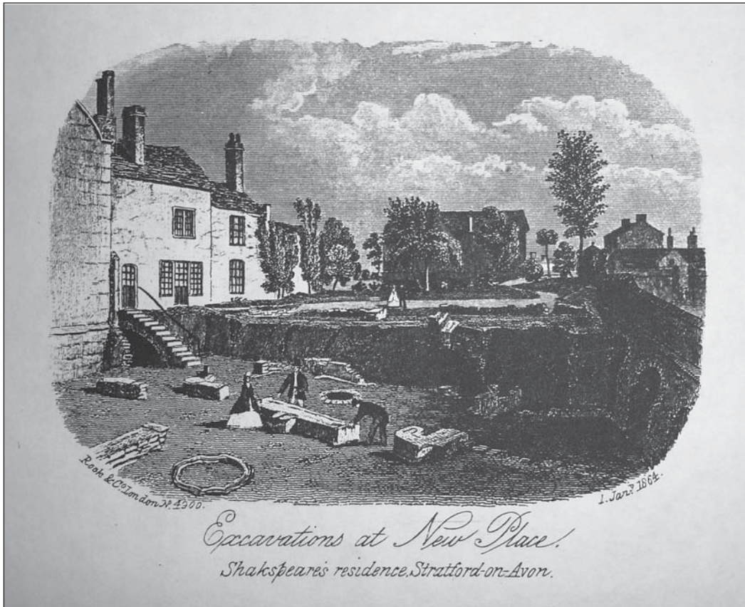
Plate 11: Excavations at New Place Shakespeare's Residence in Stratford-on-Avon, Rook and Co. 1864
