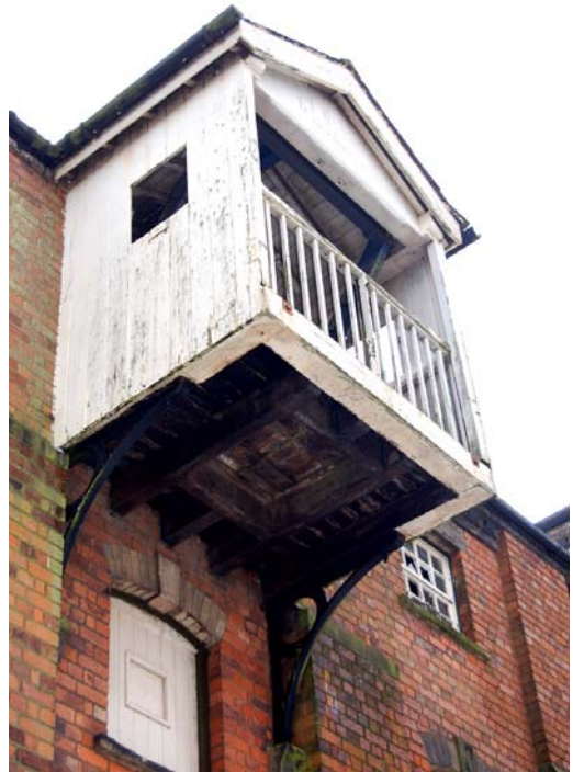
Plate 9: Working floors; 3F hoist canopy.
