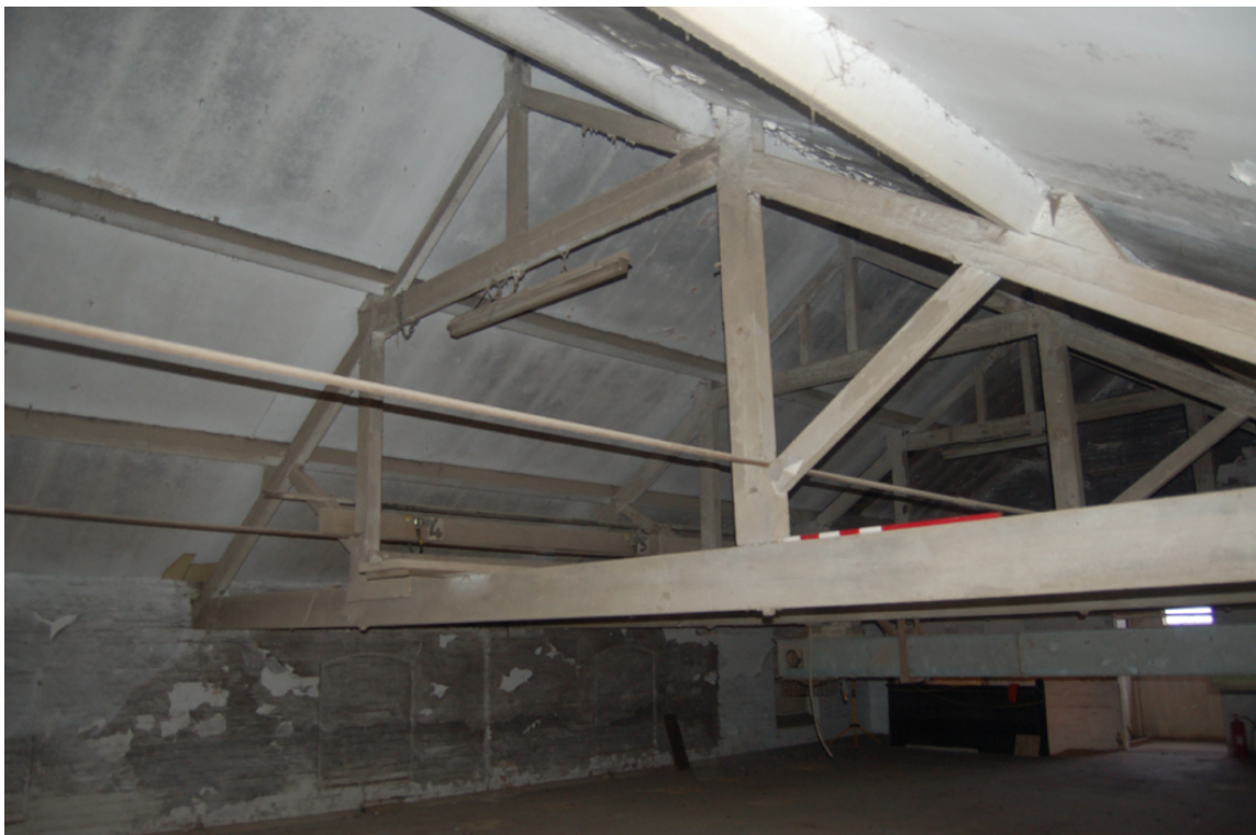
Plate 20: Barley intake range, [4F01]; detail of queen strut roof truss.
