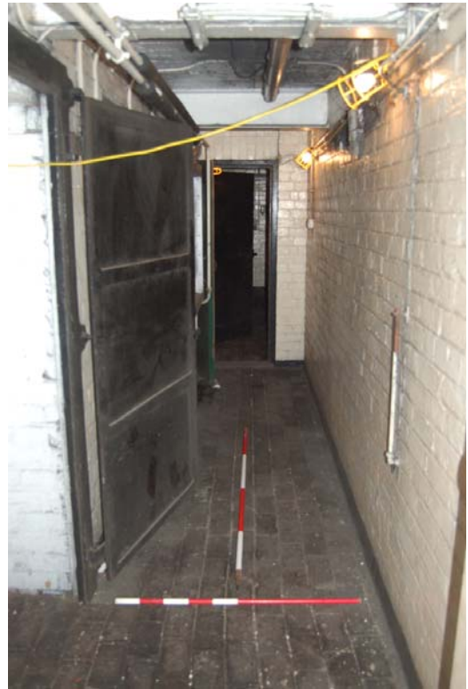
Plate 49: Kiln range; [GF04] access corridor.
