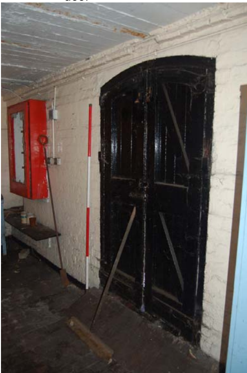
Plate 54: Kiln range, [GF10] (S); door to exterior.
