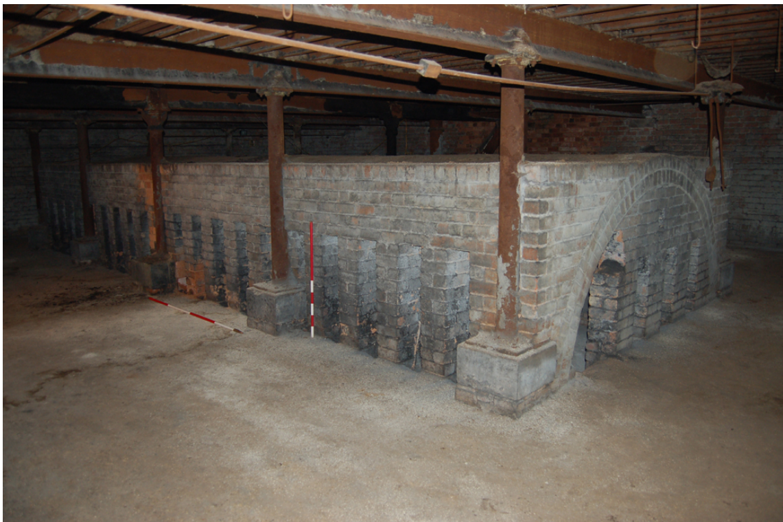
Plate 61: Heat chamber [2F02]; detail of disperser looking north-east.
