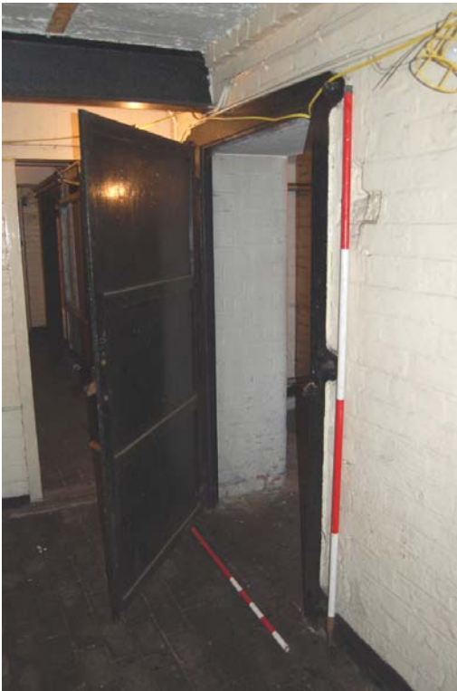
Plate 52: Kiln range, [GF04]; plate metal door
