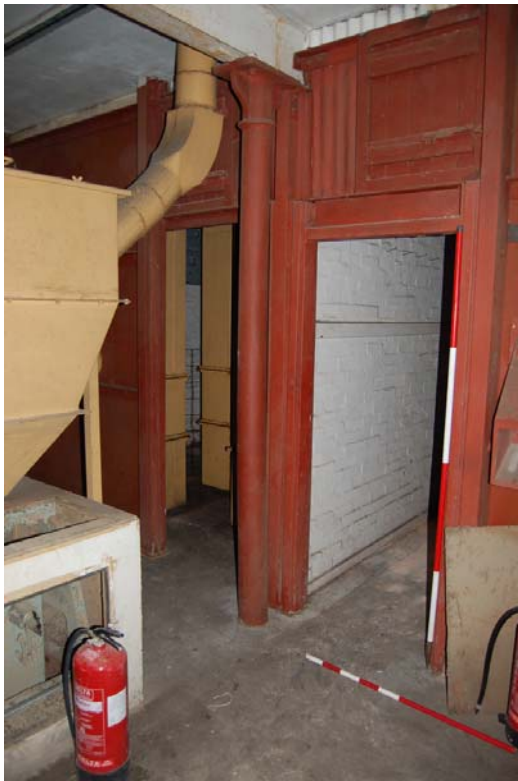
Plate 78: Out-loading bays, [2F03] timber partition.
