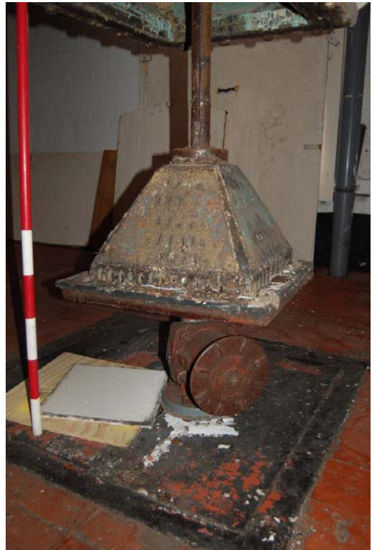
Plate 40: Hopper bottom; detail of grain outlet mechanism.
