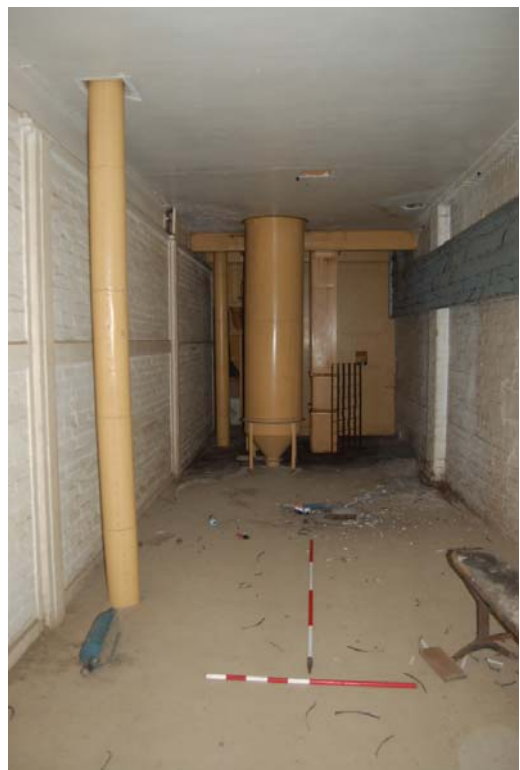
Plate 77: Out-loading bays, [2F05].
