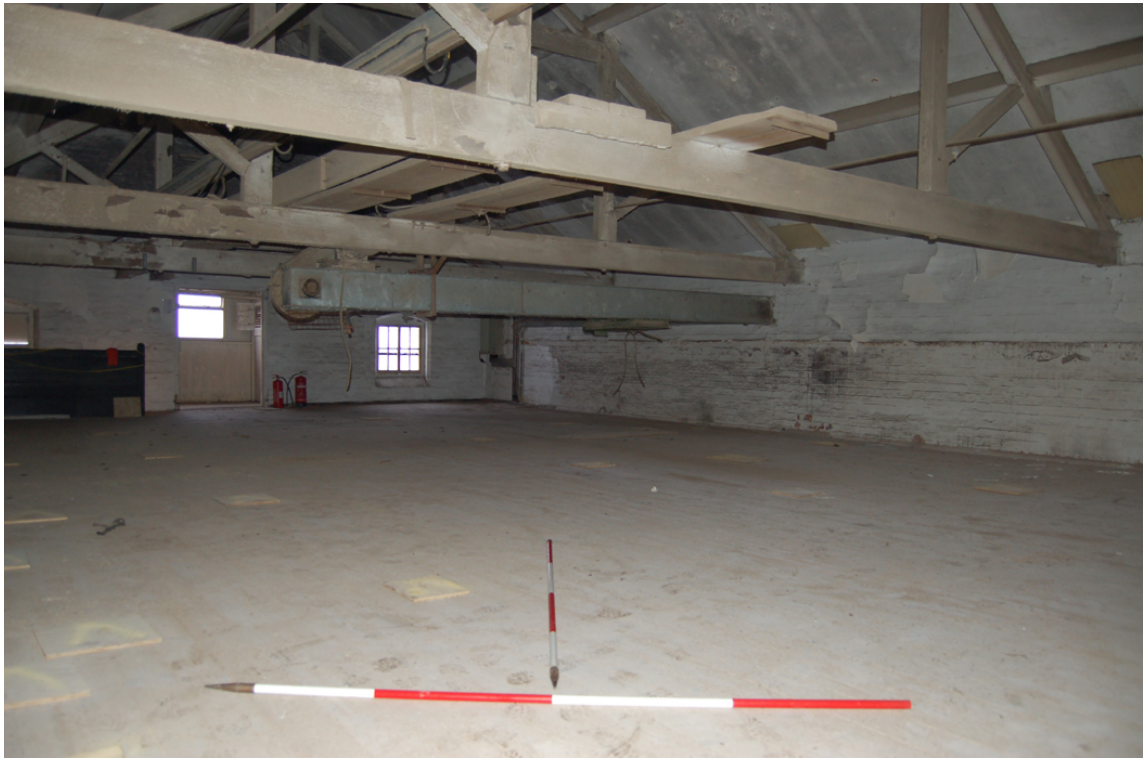
Plate 19: Barley intake range, [4F01]; general view looking north-east.
