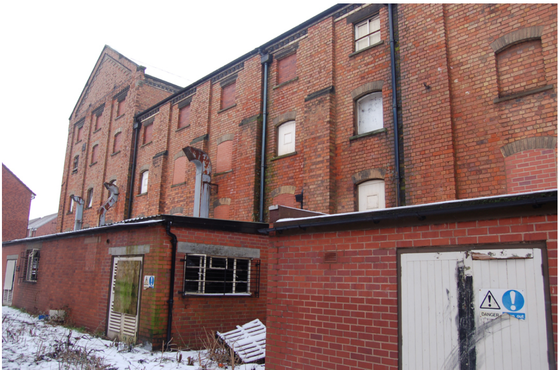
Plate 10: Working floors (centre); south elevation.
