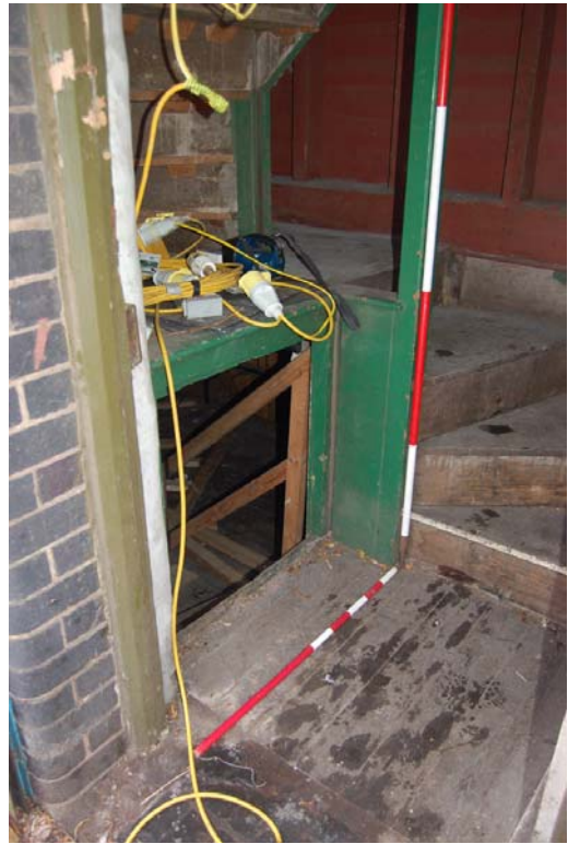
Plate 82: Access to out-loading bays semi basement [B01].
