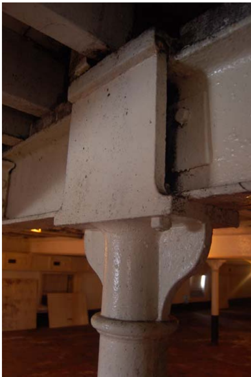
Plate 41: Barley intake range, [2F01]; detail of column head.
