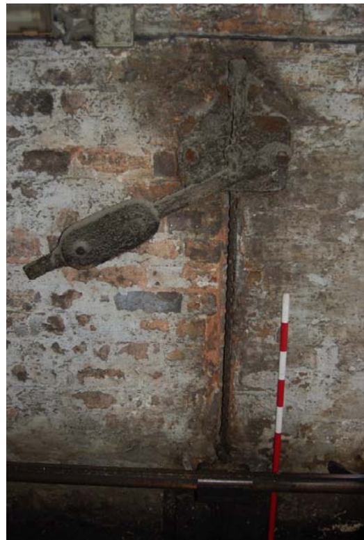
Plate 71: Drive shaft support.
