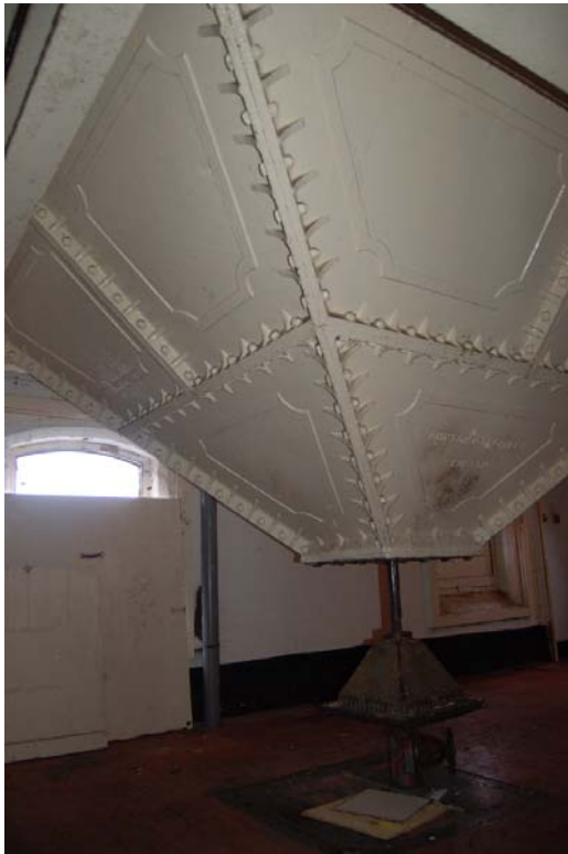
Plate 39: Detail of hopper bottom.
