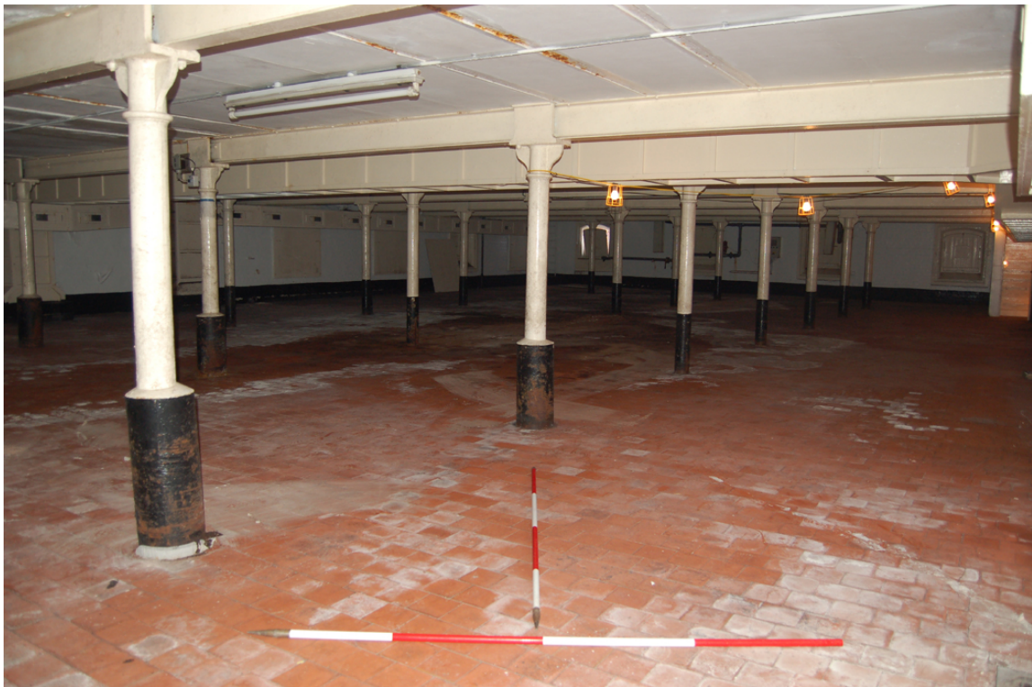
Plate 43: Working floor [1F01]; general view looking south-west.
