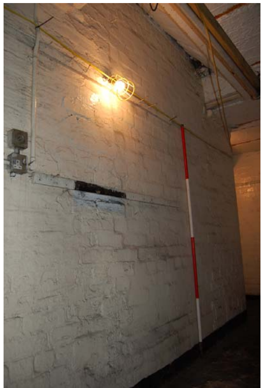
Plate 55: Kiln Range [GF10]; blocked door to flue chamber.
