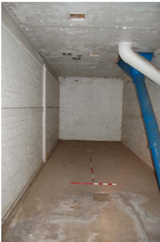
Plate 76: Out-loading bays, [2F04].
