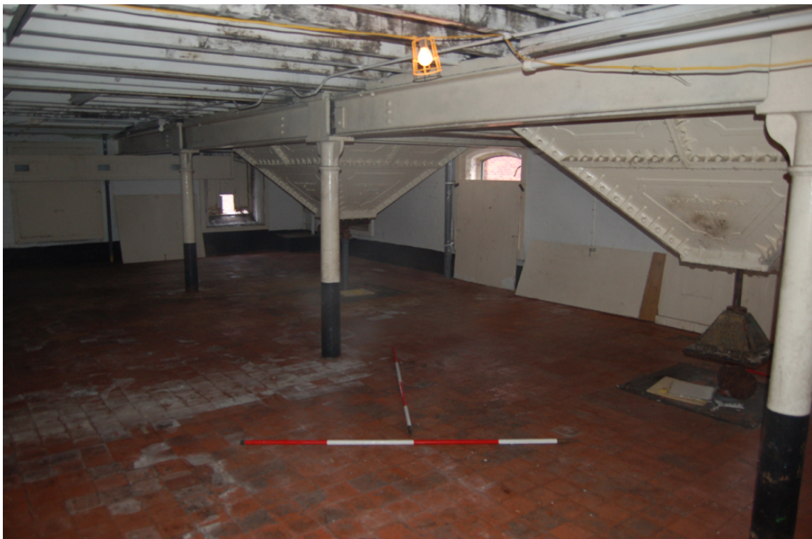
Plate 38: Barley intake range, [2F01]; hopper bottoms of steeping vessels at Bay 1.
