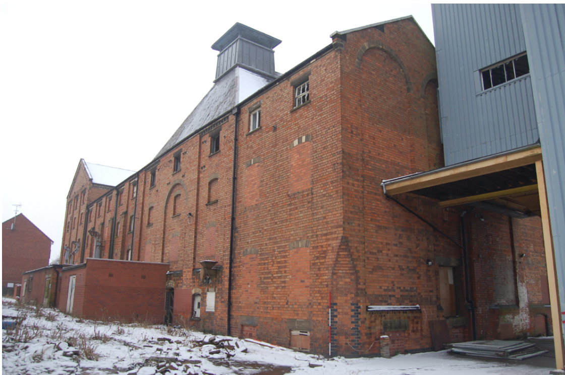
Plate 2: South elevation; general oblique view looking north west.
