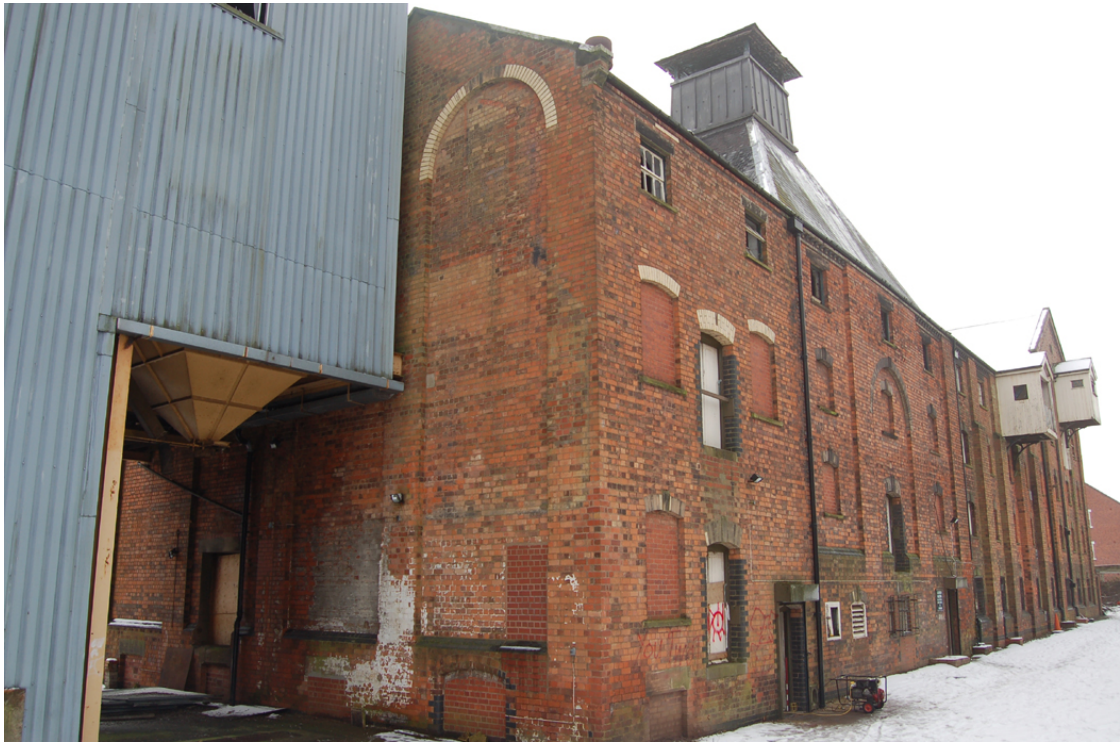
Plate 1: North elevation; general oblique view looking south-west.
