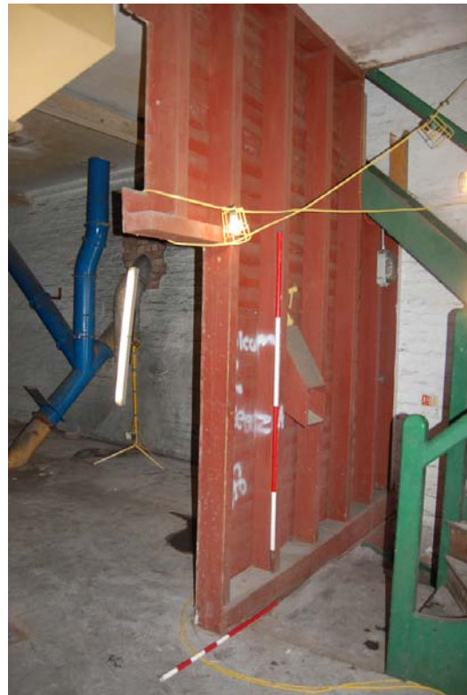
Plate 79: Out-loading bays, [1F06] timber partition (truncated).
