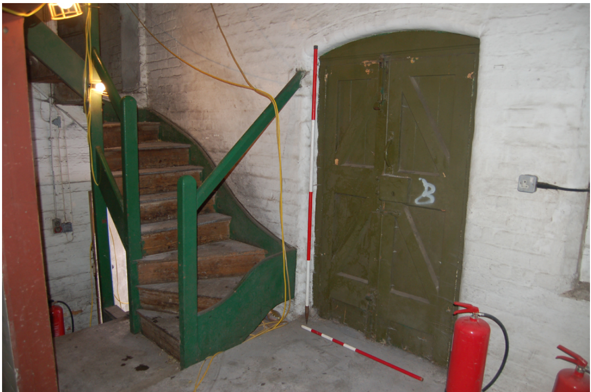
Plate 80: Out-loading bays, [1F06]; loading doors to north (right) and stair to entrance level (left).
