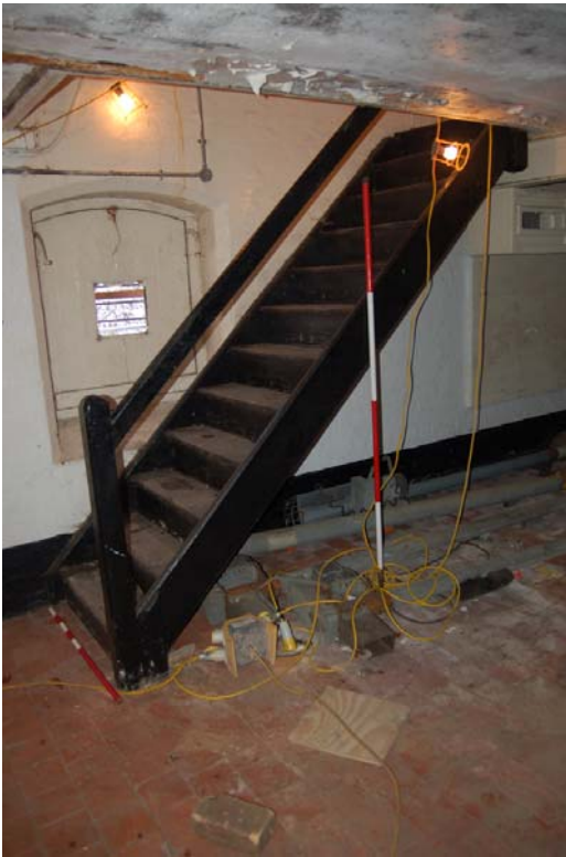
Plate 48: Barley intake range [GF01]; detail of stair.
