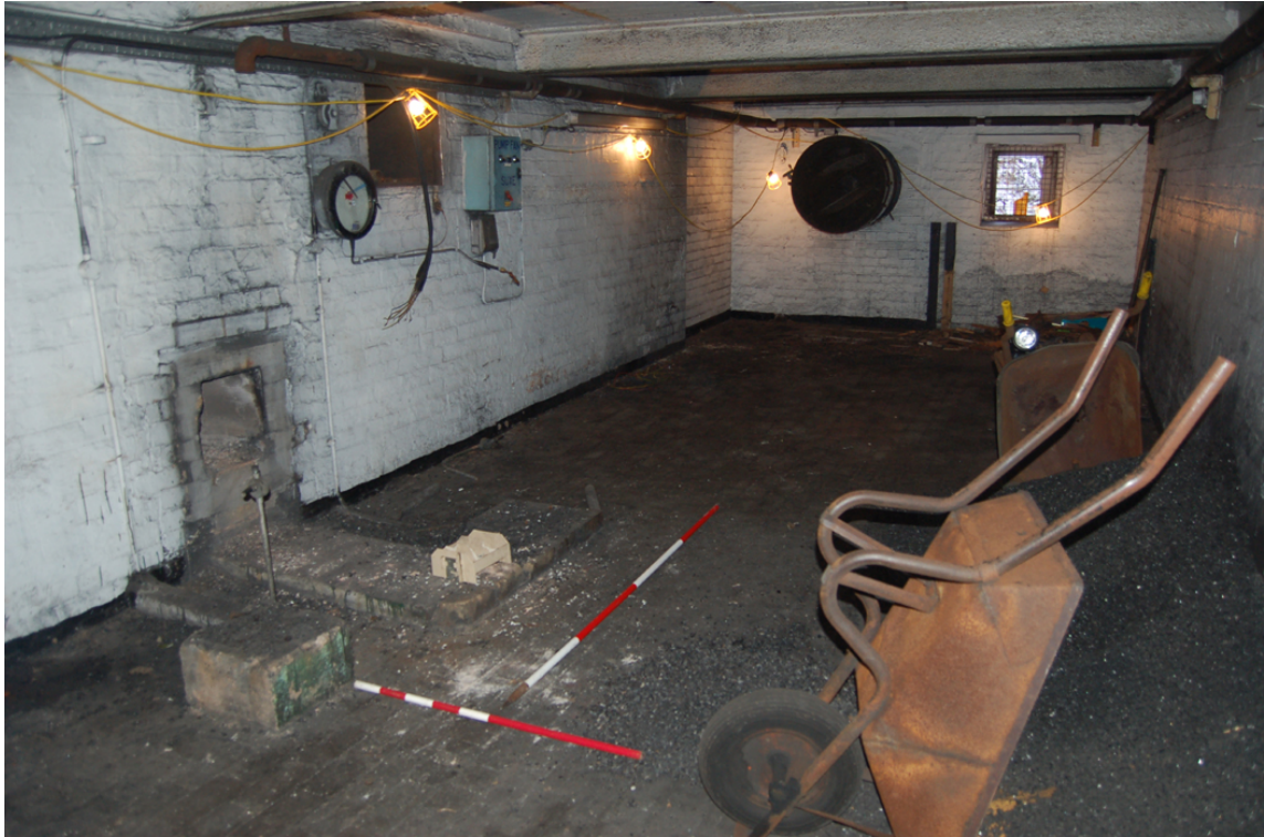
Plate 56: Kiln range, [GF11]: stoke room looking north, note setting for anthracite furnace.
