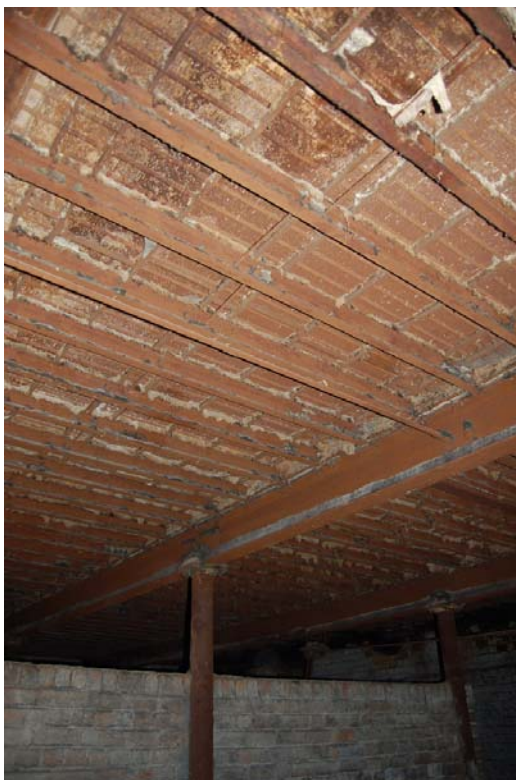
Plate 63: [2F02]; detail of u/s of wedge-wire kiln floor.
