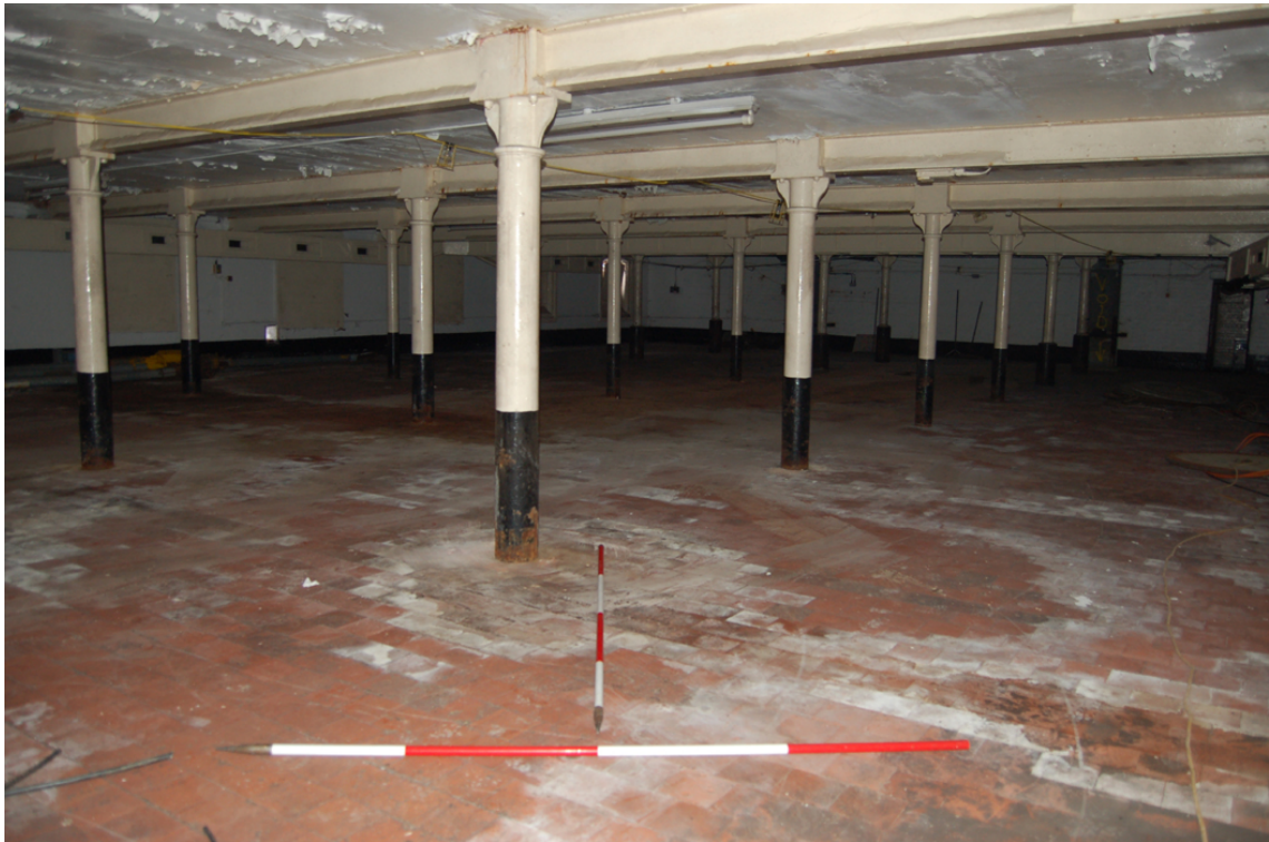
Plate 46: Working floor [GF01]; general view looking north-east.
