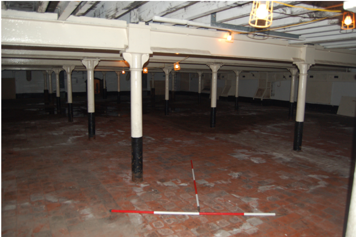
Plate 37: Working floor [2F01]; general view looking south-east.
