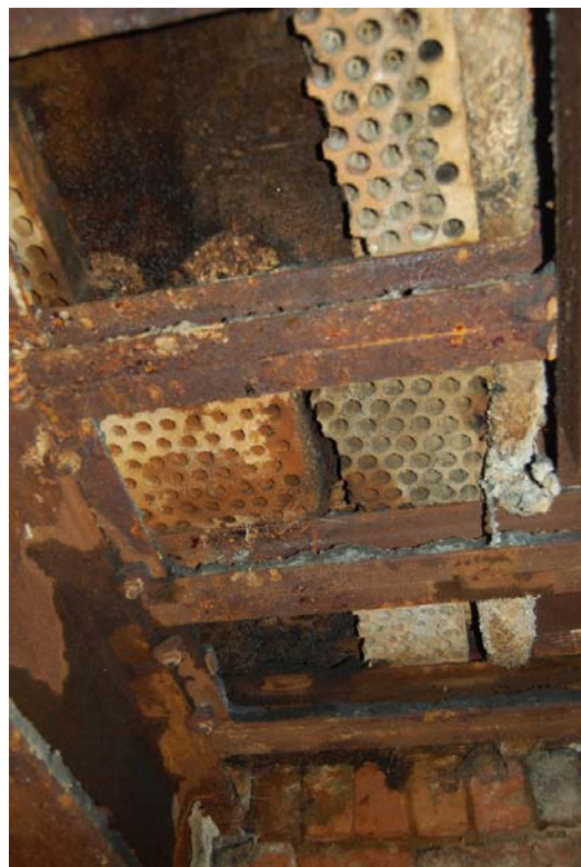
Plate 64: [2F02]; detail of in-situ primary perforated tiles.
