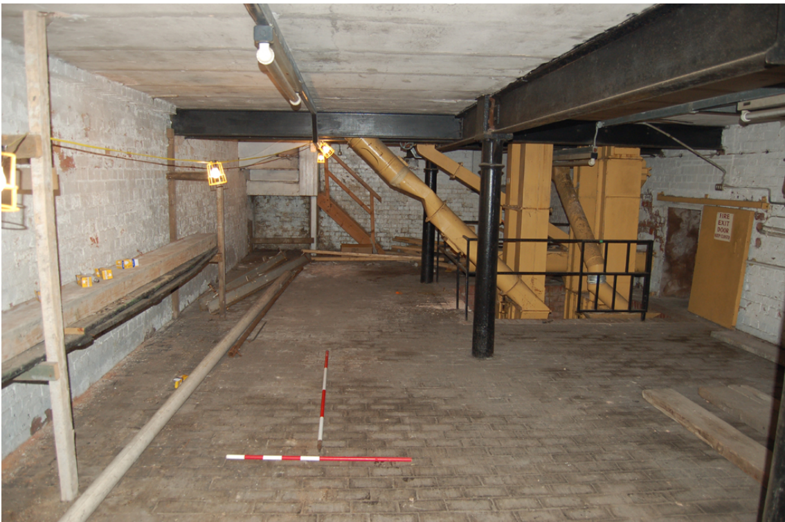
Plate 83: Out-loading bays, [B01]; general view looking north.
