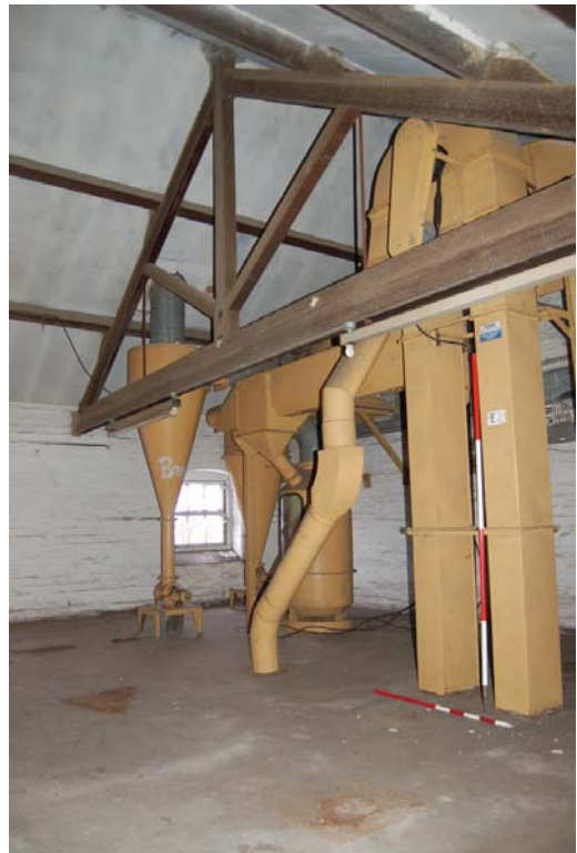
Plate 75: Out-loading bays, [3F05] roof and secondary plant.
