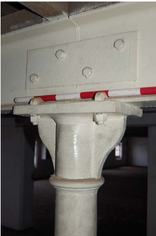
Plate 30: [3F01]; detail of column head.
