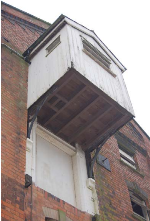
Plate 6: Barley intake range, N elevation; detail of 4F projecting hoist canopy
