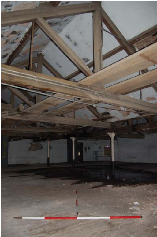
Plate 34: Room [3F02]; detail of king-post roof.
