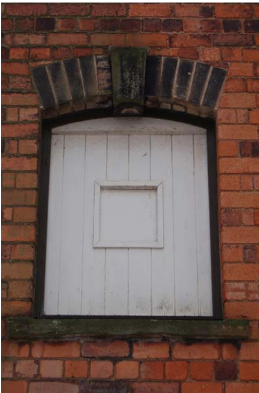
Plate 17: Secondary shutter (exterior).
