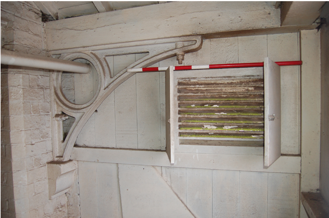
Plate 22: Barley intake range, 4F; detail of iron bracket supporting hoist canopy.
