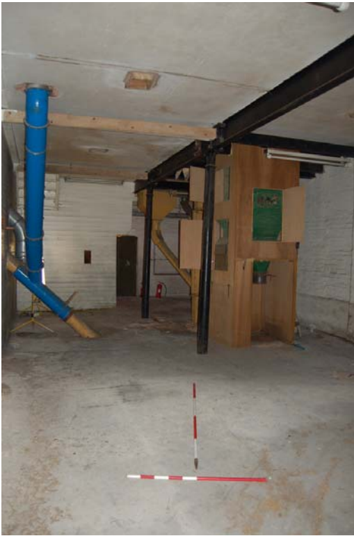
Plate 81: Out-loading bays; [B01].
