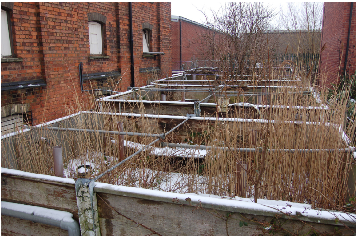
Plate 7: Steep water filtration tanks at west end of maltings.
