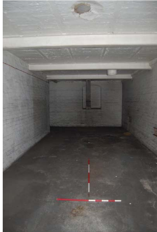
Plate 60: Kiln range, west store [1F03].
