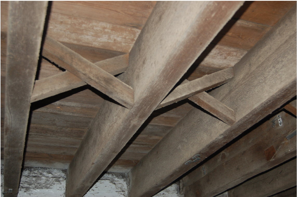
Plate 29: Barley intake range, [3F01]; ceiling structure with herring-bone strutting.
