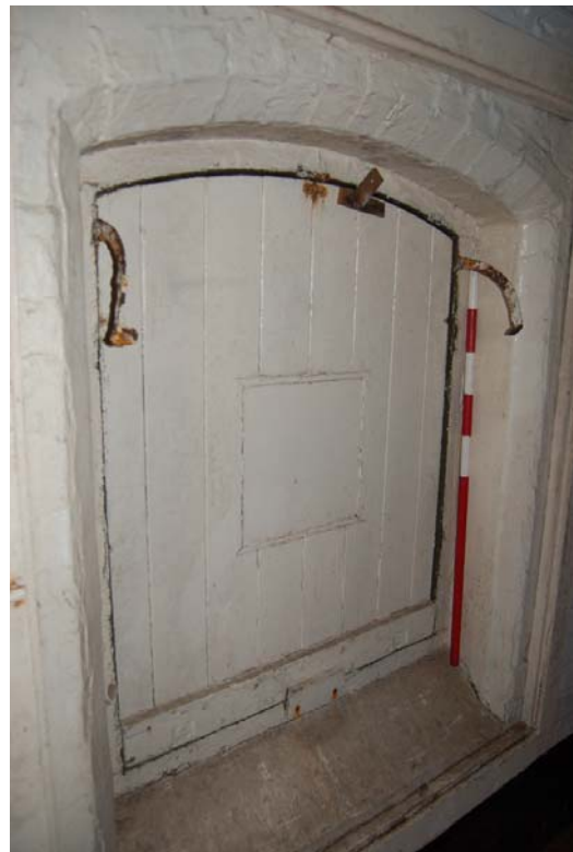
Plate 18: Secondary shutter (interior).
