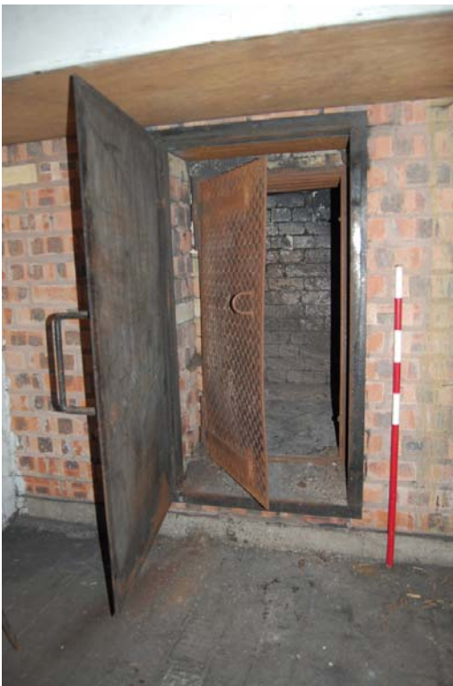
Plate 50: Kiln range [GF08]; flue doors.
