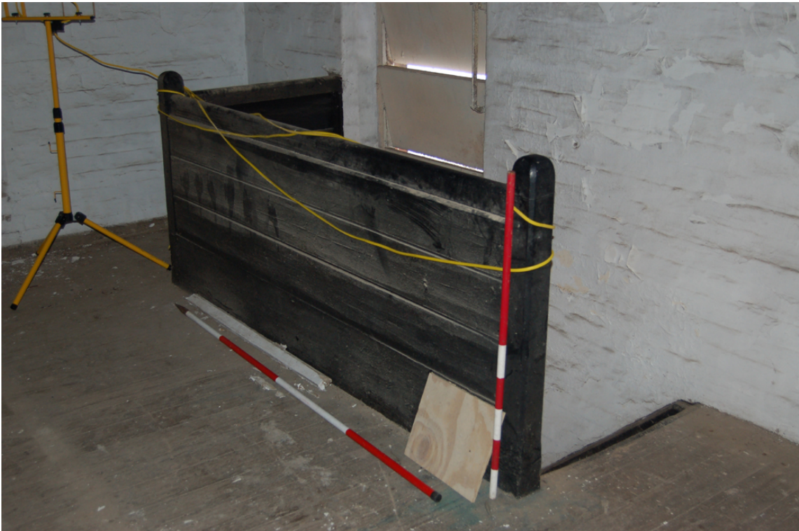
Plate 21: Barley intake range, [4F01]; primary stair at north-west corner.
