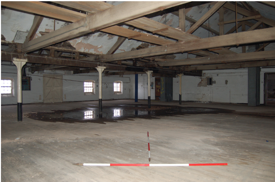
Plate 33: Room [3F02]; general view looking north-east.
