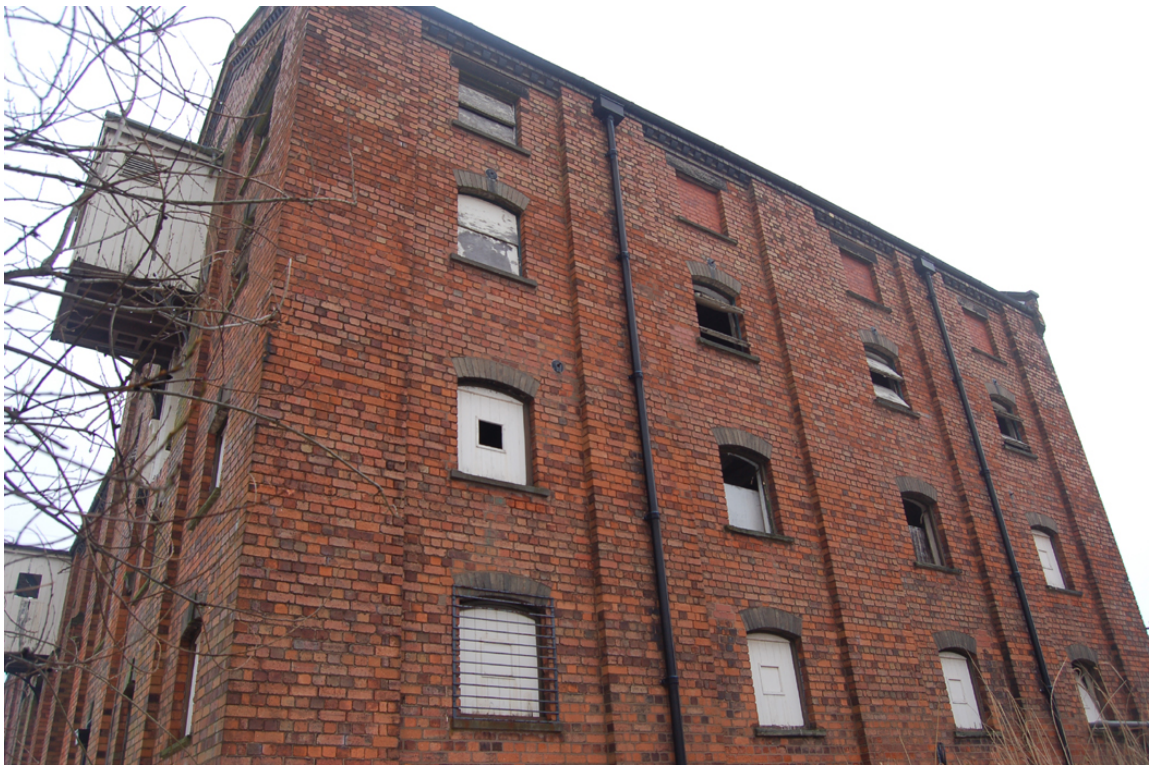
Plate 5: Barley intake range; west elevation.
