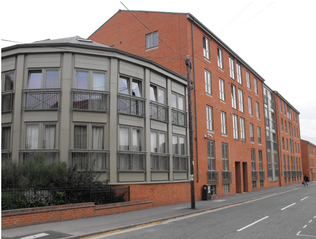
Plate 3: Chapel End and Brook House developments on north side of Brook Street.
