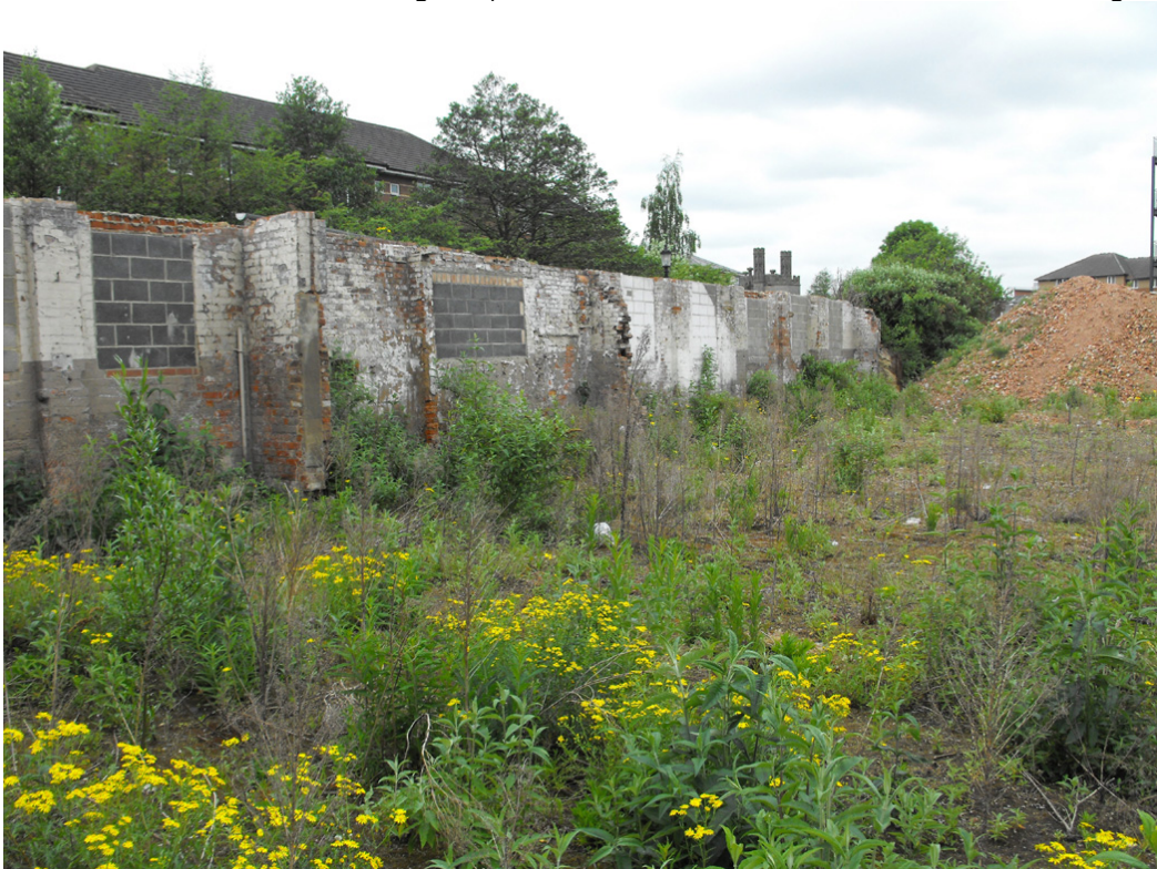
Plate 10: Southern bounding wall, note blocked windows of former ironworks ranges.
