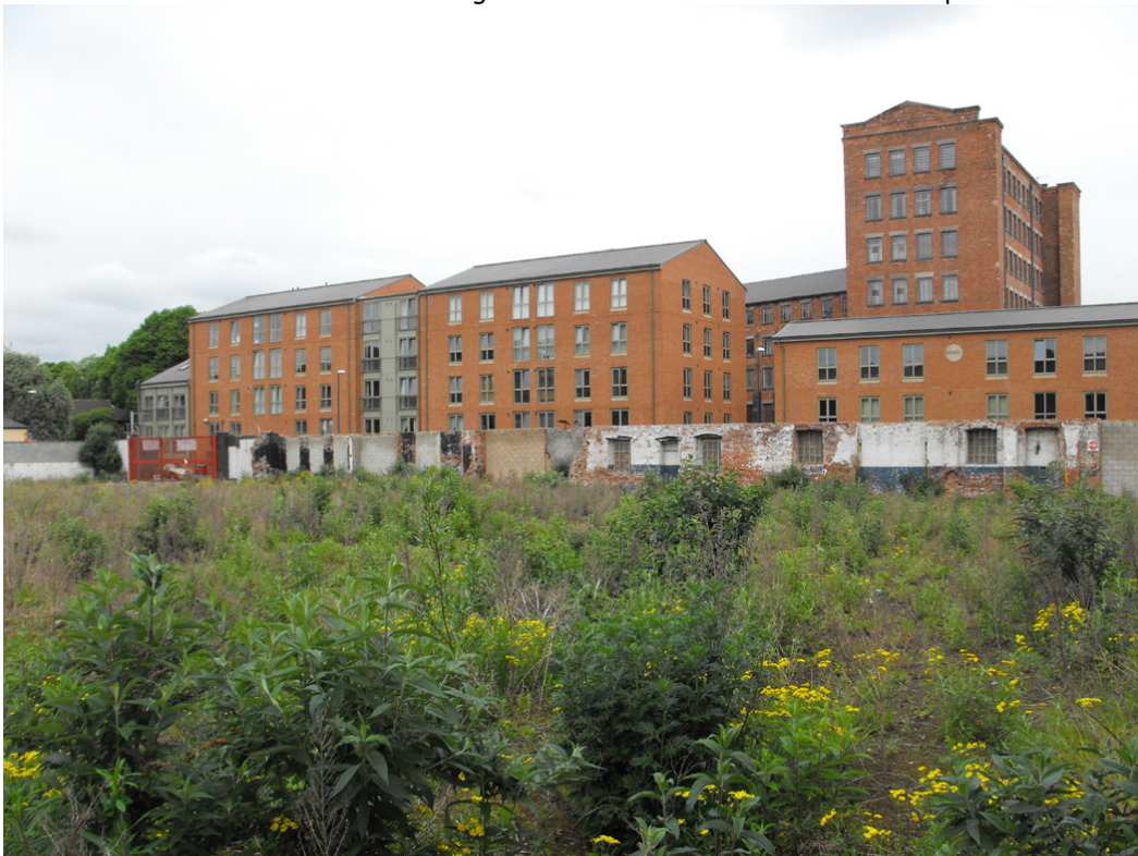
Plate 8: General view of site looking north-east towards Chapel End and Brook House (2004), Ryknield Mill ( HER 18976 ) in background.
