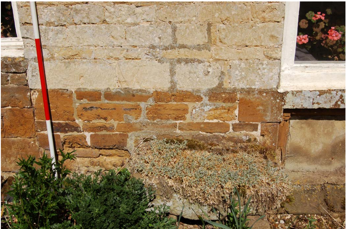
Plate 12: Lower ironstone masonry of late C17th block.
