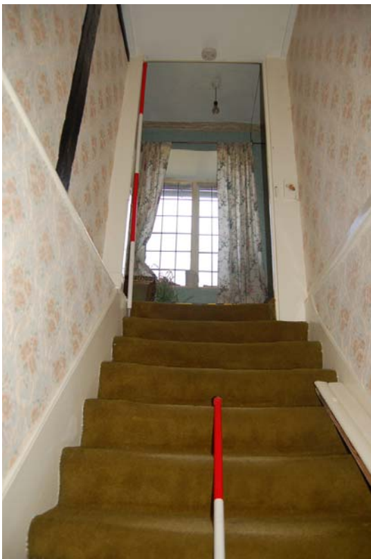
Plate 41: Stair [1F04] GF →1F.
