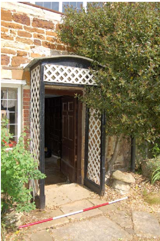
Plate 5: Doorway, east elevation.
