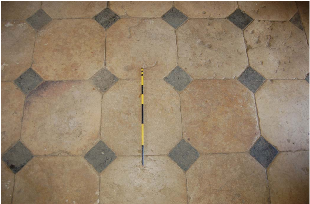
Plate 21: Room [GF06]; chequer floor of white (Culworth) and black (Byfield) stone.
