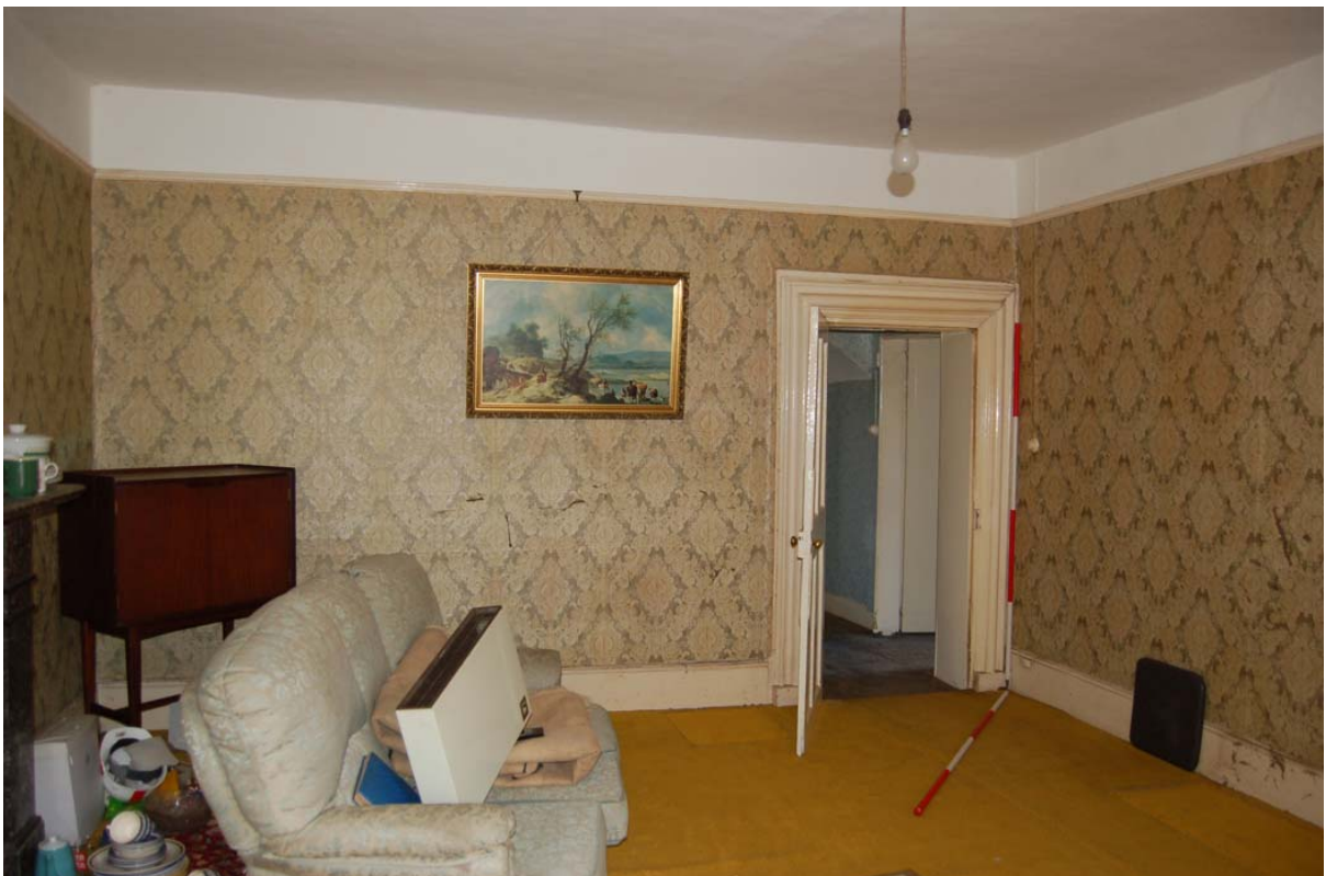
Plate 28: Room [GF10]; general view looking north; note bolection doorcase (compare Pl. 50).
