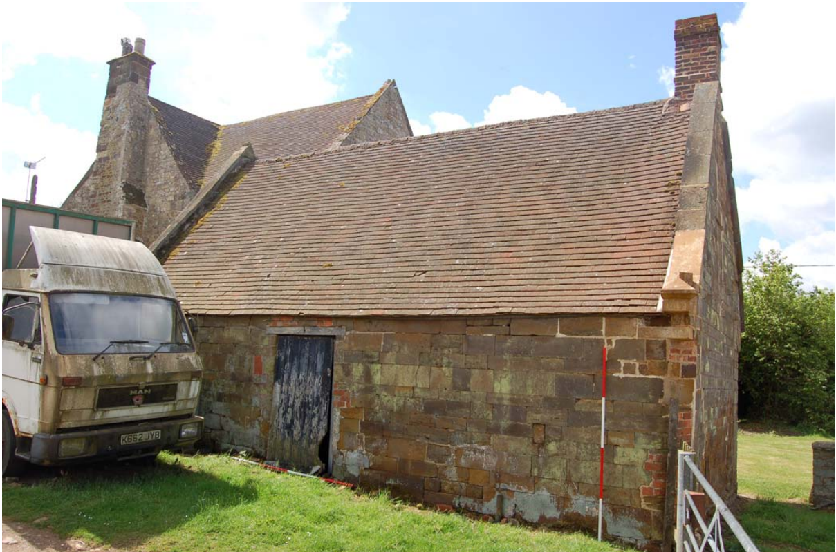
Plate 58: Outbuilding to north-west of farmhouse; looking south-east.
