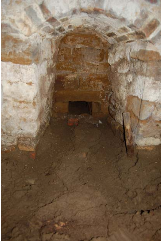
Plate 40: Drainage channel in west wall of [B01]; note original ironstone masonry of primary wall.
