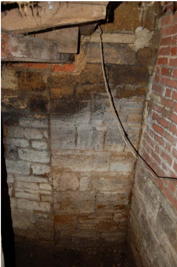
Plate 36: Room [GF11], upper section of blocked GF window visible above former ceiling level.
