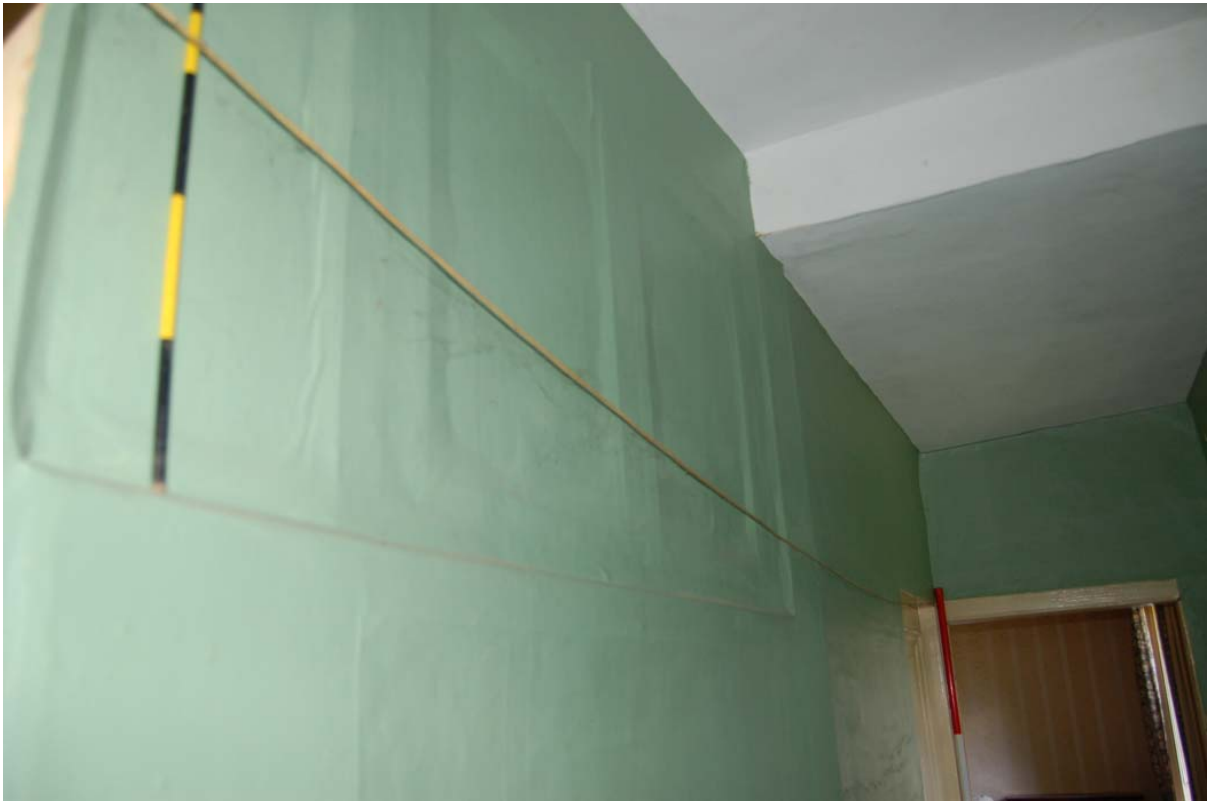
Plate 23: Obscured (?) panelling / studwork within corridor [GF05].
