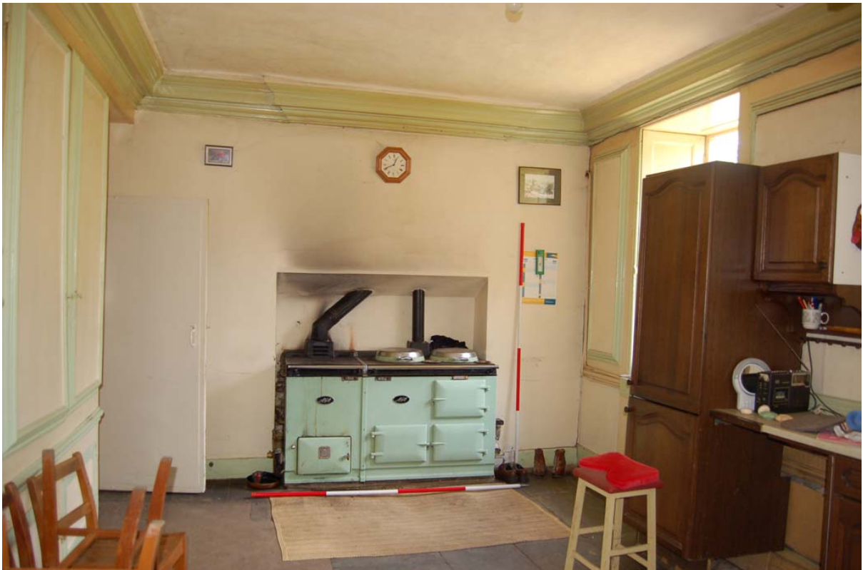
Plate 26: Room [GF07]; general view looking north.
