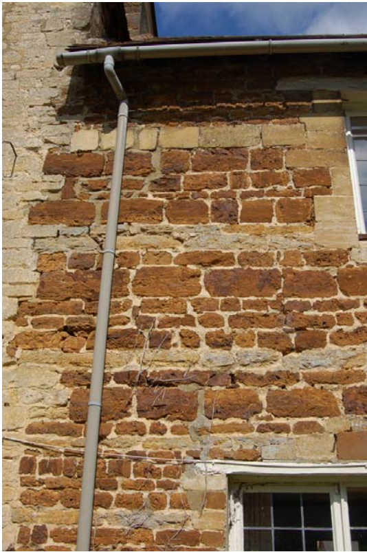
Plate 7: Phase break in east elevation.
