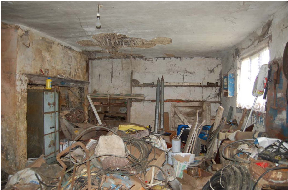
Plate 33: Room [GF11], general view looking west.
