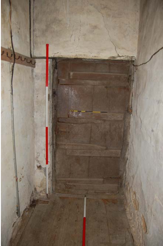
Plate 27: Corridor [GF09] looking west.
