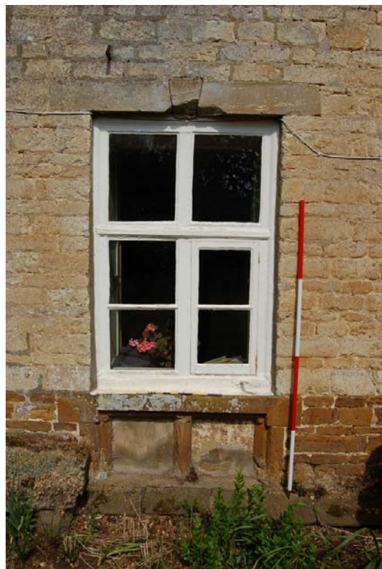
Plate 10: Moulded basement window to late C17th block.
