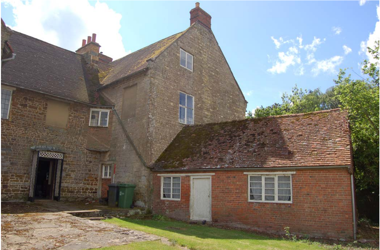
Plate 16: Oblique view of southern extension, later structures to right.
