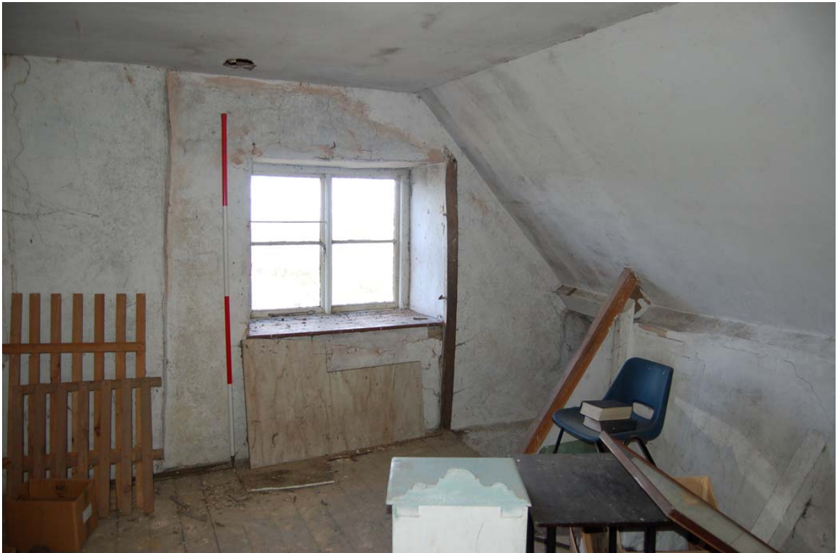
Plate 55: Room [2F01] looking west.
