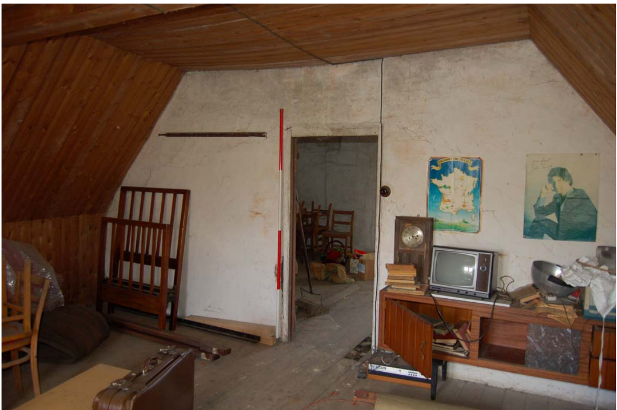
Plate 56: Stair [2F02] looking south-west.
