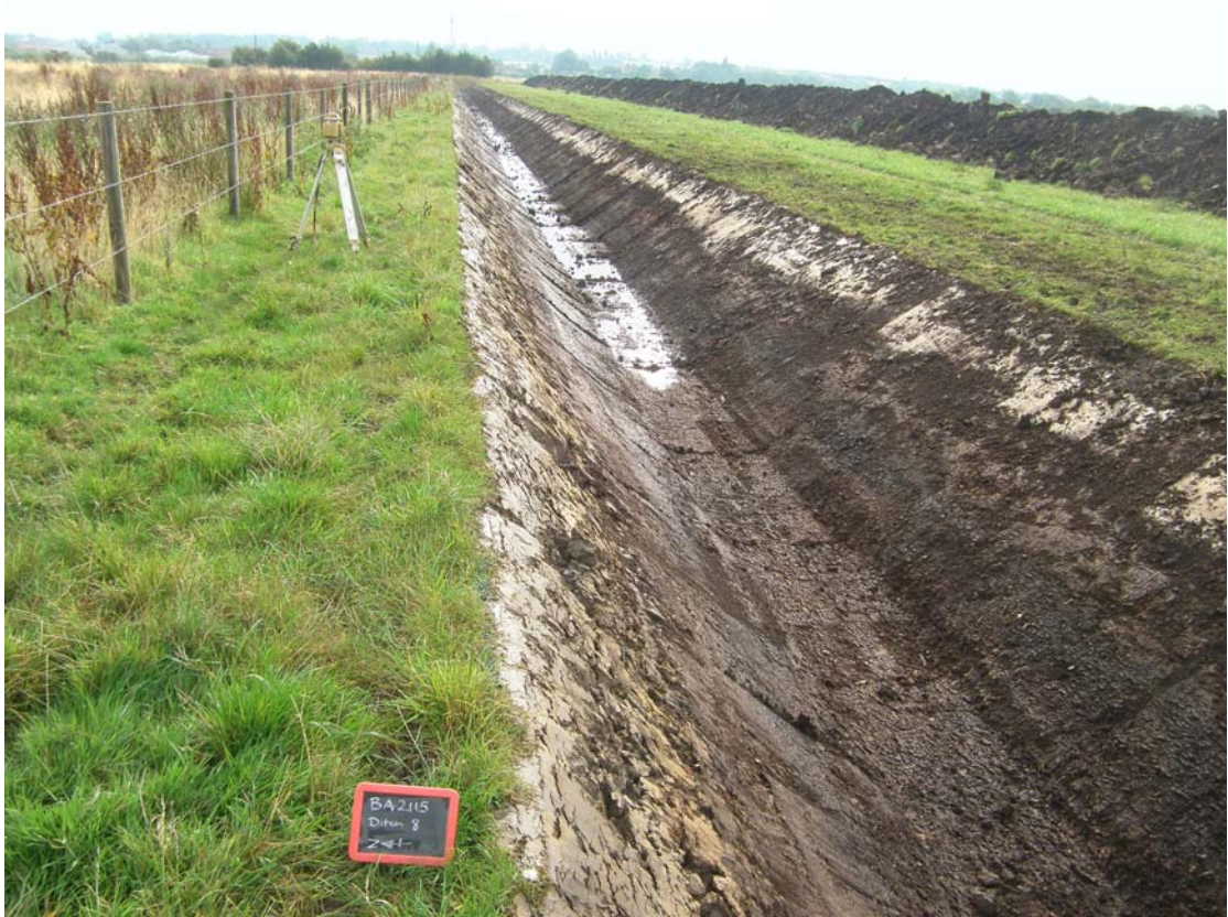
Plate 1: Ditch 8 looking east
