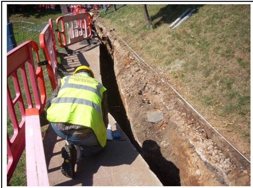
Plate 4: Excavated service trench, west facing
