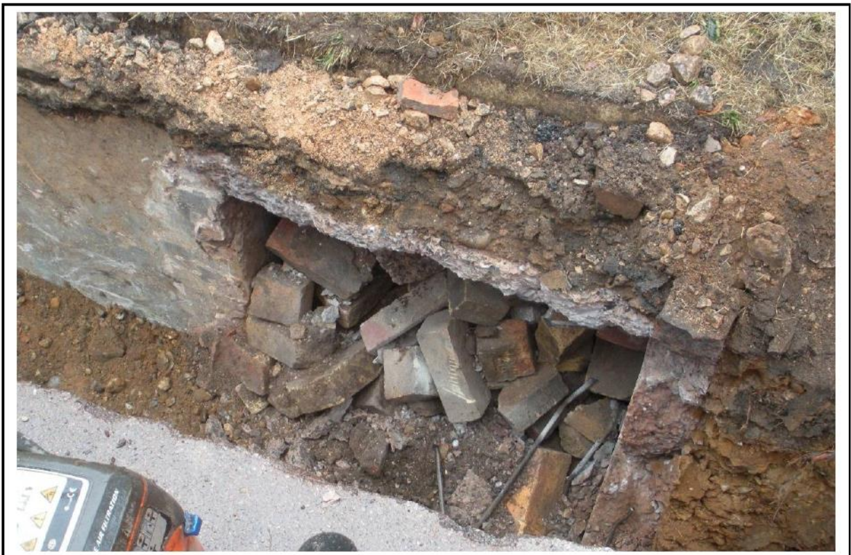
Plate 6: Entrance to Shelter AR2, north facing
