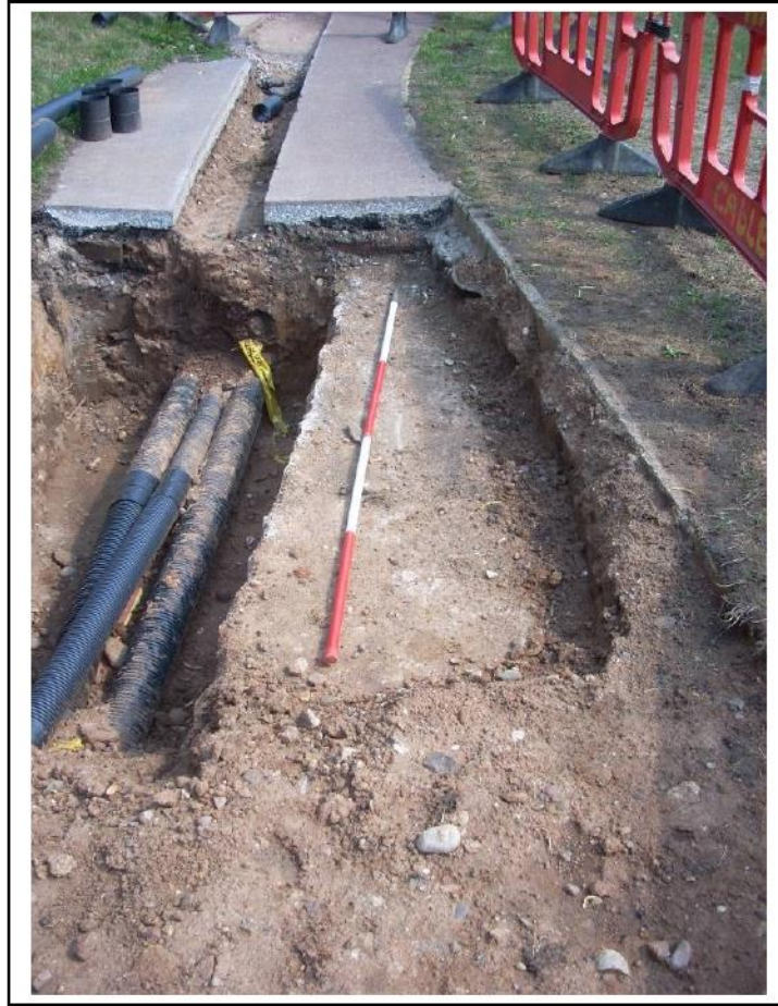
Plate 3: Excavated rear (north) wall of Shelter AR1
