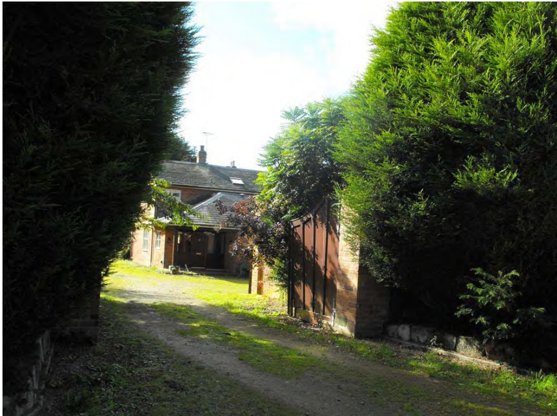
Plate 7: Entrance to walled garden from north (Coach House in background).
