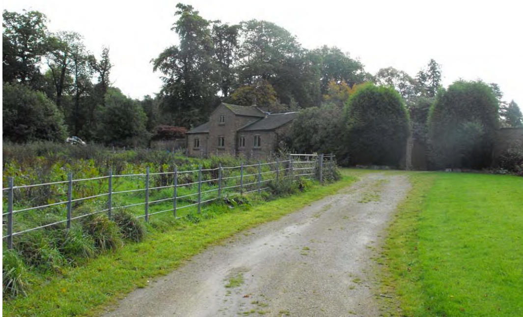
Plate 5: Walled garden (exterior) from northwest.
