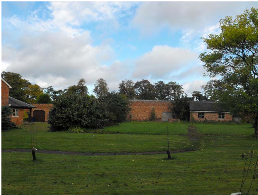
Plate 10: Walled garden (interior) from south.
