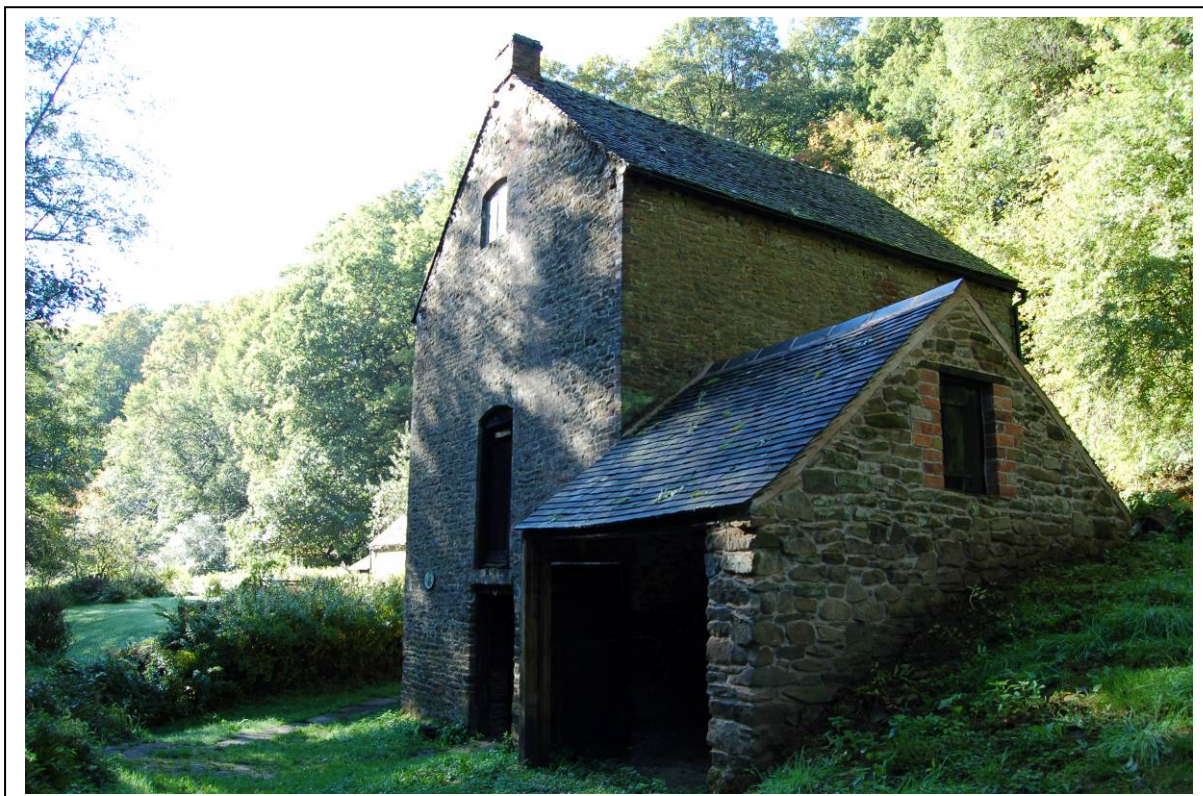
Plate 2: Knowles Mill – Eastern Elevation
