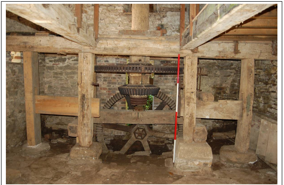
Plate 12: Mill machinery, ground floor, west facing
