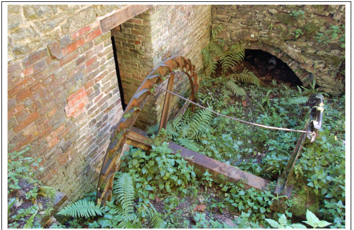
Plate 8: Wheel pit and remains of the wheel, pre-excitation
