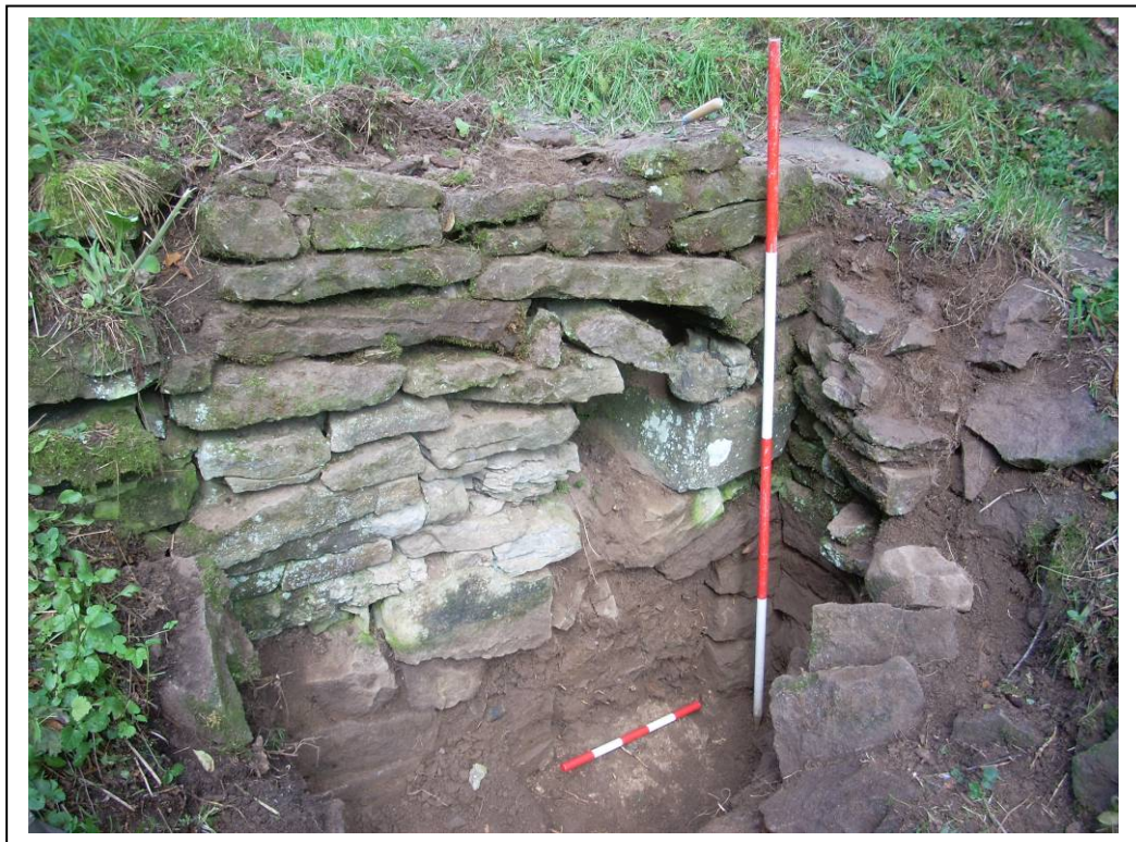
Plate 30: Trench 3, weir/ bridge, south facing elevation
