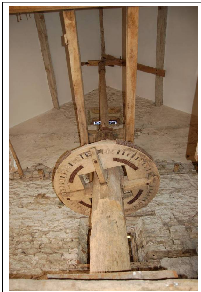
Plate 25: Crown wheel, main axle and sack hoist mechanism
