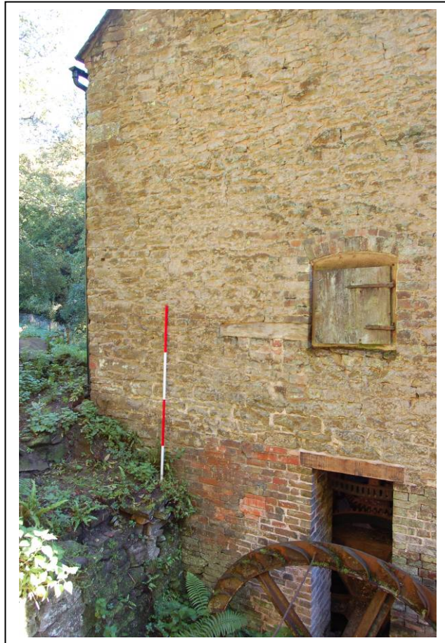
Plate 9: West elevation including wheel pit
