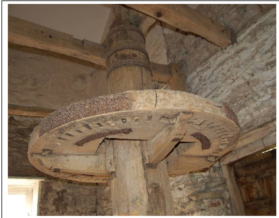
Plate 24: Crown wheel, detail
