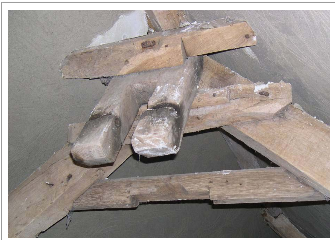
Plate 16: Sack-hoist pulley mount, in apex of roof truss
