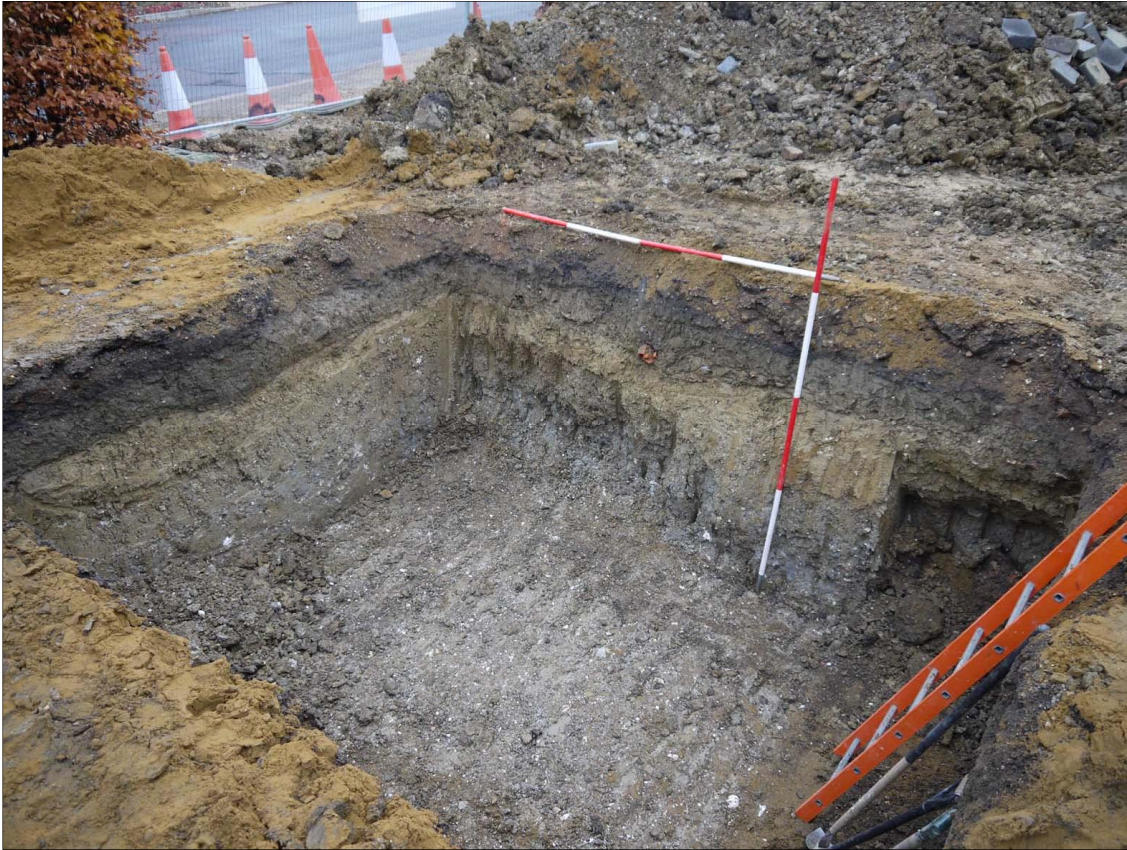
Figure 19. Gas tank pit: Sections 8 (left) and 9 (right). Facing northeast
