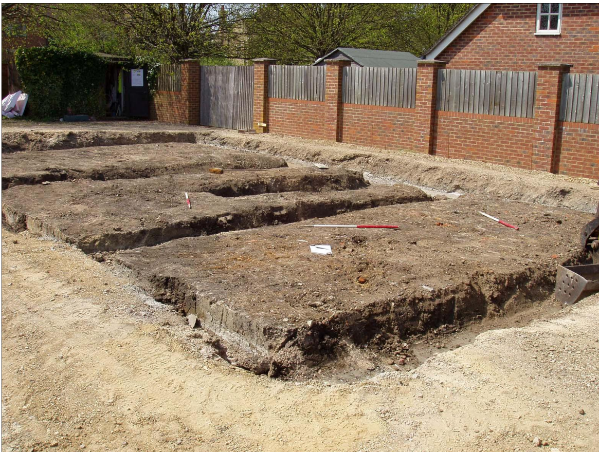
Figure 14. Building footprint showing final reduced ground level, facing west
