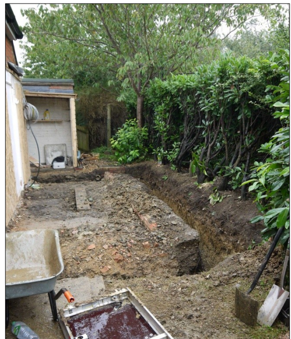
13.10. Overview of foundation trenches. Facing NE
