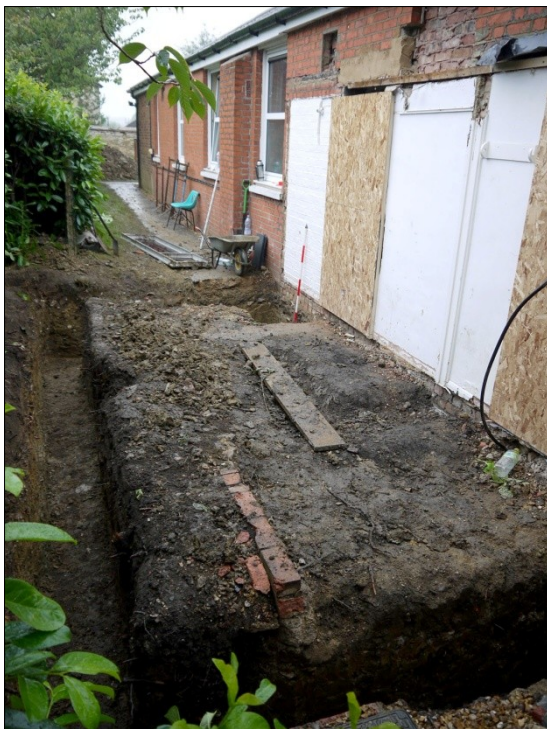
13.9. Overview of foundation trenches. Facing SW
