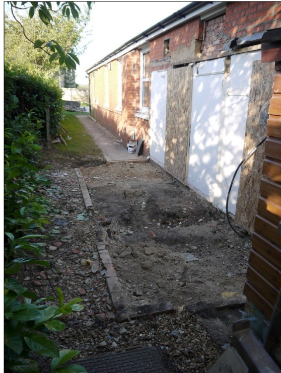
13. 2. Overview of site prior to investigation. Facing SW
