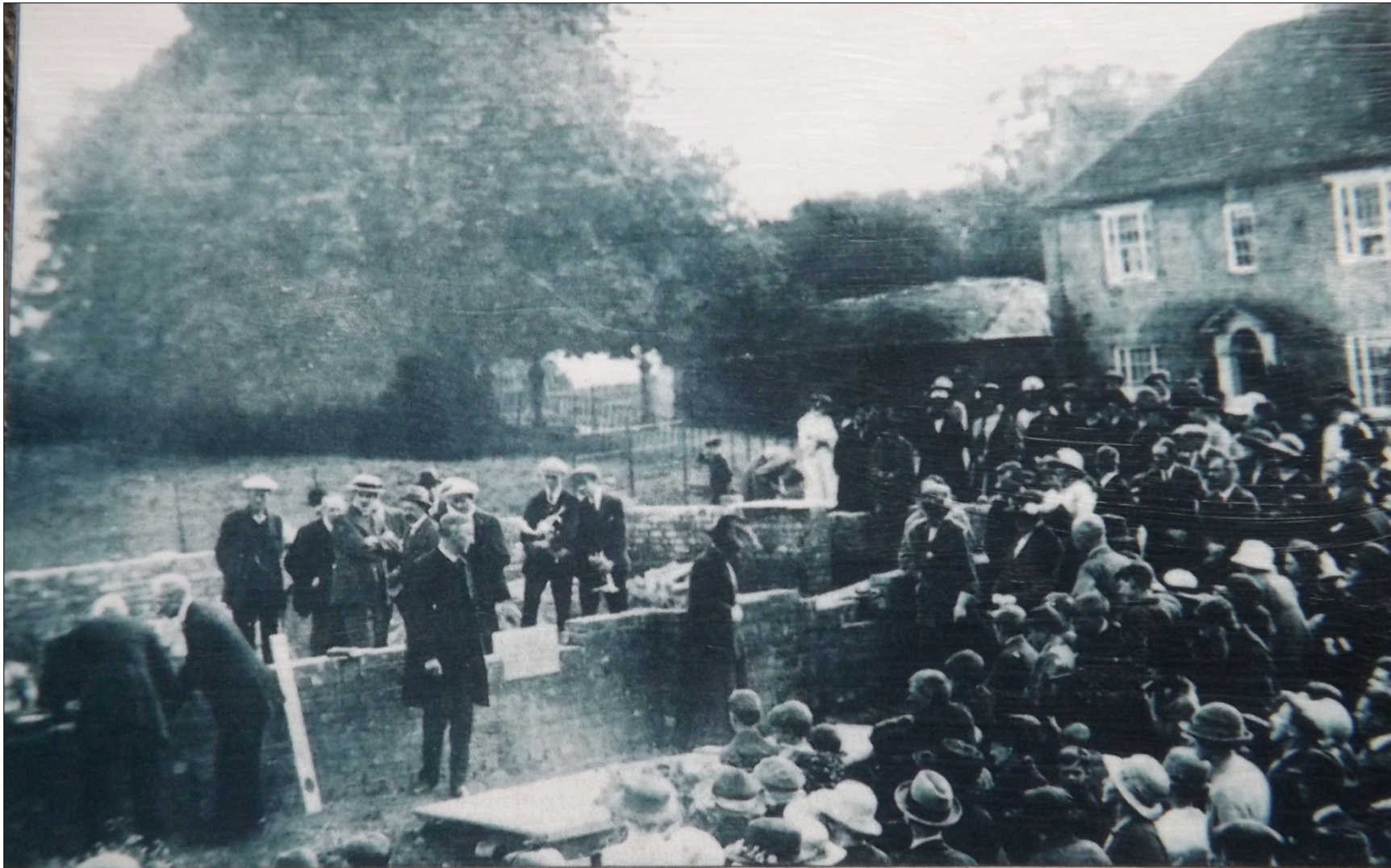
Figure 6. Laying the foundation stone of Bradwell Memorial Hall c. 1924. Facing south; the bailey earthwork is visible behind the building site. (photograph courtesy of the Bradwell Hall Memorial Hall Committee).
