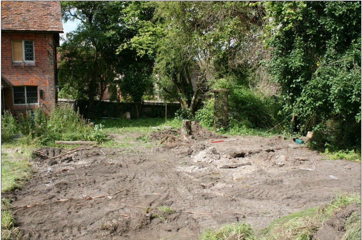
Figure 7. Overview of development plot prior to ground reduction and trenching. Facing NW
